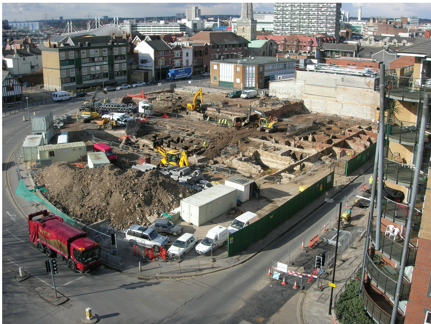
Fig. 1.4 The site under excavation, facing north-west
