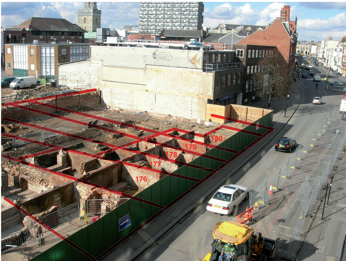
Fig. 4.19 Tenements 176-180 superimposed over excavation photograph, facing north/north-west
