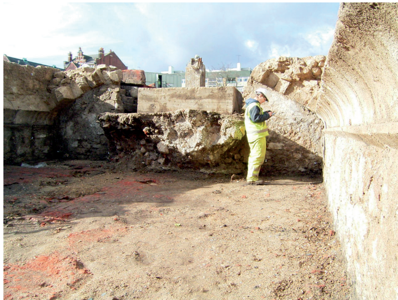
Fig. 4.16 Tenement 173, the cellar during recording, facing west
