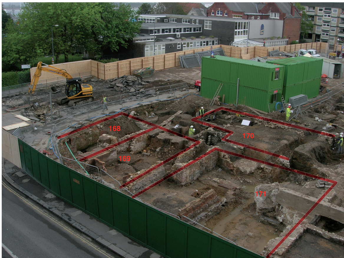
Fig. 4.7 Tenements 168-170 superimposed over excavation photograph, facing south-west
