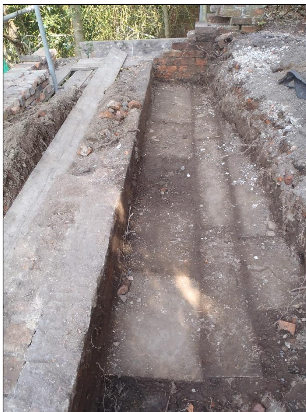
Plate 2: Detail of stone flags 1004, looking north (no scale)
