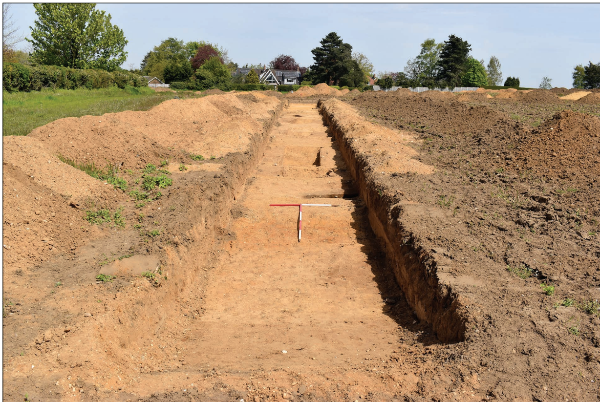
Plate 21: Trench 20, looking north-north-east
