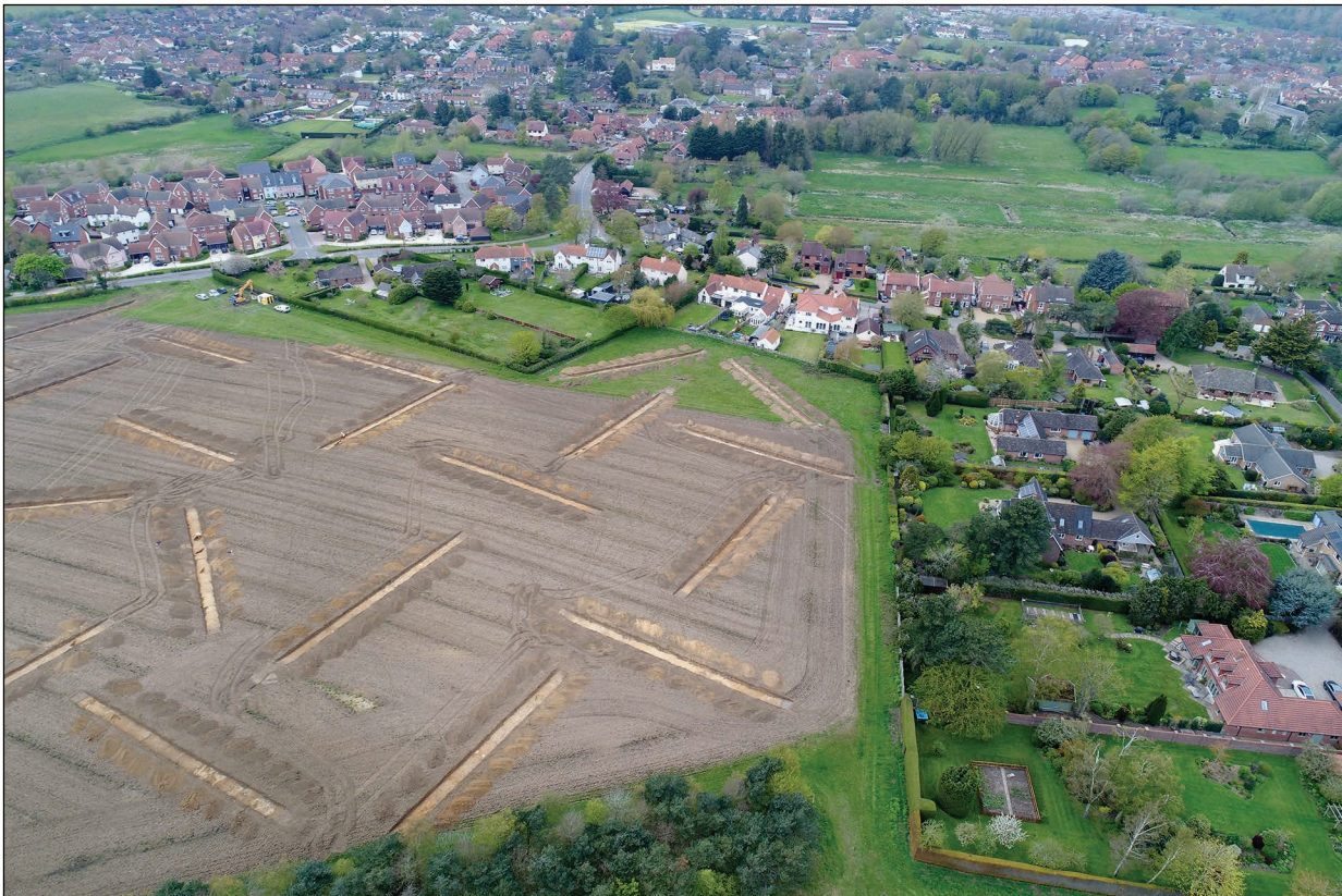
Plate 2: Aerial view of the site, looking west
