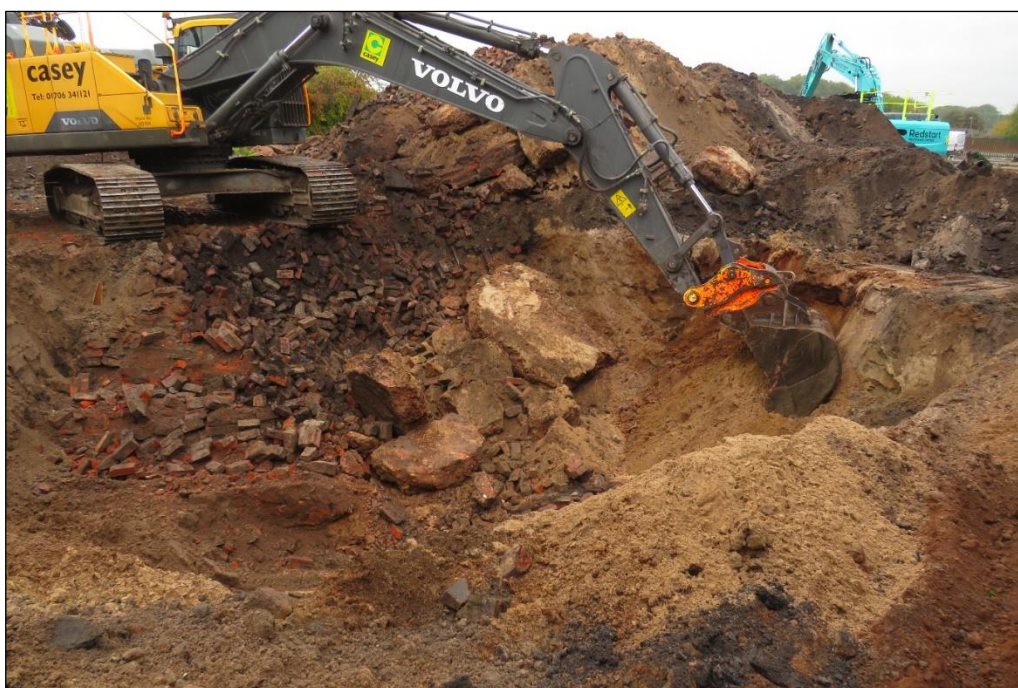
Plate 9: Working shot showing bricks, concrete blocks and natural sand (no scale)
