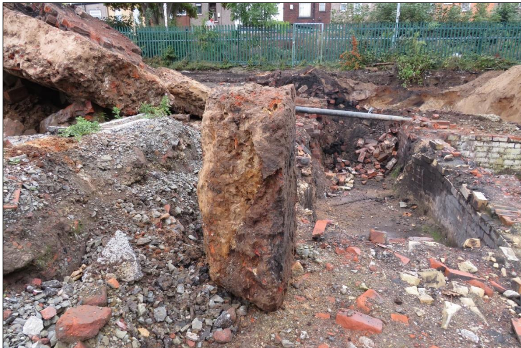
Plate 8: Example of large concrete block found during excavations in south-east corner of site, looking east (no scale)
