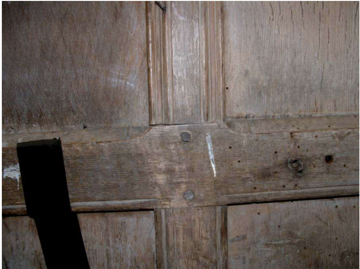
Plate 4: Detail of mouldings and bar stops on panel 5
