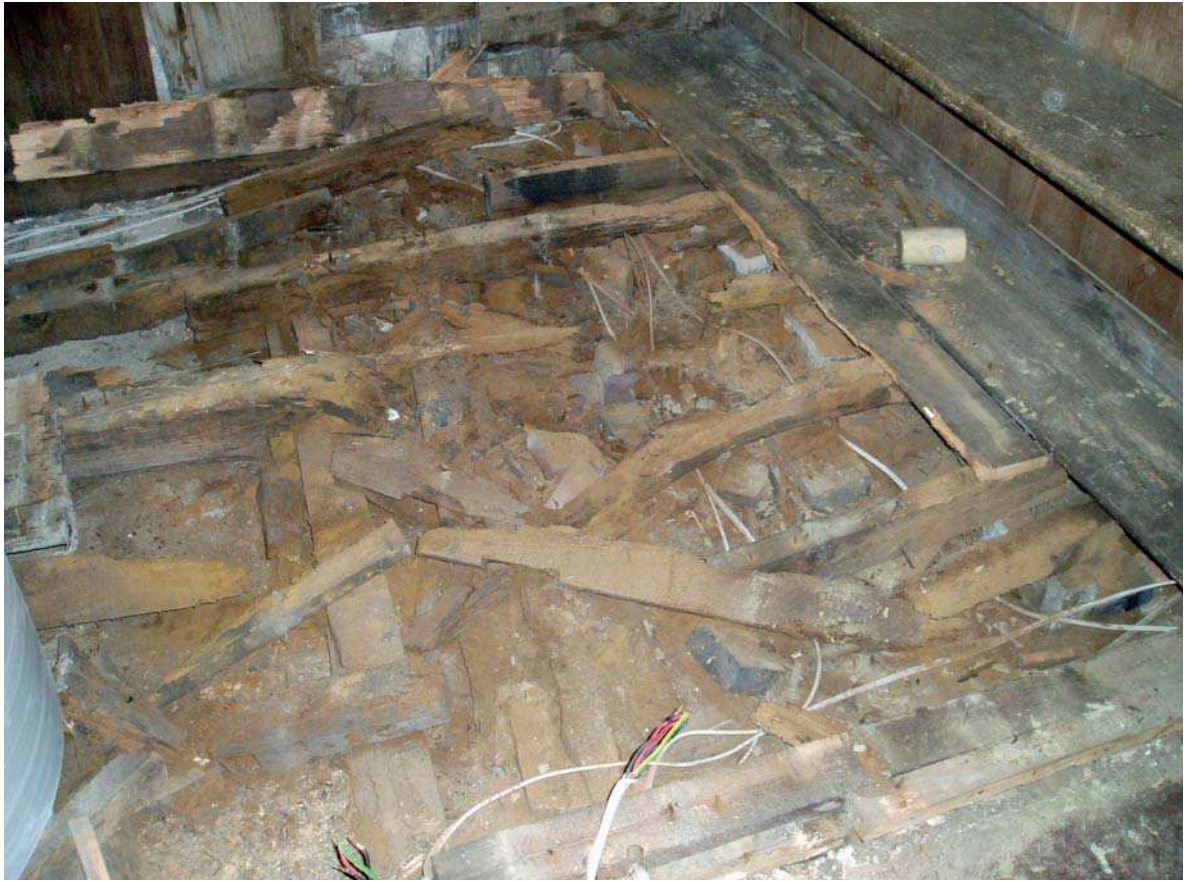
Plate 19: Pew base members before removal showing reused timbers (photo courtesy of Ward and Co.)
