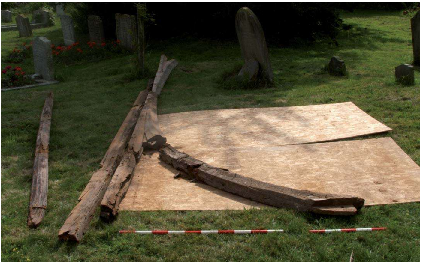
Plate 20: Reconstruction of roof truss from reused members from pew bases (1m and 0.5m scales)
