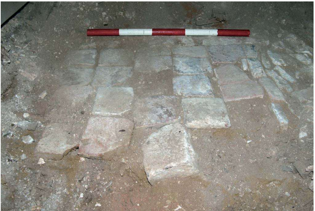
Plate 14: Tiles in recess at west end of south side of Nave (looking west, 0.5m scale)
