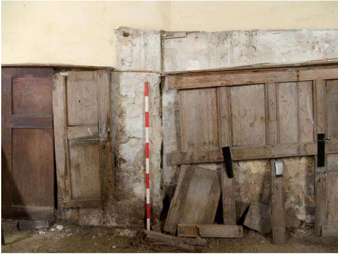
Plate 1: East jamb of blocked north door with panel 5 to right
