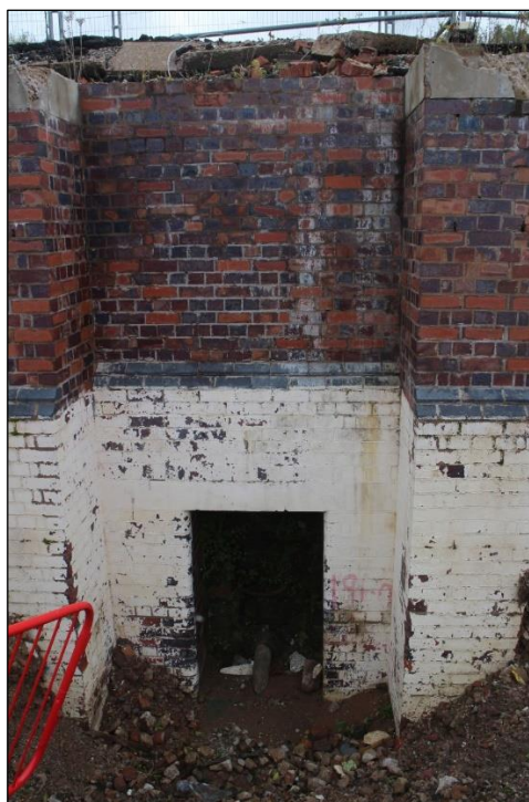
Plate 3: Retaining wall along the southern edge of the development, looking south
