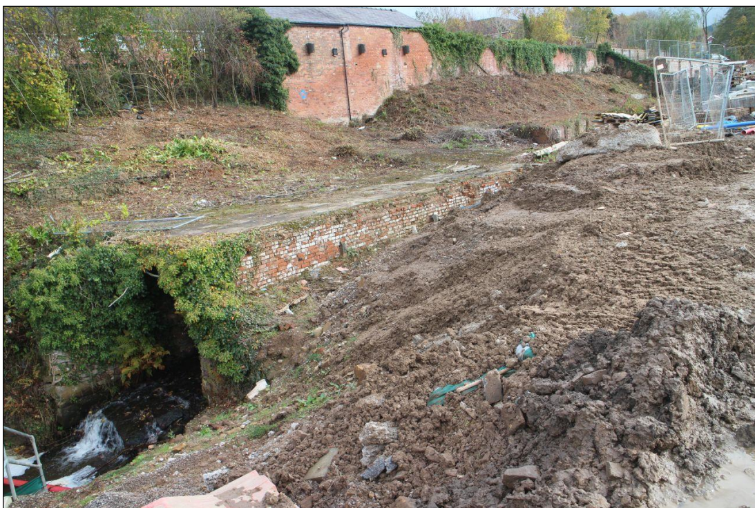
Plate 5: Culvert over Bollin Head Brook looking south-east
