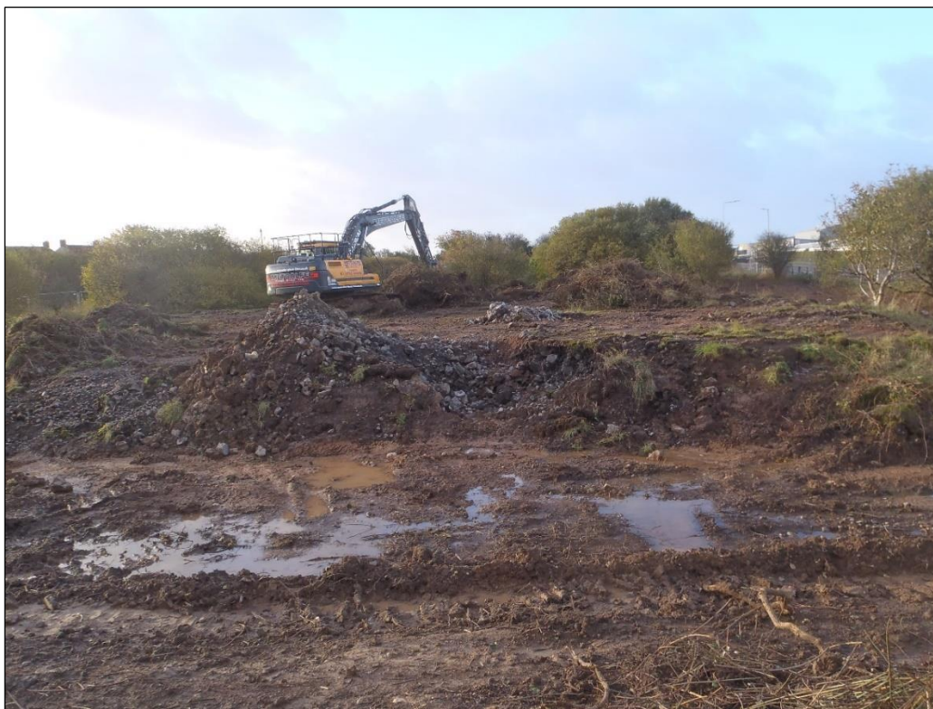
Plate 3: Clearing of made ground, southern end of the site, looking south
