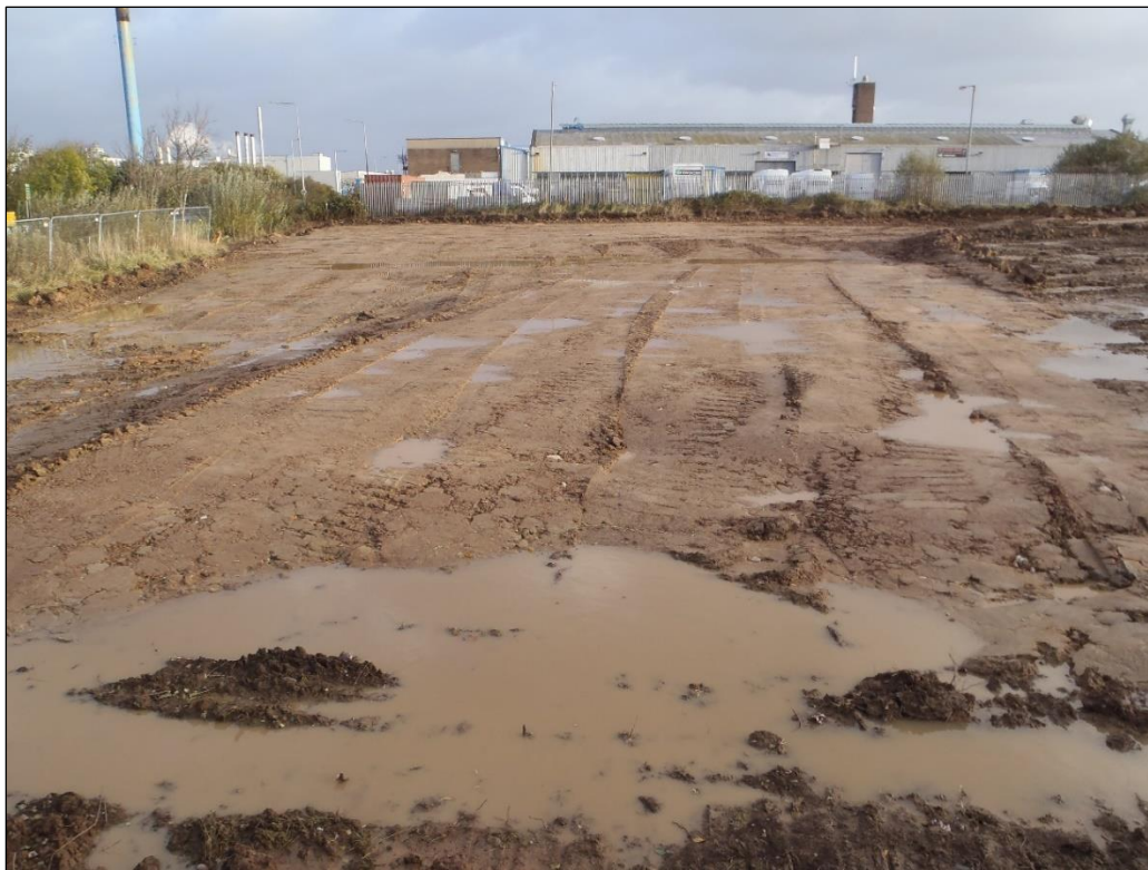
Plate 2: Northern end of main strip area stripped, looking north
