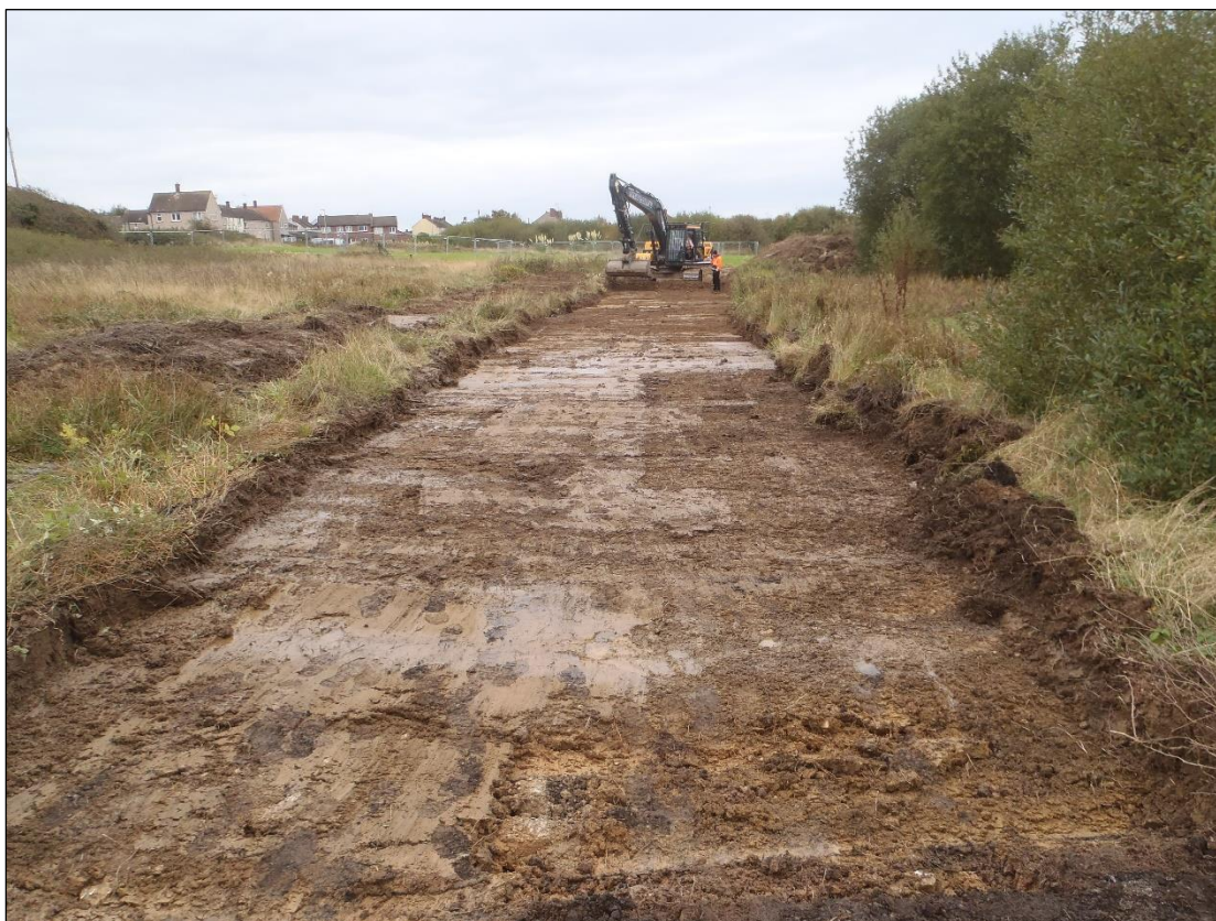
Plate 1: Stripping of haul road in progress, looking south
