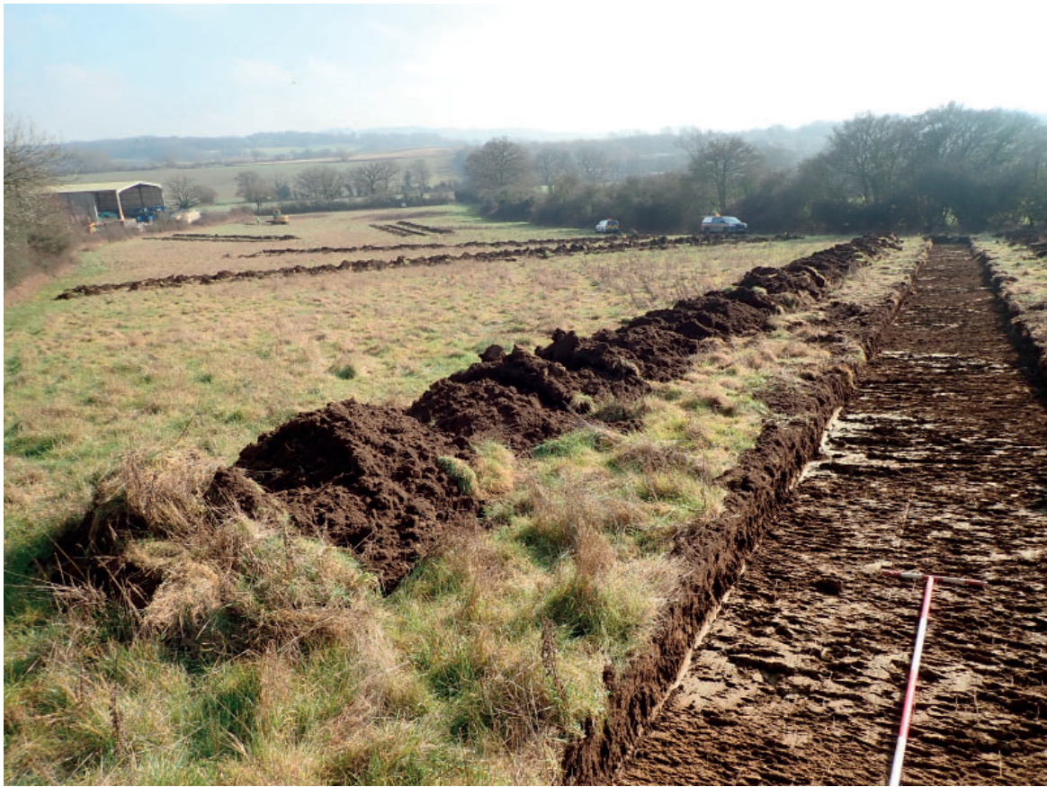
Plate 1: General view of trenching from Trench 1, facing south-east
