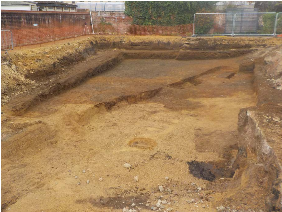
Plate 7: Quarrying in south-western corner of the site
