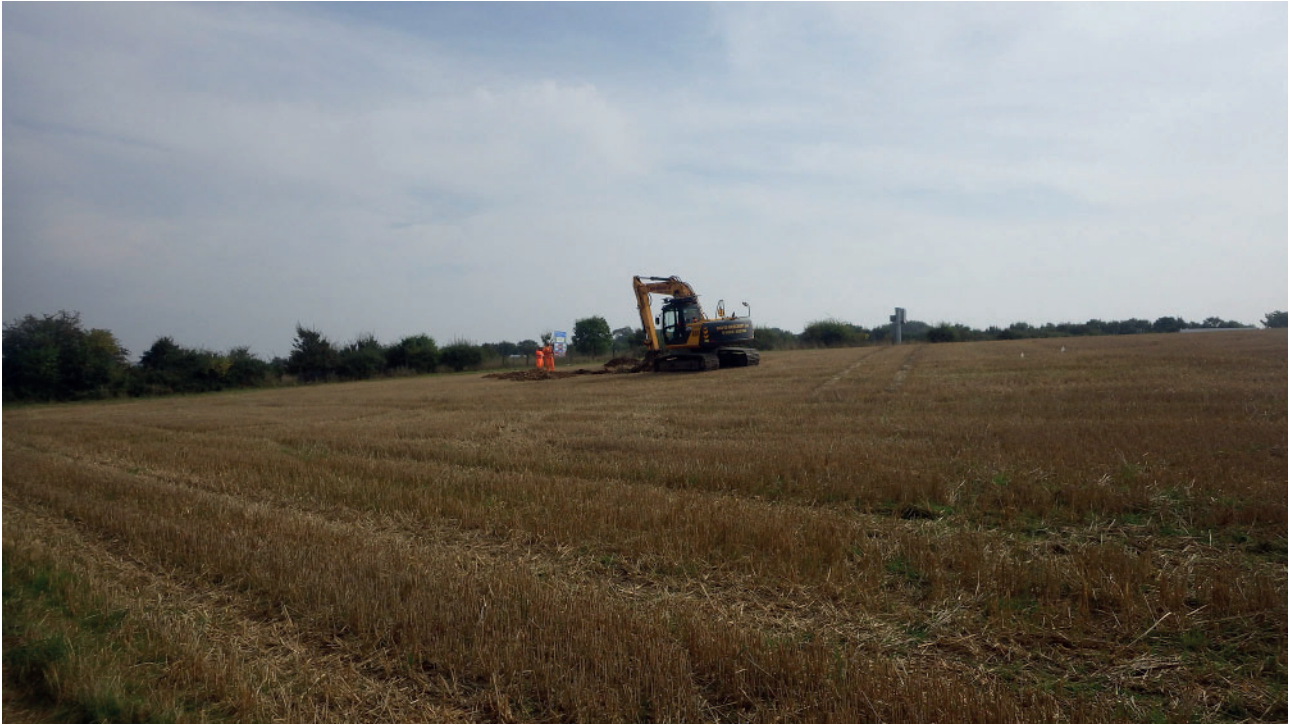
Plate 1: General view of site, looking north
