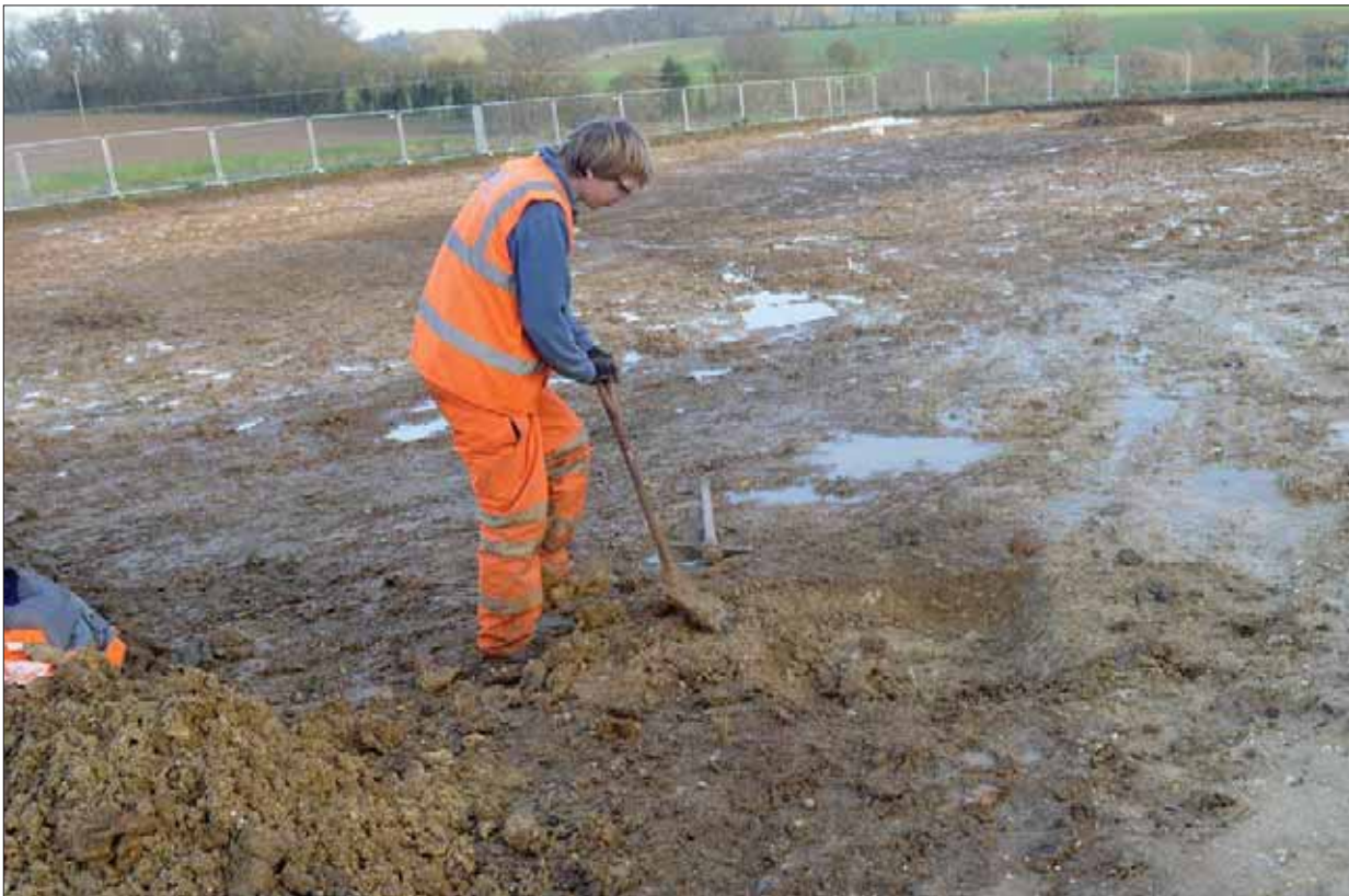
Plate 5: Hand excavation in Area 2, looking north
