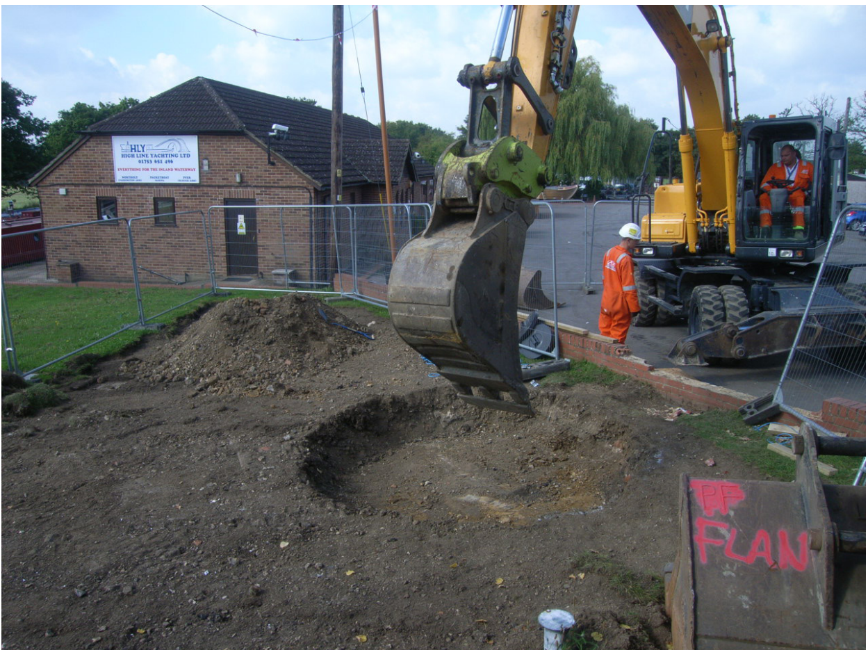
Plate 4: Excavating the reception pit
