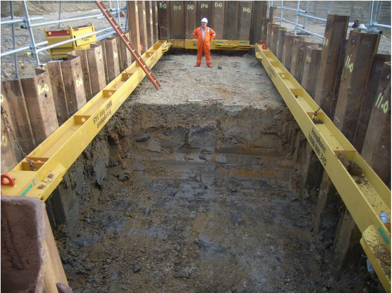
Plate 7: The thrust pit fully excavated
