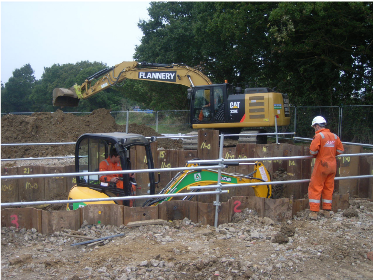
Plate 6: Mini-digger excavating the thrust pit
