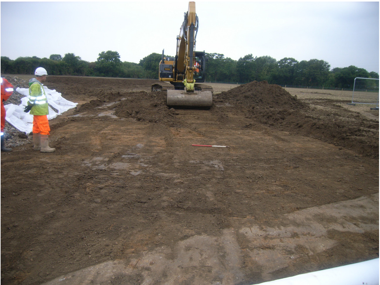
Plate 1: Topsoil stripping in the compound
