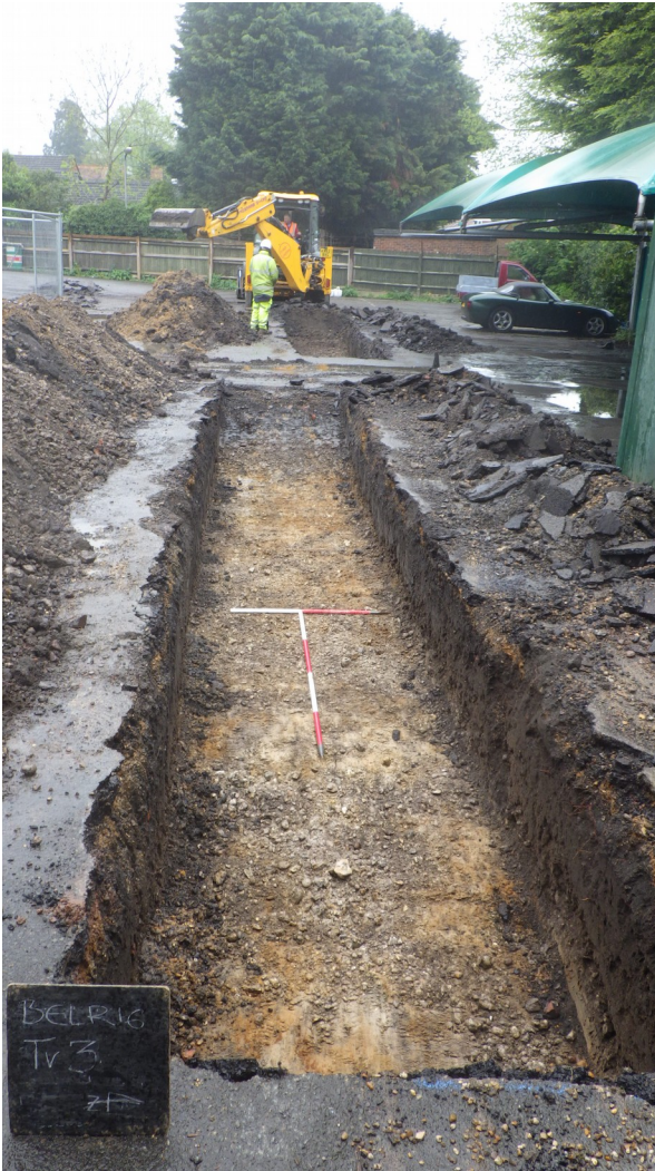
Plate 3: Trench 3 looking east (scale 1x1m and 1x2m)
