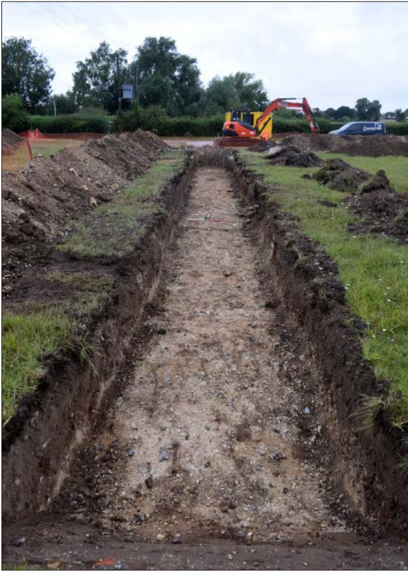
Plate 3: Trench 4 from the south-east
