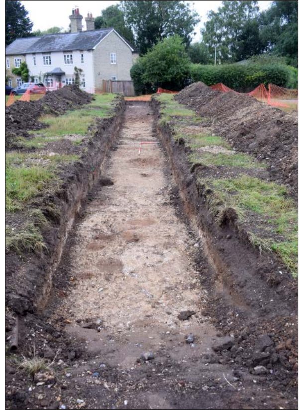
Plate 4: Trench 5 from the north-east
