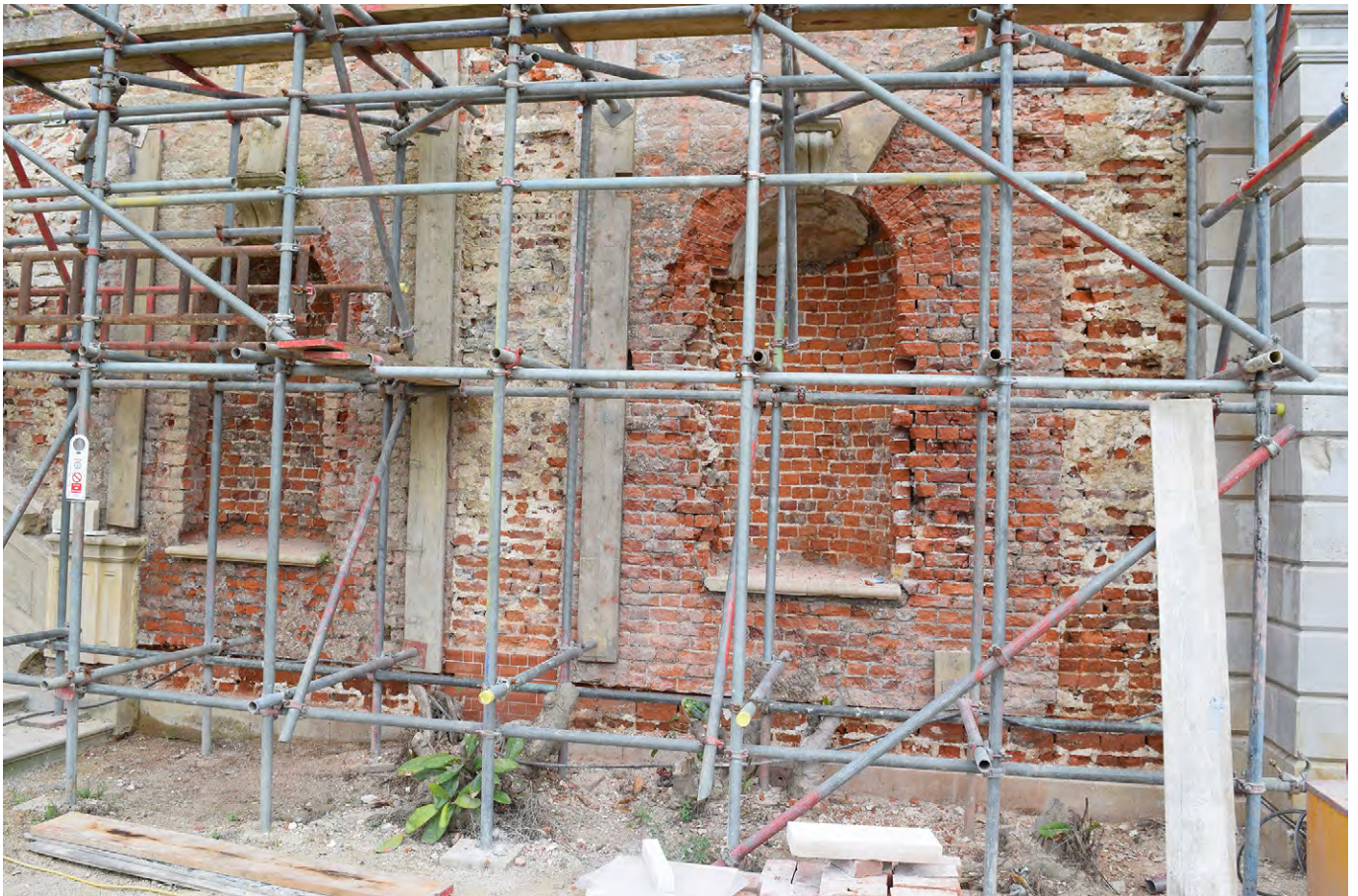
Plate A.16: Western face of stairs after removal of render
