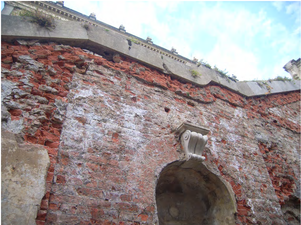
Plate A.18: Fine brickwork on west side after removal of render
