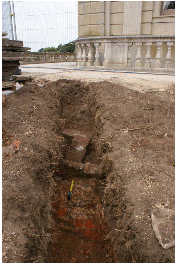
Plate I.9: Wall exposed at south-west corner of Duke's Lawn [I.105.1]
