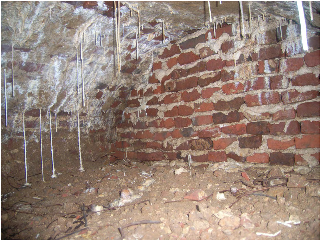
Plate A.41: Vault beneath western lower landing
