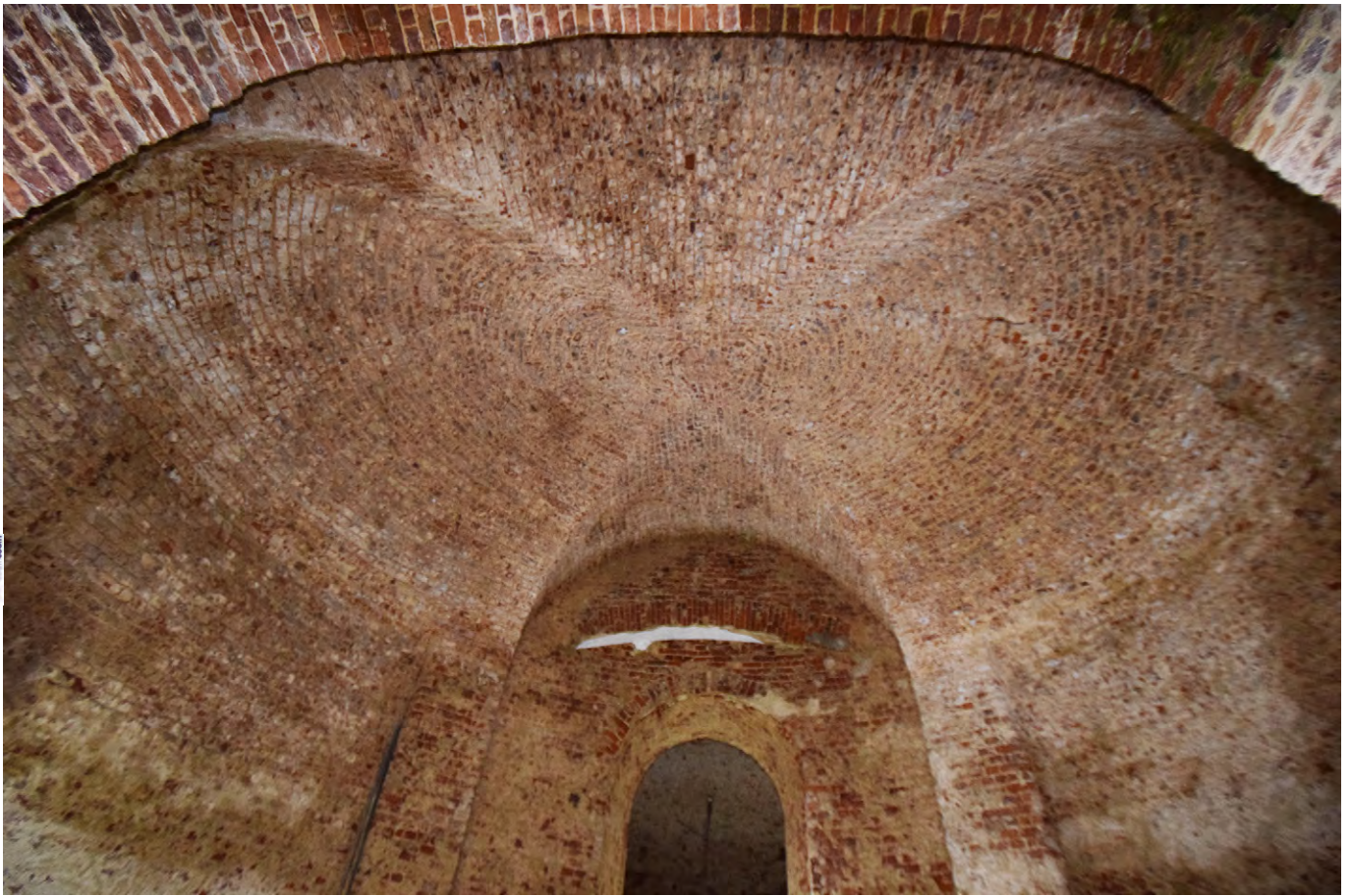
Plate D.3: Vault of central chamber [D.2] after plaster removal, looking north
