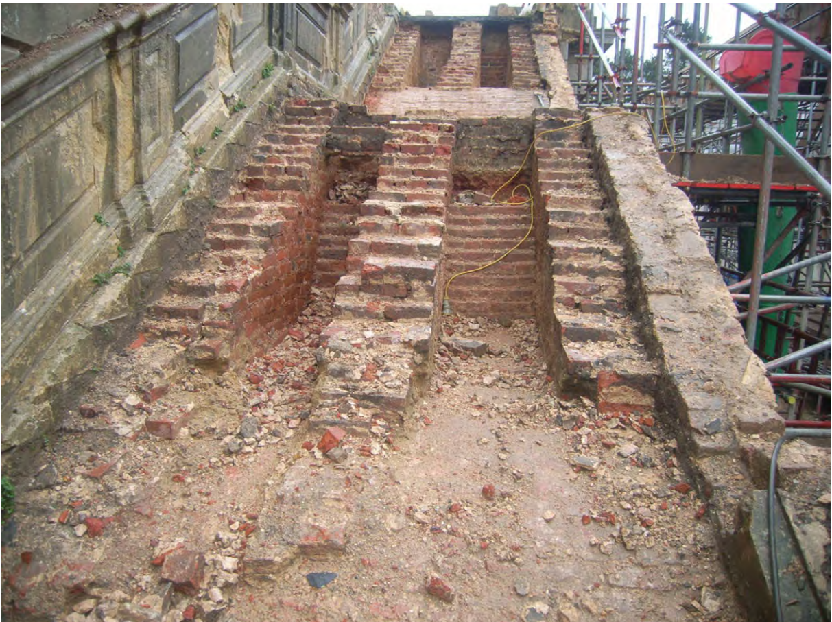
Plate A.34: West side of stairs during dismantling
