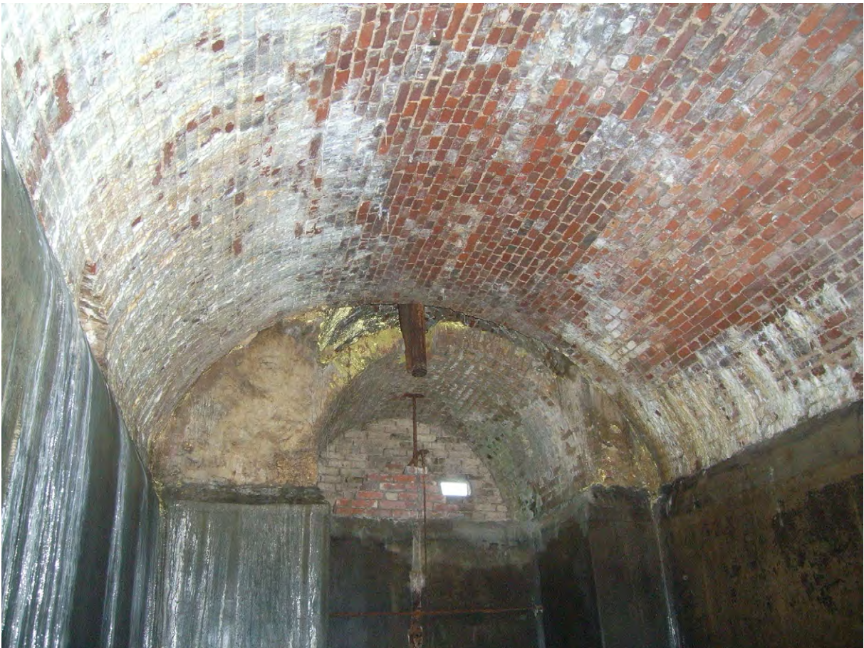
Plate E.11: Interior of East Barrel Vaulted Chamber looking south
