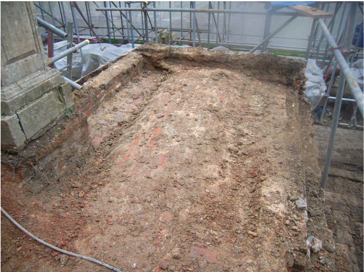
Plate A.32: Vault after removal of western lower landing
