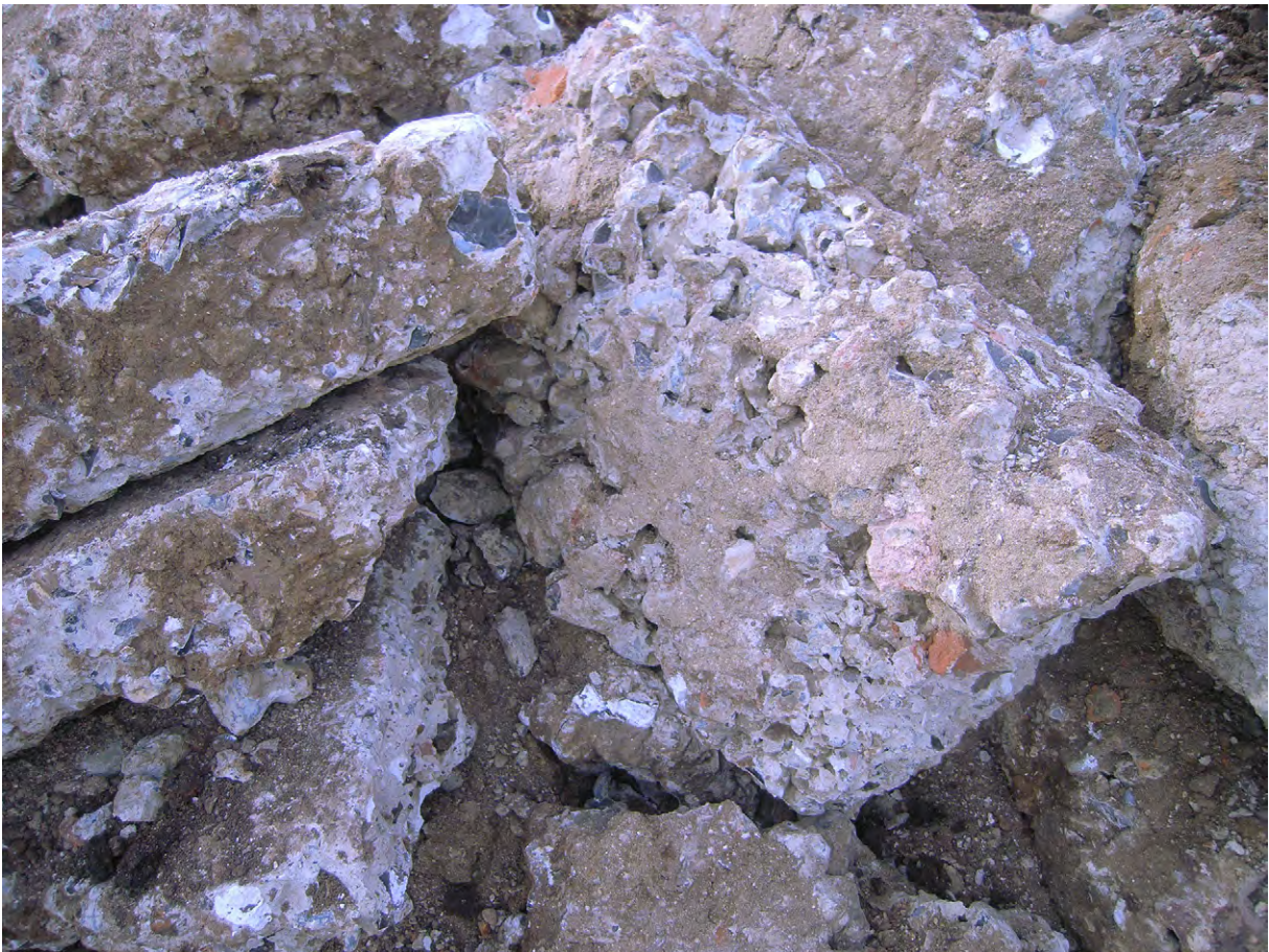
Plate G.43: Detail of 'lumpy' limecrete edging after removal
