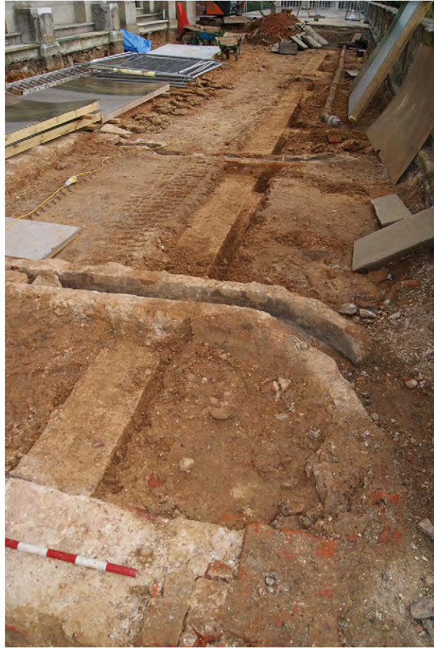
Plate F.43: East-to-west wall [F.2.1] towards front of terrace and overlying drains, looking east
