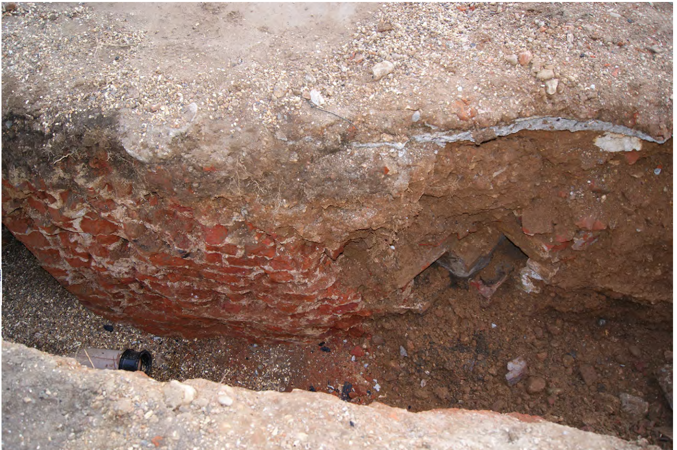
Plate F.66: Former north wall of terrace [F.106.1] and drainage channels, looking SE
