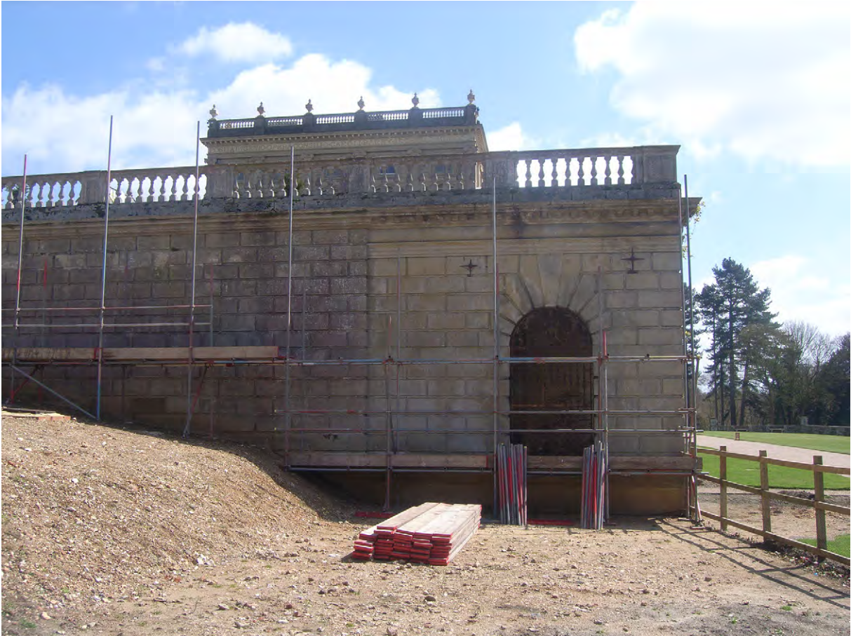
Plate C.3: West elevation of West Fernery, looking east
