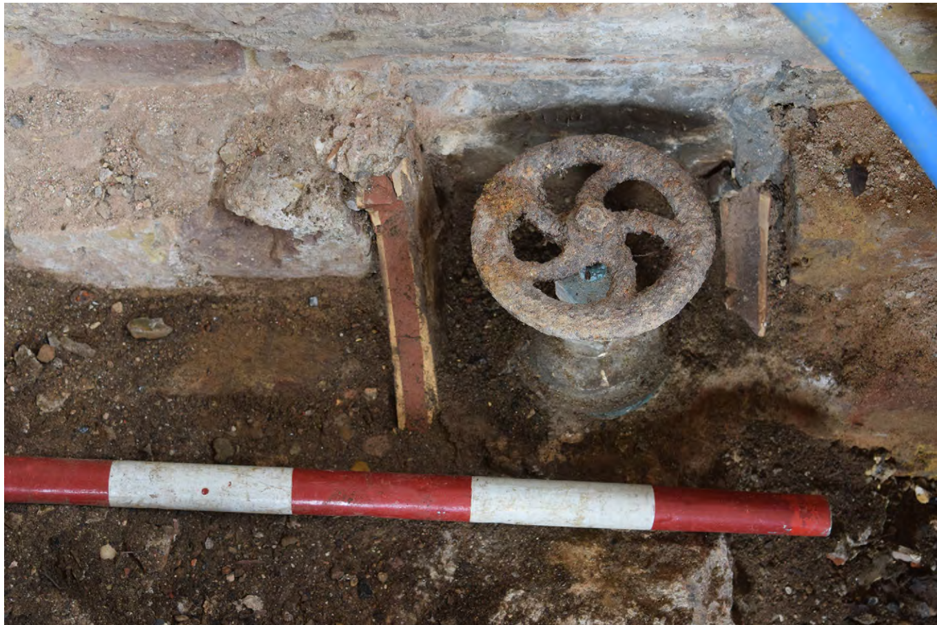
Plate C.15: Tap at SE corner of West Fernery, looking east [C.1.9]
