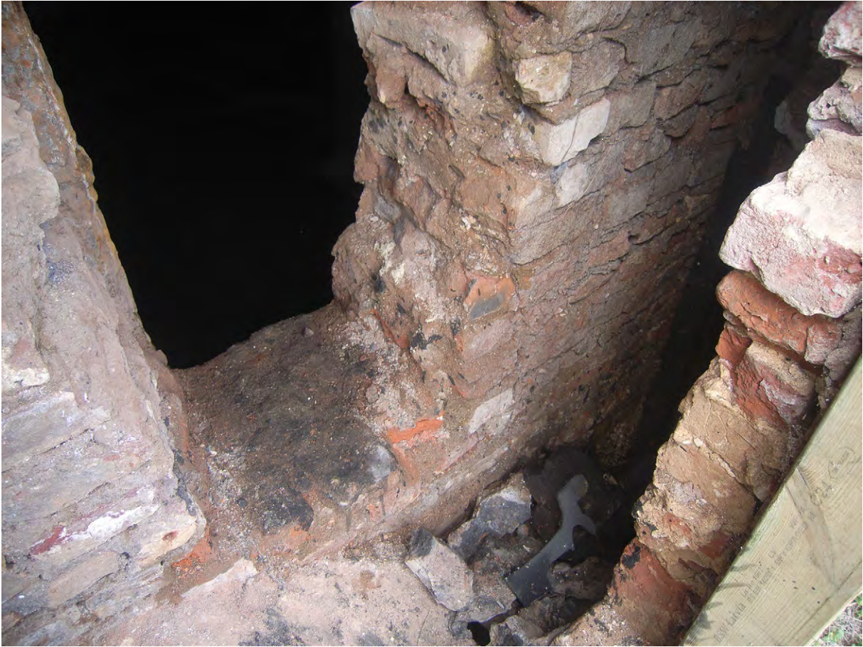
Plate E.10: Detail of entrance formed into East Barrel Vault Chamber
