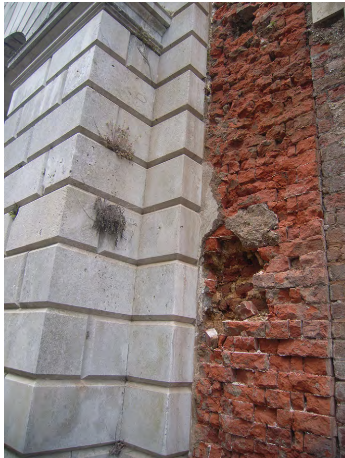
Plate A.48: Portico and brick junction on east side
