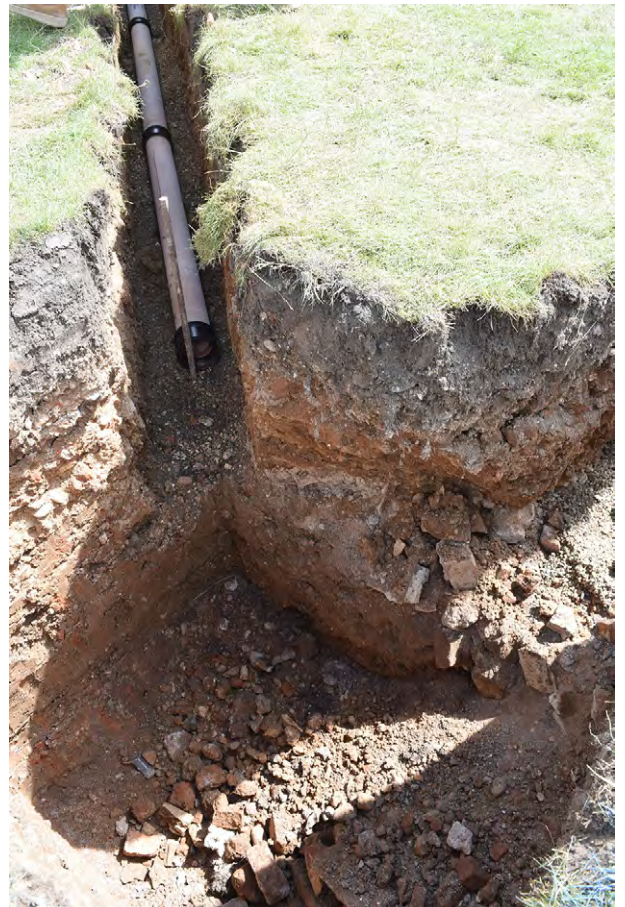
Plate I.5: Trench into soakaway [I.101] towards centre of West Lawn, looking south-east
