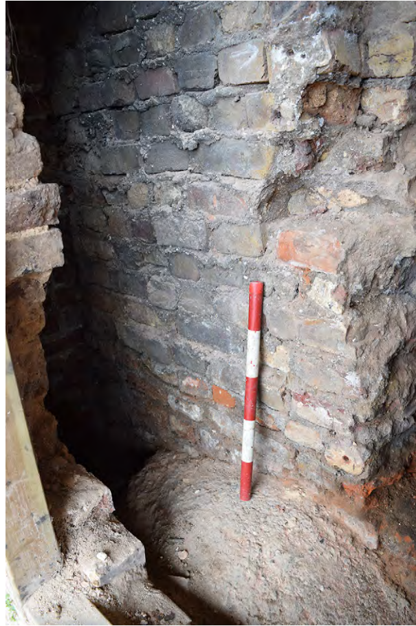
Plate E.3: Rear of late 19th-century wall behind blind arcade to West Barrel Vaulted Chamber
