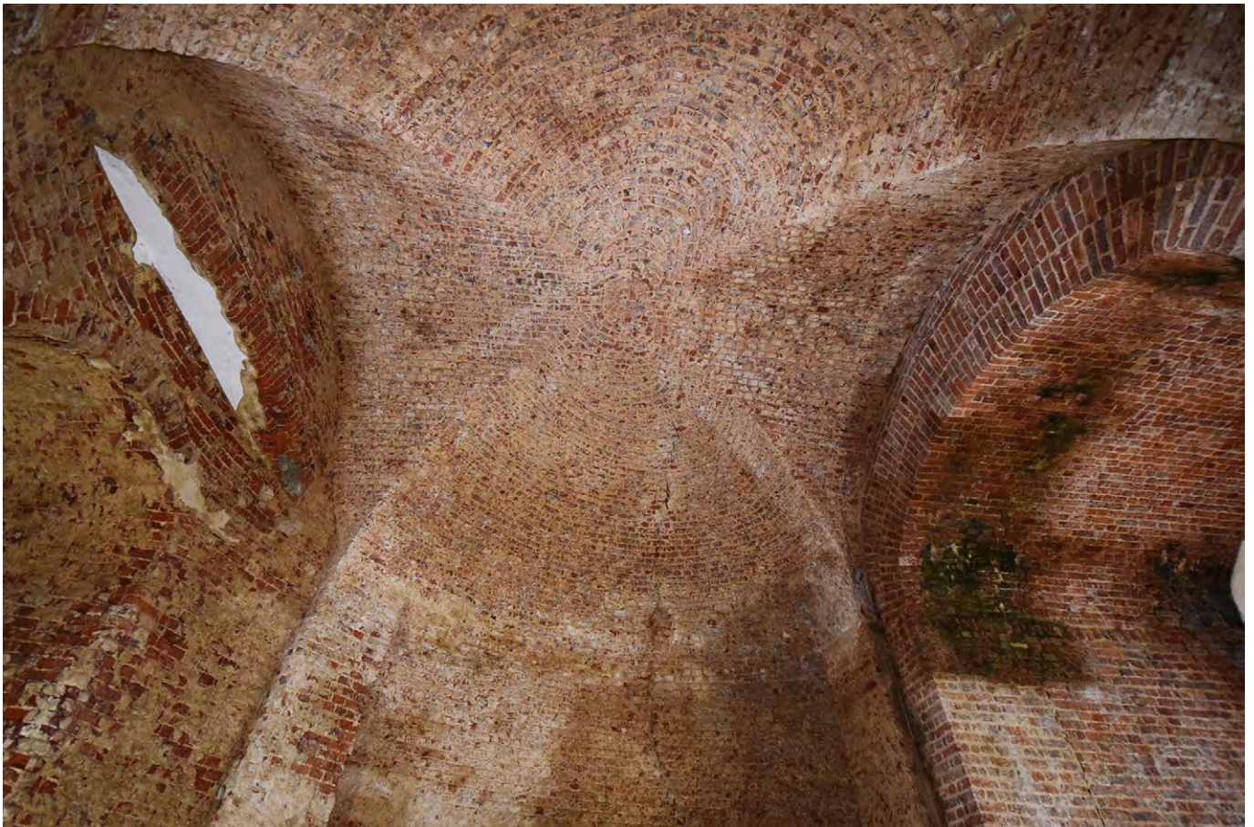
Plate D.4: Vault of central chamber [D.2] after plaster removal, looking east
