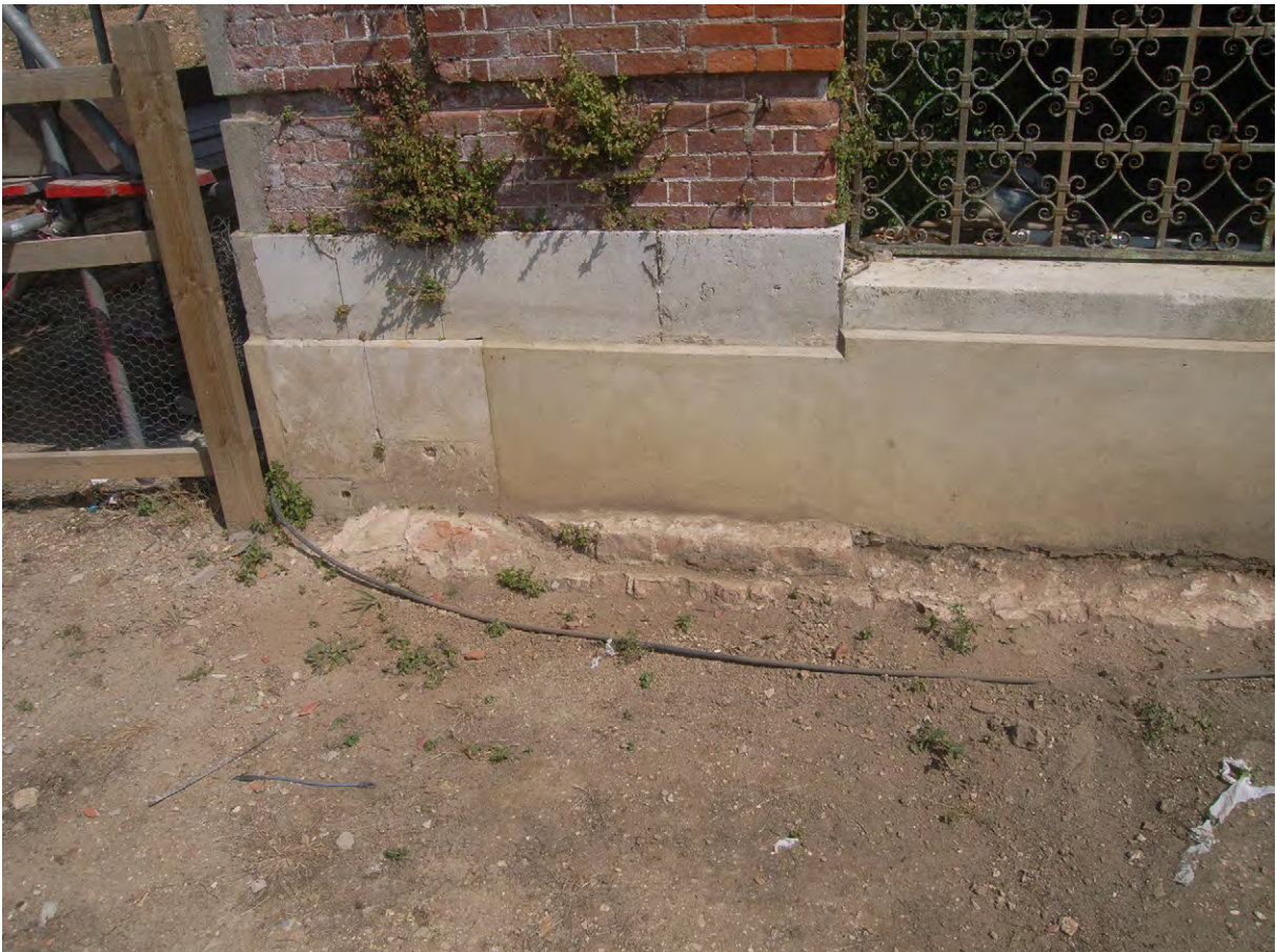
Plate C.4: Footings visible beneath front wall of West Fernery, looking north
