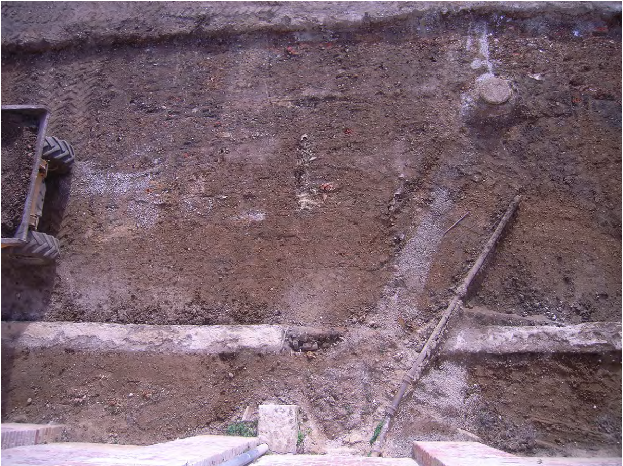
Plate G.40: West side of Blind Arcade with exposed limecrete edging in front [G.119.3]
