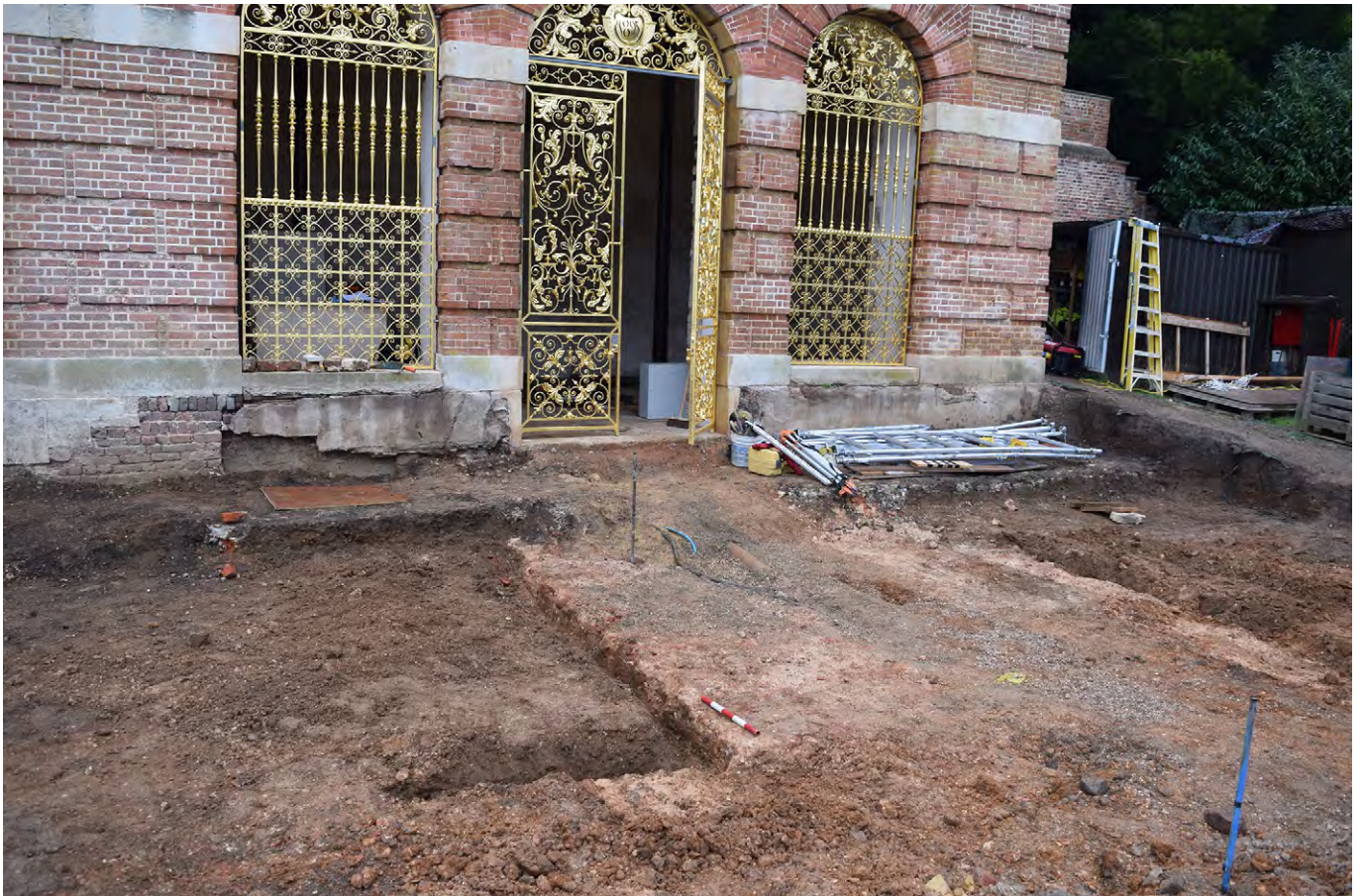
Plate G.23: Trace of brick base exposed in front of East Fernery [G.119.1], looking north
