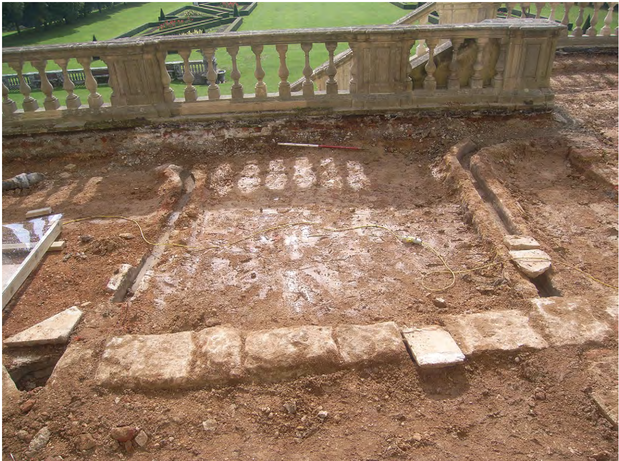
Plate F.29: Area of terrace just to east of centre showing Drain 8 [F.2.13], Drain 9 [F.2.14] and Drain 10 [F.2.15], looking south
