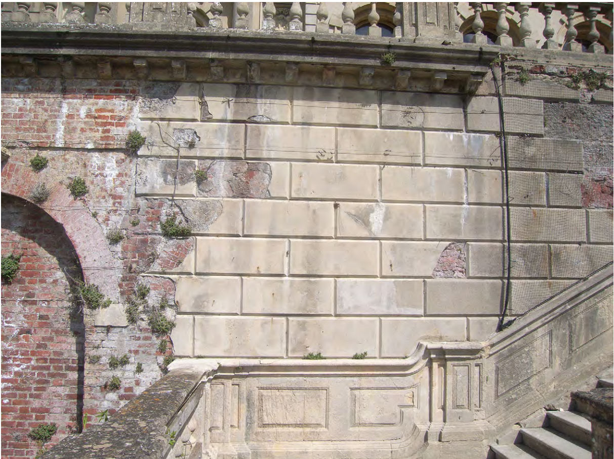
Plate B.8: Rustication behind west side of stairs
