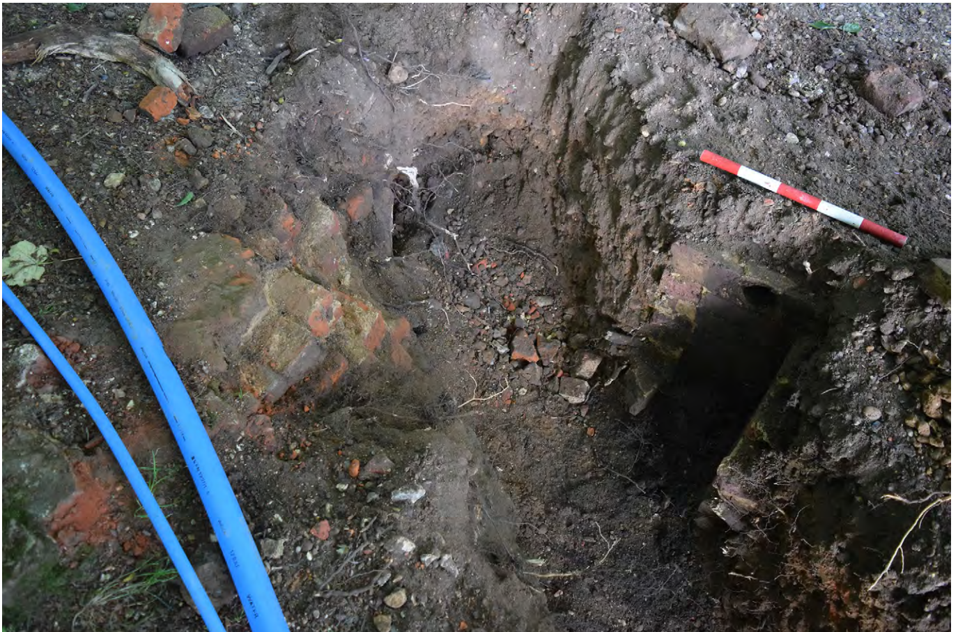
Plate J.11: Wall [J.1.1] to left and small brick sump [J.1.2] exposed to east of terrace, looking north
