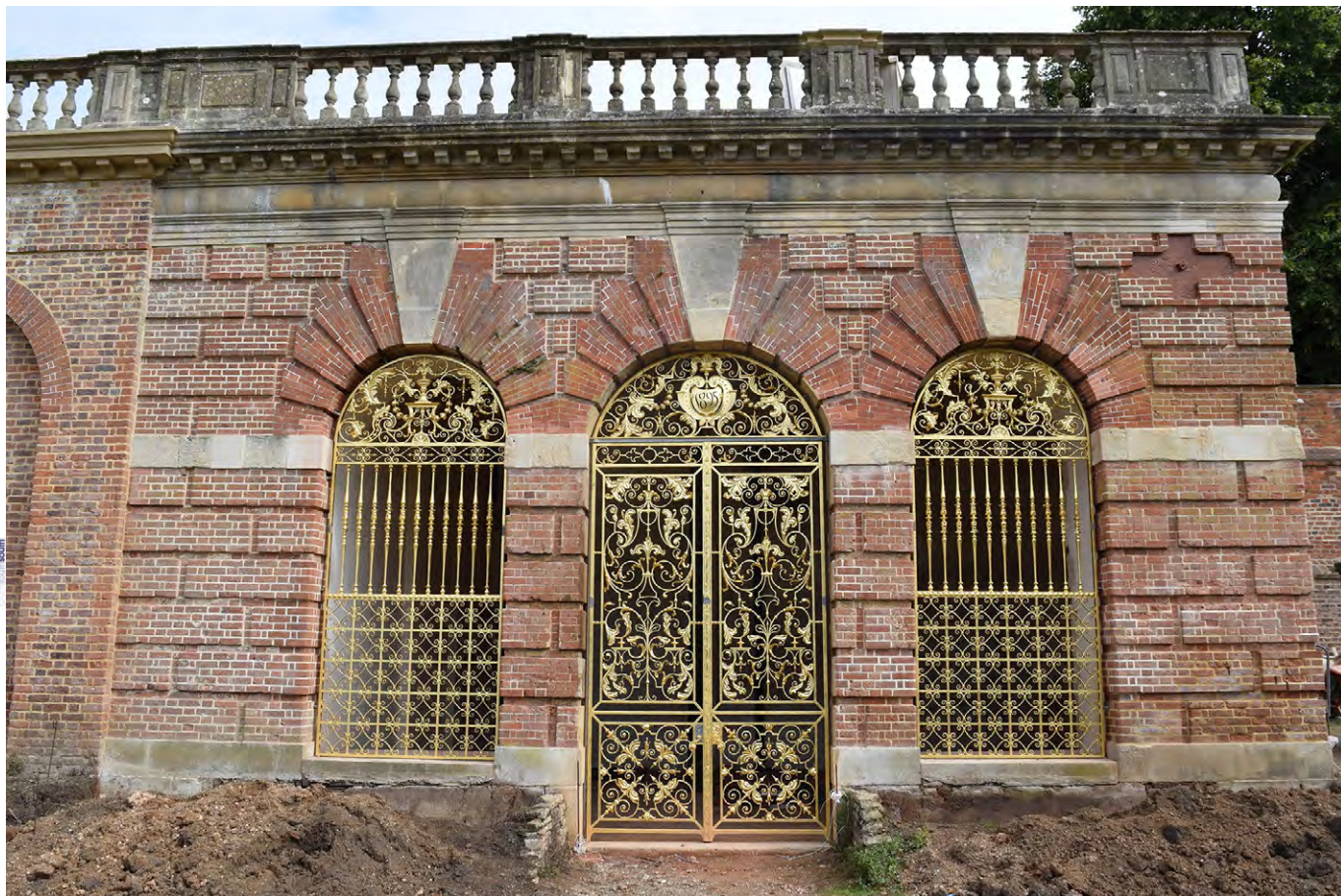
Plate C.46: South face of East Fernery with lower banks removed
