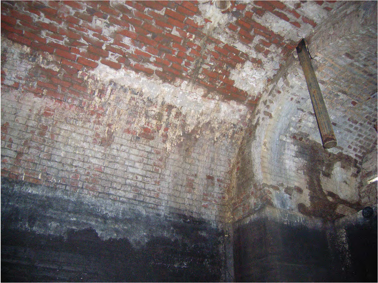
Plate E.5: Southern end of West Barrel Vaulted Chamber
