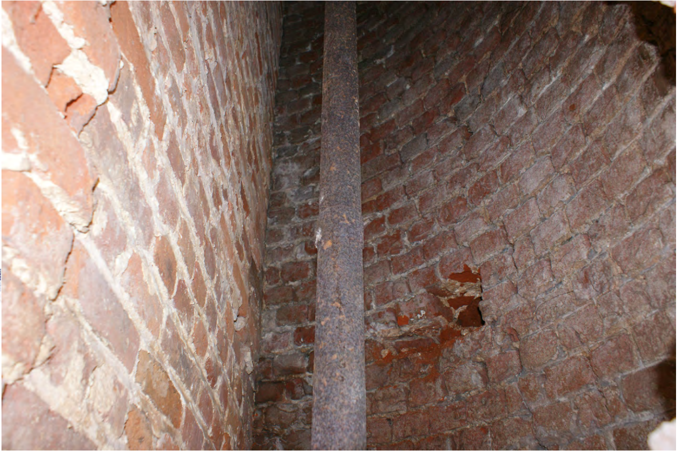
Plate B.21: Hidden brickwork from former niche behind later blind arcade exposed by NT in 2012
