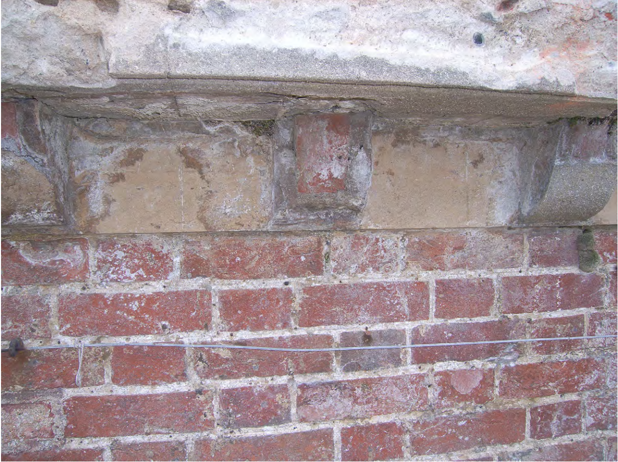
Plate B.19: Detail of exposed rendered brick bracket in cornice
