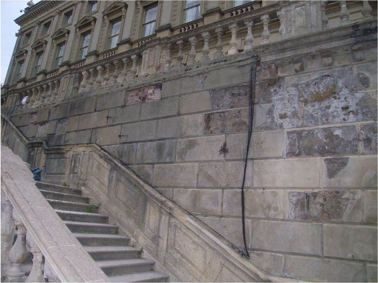
Plate B.9: Upper part of eastern rustication
