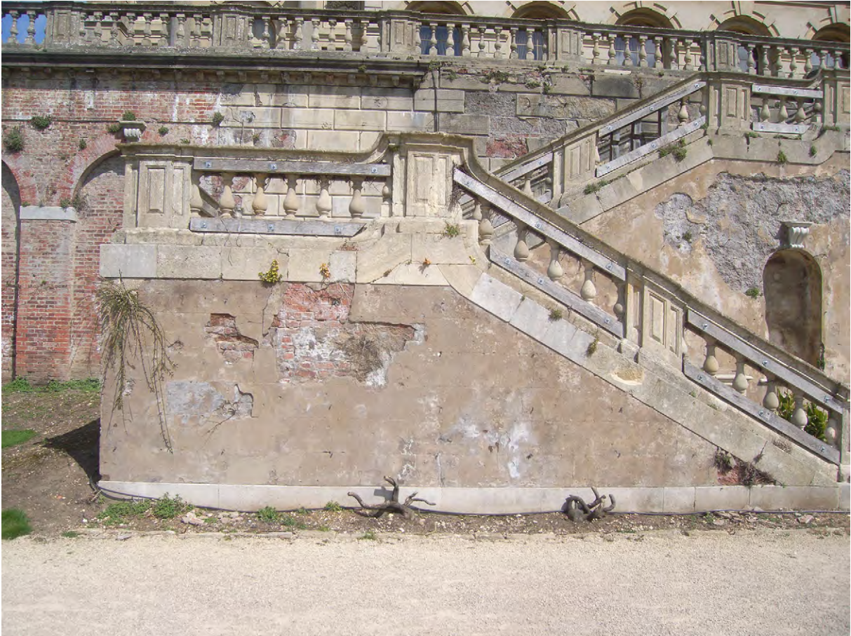
Plate A.3: West lower flight prior to start of works
