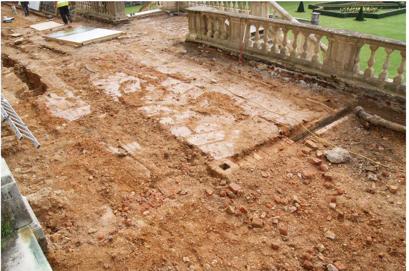
Plate F.18: Central part of terrace looking south-east. Note puddling clay and drain 1 [F.2.6]
