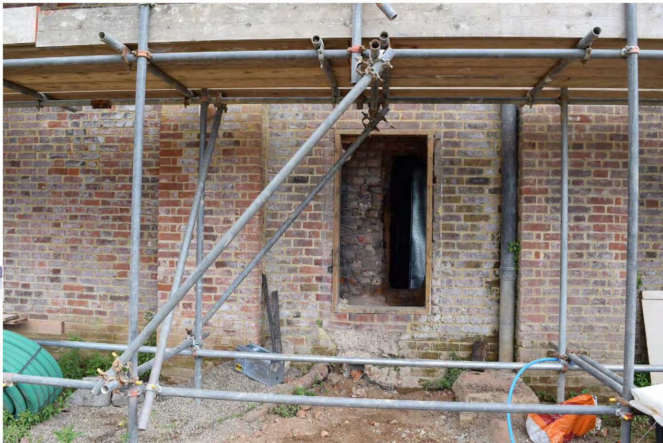
Plate E.1: Entrance formed in blind arcade to West Barrel Vaulted Chamber
