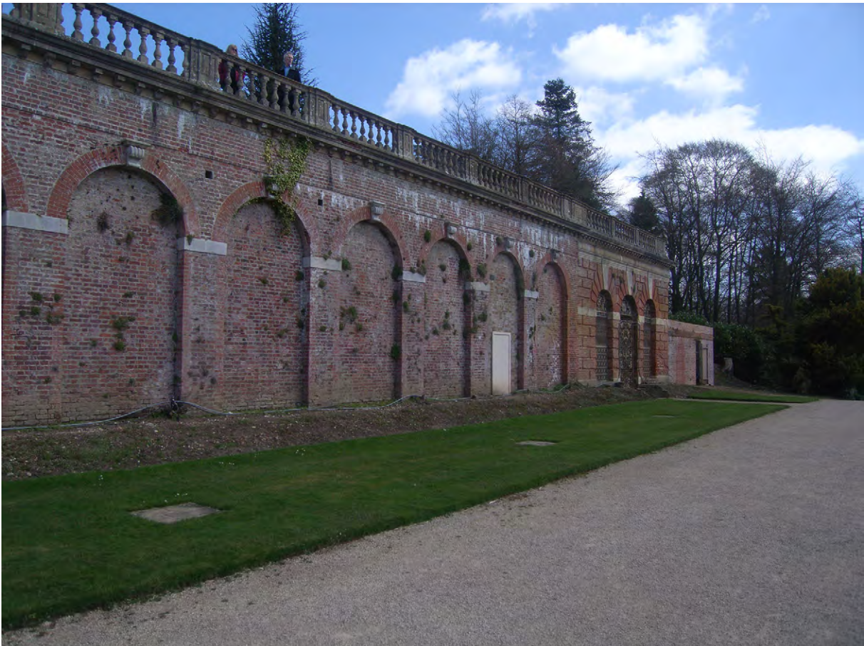
Plate B.6: General view of east blind arcade
