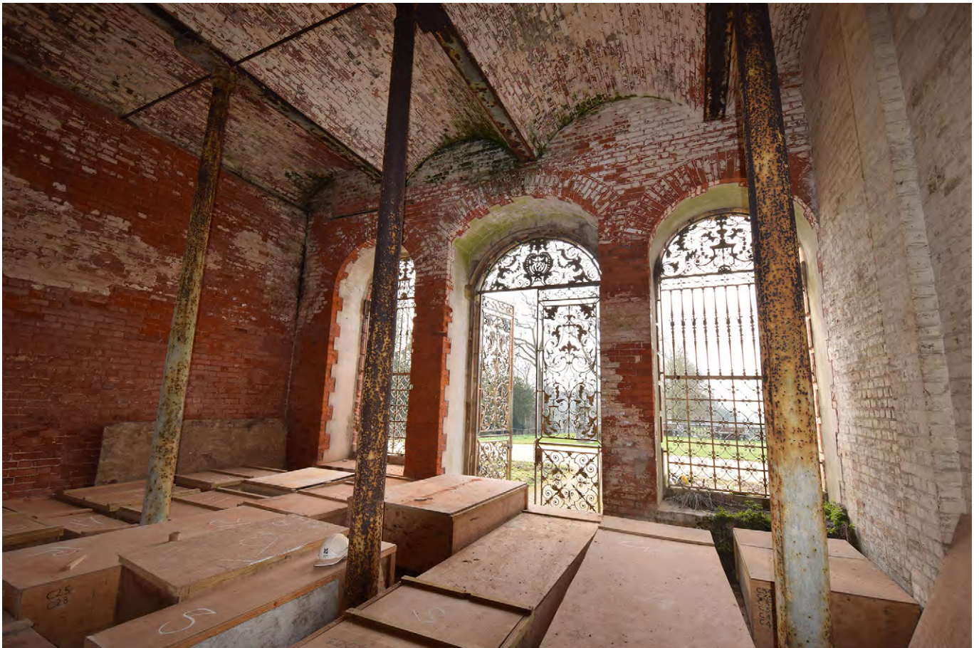
Plate C.29: Interior of East Fenery (south wall), looking south
