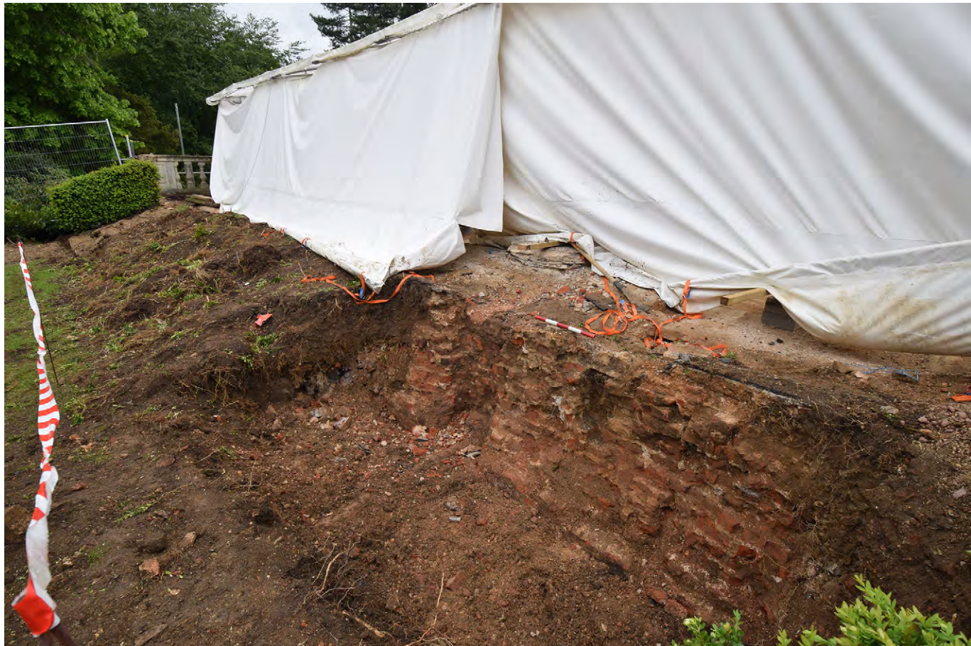
Plate I.7: Cut-back north face of Terrace facing Duke's Lawn [F.3.11], looking south-east
