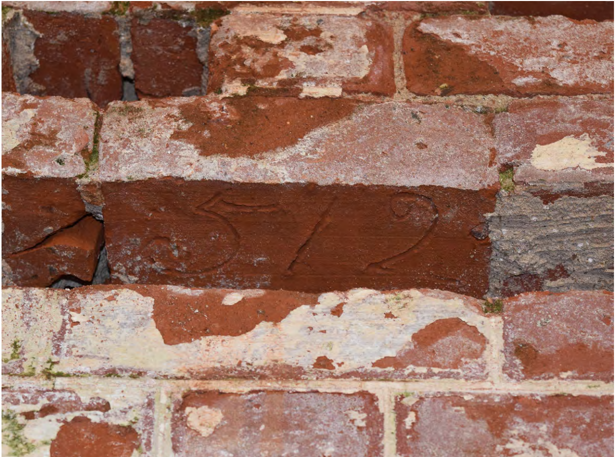
Plate C.17: '5.1.2' batch mark on underside of brick in West Fernery, looking north
