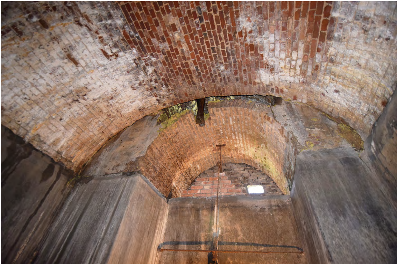
Plate E.15: Southern end of East Barrel Vaulted Chamber
