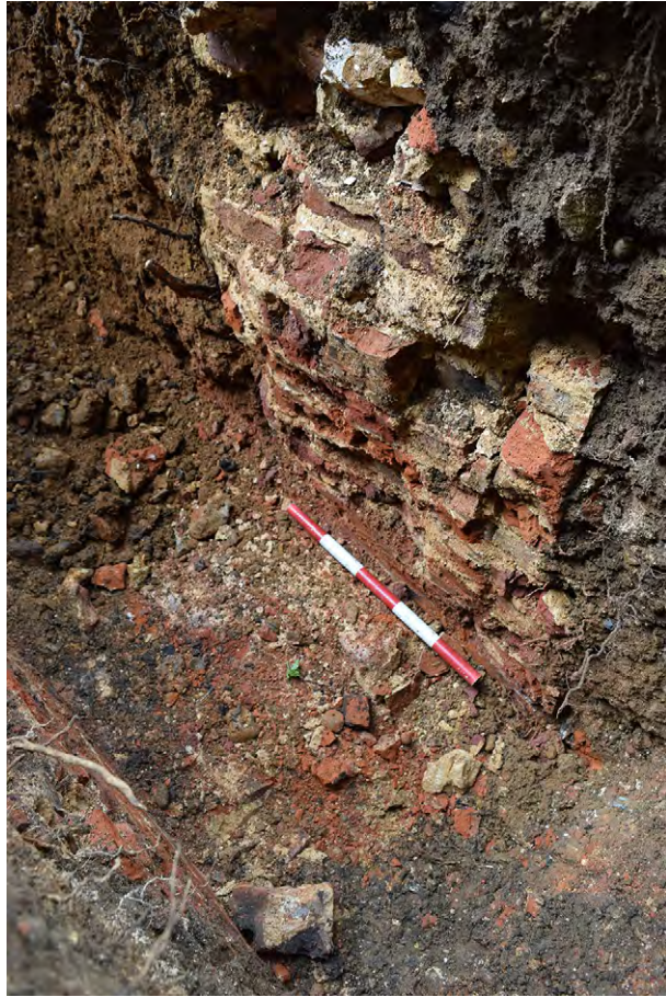
Plate J.4: Wall [J.102.1] after truncation in current works, looking south-east
