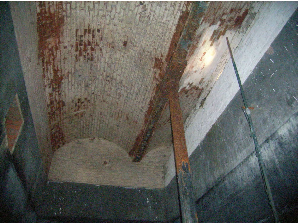
Plate C.39: Vault detail in West Fernery Water Tank, looking south
