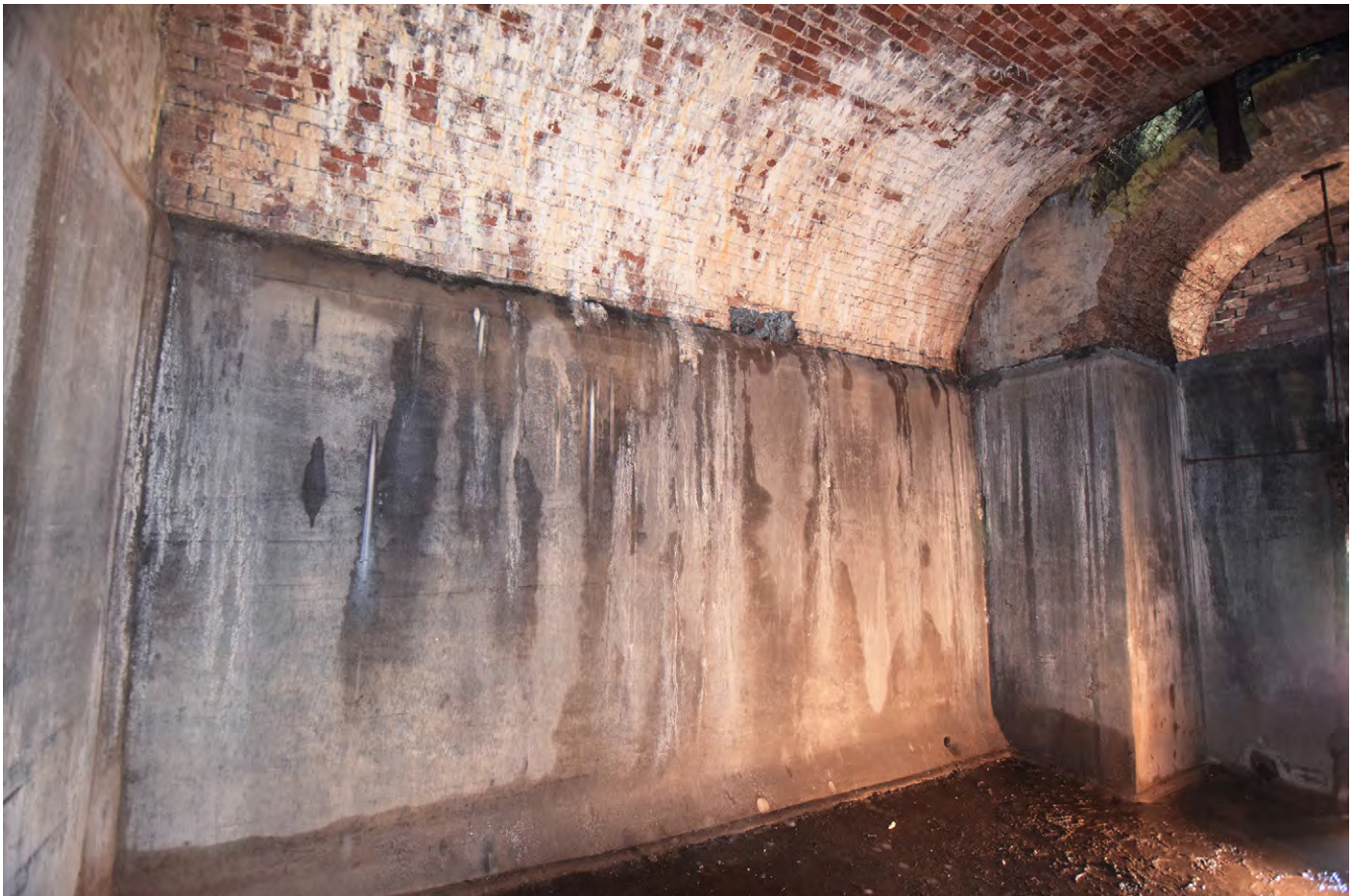
Plate E.13: Interior of East Barrel Vaulted Chamber looking south-east
