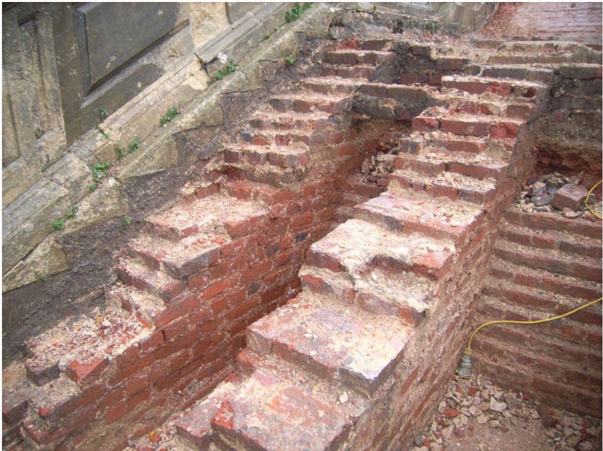
Plate A.35: West side of stairs during dismantling
