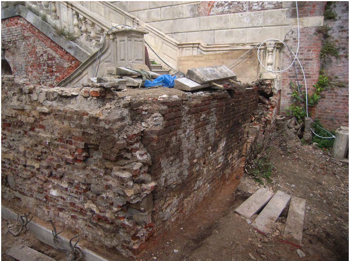
Plate A.49: Eastern stairs during dismantling [A.3.1 & A.3.2]
