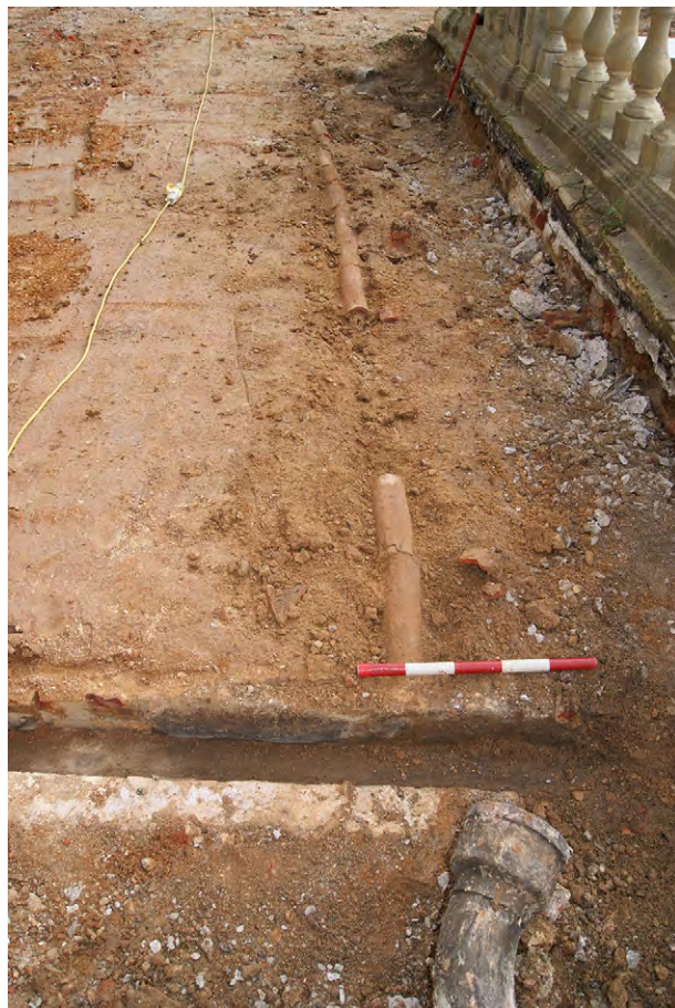
Plate F.24: Horseshoe pipe extending eastwards from Drain 1 [F.2.6], looking east
