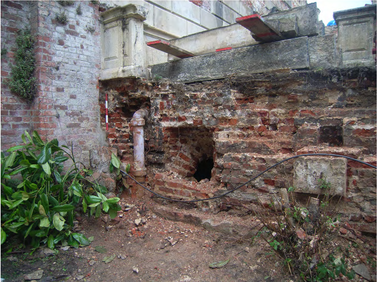
Plate A.25: Detail of west wall [A.4.1 and A.4.2]
