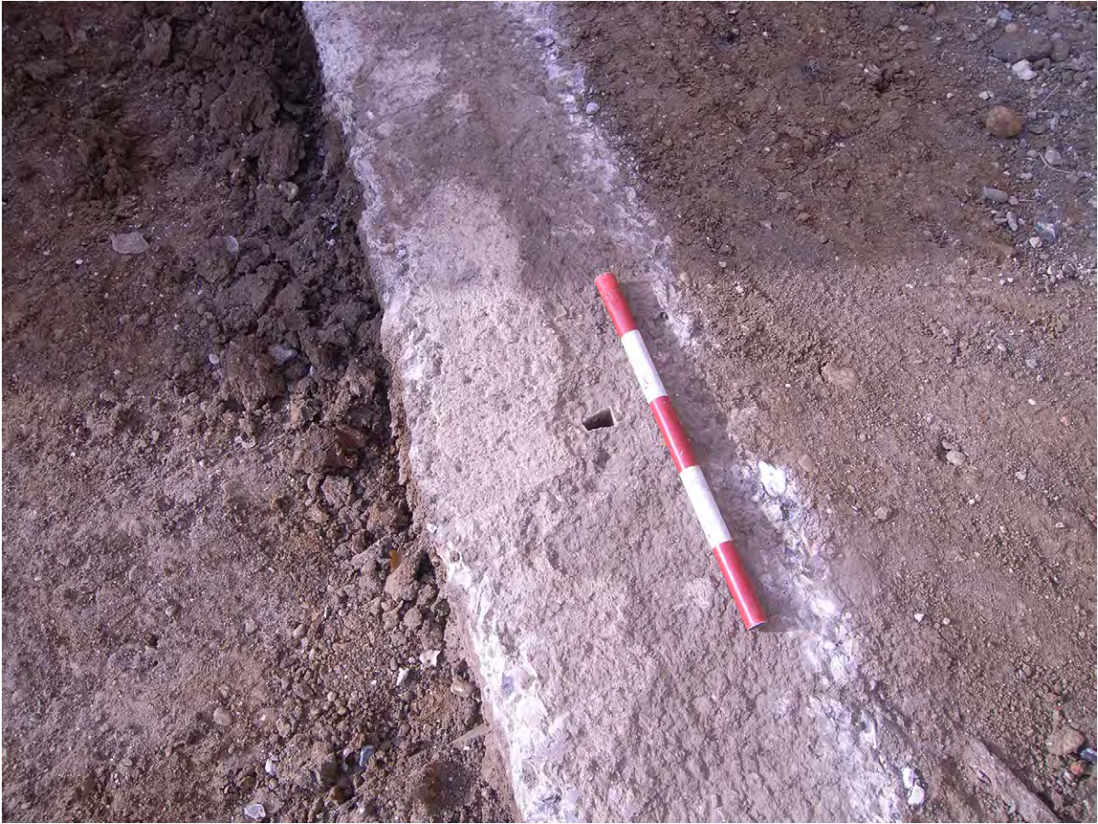
Plate G.42: Detail of limecrete edging with setting-out peg hole
