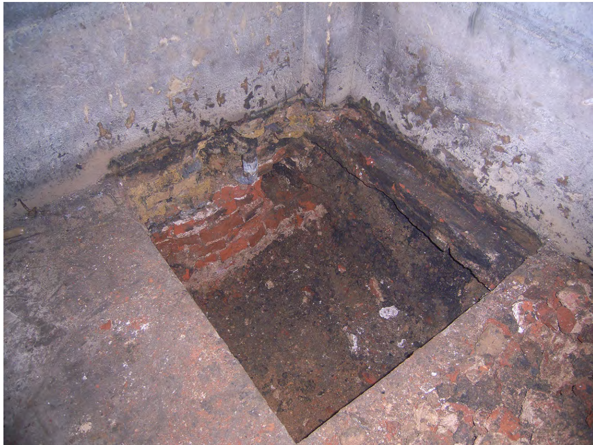
Plate C.43: Pit dug in floor of East Fernery Water Tank , looking south-east
