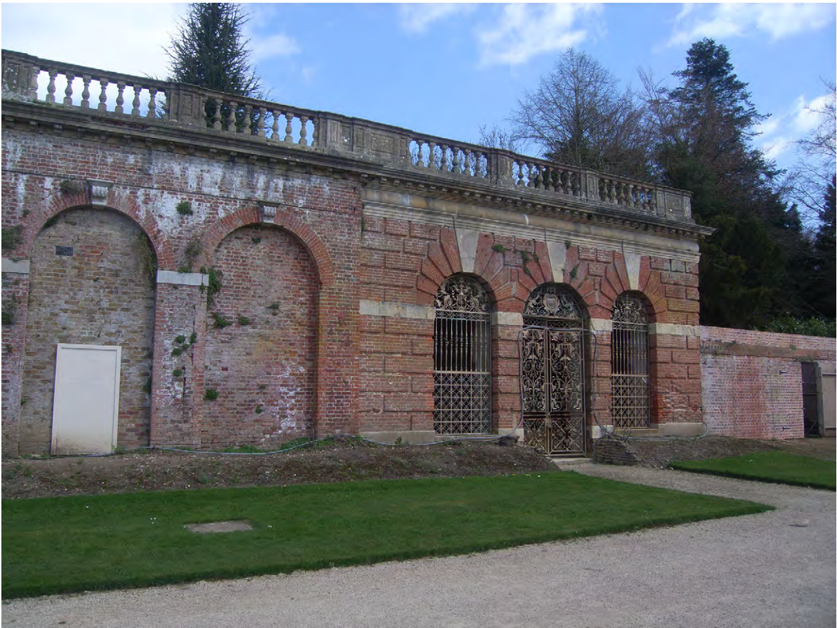
Plate C.23: South face of East Fernery
