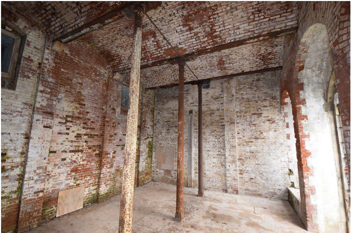
Plate C.6: Interior of West Fernery, looking east
