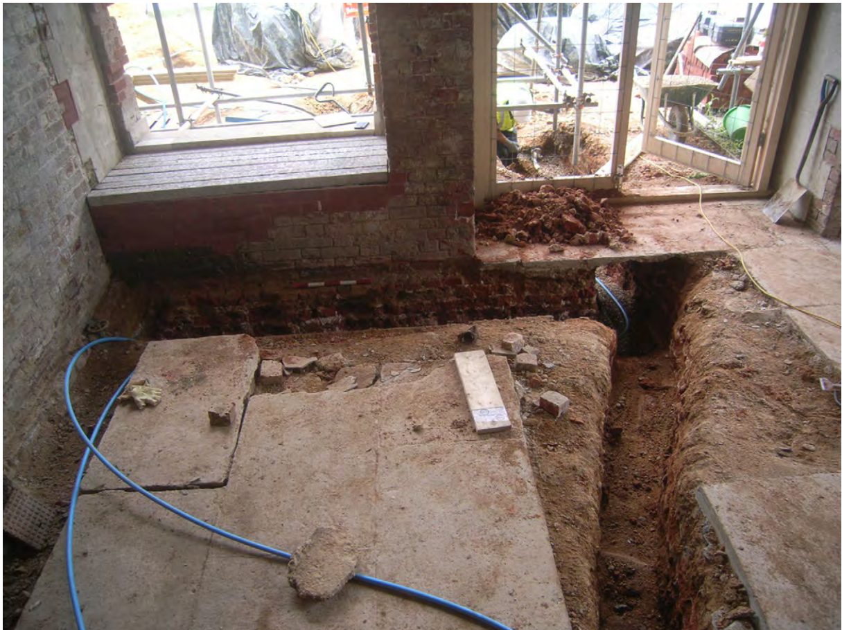
Plate C.20: General view of excavations in West Fernery, looking south
