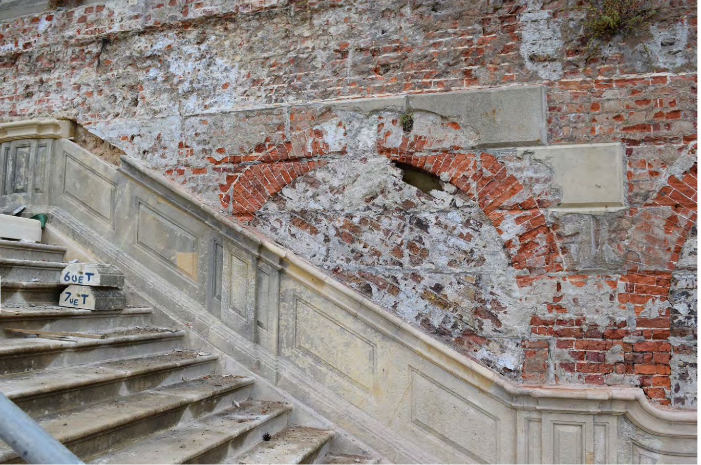
Plate B.15: Arch in east side after rustication removal
