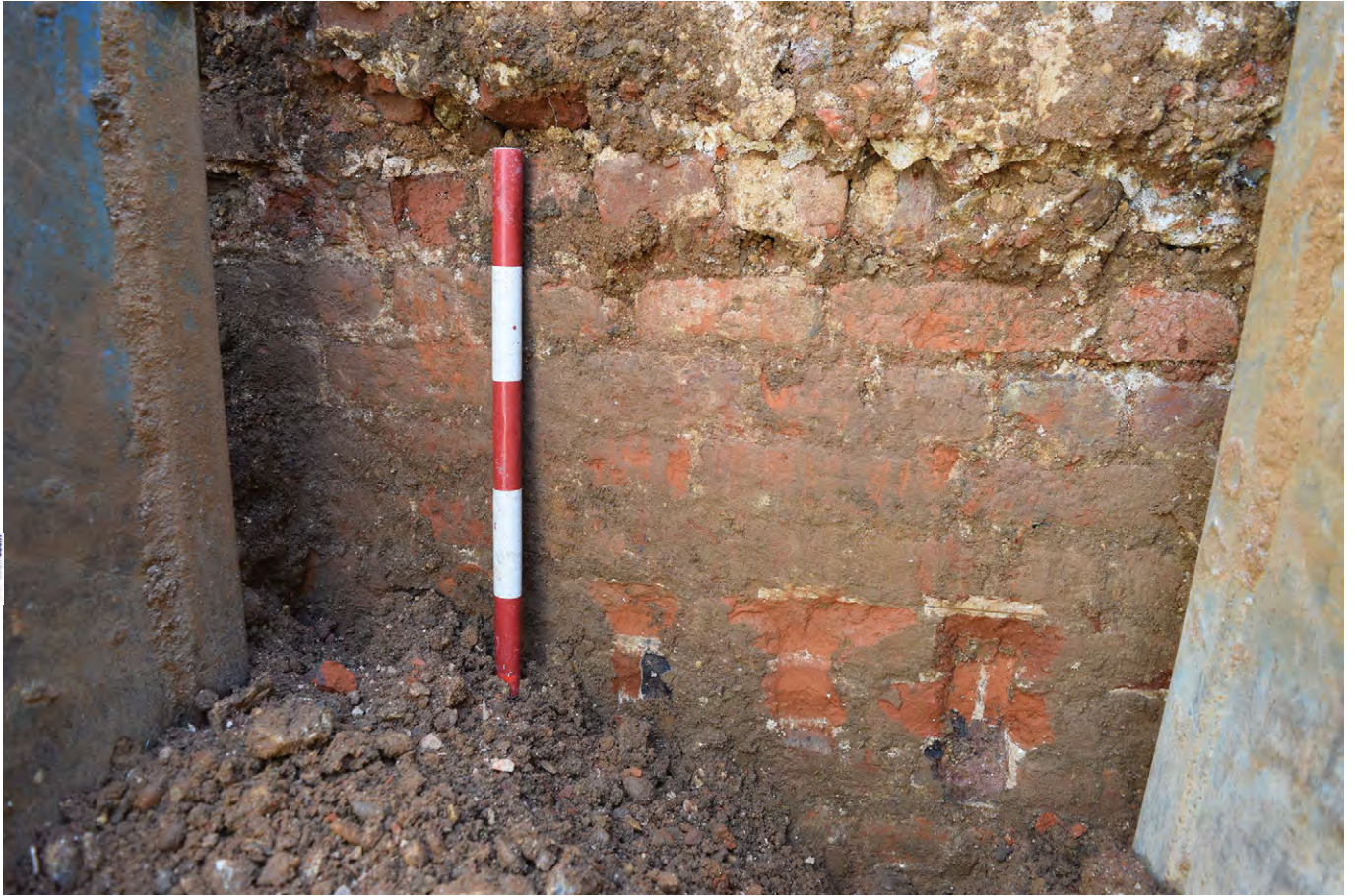
Plate G.9: Detail of large wall found [G.100.17], looking east
