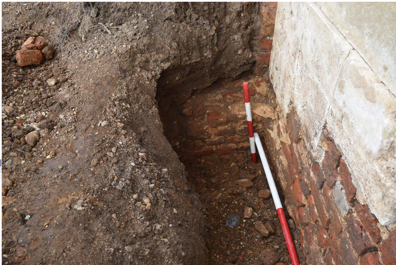
Plate C.48: Brick footing looking west exposed by East Fernery. Possibly supported lower step
