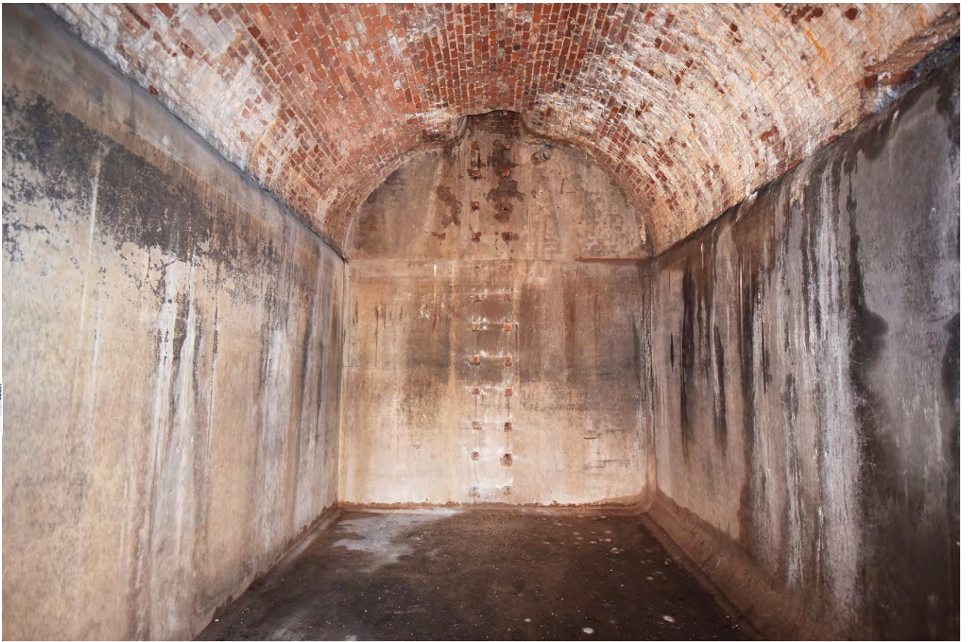
Plate E.12: Interior of East Barrel Vaulted Chamber looking north
