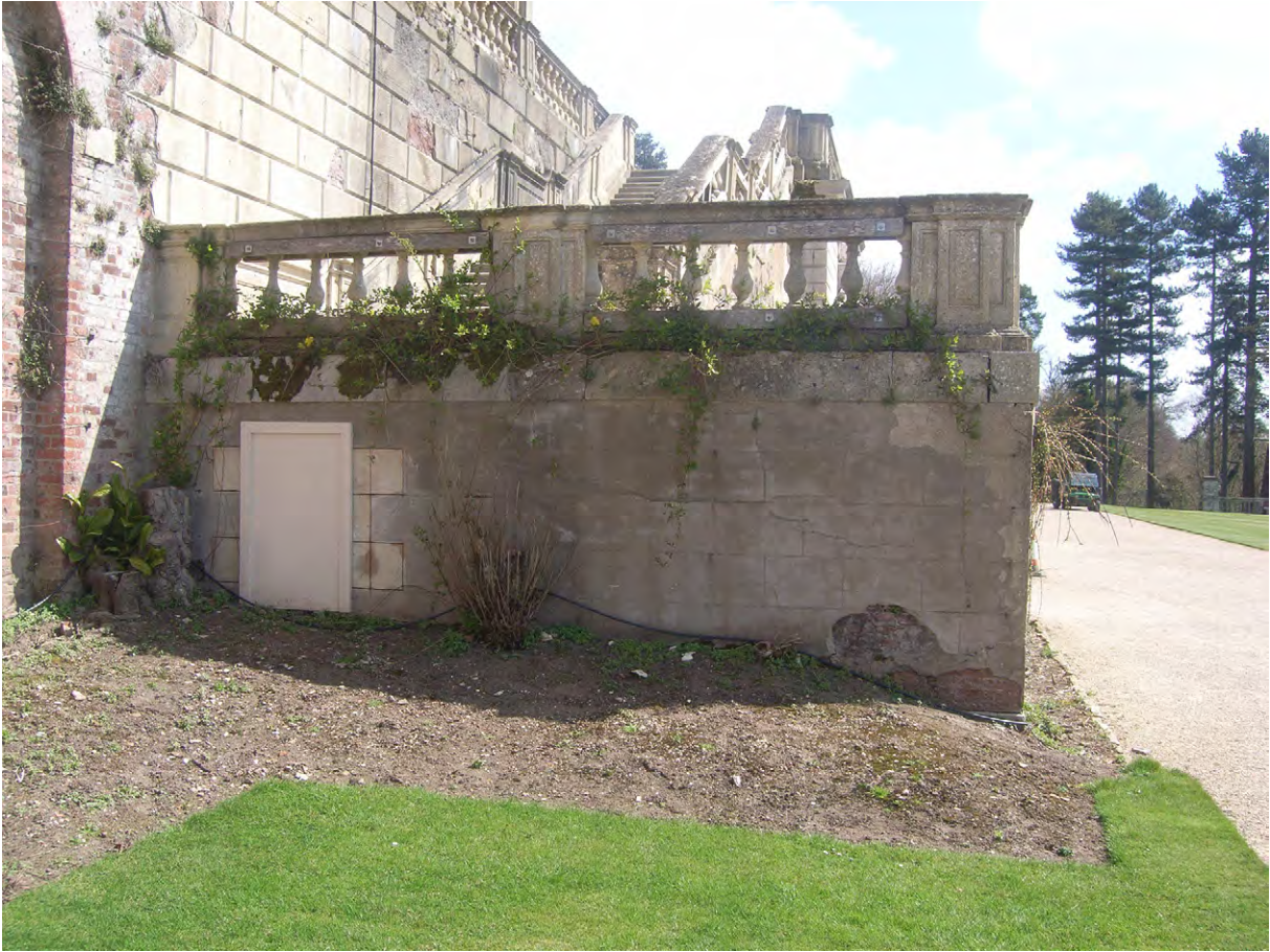
Plate A.5: West return wall in staircase
