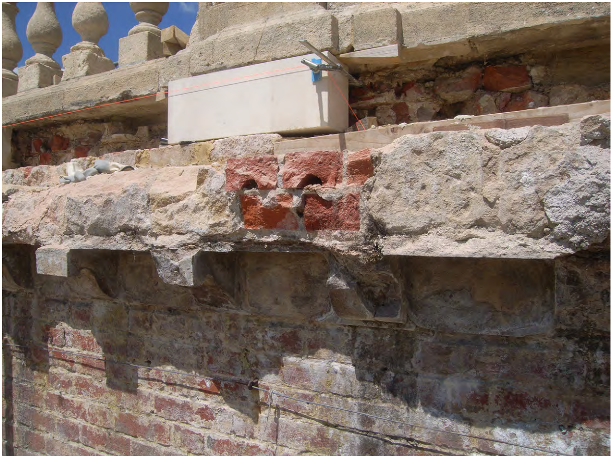
Plate B.18: Detail of cornice
