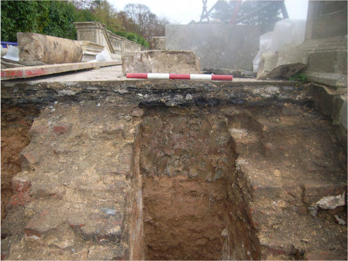
Plate A.39: Clay at top of west side of stairs
