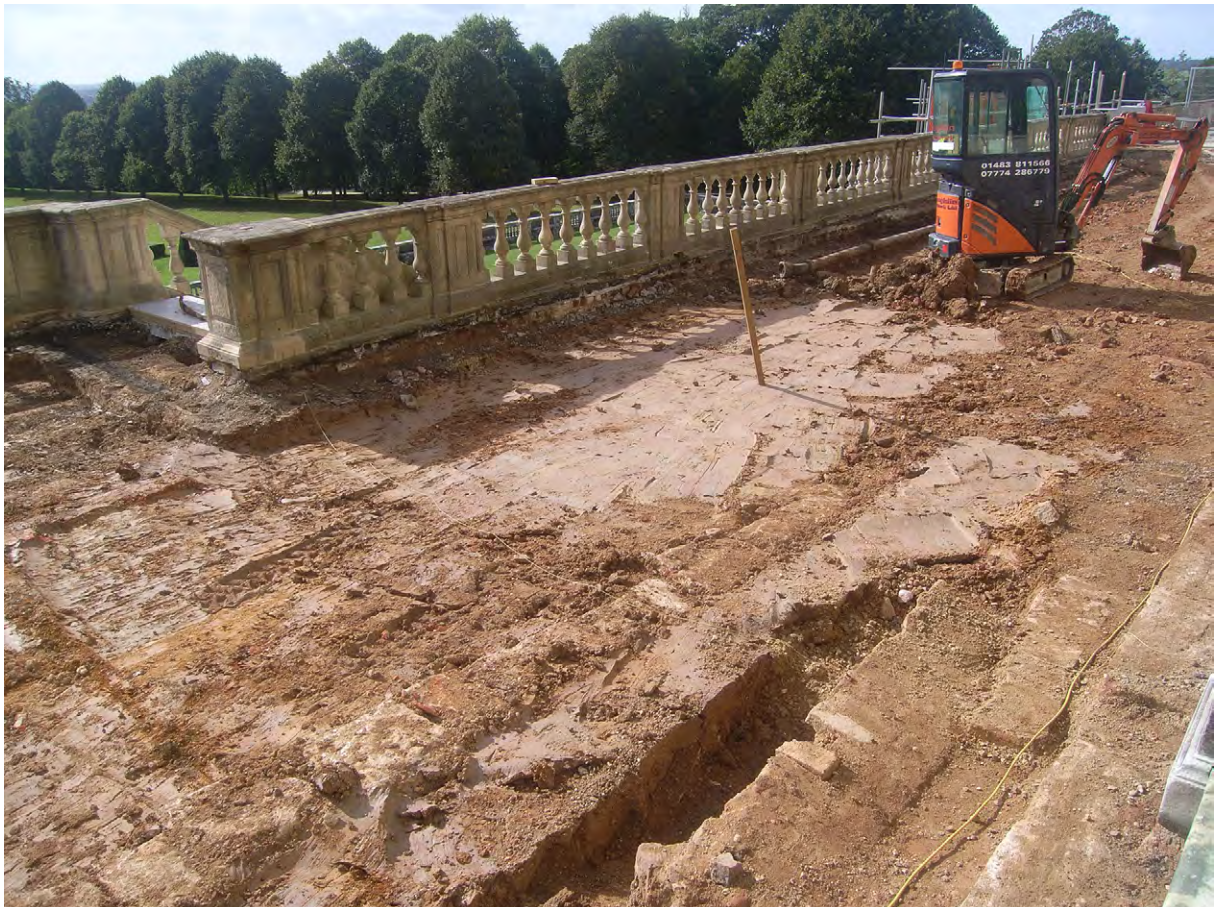
Plate F.17: Central part of terrace looking south-west after removal of paving and upper loose fill. (note clay pudding)
