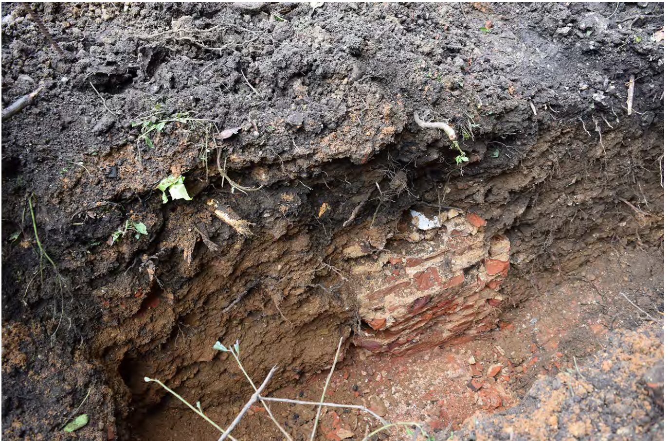
Plate J.3: Wall [J.102.1] after truncation in current works, looking south-west
