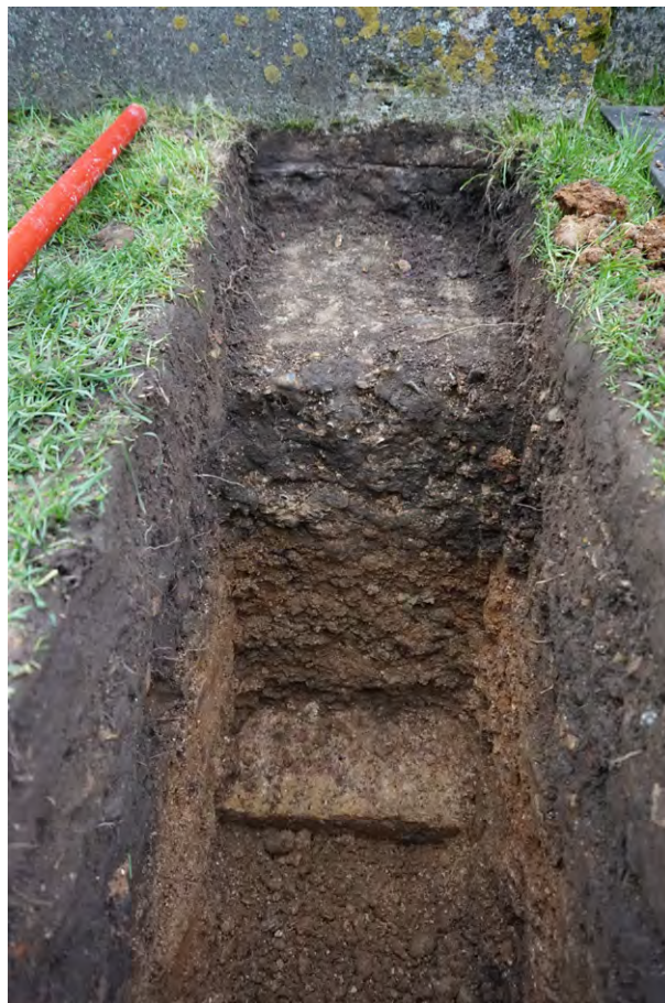
Plate G.51: Footings exposed beneath Borghese Balustrade within trial pit [G.113]
