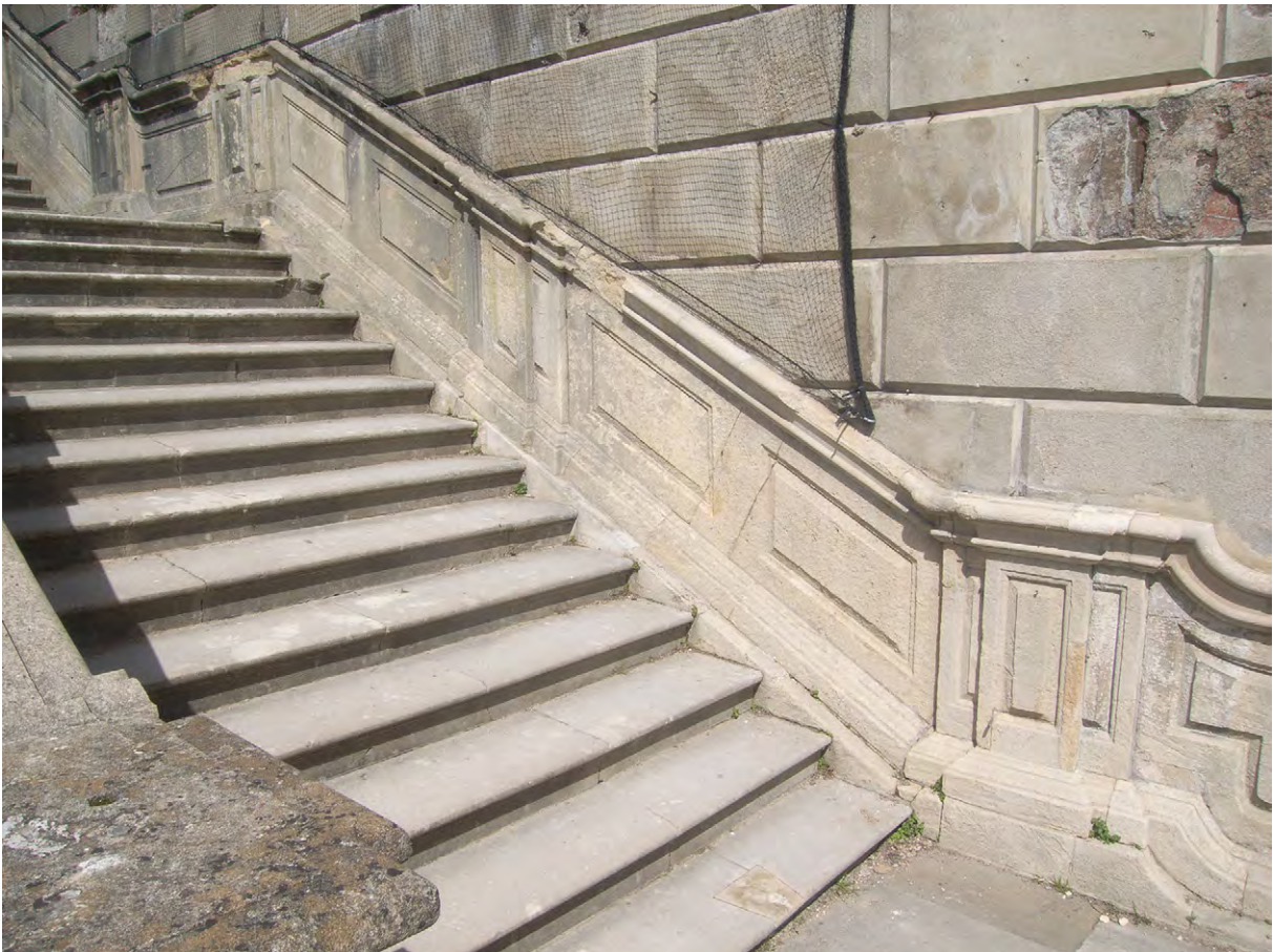
Plate A.14: Stairs on east side
