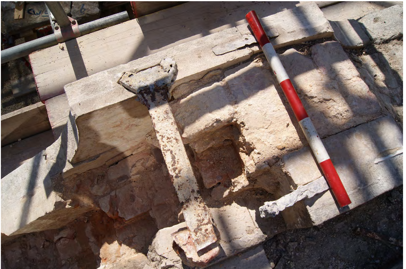
Plate A.58: Cast iron clamp on south side of west lower landing
