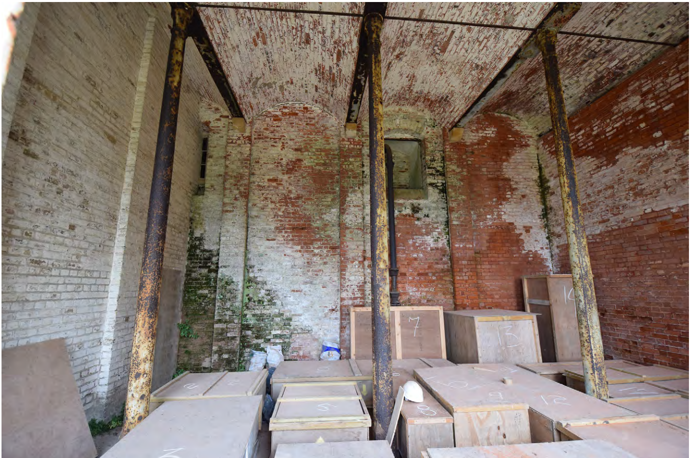
Plate C.27: Interior of East Fernery (north wall), looking north
