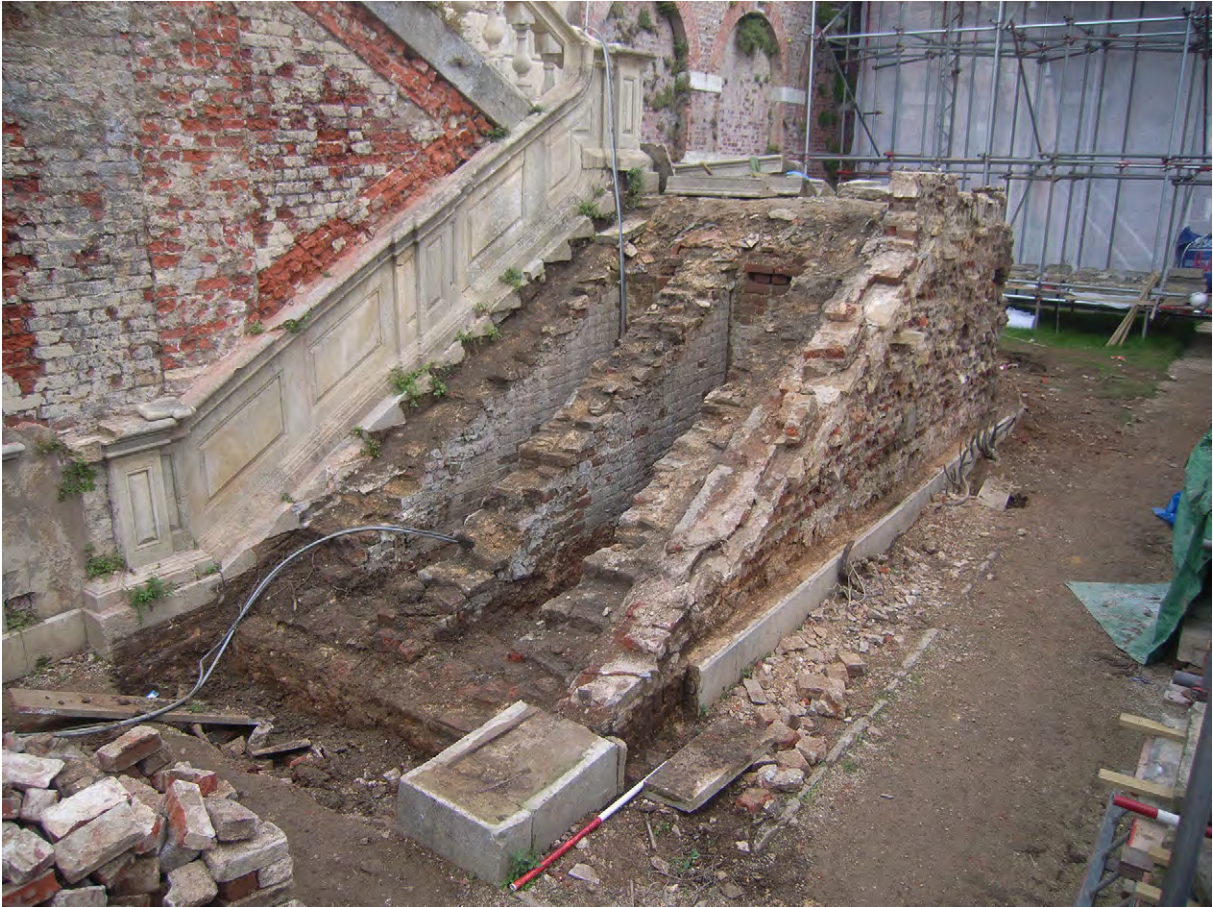
Plate A.57: Exposed eastern lower flight during works
