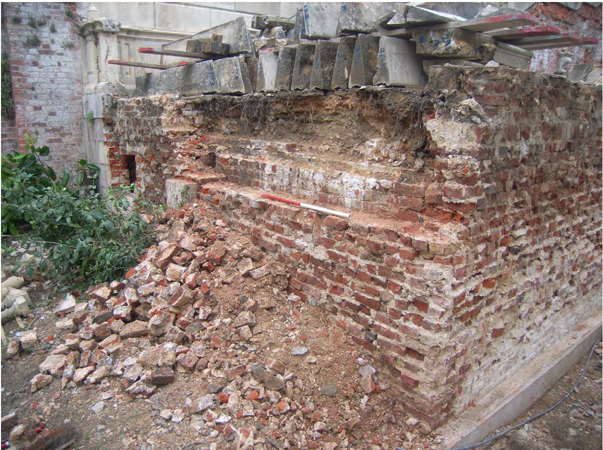
Plate A.30: West lower flight during dismantling [A.4.1 and A.4.2]
