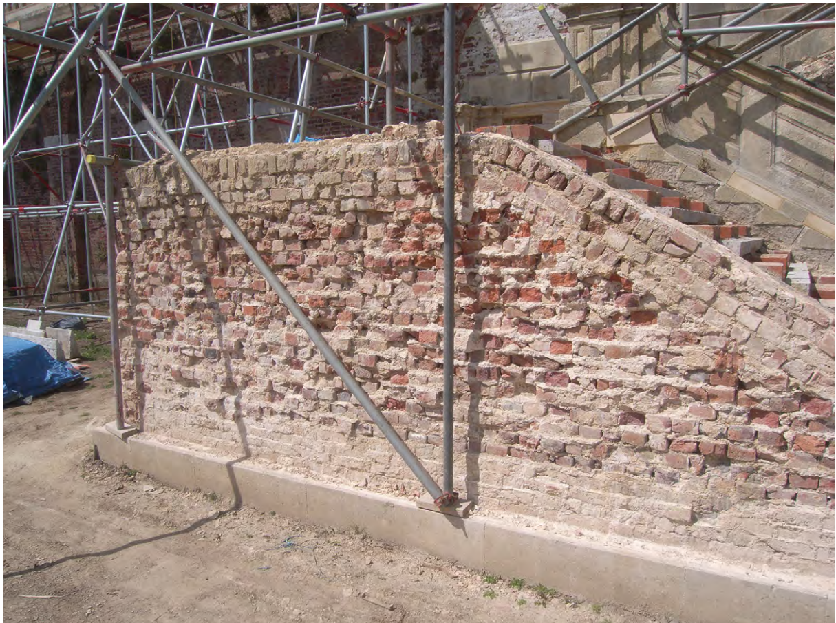
Plate A.24: West lower flight after removal of fine brick skin [A.4.1]
