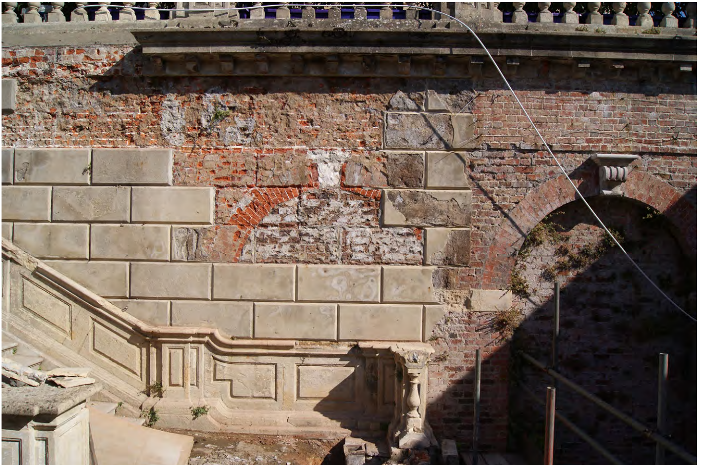
Plate B.10: Arch exposed behind rustication on east side
