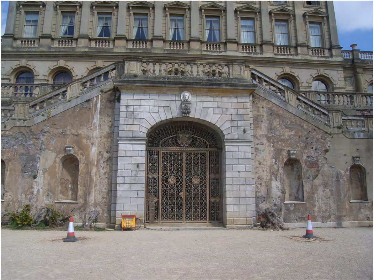
Plate A.1: Portico and staircase prior to works
