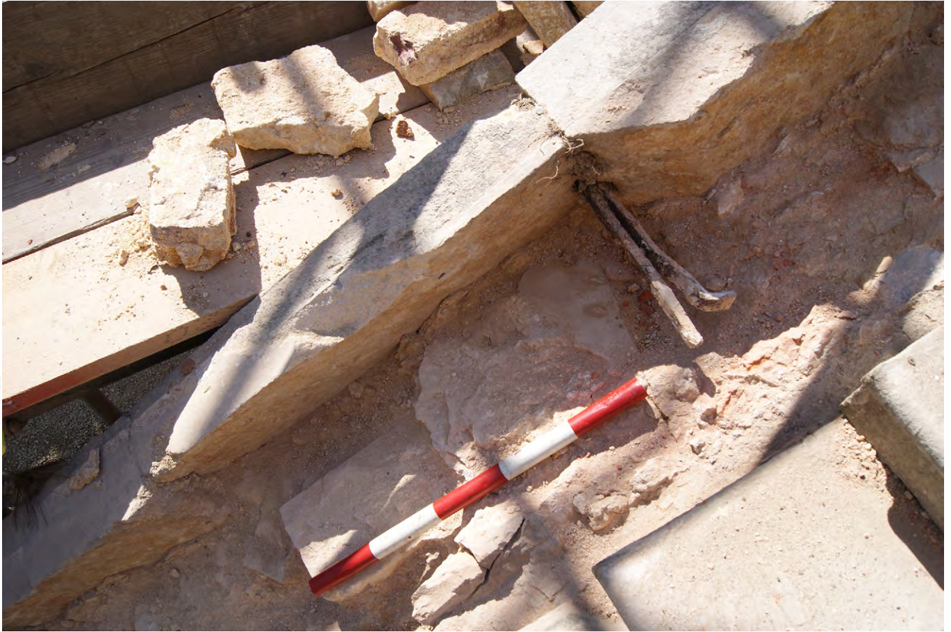
Plate A.59: Typical iron fixing in western lower flight
