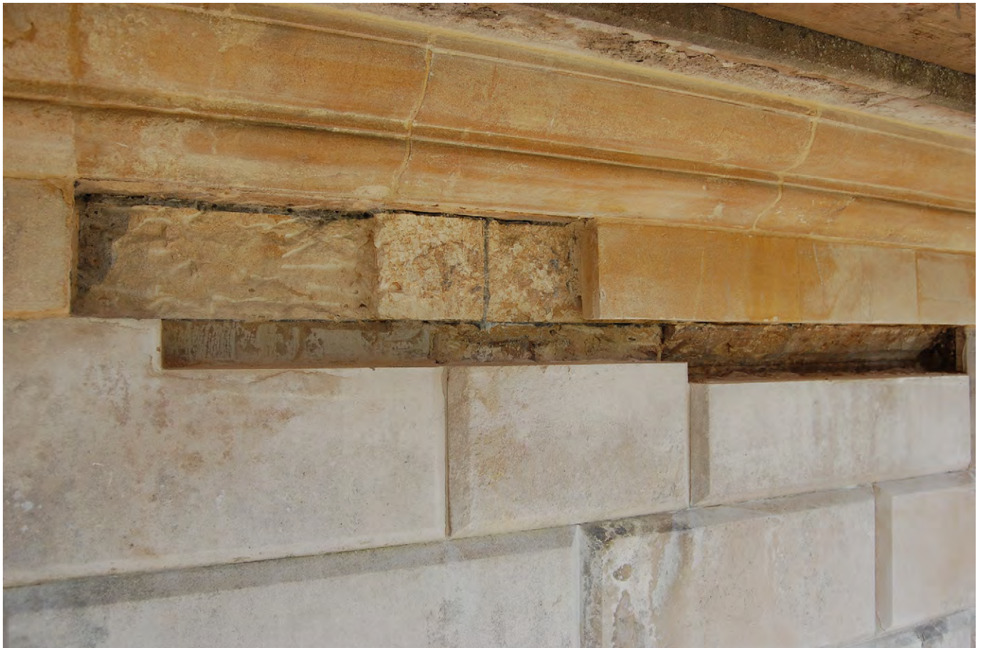
Plate A.62: Exposed fragment of older cornice behind Portico cladding [A.5.1]
