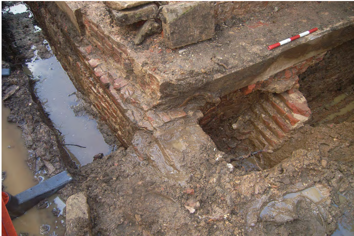
Plate A.54: Foundations beneath east side of stairs [A.3.3-A.3.5]
