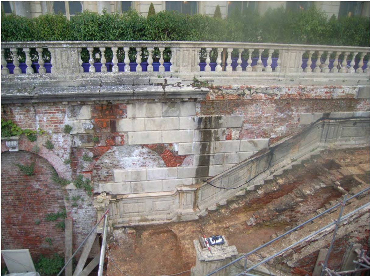
Plate B.14: General view of west side during removal of rustication
