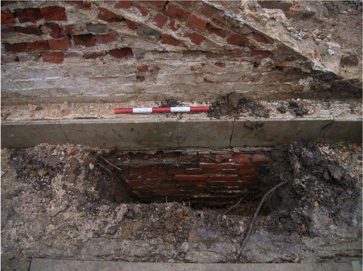
Plate A.29: Older foundations [A.4.3] beneath west flight of steps
