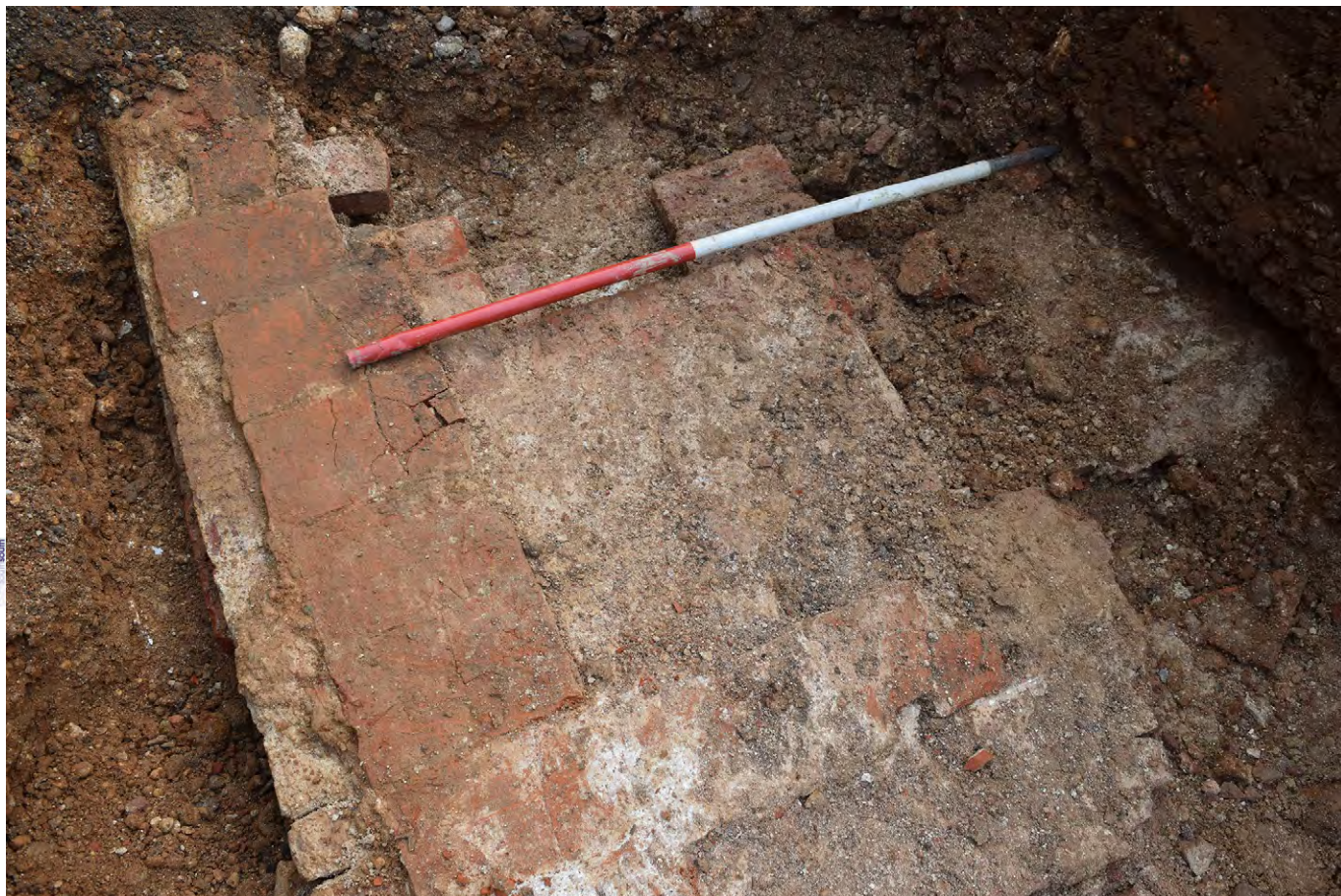
Plate G.32: Brick wall exposed in trial pit in front of west half of Blind Arcade [G.121.2], looking south-east
