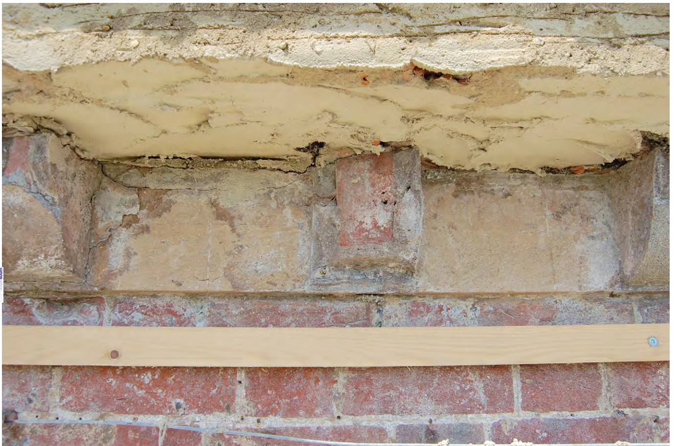
Plate B.17: Detail of cornice with ashlar grooves between brackets
