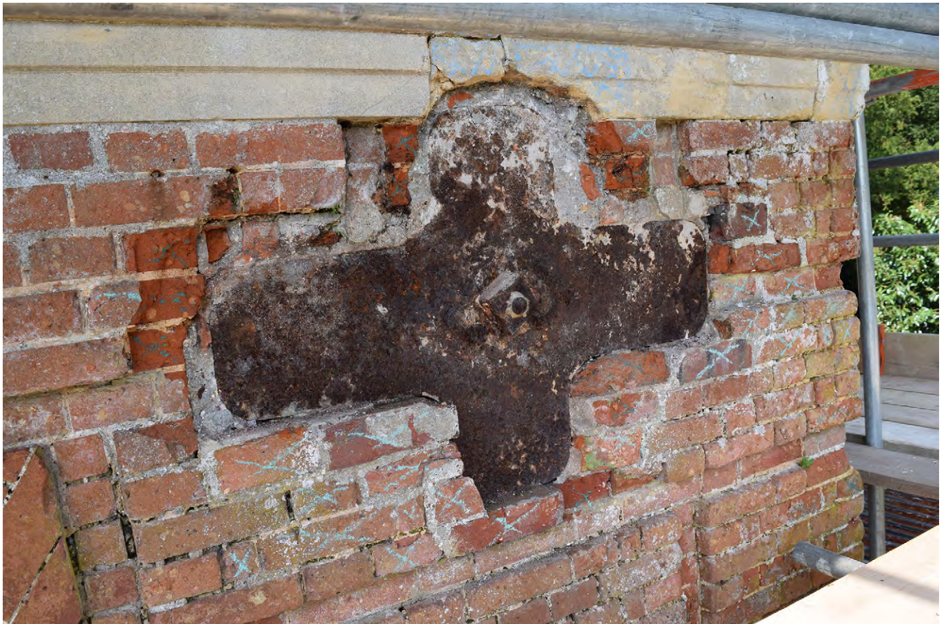
Plate C.25: Large iron tie-bar in south wall of East Fenery, looking north
