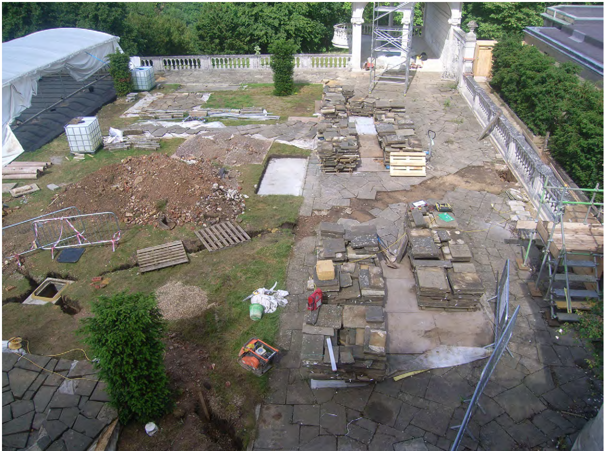
Plate I.2: General view of West Lawn during works, looking west
