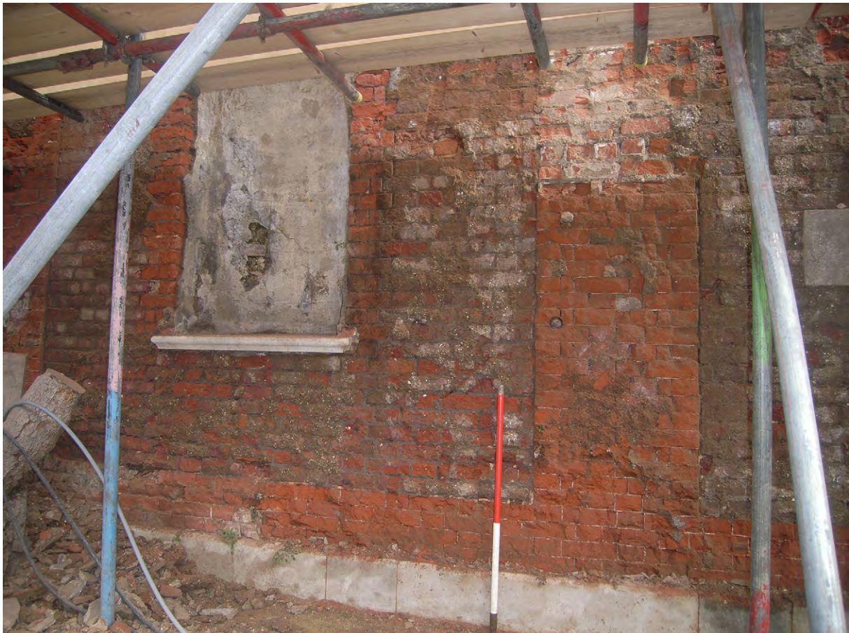
Plate A.46: Detail of fine brick on east side of stairs
