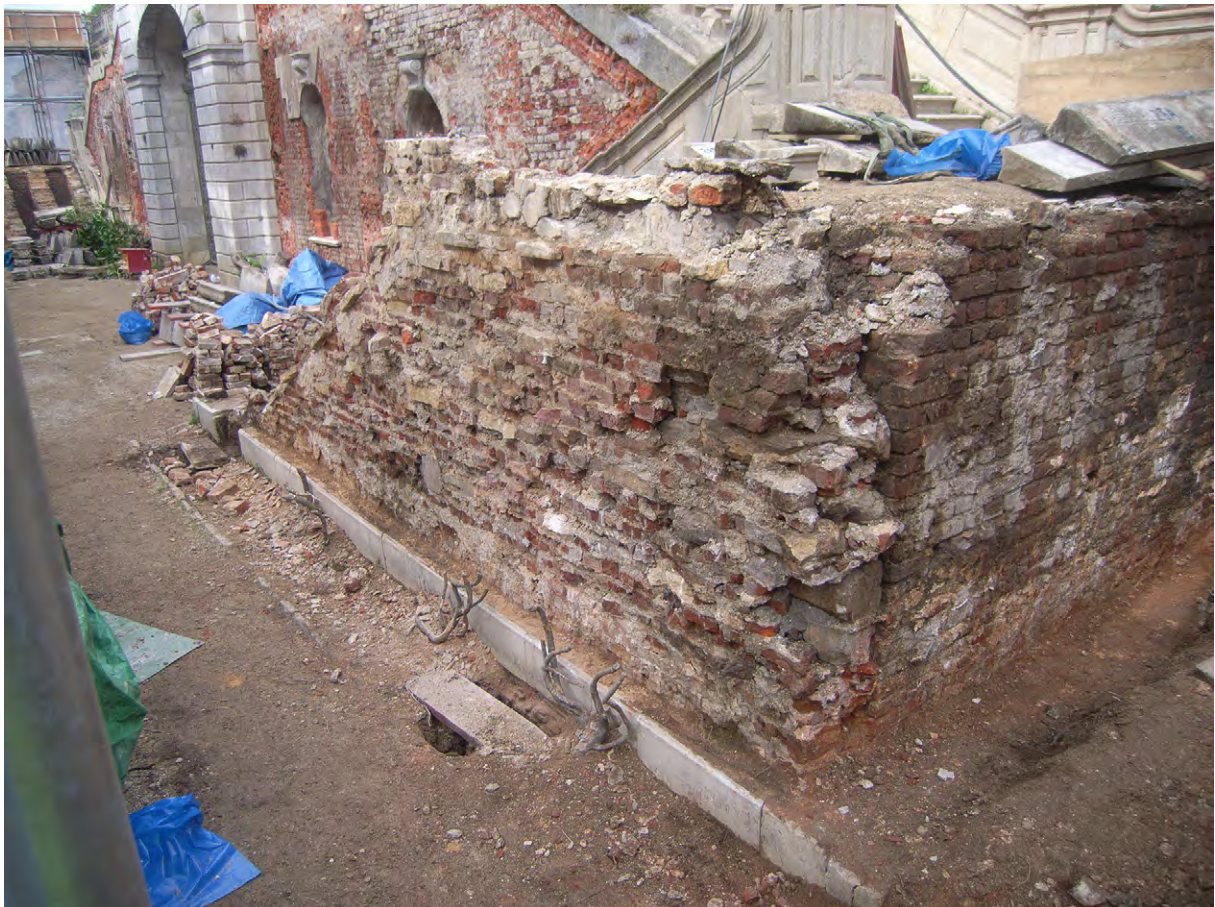
Plate A.50: Eastern stairs during dismantling [A.3.1 & A.3.2]
