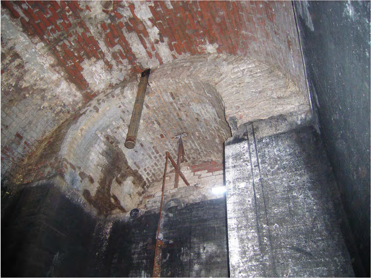
Plate E.7: Southern end of West Barrel Vaulted Chamber
