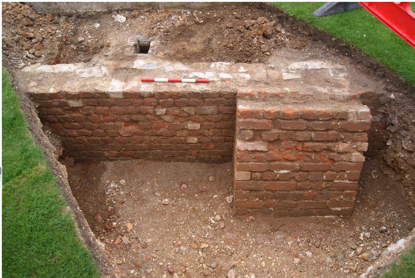
Plate F.10: Former north wall of terrace exposed in Pit F.101, looking south
