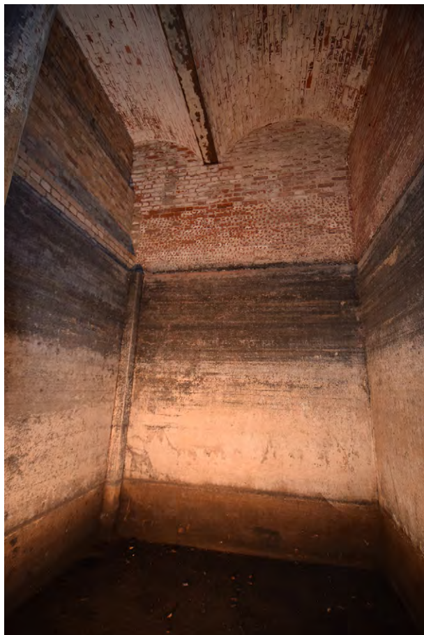
Plate C.42: West Fernery Water Tank looking south
