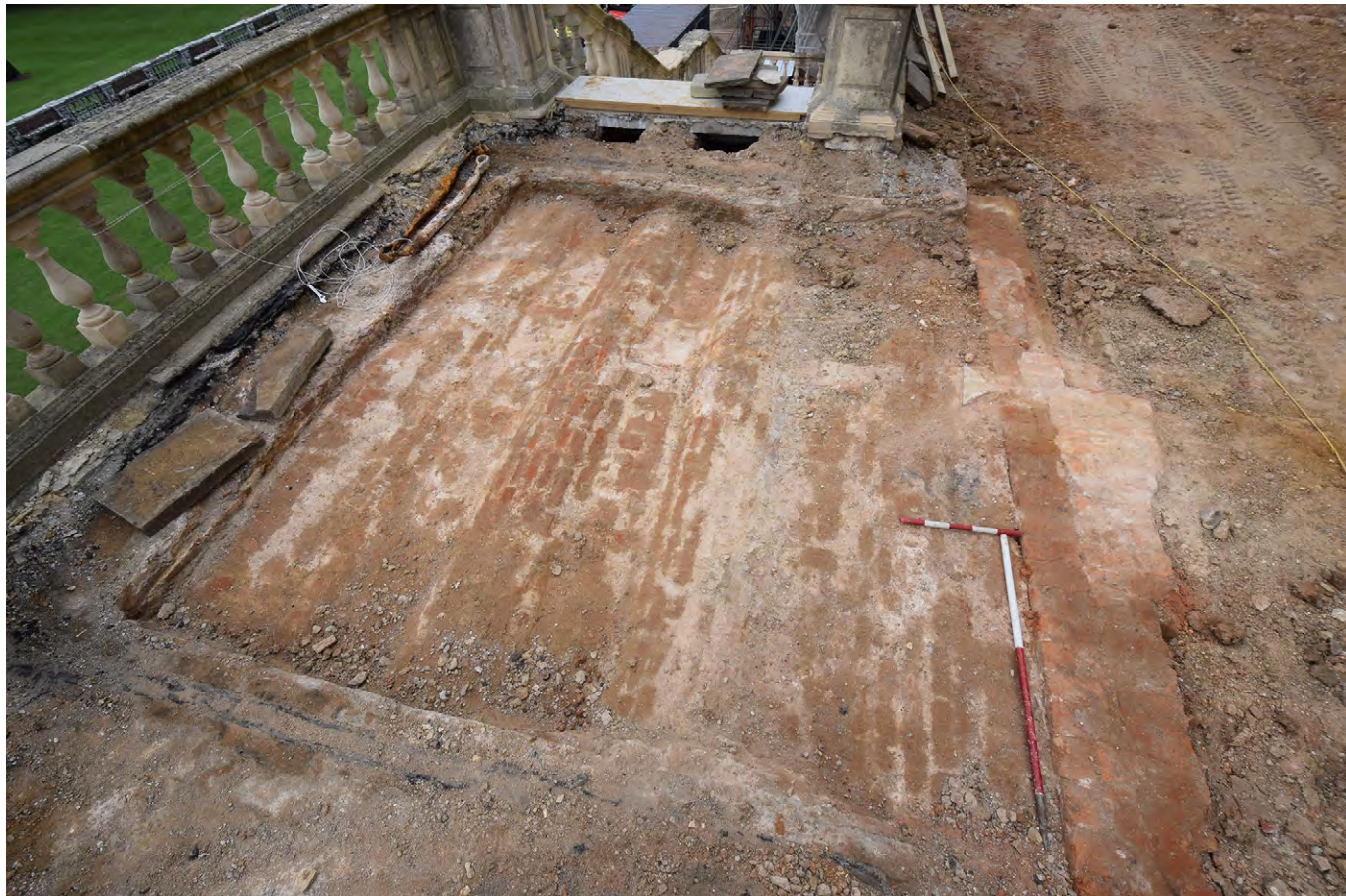
Plate F.36: Vaults over landing at top of staircase, looking west
