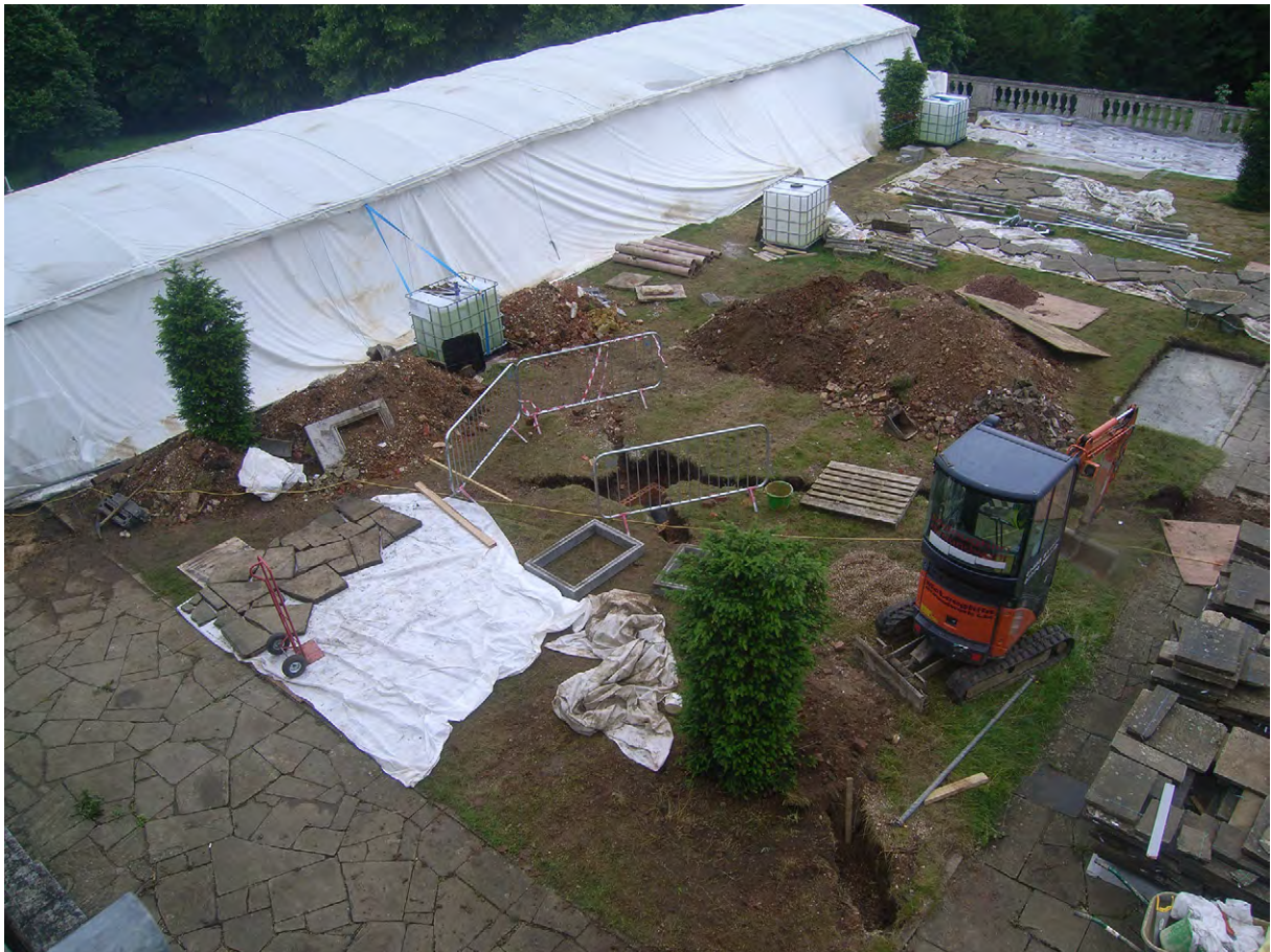
Plate I.1: General view of West Lawn during works, looking south-west
