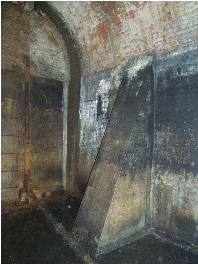
Plate E.8: Buttress in West Barrel Vaulted Chamber, looking north-east
