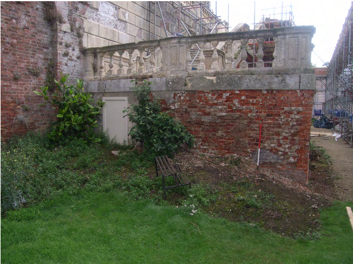
Plate A.22: West wall after removal of render
