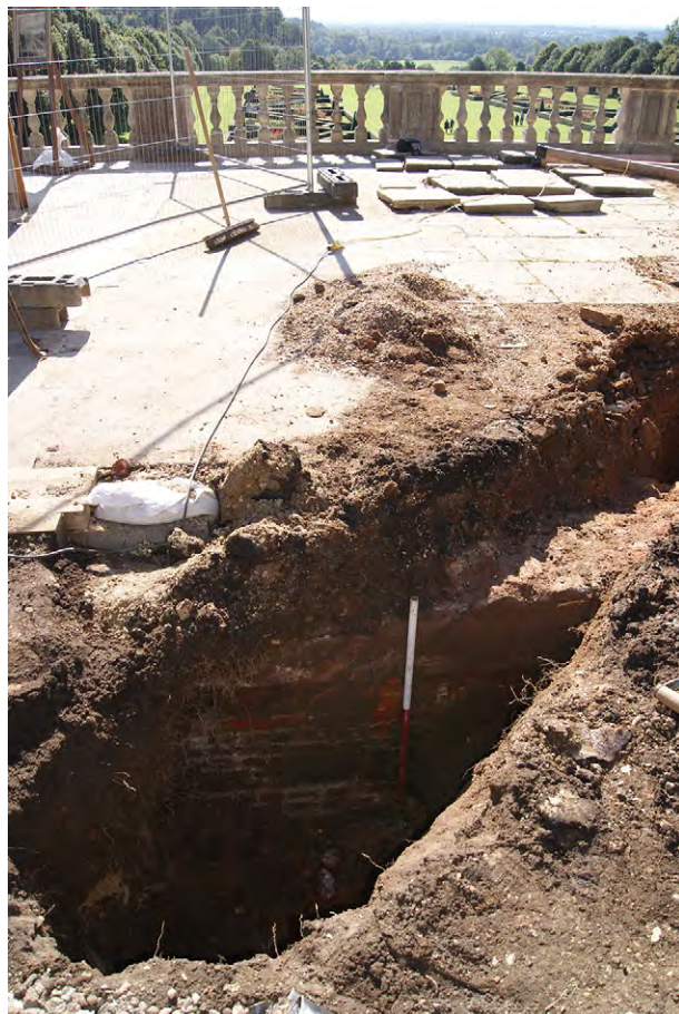
Plate F.62: Former north wall of terrace [F.106.1] exposed in pit just to SE of mansion, looking south
