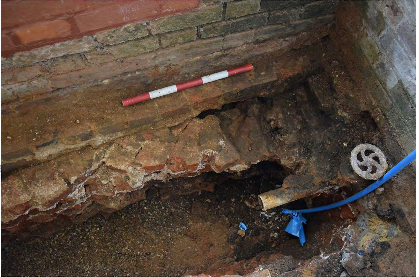
Plate C.34: Excavations at SW corner of East Fernery, looking south-west
