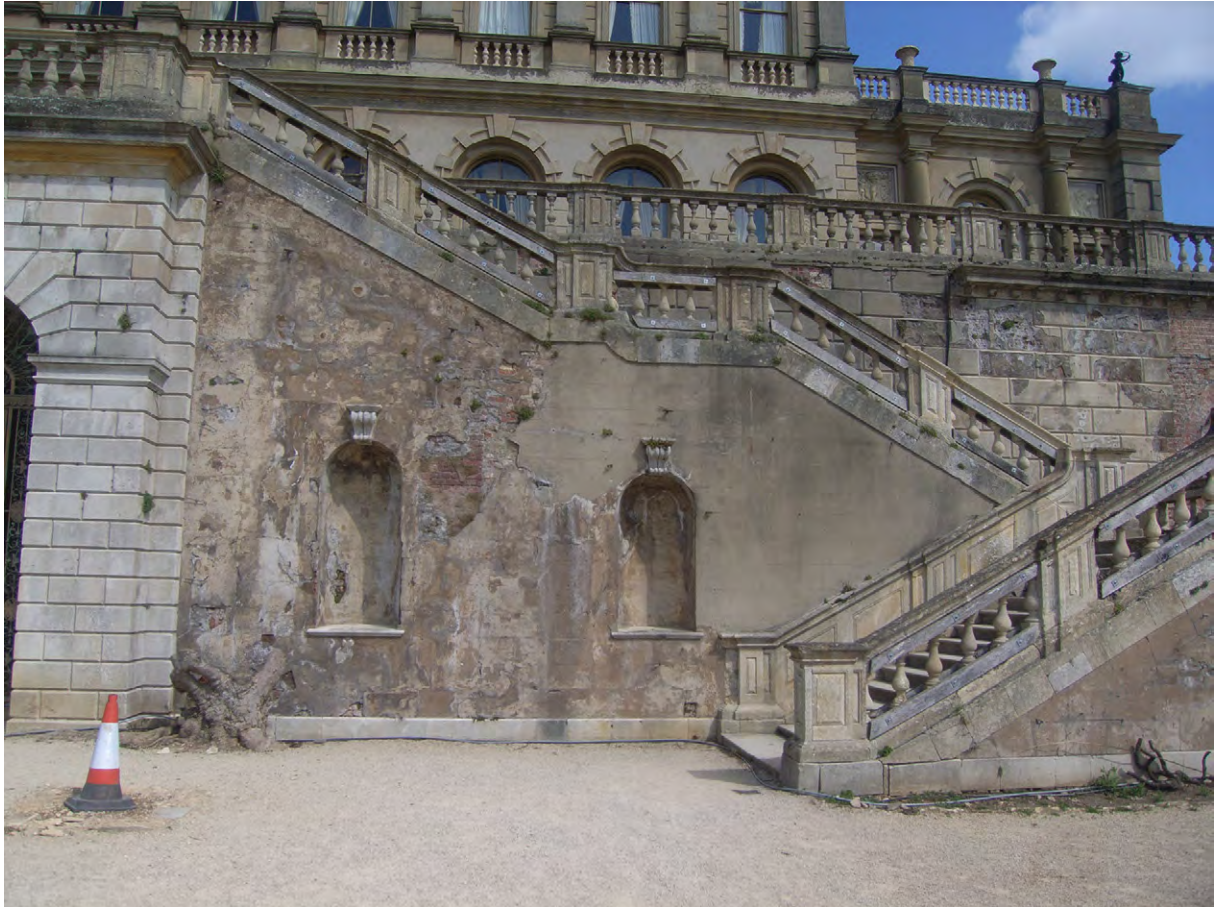
Plate A.9: East side of stairs prior to works
