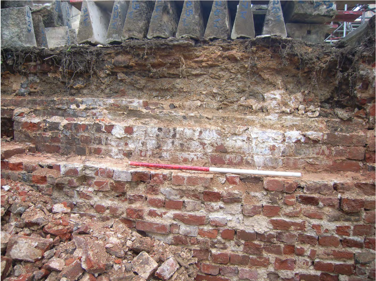
Plate A.31: Detail of west lower flight during dismantling [A.4.1 and A.4.2]
