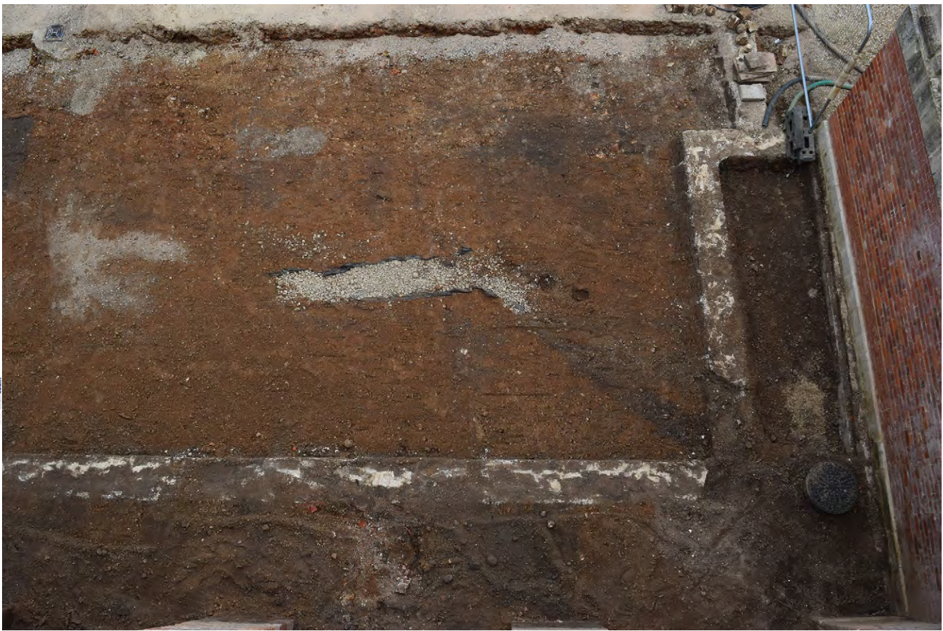
Plate G.28: Limecrete edging in front of east side of Blind Arcade [G.119.4], looking down from terrace
