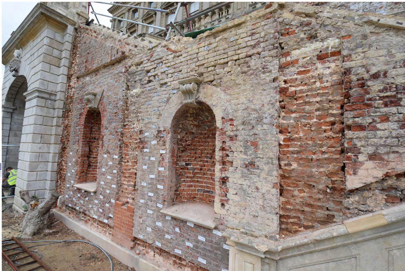
Plate A.43: Exposed east face of stairs
