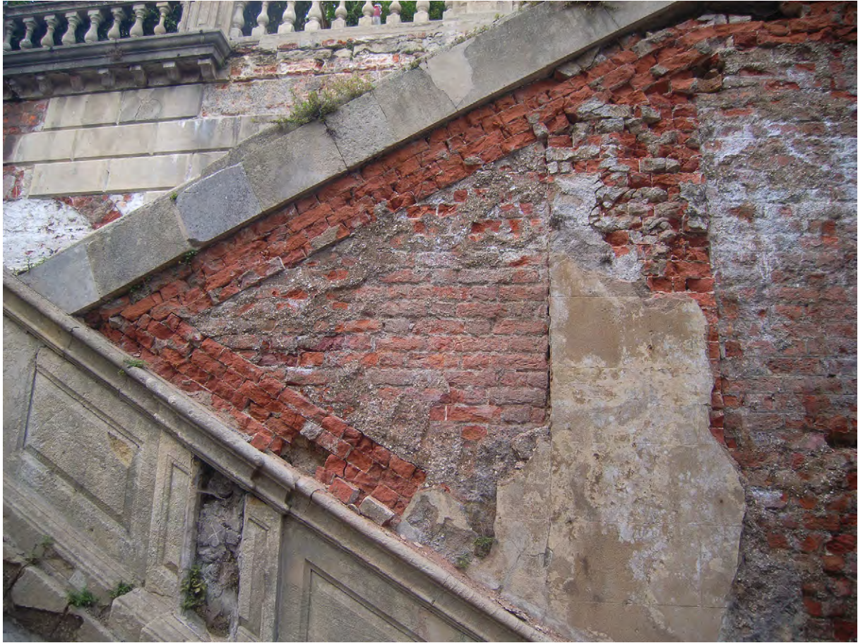
Plate A.17: Fine brickwork on west side after removal of render
