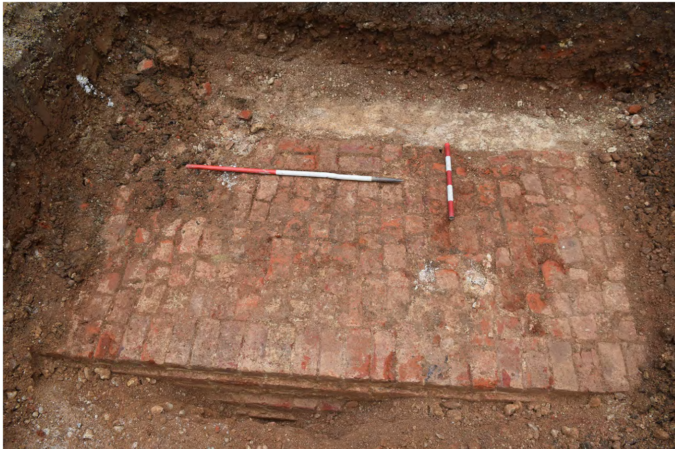
Plate G.33: Brick wall exposed in trial pit in front of west half of Blind Arcade [G.122.1], looking north
