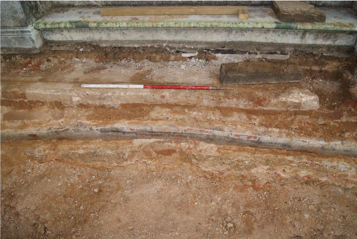
Plate F.51: Drains in front of mansion after removal of brick capping, looking north
