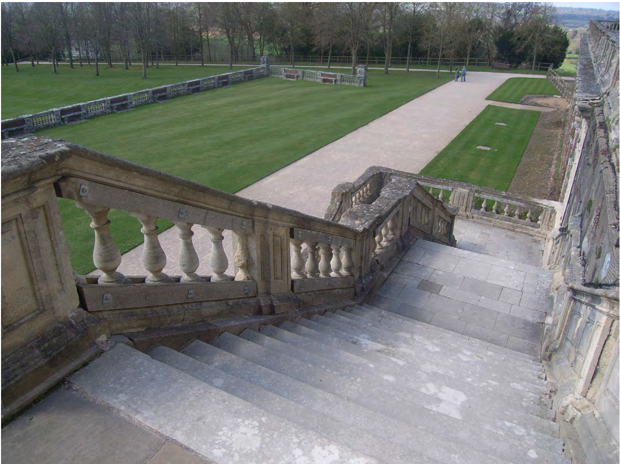
Plate A.6: Western stairs
