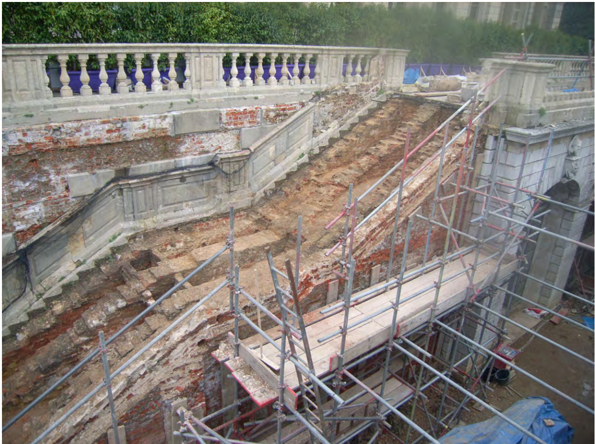
Plate A.38: West side of stairs during works
