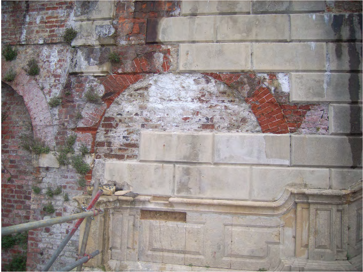
Plate B.11: Arch exposed behind rustication on west side
