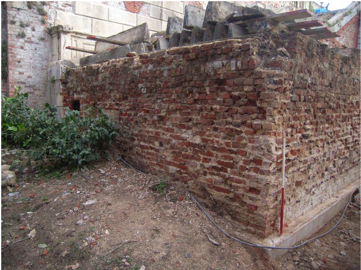
Plate A.23: West wall after removal of fine brick skin [A.4.1]
