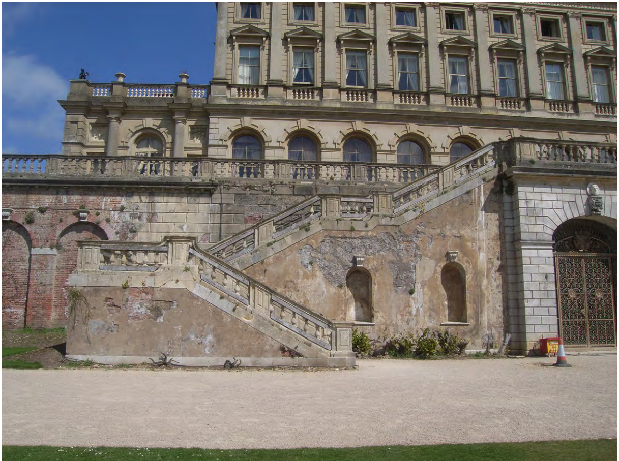
Plate A.2: West side of stairs prior to works
