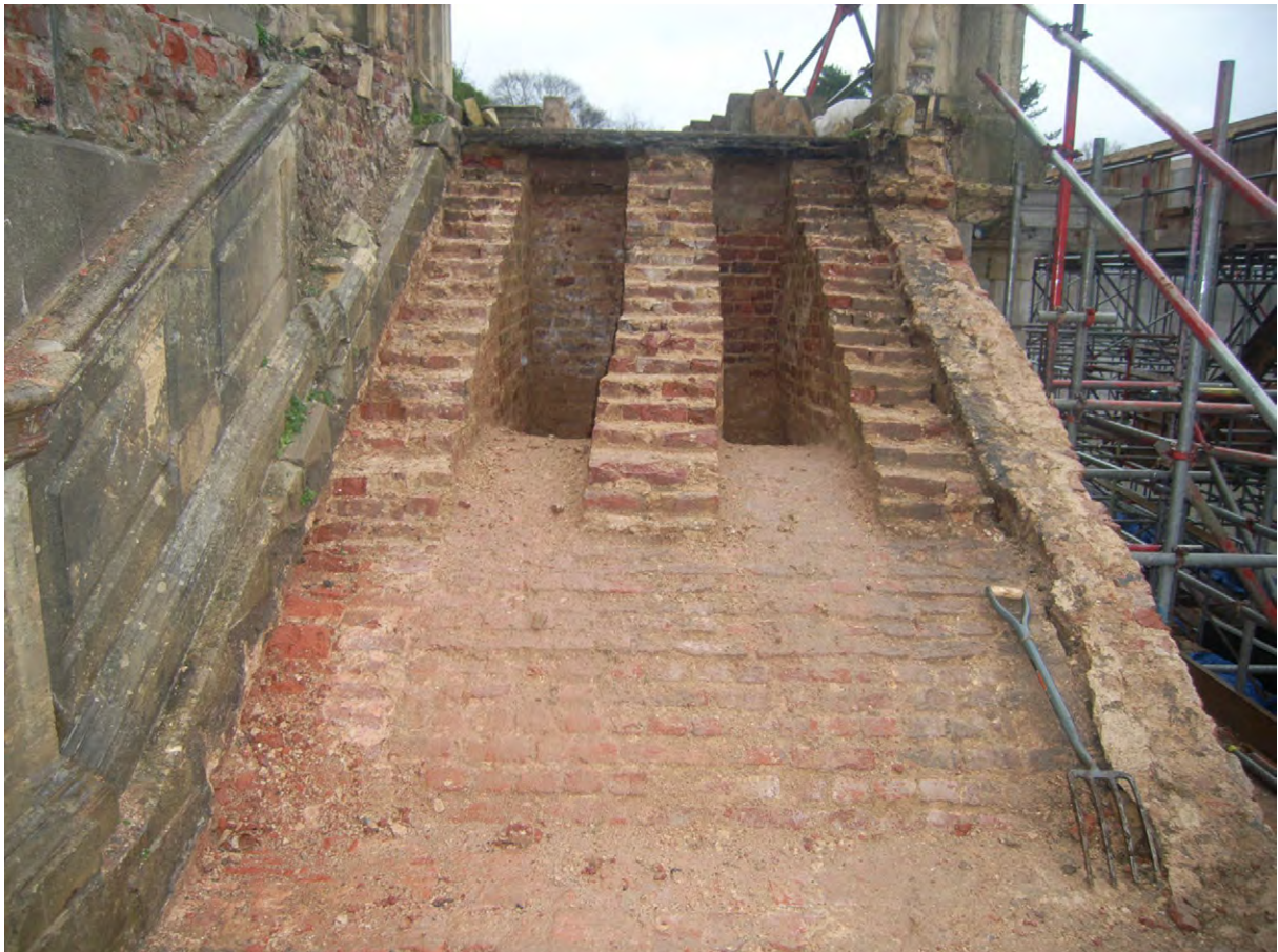
Plate A.36: Upper part of west side of stairs during works
