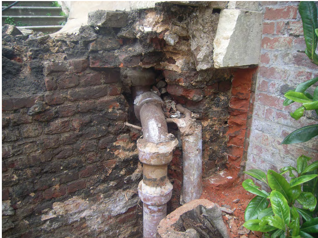
Plate A.52: North wall of east side of stairs with blackened core [A.3.1, A.3.2] and pristine face [A.2.1]
