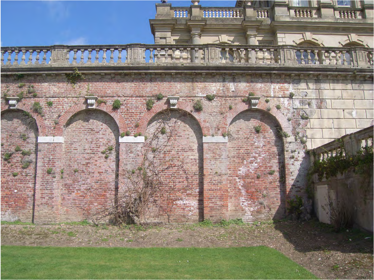
Plate B.1: Blind arcade immediately west of staircase
