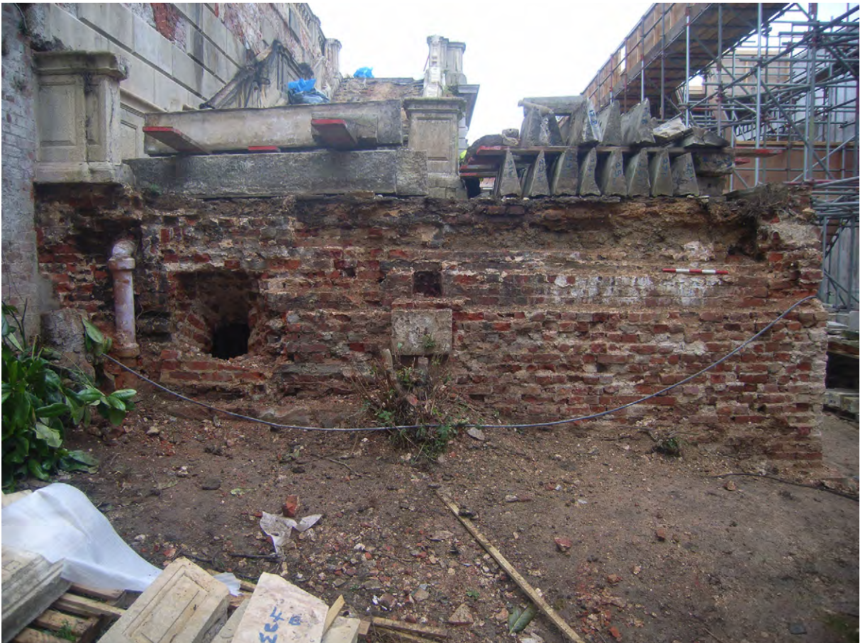
Plate A.26: Exposed core of west wall [A.4.1 and A.4.2]
