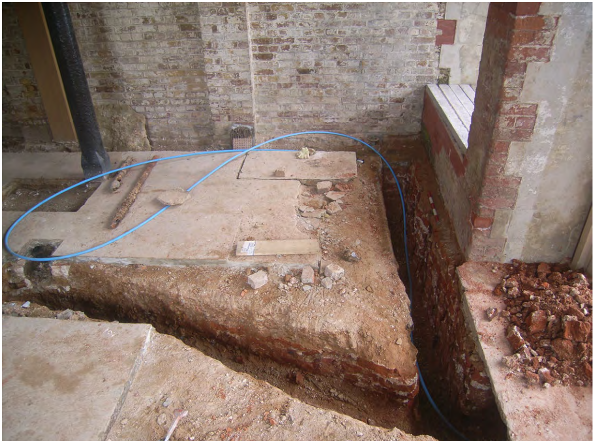
Plate C.21: Excavations in West Fernery with exposed wall [C.1.8], looking east
