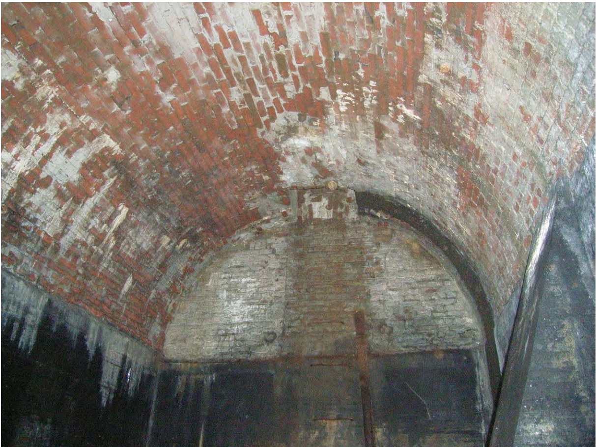
Plate E.6: Looking north in West Barrel Vaulted Chamber
