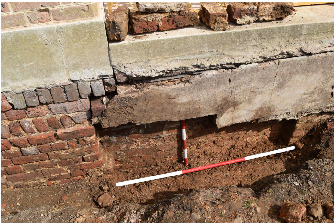
Plate C.51: Lower part of south wall of East Fernery
