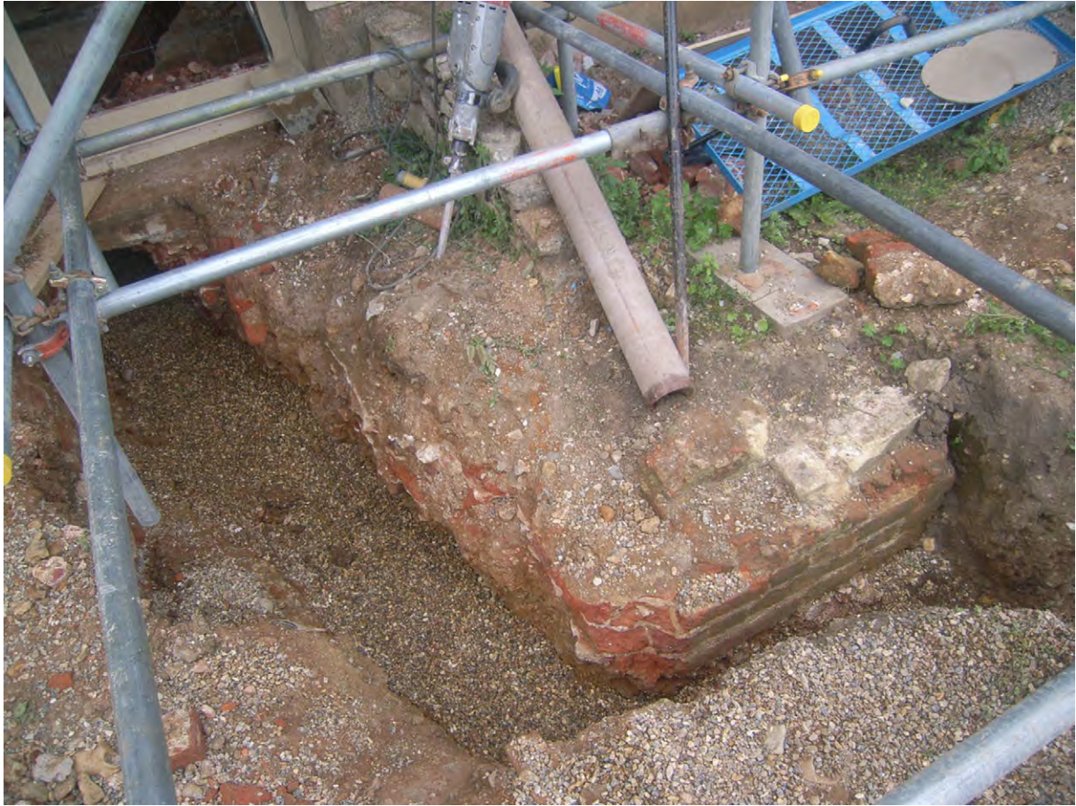
Plate C.5: Exposed footings in front of West Fernery [G.117.1], looking north-east
