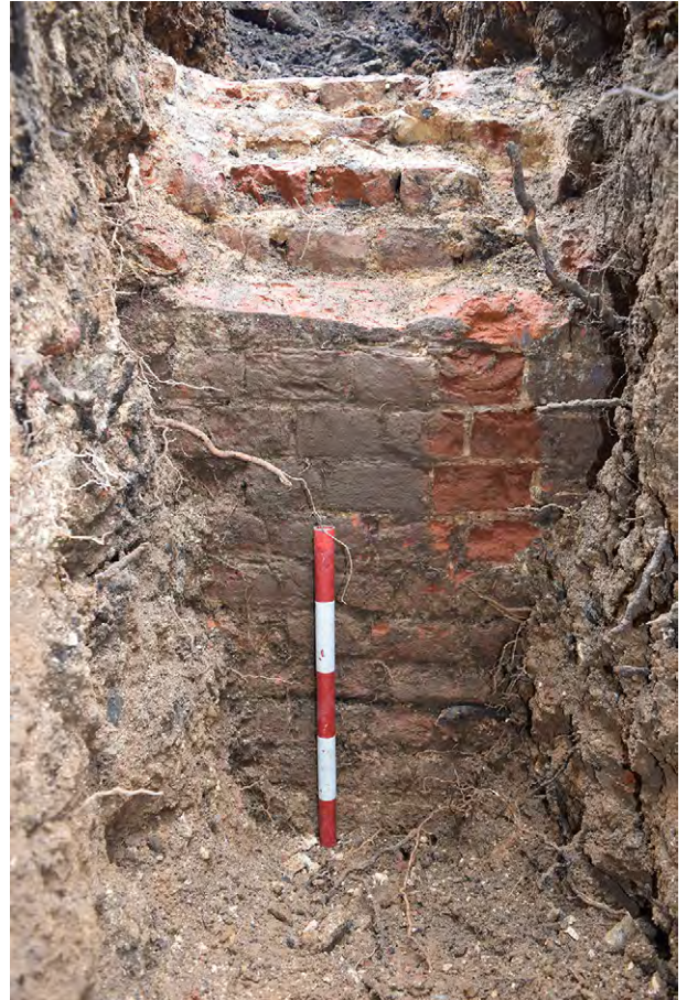
Plate J.2: Wall [J.102.1] exposed at top of bank to east of Duke's Lawn, looking west
