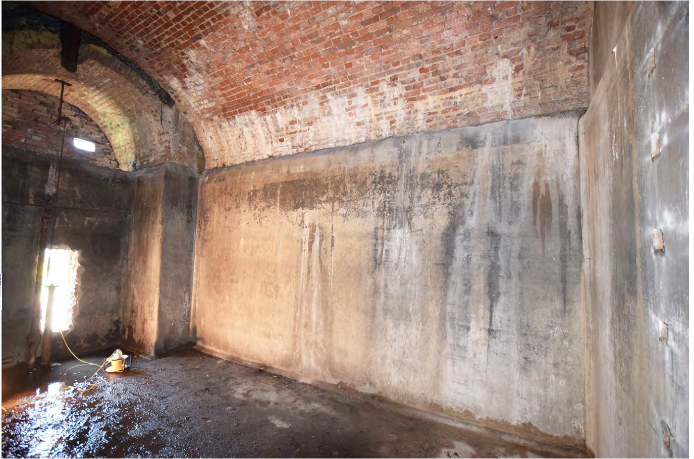
Plate E.14: Interior of East Barrel Vaulted Chamber looking south-west
