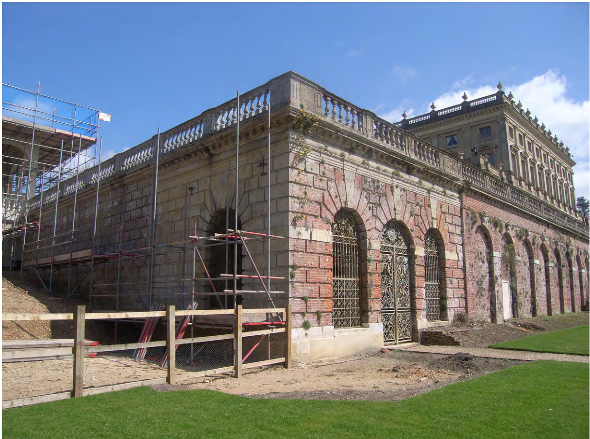
Plate C.2: West Fernery from south-west
