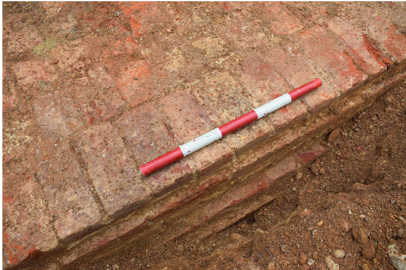
Plate G.35: Detail of wall in trial pit [G. 122. 1], looking north-east
