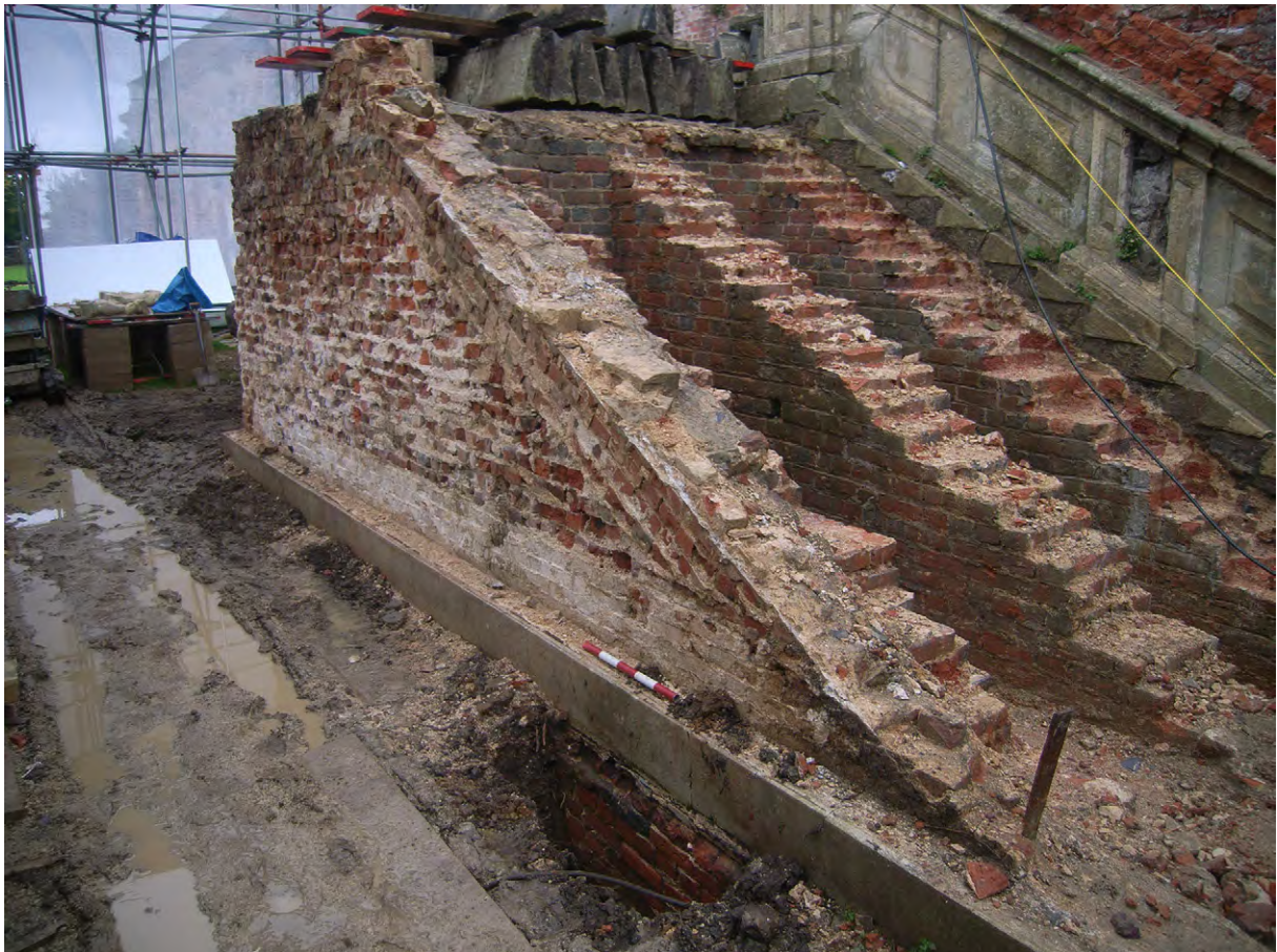
Plate A.28: Lower flight after removal of steps
