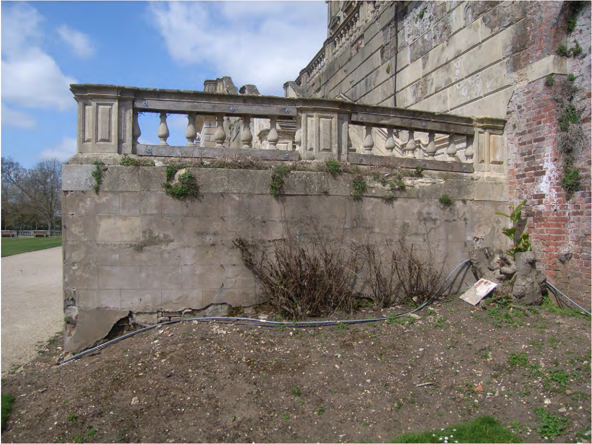
Plate A.13: East return wall of stairs
