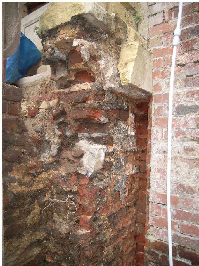
Plate A.51: Junction between east side of stairs and blind arcade
