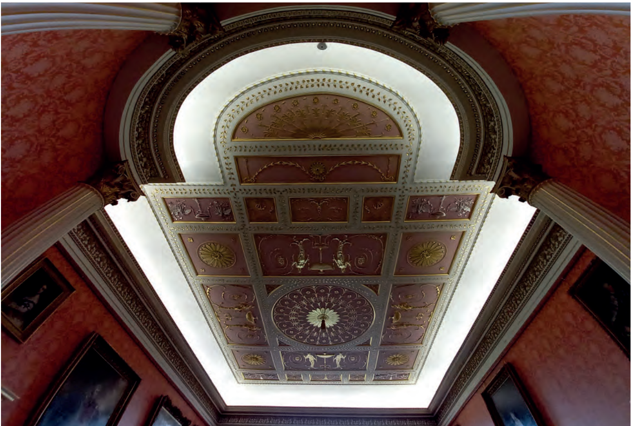
Plate 18: Temple Room, ceiling, following the conservation work
