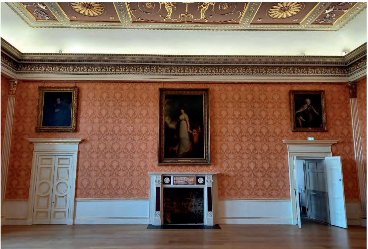
Plate 8: Temple Room, west wall, following the conservation work
