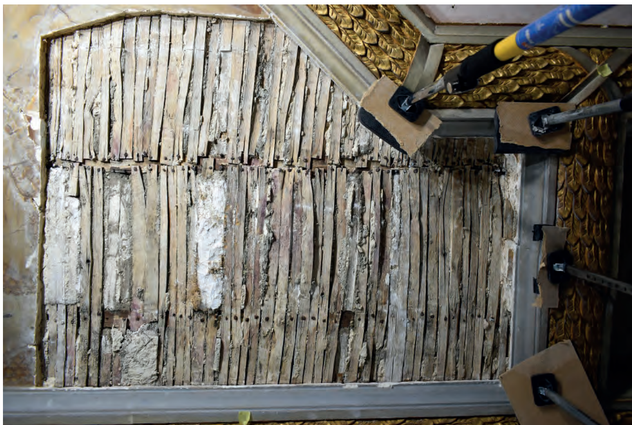
Plate 120: Dining Room, ceiling, during repair to the west end
