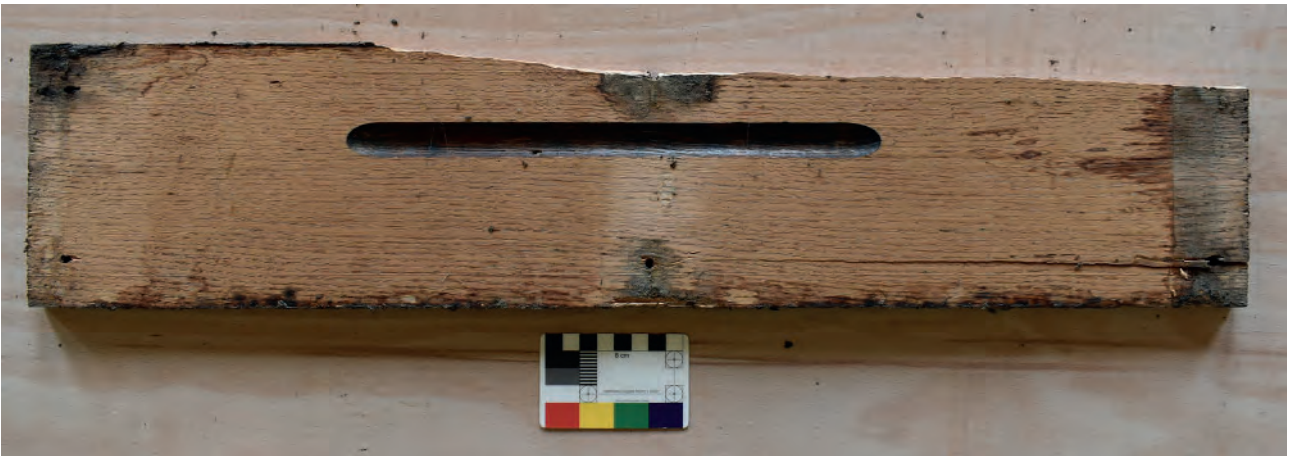
Plate 146: Dining Room, floor, example of furniture used to patch the floorboards
