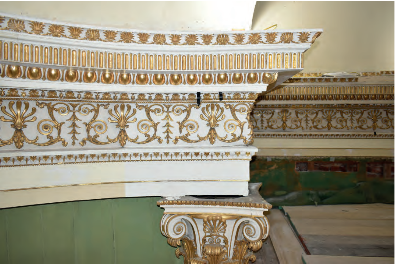
Plate 15: Temple Room, cornice, example of cleaning
