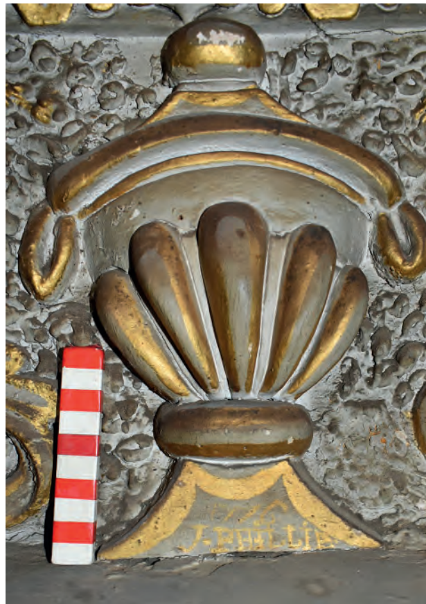
Plate 128: Dining Room, ceiling, example of graffiti
