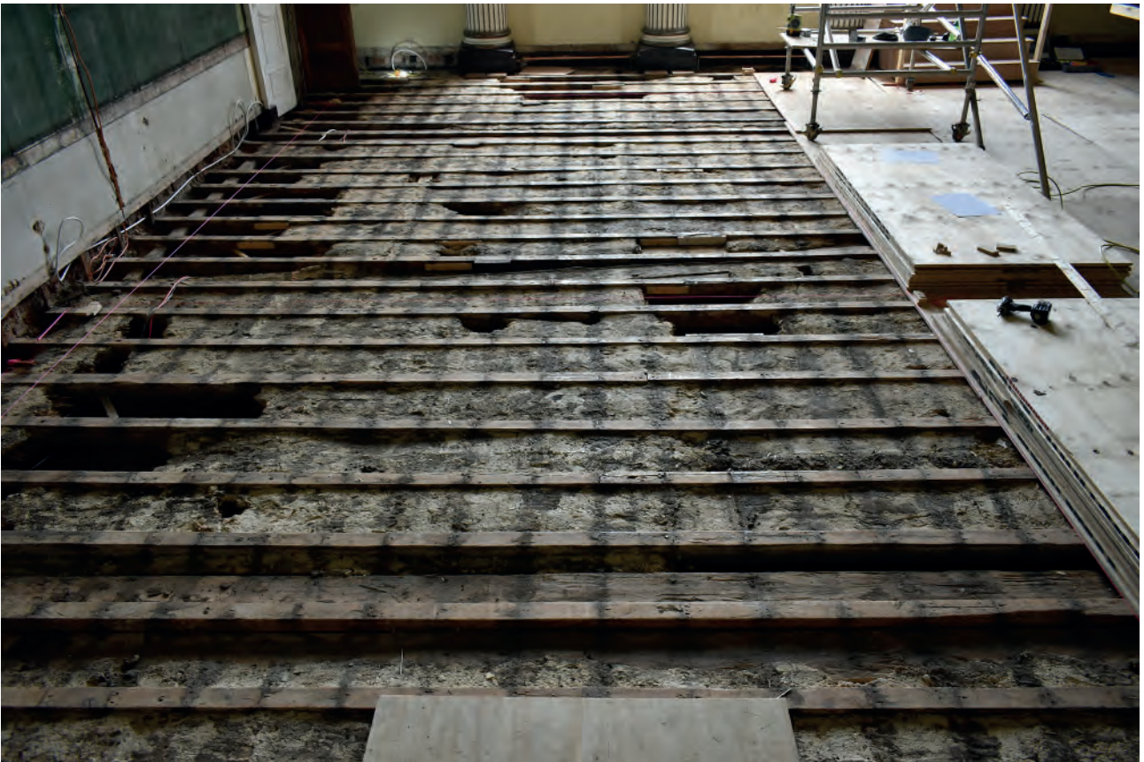
Plate 74: Temple Room, floor, east end, following stripping of floorboards
