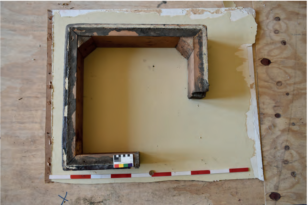
Plate 53: Temple Room, north wall, example of pilaster base construction
