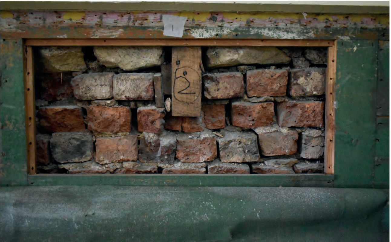
Plate 32: Temple Room, west wall, exposed brickwork
