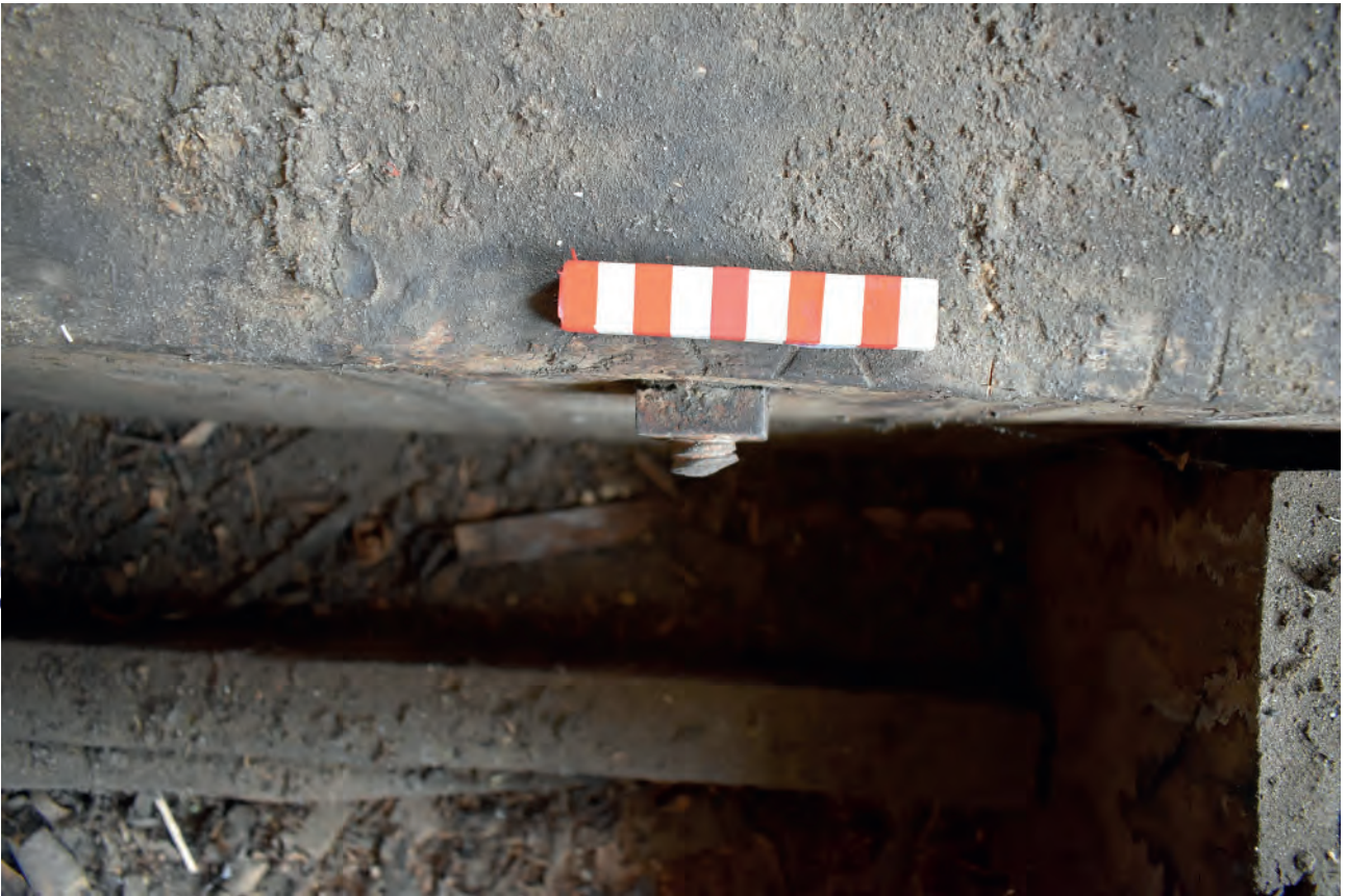
Plate 157: Dining Room, floor, example of ironwork
