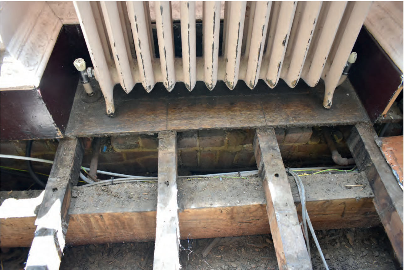
Plate 138: Dining Room, wall, example of relieving arch beneath windows
