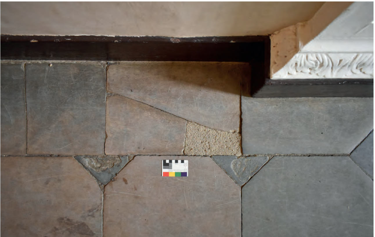
Plate 180: West Corridor, floor, example of concrete repair
