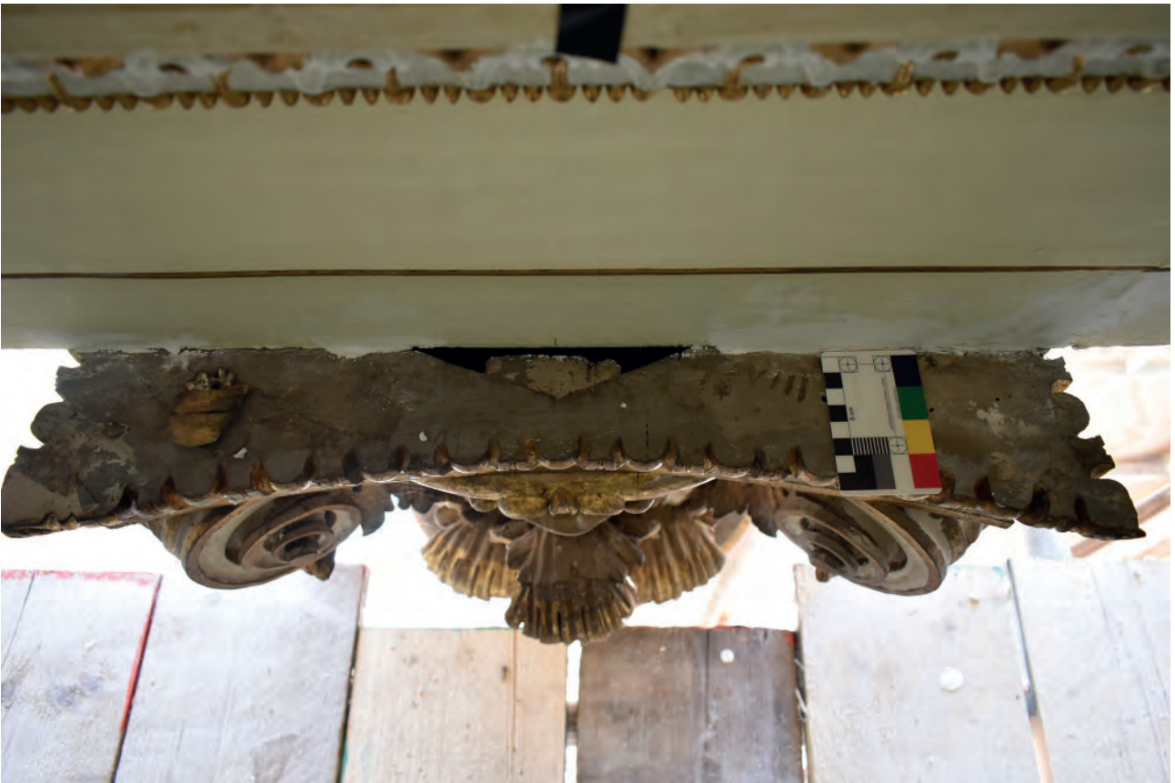
Plate 52: Temple Room, south wall, example of numbered pilaster
