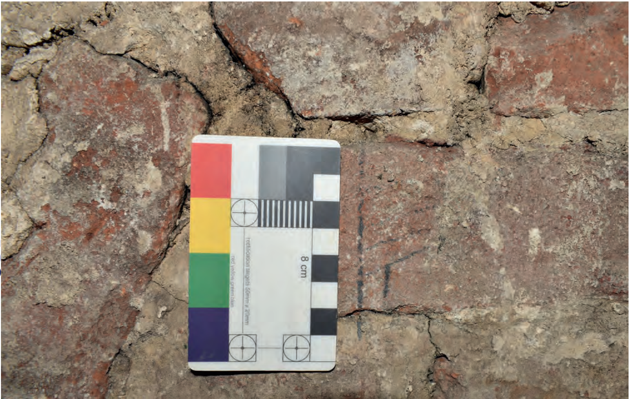
Plate 59: Temple Room, 1922 fireplace construction marks
