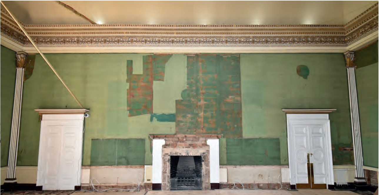
Plate 21: Temple Room, west wall, following stripping
