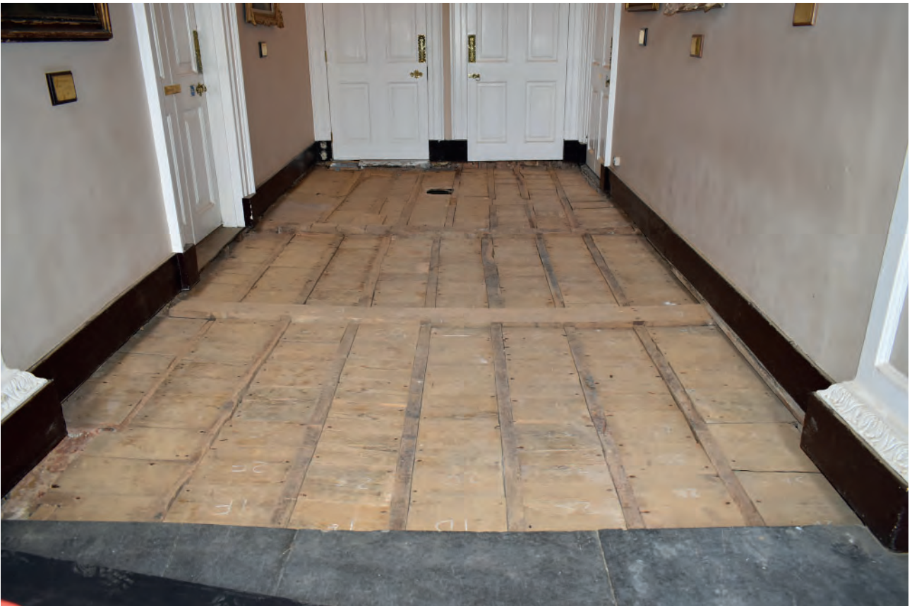
Plate 186: West Corridor, floor, exposed pugging boards, looking east
