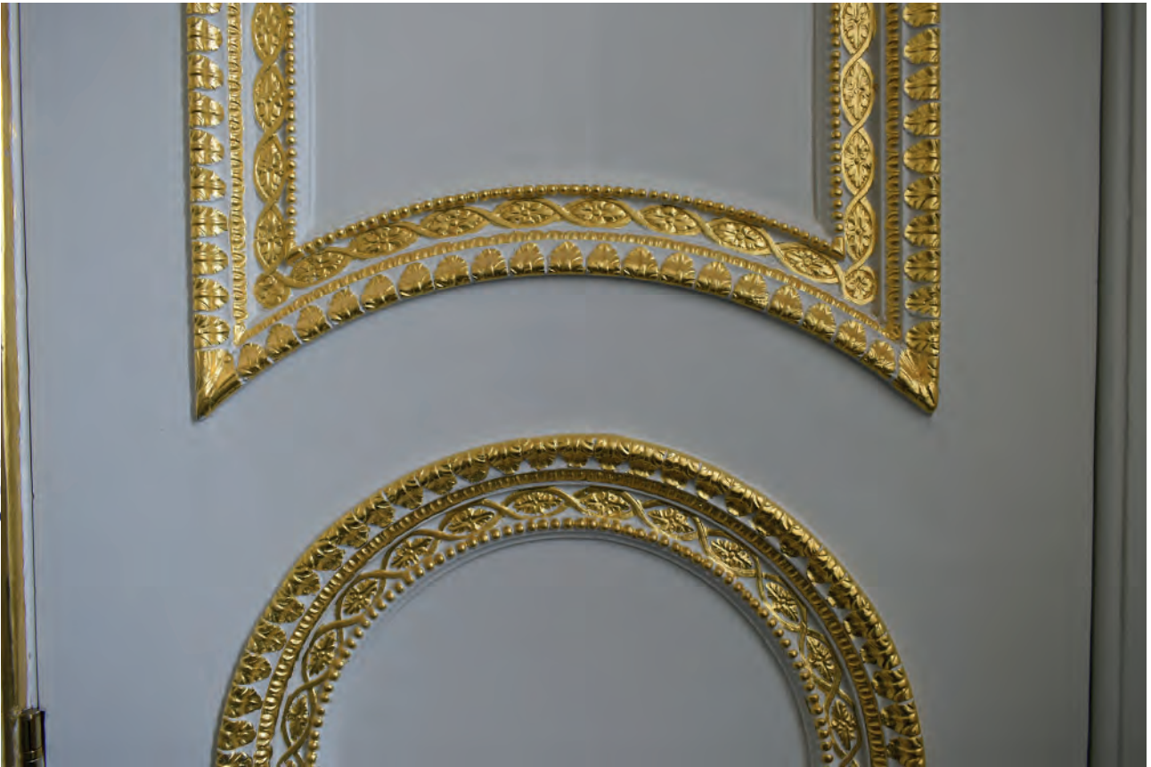
Plate 47: Temple Room, example of regilded moulding
