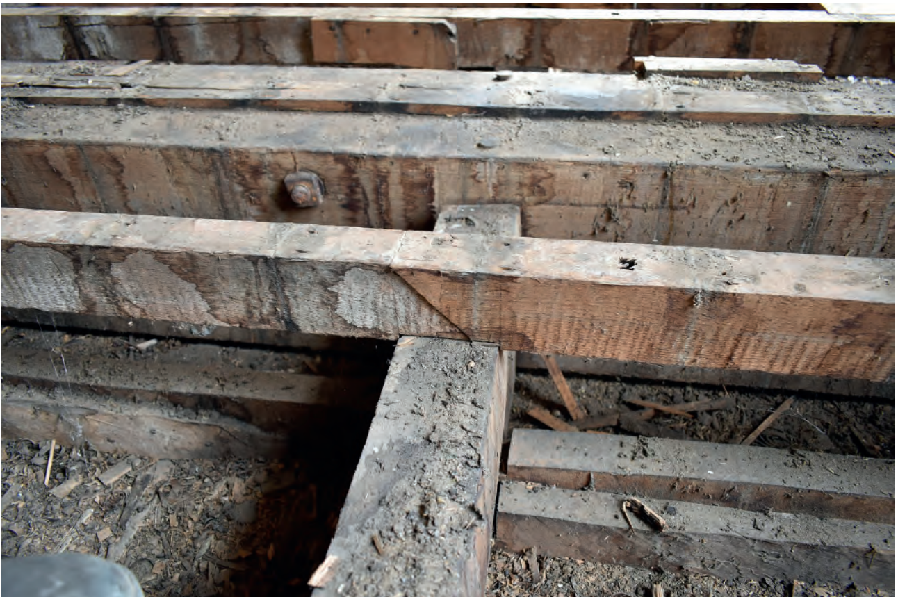
Plate 162: Dining Room, floor, example of jointed joists
