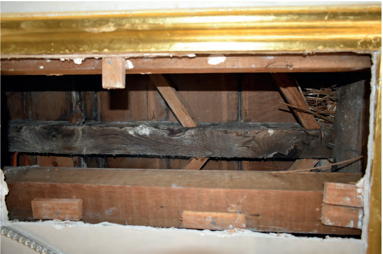
Plate 12: Temple Room, ceiling, 1965 panel towards the south east
