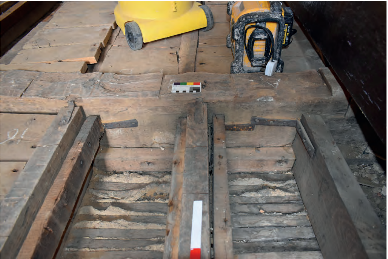
Plate 189: West Corridor, floor, detail of the altered easternmost beam
