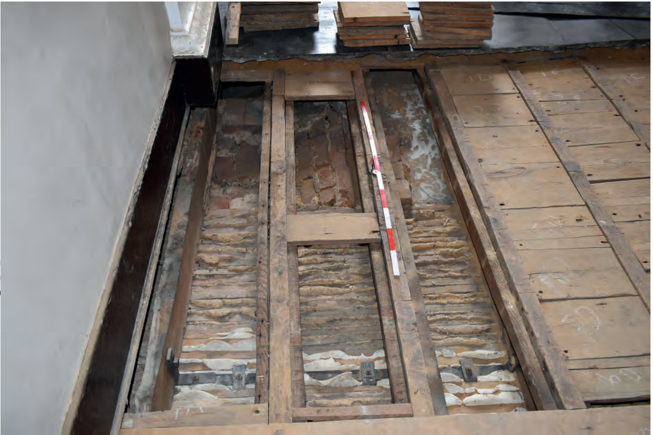
Plate 193: West Corridor, floor, brick vault beneath floor, looking west
