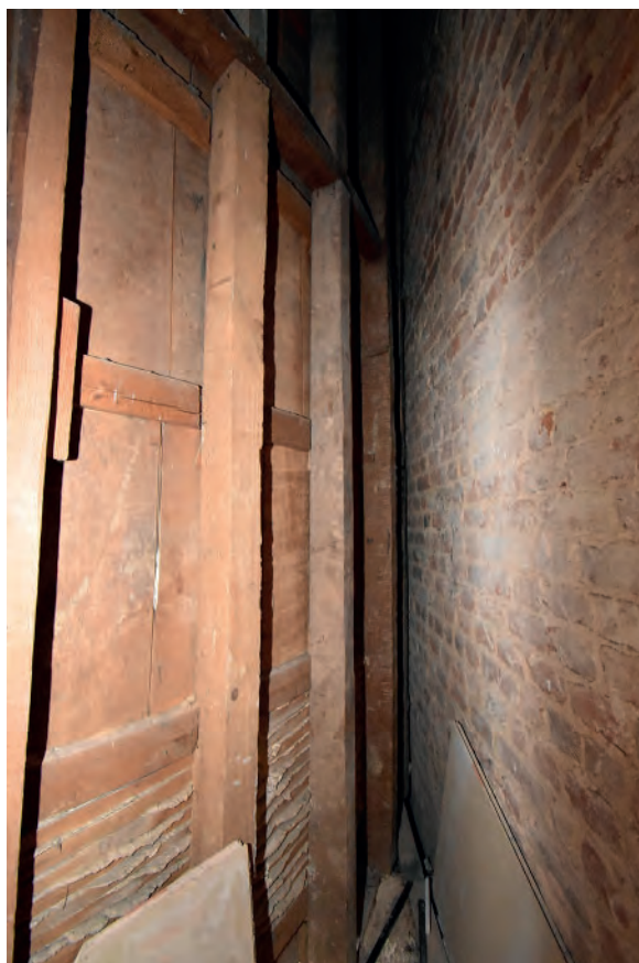
Plate 85: Void behind Temple Room apse, structure of apse
