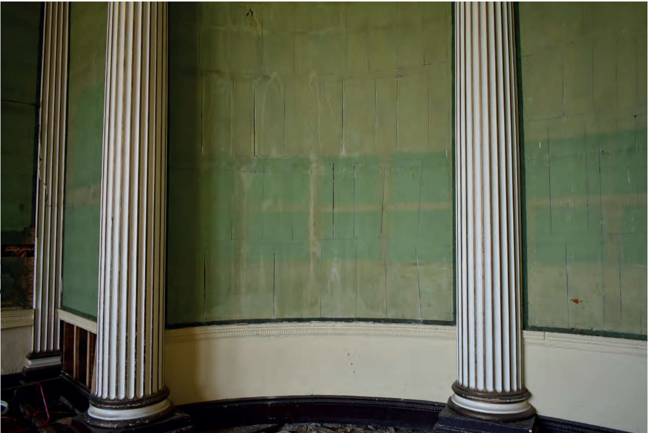
Plate 29: Temple Room, wall, example of light green paint fading around pictures
