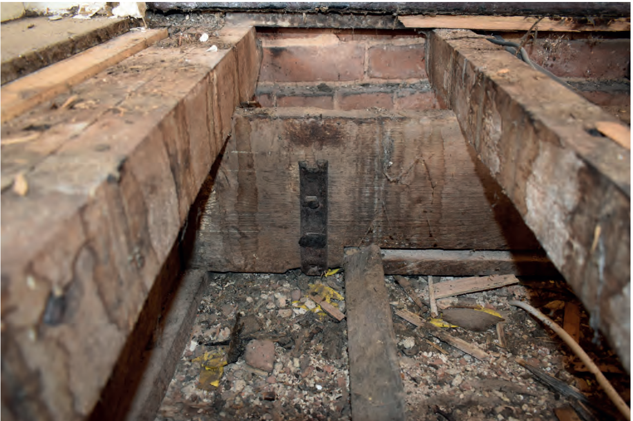
Plate 160: Dining Room, floor, example of ironwork
