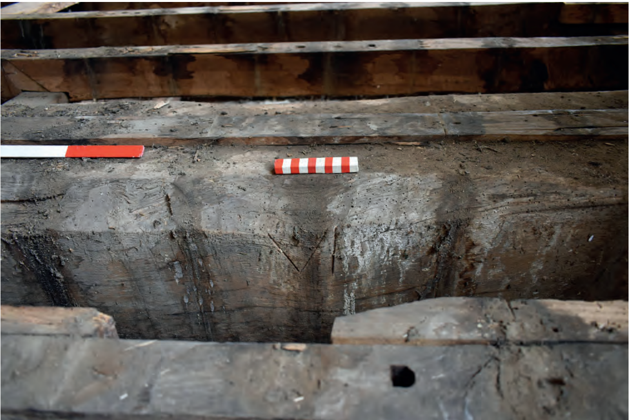
Plate 170: Dining Room, floor, example of carpenter's marks
