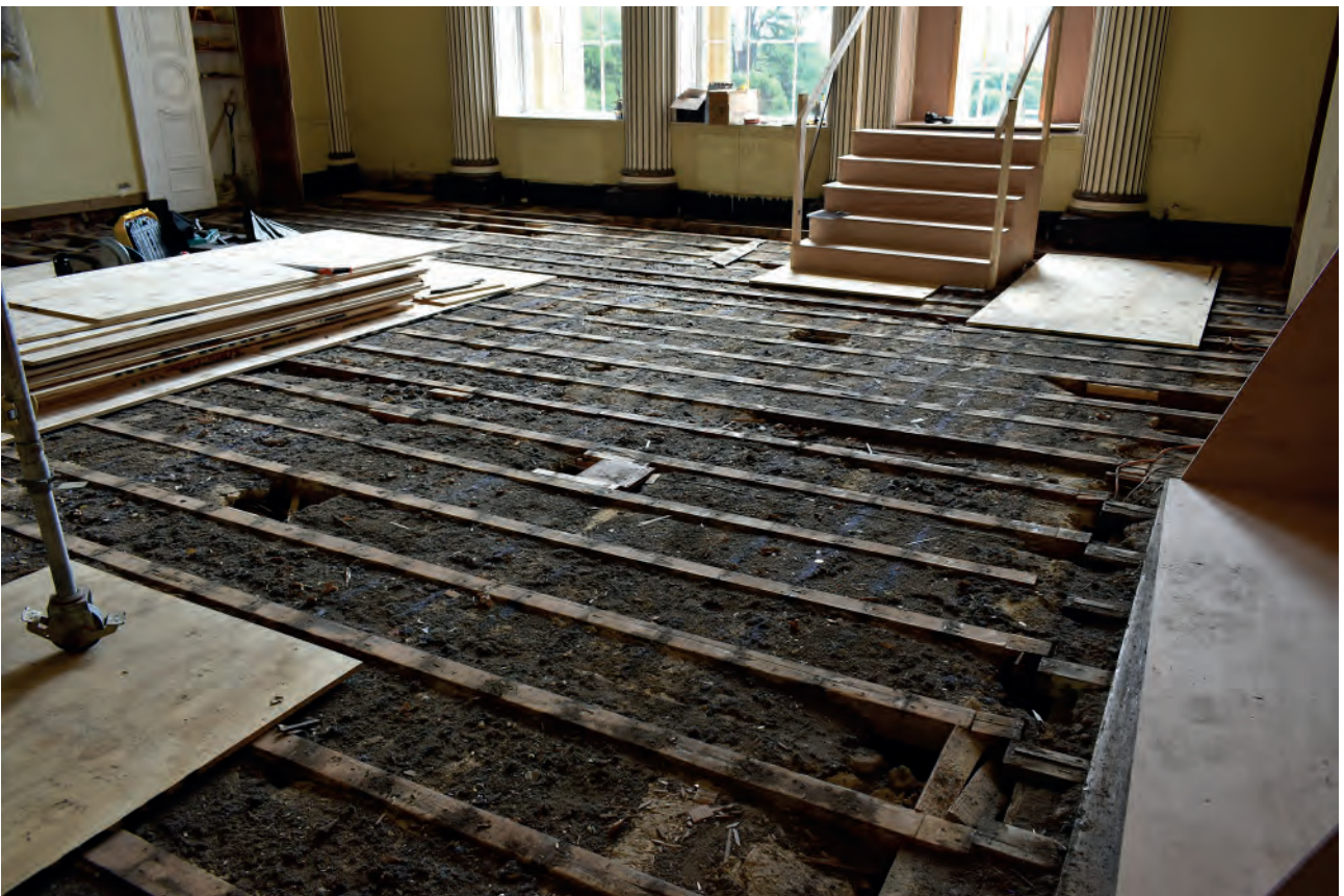
Plate 72: Temple Room, floor, south end, following stripping of floorboards
