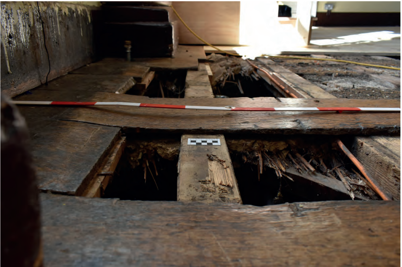
Plate 70: Temple Room, floor, example of floorboard wear in front of the window
