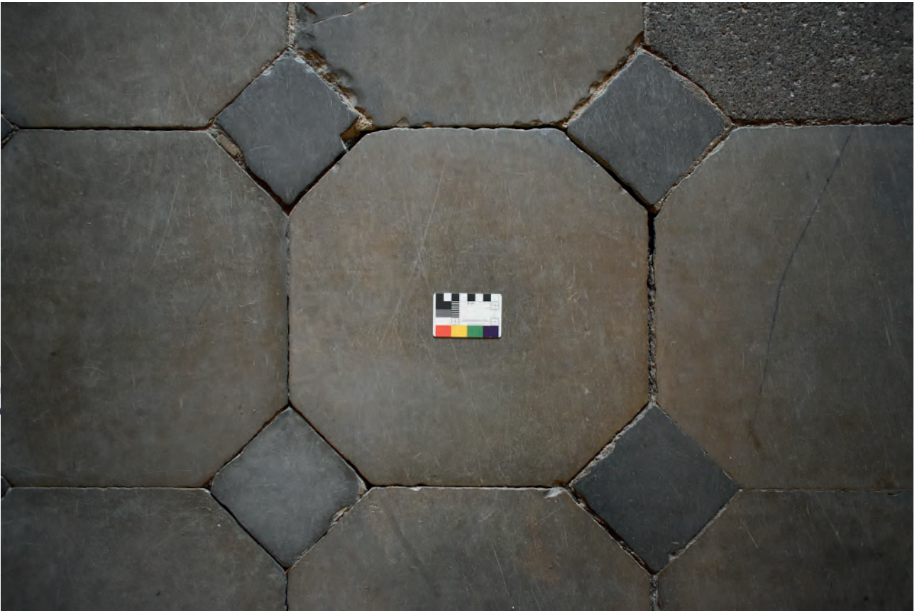
Plate 175: West Corridor, floor, example of original stone floor covering
