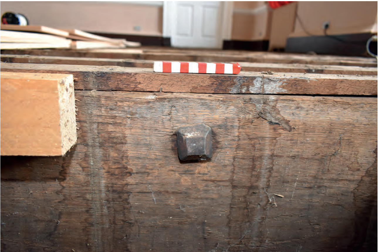
Plate 158: Dining Room, floor, example of ironwork
