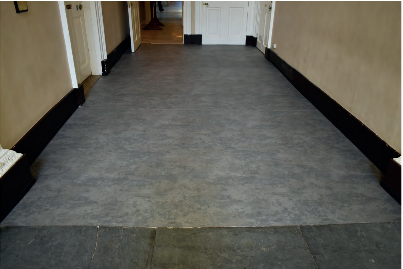
Plate 195: West Corridor, floor, temporary floor covering
