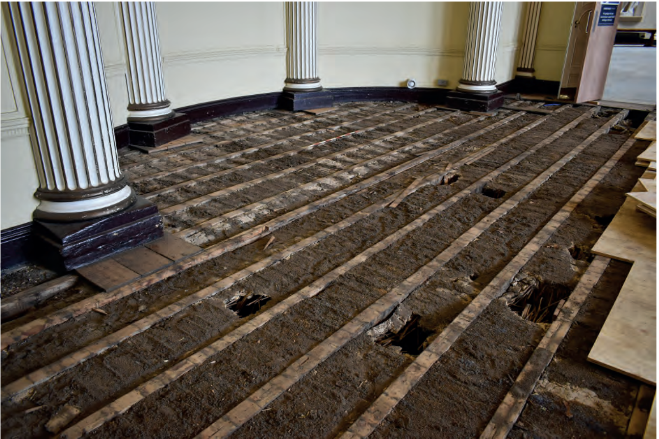
Plate 71: Temple Room, floor, north end, following stripping of floorboards
