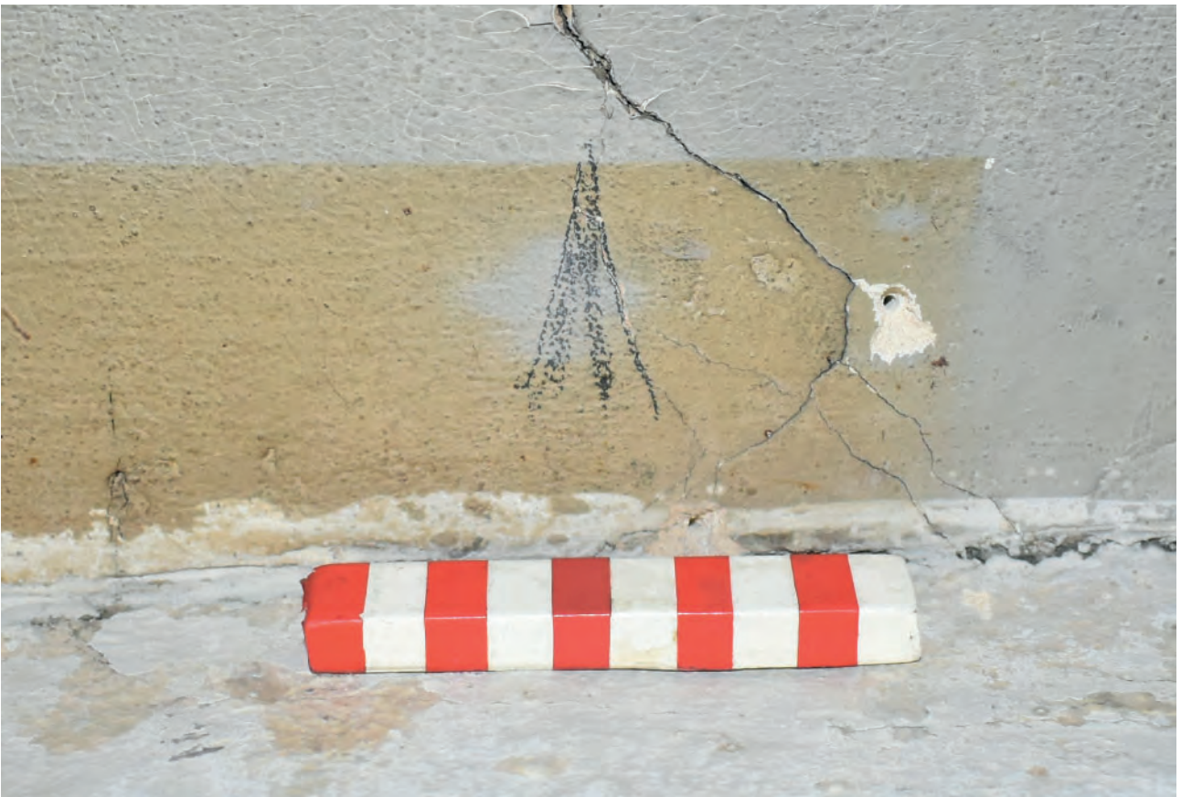
Plate 132: Dining Room, ceiling, example of graffiti
