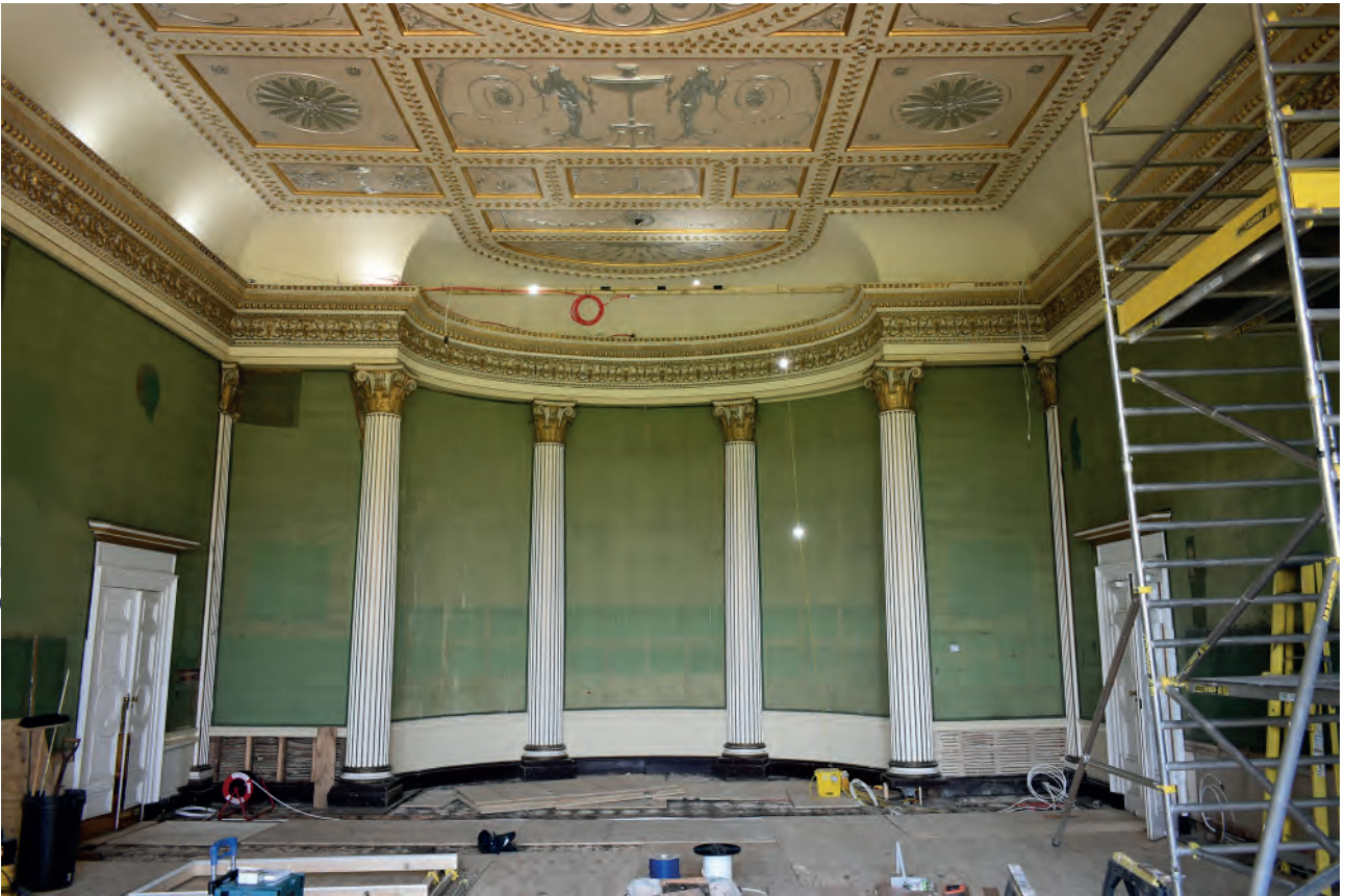
Plate 19: Temple Room, north wall, following stripping
