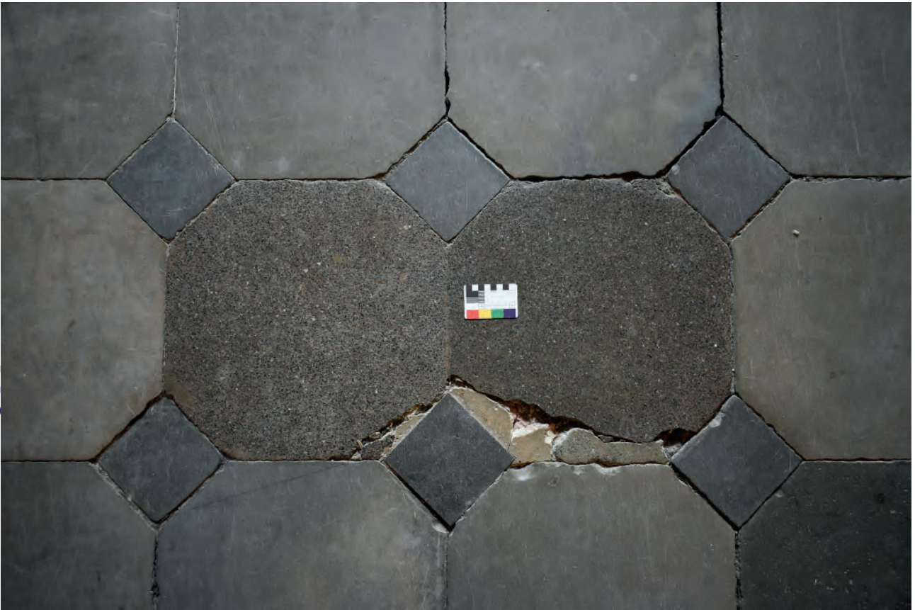
Plate 179: West Corridor, floor, example of concrete repair
