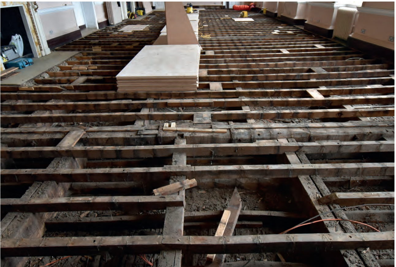
Plate 154: Dining Room, floor, following stripping of the floorboards
