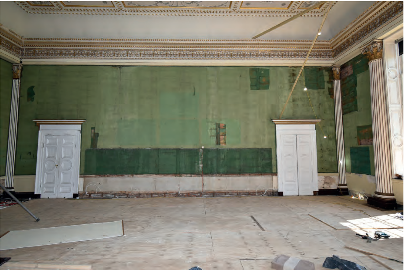
Plate 20: Temple Room, east wall, following stripping
