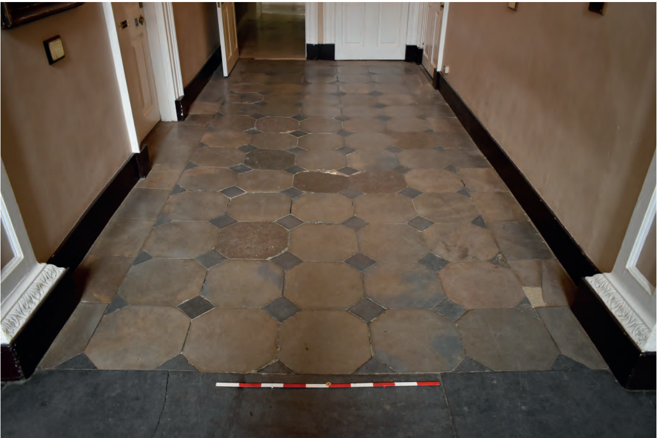
Plate 174: West Corridor, floor, before replacement, looking east
