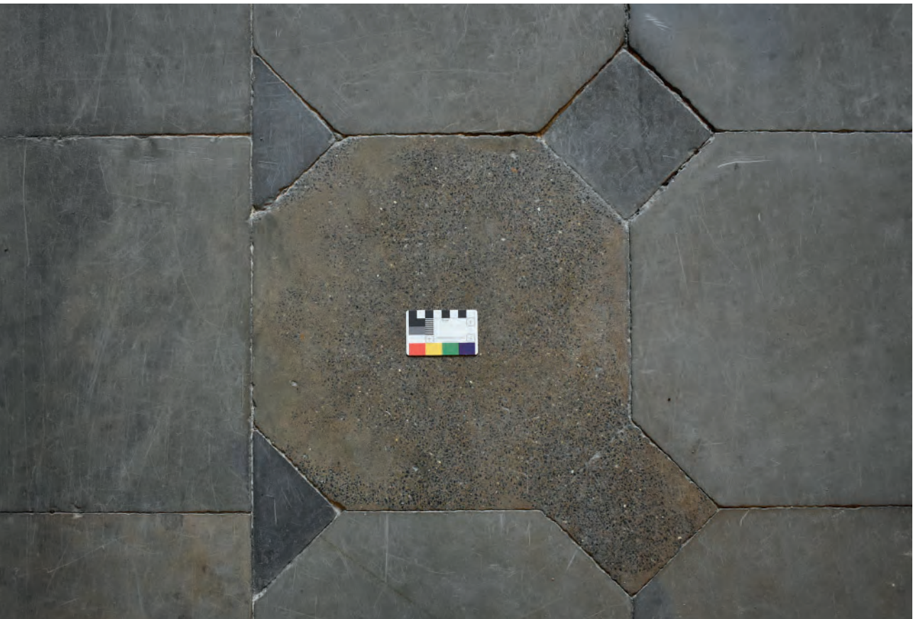
Plate 178: West Corridor, floor, example of concrete repair
