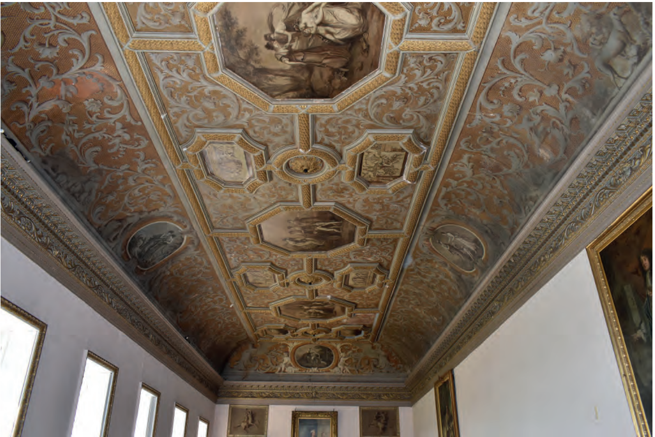
Plate 102: Dining Room, ceiling, before conservation work, looking west
