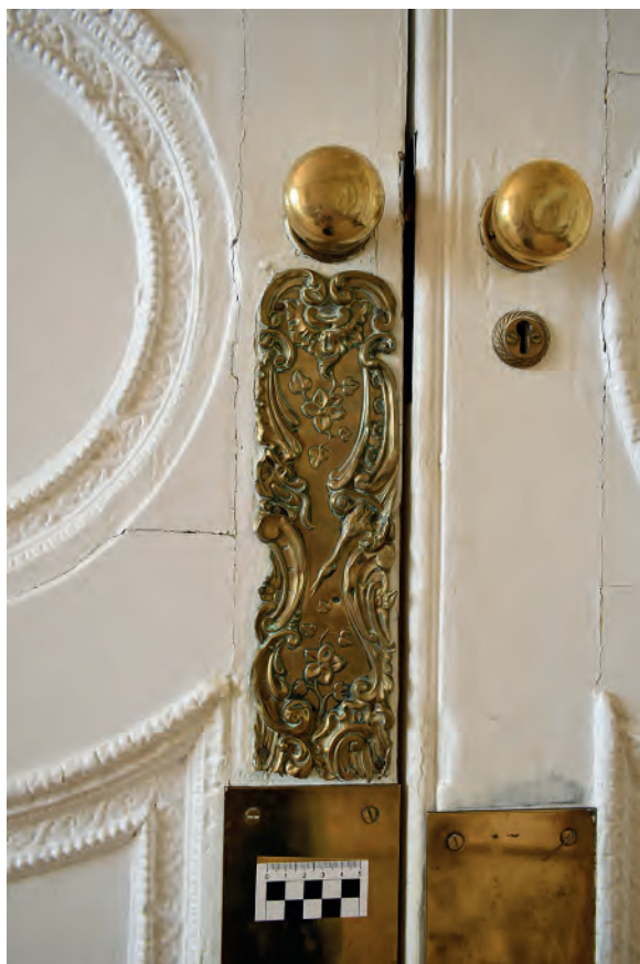
Plate 43: Temple Room, door to Dining Room, detail
