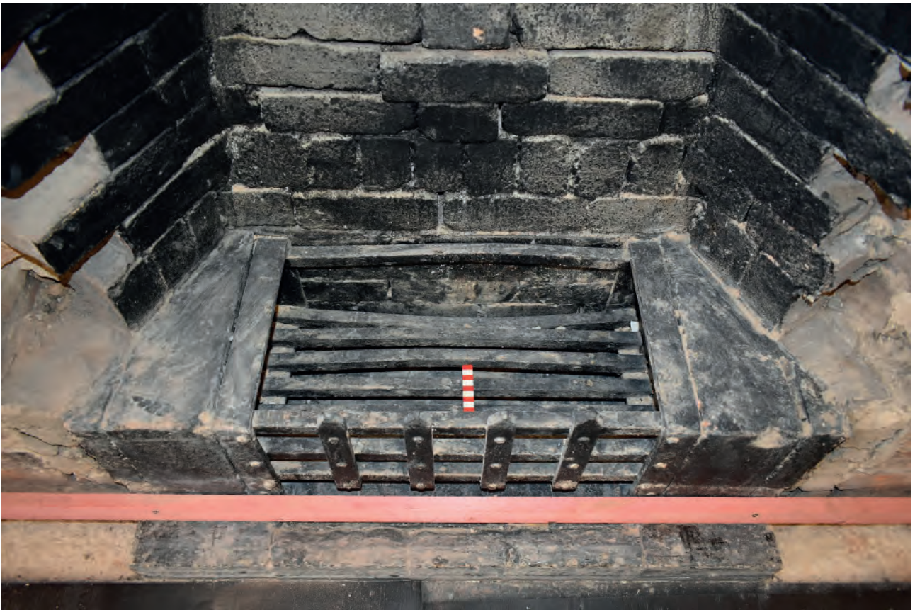
Plate 56: Temple Room, 1922 fireplace
