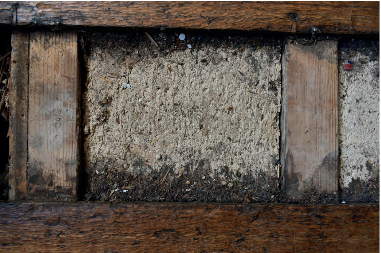
Plate 82: Temple Room, floor, upper surface of pugging
