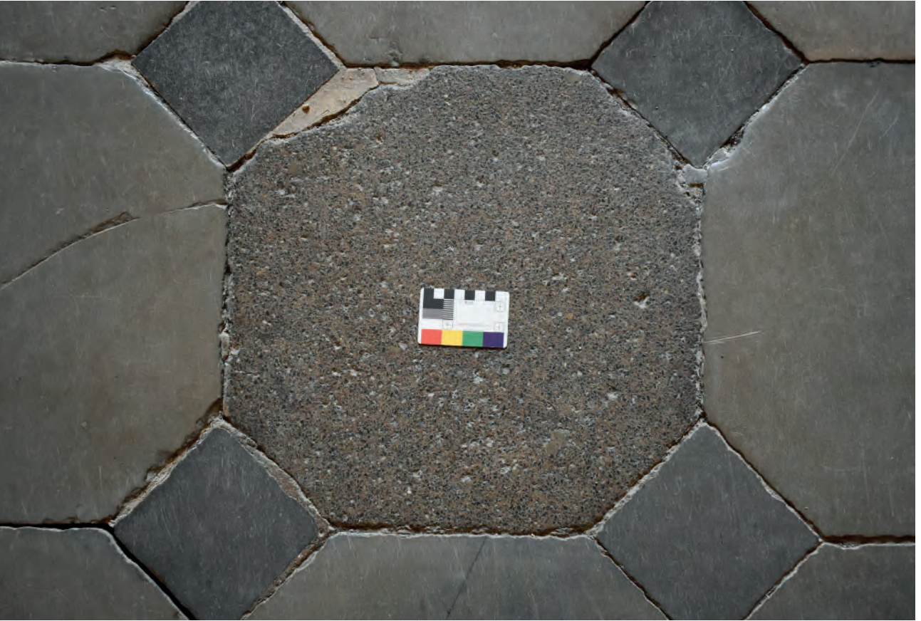
Plate 177: West Corridor, floor, example of concrete repair
