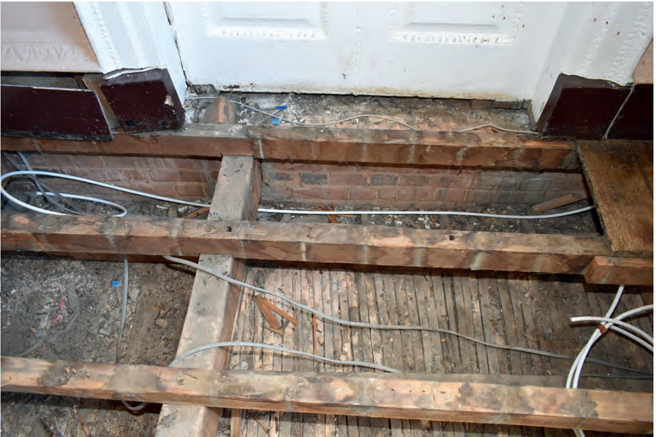
Plate 139: Dining Room, wall, modern brickwork beneath false door to the east wall
