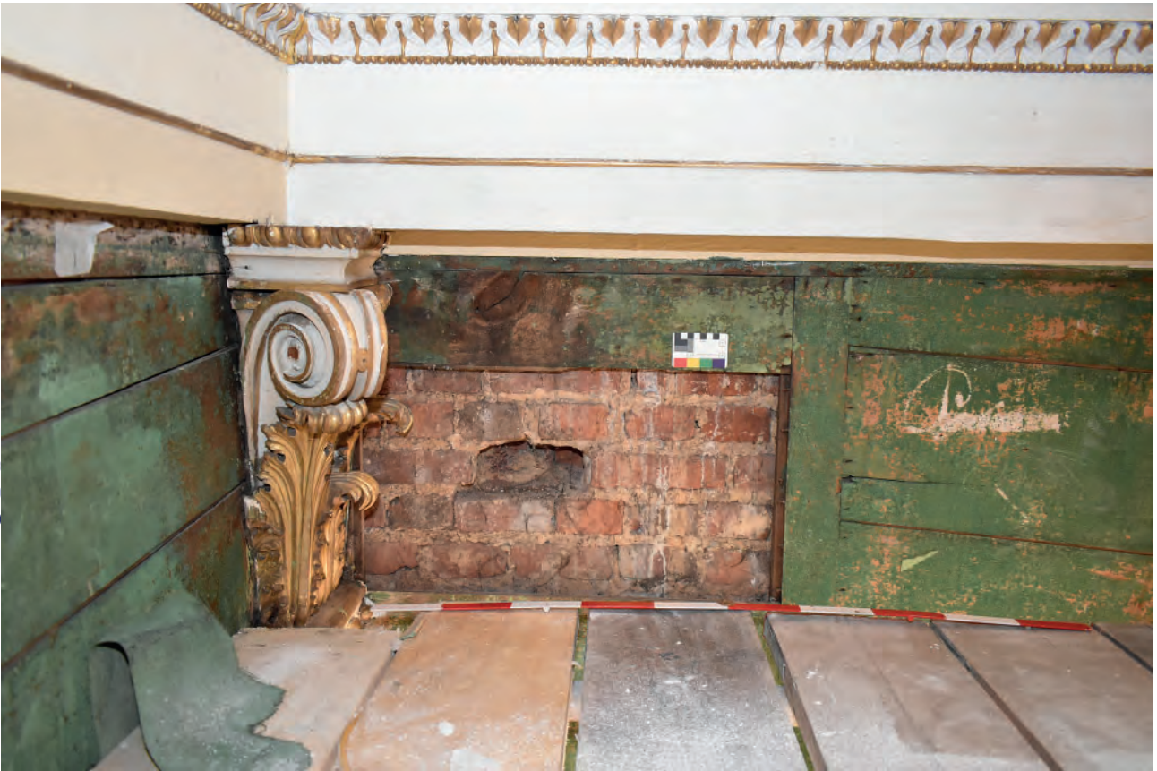
Plate 35: Temple Room, south wall, exposed brickwork
