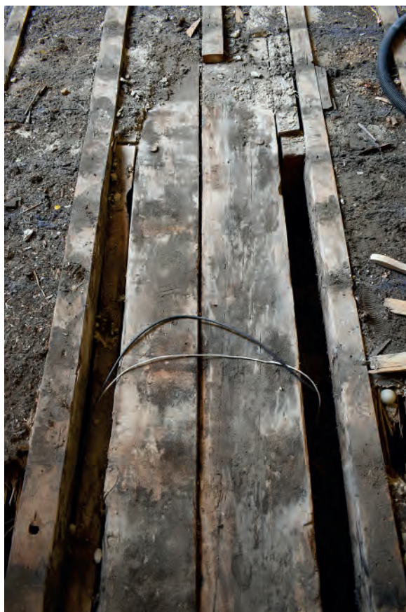
Plate 75: Temple Room, floor, example of a primary beam
