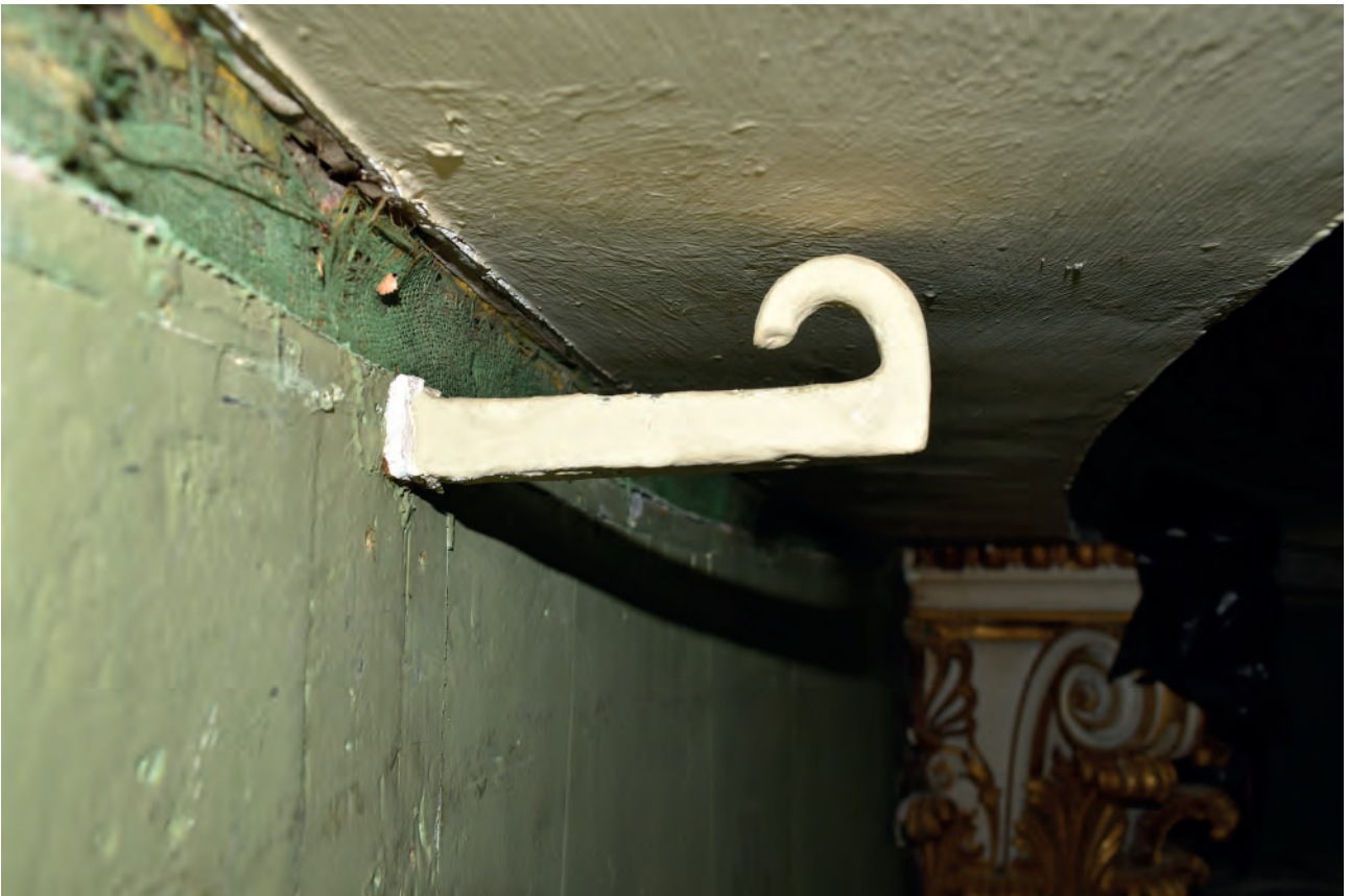
Plate 24: Temple Room, wall, hook in the north wall
