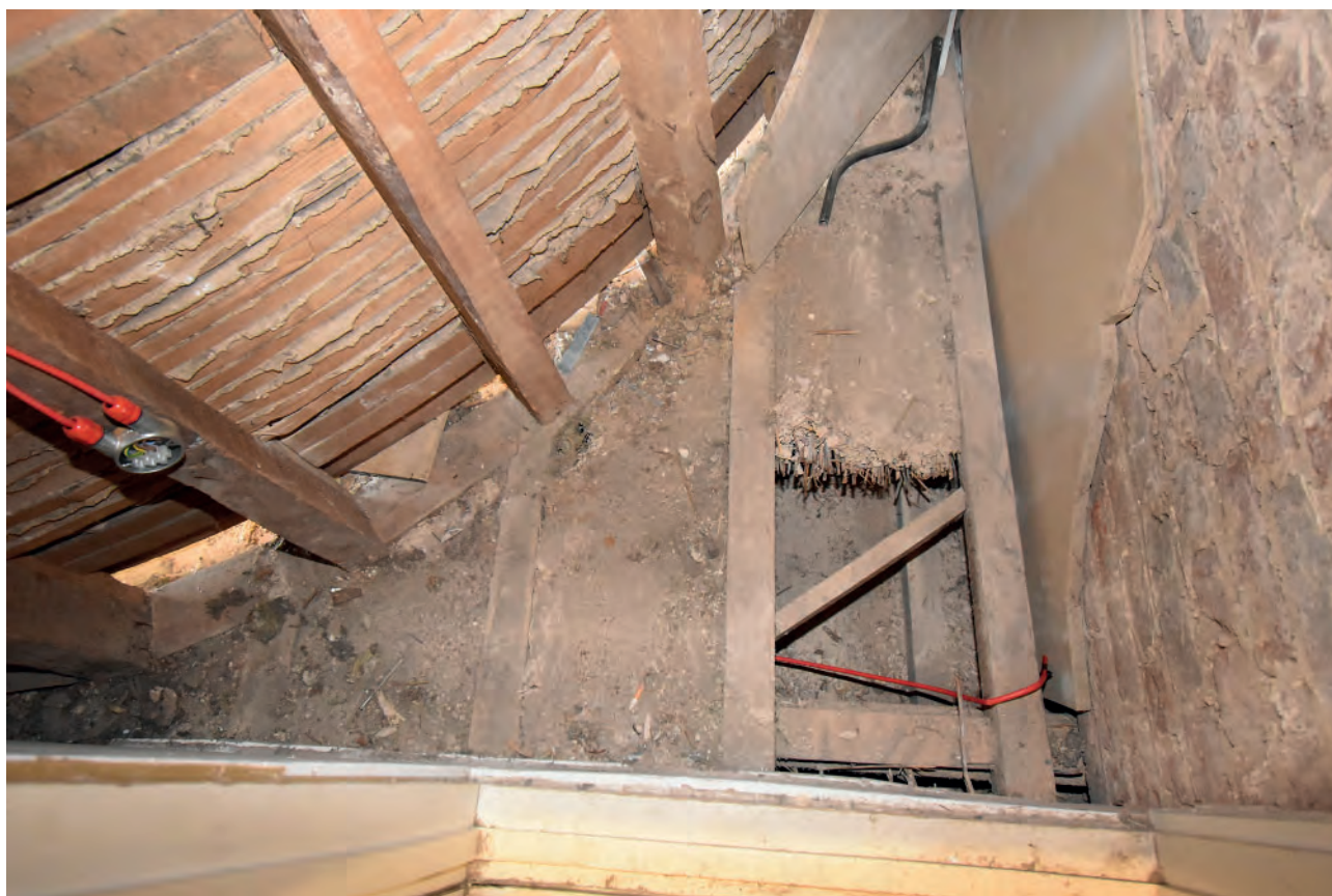
Plate 86: Void behind Temple Room apse, structure of apse
