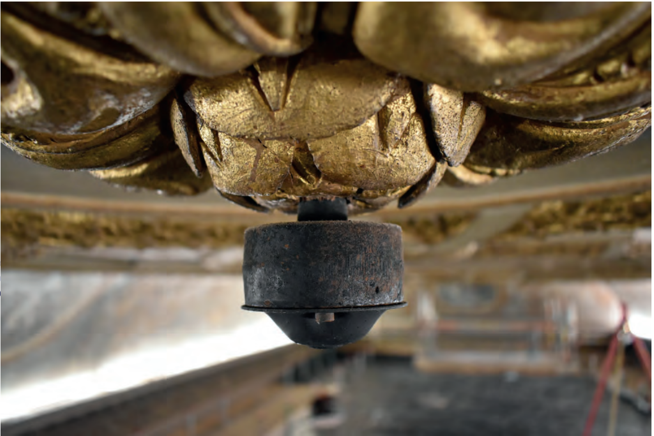
Plate 133: Dining Room, ceiling, redundant gas light fitting
