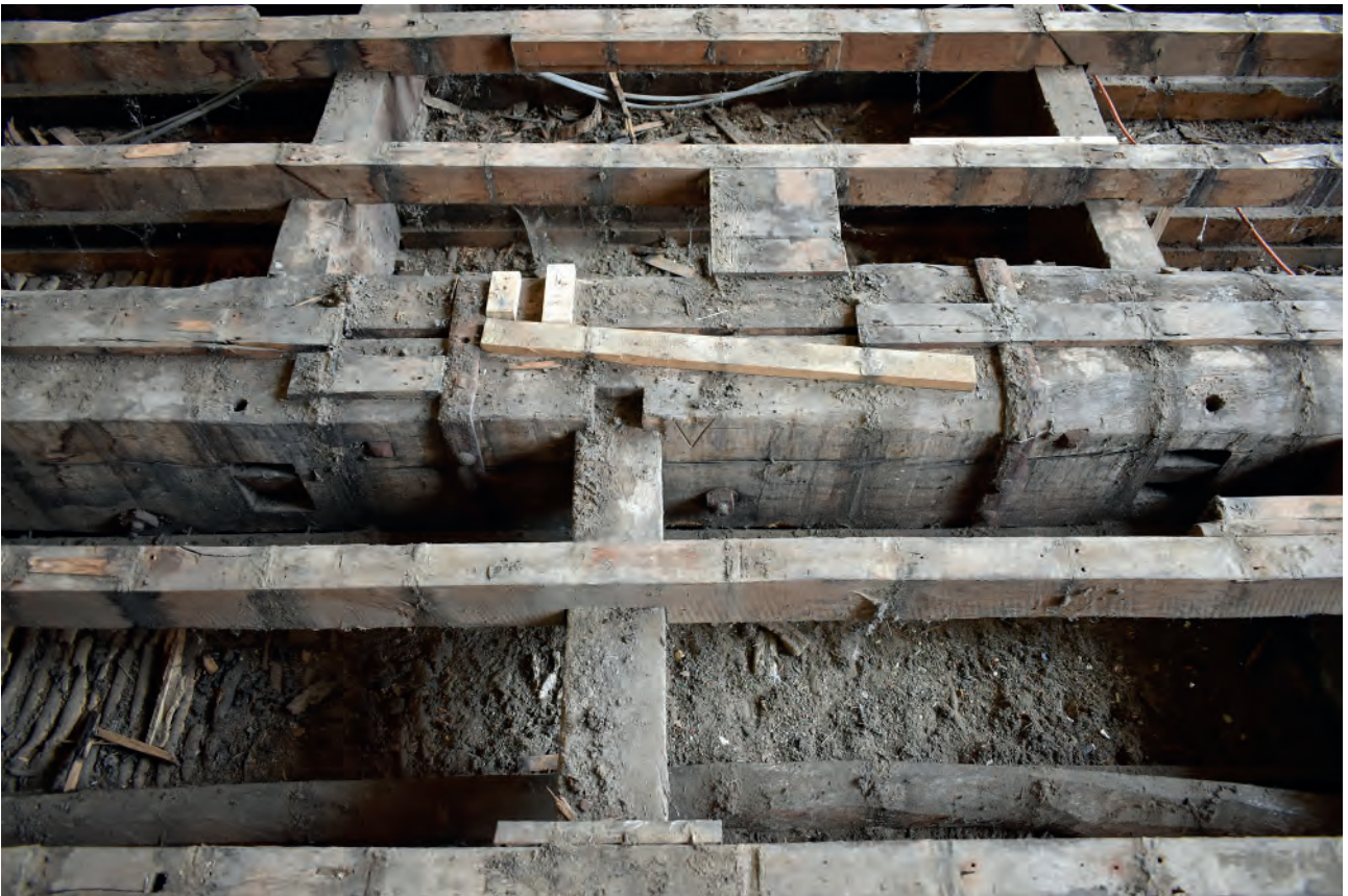
Plate 168: Dining Room, floor, evidence of reconfiguration at the west end of the room
