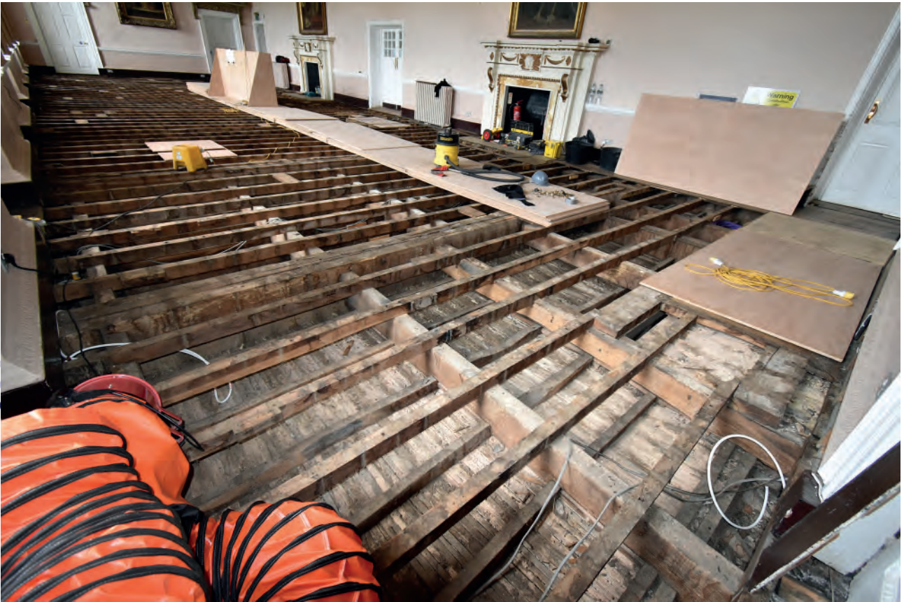
Plate 153: Dining Room, floor, following stripping of the floorboards
