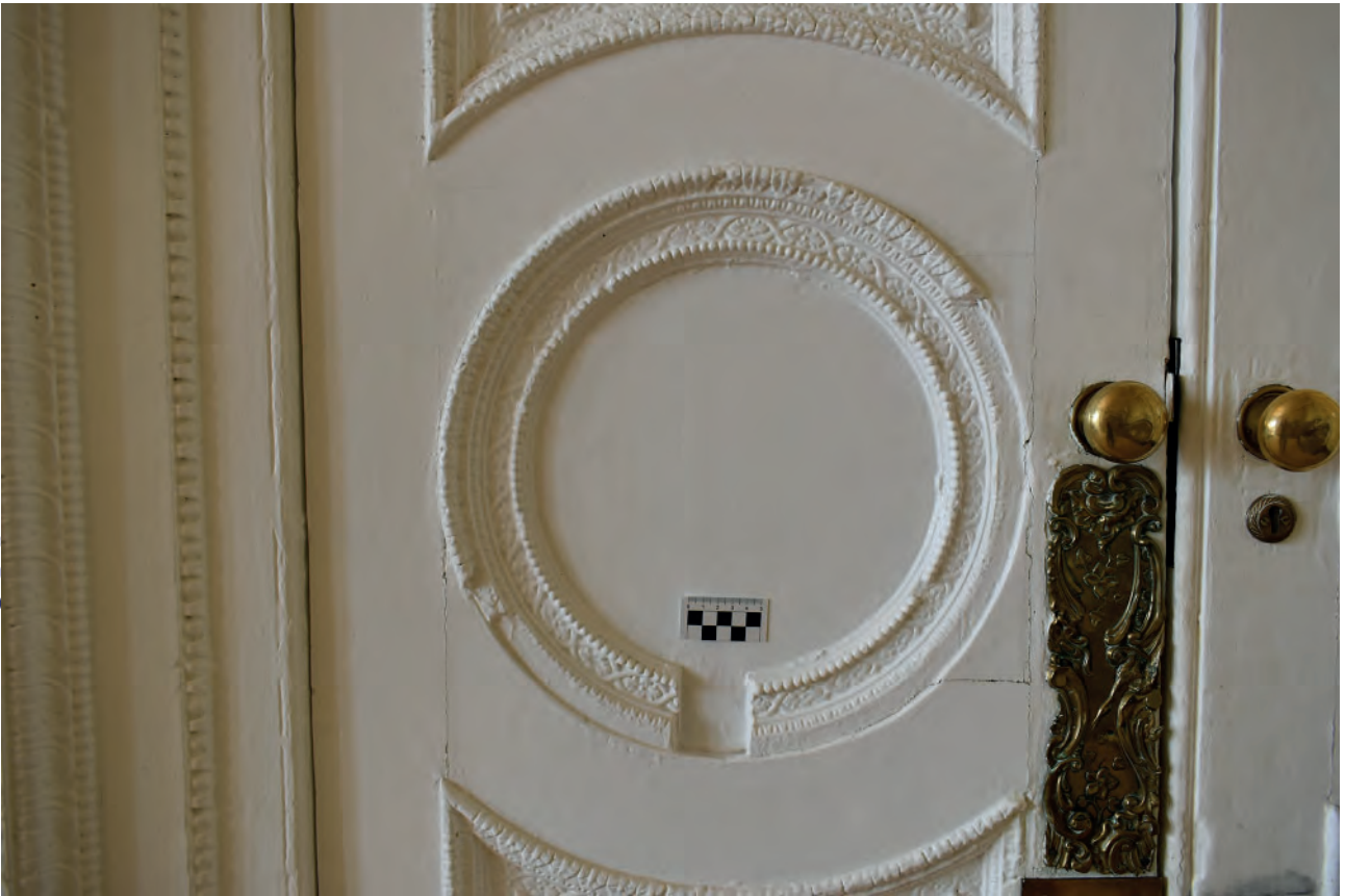
Plate 45: Temple Room, door to Dining Room, damage to moulding
