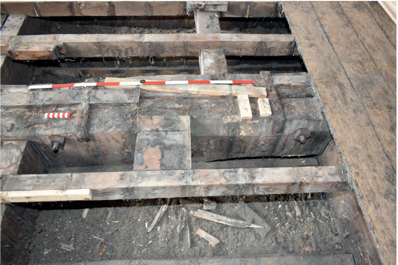
Plate 155: Dining Room, floor, example of a primary beam and ironwork
