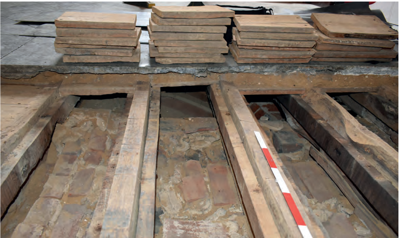
Plate 194: West Corridor, floor, brick vault beneath floor, looking west
