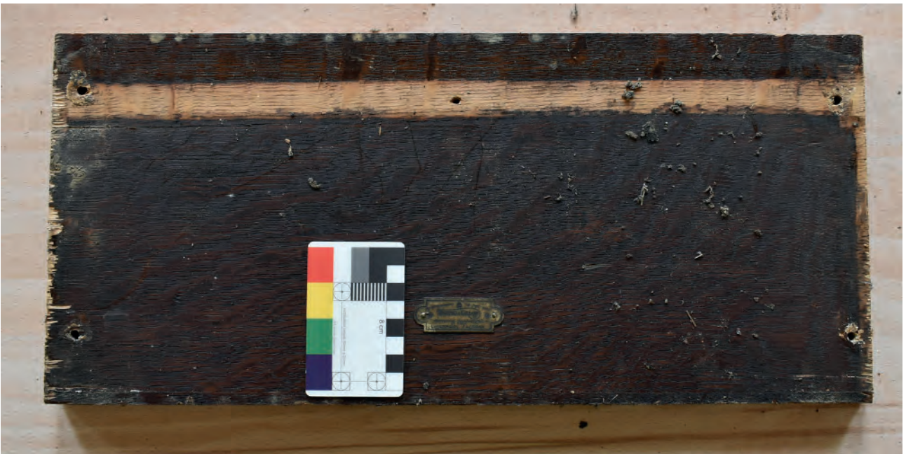
Plate 148: Dining Room, floor, example of furniture used to patch the floorboards
