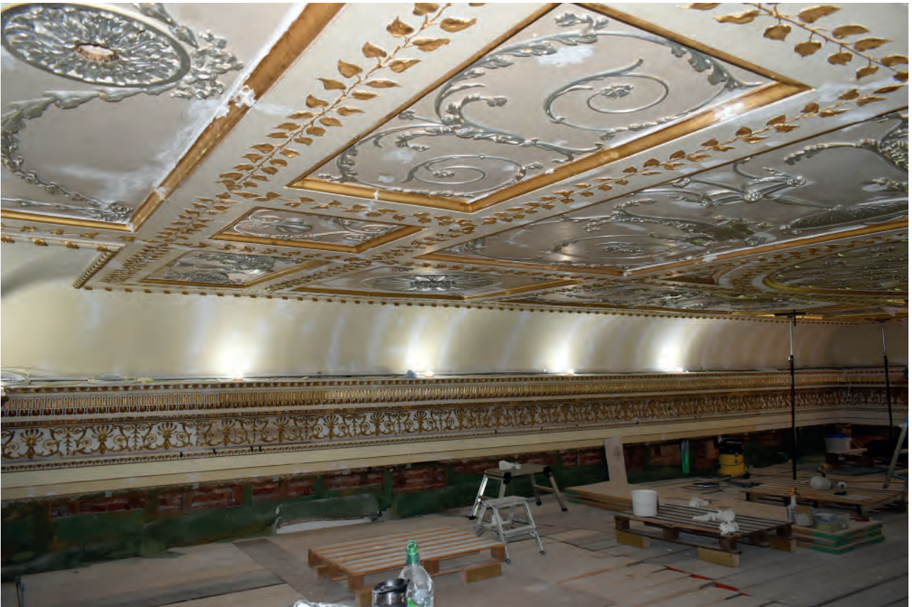
Plate 10: Temple Room, ceiling, during conservation work
