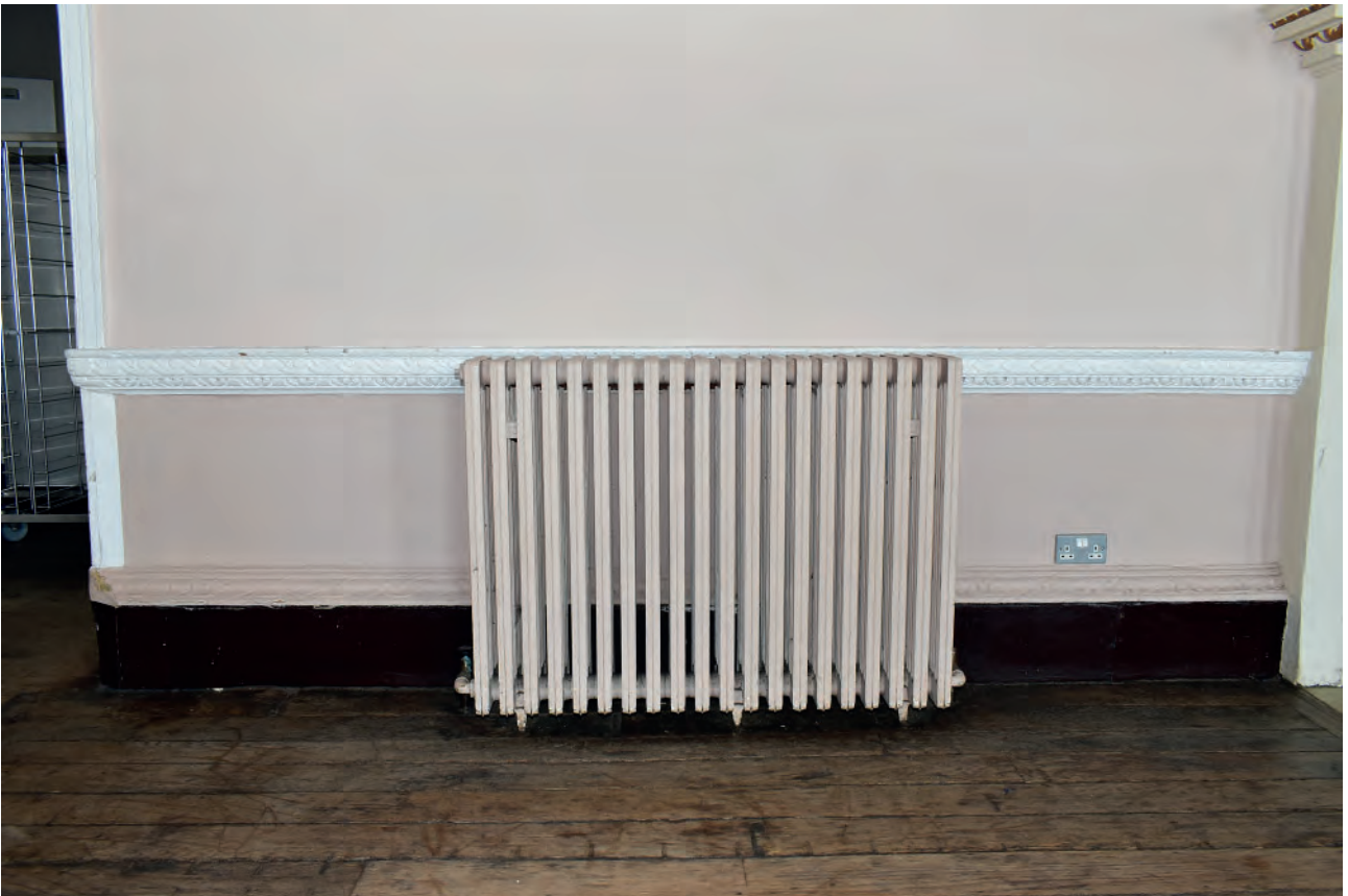
Plate 98: Dining Room, example of a radiator to the north wall
