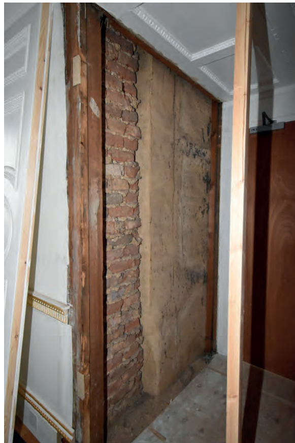
Plate 30: Temple Room, doorway to Dining Room, south return and later brickwork
