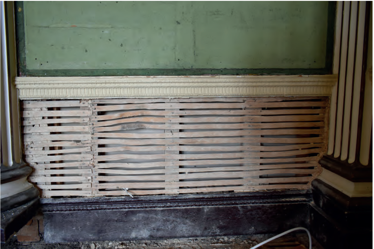
Plate 25: Temple Room, wall, example of lath and plaster
