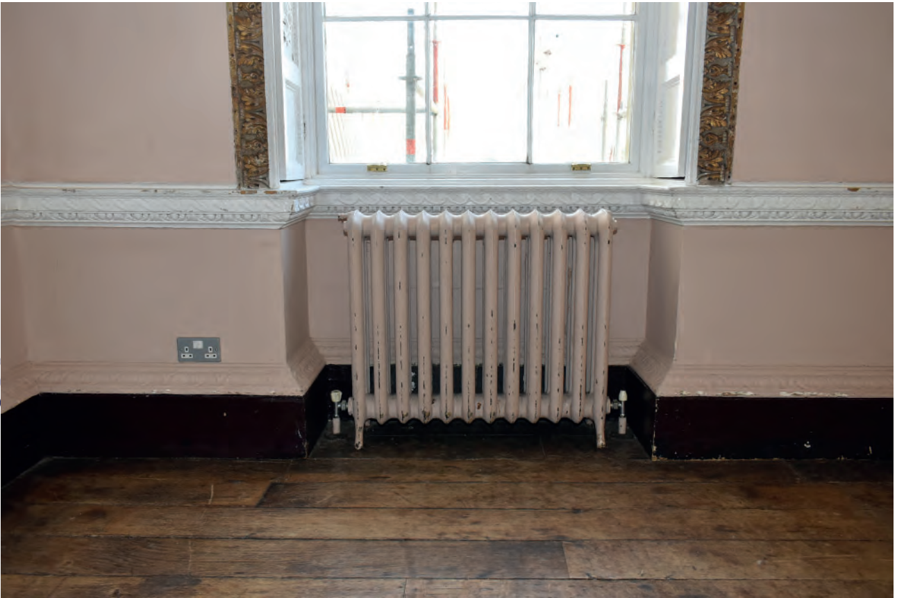
Plate 97: Dining Room, example of a radiator to the south wall
