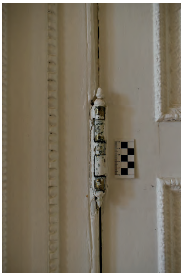
Plate 44: Temple Room, door to Dining Room, detail
