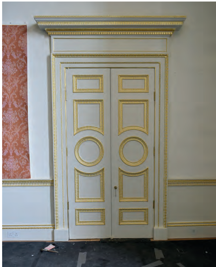
Plate 48: Temple Room, example of door following conservation work
