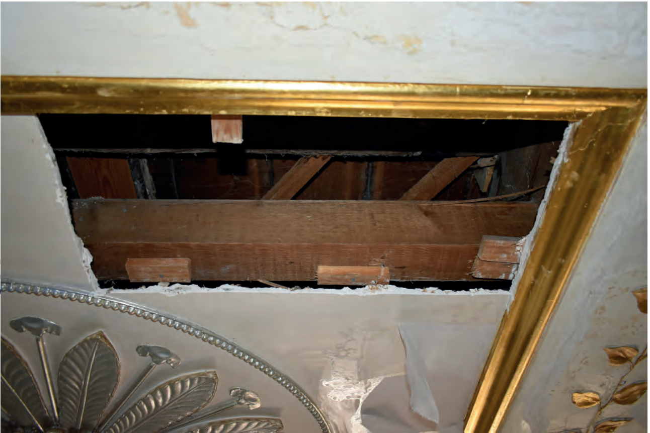
Plate 11: Temple Room, ceiling, 1965 panel towards the south east
