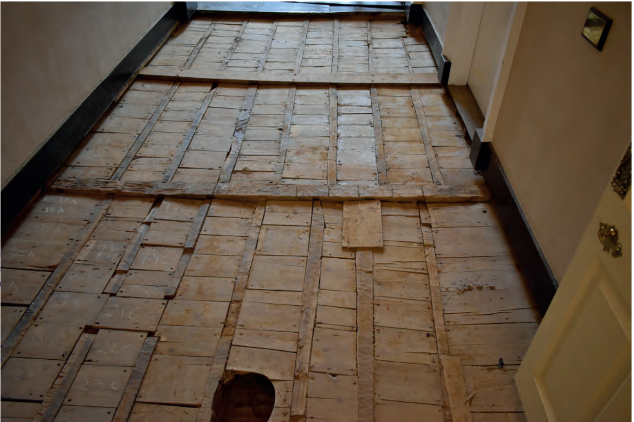
Plate 187: West Corridor, floor, exposed pugging boards, looking west
