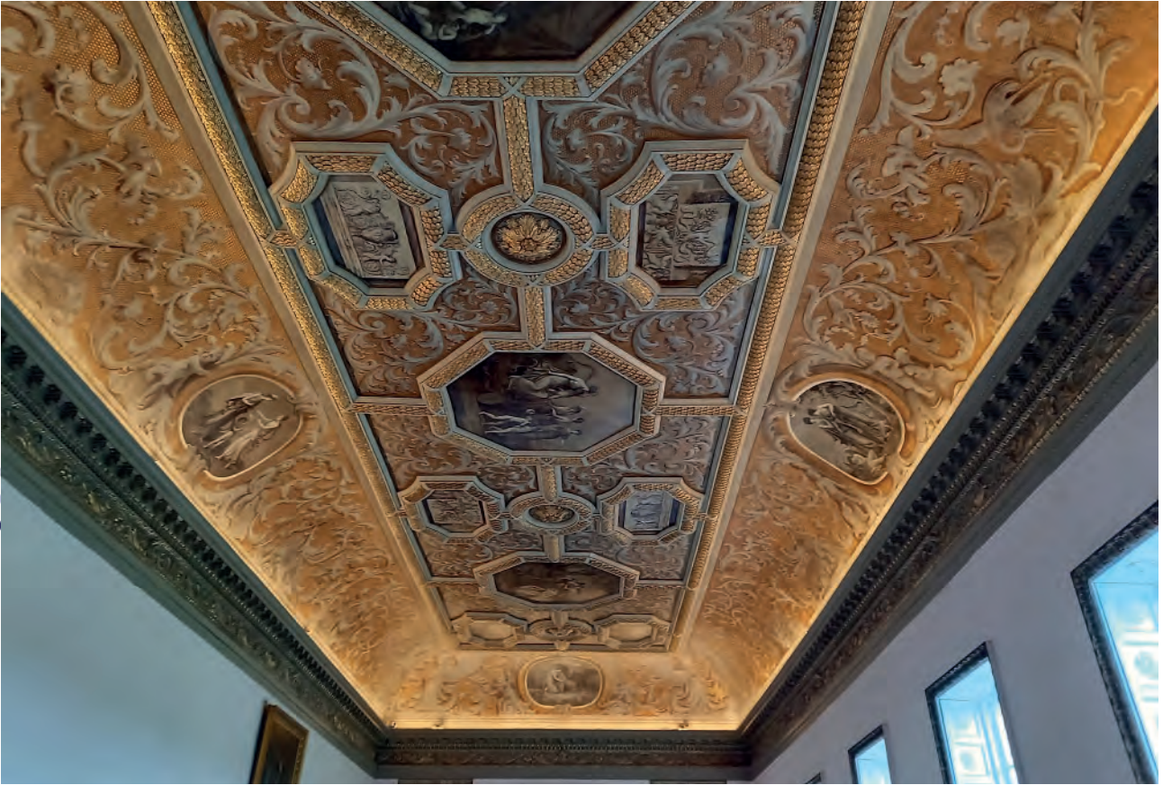
Plate 135: Dining Room, ceiling, following conservation, looking east
