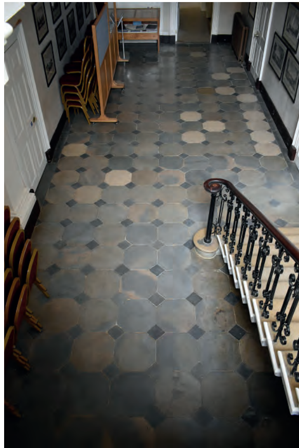
Plate 183: East Corridor, floor following repair work in 2013
