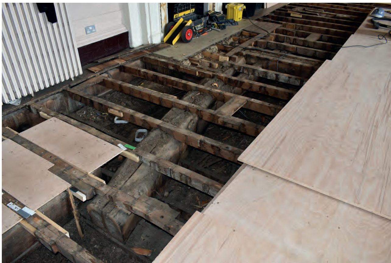
Plate 164: Dining Room, floor, diagonal beam
