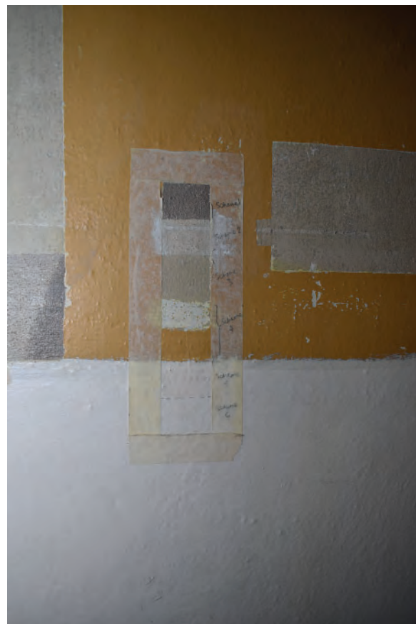
Plate 204: East Corridor Wall Paintings, example of sequence of layers of finishes
