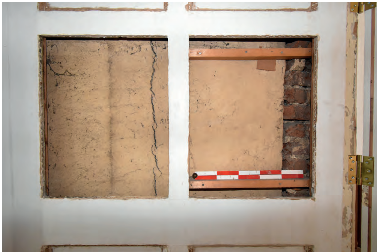
Plate 40: Temple Room, doorway to Dining Room, evidence of panel repair
