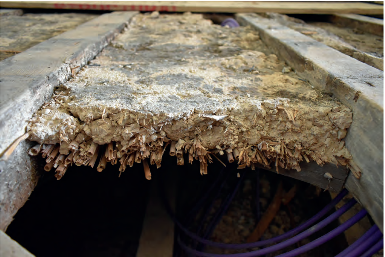
Plate 81: Temple Room, floor, section through pugging
