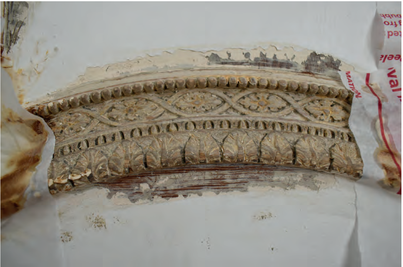
Plate 46: Temple Room, example of stripping moulding
