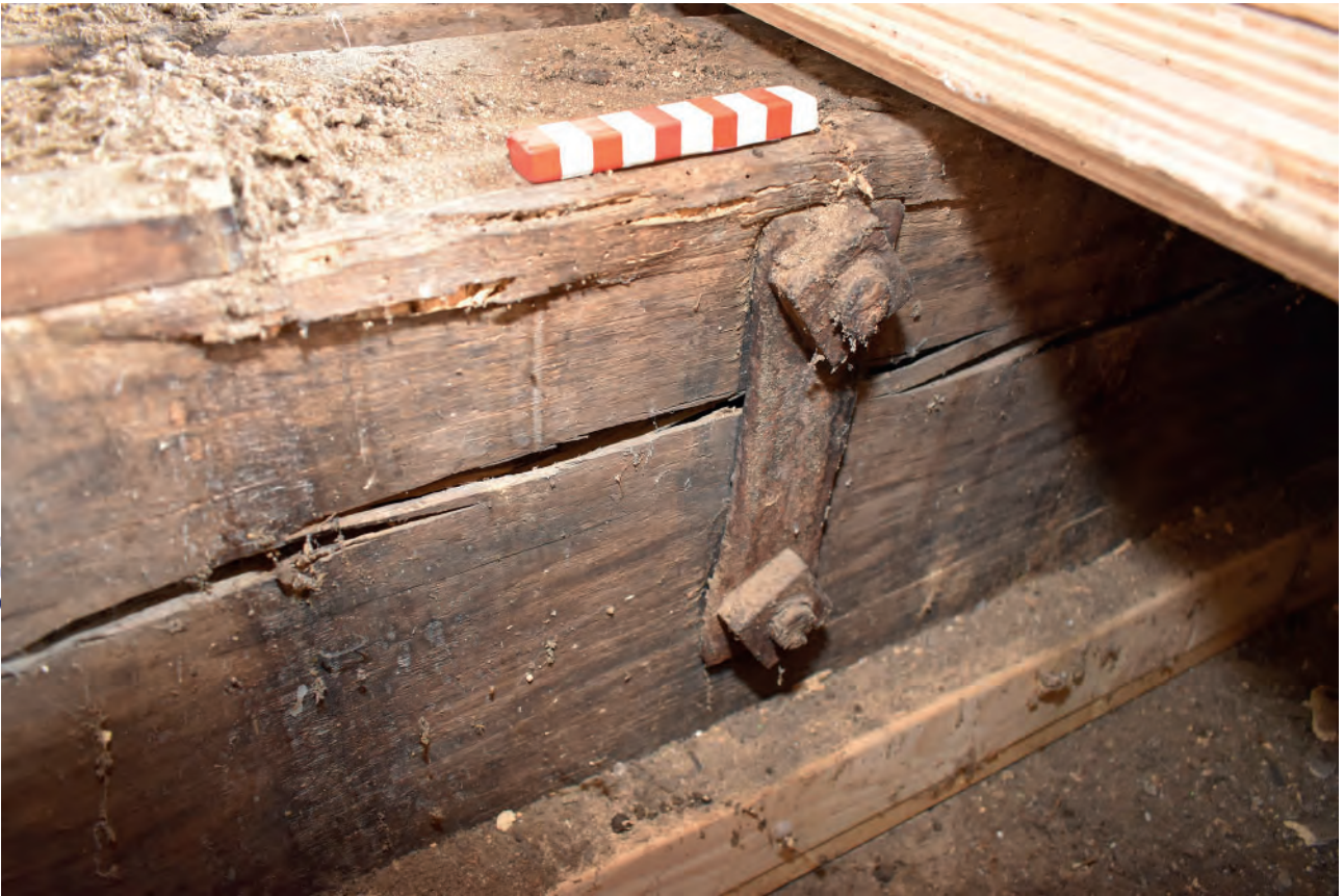
Plate 159: Dining Room, floor, example of ironwork
