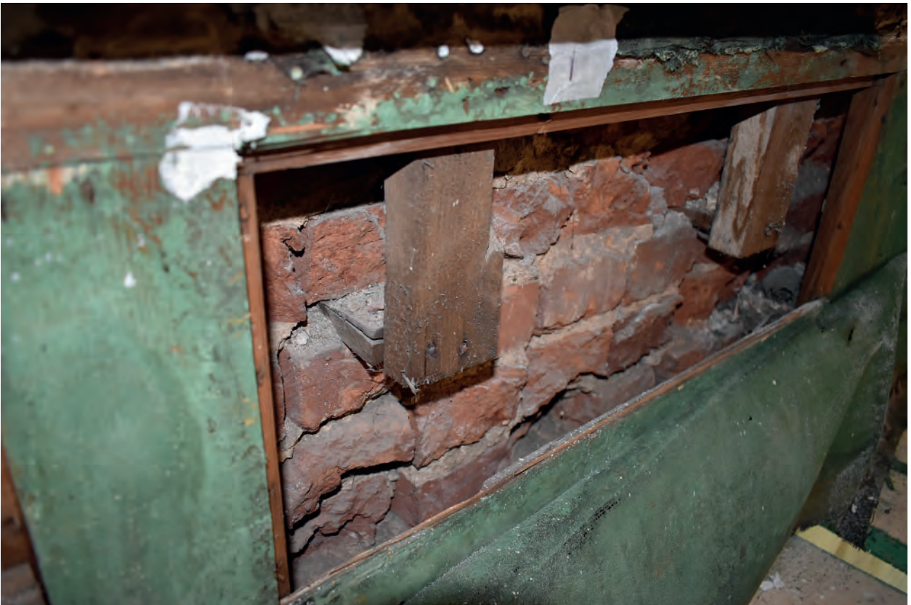
Plate 34: Temple Room, east wall, exposed brickwork
