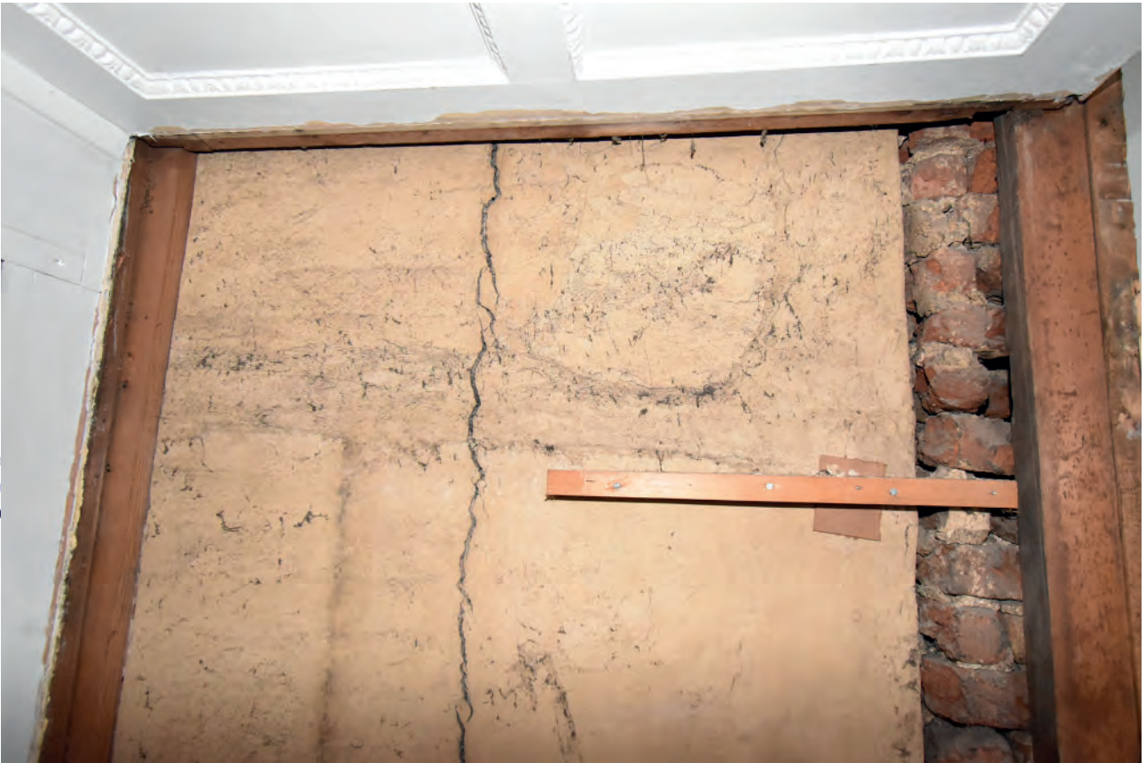
Plate 31: Temple Room, doorway to Dining Room, north return and later brickwork
