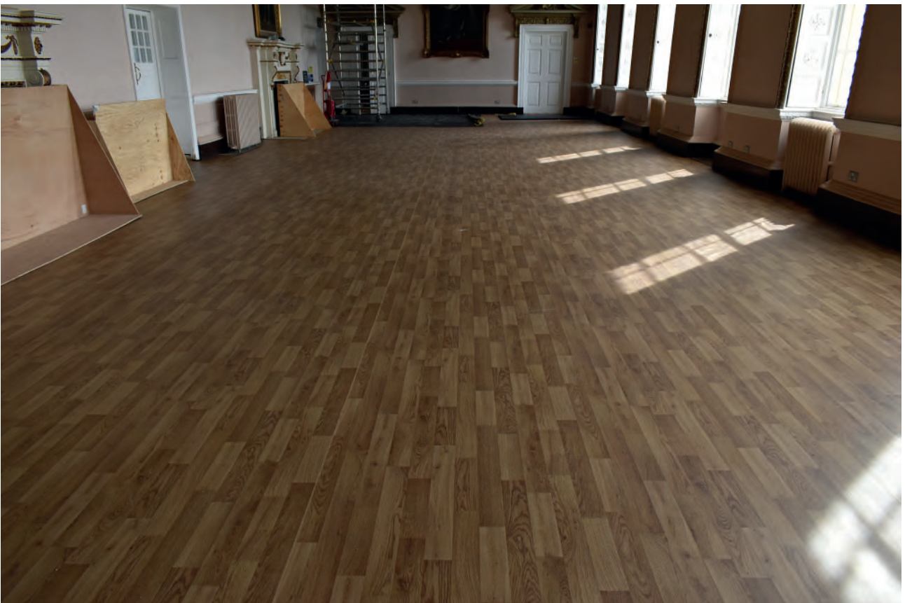
Plate 172: Dining Room, floor, temporary floor covering
