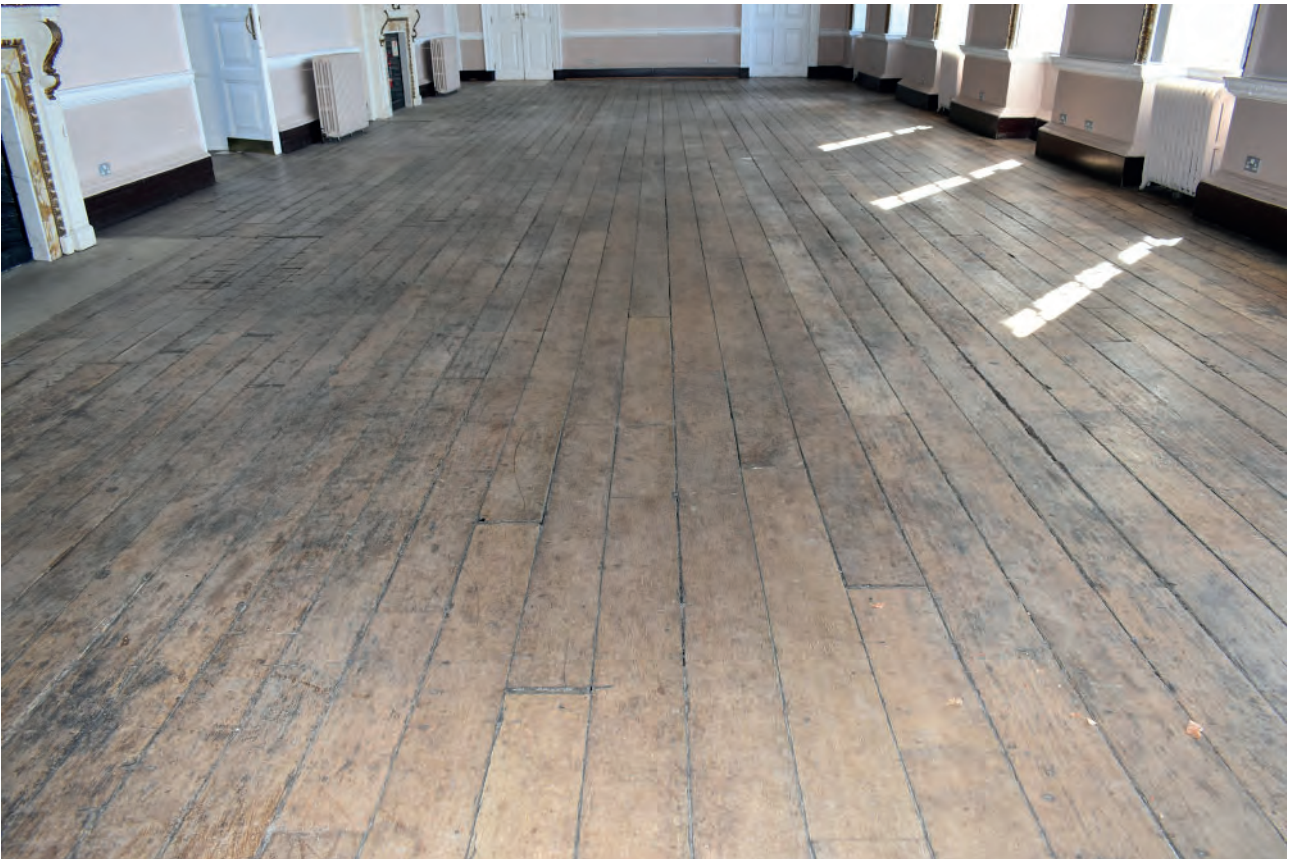
Plate 142: Dining Room, floor, at the start of the project, looking east
