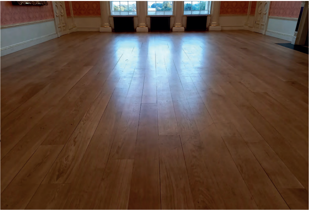
Plate 83: Temple Room, floor, following replacement
