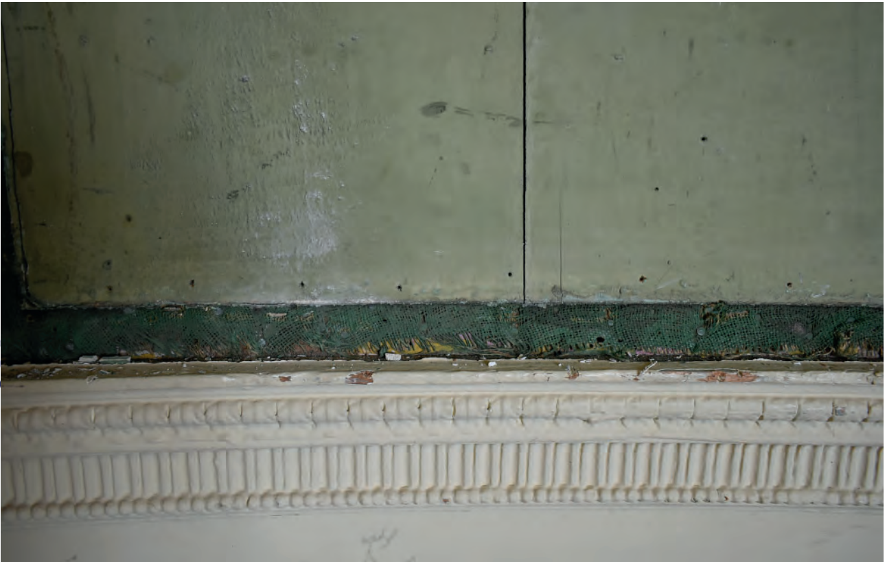
Plate 27: Temple Room, wall, example of strip of hessian remaining around joinery
