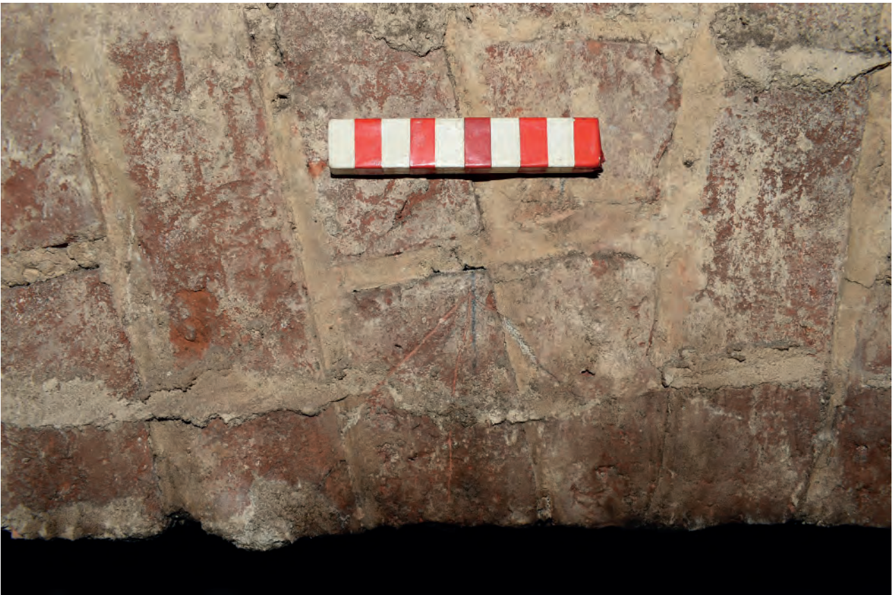
Plate 58: Temple Room, 1922 fireplace construction marks
