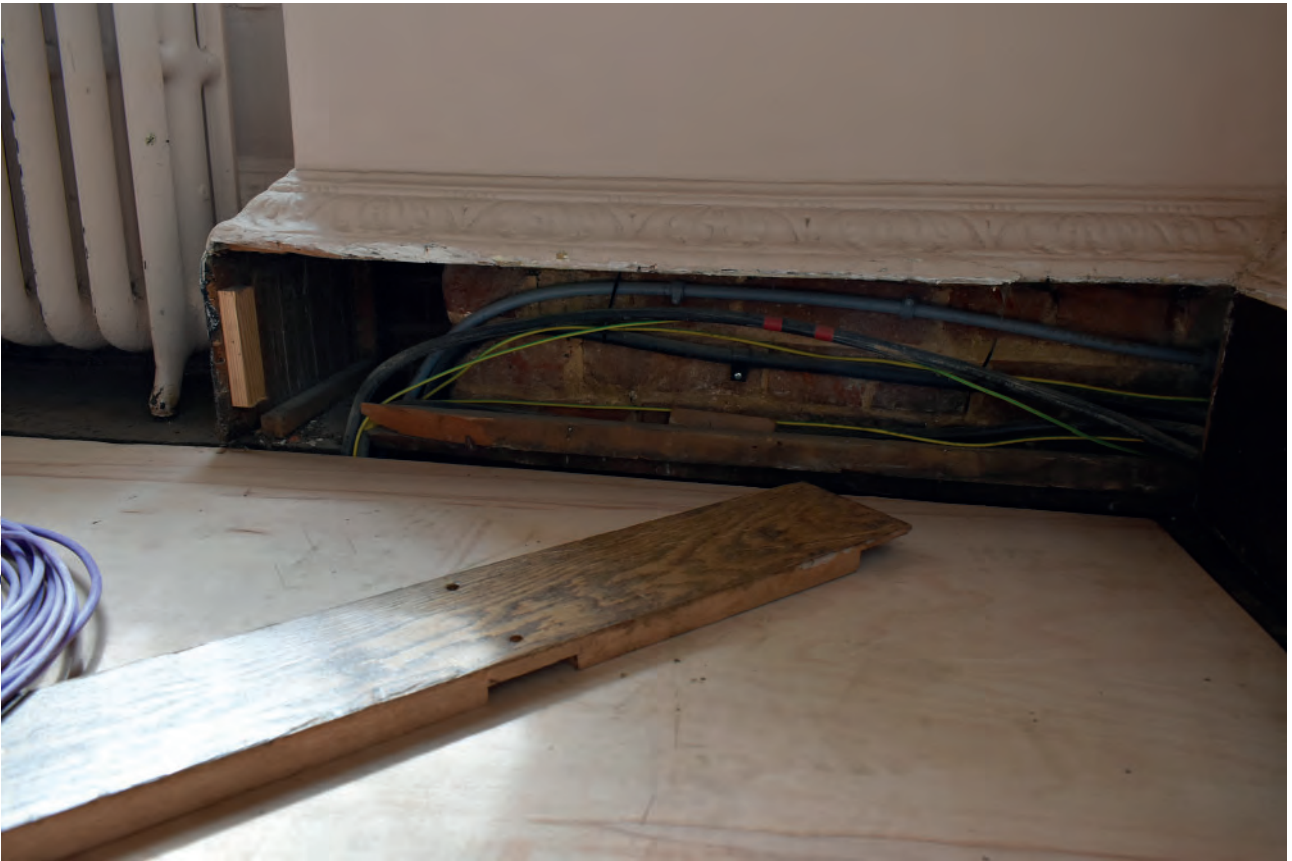
Plate 137: Dining Room, wall, example of brickwork set behind wall surface
