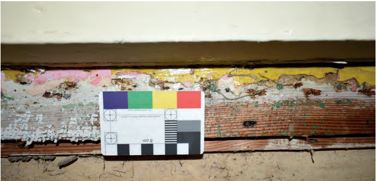
Plate 6: Temple Room, partial sequence of decorative finishes
