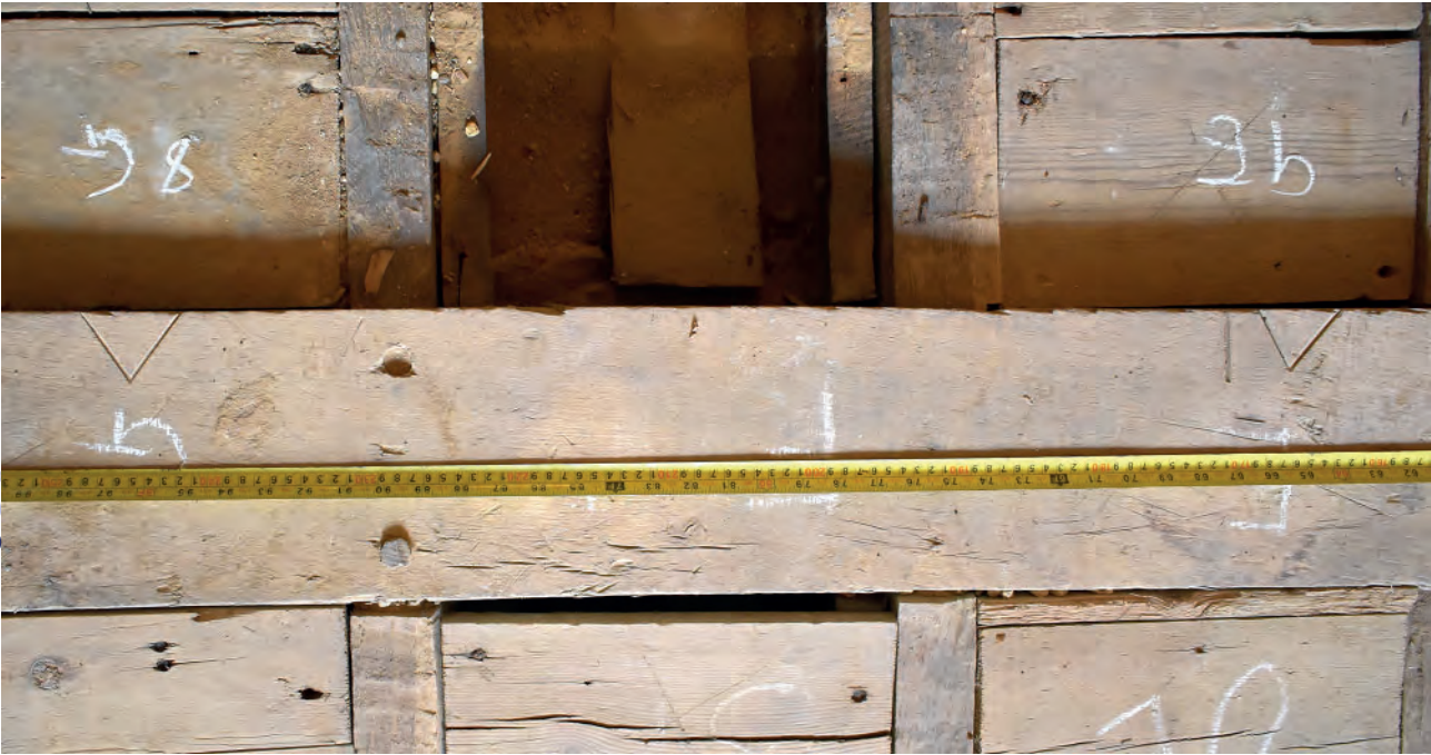
Plate 191: West Corridor, floor, example of carpenter's marks to the westernmost beam
