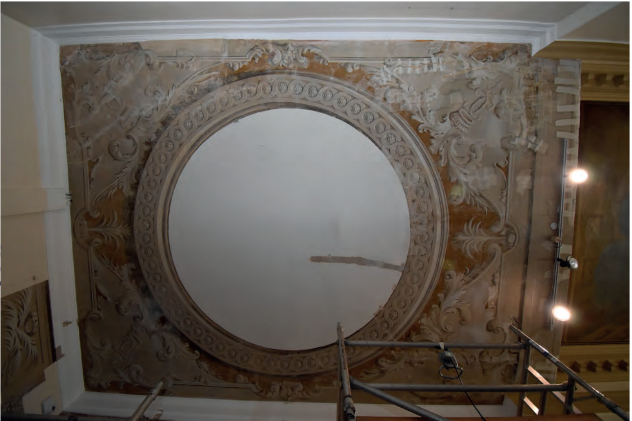
Plate 197: East Corridor Wall Paintings, ceiling above landing
