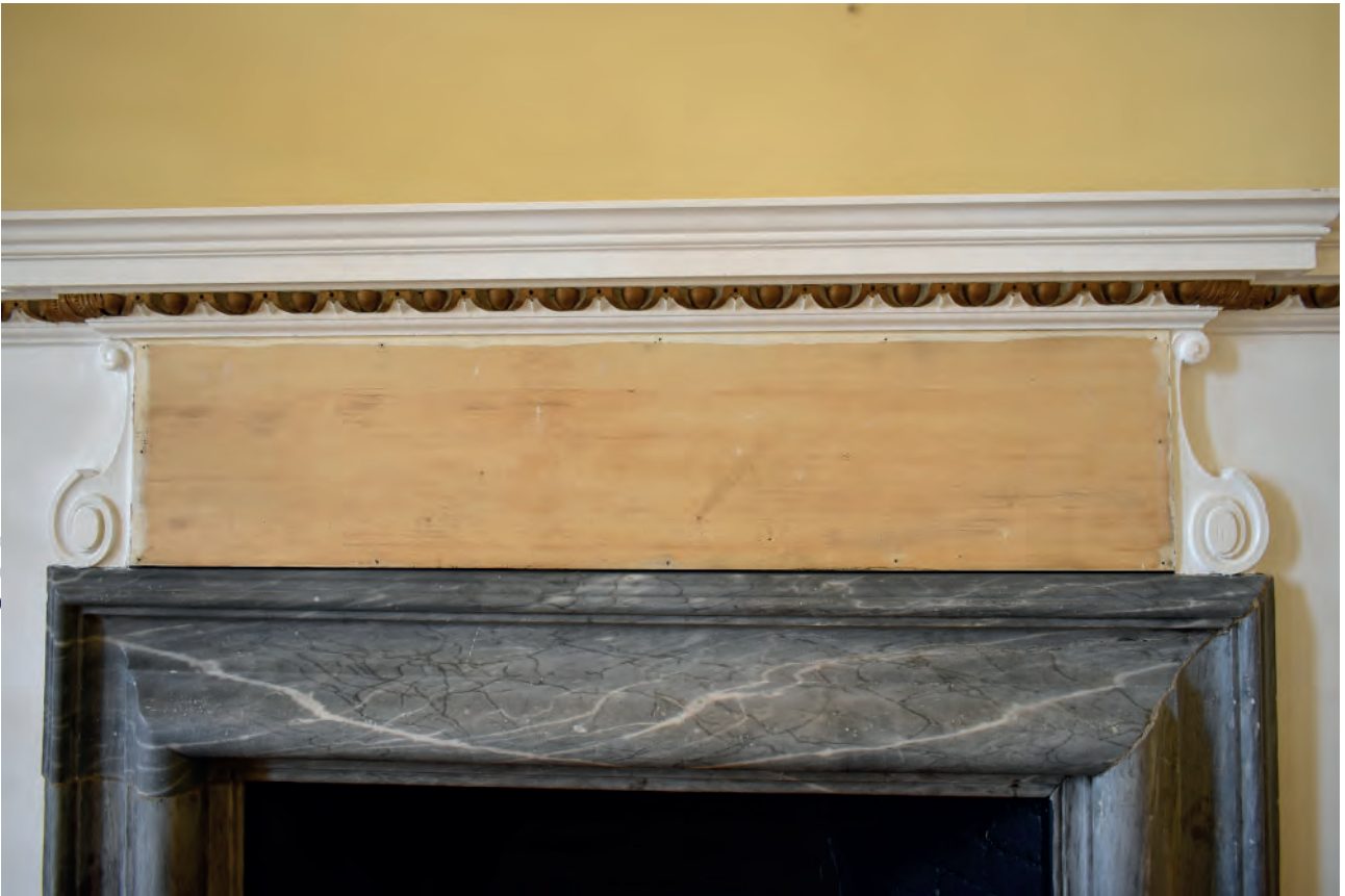
Plate 55: Temple Room, 1922 fireplace
