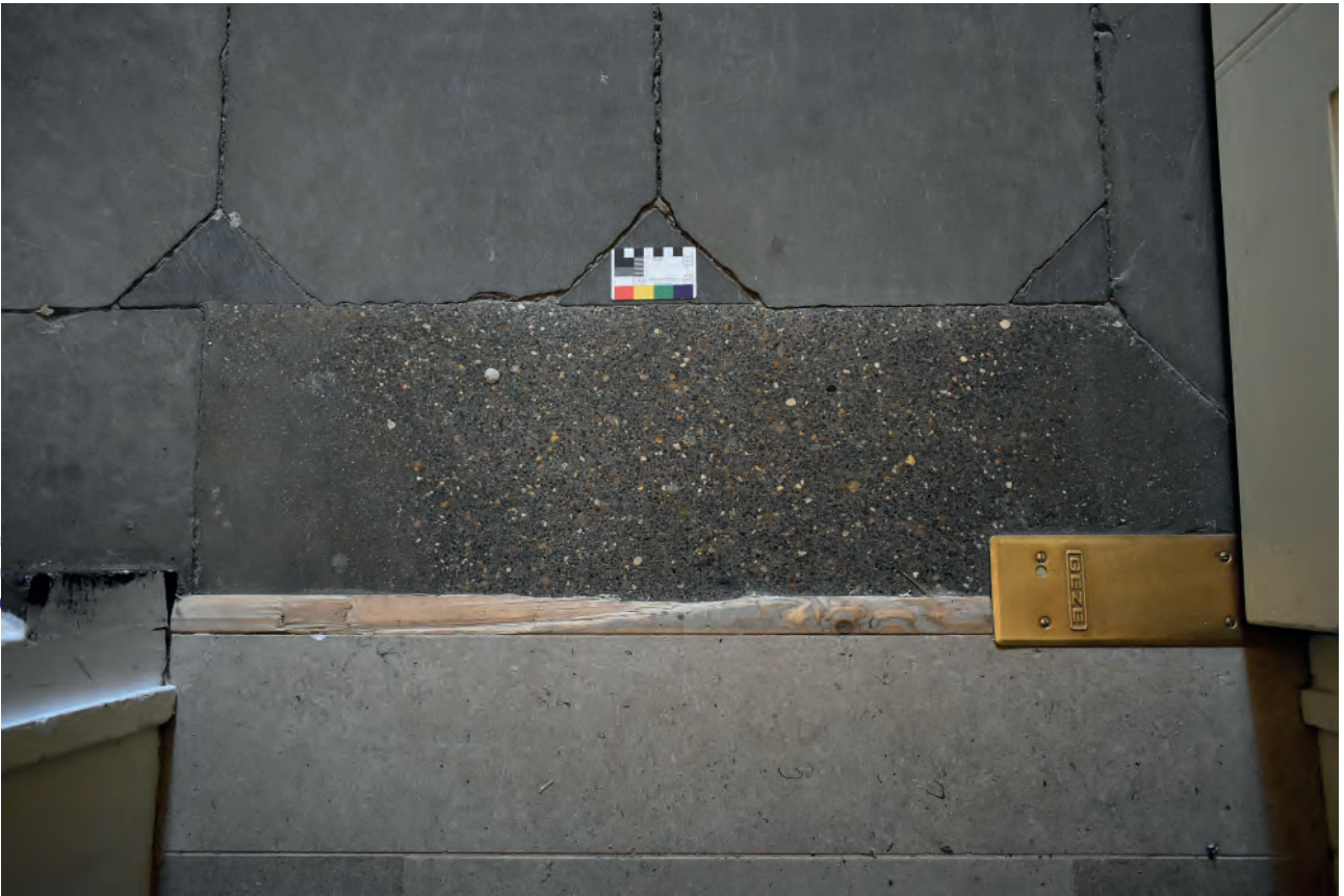
Plate 181: West Corridor, floor, example of concrete repair
