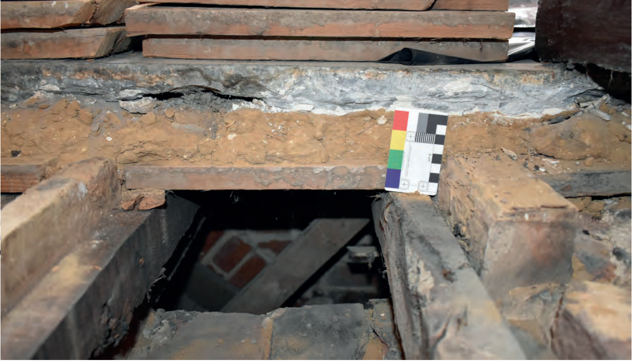
Plate 185: West Corridor, floor, sandy levelling layer
