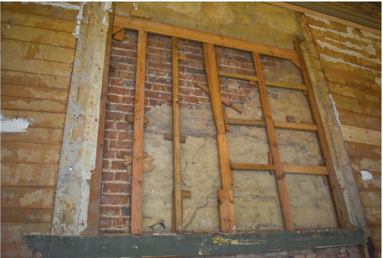
Plate 18: North wall, lime plaster behind east overmantel
