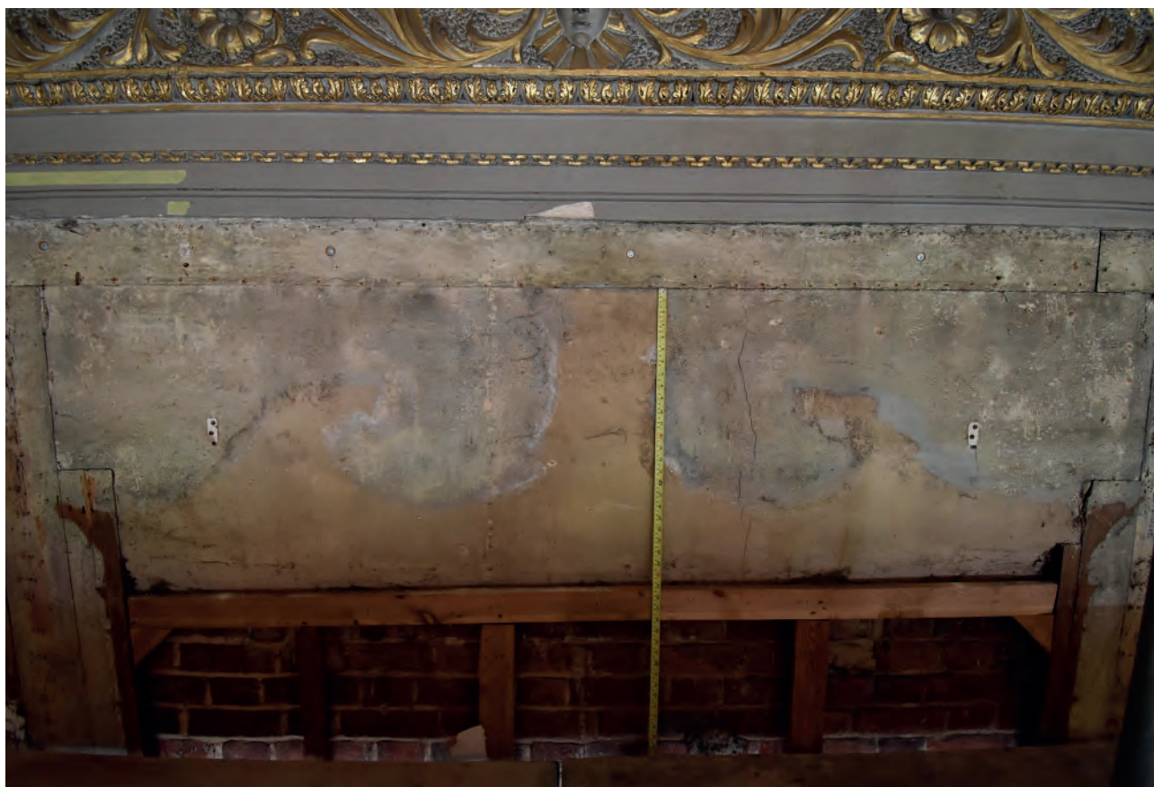
Plate 29: North wall, west crown of overmantel, greenish lime plaster
