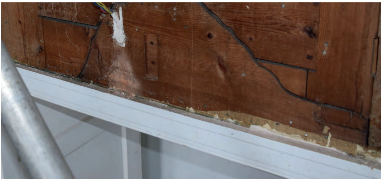
Plate 115: North wall, lower part of reused door, remnants of a green jute cloth
