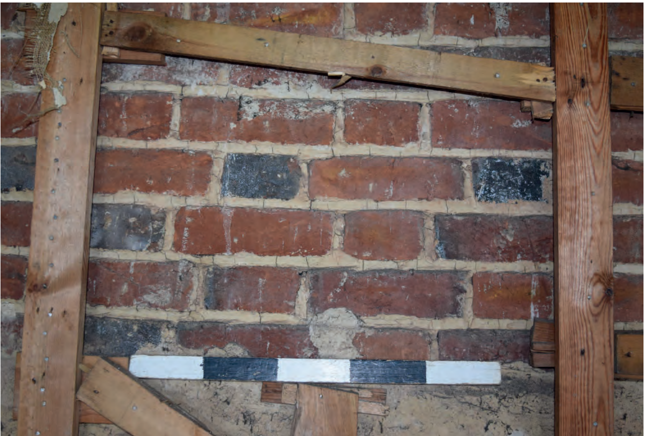
Plate 12: North wall, west overmantel, example of brickwork
