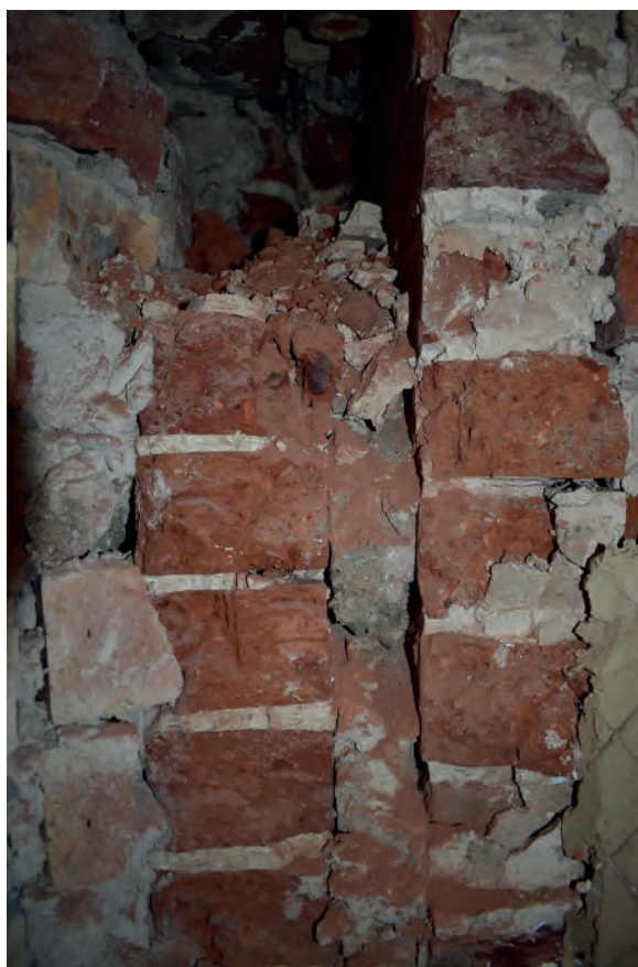
Plate 133: North wall, east part of east fireplace, development phases, Victorian period
