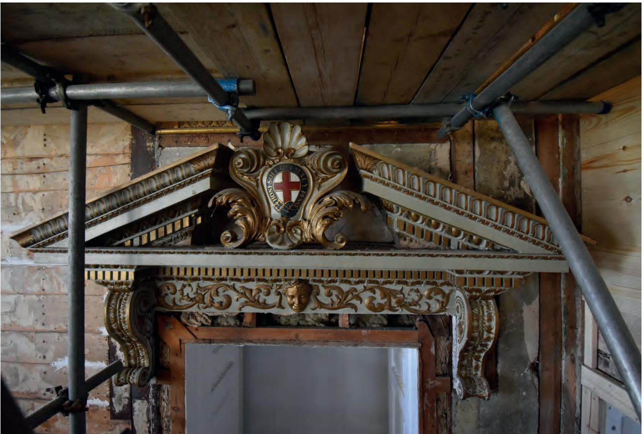
Plate 31: West wall, north door pediment
