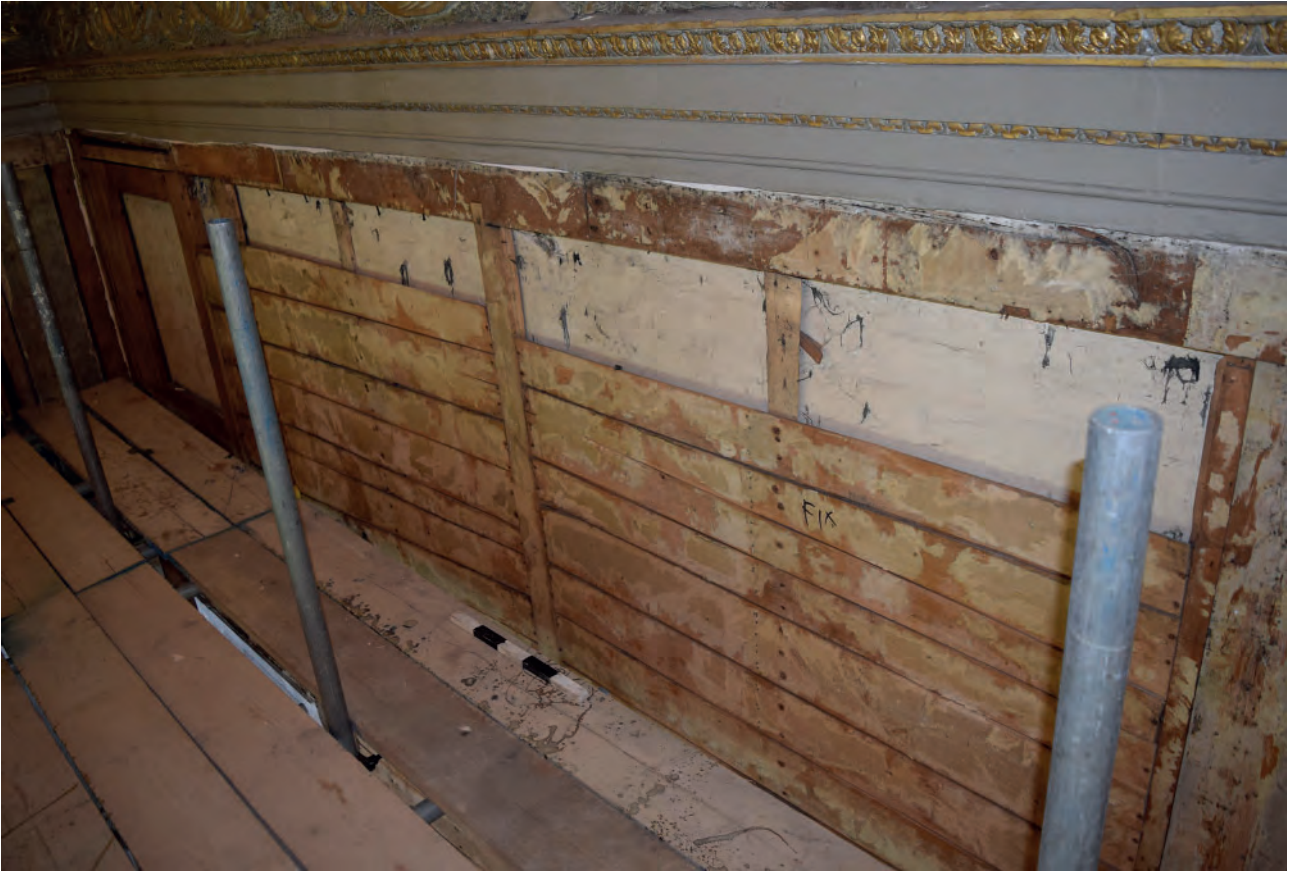
Plate 15: North wall, lime plaster behind sarking boards
