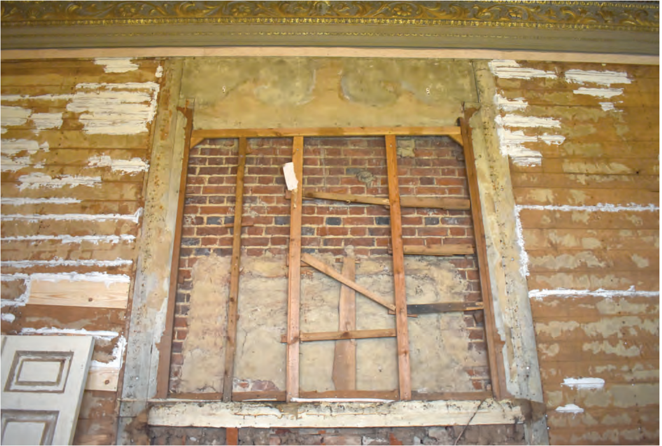
Plate 17: North wall, lime plaster behind west overmantel
