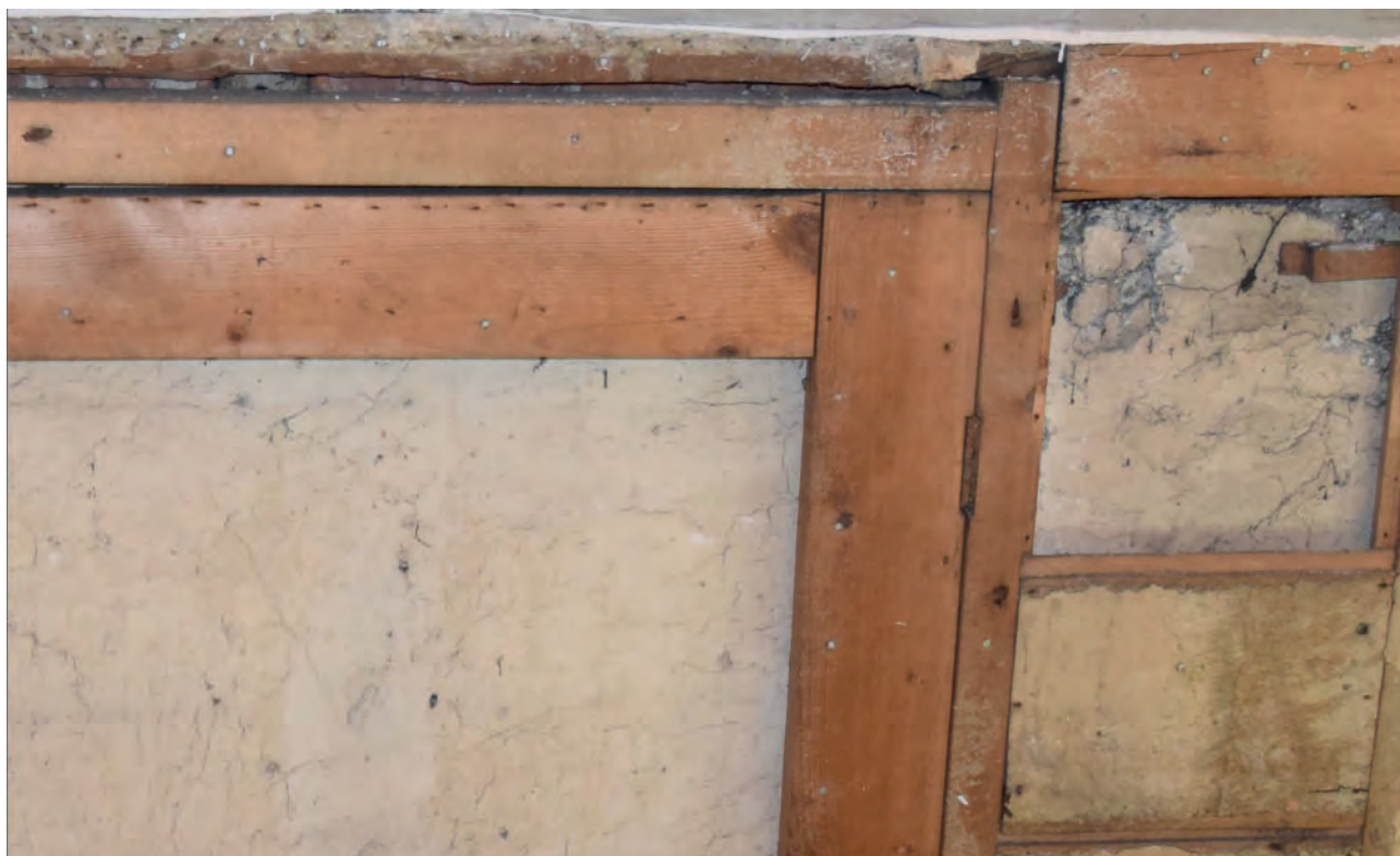
Plate 112: North wall, upper part of reused door, masked place of removal of upper hinge
