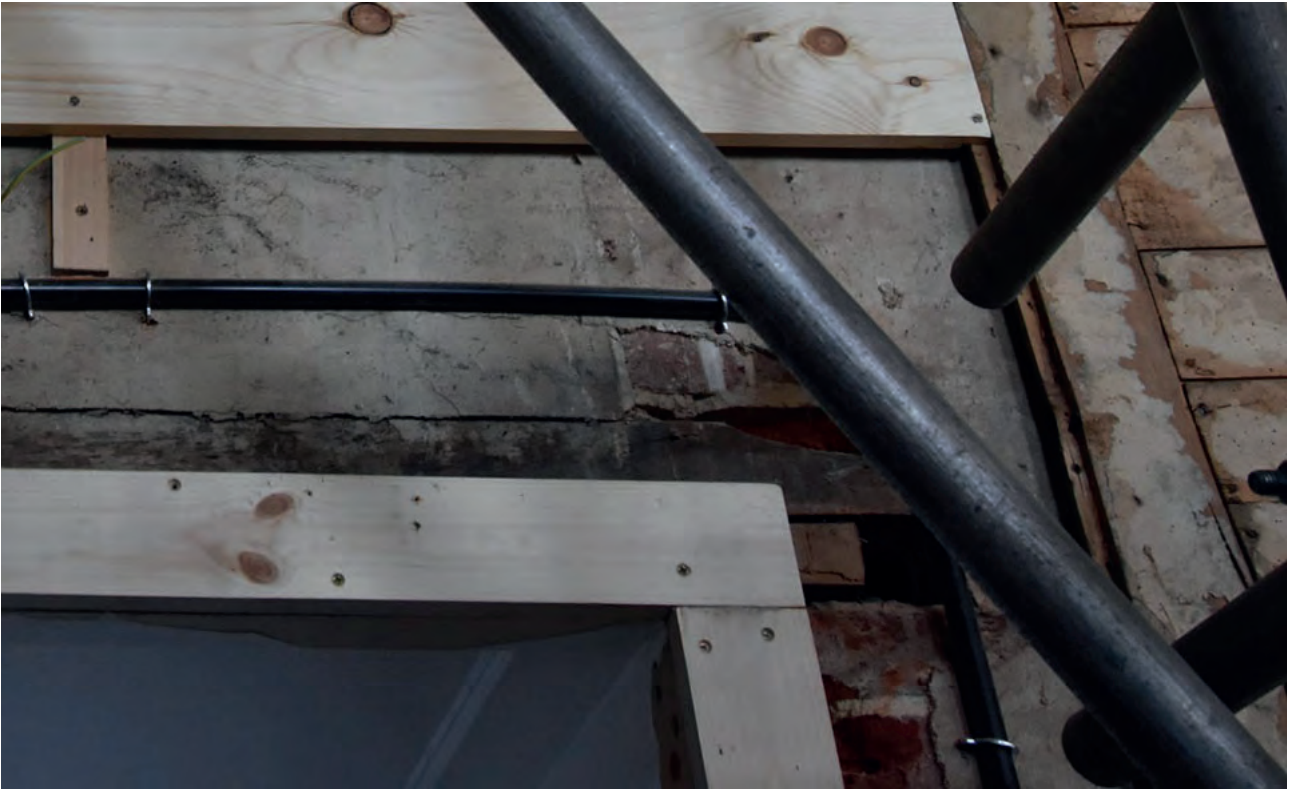
Plate 42: North wall, west door, timber lintel
