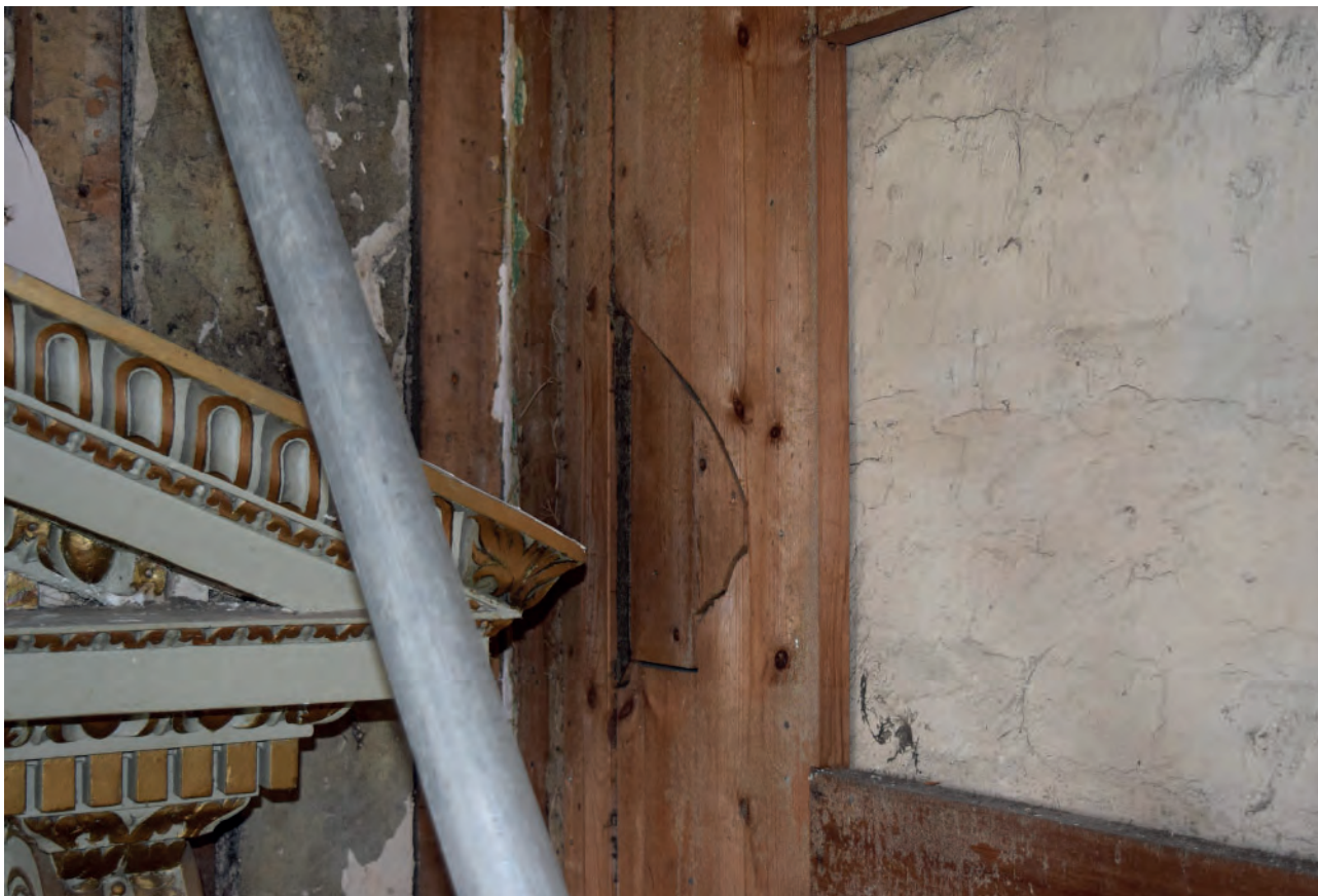
Plate 114: North wall, lower part of reused door, irregular shape cut
