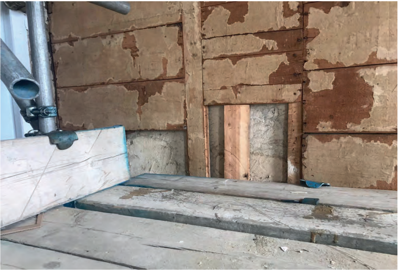
Plate 21: East wall, lime plaster behind sarking boards
