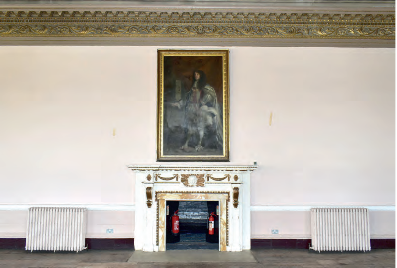
Plate 7: Example of a later fireplace
