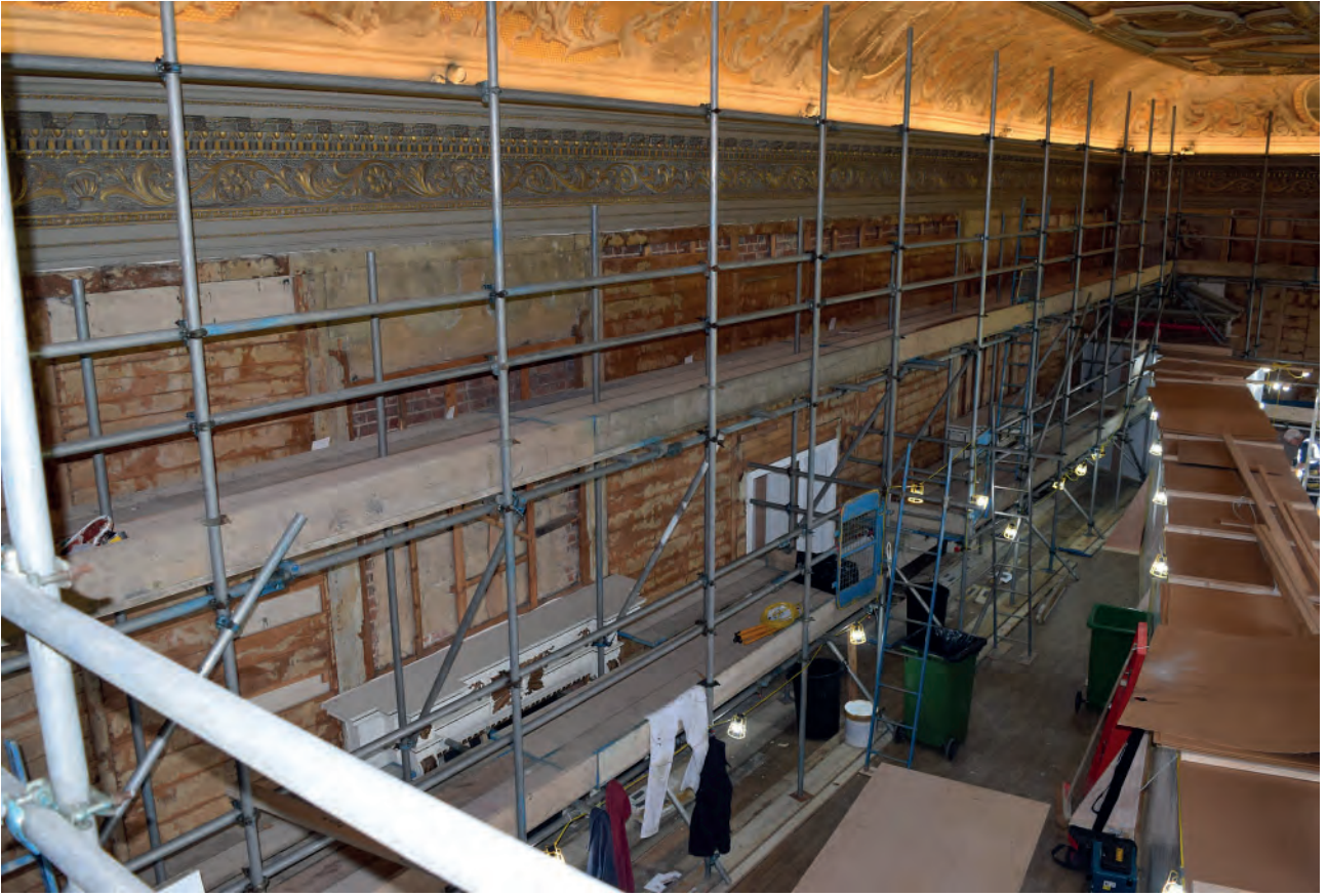
Plate 48: North wall, sarking boards
