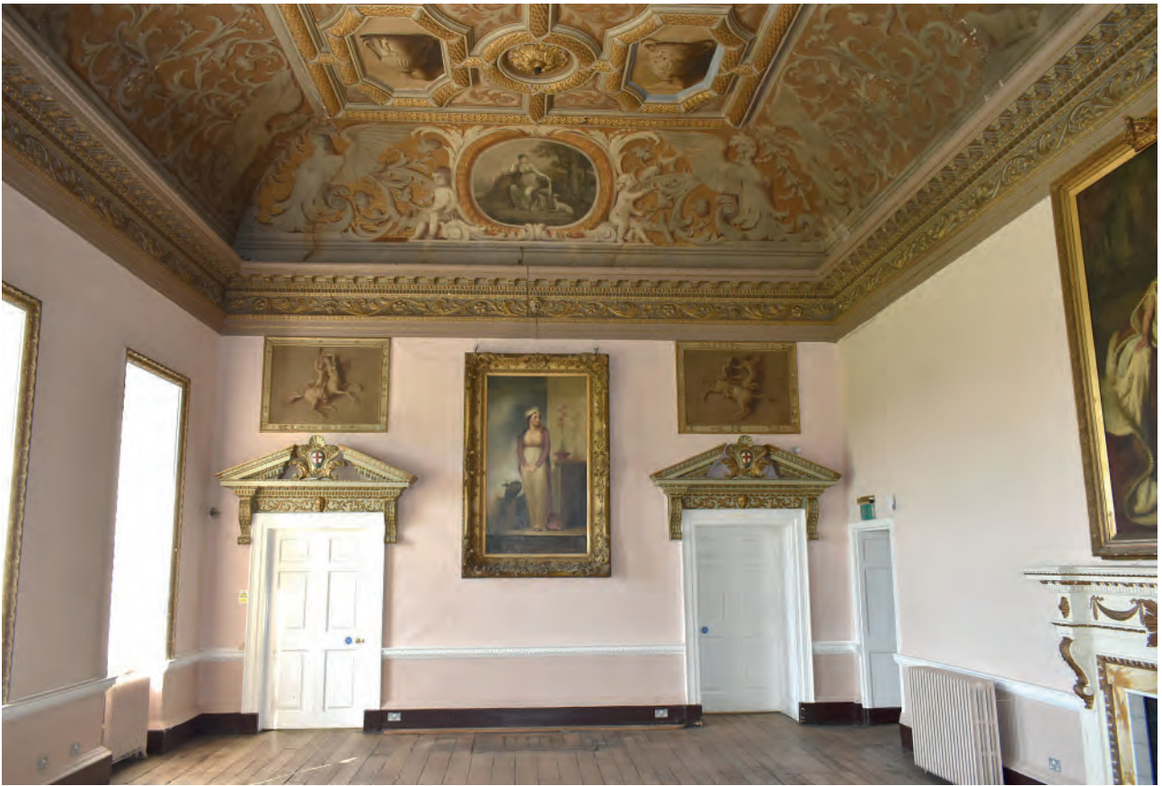
Plate 3: West wall, at the start of the project
