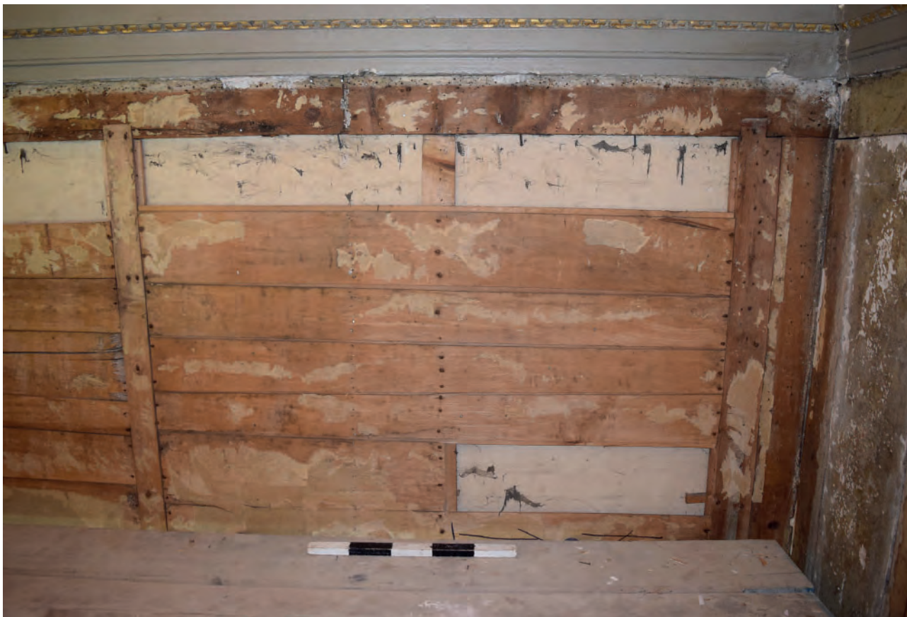
Plate 13: North wall, lime plaster behind sarking boards
