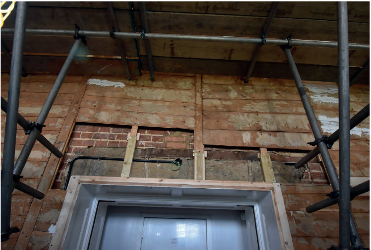
Plate 39: North wall, middle door, concrete lintel
