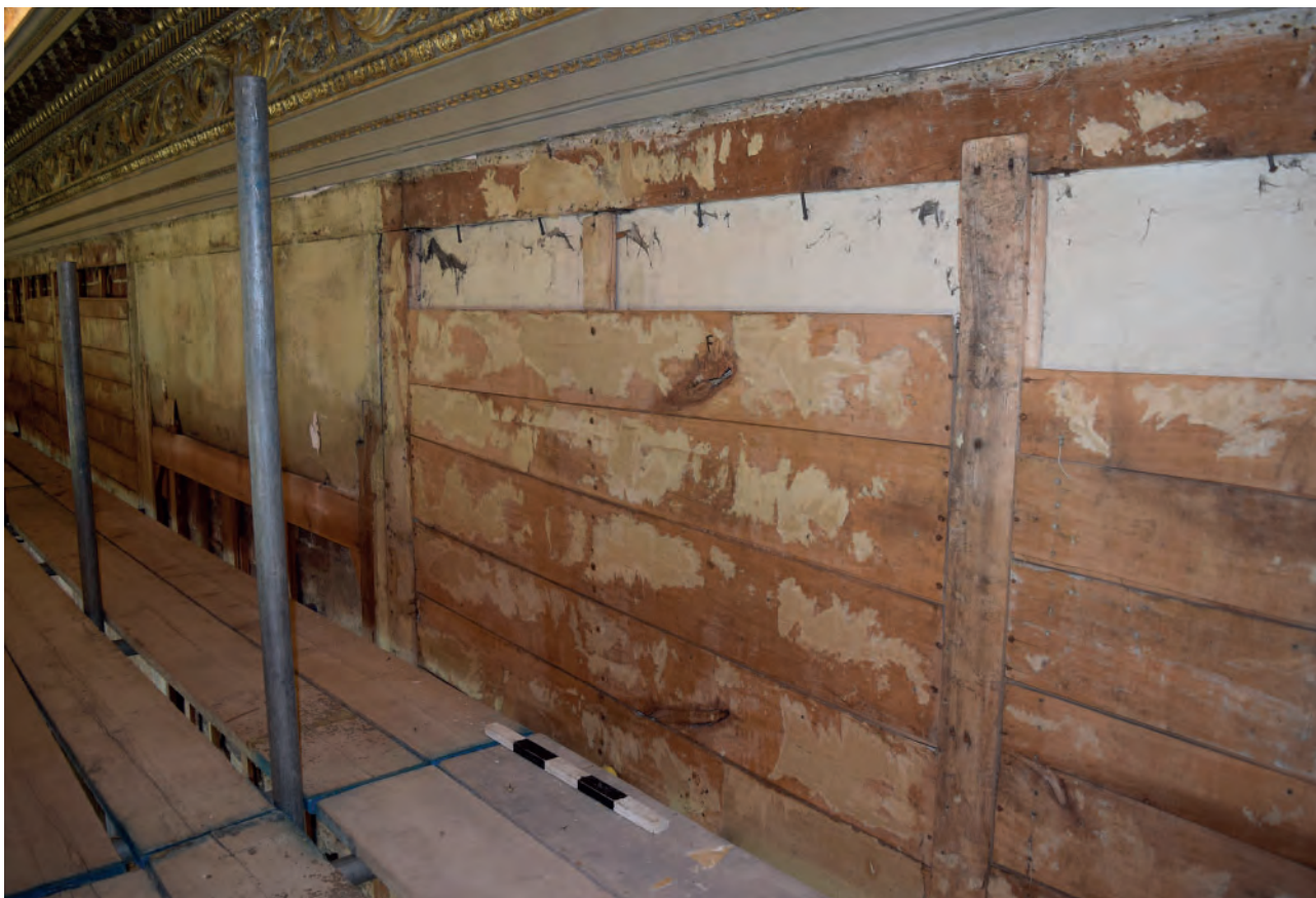
Plate 14: North wall, lime plaster behind sarking boards
