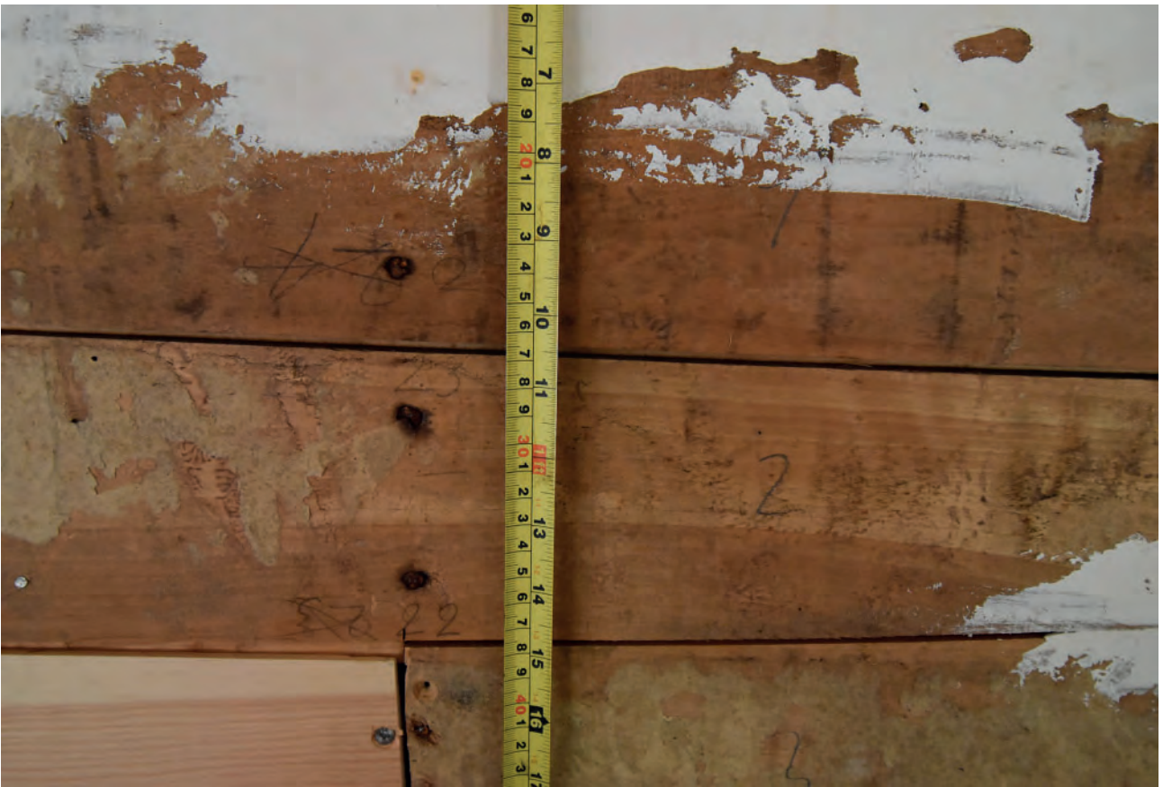
Plate 89: North wall, panel 8, example of second and third type of numbering
