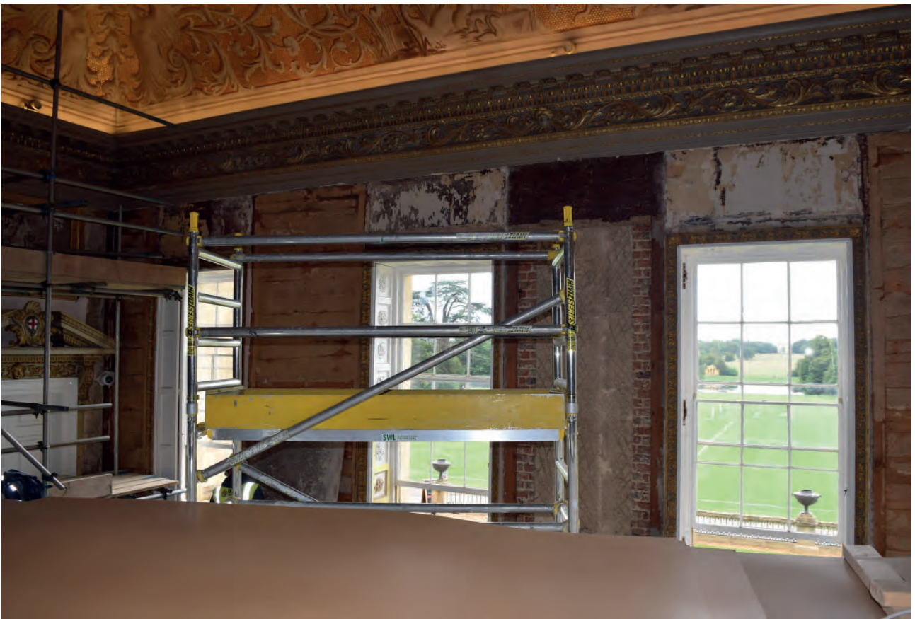
Plate 47: South wall, sarking boards
