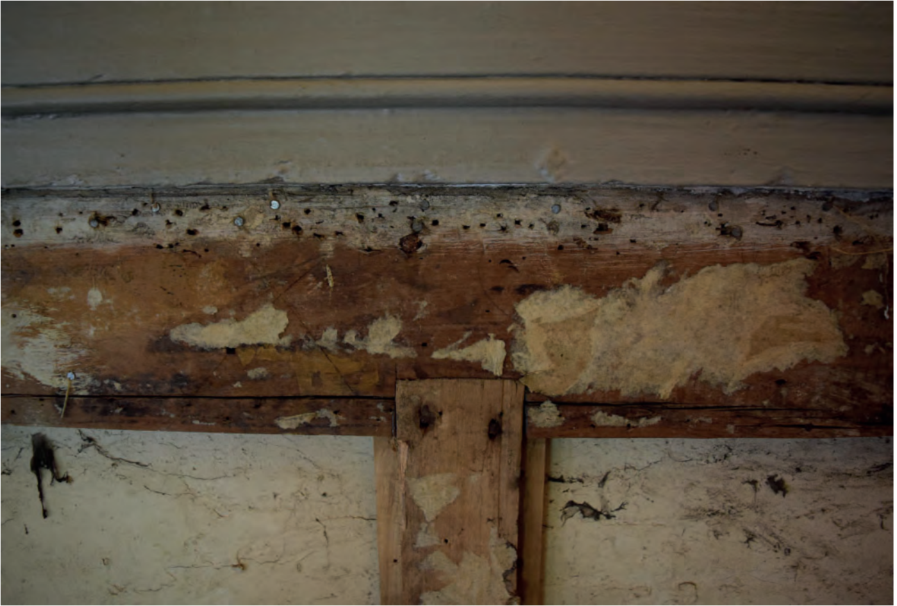
Plate 52: North wall, carpentry joints
