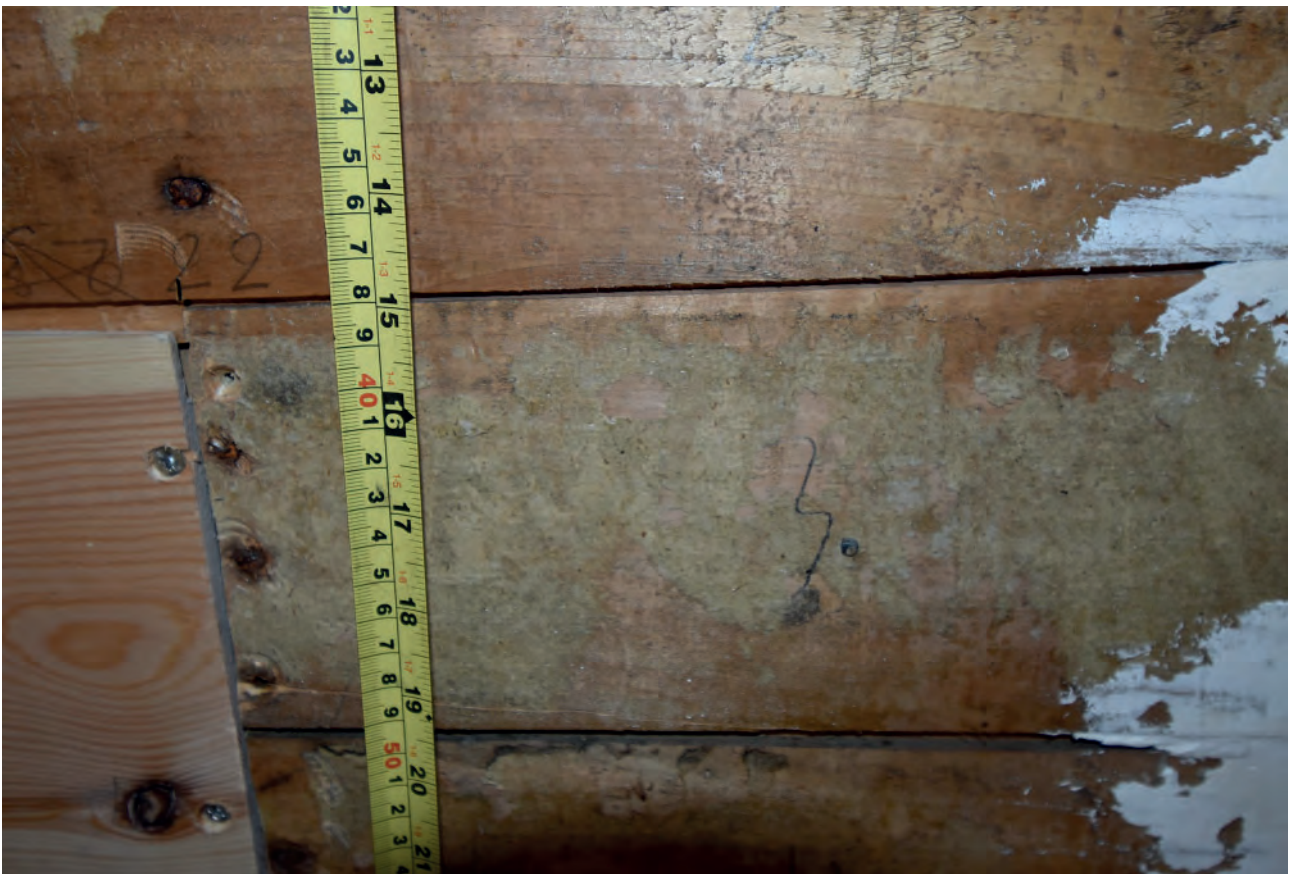
Plate 90: North wall, panel 8, example of second type of numbering
