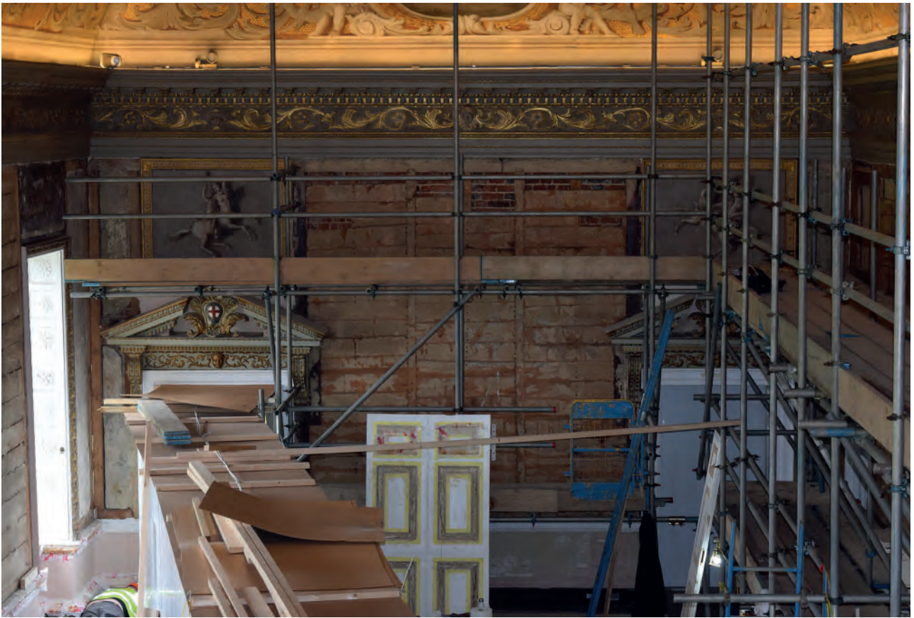
Plate 44: West wall, sarking boards
