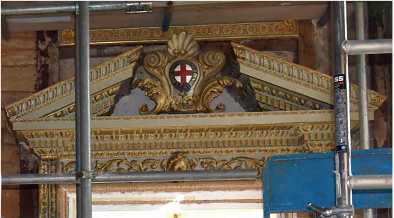
Plate 34: East wall, south door pediment
