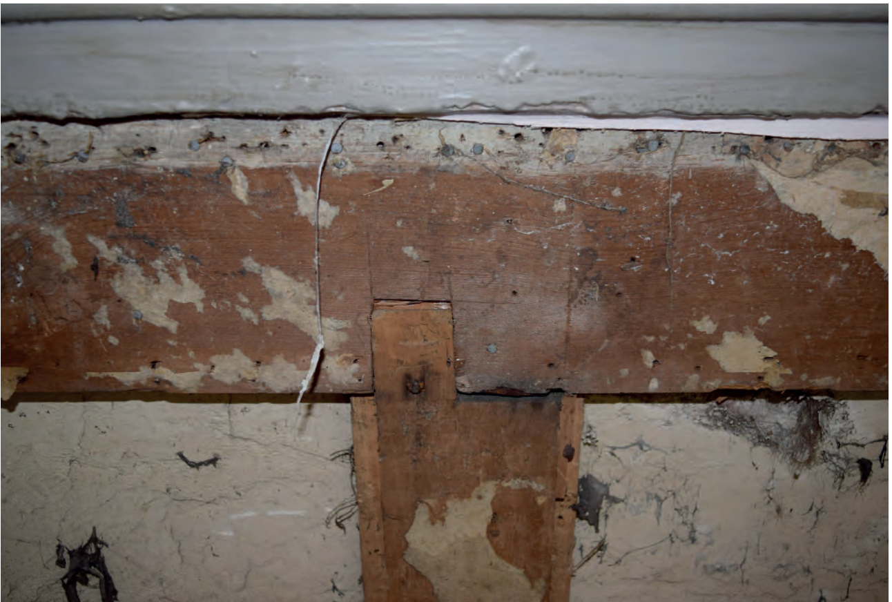
Plate 109: North wall, original frame, exemplar of carpenter's mark
