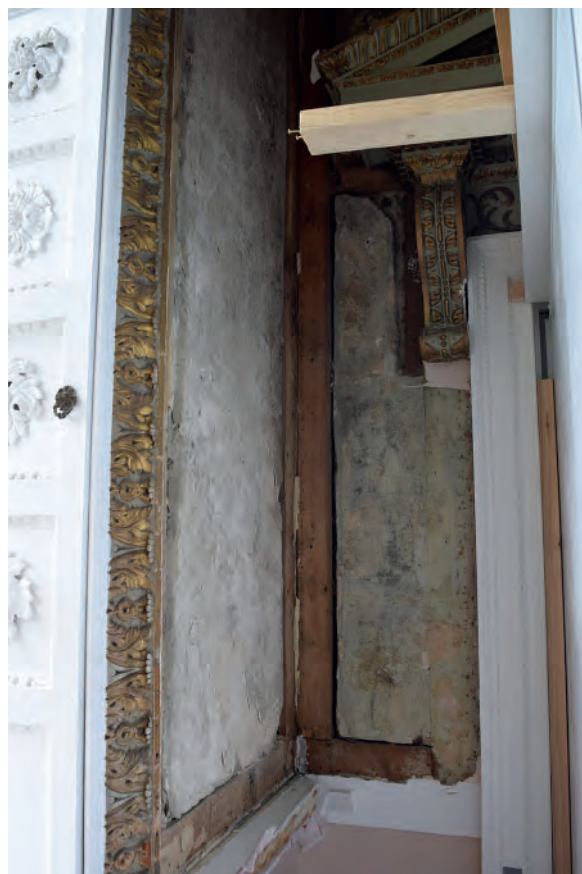
Plate 28: South and west walls, south corner, greenish lime plaster
