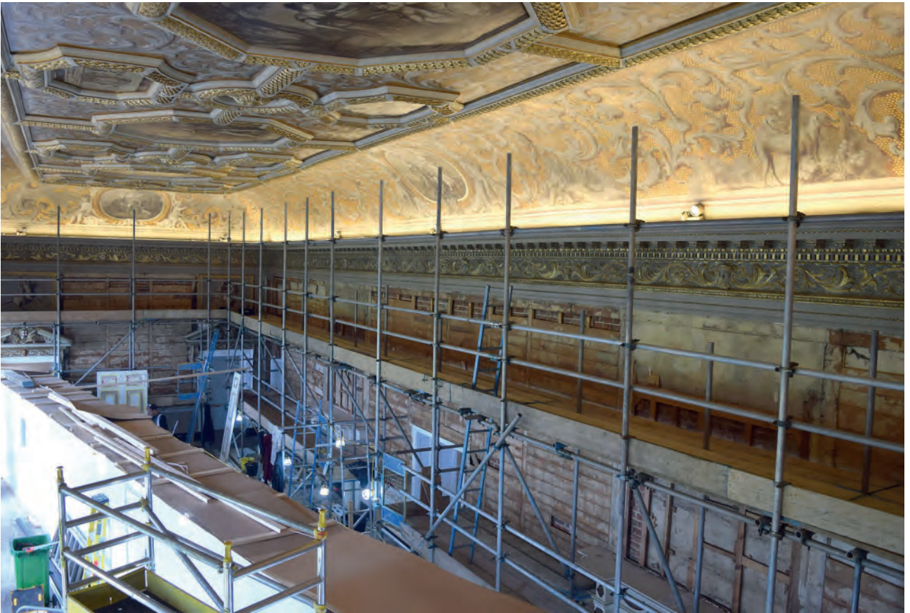
Plate 49: North wall, sarking boards
