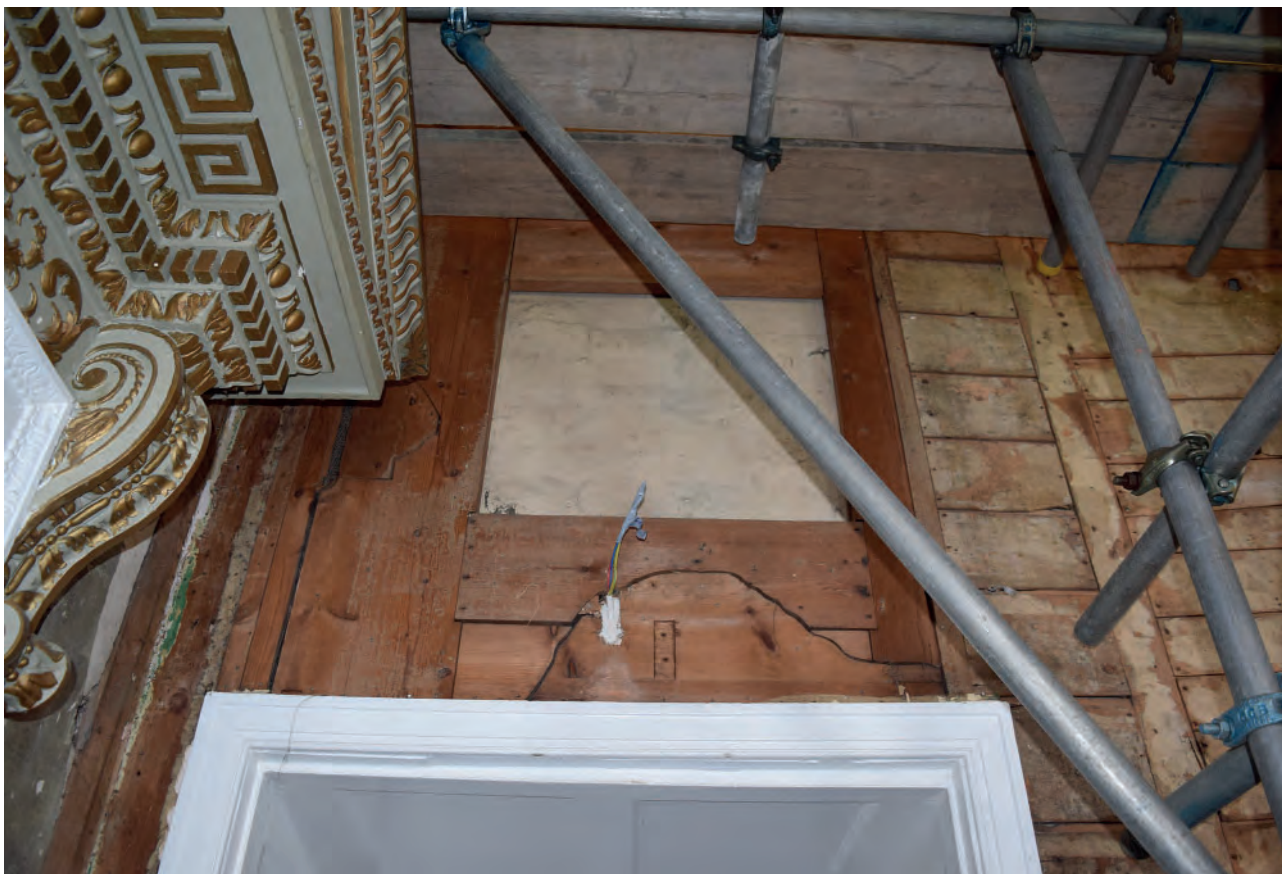
Plate 111: North wall, lower part of reused door
