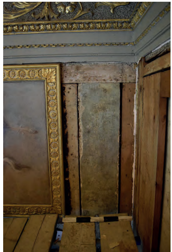
Plate 25: West wall, north corner, greenish lime plaster
