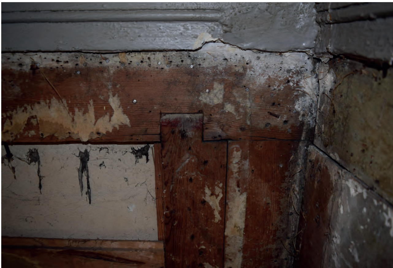
Plate 51: North wall, carpentry joints
