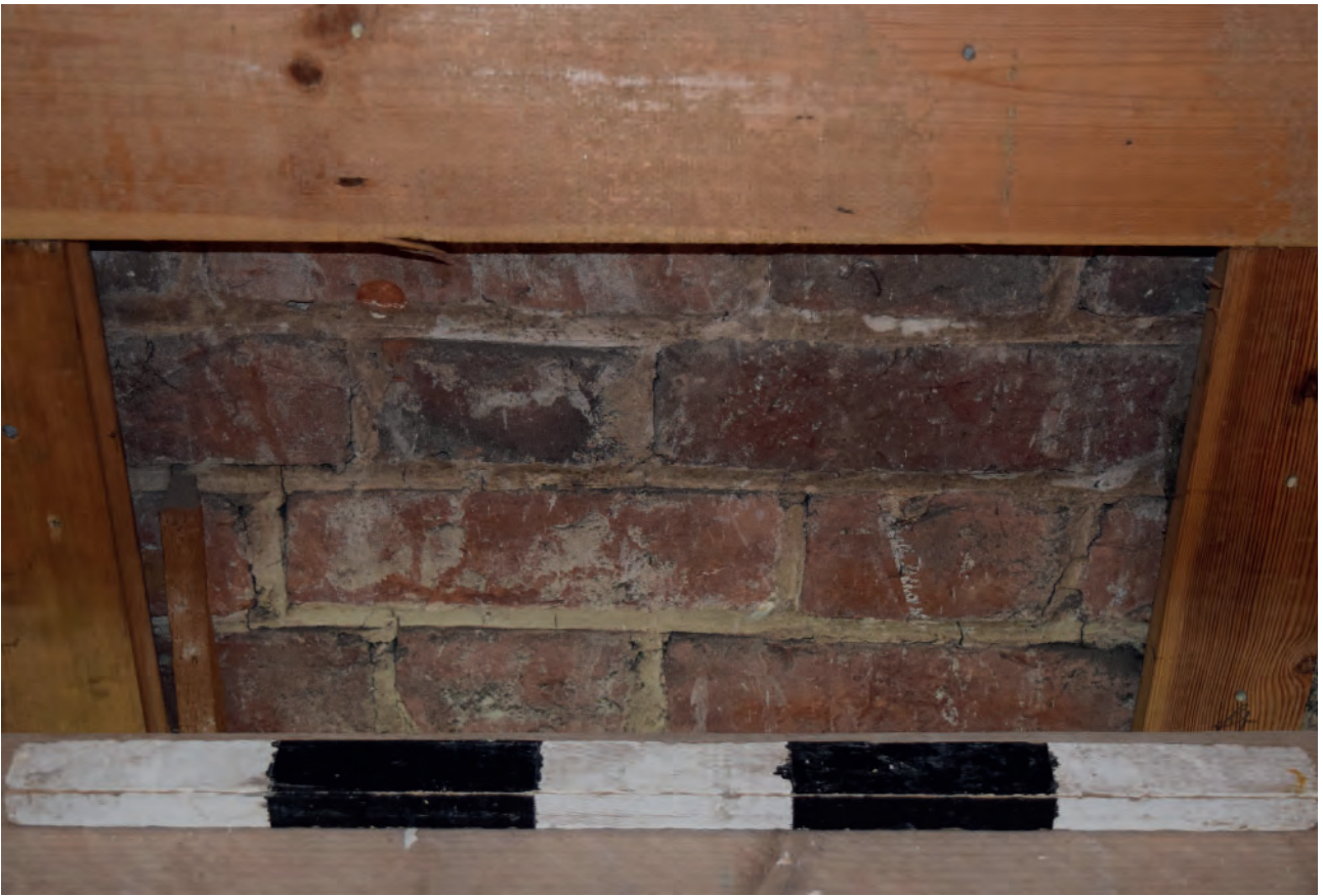
Plate 11: North wall, example of brickwork
