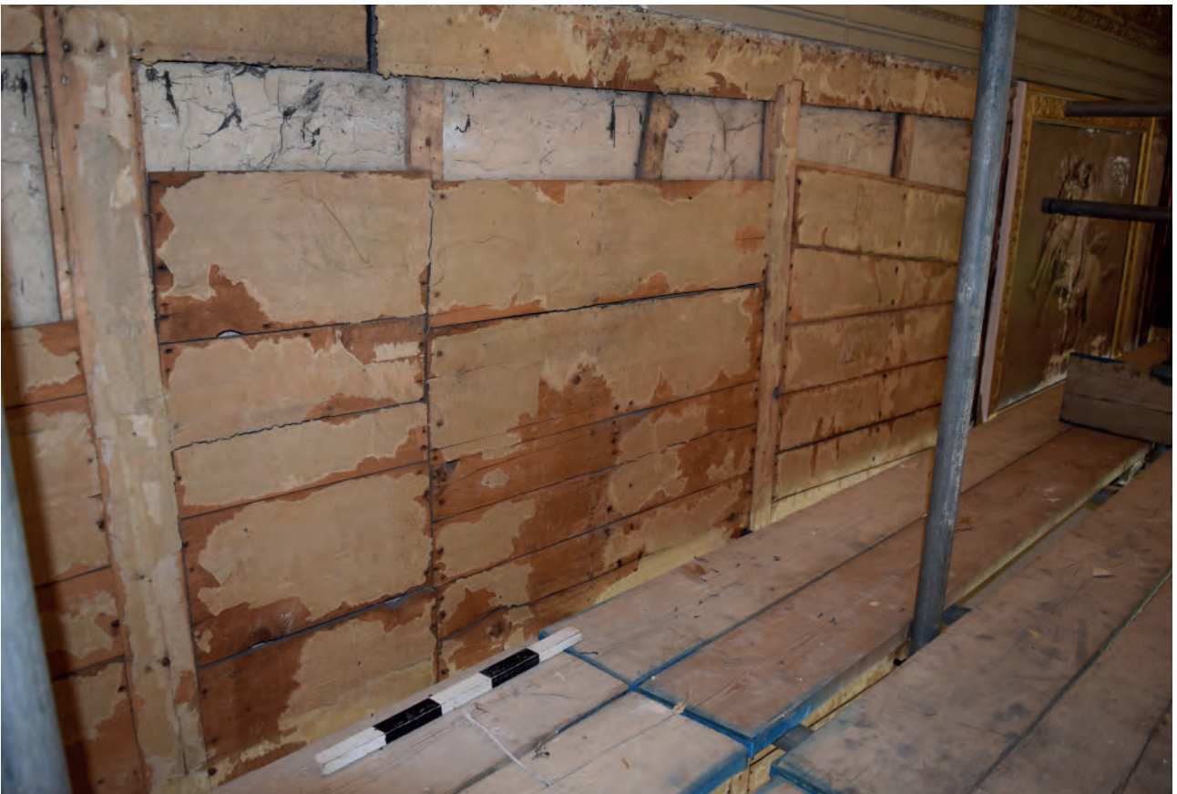
Plate 20: East wall, lime plaster behind sarking boards
