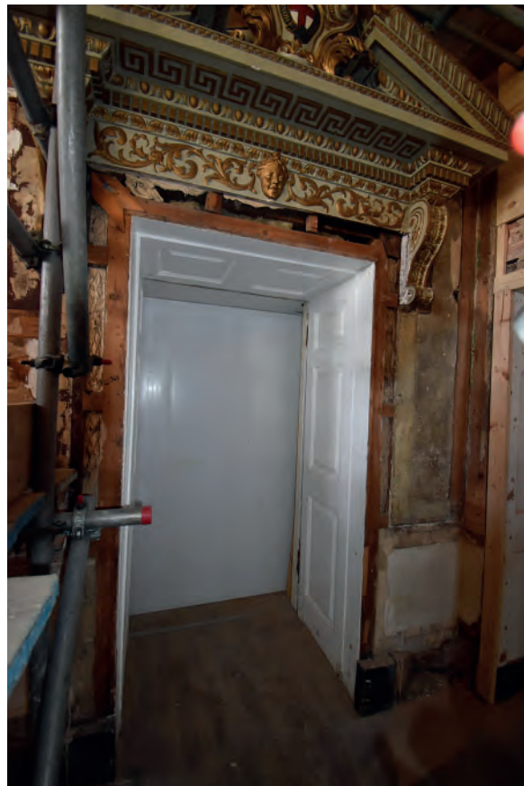
Plate 155: West wall, north door frame
