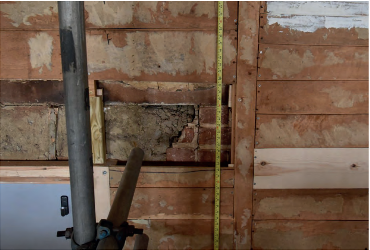
Plate 40: North wall, middle door, timber lintel
