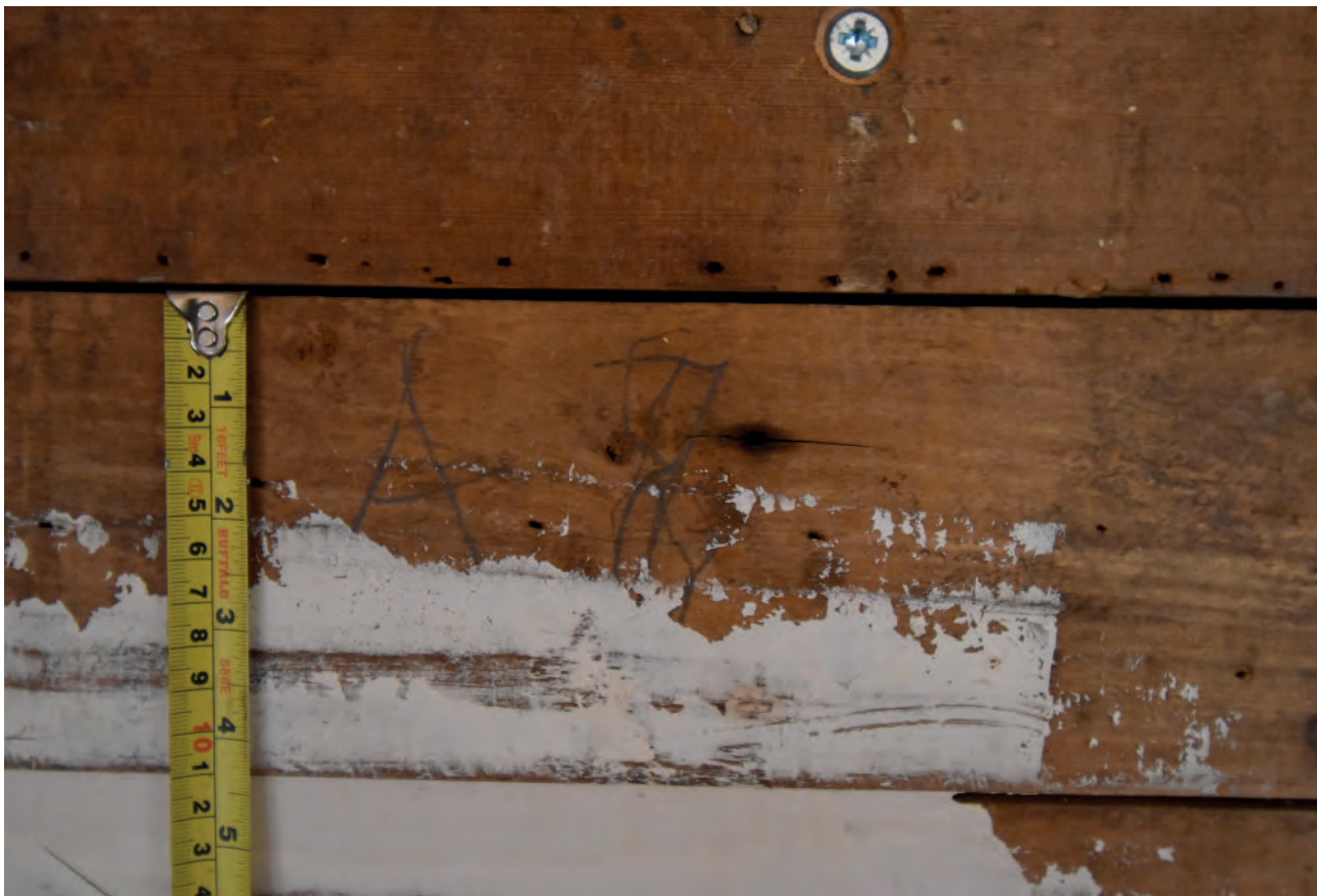
Plate 74: North wall, panel 5, example of first type of numbering
