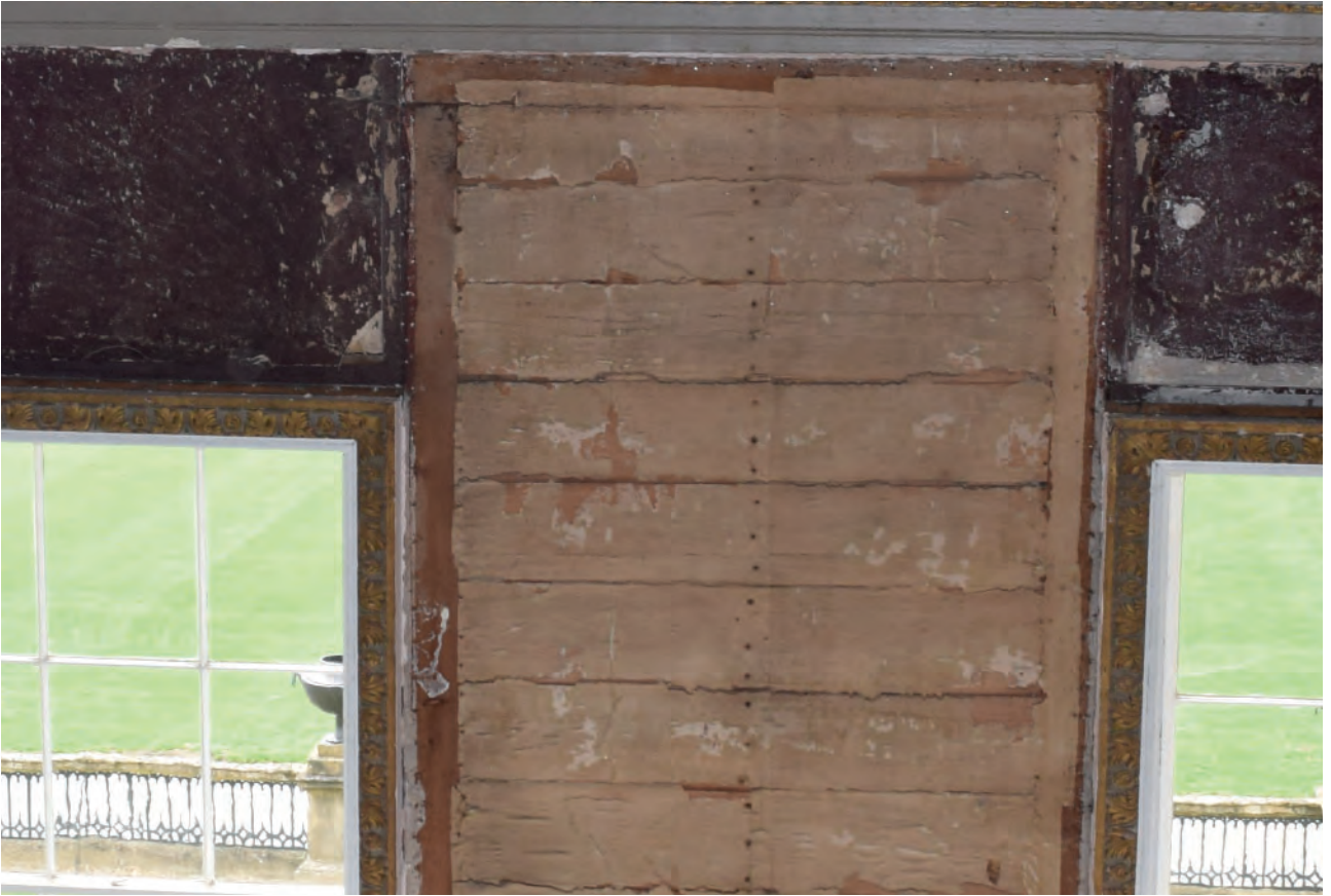
Plate 36: South wall, original plaster over windows
