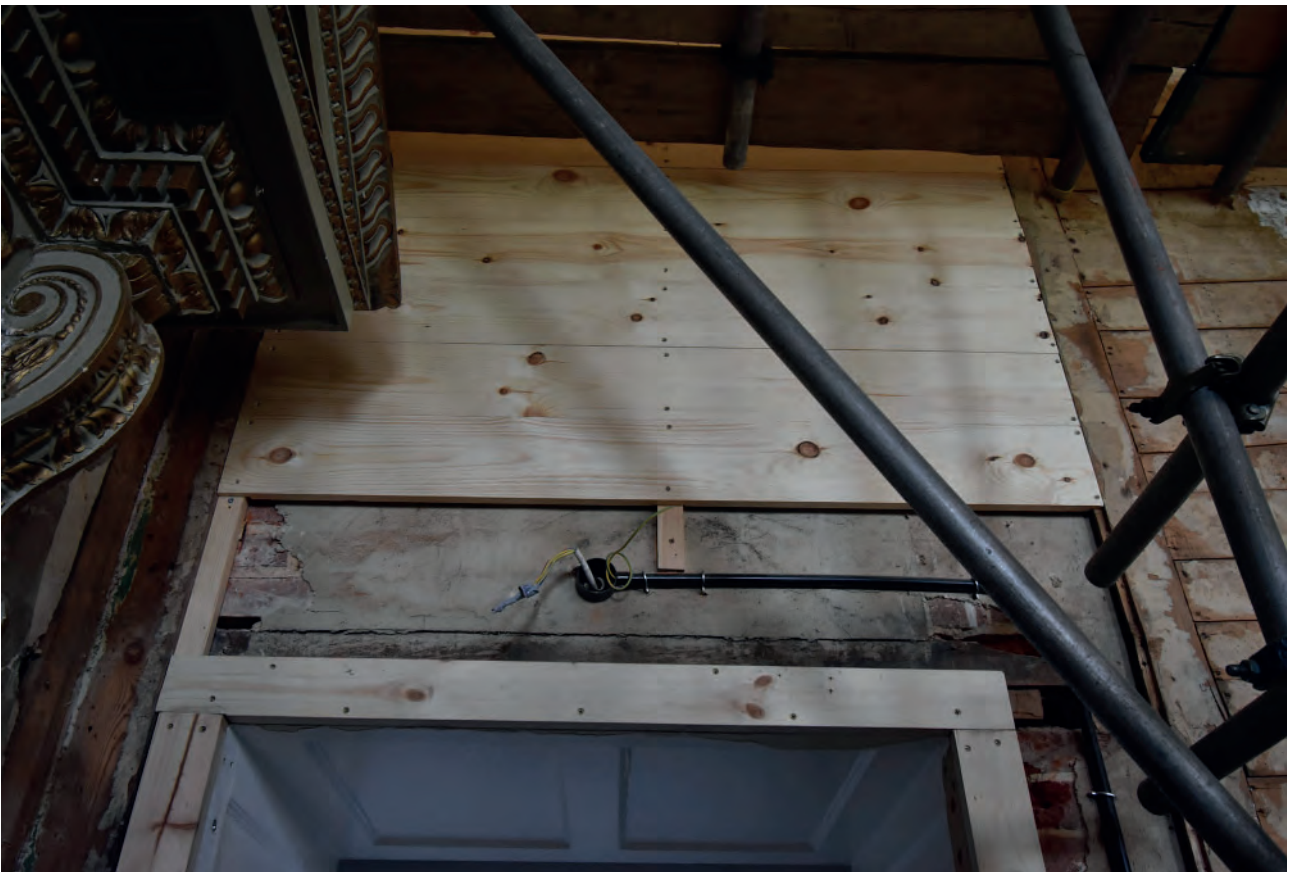
Plate 41: North wall, west door, timber lintel
