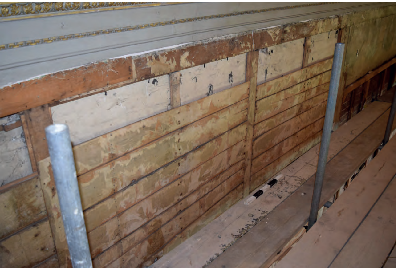
Plate 16: North wall, lime plaster behind sarking boards
