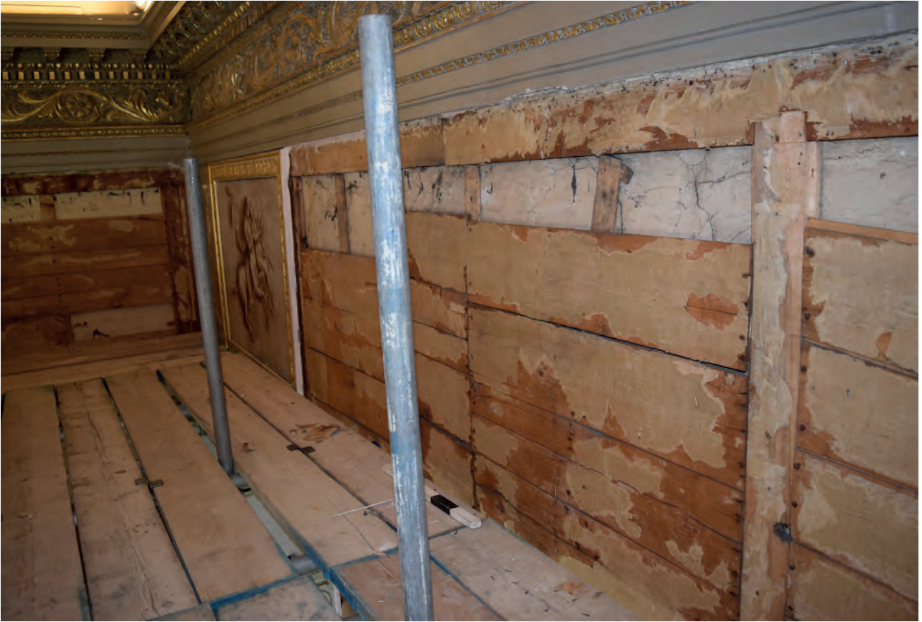
Plate 19: East wall, lime plaster behind sarking boards
