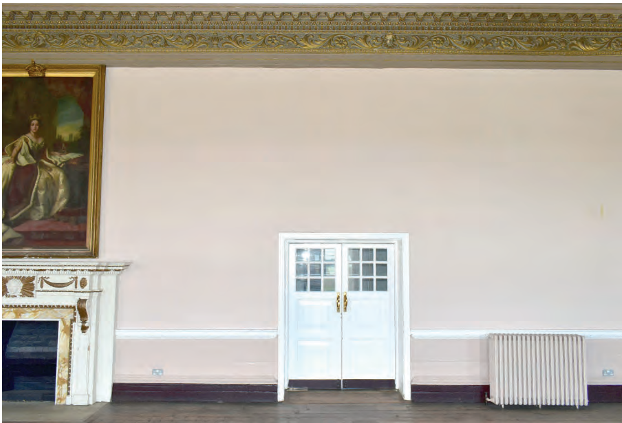
Plate 1: North wall, example of an early 20th-century doorway
