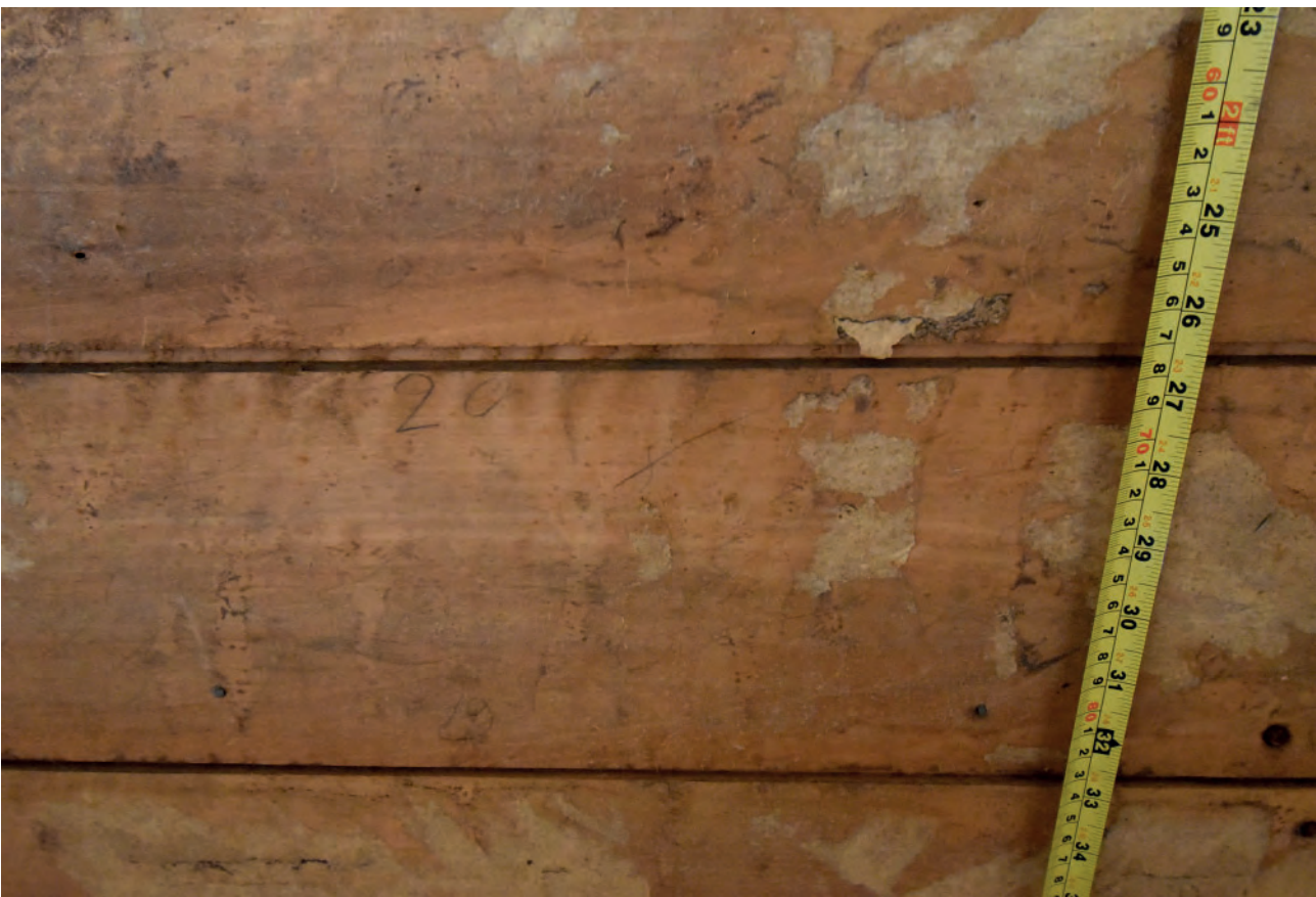
Plate 93: North wall, panel 9, example of second type of numbering
