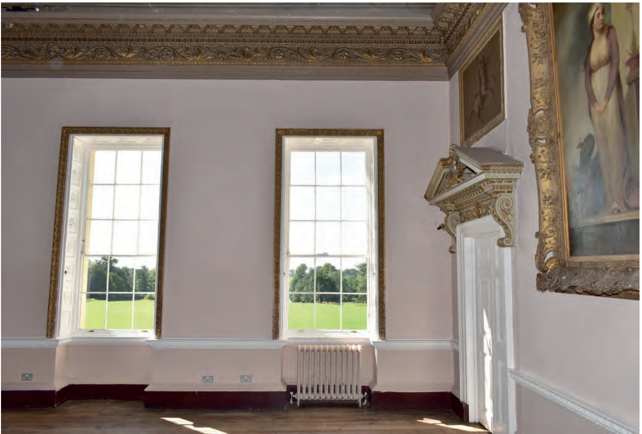
Plate 4: South wall, example of windows at the start of the project
