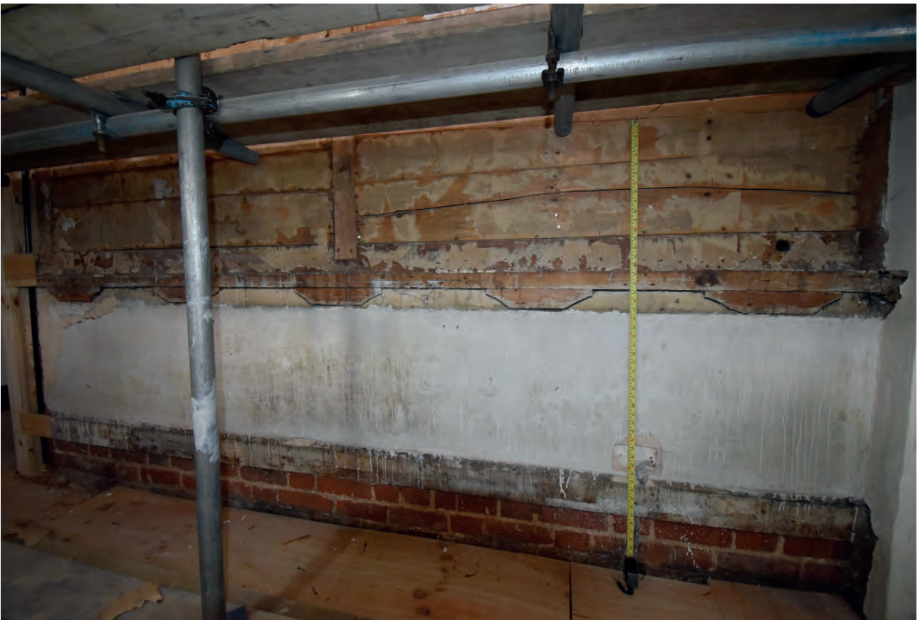
Plate 117: North wall, dado between west door and west fireplace
