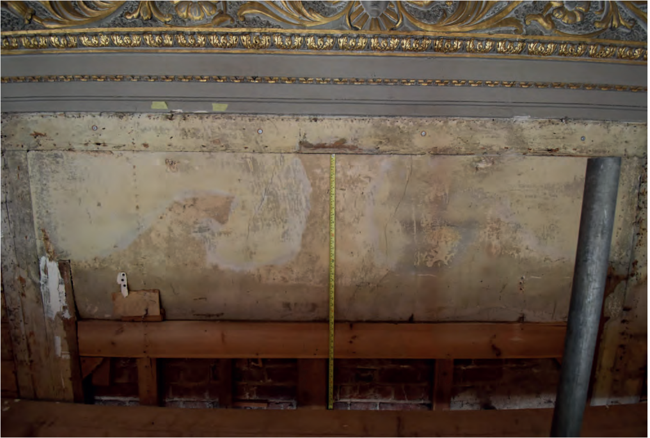
Plate 30: North wall, east crown of overmantel, greenish lime plaster
