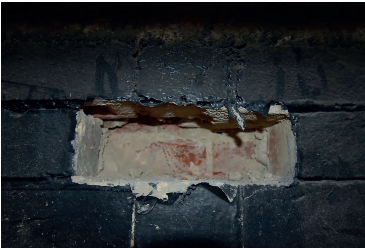
Plate 126: North wall, east fireplace, Gregorian brick behind brick from 1920s fireplace
