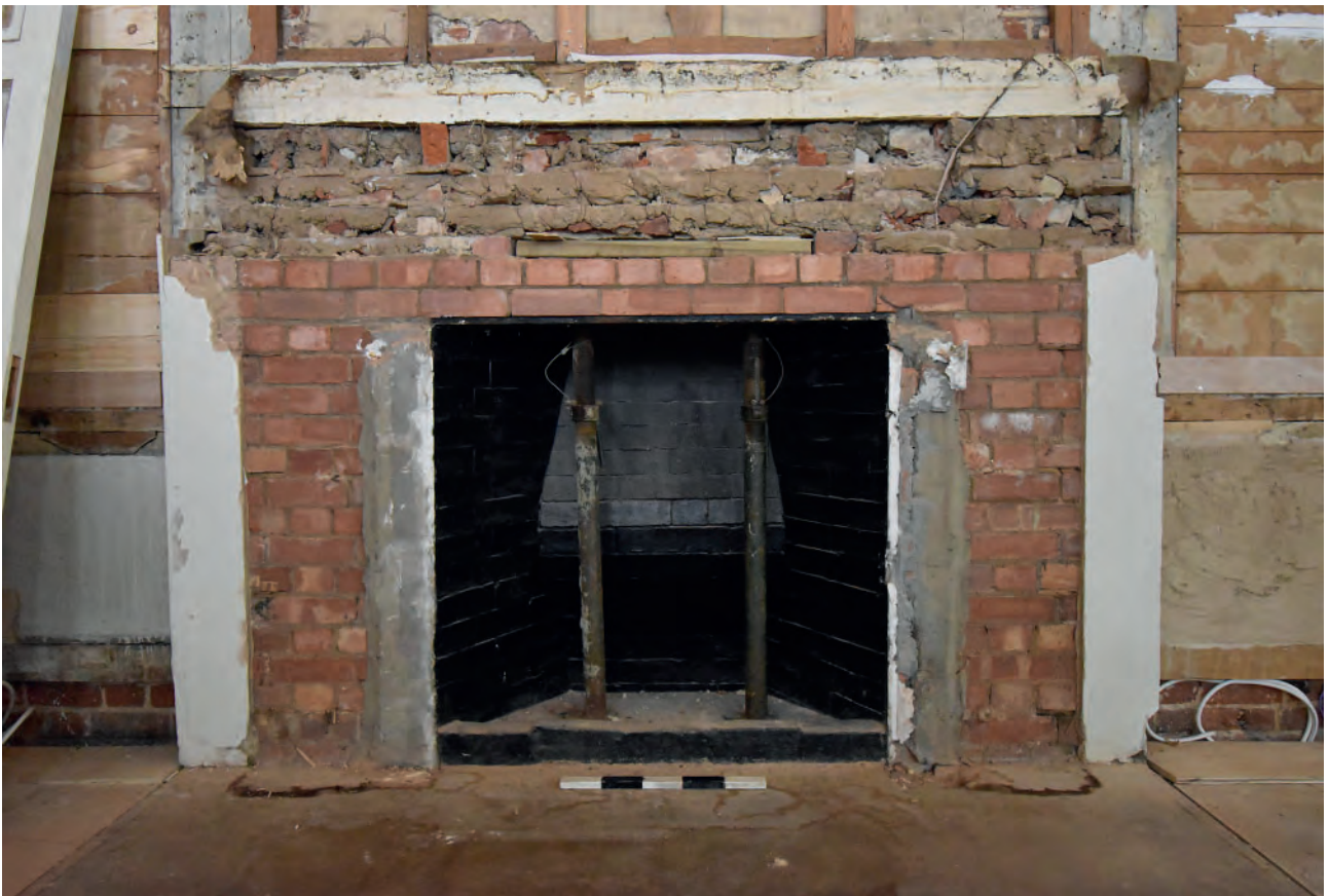
Plate 123: North wall, west fireplace
