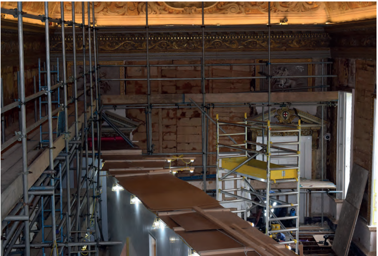
Plate 45: East wall, sarking boards
