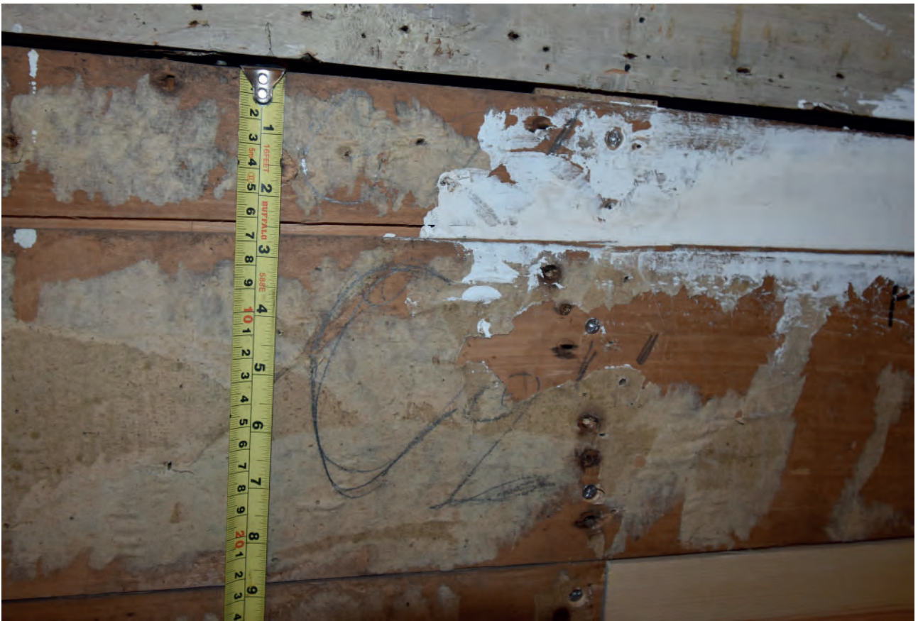
Plate 79: West wall, panel 2, example of first type of numbering
