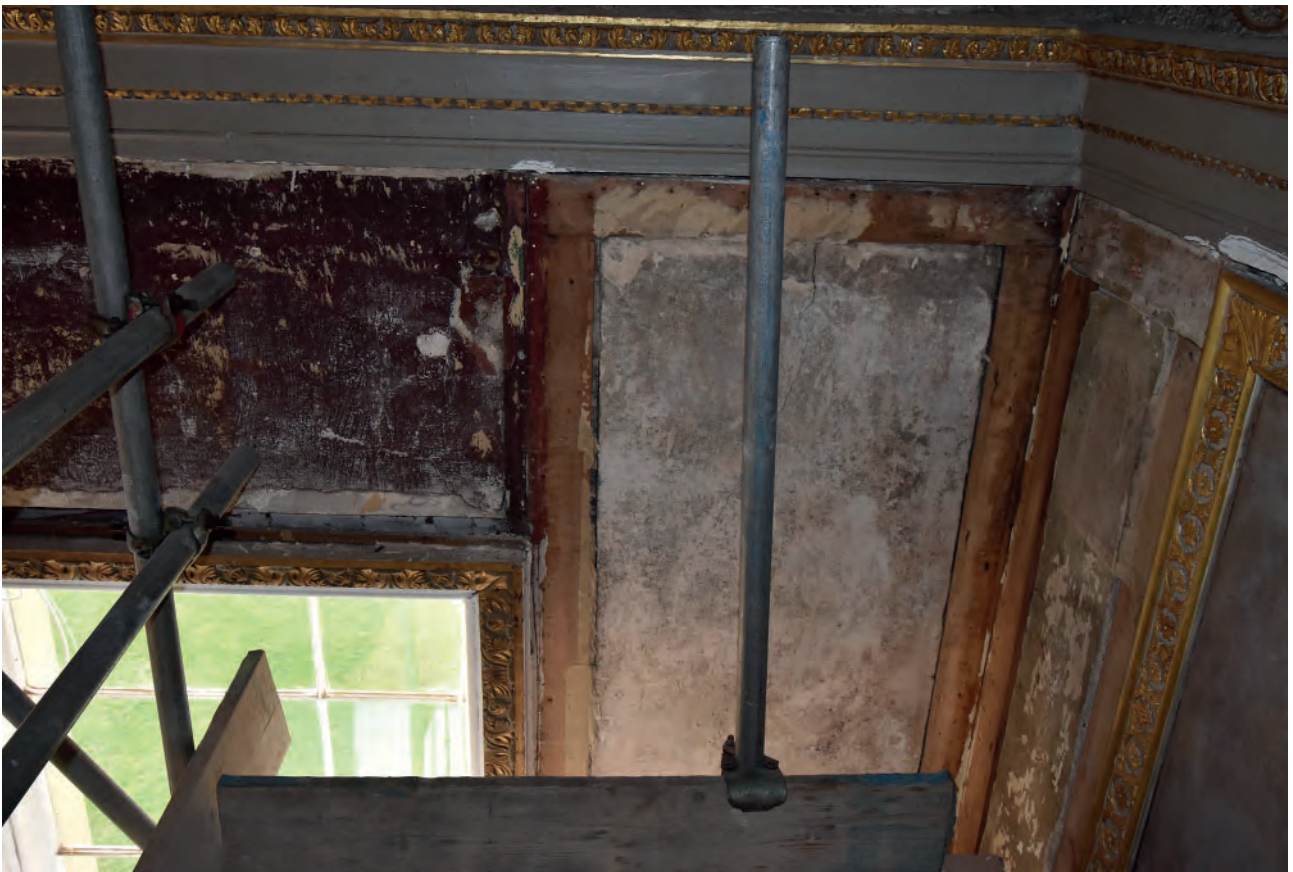
Plate 27: South and west walls, south corner, greenish lime plaster
