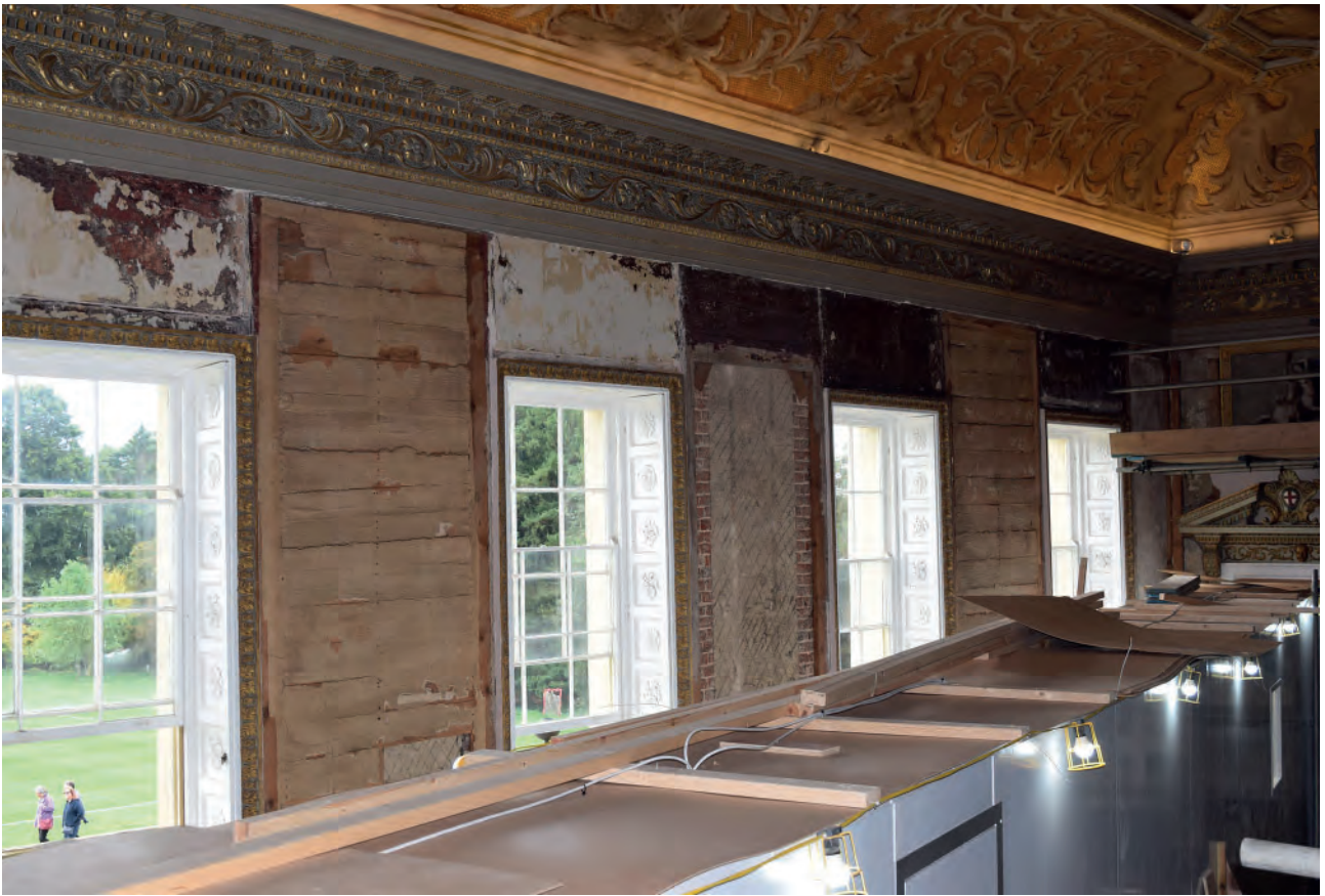
Plate 46: South wall, sarking boards
