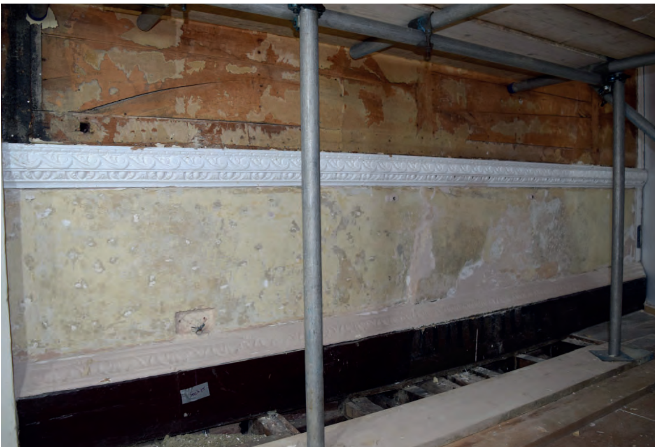
Plate 119: North wall, dado between east fireplace and east door
