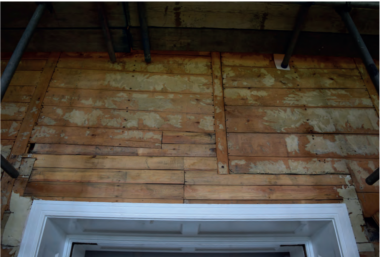
Plate 43: North wall, middle door, replaced sarking boards
