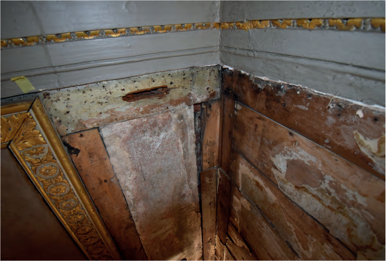
Plate 23: East wall, south corner, greenish lime plaster
