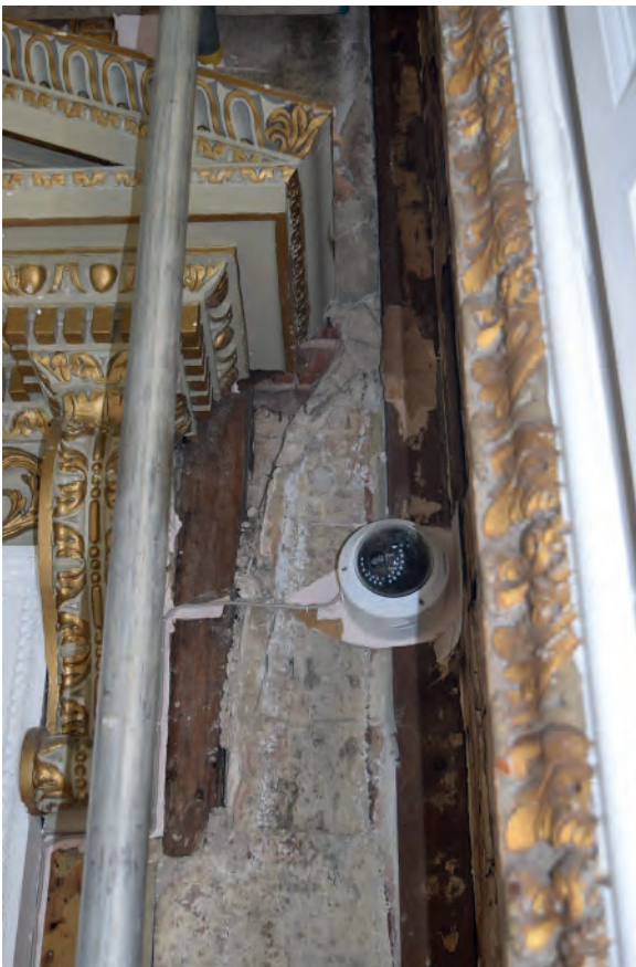
Plate 24: East wall, south corner, greenish lime plaster
