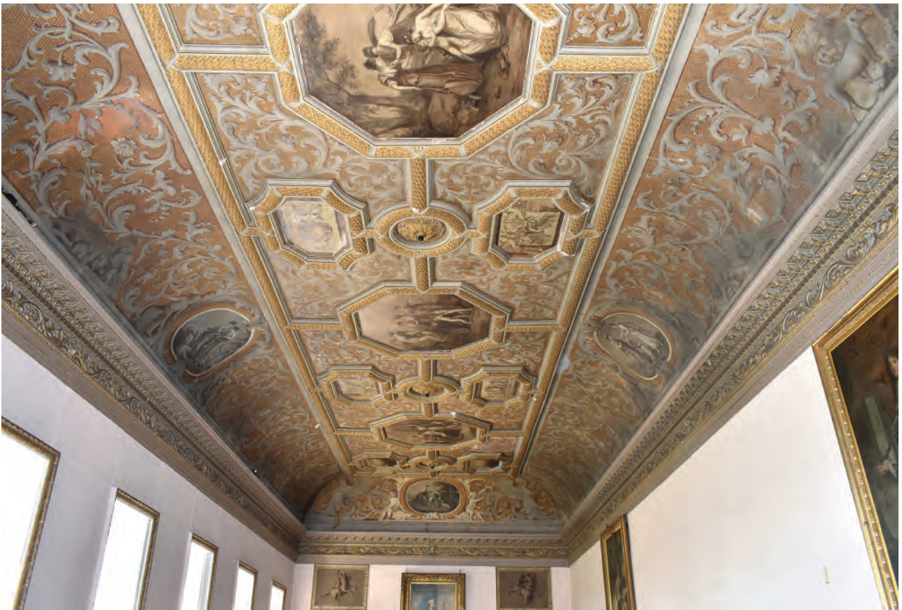
Plate 10: Ceiling, before conservation work, looking west
