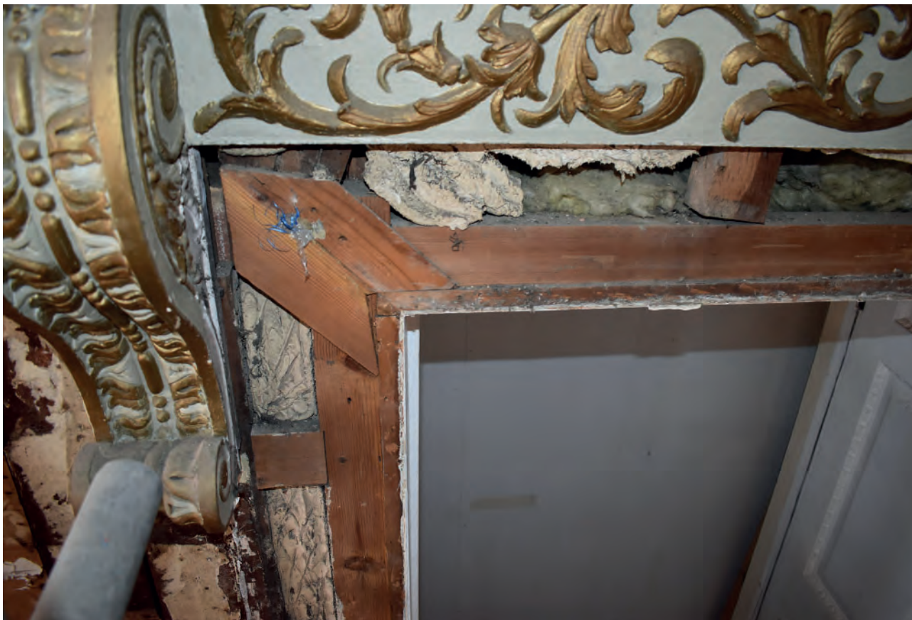
Plate 156: West wall, north door frame
