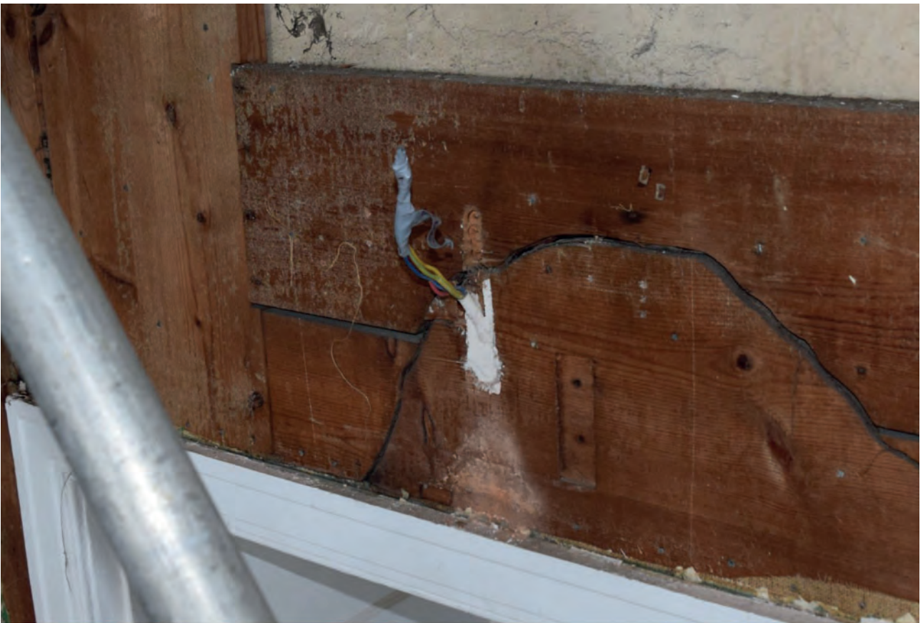
Plate 57: North wall, panel 1, example of graffiti
