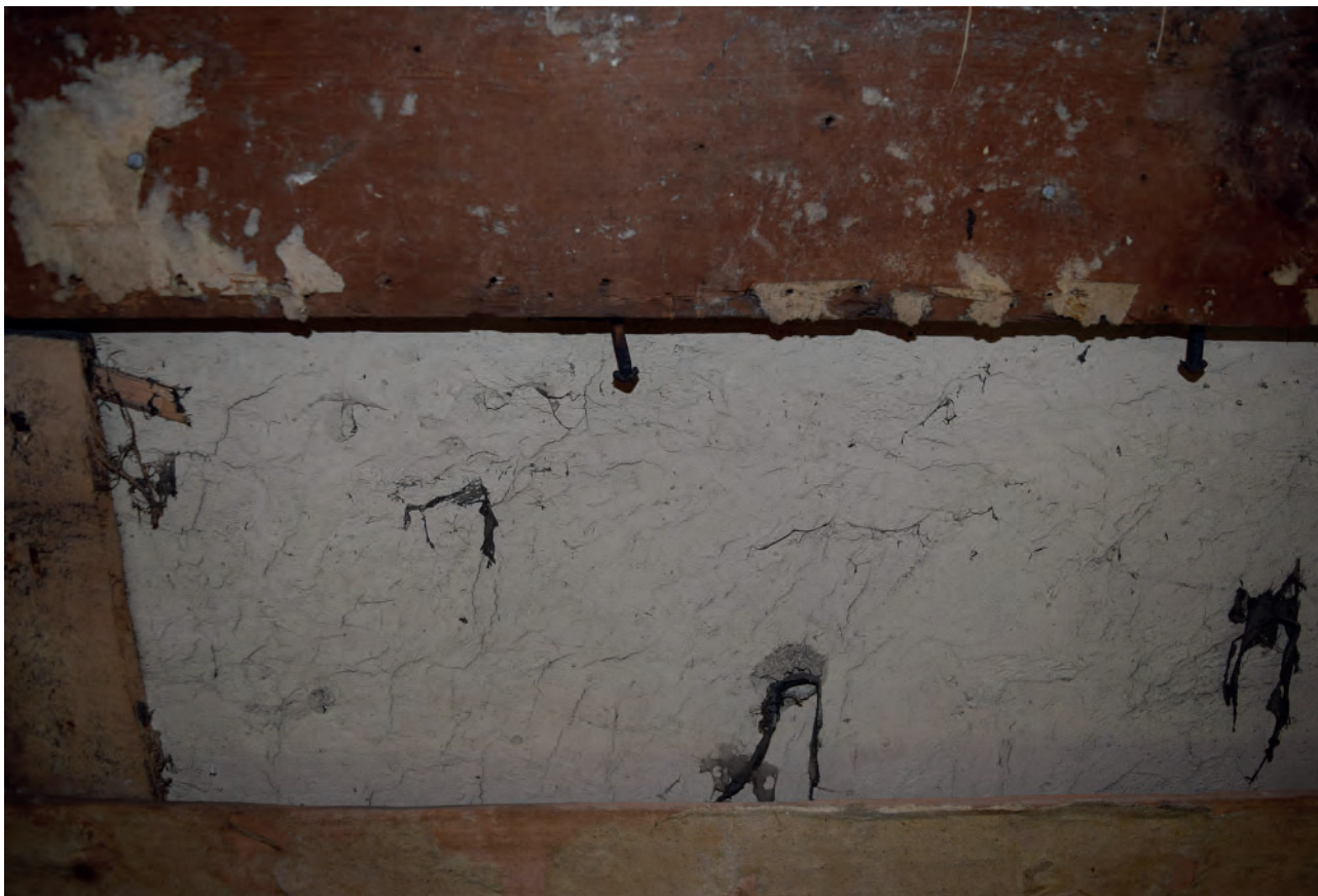
Plate 50: North wall, example of original nails
