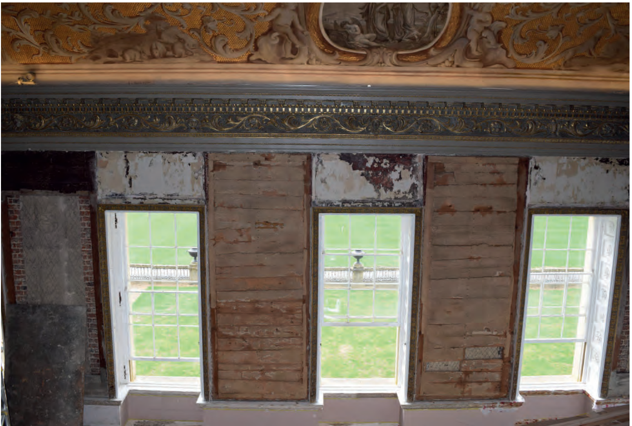
Plate 35: South wall, original plaster over windows
