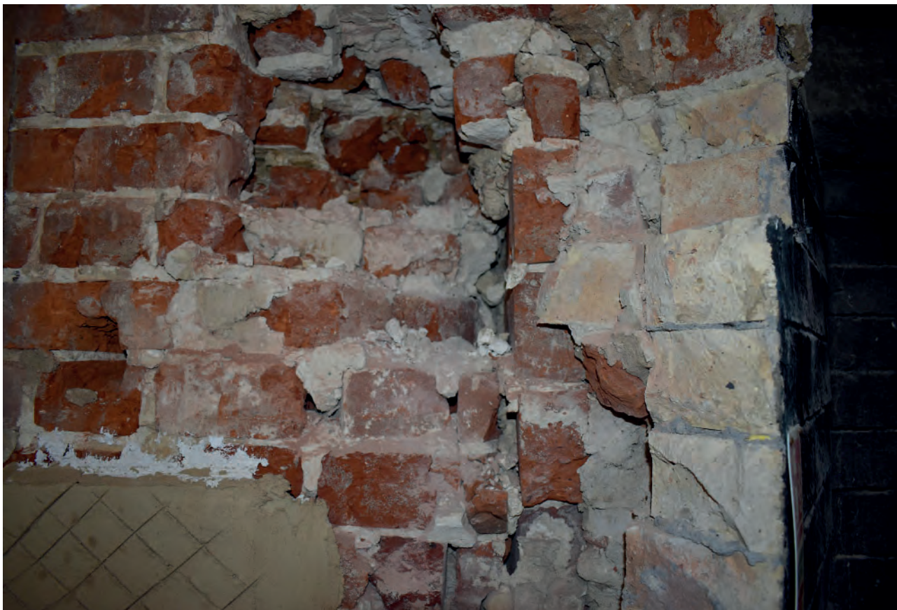
Plate 132: North wall, west part of east fireplace, development phases, Victorian period
