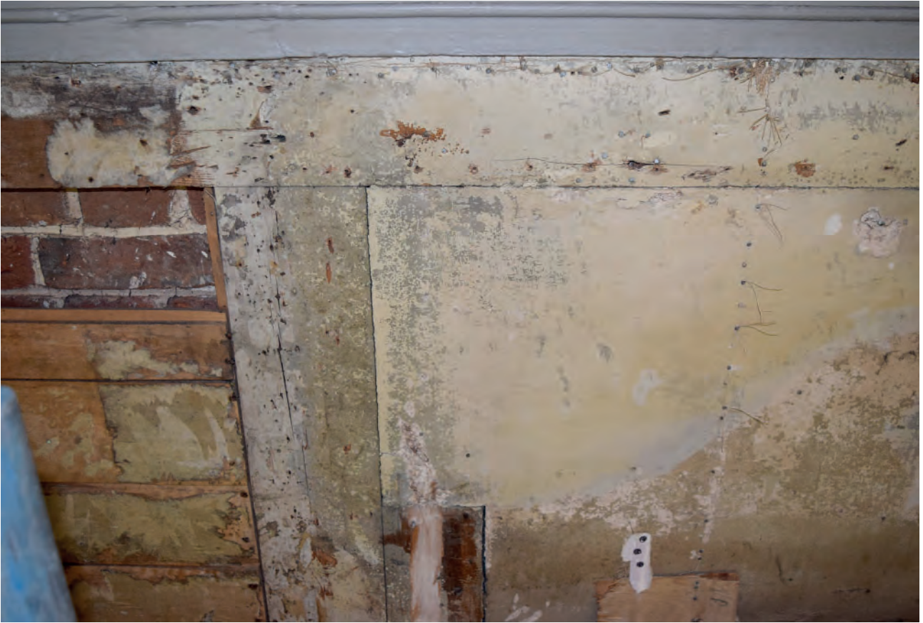
Plate 116: North wall, east upper part of overmantel, example of hessian threads
