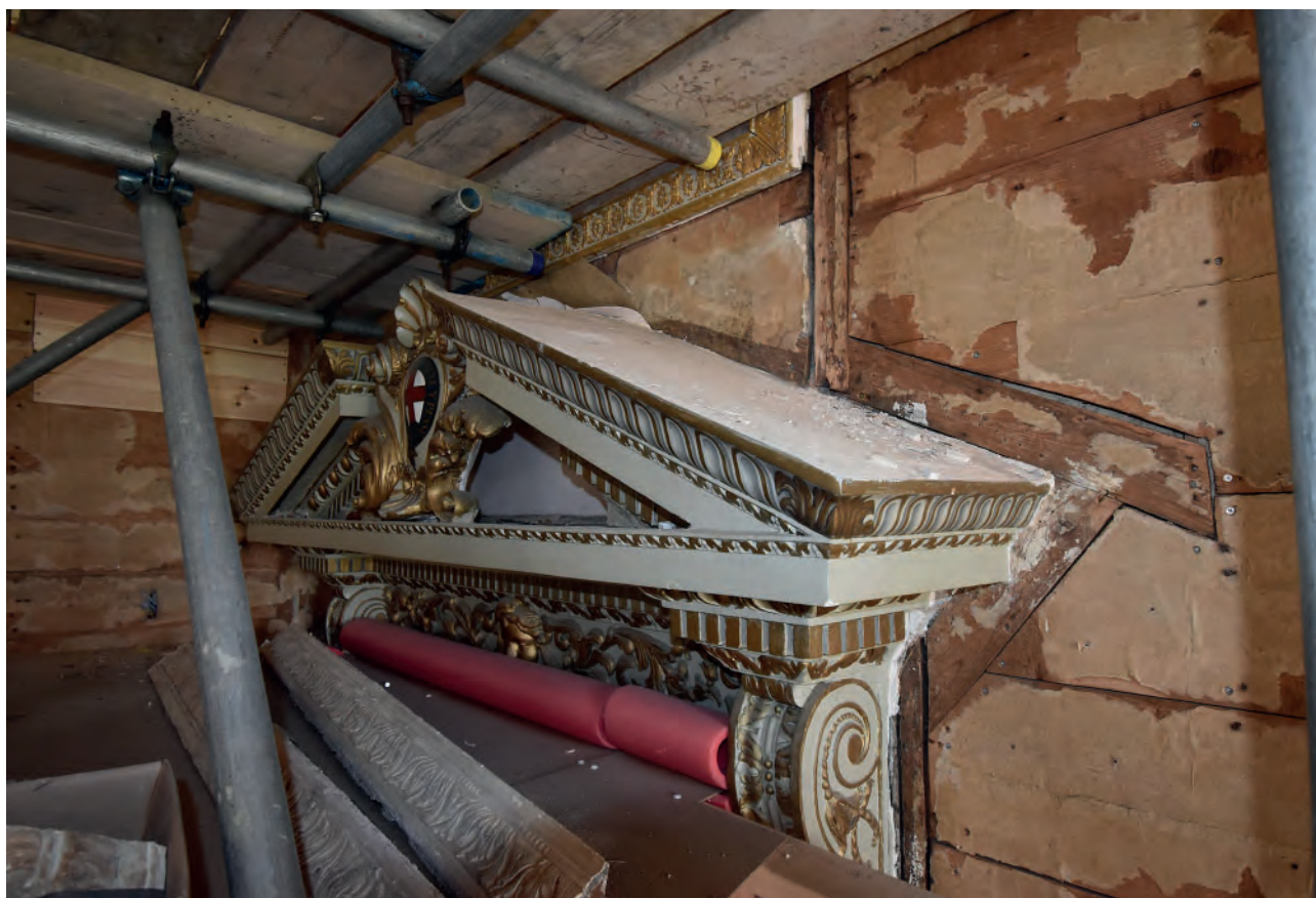
Plate 147: East wall, north door pediment, remodeled sarking boards
