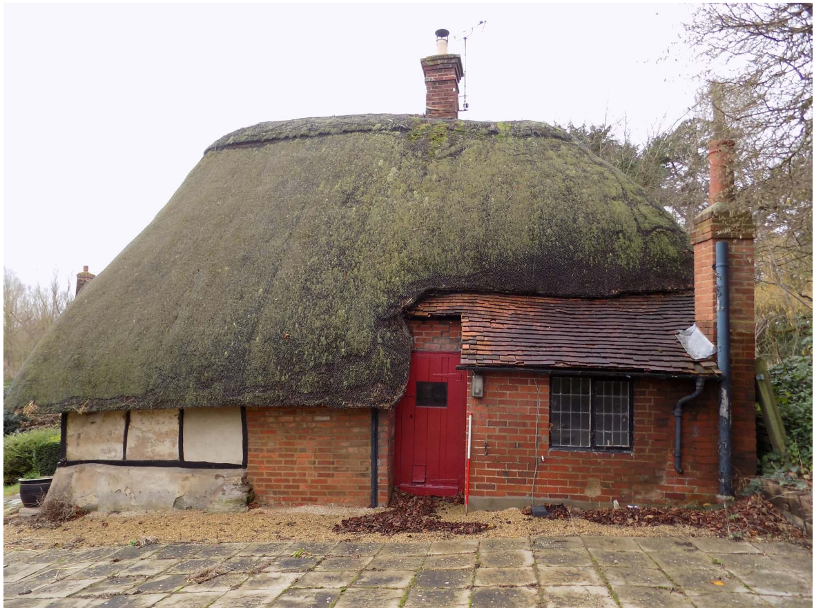
Plate 2: North east elevation of Bridge End Cottage
