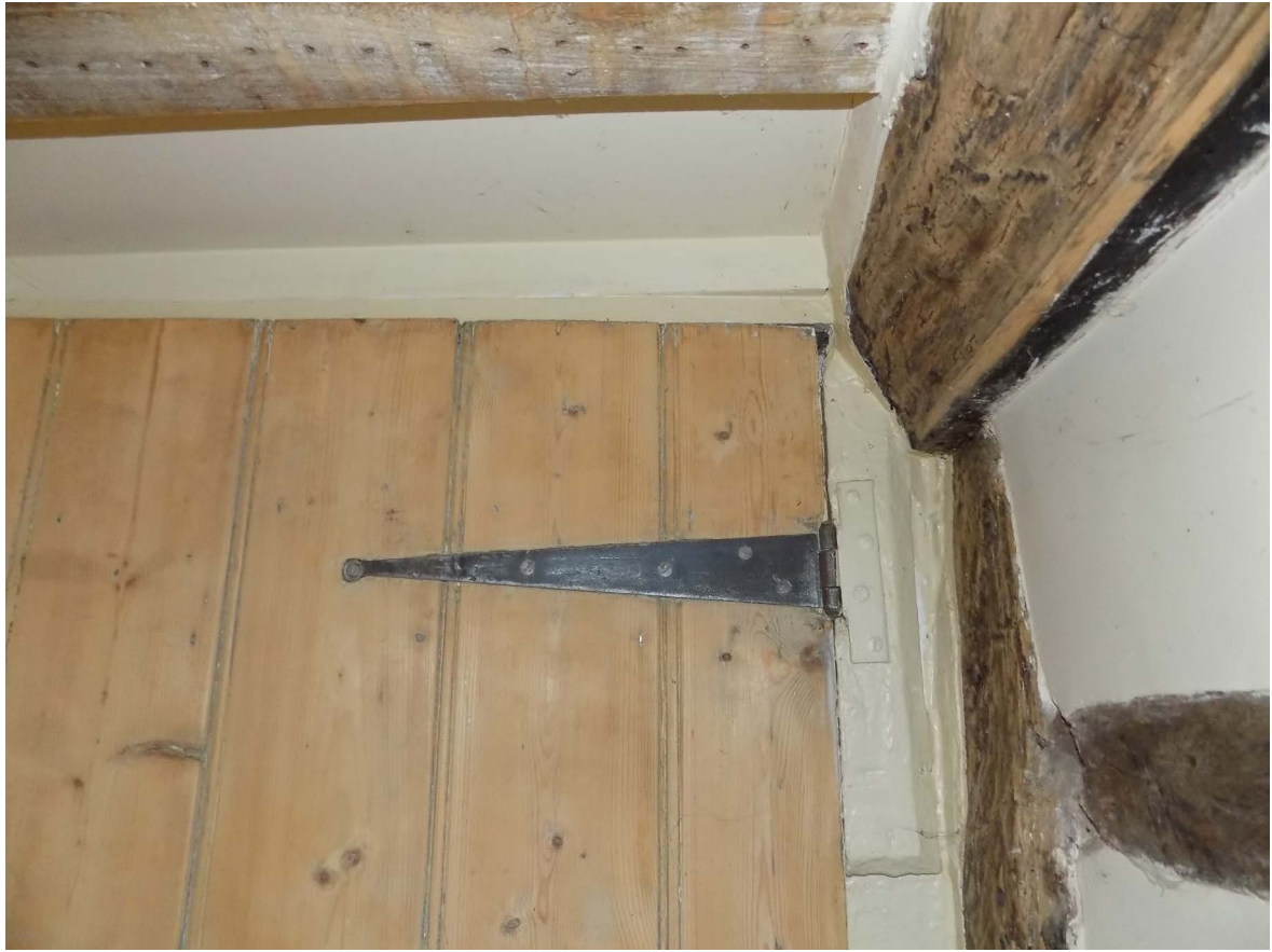
Plate 7: Detail of door strap hinge
