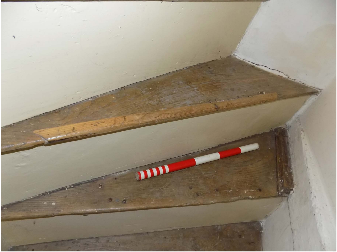
Plate 13: Detail of stair tread showing inserted wood section
