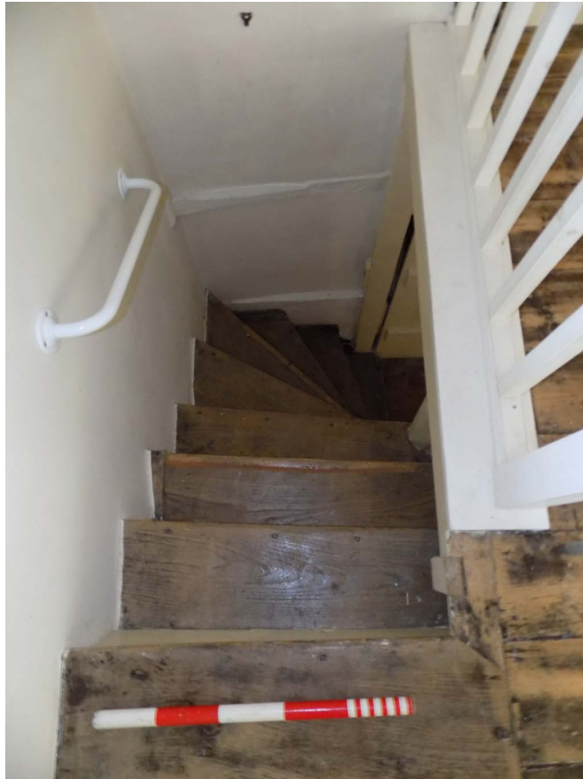
Plate 10: Staircase viewed from above
