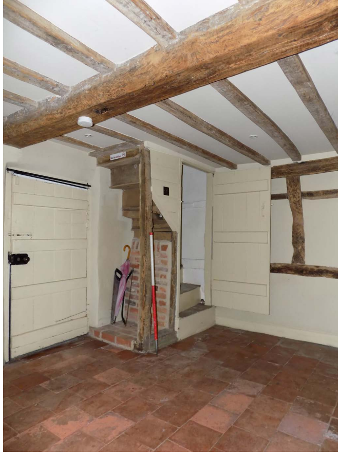
Plate 5: Staircase viewed from ground floor (N)
