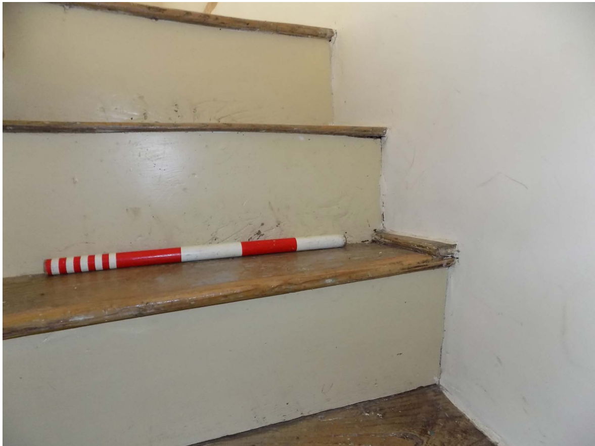
Plate 12: Detail of stair tread showing additional timber
