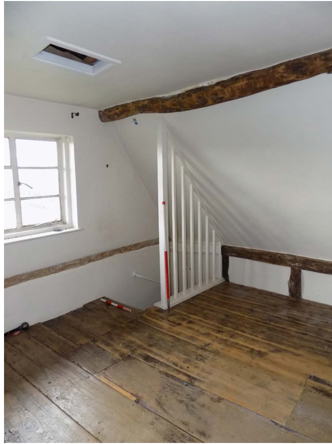
Plate 11: View of staircase from first floor (N)
