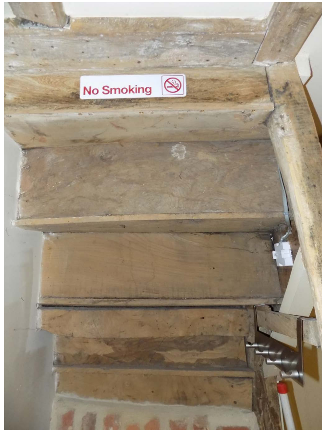
Plate 14: Detail showing rear of stair risers and underside of treads.
