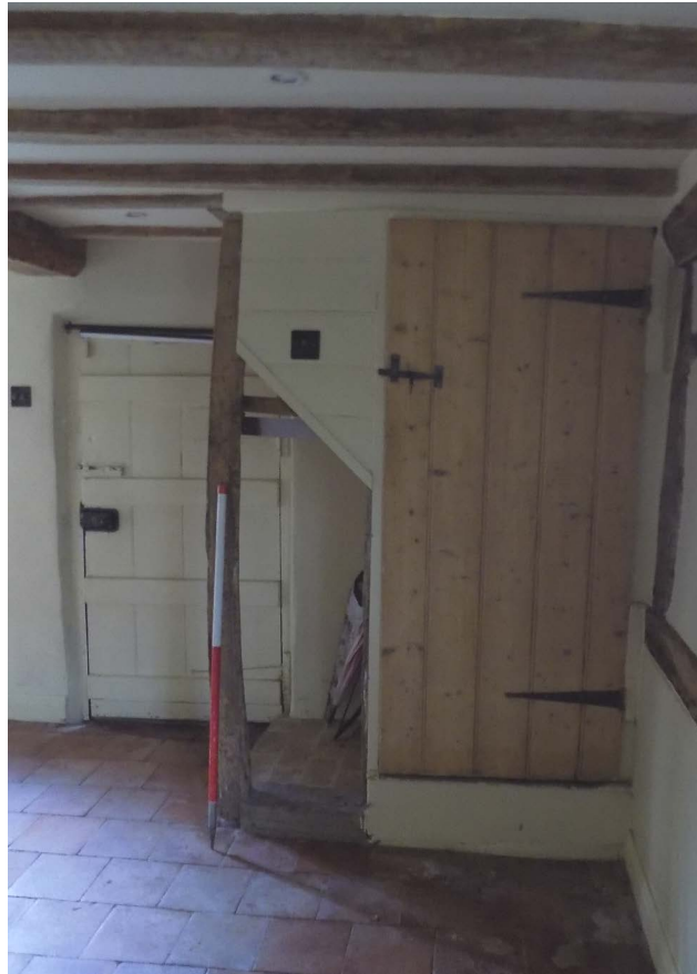
Plate 6: Staircase with door closed (NW)
