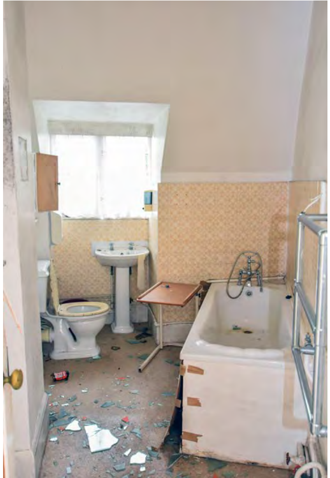
Plate 80: Bathroom in the loft of Harecombe Manor, looking north
