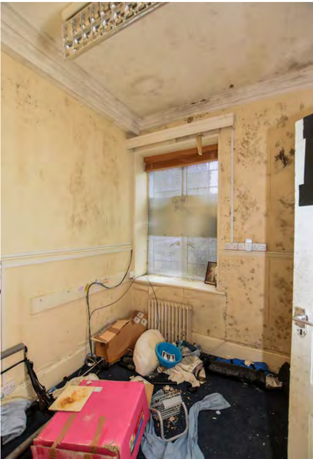
Plate 36: Small room on the ground floor of Harecombe Manor, looking north
