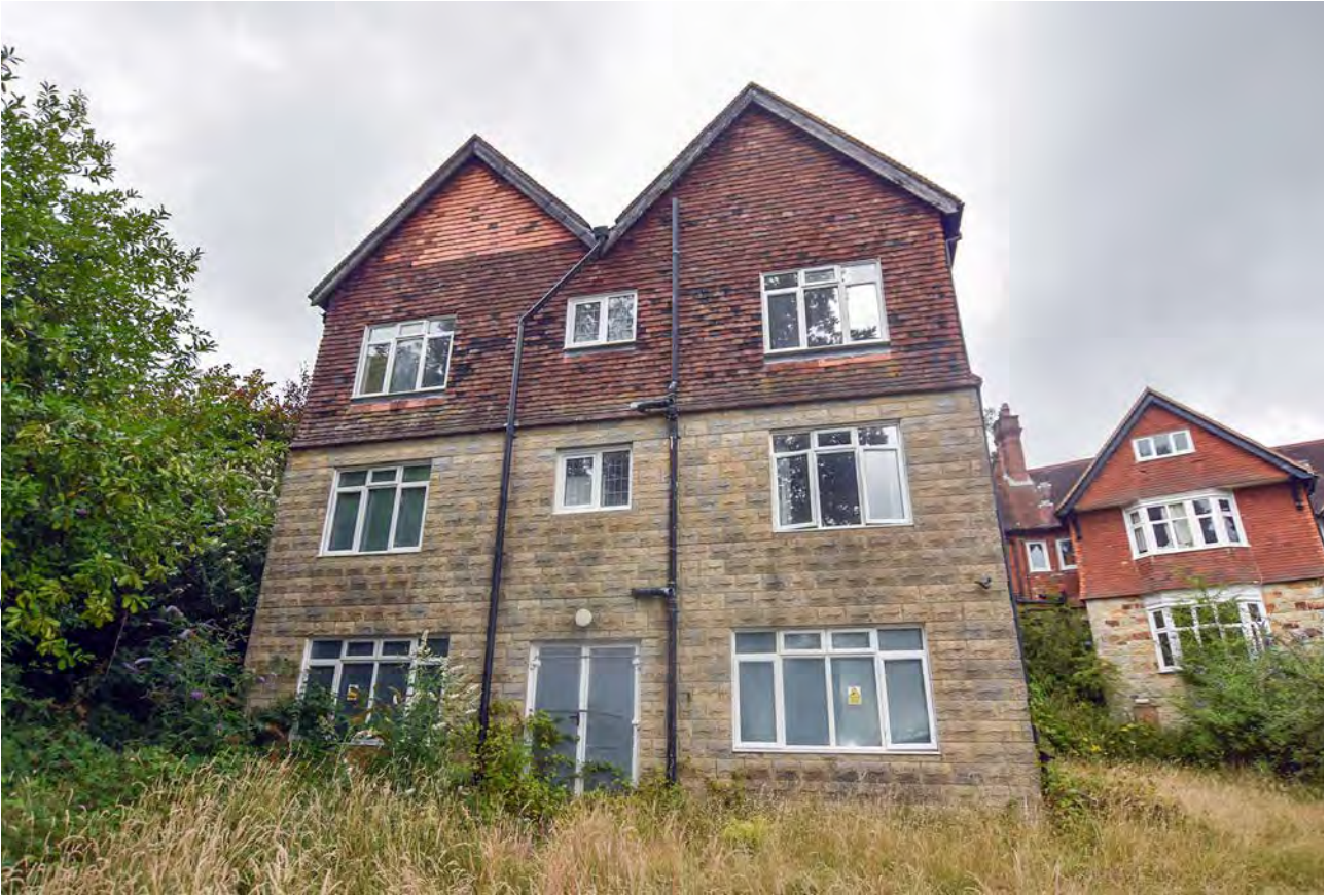
Plate 5: The west extension of Harecombe Manor, looking north
