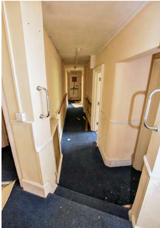
Plate 68: Hallway of the service wing on the first floor of Harecombe Manor, looking west
