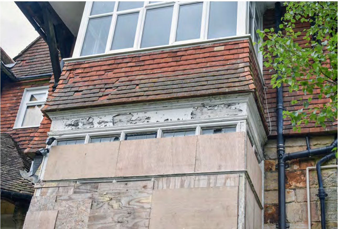
Plate 17: Detail of the east elevation of Harecombe Manor, looking west
