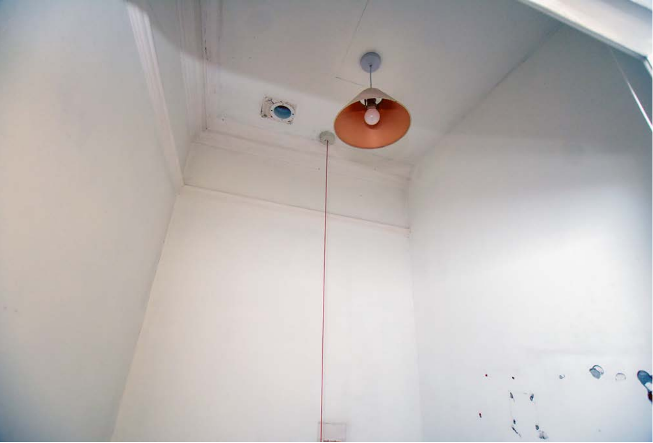
Plate 65: Ensuite in the first floor of the east wing, Harecombe Manor, looking east
