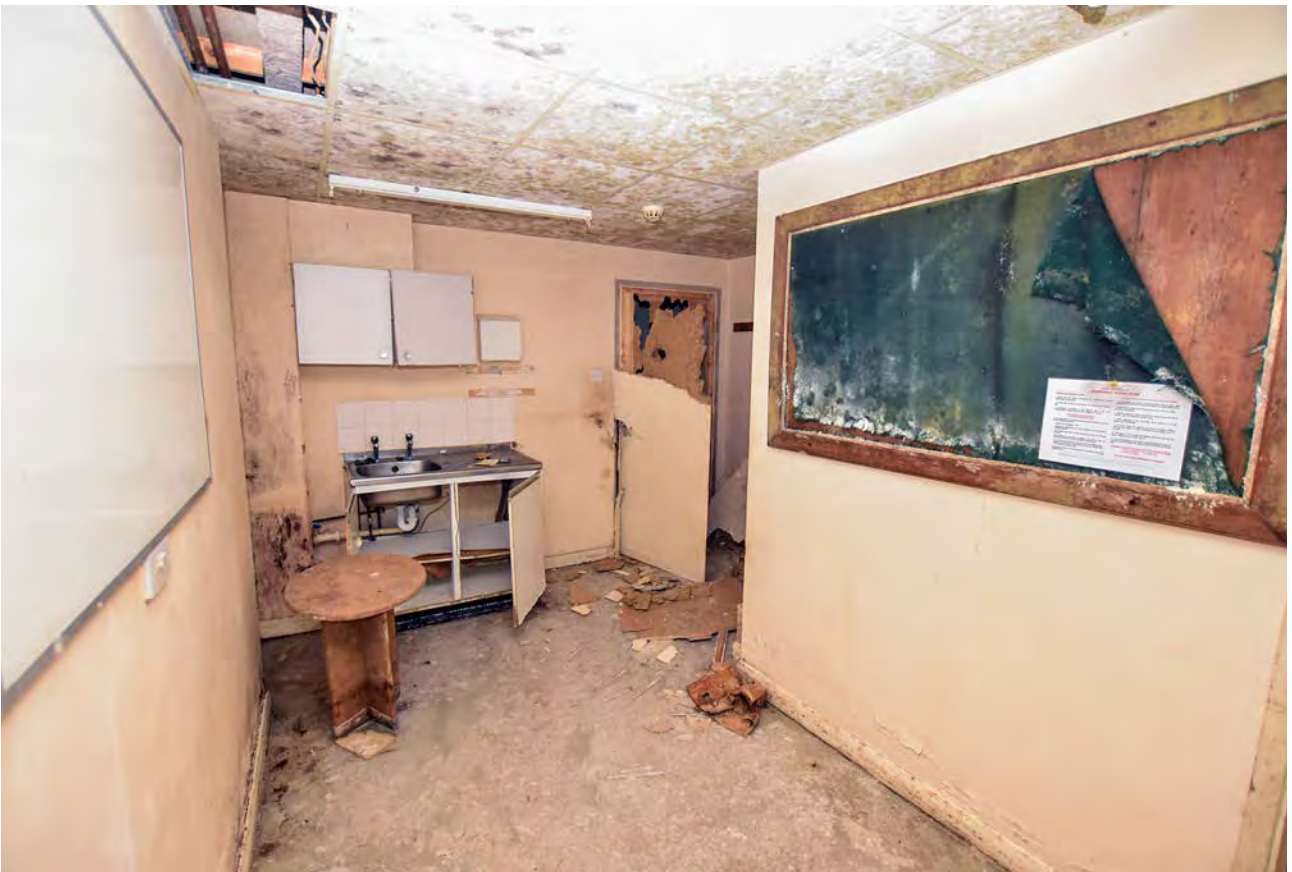
Plate 87: Staffroom in the basement of the west extension, looking east
