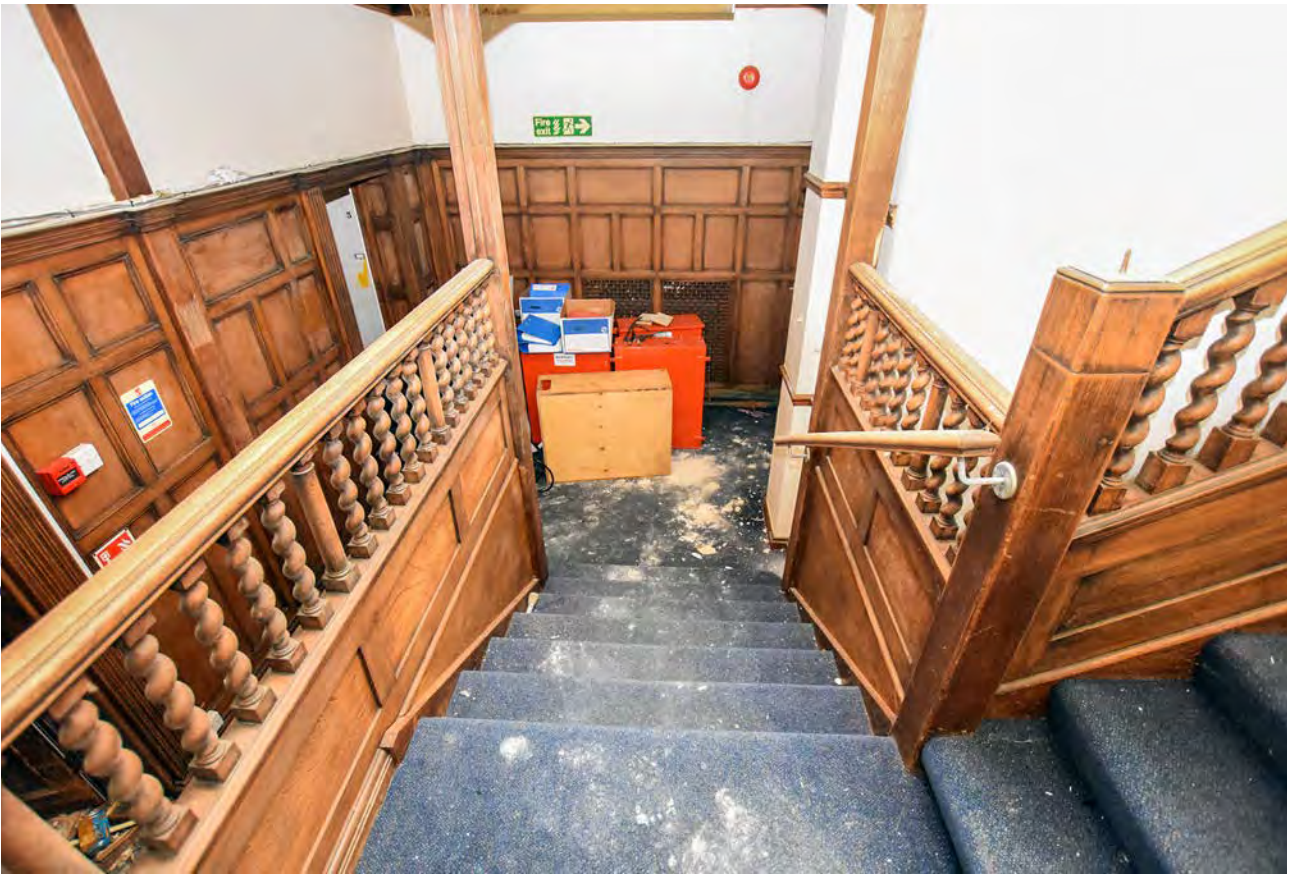
Plate 50: The main stairway from the ground to the first floor in Harecombe Manor, looking south
