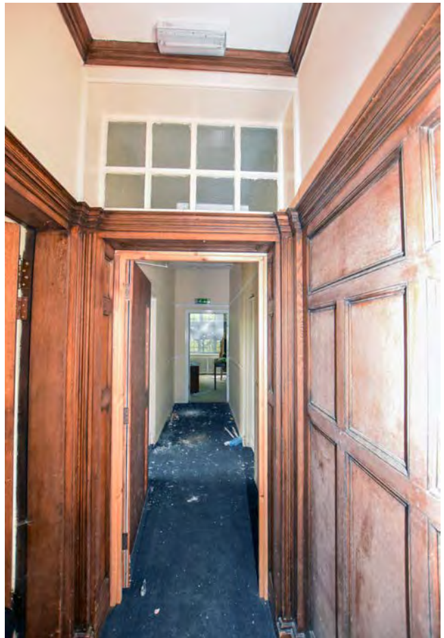
Plate 37: Hallway on the ground floor of Harecombe Manor, looking north
