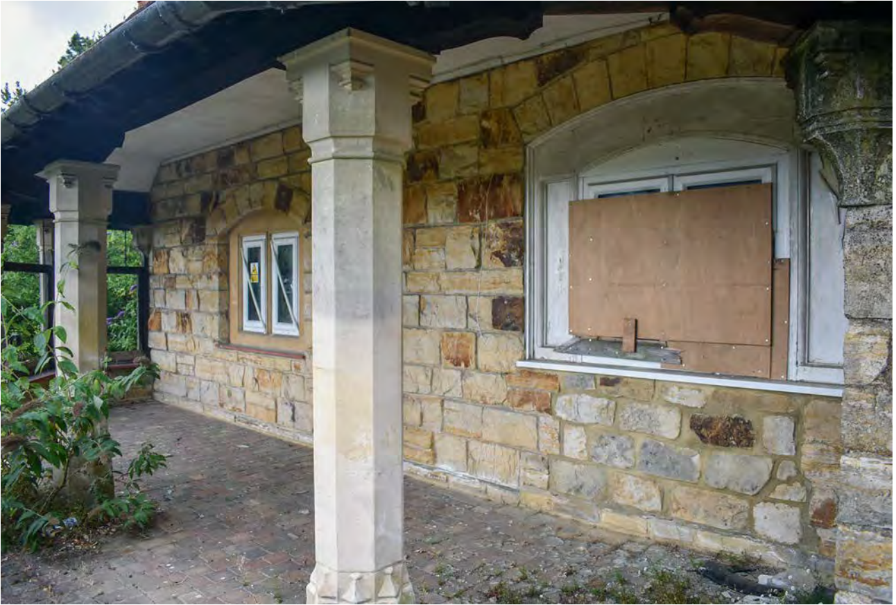
Plate 18: The porch on the east elevation of Harecombe manor, looking south-west
