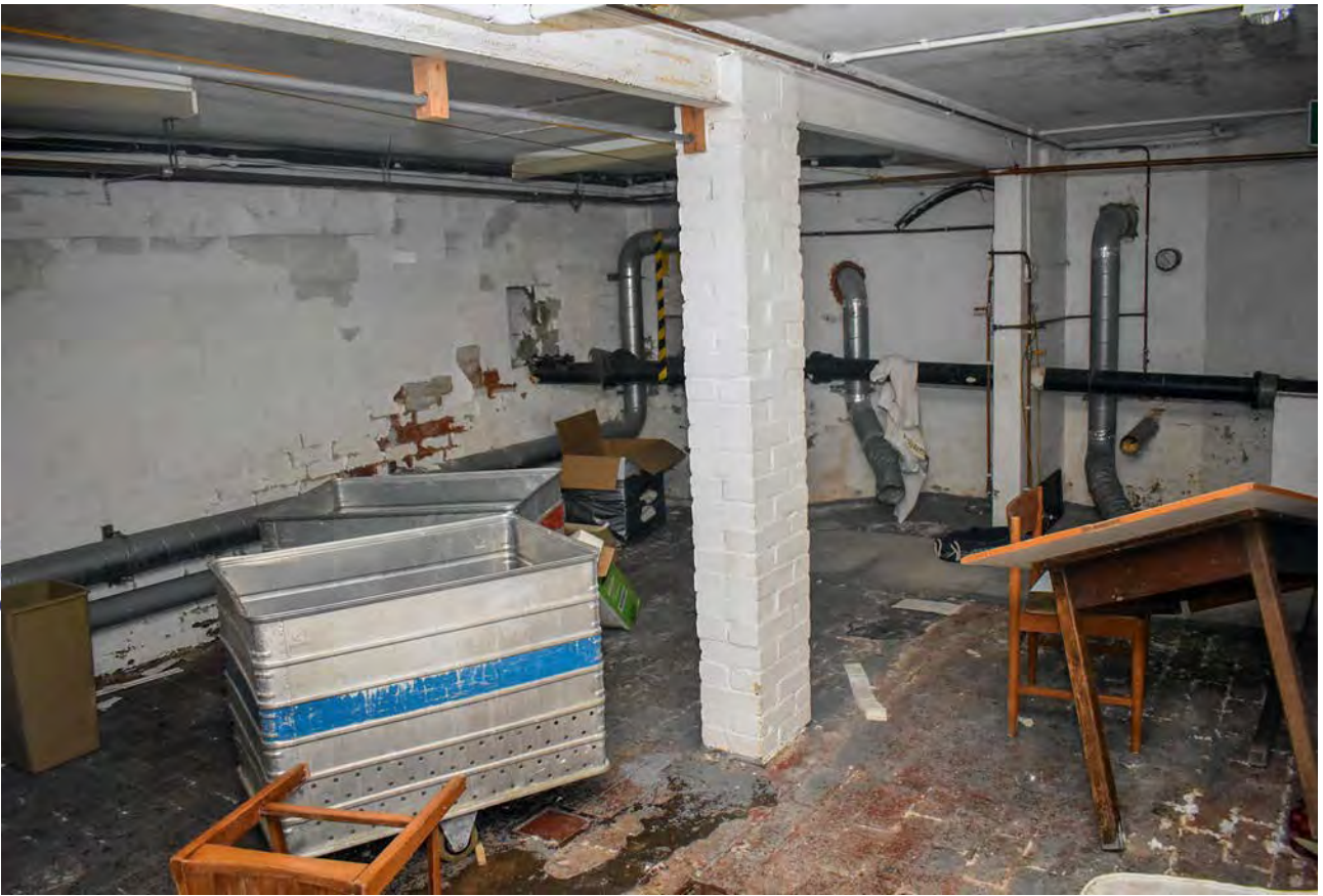
Plate 26: The central basement of Harecombe Manor, looking south-east
