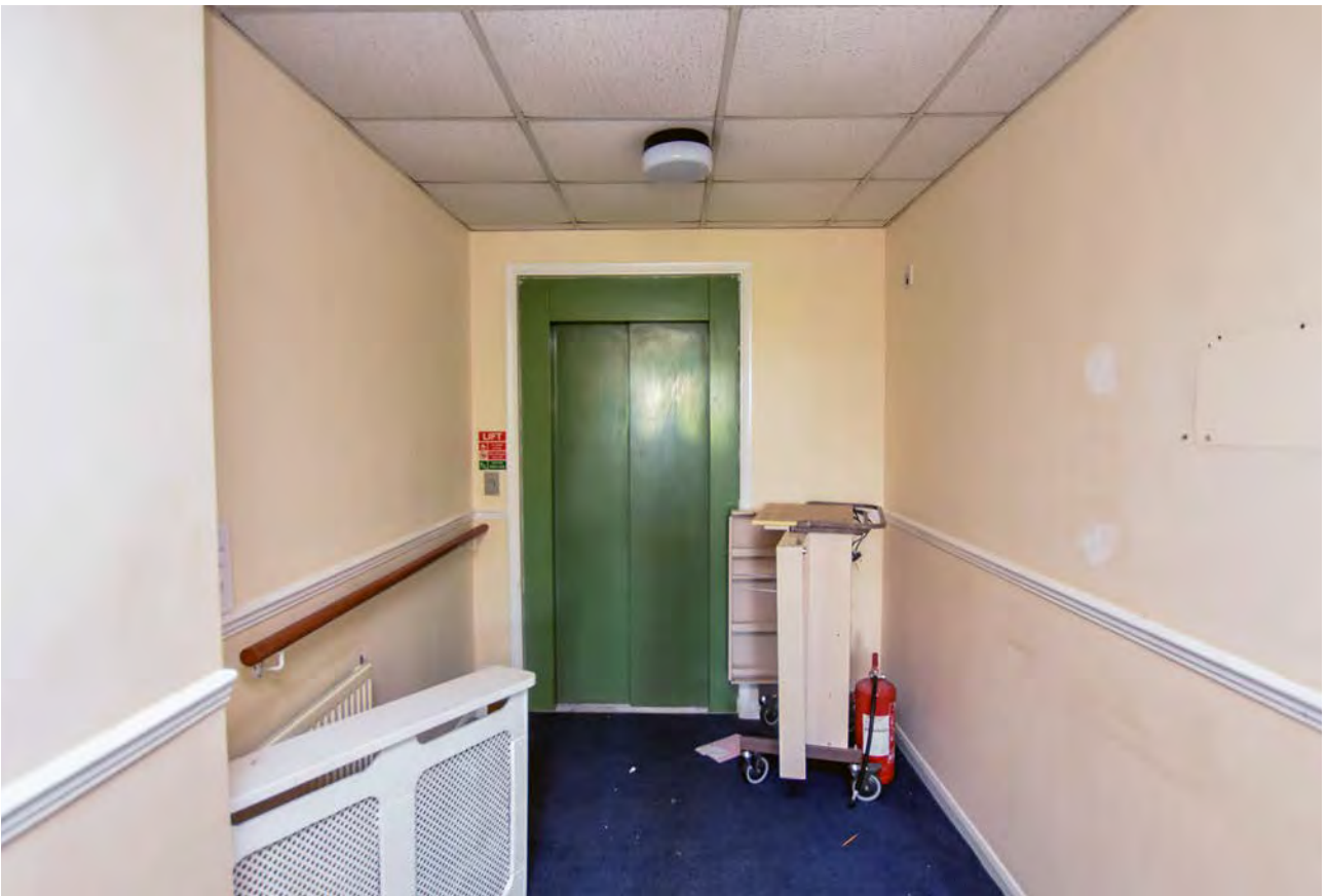
Plate 83: Lift in the west extension, looking west
