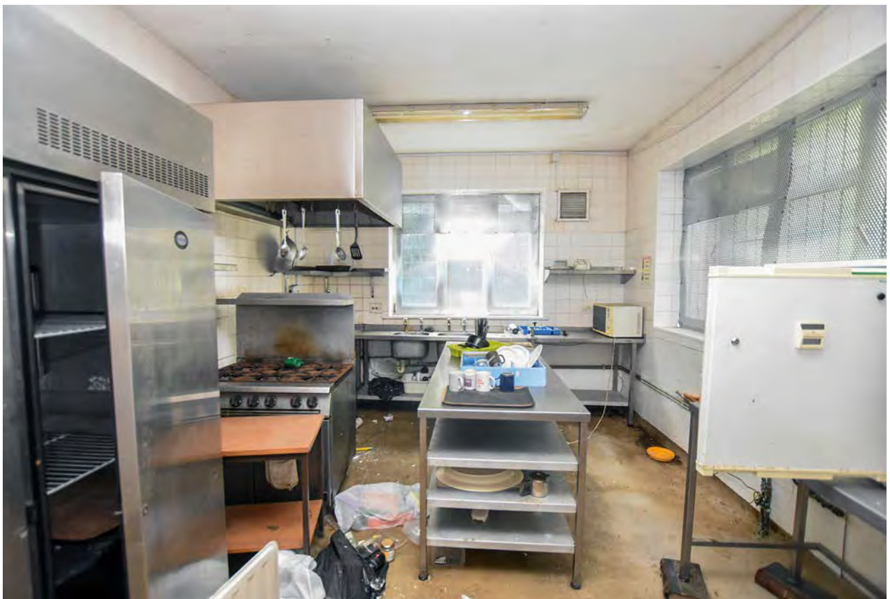
Plate 89: Kitchen in the ground floor of the west extension, looking west
