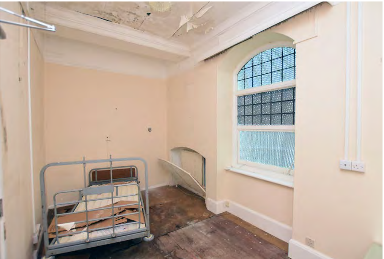
Plate 44: Small room in the ground floor of Harecombe Manor, looking north-east
