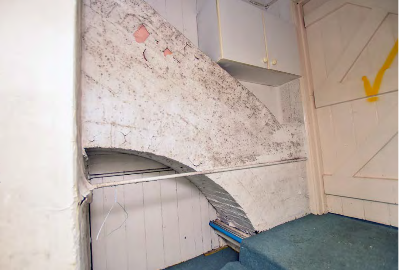
Plate 73: Buttress in the loft of Harecombe manor, looking south-east
