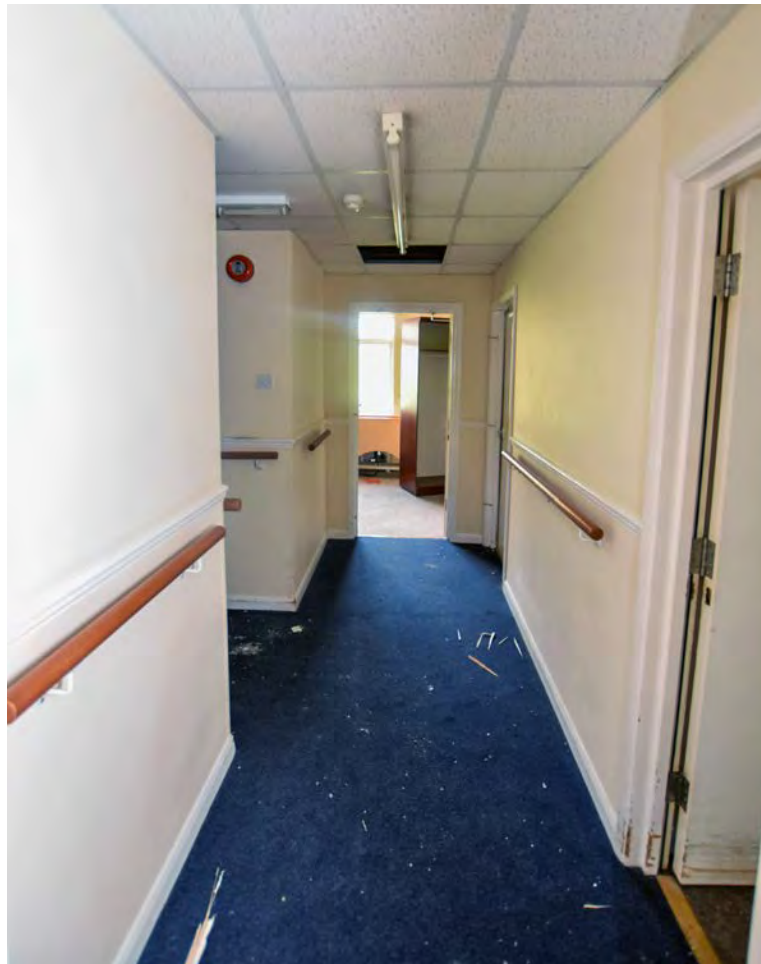
Plate 88: Hallway in the ground floor of the west extension, looking east
