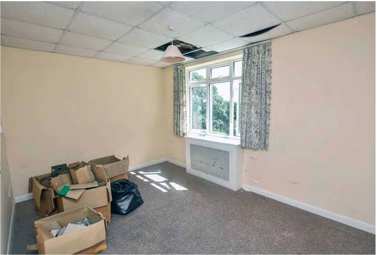
Plate 90: Bedroom in the ground floor of the west extension, looking south-east
