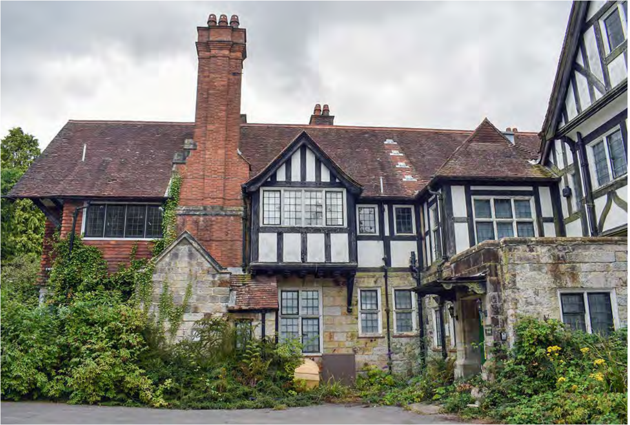
Plate 14: The west facing elevation of the east wing of Harecombe Manor, looking east
