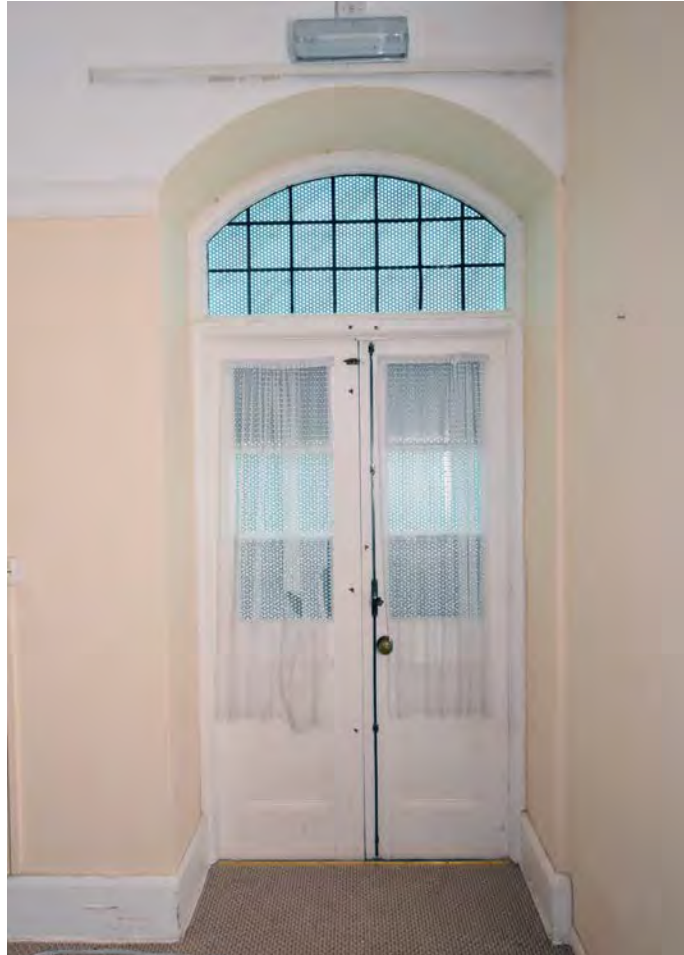
Plate 43: Door in sitting room on the ground floor of Harecombe Manor, looking east
