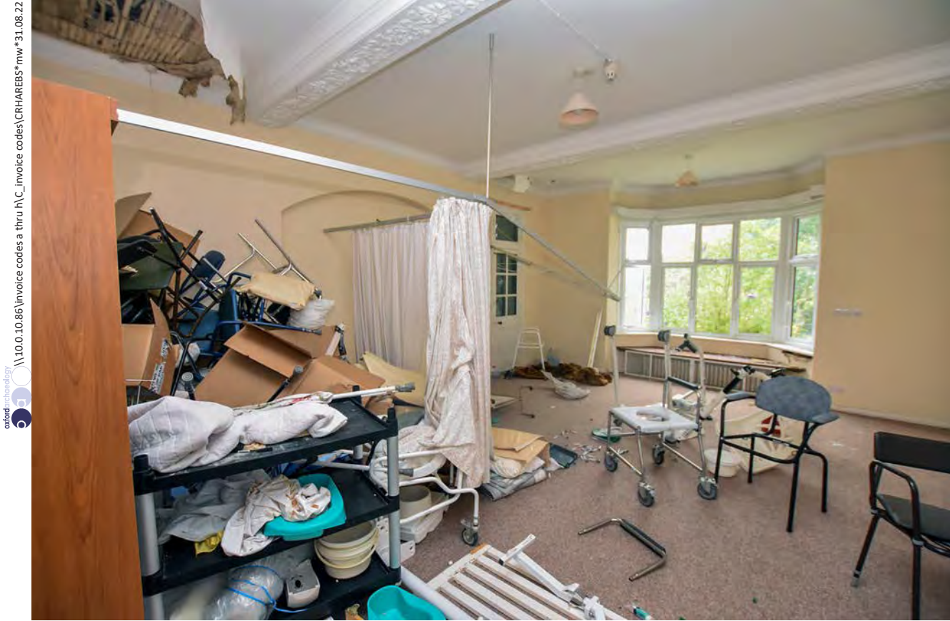
Plate 32: Lounge on the ground floor of Harecombe Manor, looking south-east
