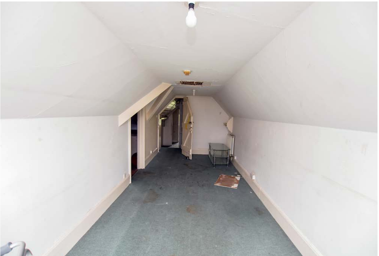
Plate 74: South room in the loft of Harecombe Manor, looking north
