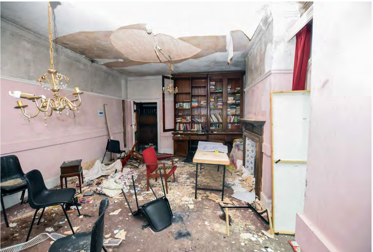
Plate 38: Library on the ground floor of Harecombe Manor, looking west
