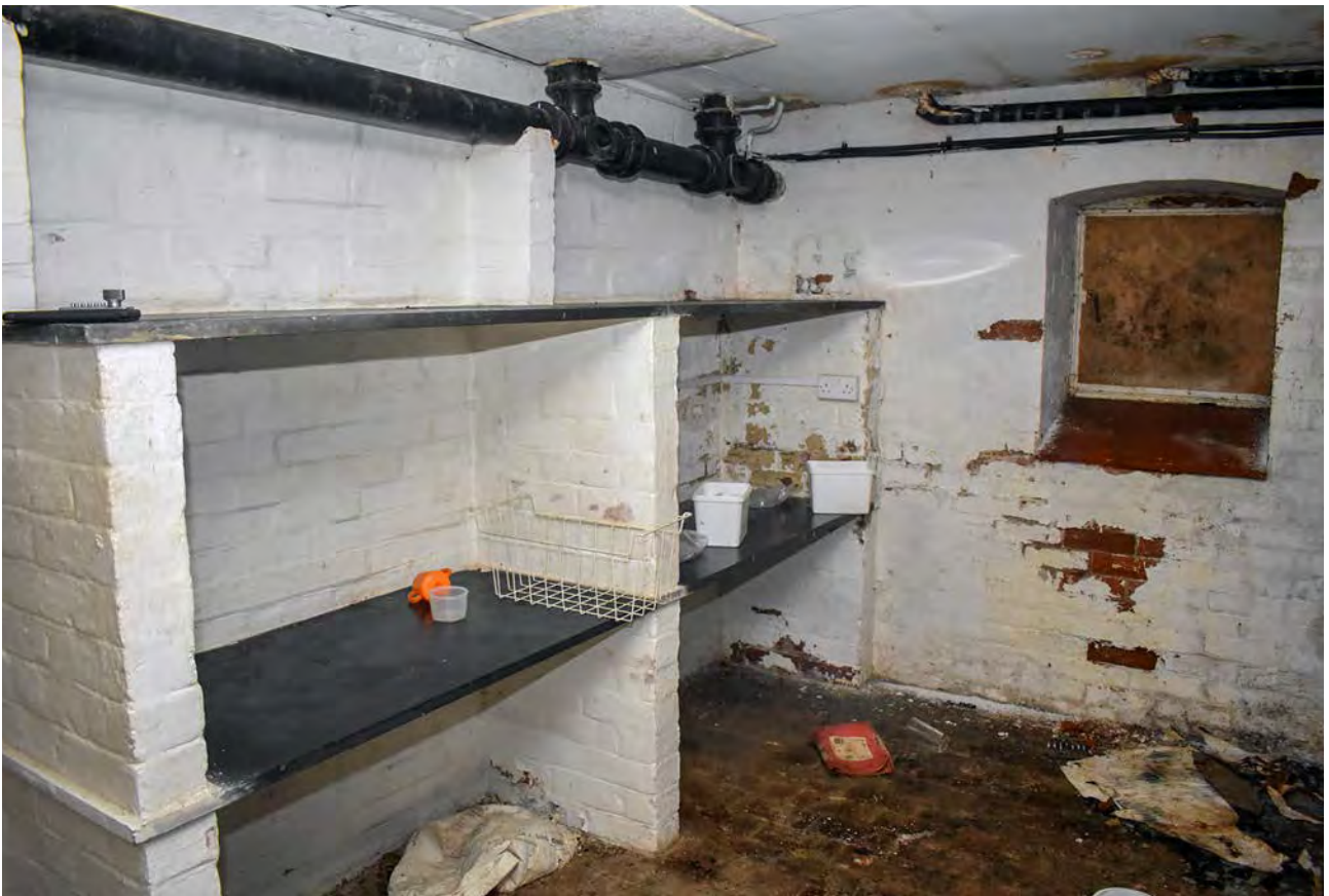
Plate 25: The central basement of Harecombe Manor, looking north-west
