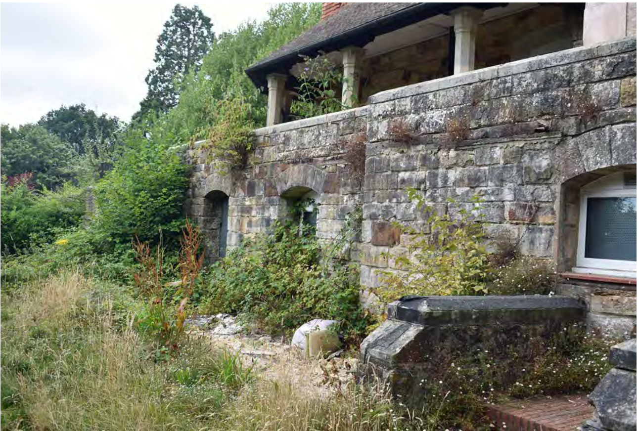
Plate 19: The terrace under the east elevations of Harecombe Manor, facing south-west
