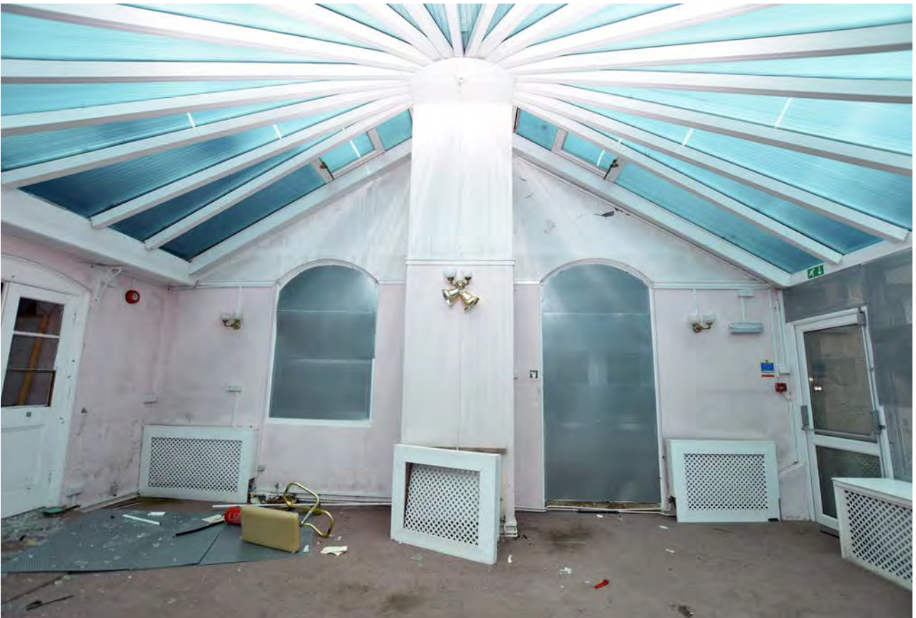
Plate 40: Conservatory on the ground floor of Harecombe Manor, looking west
