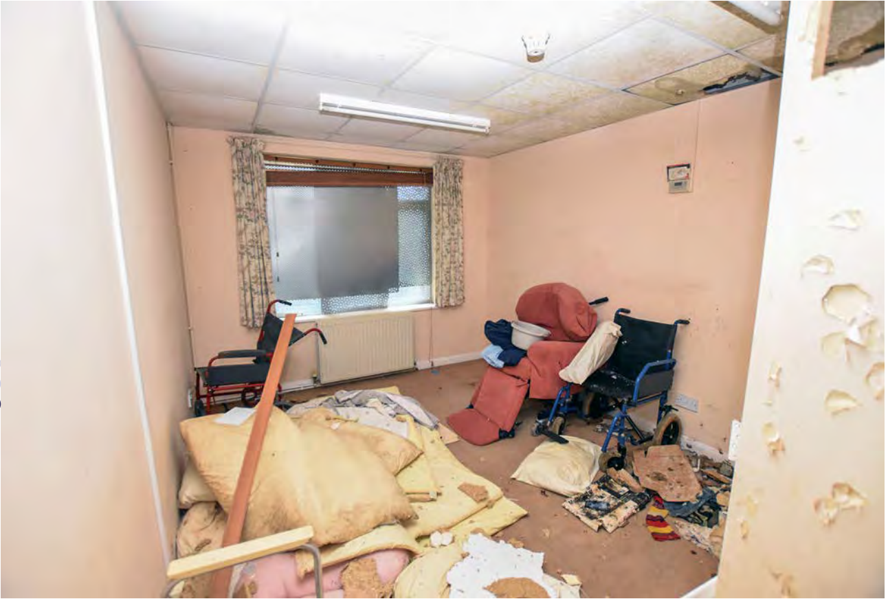
Plate 86: Staffroom in the basement of the west extension, looking east
