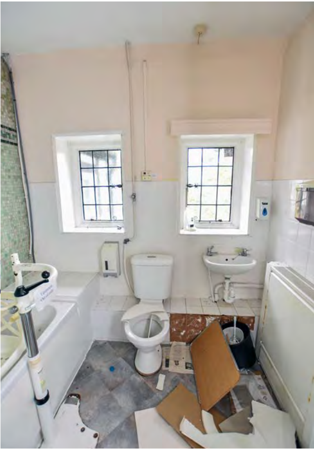
Plate 66: Bathroom on the first floor of the east wing, Harecombe Manor, looking west
