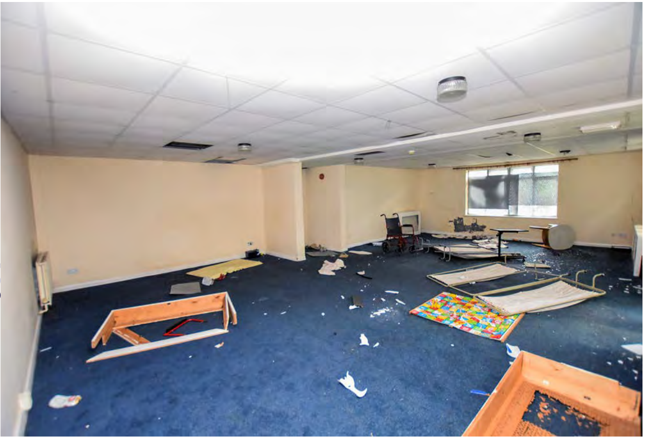
Plate 84: Lounge in the basement of the west extension, looking north-east
