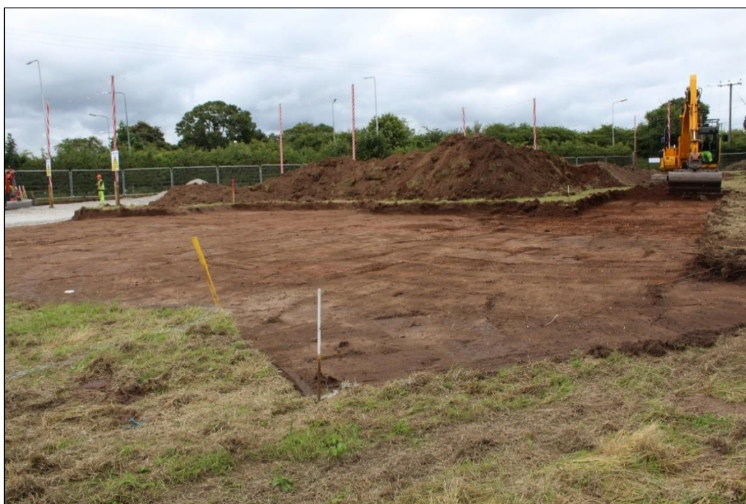
Plate 1: Topsoil stripping, Tarvin Road roundabout compound
