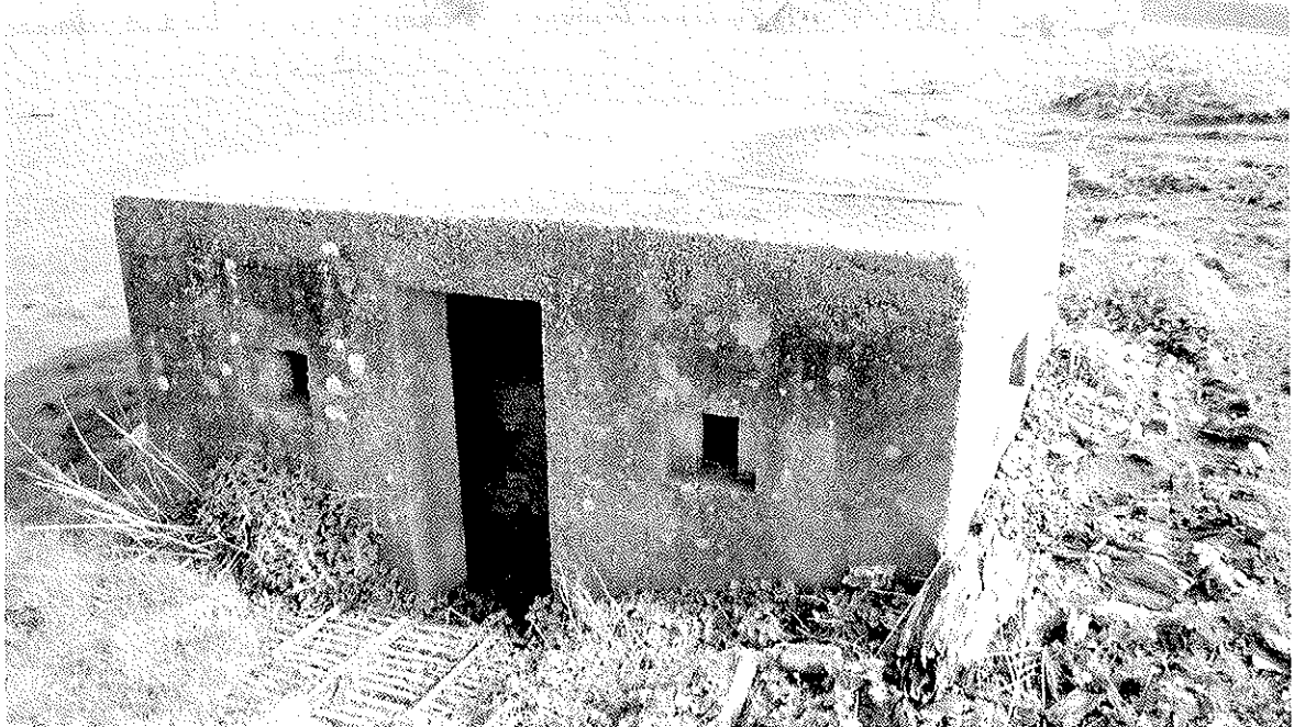
Plate 1: Pill Box A, south-west elevation
