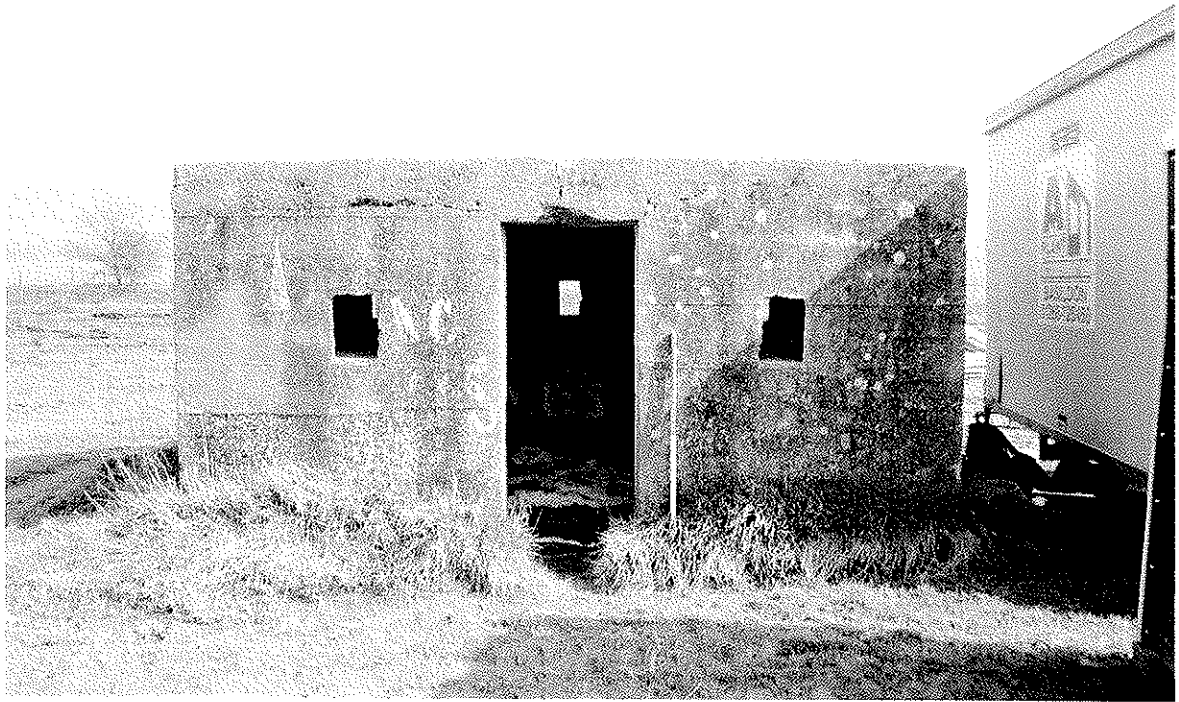
Plate 5: Pill Box B, south-west elevation
