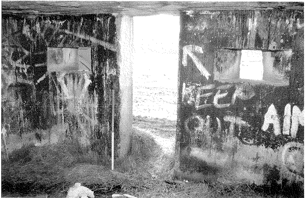
Plate 6: Interior of Pill Box B
