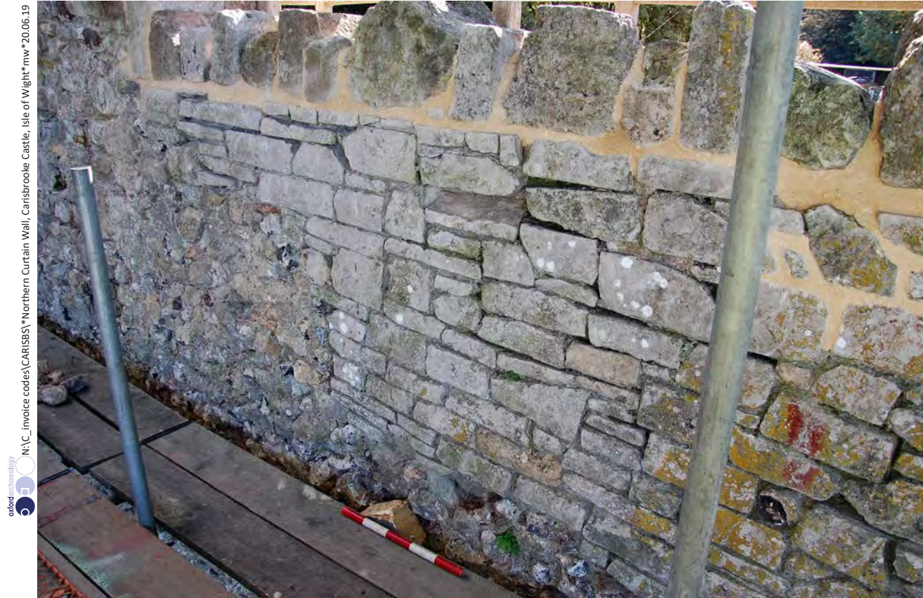
Plate 16: Rebuilt patch at level 3
