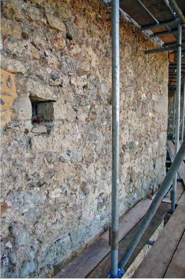
Plate 21: Putlog holes at level 3
