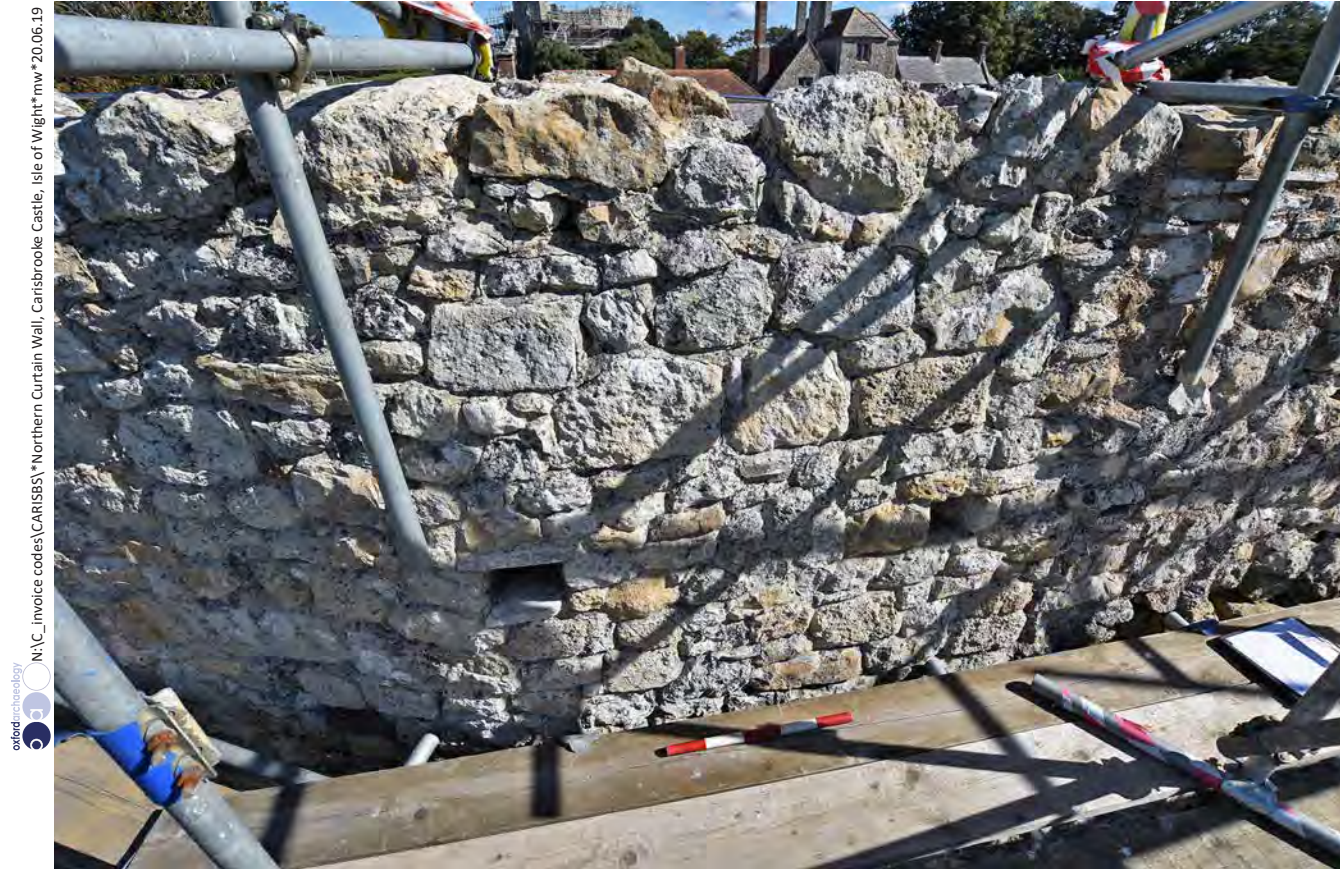
Plate 39: Pair of putlogs at level 5 t
