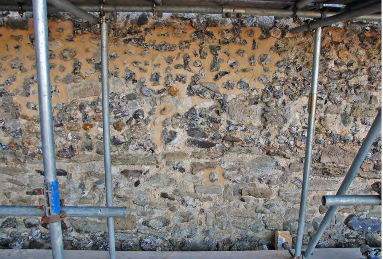
Plate 11: Northern curtain wall at level 1
