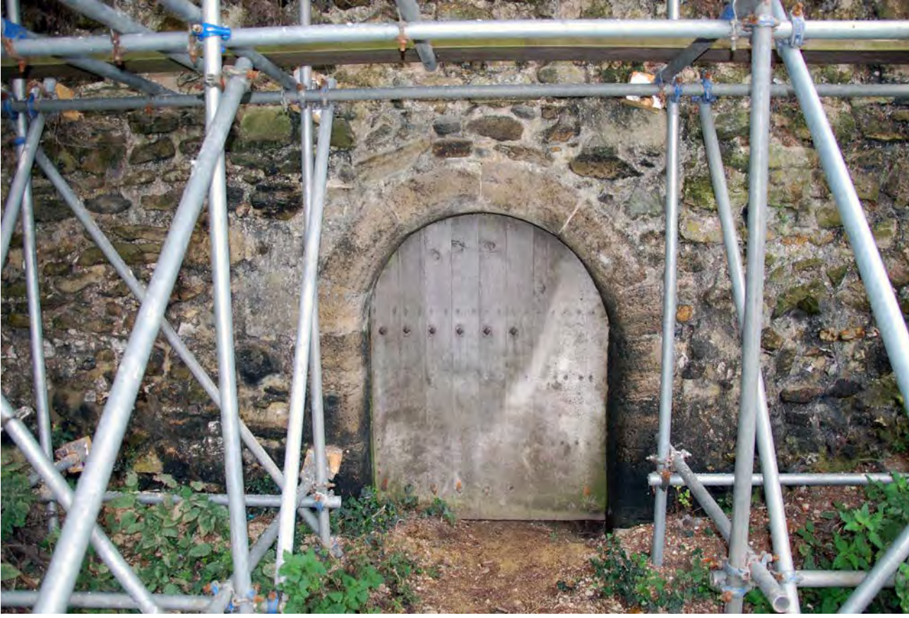
Plate 10: Postern at base of northern curtain wall
