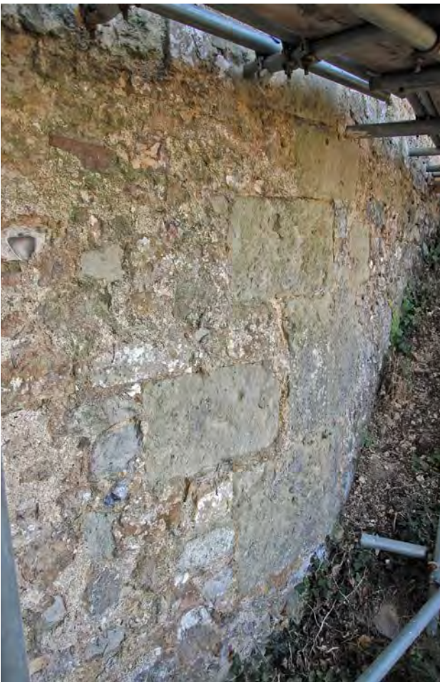
Plate 12: Curtain wall at level 2
