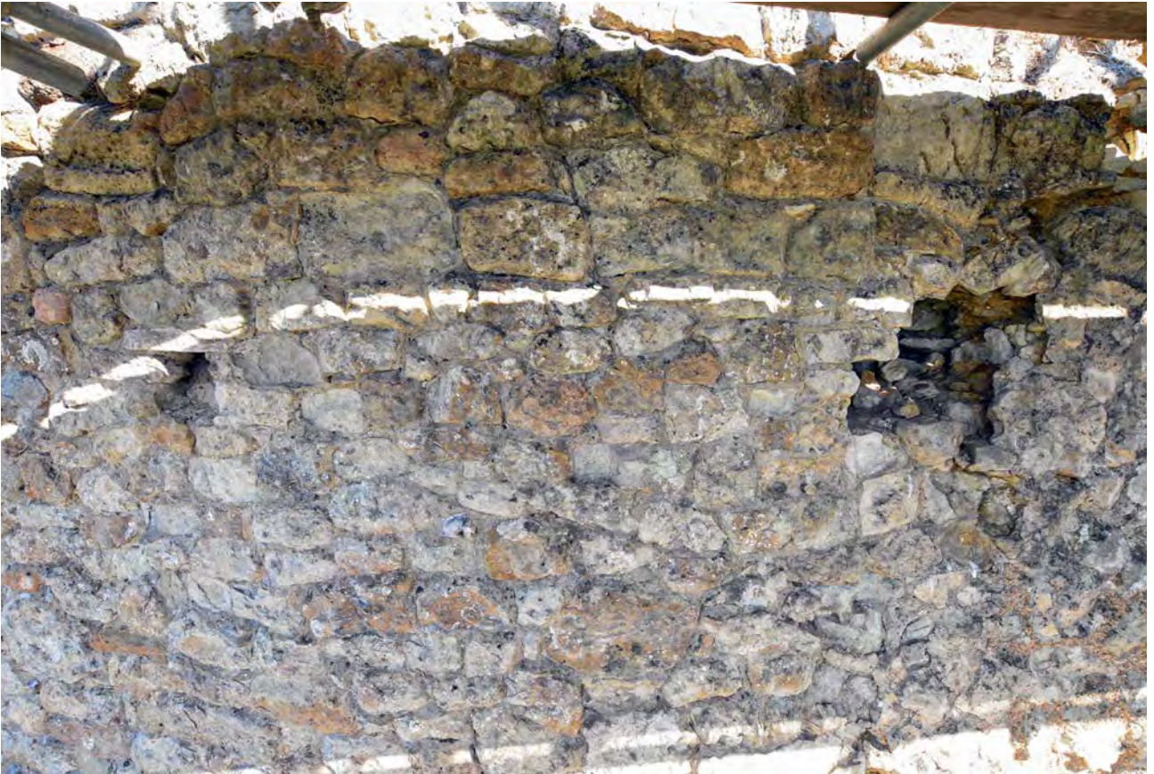
Plate 34: Void D1 and putlog
