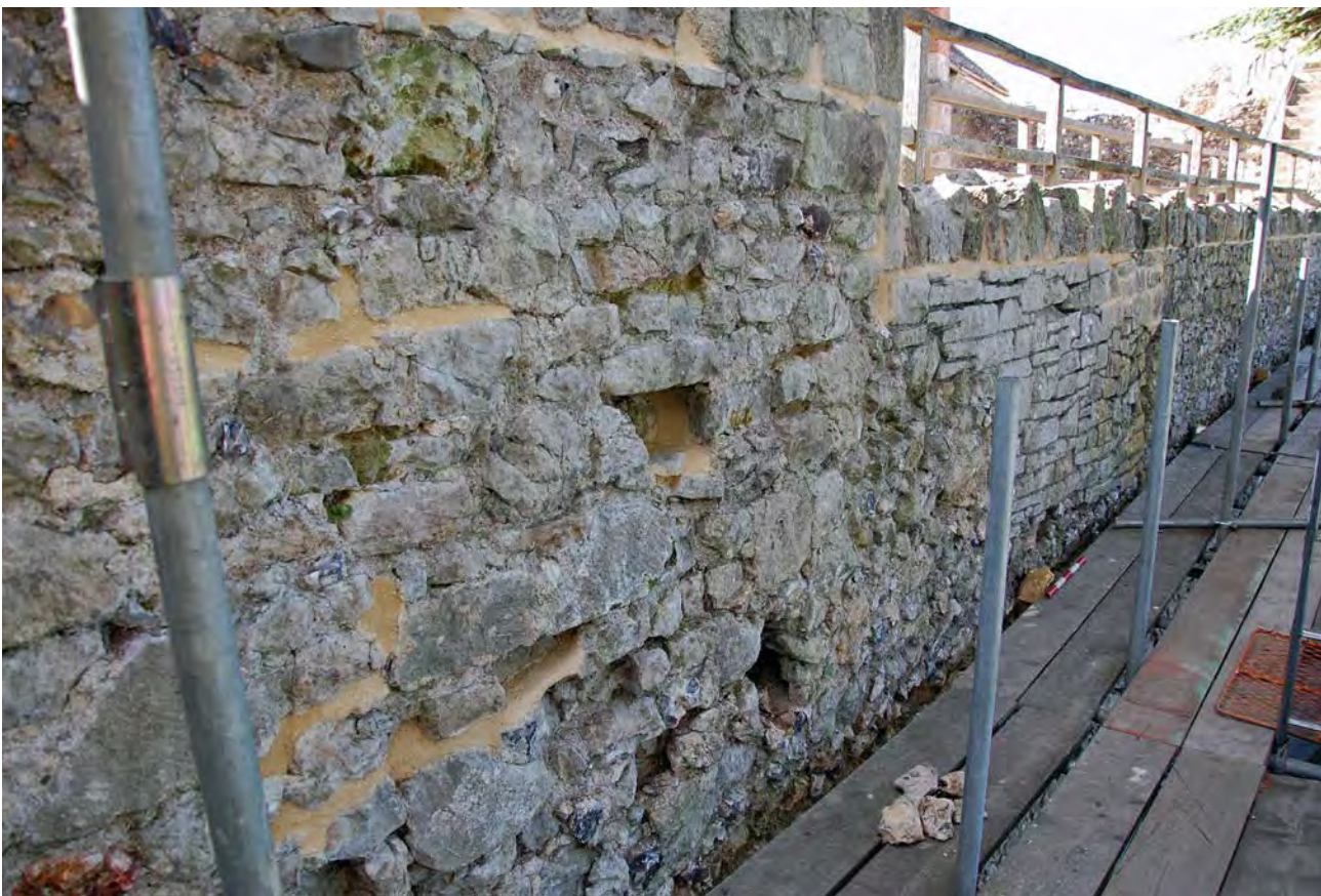
Plate 17: Curtain wall at level 3
