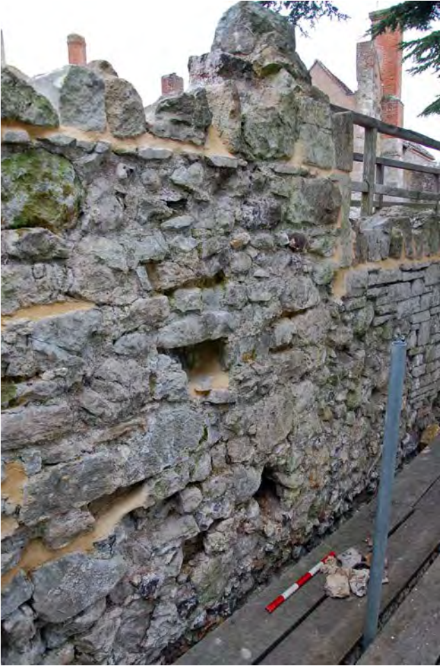
Plate 18: Curtain wall at level 3
