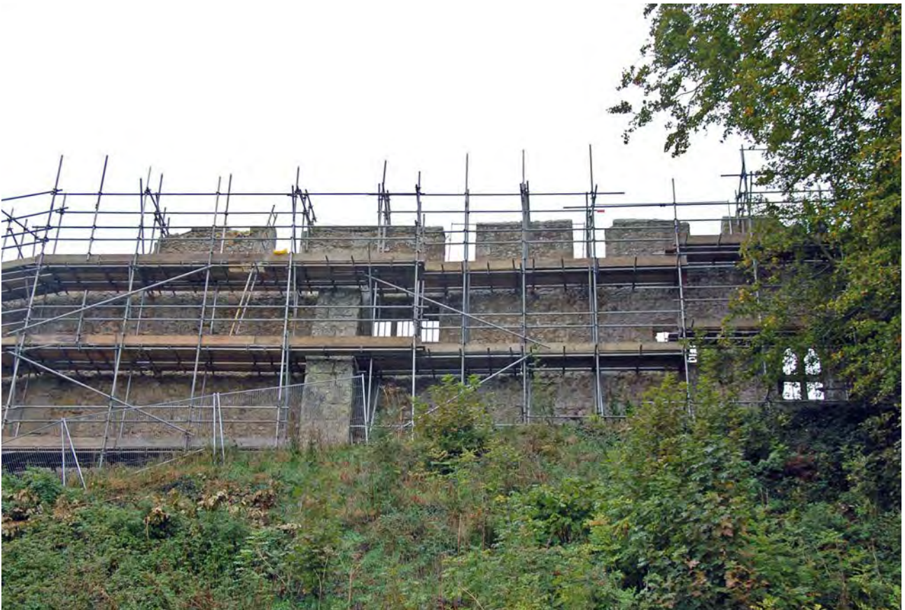
Plate 4: Central part of northern curtain wall
