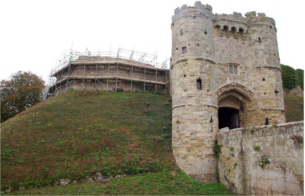
Plate 1: Gatehouse and adjacent section of curtain wall
