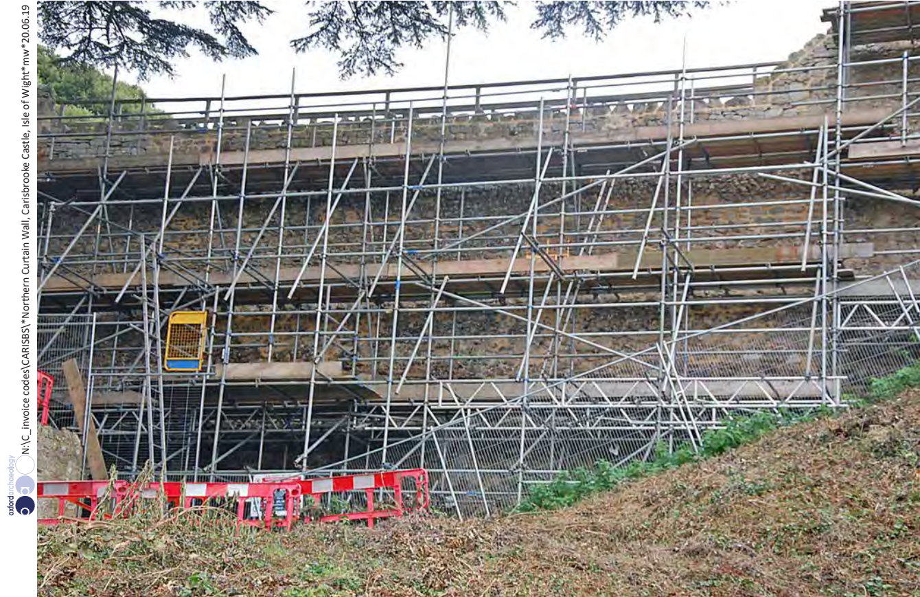
Plate 7: Northern curtain wall above postern
