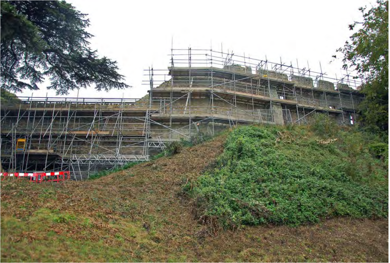
Plate 5: Central part of northern curtain wall
