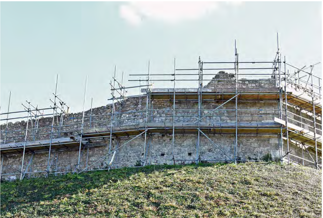
Plate 2: North-west part of curtain wall
