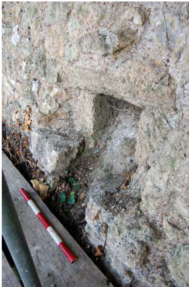
Plate 45: Garderobe outlet at level 8
