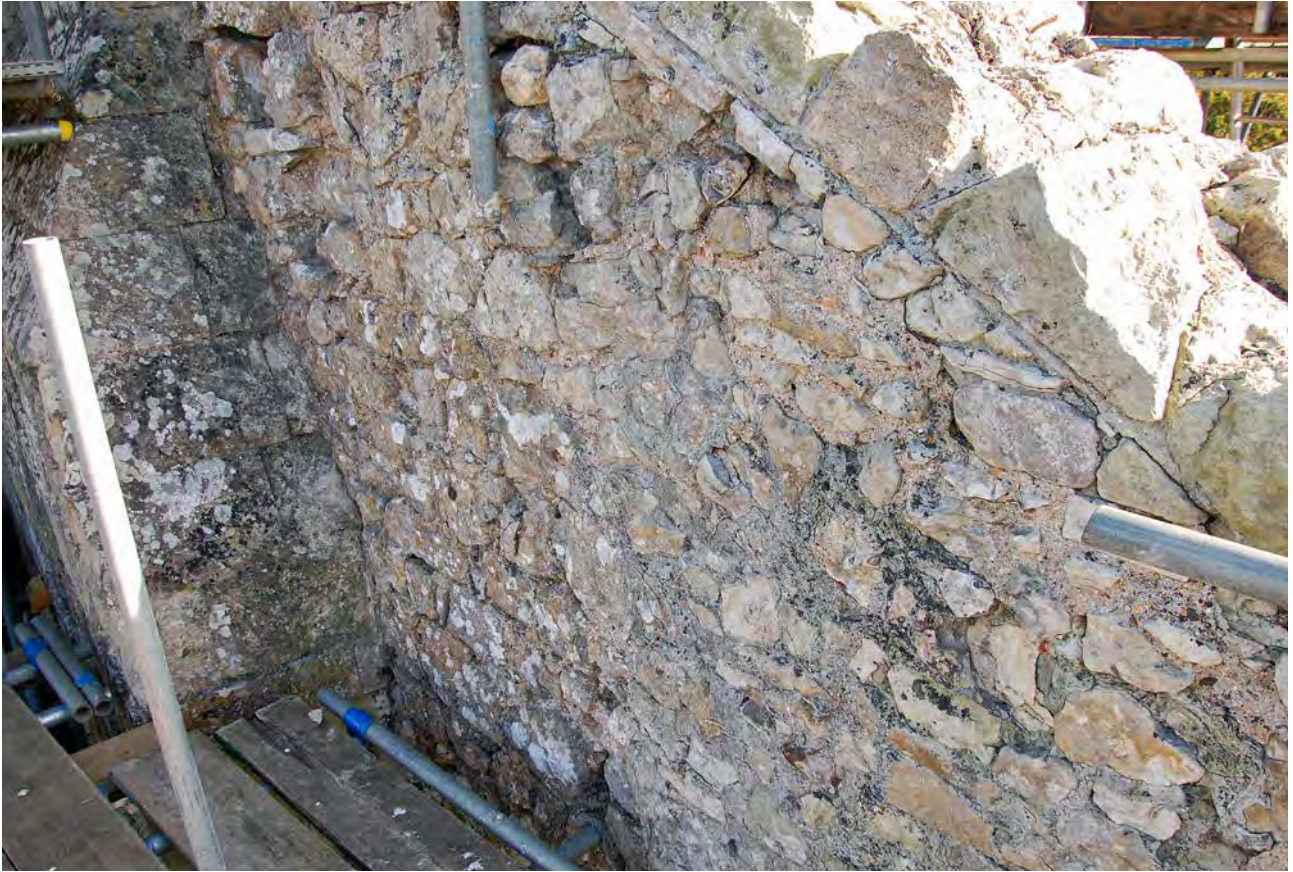
Plate 44: General view of wall at level 8
