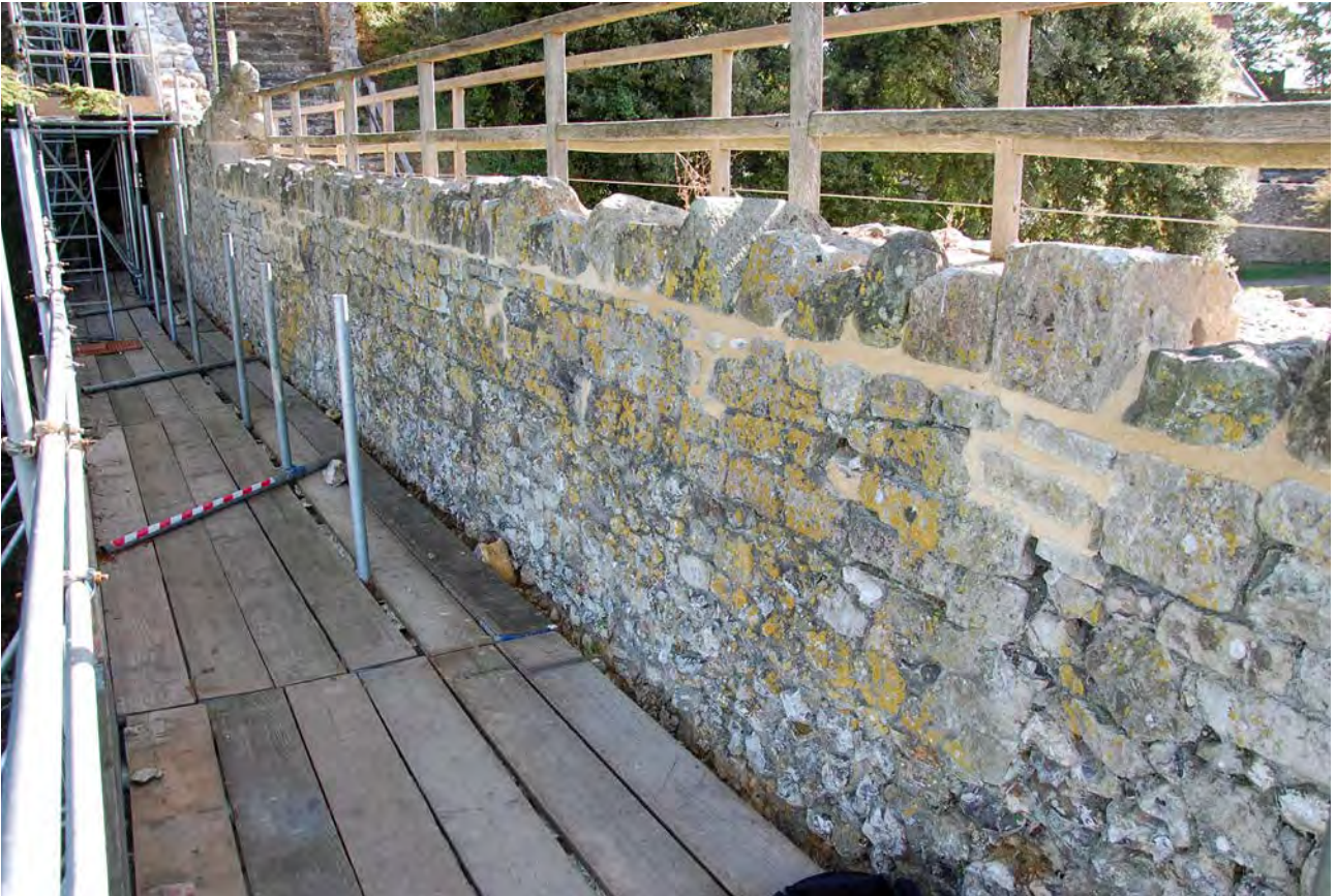
Plate 20: Wall top at level 3
