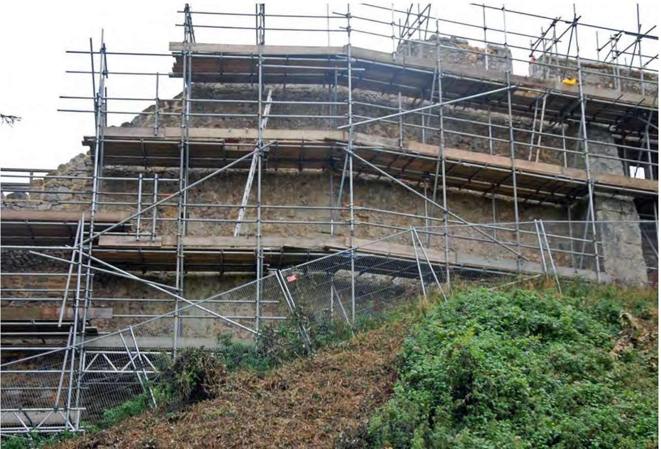
Plate 6: Central part of northern curtain wall
