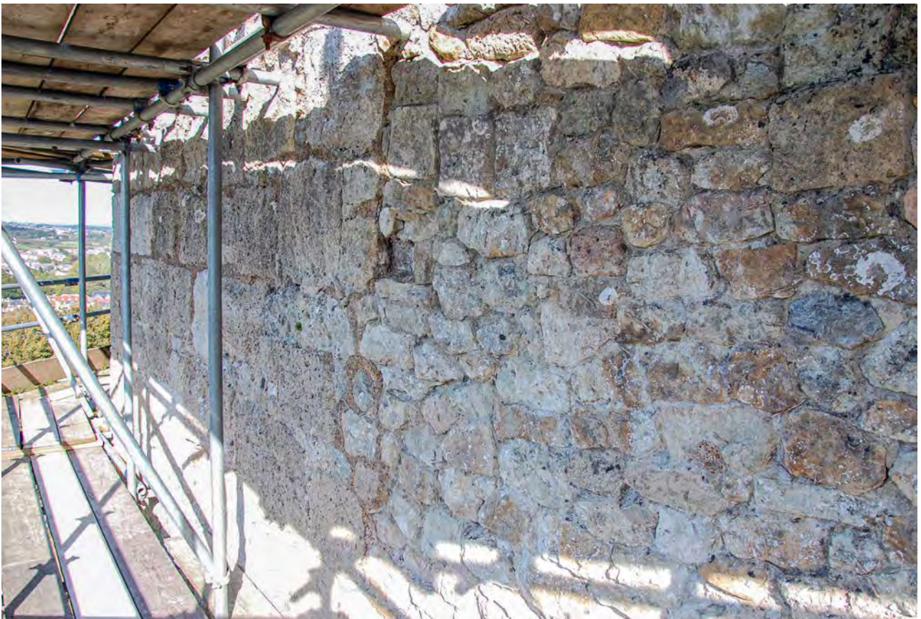
Plate 27: Construction break at level 4
