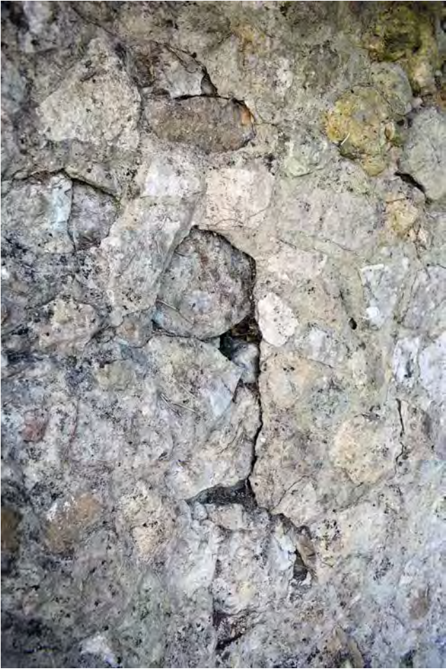
Plate 28: Skim of 20th-century render with stones embedded (level 4)
