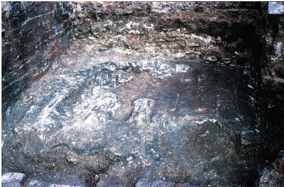
Plate 3.15 Site 29 the Oracle: view looking NW at a detail of demolished or collapsed workhouse wall and ceiling plaster showing the impressions of laths in the untruncated northern part of the west range (Project Phase 8)
