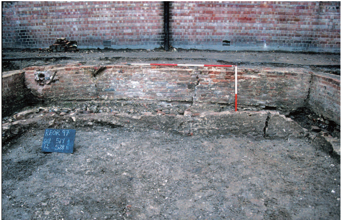
Plate 3.29 Site 12: the Yield Hall: view looking NW showing the problems of subsidence affecting two phases of walls (Project Phase 8)
