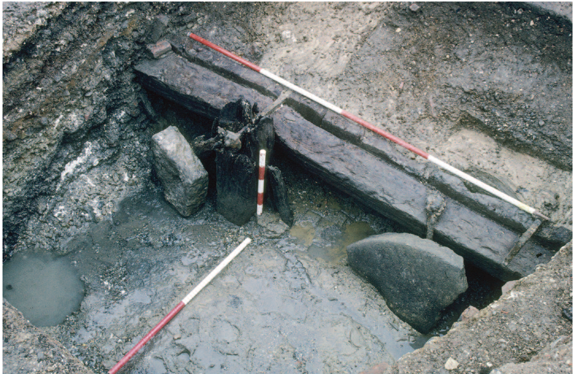
Plate 3.44 Site 300 St Giles Mill: view looking NW showing the mill tail revetment structure as seen in Test Pit 362 (Project Phase 9)
