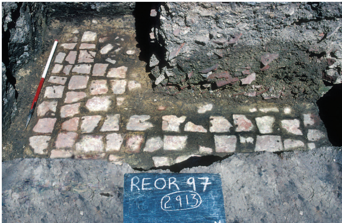
Plate 3.26 Site 12: the Yield Hall (above) view looking NE showing cellar 967 with a later brick reflooring, and (below) with original flooring of reused ceramic rooftiles (Project Phase 7)
