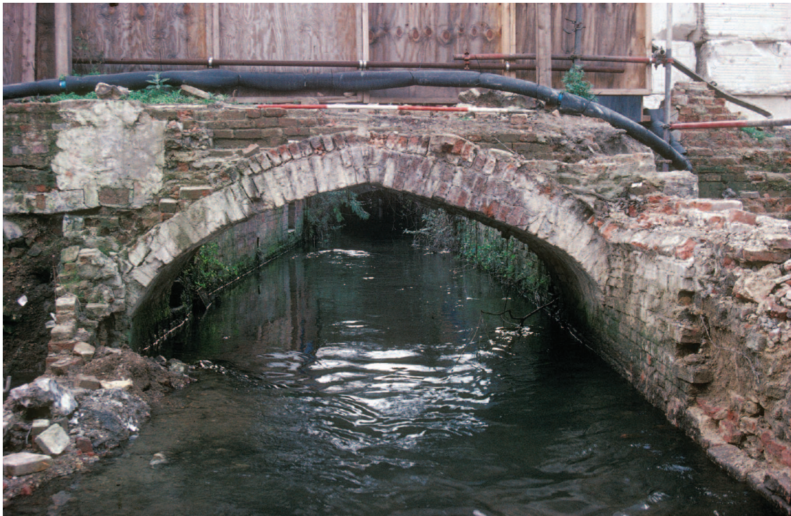
Plate 3.8 Site 29 the Oracle: view looking SW at original brick bridge 6015 which carried the western range of the workhouse over the Holy Brook (Project Phase 7)
