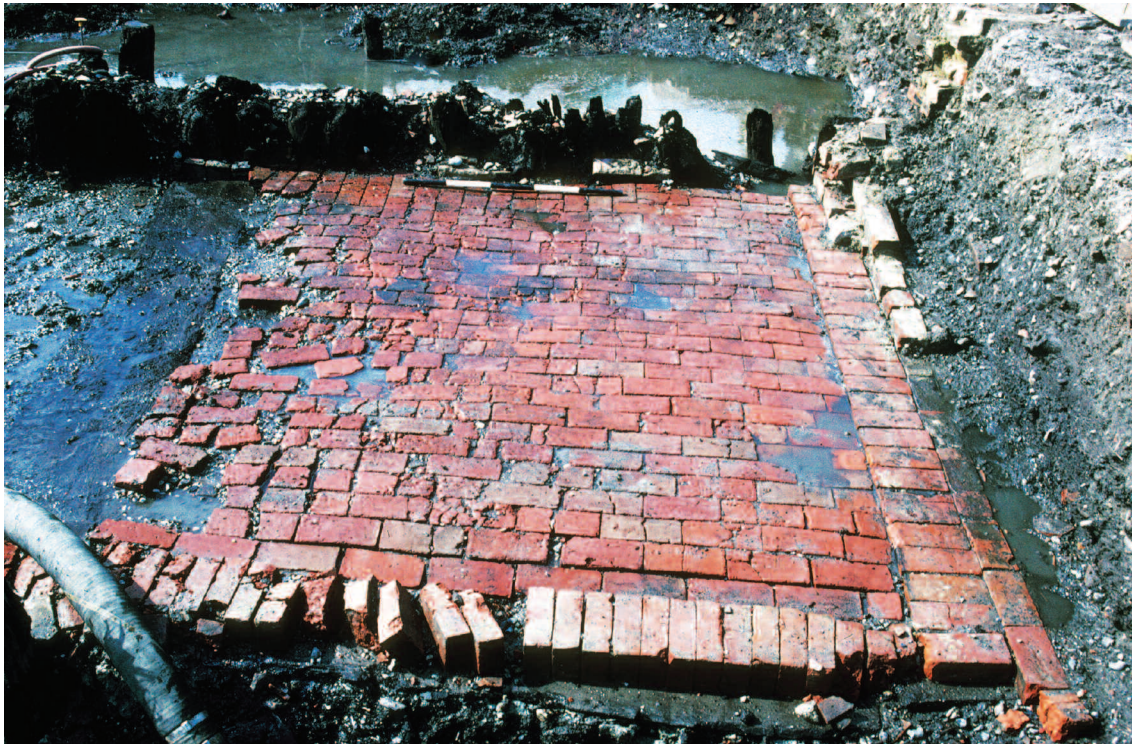
Plate 3.33 Site 101: the Back Brook, view looking NW showing the well-built brick surface 7122 constructed on the southern bank of the Back Brook (Project Phase 7); the Back Brook and its substantial revetment can be seen in the background
