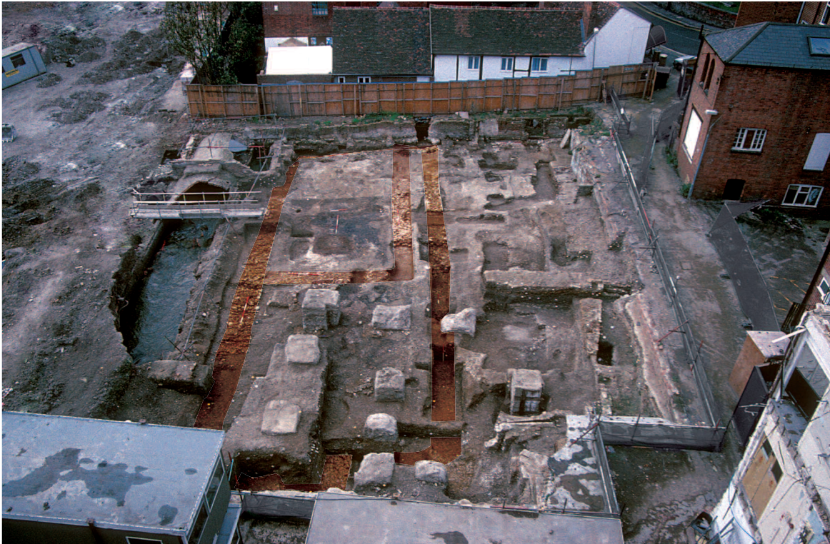
Plate 2.10 Site 29: view looking SW showing Building 5860 (highlighted, along with Building 5840) (Project Phase 4). It is interesting to note that the northern wall of this building (partially robbed) is on the same alignment as the boundary between the two standing buildings immediately beyond the site
