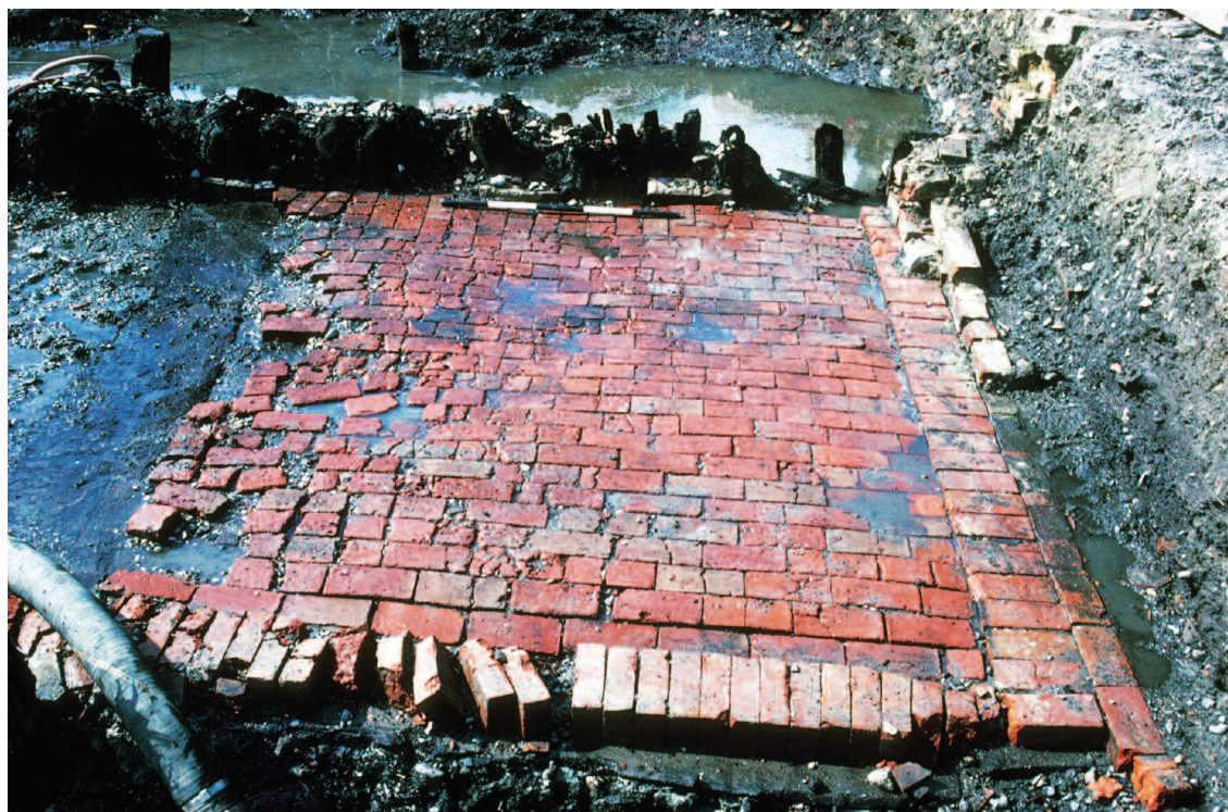
Plate 3.33 Site 101: the Back Brook, view looking NW showing the well-built brick surface 7122 constructed on the southern bank of the Back Brook (Project Phase 7); the Back Brook and its substantial revetment can be seen in the background
