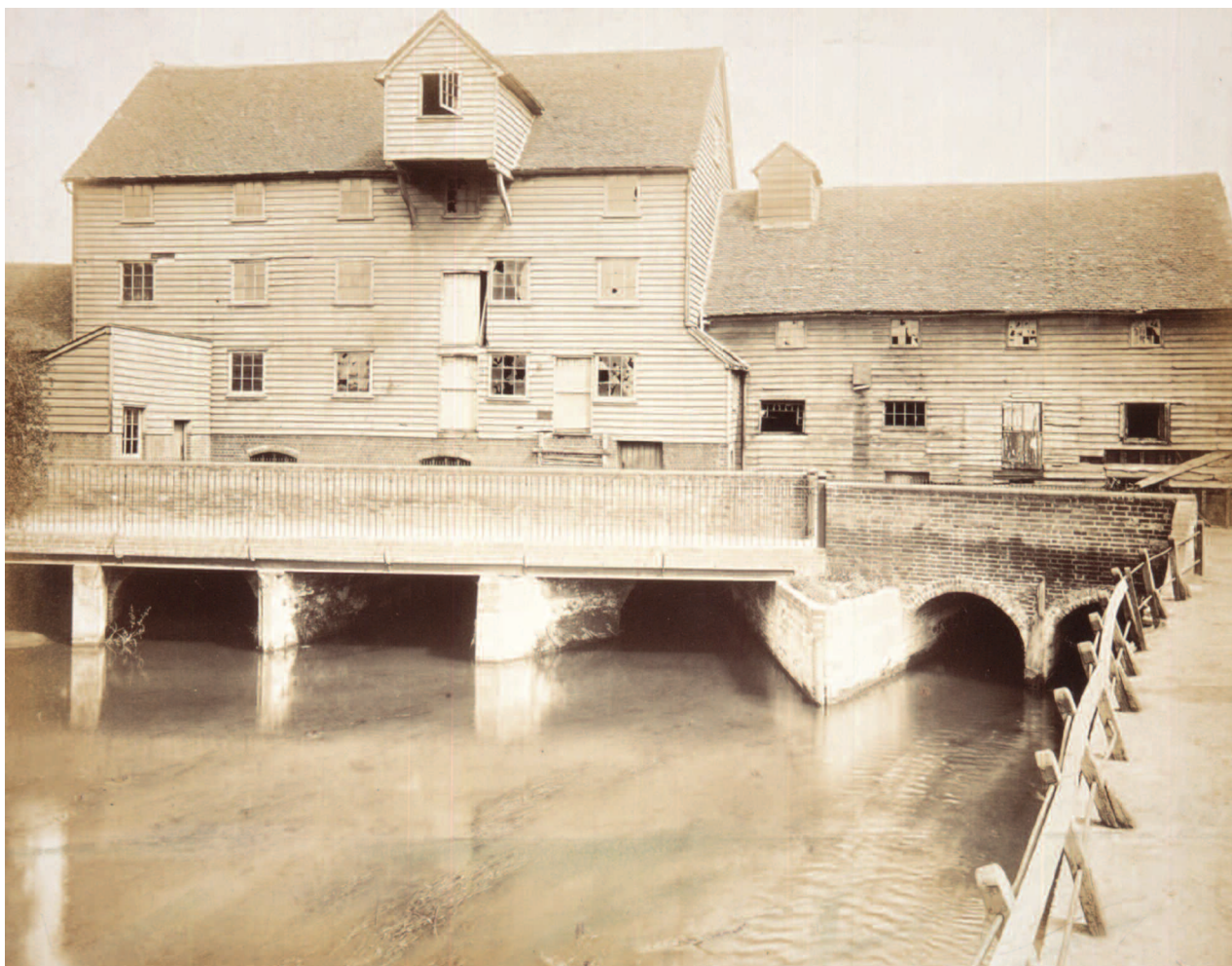
Plate 3.40 Site 300 St Giles Mill, photograph looking NE of the south-west elevation of the mill taken around 1900; the larger buildings added in the 18th century are on the left, with the smaller 17th-century buildings on the right
