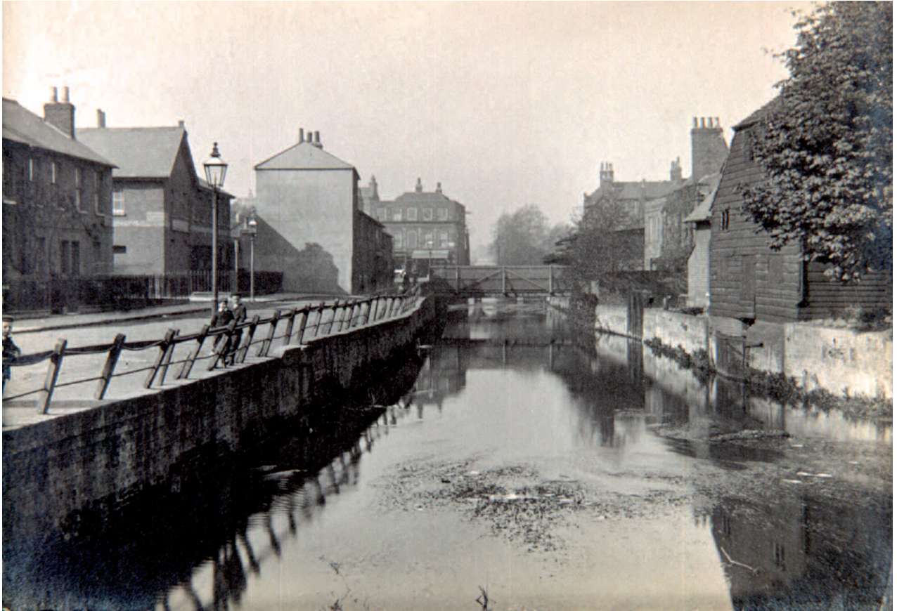
Plate 3.39 Photograph looking NW along Mill Lane showing the water pumping mill towards the centre of the photograph, immediately behind the tree, view c 1900
