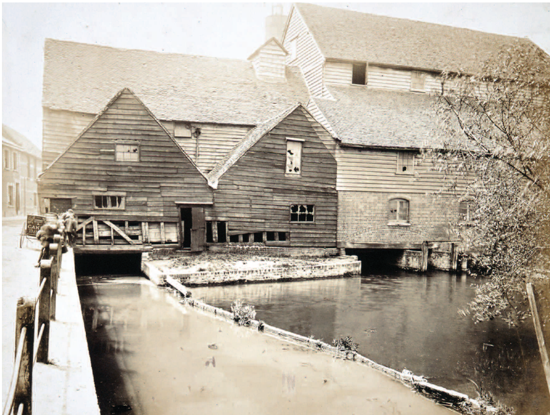
Plate 3.36 Site 300 St Giles Mill: photograph looking SW of the east elevation of the mill taken c 1900; on the left is the 17th-century mill, with the more substantial buildings of the 18th-century rebuild to the right (Project Phase 7)
