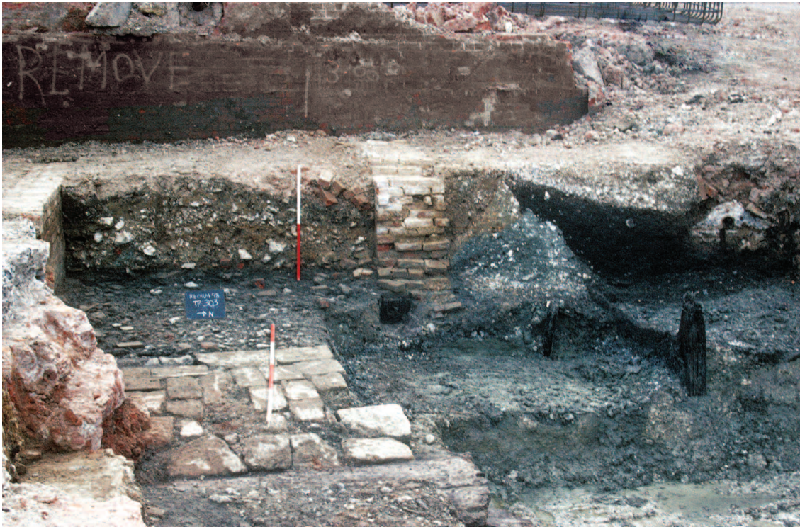
Plate 3.41 Site 300 St Giles Mill: view looking SW showing a section through the central mill channel and retaining wall upstream from the mill (Project Phase 9)
