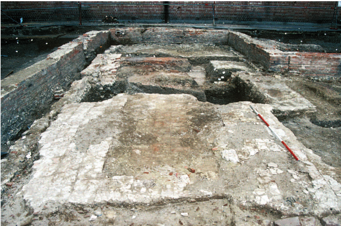
Plate 3.25 Site 12: the Yield Hall, view looking NW showing mortar bedding layer with the impressions of ceramic tiles or bricks for floor 716 in Room 4 (Project Phase 7)
