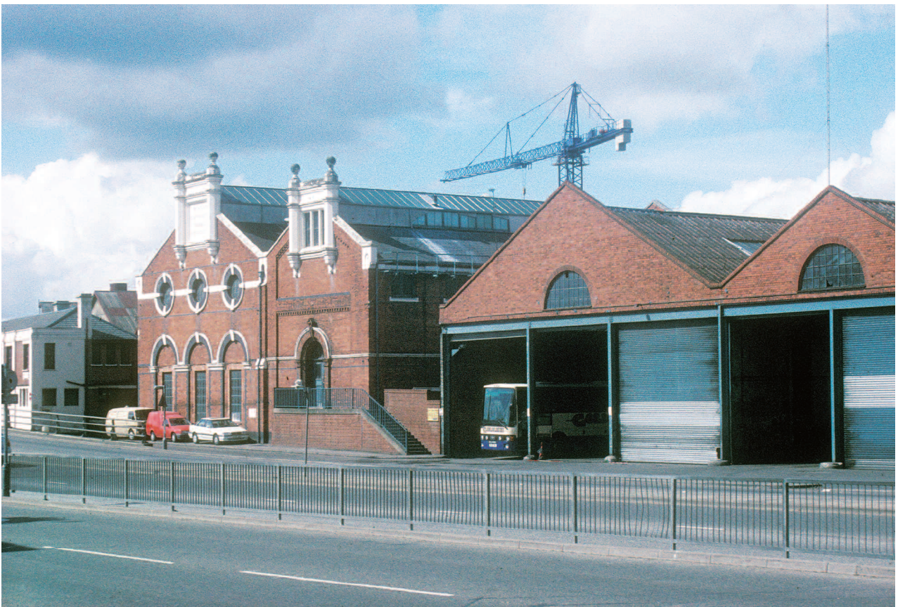
Plate 3.49 View looking W of Reading Bus Depot immediately prior to demolition
