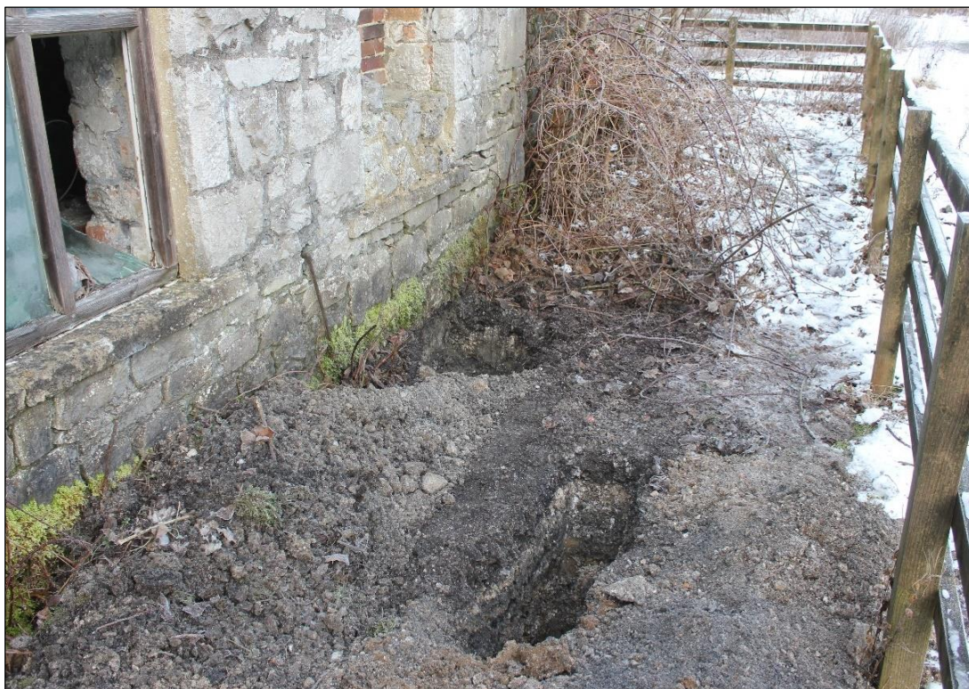
Plate 4: Test-pits against the eastern elevation of the single-storey shed (OA3)
