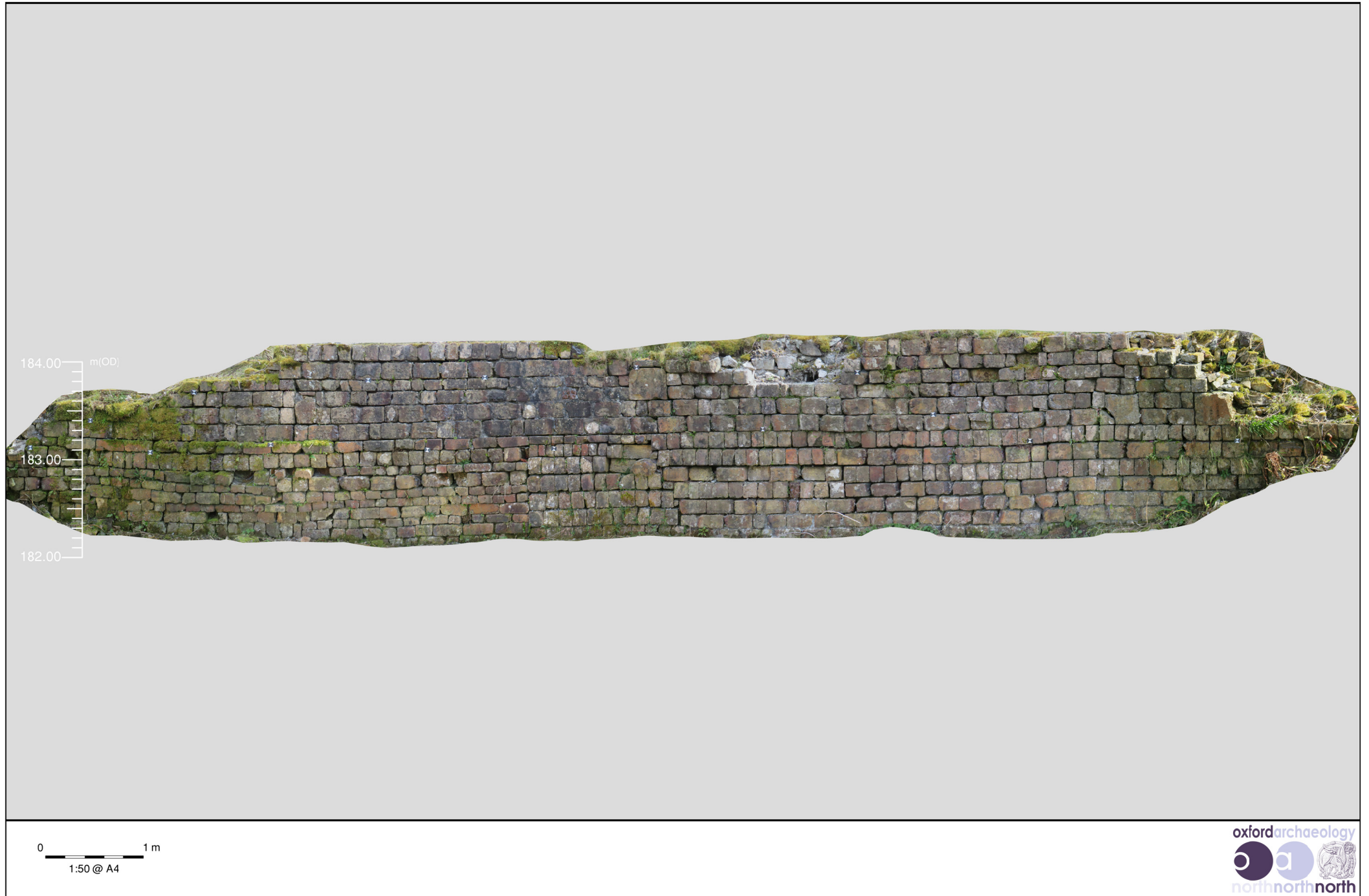
Figure 9: Photogrammetric model of the extant remains of the loading bay wall
