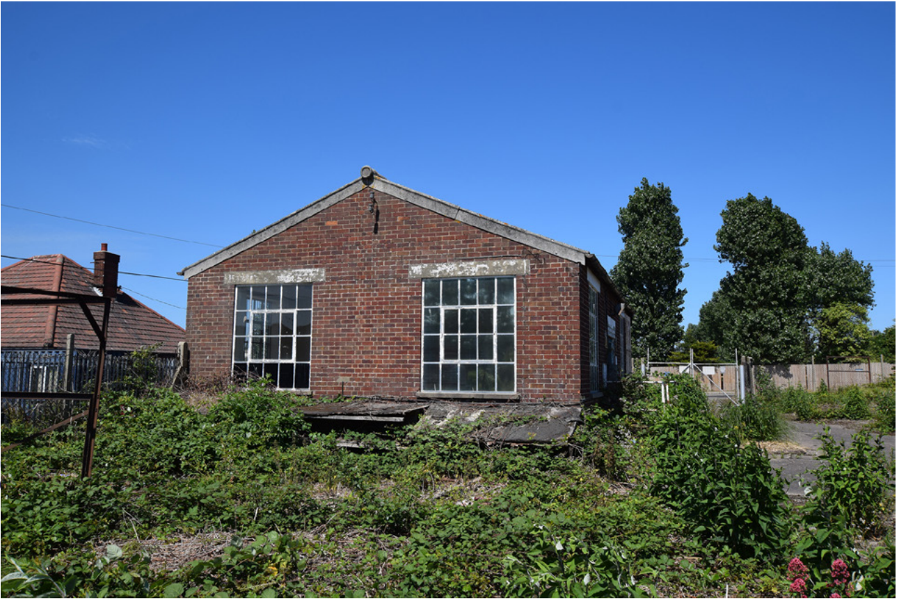
Plate 43: The south elevation of the office building
