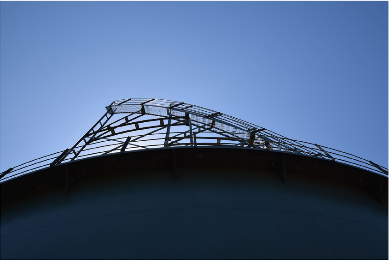
Plate 15: The steps to the lifts
