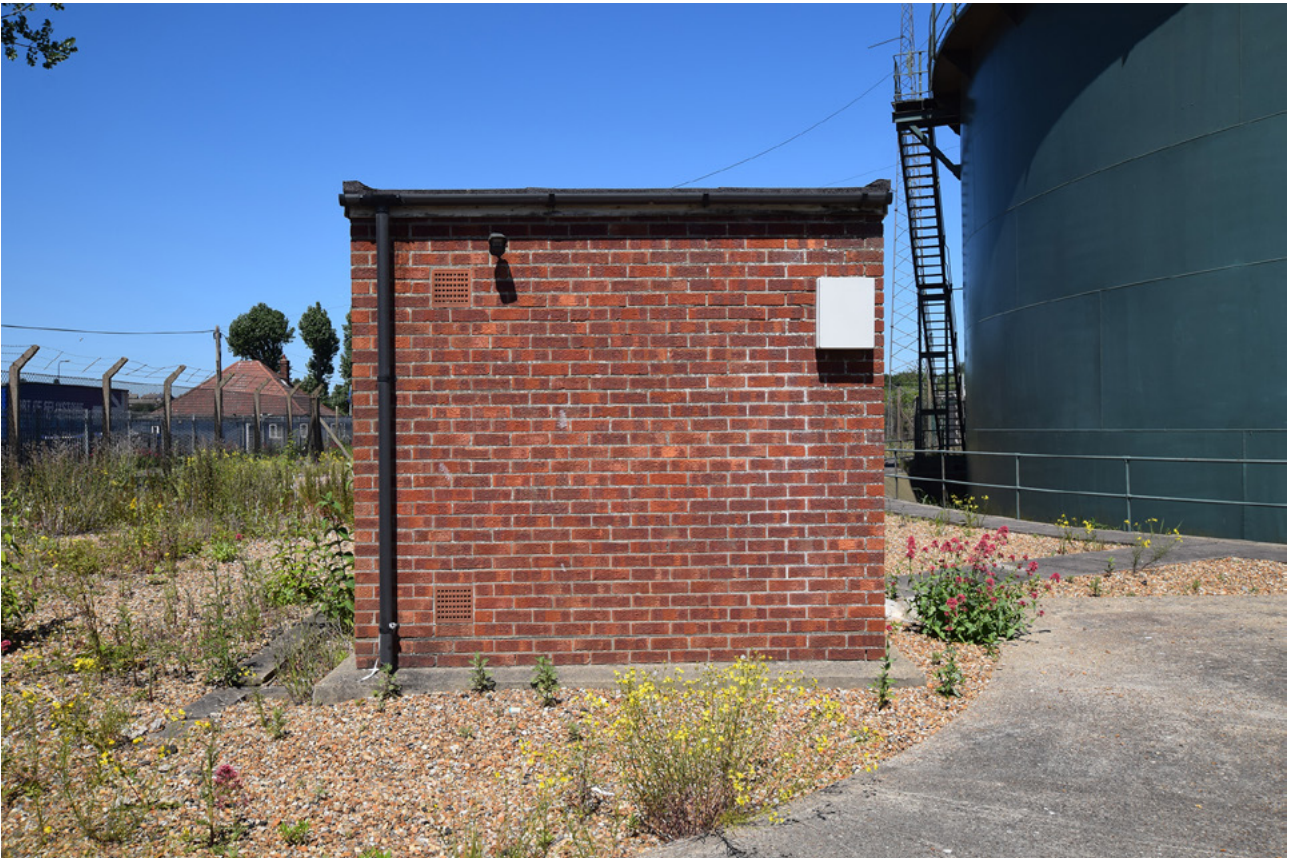
Plate 32: The south elevation of the brick building
