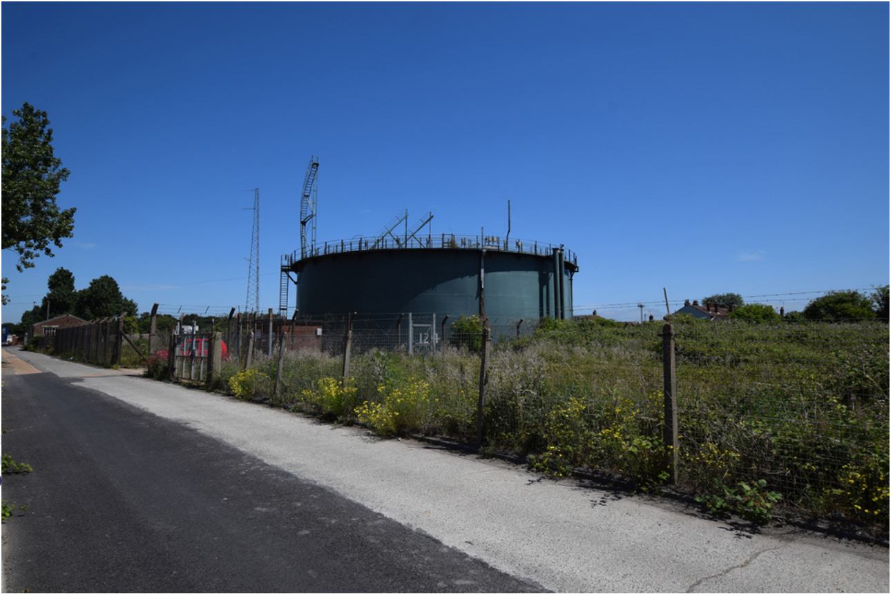
Plate 7: The view of the site from the service road, looking north-east
