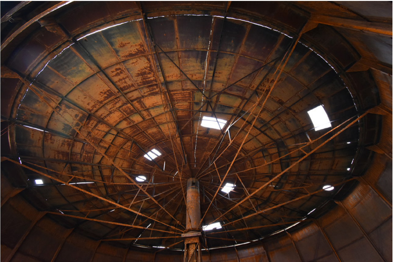
Plate 26: The crown structure
