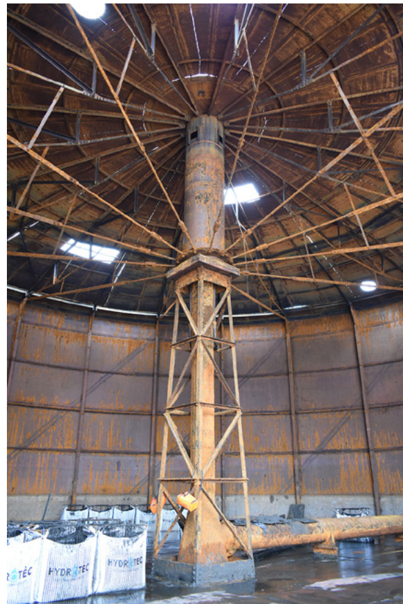
Plate 28: The support structure
