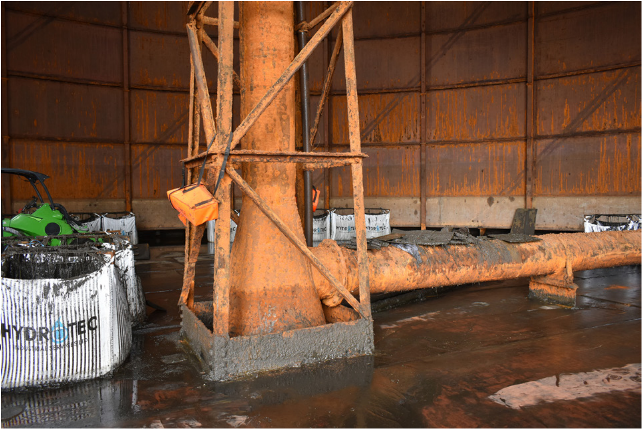
Plate 29: The base of the support structure
