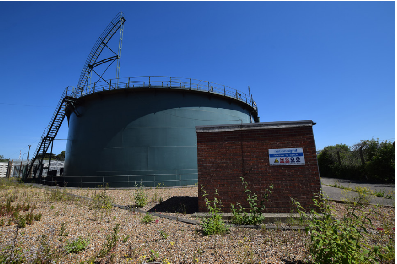
Plate 31: The brick building in relation to the gasholder, looking east
