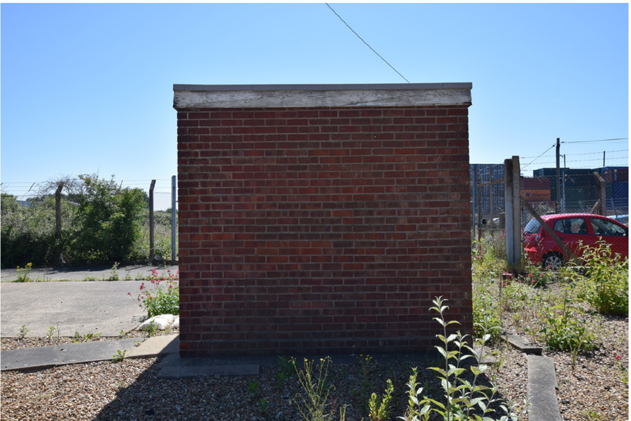
Plate 34: The north elevation of the brick building
