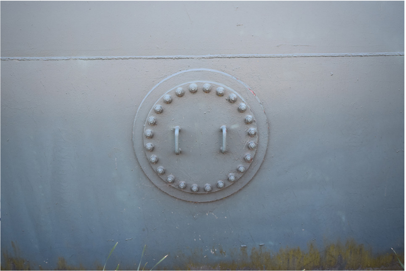
Plate 11: The access hatch at the north of the gasholder
