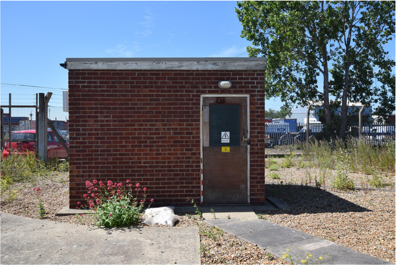
Plate 33: The east elevation of the brick building
