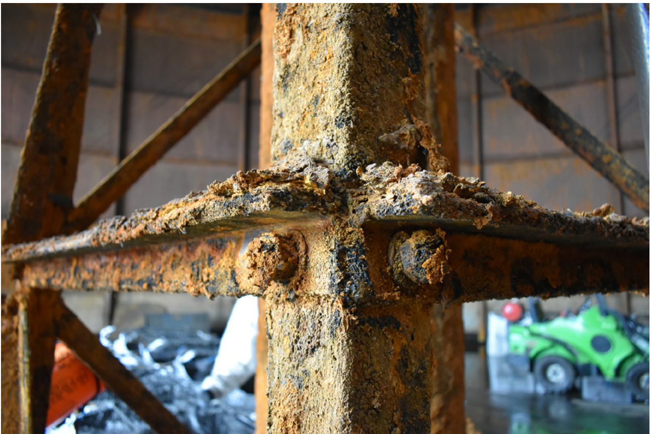
Plate 30: An example of the bolted joints
