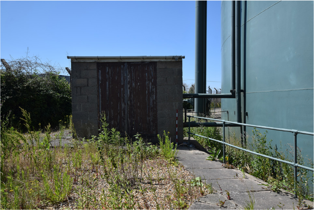
Plate 37: The east elevation of the concrete block building
