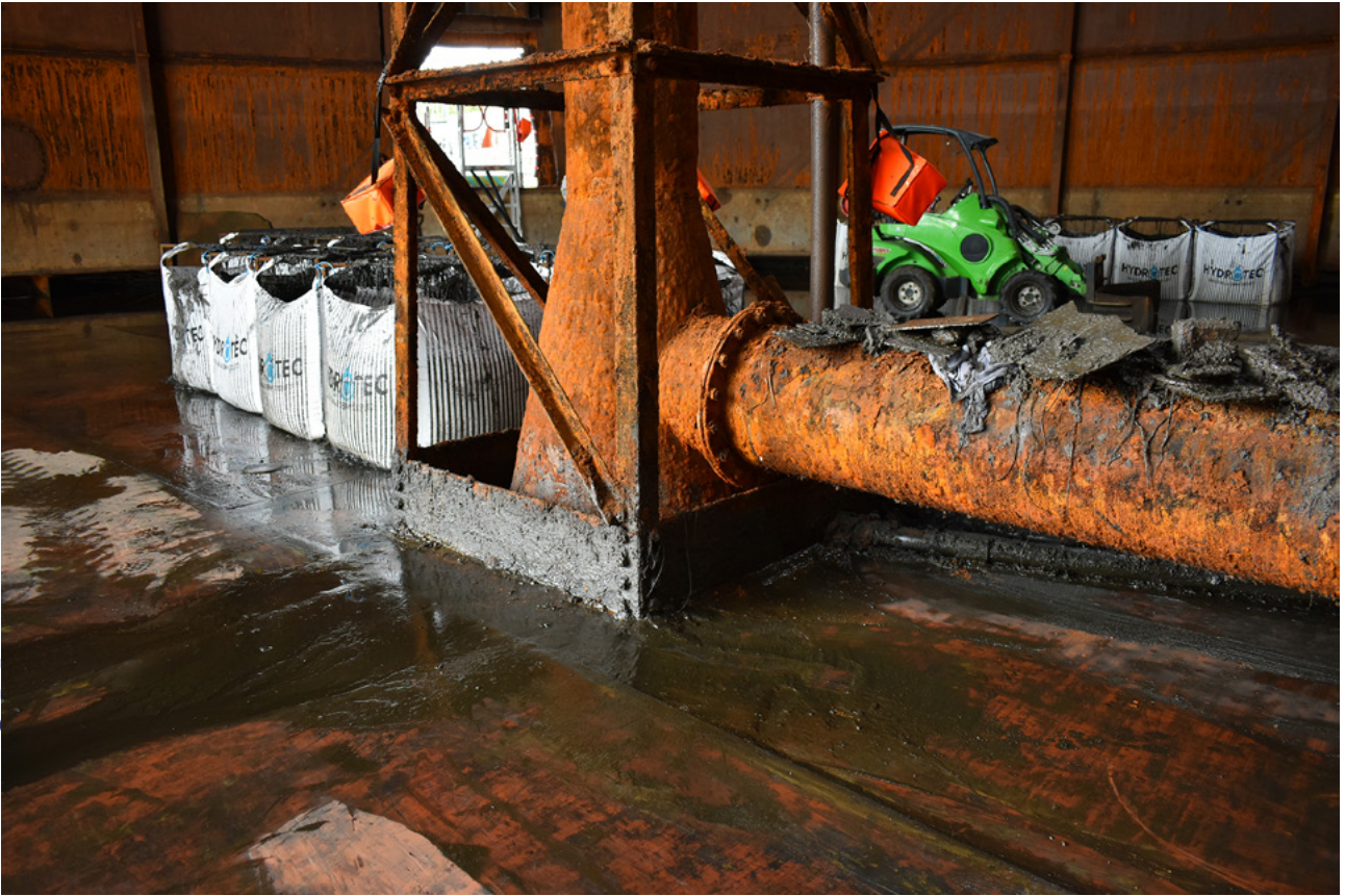
Plate 25: The inlet/outlet pipe inside the support post
