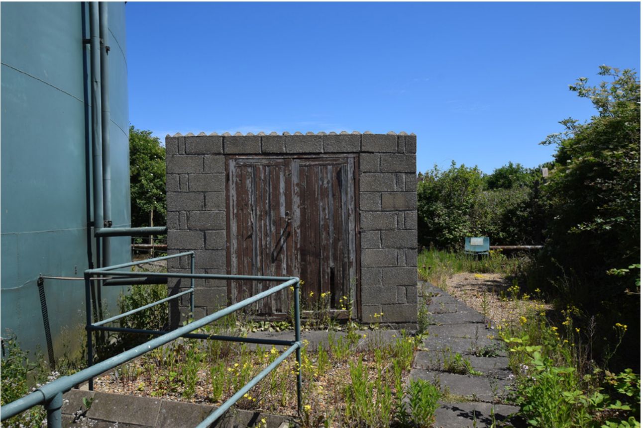
Plate 38: The west elevation of the concrete block building
