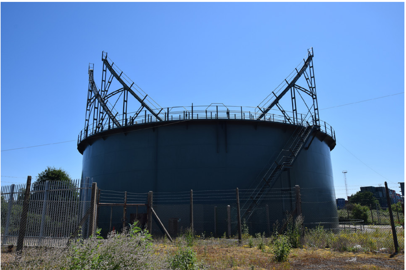
Plate 14: The steps to the top of the tank and lifts
