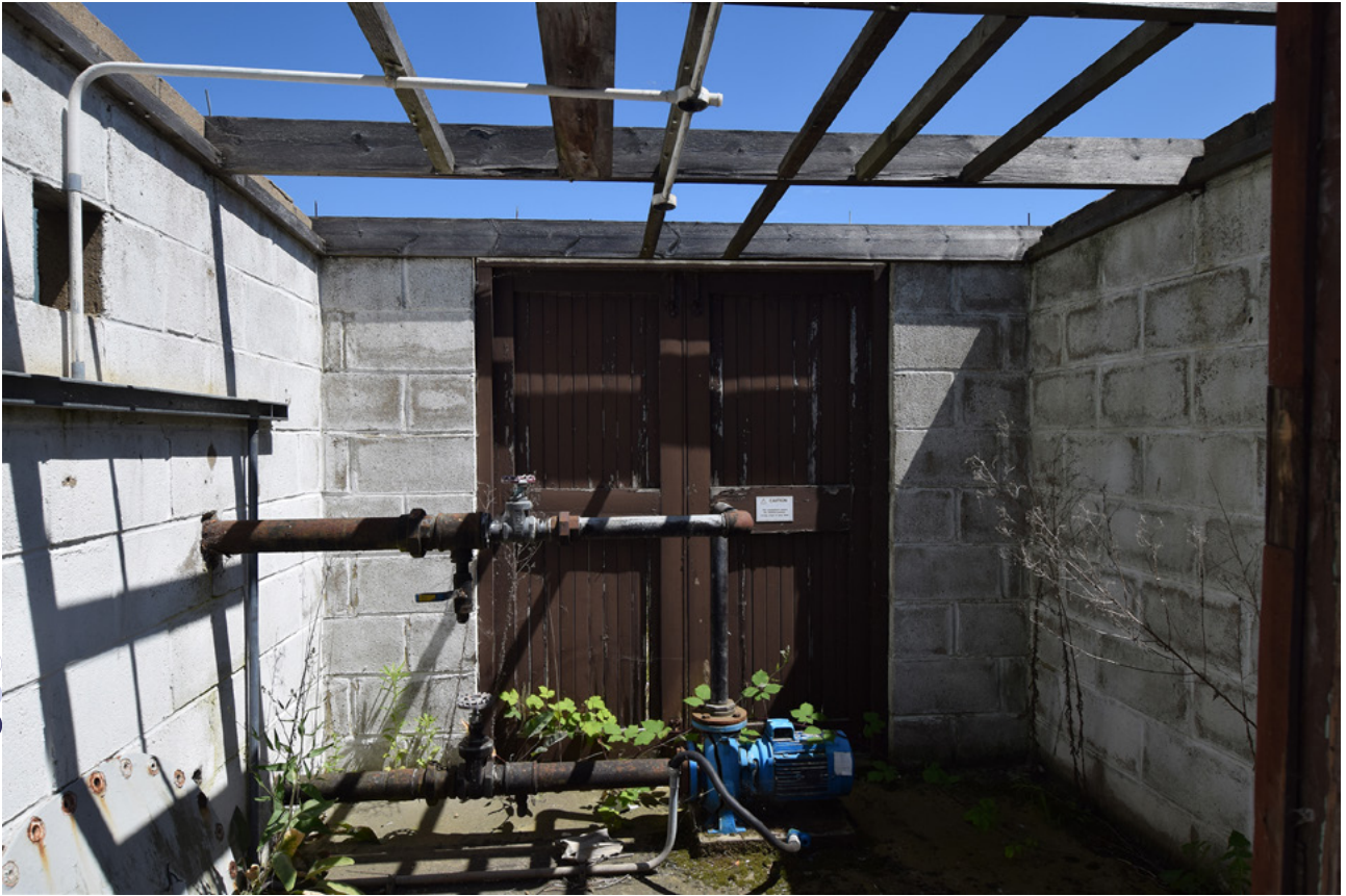
Plate 39: The interior of the concrete block building, looking east
