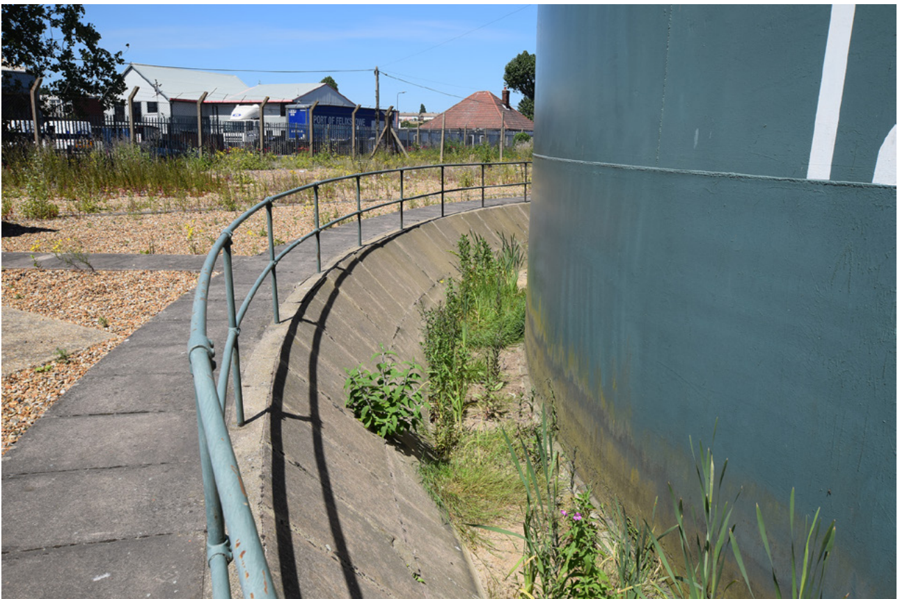
Plate 10: The bund surrounding the gasholder
