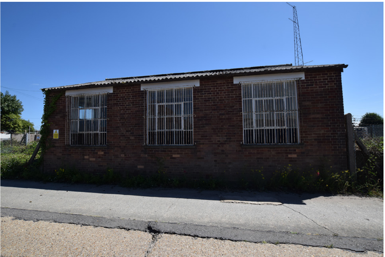
Plate 42: The west elevation of the office building
