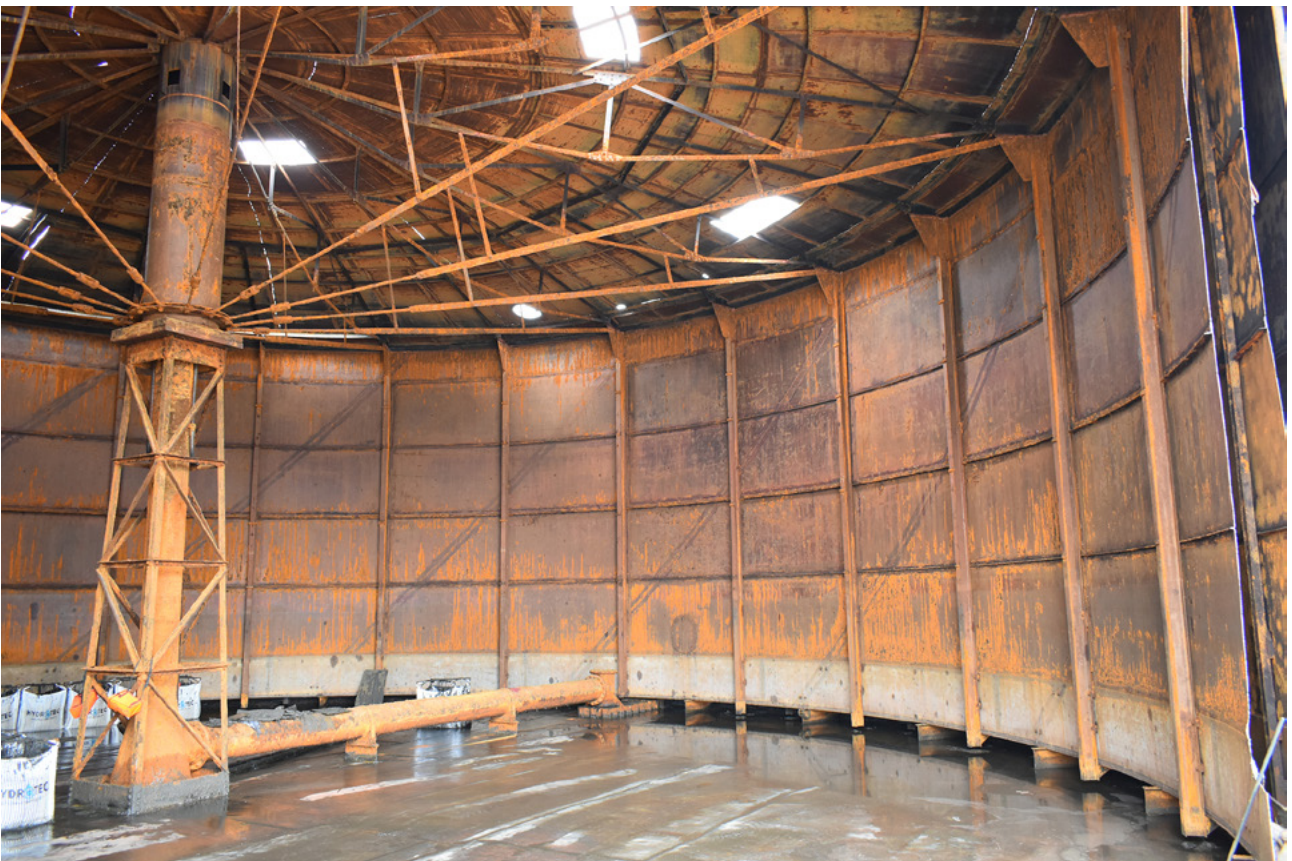
Plate 22: The interior of the gasholder, looking south
