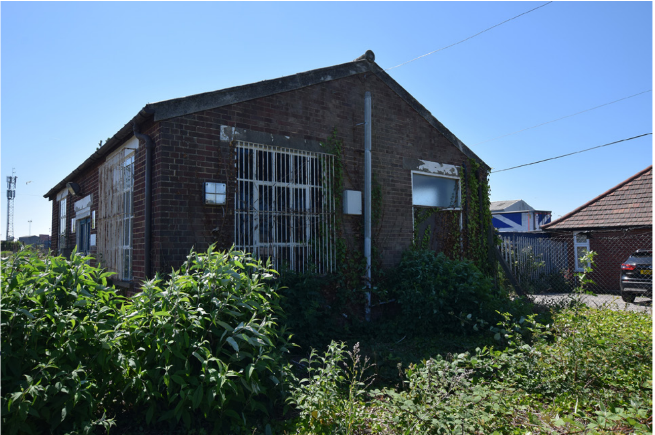
Plate 41: The north elevation of the office building
