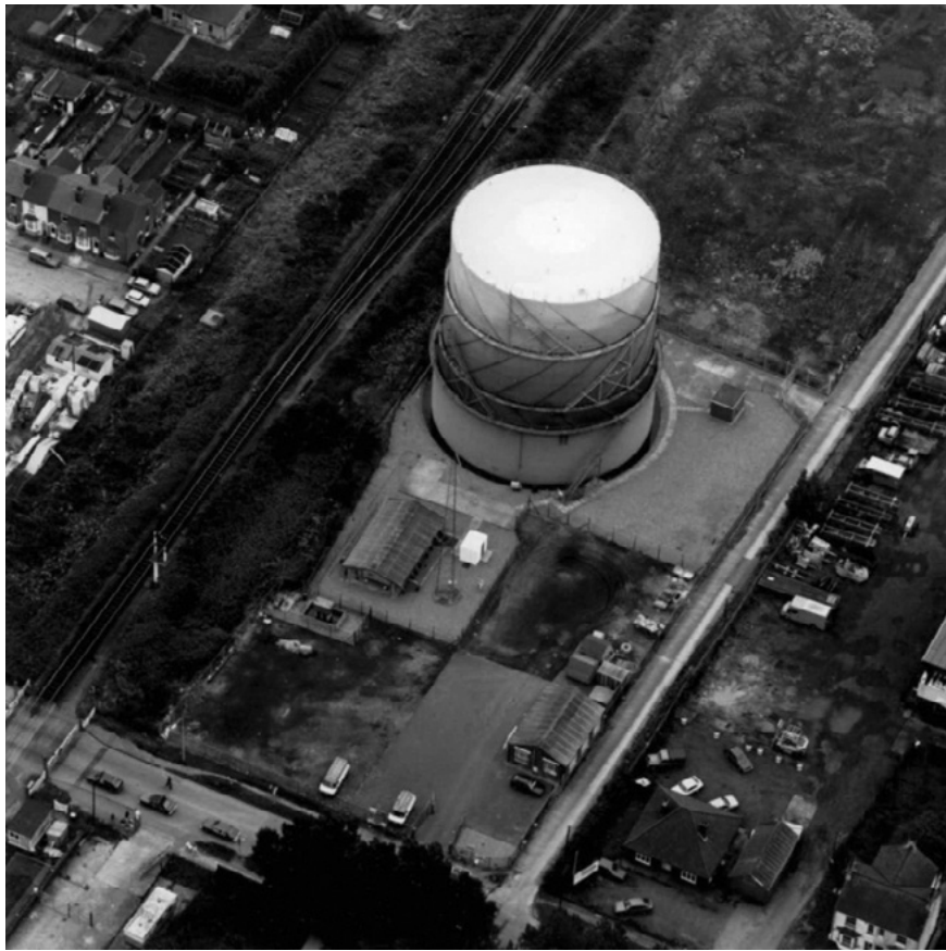
Plate 5: Undated aerial view of the site, looking approximately south. c1970s or 1980s. National Gas Archive Document Reference: EA/DX/E/F/3/xg02643
