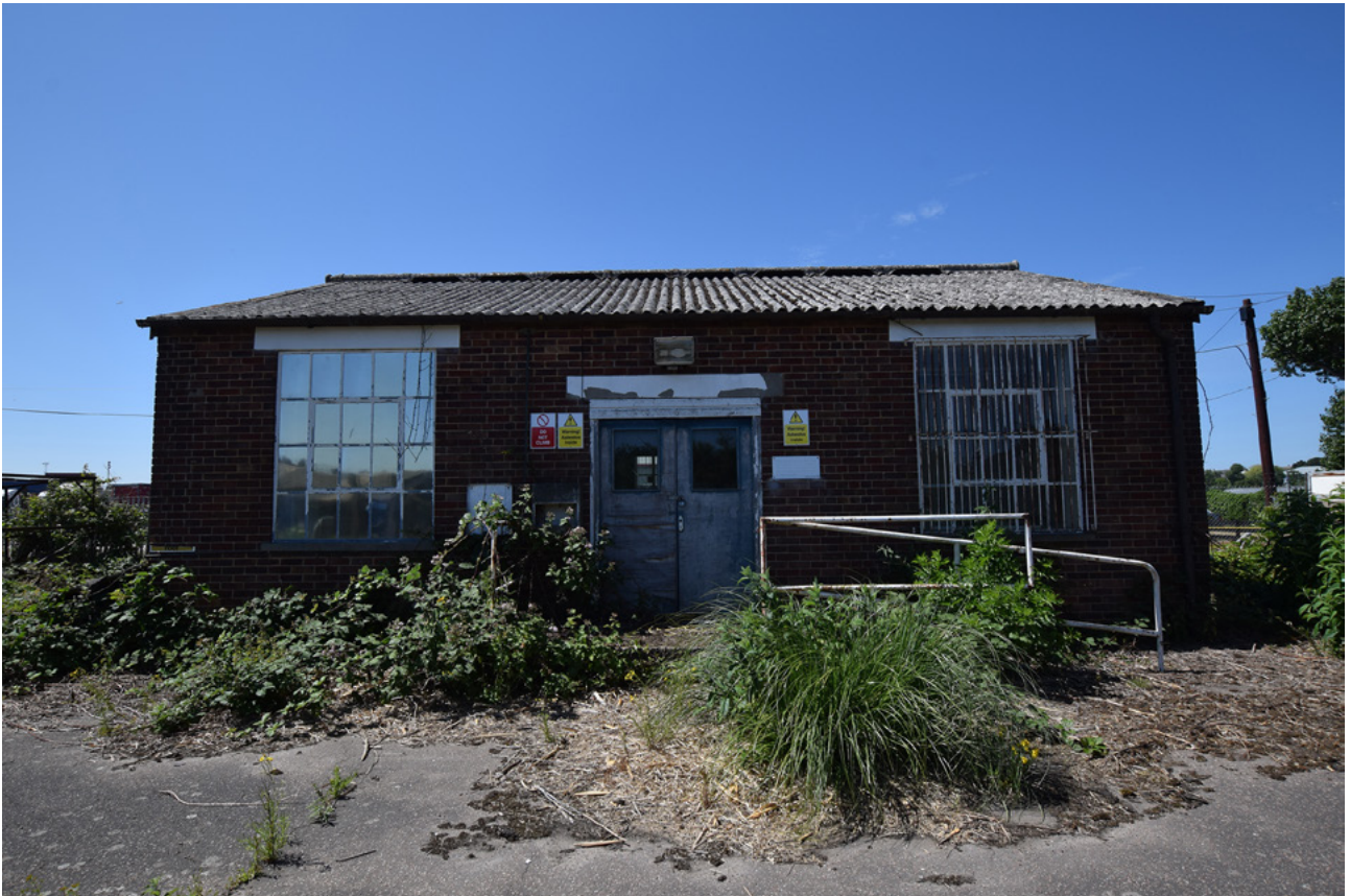
Plate 40: The east elevation of the office building
