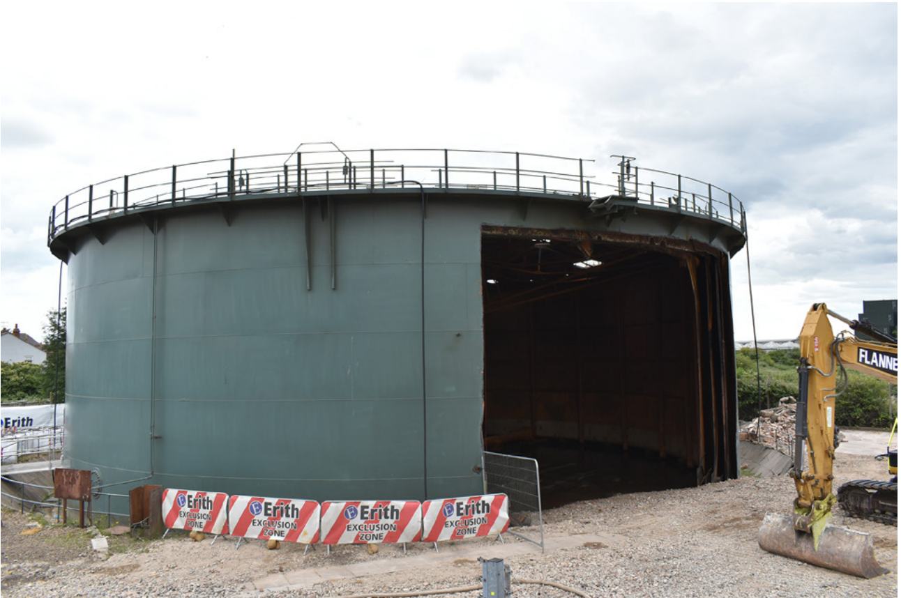
Plate 16: The tank after opening-up and desludging, looking south-east
