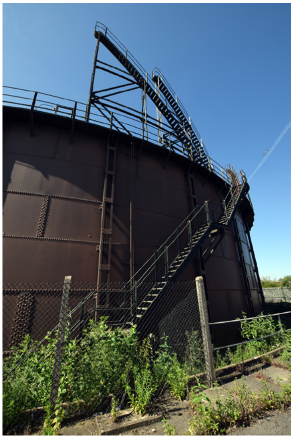
Plate 11: The access stairs viewed from the north-east
