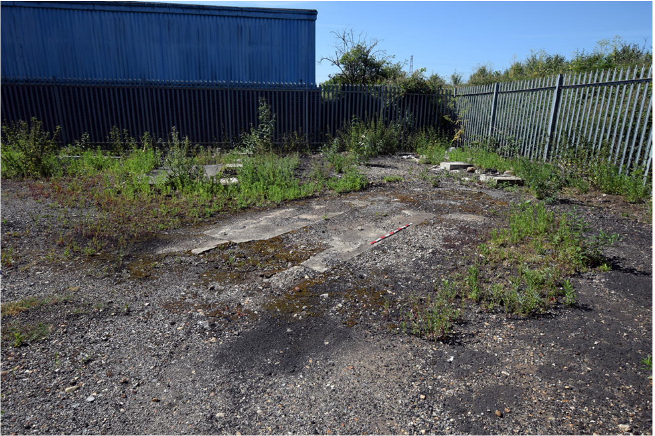
Plate 28: The concrete bases at the south-west of the site, viewed from the north
