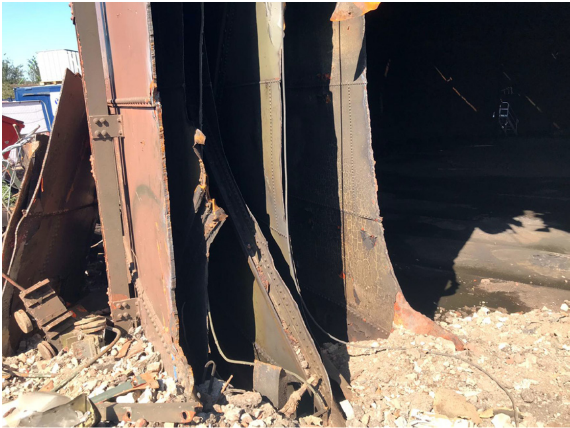
Plate 17: A cross section of the tank and lifts. Photograph provided by Erith Contractors Ltd
