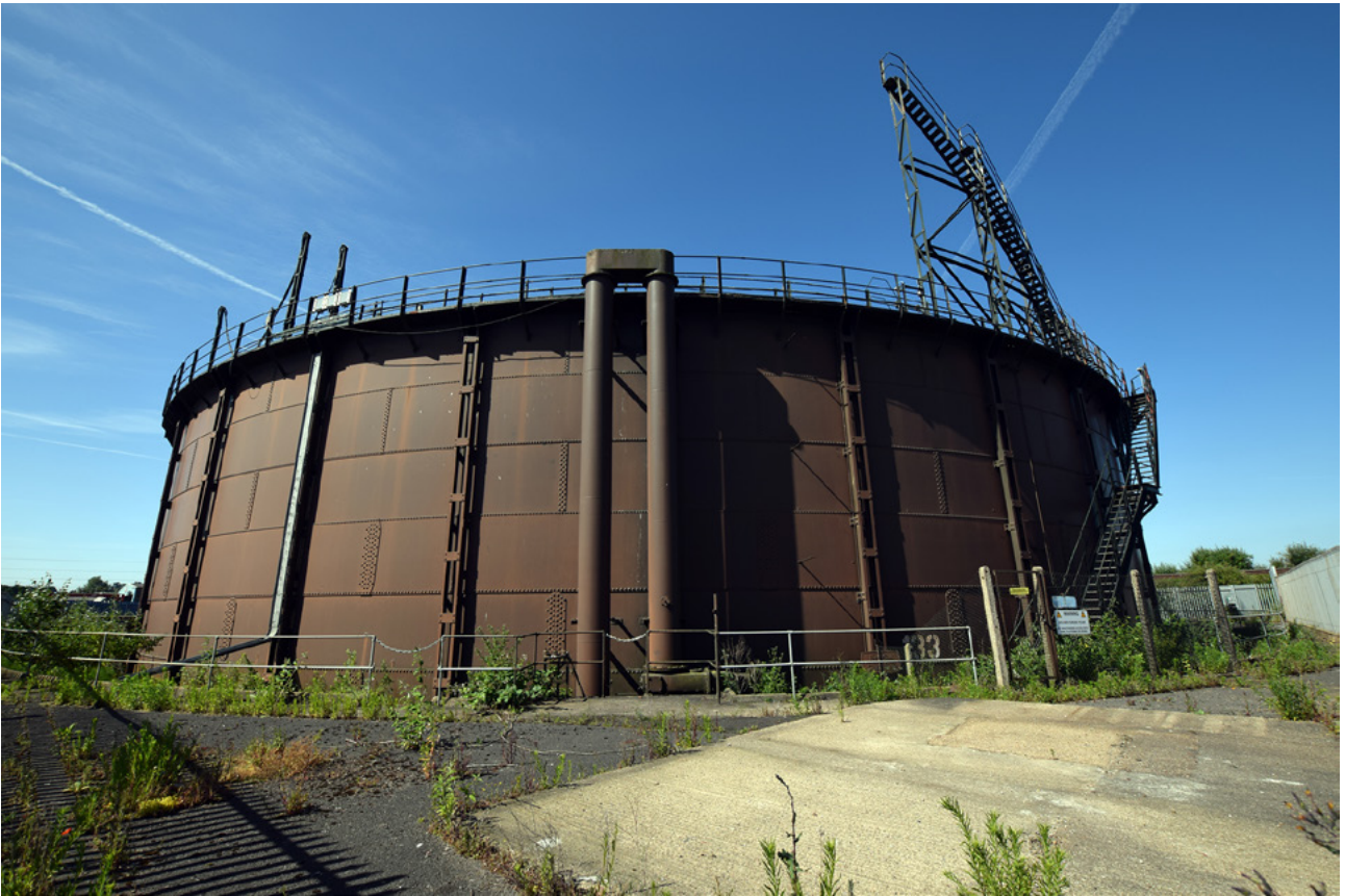
Plate 6: Gasholder viewed from the north-east
