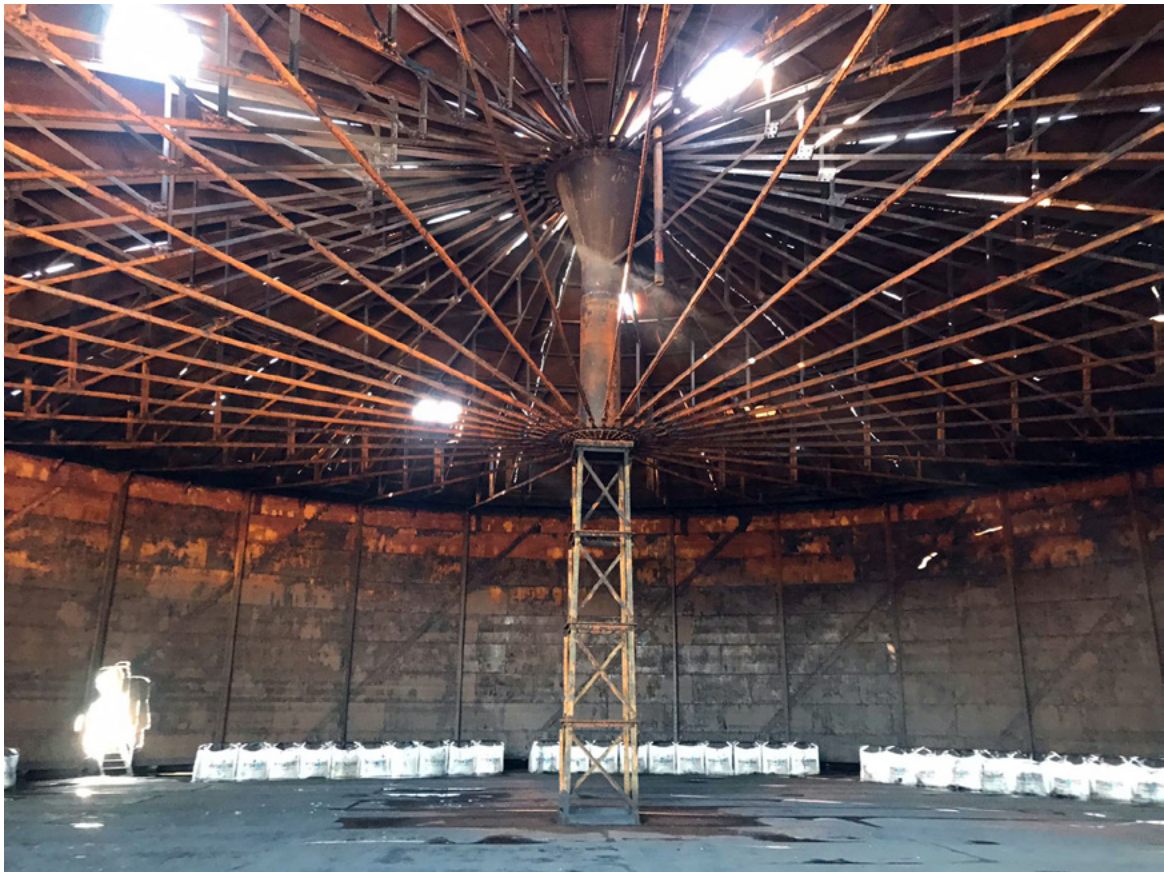
Plate 23: The crown support. Photograph provided by Erith Contractors Ltd
