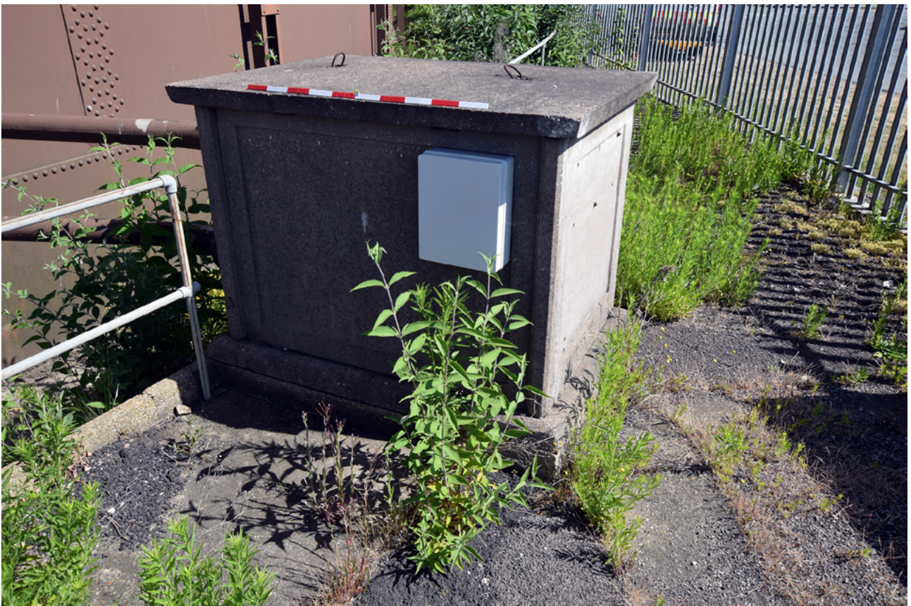
Plate 24: The concrete cabinet at the south east of the gasholder
