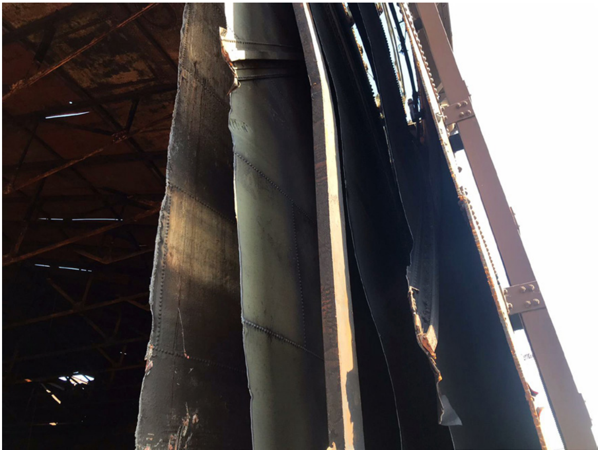
Plate 18: A cross section of the tank and lifts. Photograph provided by Erith Contractors Ltd
