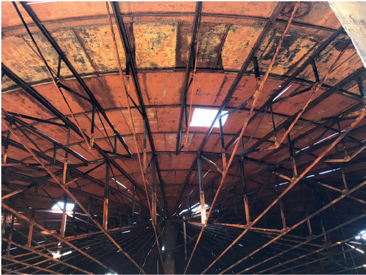
Plate 21: The crown and trusses. Photograph provided by Erith Contractors Ltd
