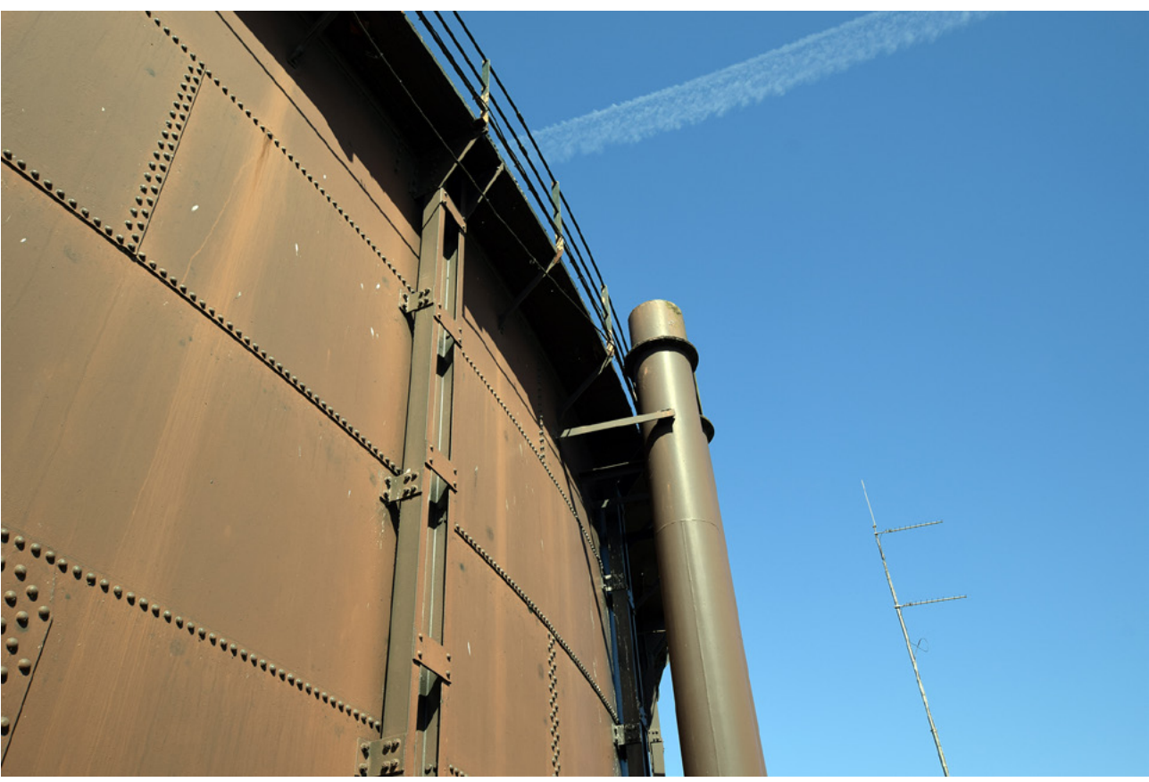
Plate 12: An example of a column and walkway fixing
