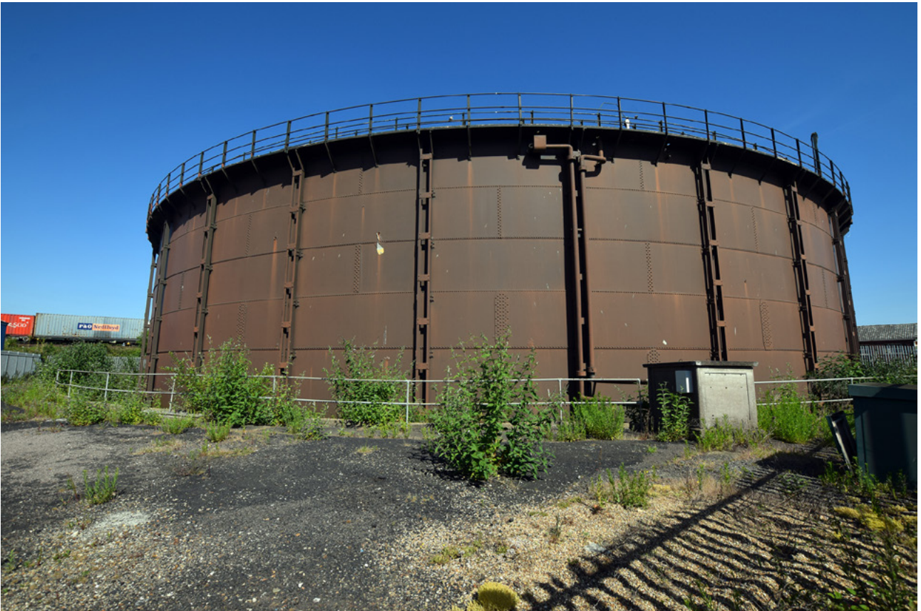
Plate 4: Gasholder viewed from the south-east
