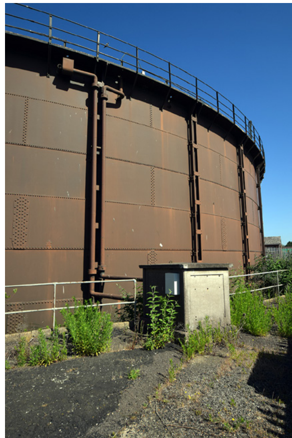
Plate 15: The concrete cabinet and pipework to the south-east of the gasholder
