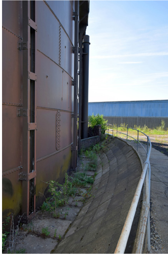
Plate 5: Bund surrounding the gasholder, west side of the gasholder
