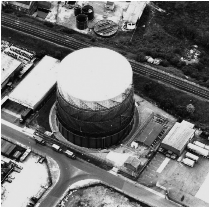
Plate 8: The gasholder almost fully extended. National Gas Archives Document Reference: EA/DX/E/F/5/xg02861
