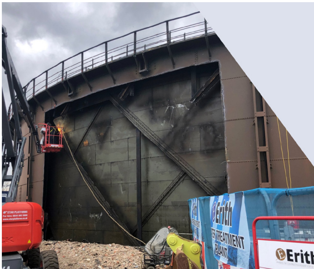
Plate 16: The gasholder during cutting. Photograph provided by Erith Contractors Ltd
