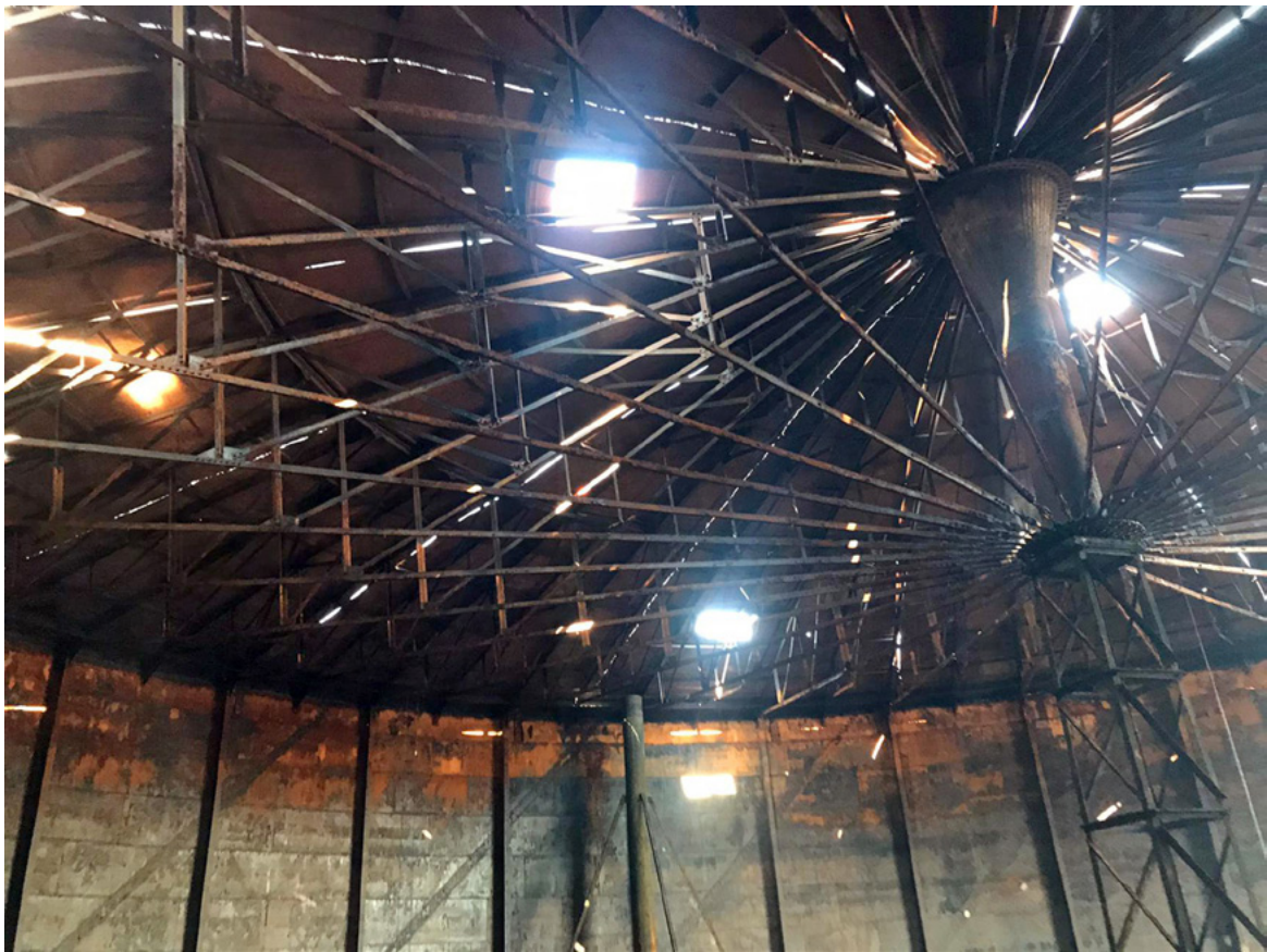
Plate 22: The trusses. Photograph provided by Erith Contractors Ltd
