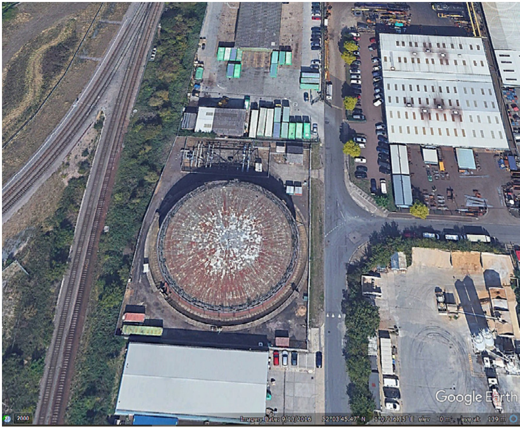
Plate 9: The gasholder station from above. Taken from Google Earth. ©Google
