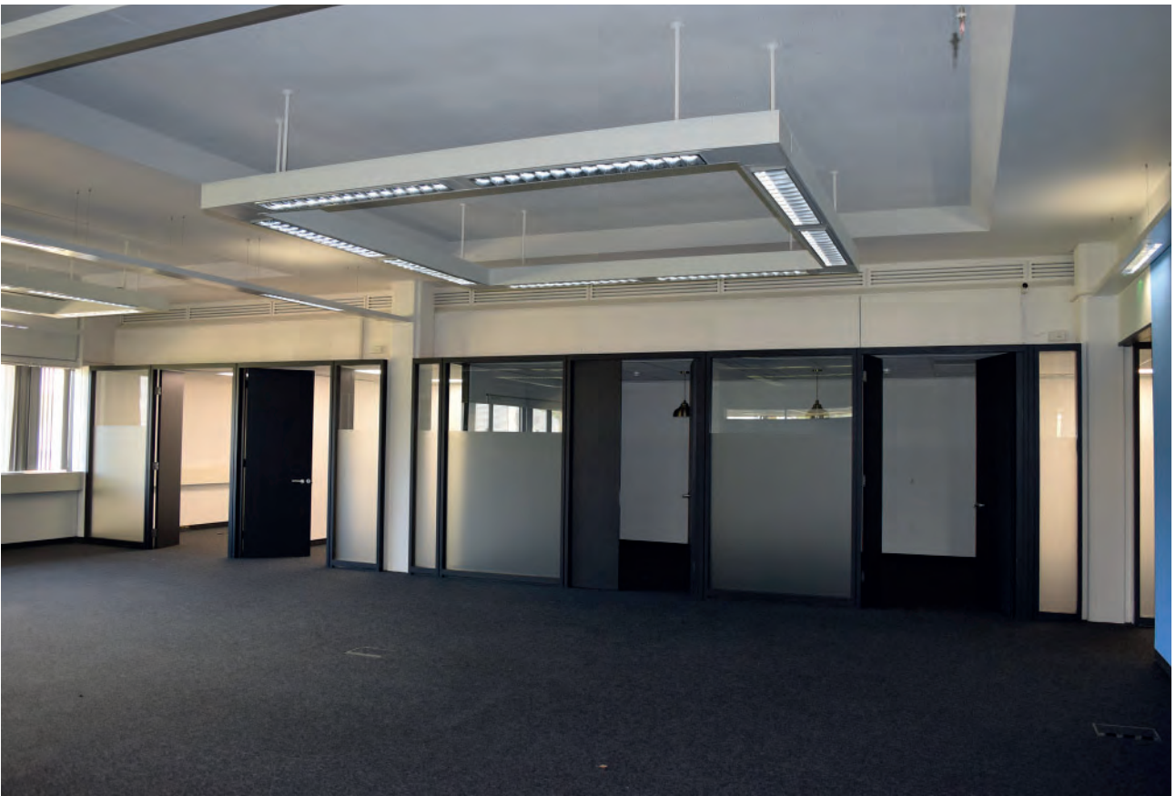
Plate 123: West wing of Building 6000, south office space, office cubicles set, looking north- west.
