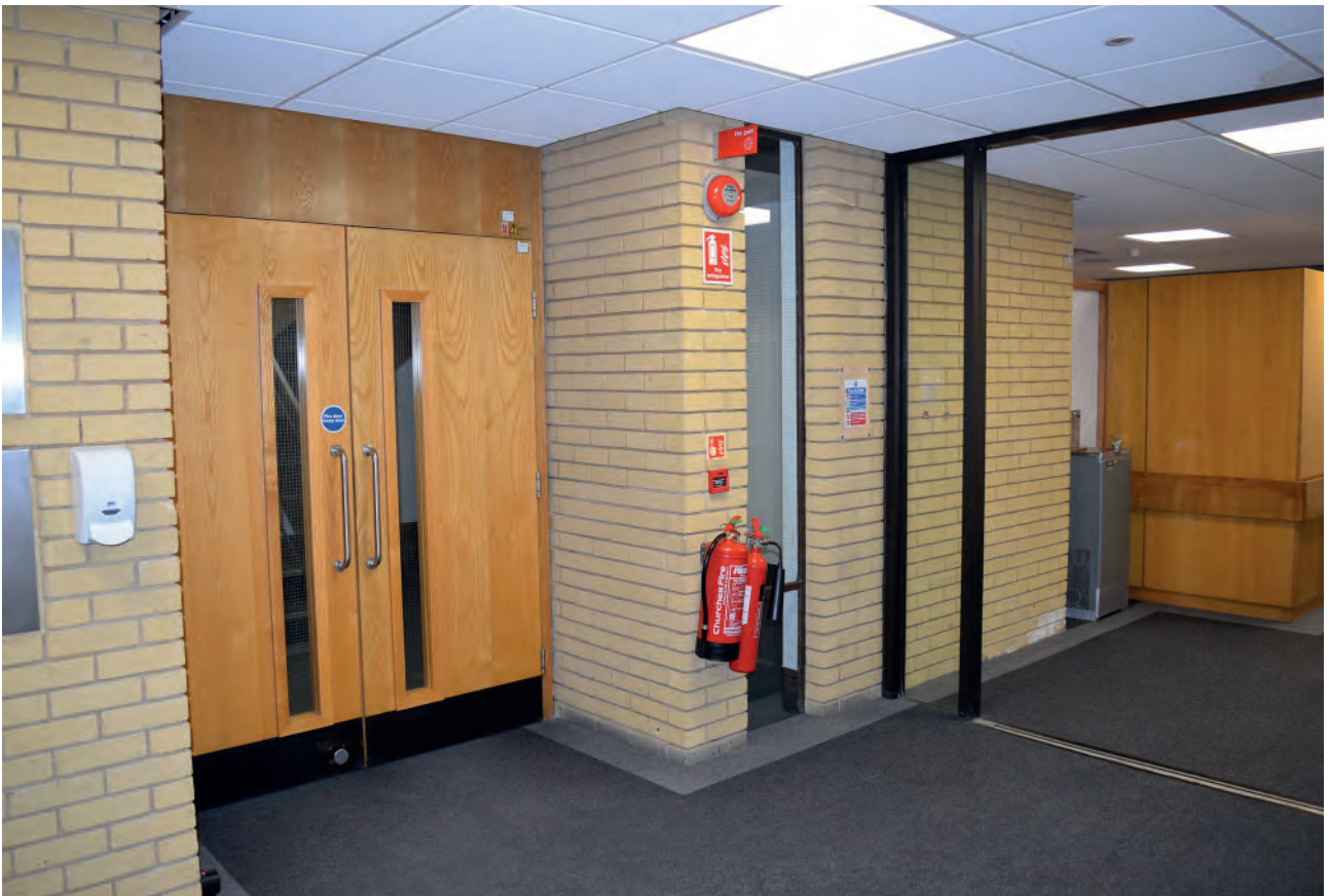
Plate 144: North part of Building 6000, north corridor, stairway entrance, looking south- west.
