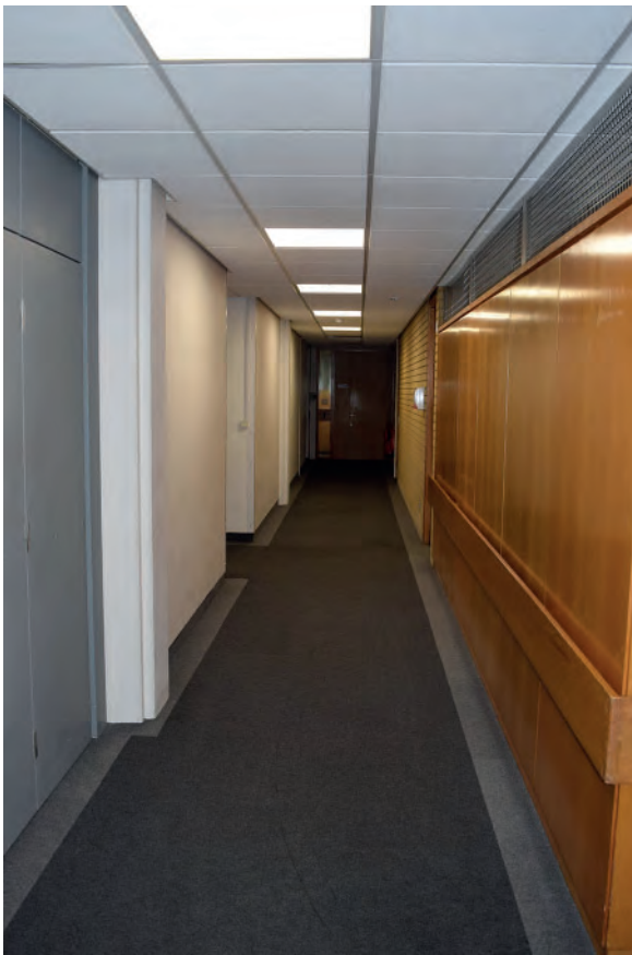
Plate 215: South part of Building 6000, east corridor, looking south.
