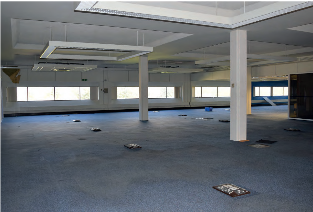
Plate 359: East wing of Building 6000, middle office space, looking south- east.
