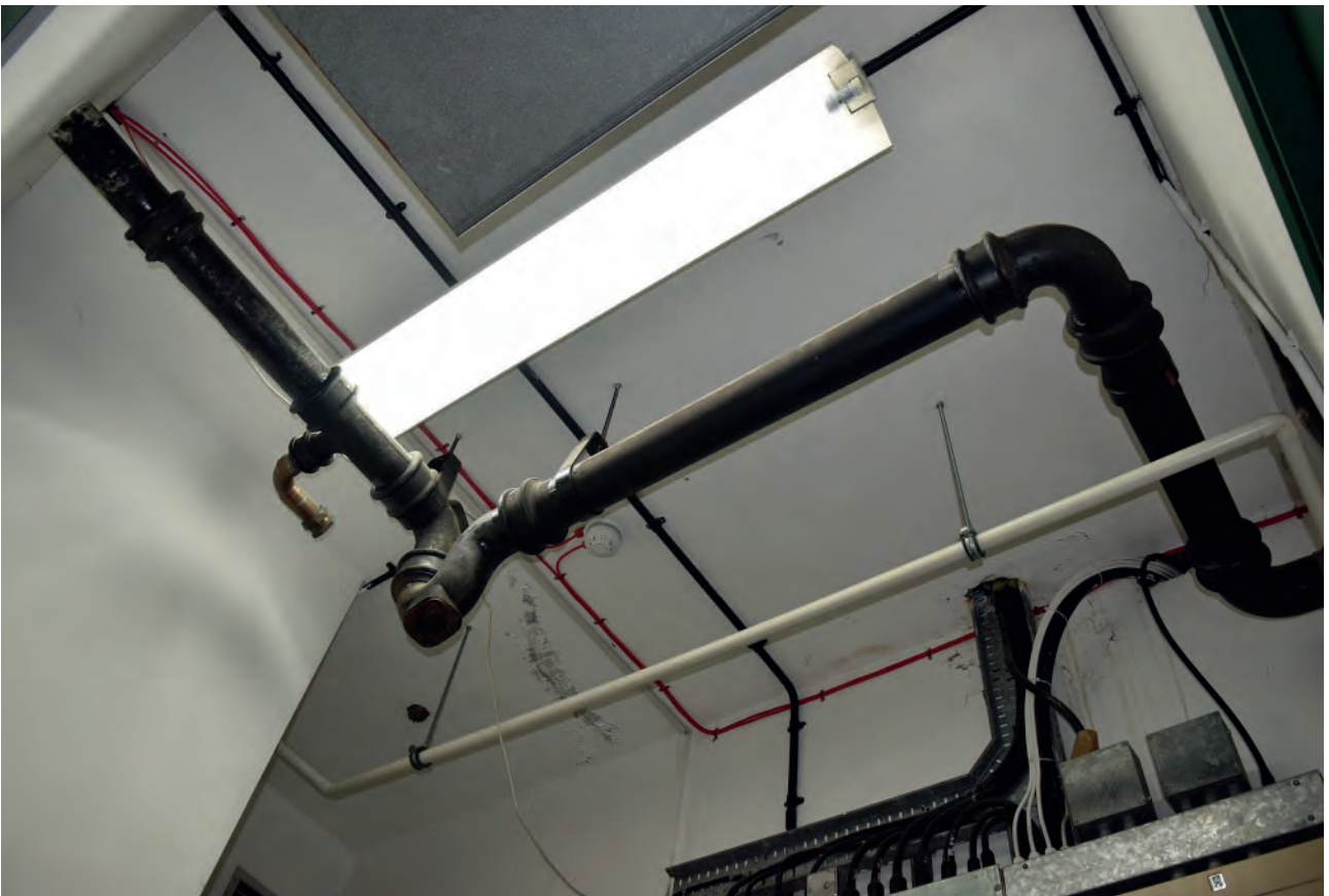
Plate 91: South part of Building 6000, east corridor, ceiling of engine room.
