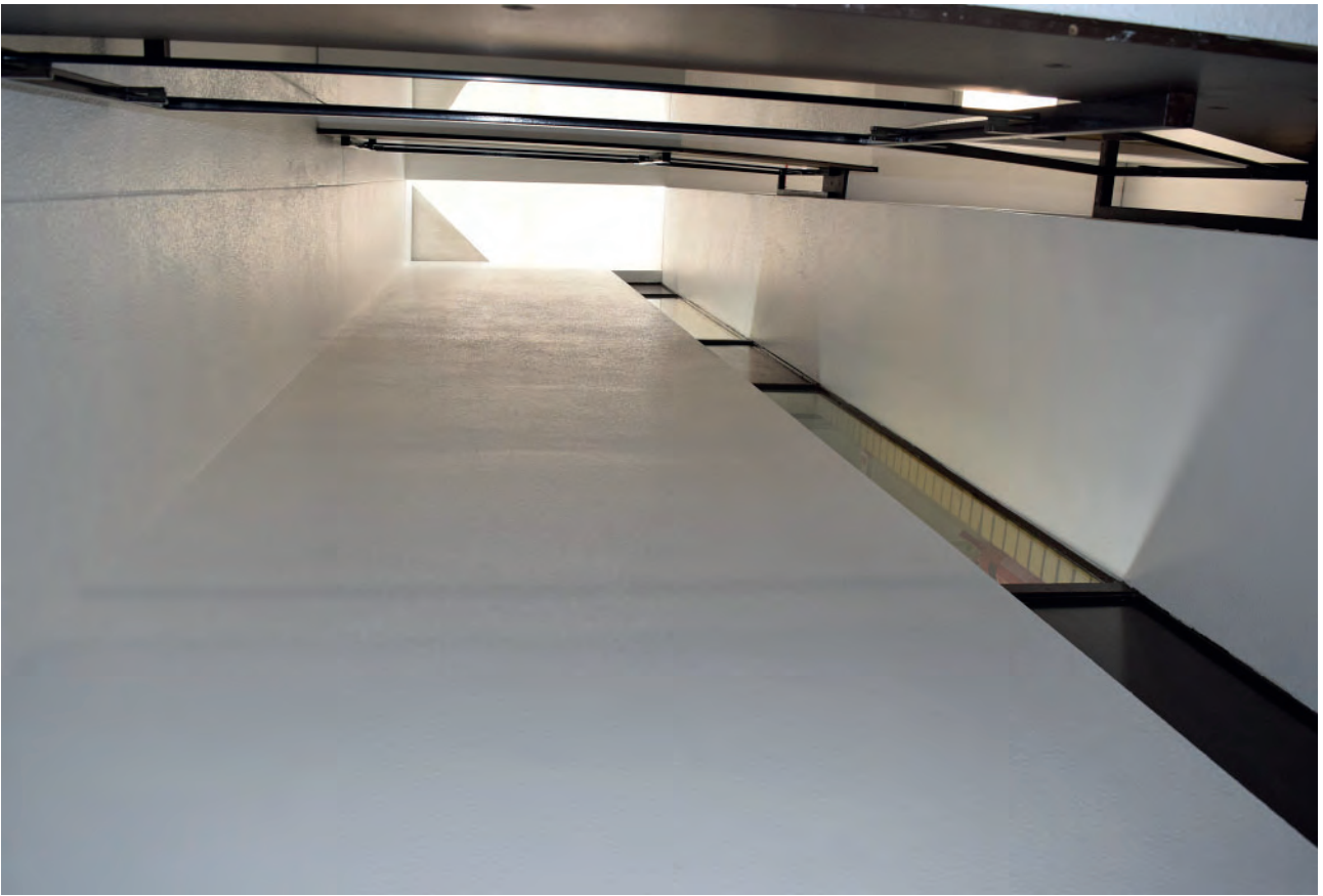
Plate 157: North part of Building 6000, staircase skylight.
