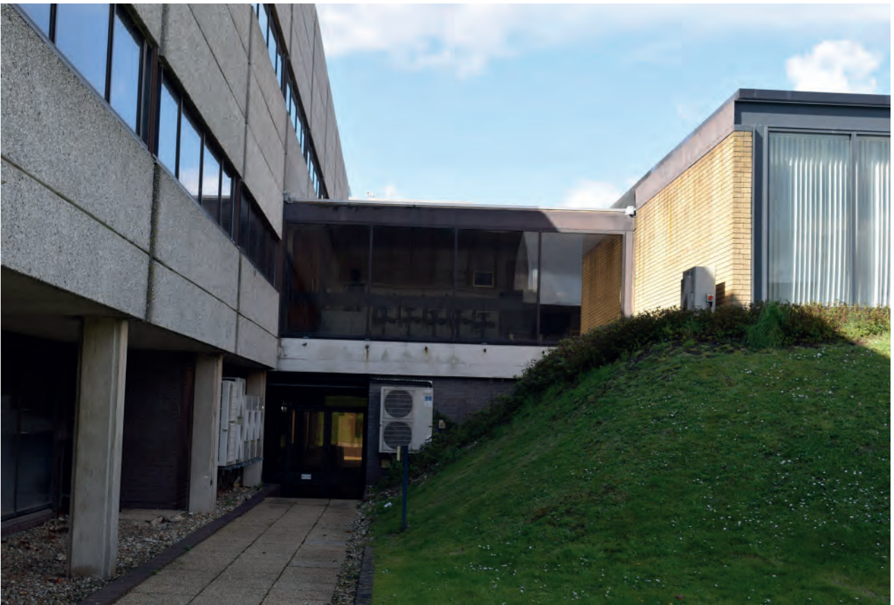
Plate 52: Connection between buildings 6000 and 4000, looking west.
