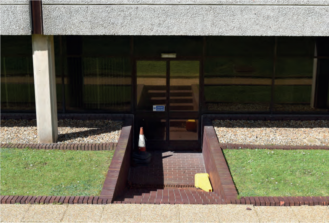
Plate 45: East elevation, one of the glazed emergency exits, looking west.
