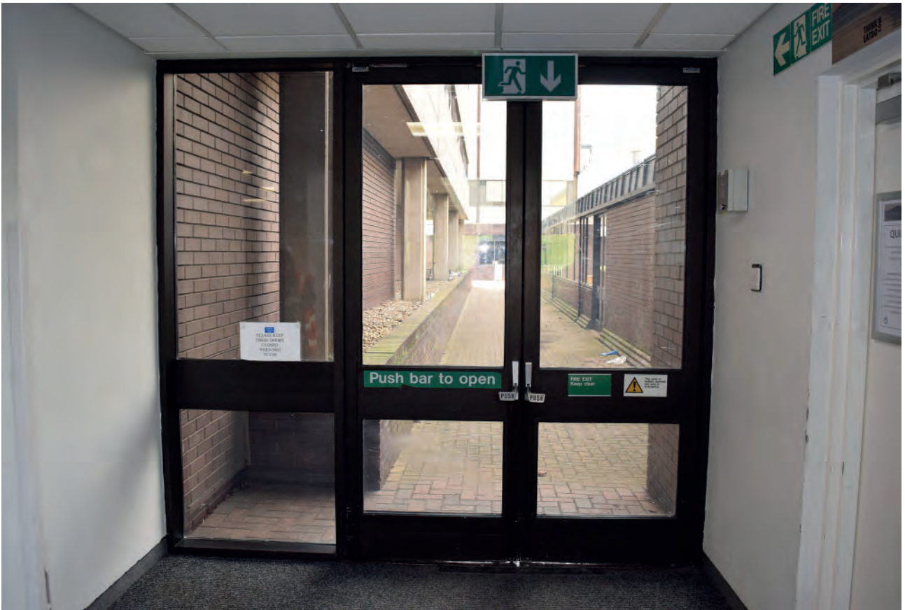
Plate 152: North part of Building 6000, connection between Buildings 6000 and 4000, western emergency door, looking west.
