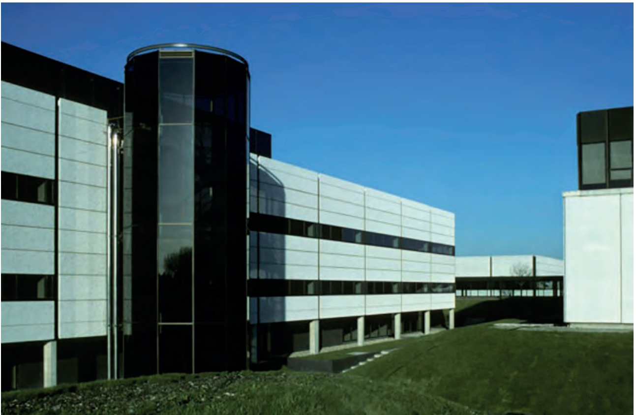
Plate 6: East staircase tower, looking north- west, 1979.
