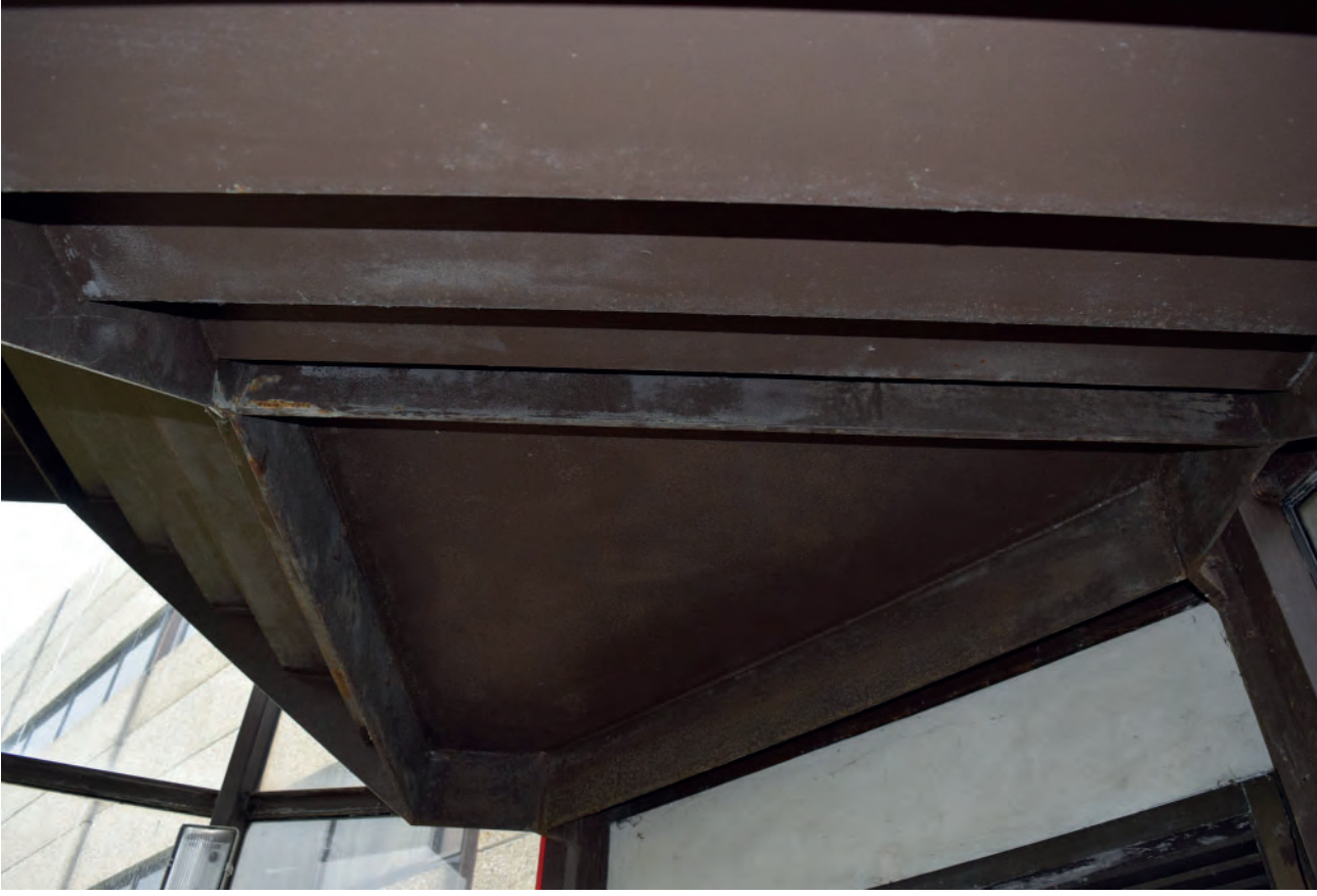
Plate 455: Construction of stairs, landing.
