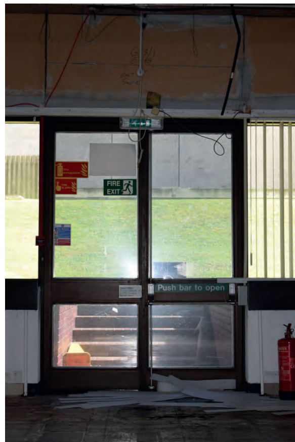
Plate 113: East wing of Building 6000, north office space, emergency exit, looking east.
