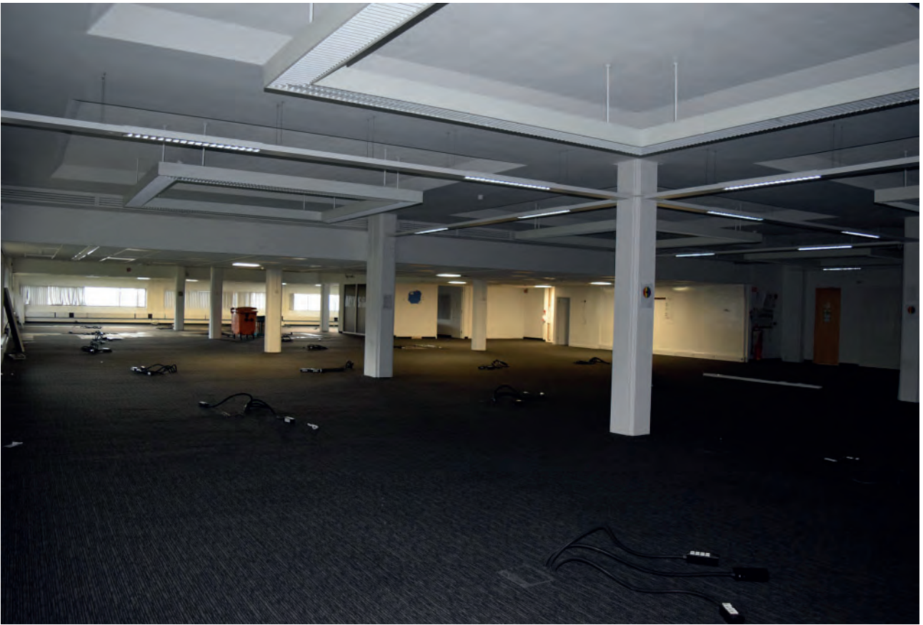
Plate 233: East wing of Building 6000, middle office space, looking south- west.
