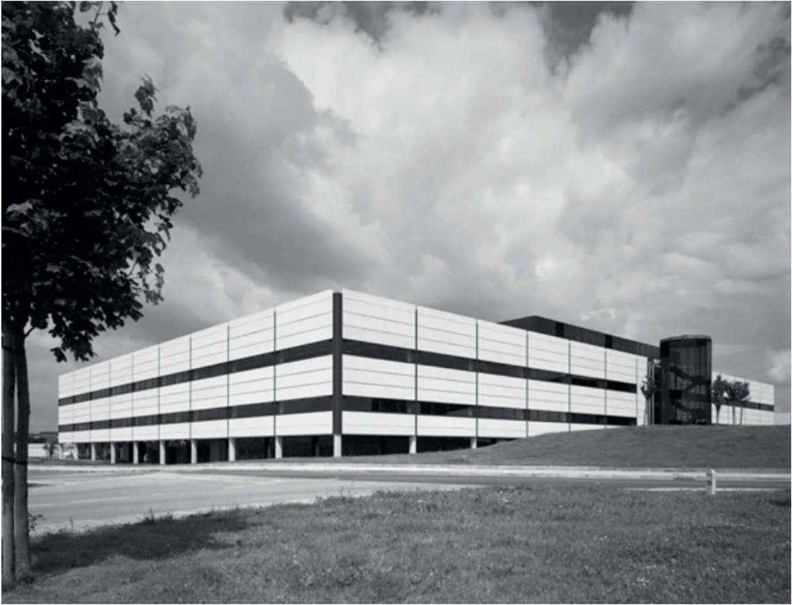
Plate 3: Southeast corner of Building 6000, looking north- west, 1980.
