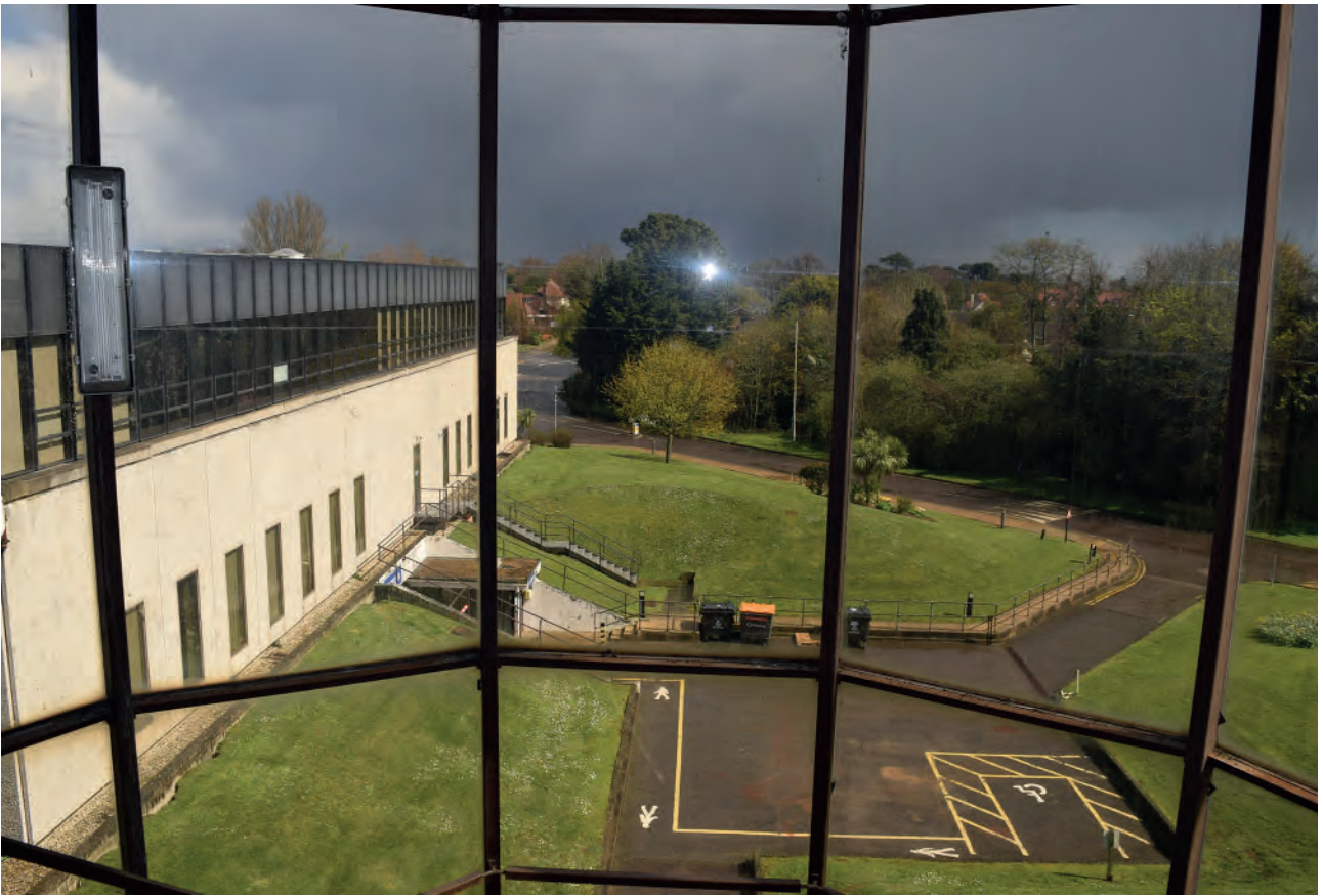
Plate 472: Roof level, looking east.
