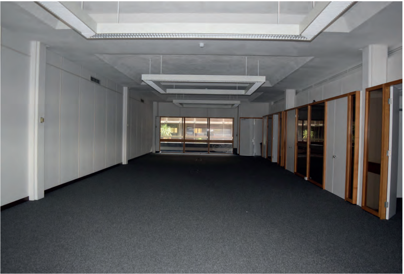
Plate 307: West wing of Building 6000, middle office space, looking east.
