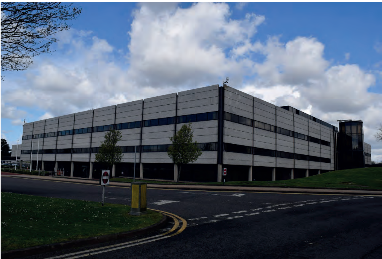
Plate 33: Southeast corner of Building 6000, looking north- west.
