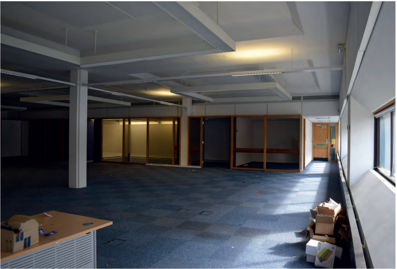
Plate 292: West wing of Building 6000, north office space, looking south.
