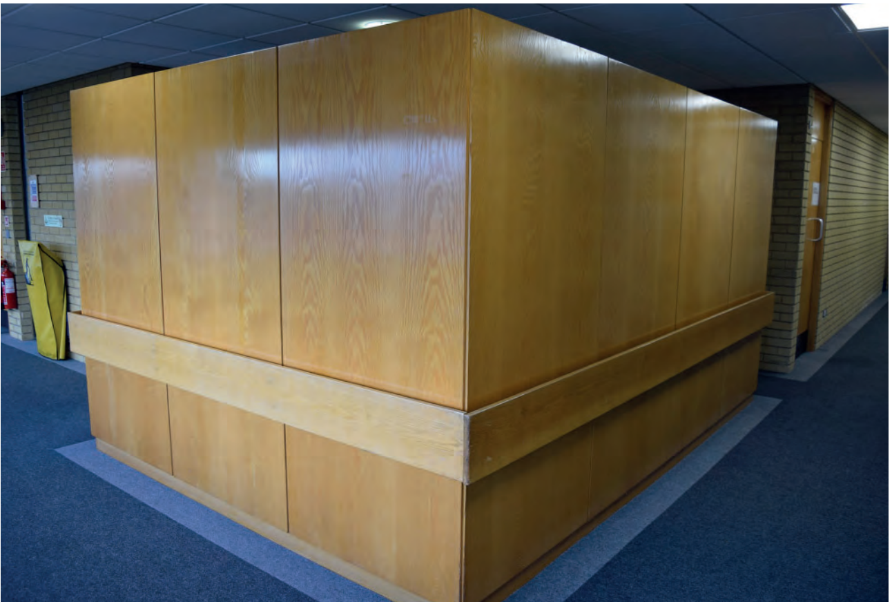
Plate 392: North part of Building 6000, west corridor, wooden structure, looking south-east.
