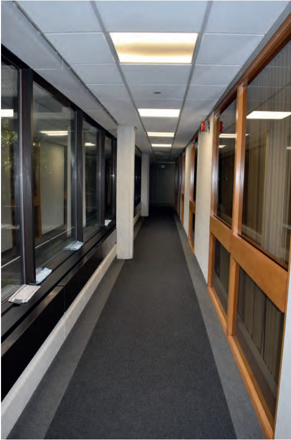
Plate 243: North part of Building 6000, corridor along the north side of the courtyard, looking west.
