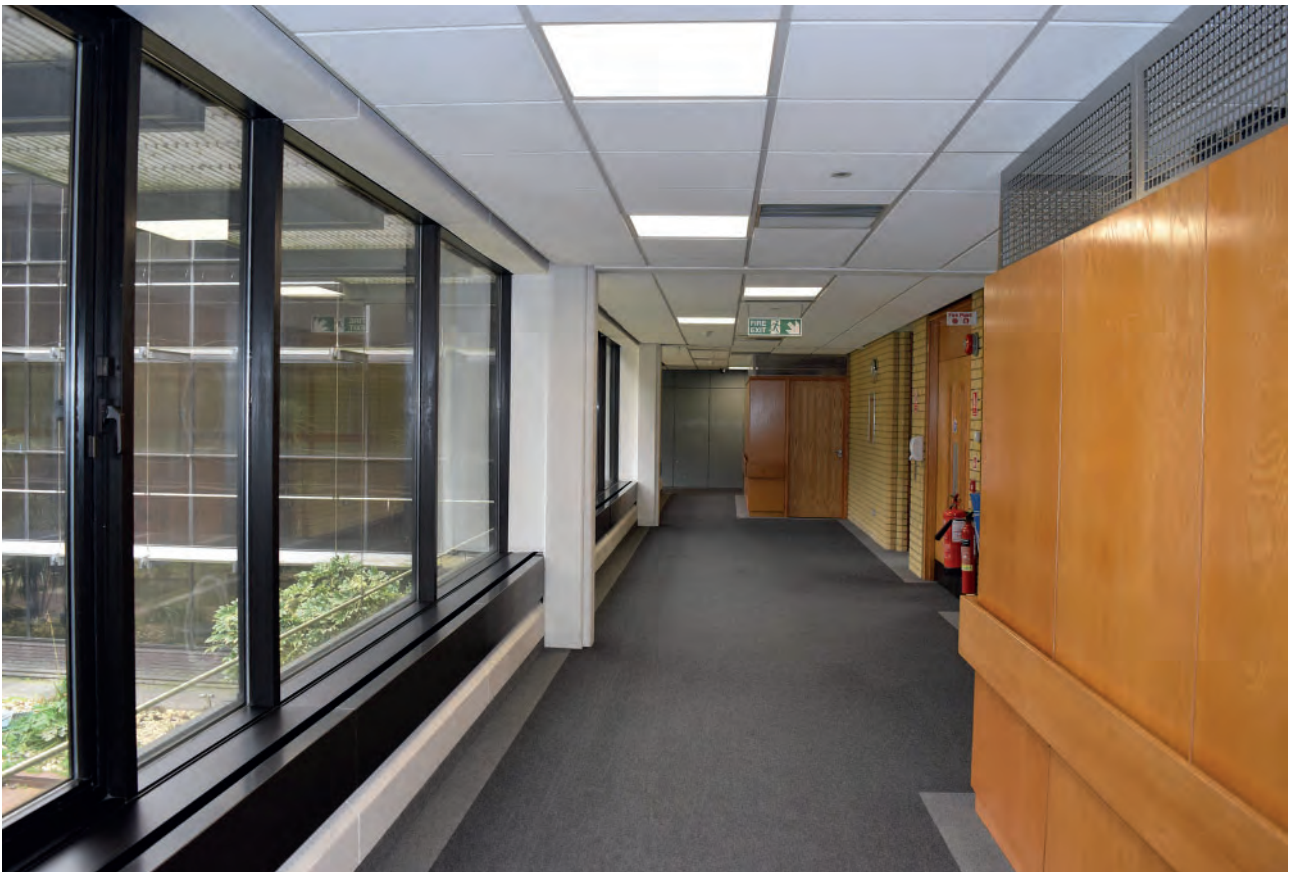
Plate 193: South part of Building 6000, south corridor, looking east.
