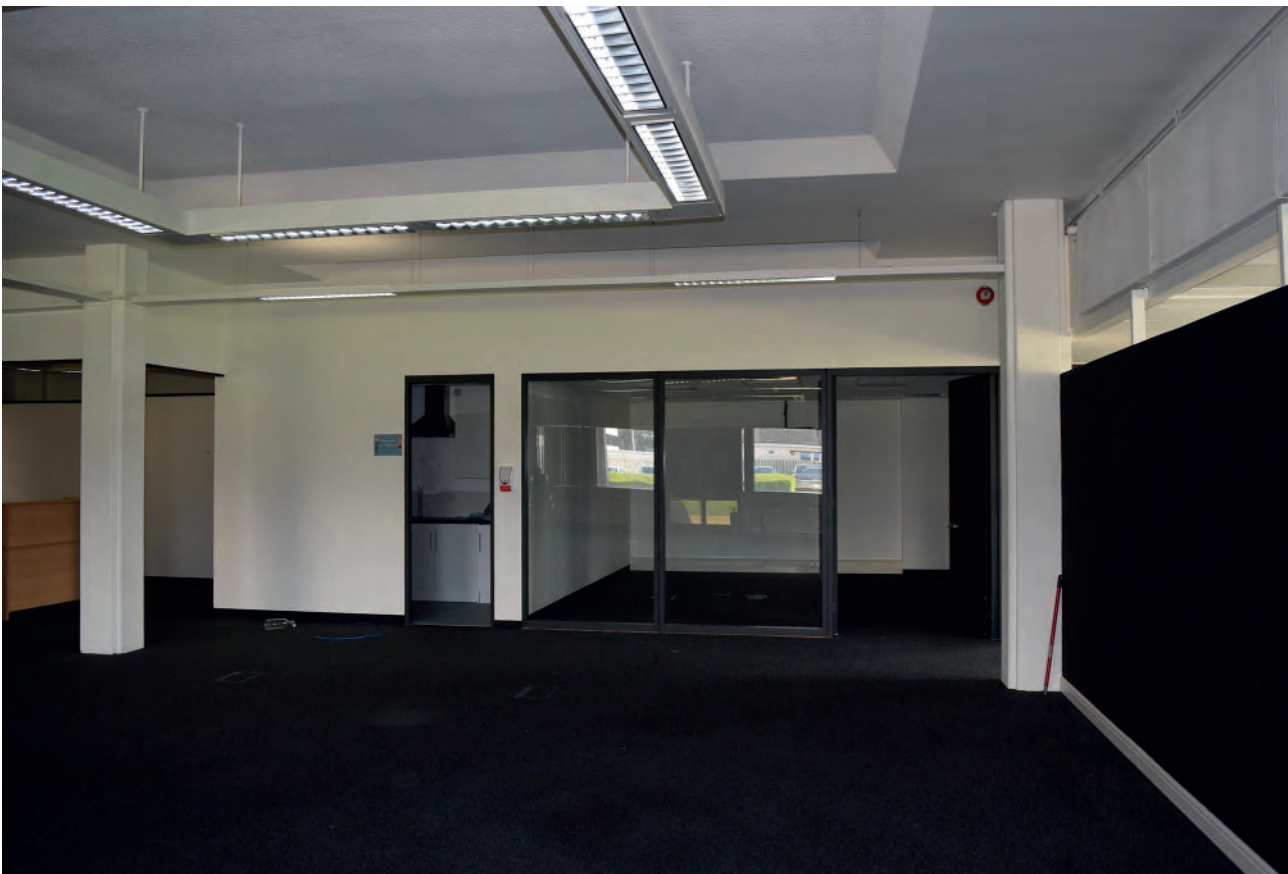
Plate 124: West wing of Building 6000, south office space, looking east.
