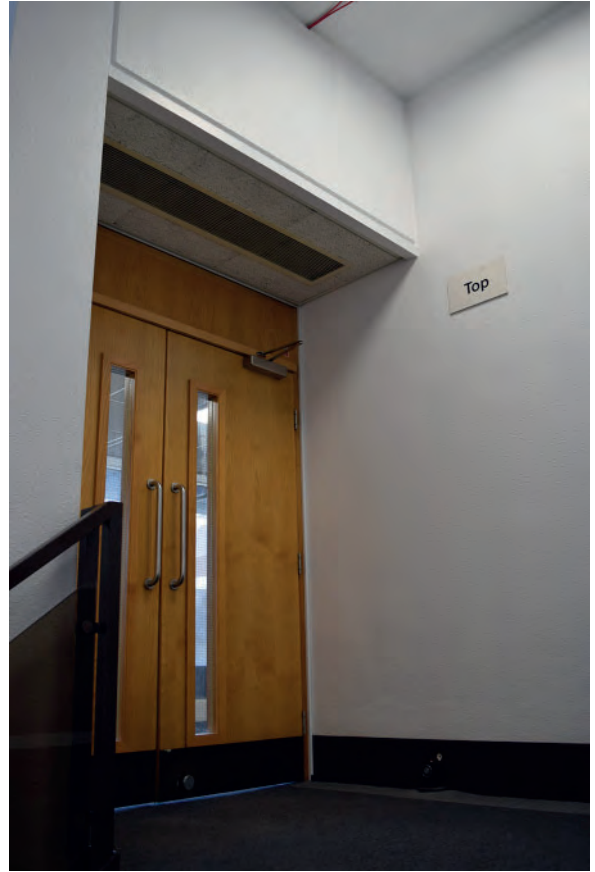
Plate 328: South part of Building 6000, staircase, looking north- east.
