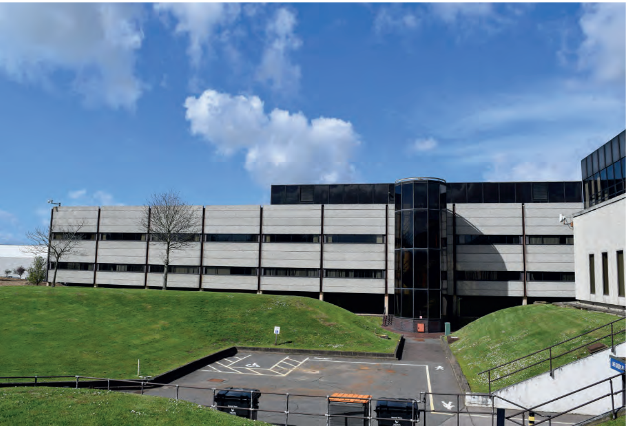
Plate 36: East elevation of Building 6000, looking west.
