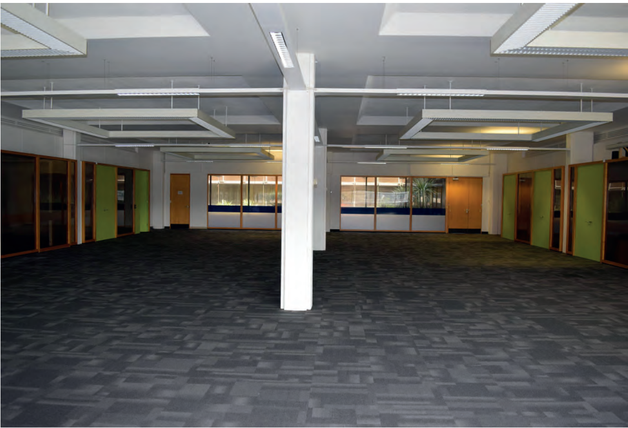
Plate 314: West wing of Building 6000, middle office space, looking east.
