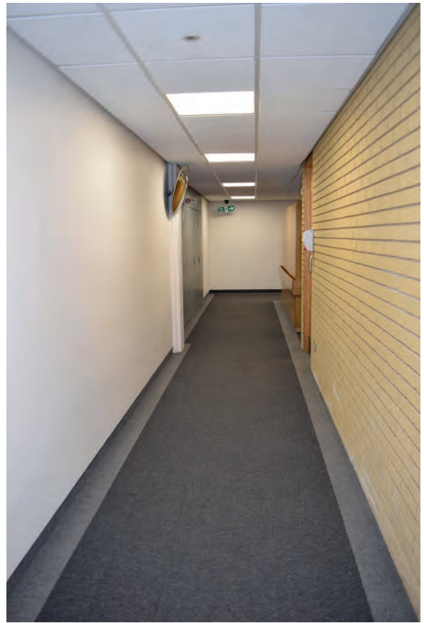
Plate 137: North part of Building 6000, west corridor, looking north.
