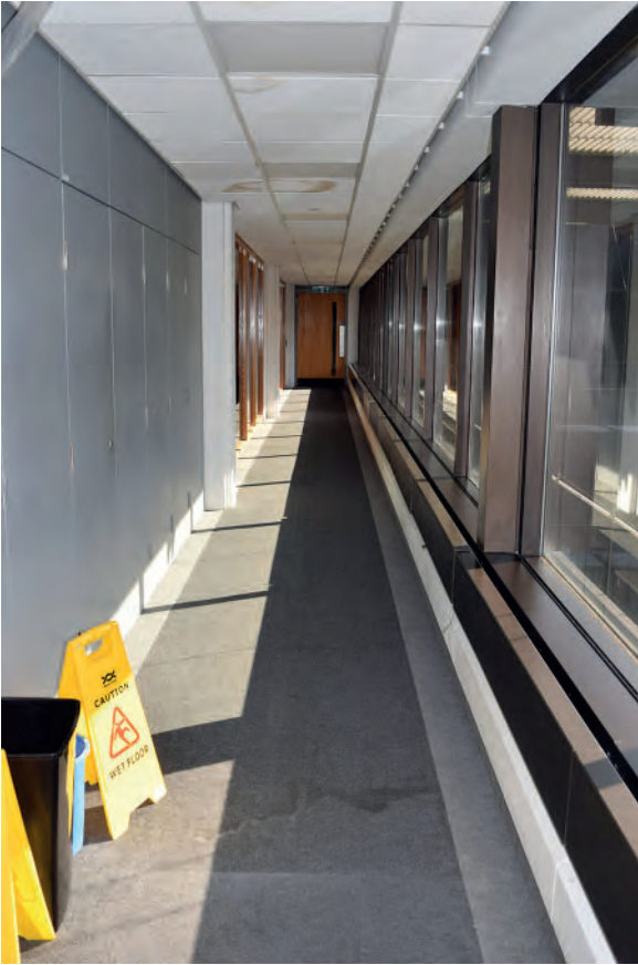
Plate 365: East wing of Building 6000, middle part of east corridor, looking south.
