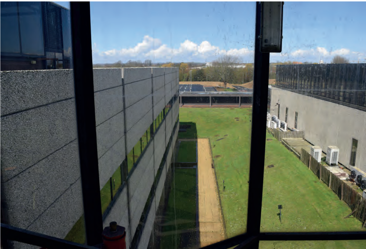
Plate 471: Roof level, looking north.
