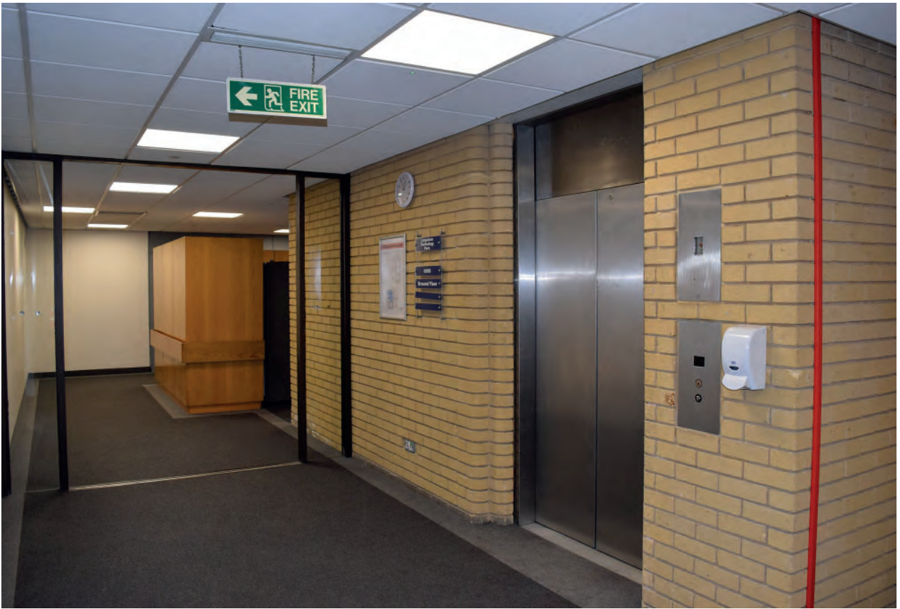
Plate 145: North part of Building 6000, north corridor, elevator entrance, looking south- east.
