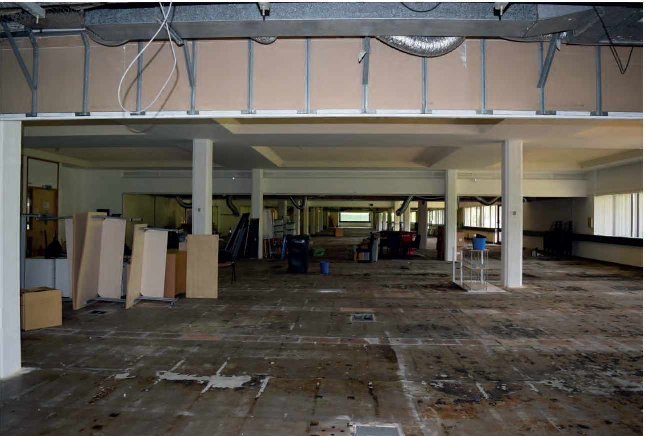
Plate 95: East wing of Building 6000, south office south office space, looking north.
