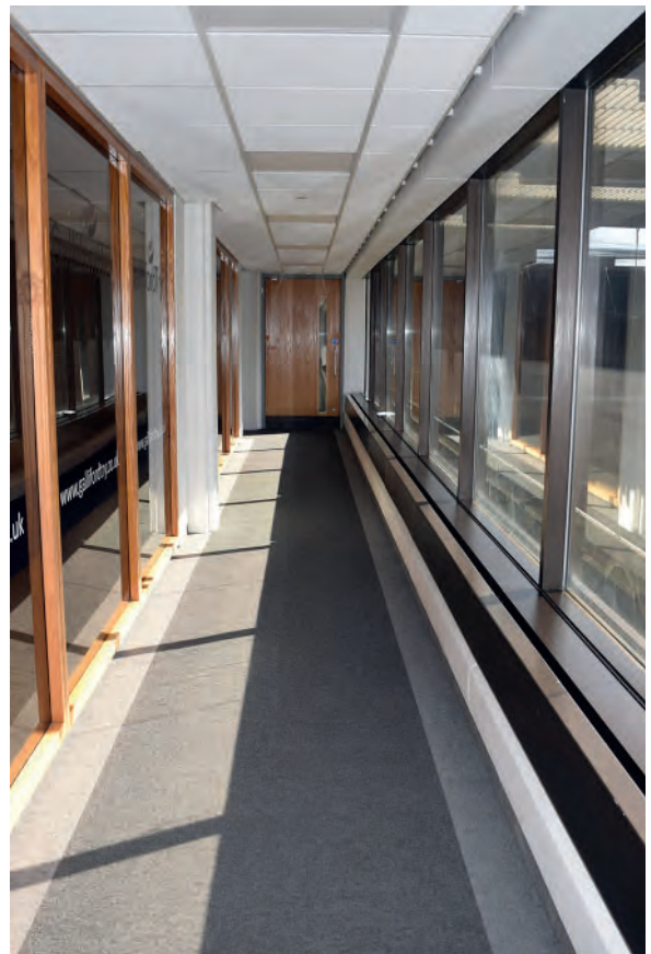
Plate 368: East wing of Building 6000, middle part of east corridor, looking south.
