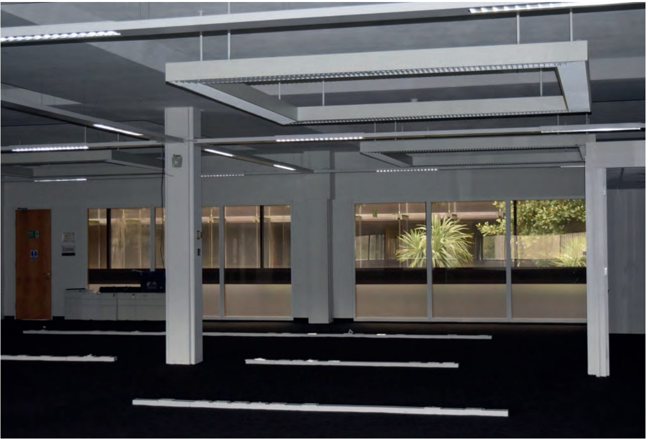
Plate 241: East wing of Building 6000, middle office space, looking west.
