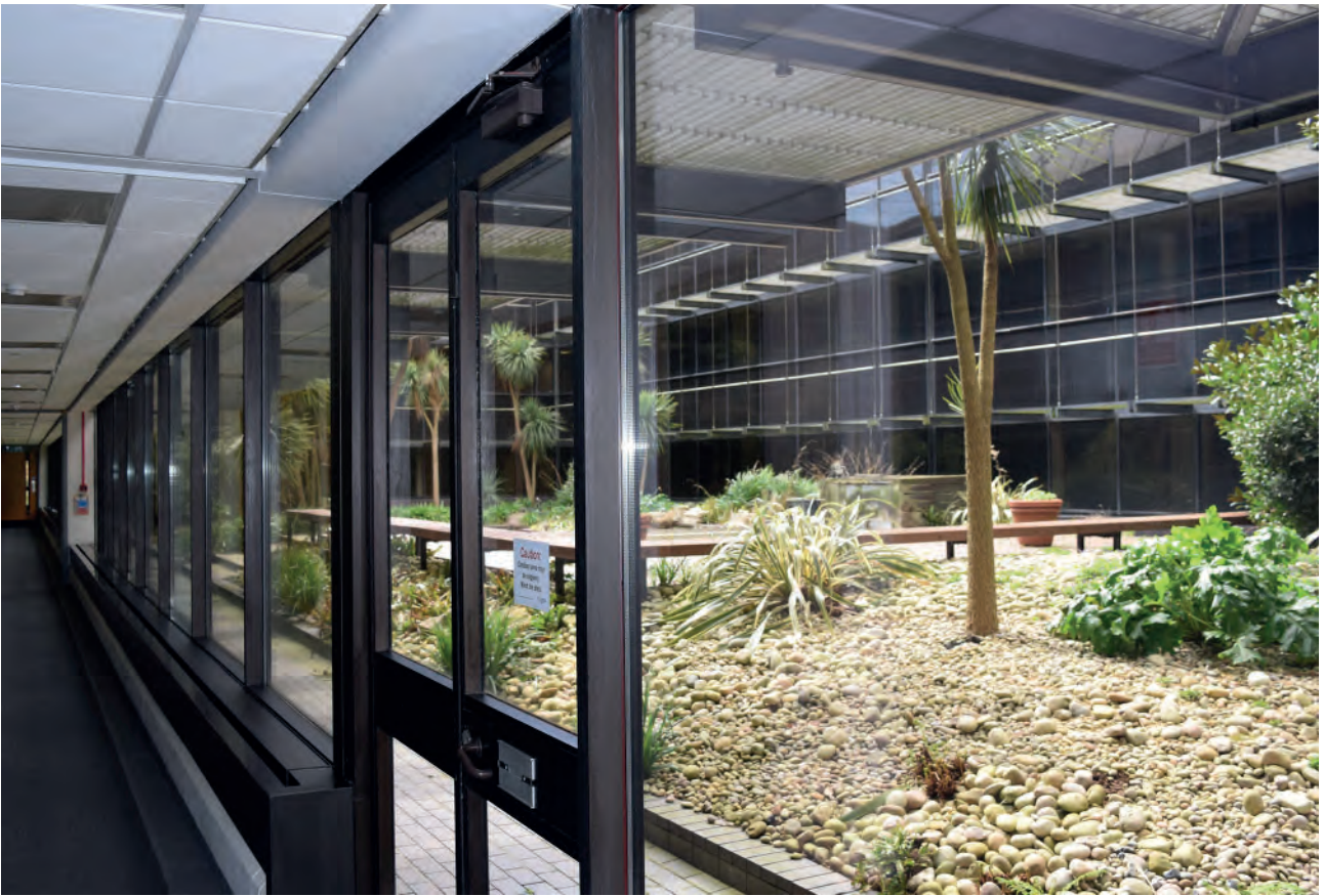
Plate 162: East wing of Building 6000, middle part of east corridor, view of the courtyard, looking south-west.
