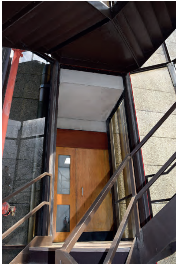
Plate 482: First Floor, emergency door, looking east.
