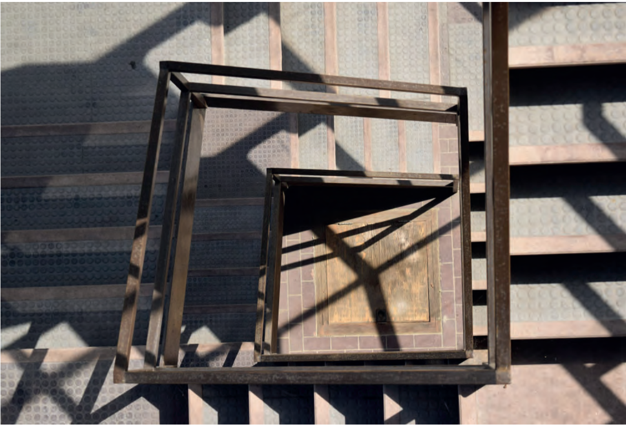
Plate 470: Construction of stairs, ground floor view.
