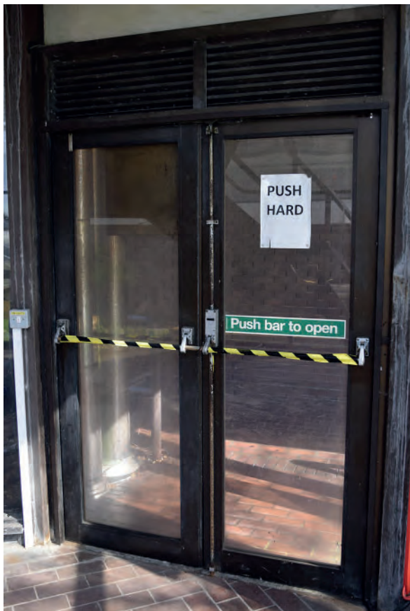
Plate 476: Ground Floor, emergency door, looking east.
