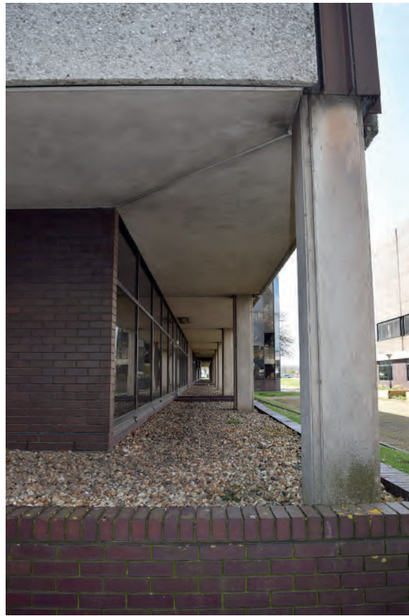
Plate 64: West concrete portico with glazing of the offices, looking south.
