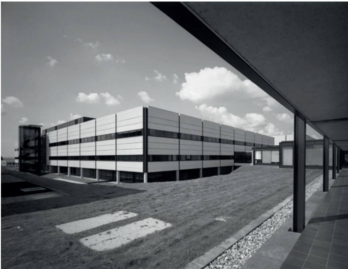
Plate 8: Northeast corner of Building 6000, looking south- west, 1980.
