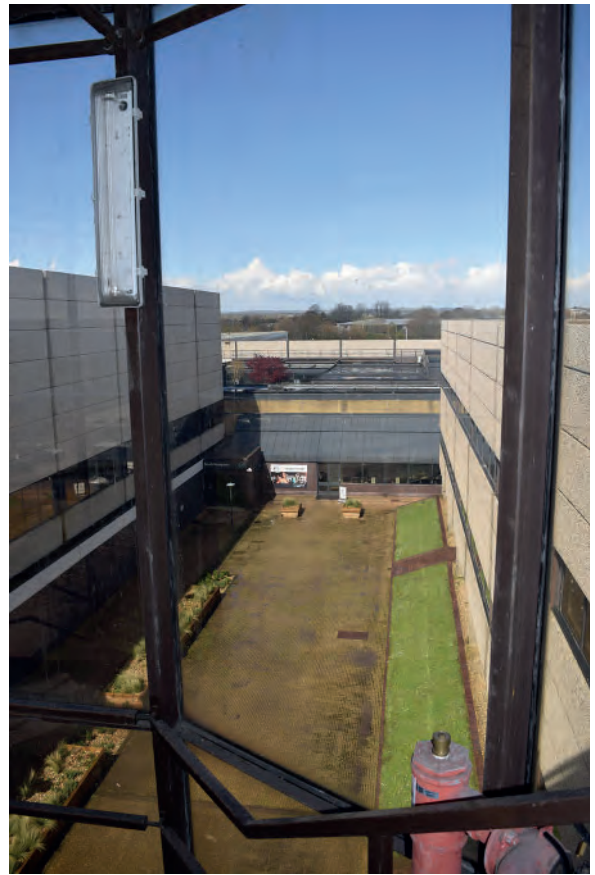
Plate 493: Roof level, looking north.
