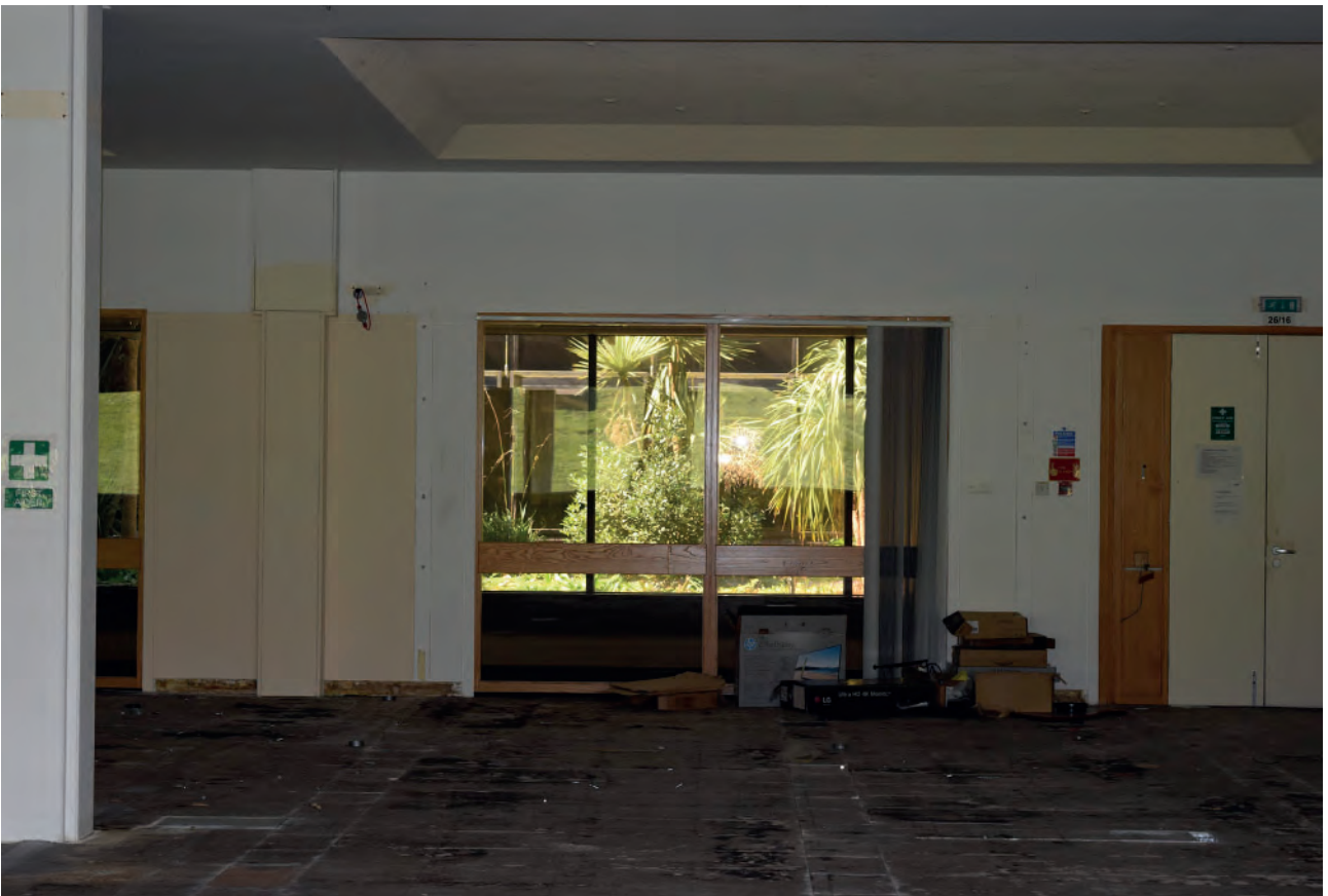
Plate 101: East wing of Building 6000, middle office space, looking west.
