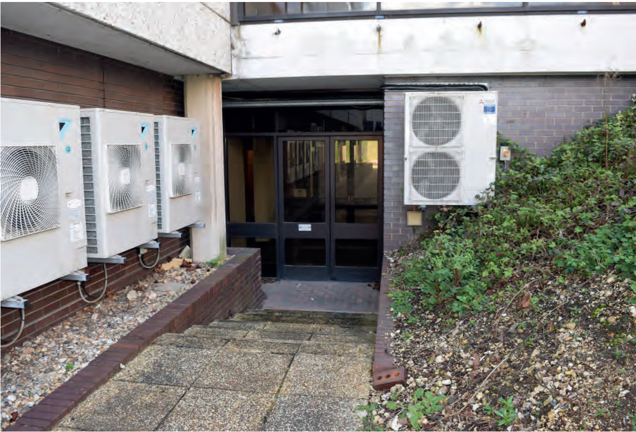
Plate 53: Connection between buildings 6000 and 4000, emergency exit, looking west.
