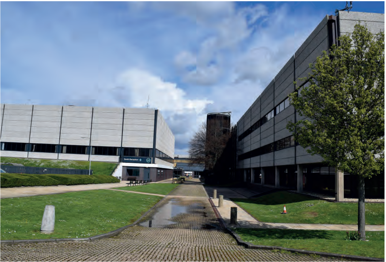
Plate 57: Walkway between Buildings 6000 and 5000, looking north.
