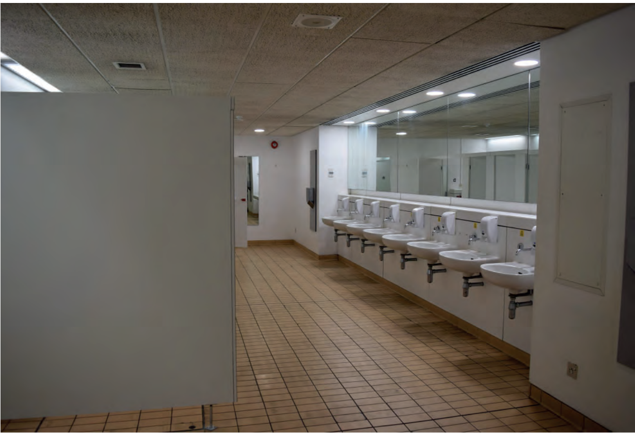
Plate 150: North part of Building 6000, west corridor, men's toilet, looking north- west.
