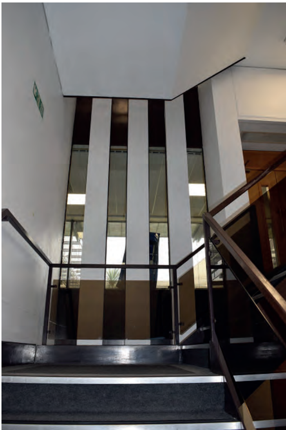
Plate 190: South part of Building 6000, staircase glazing, looking north.
