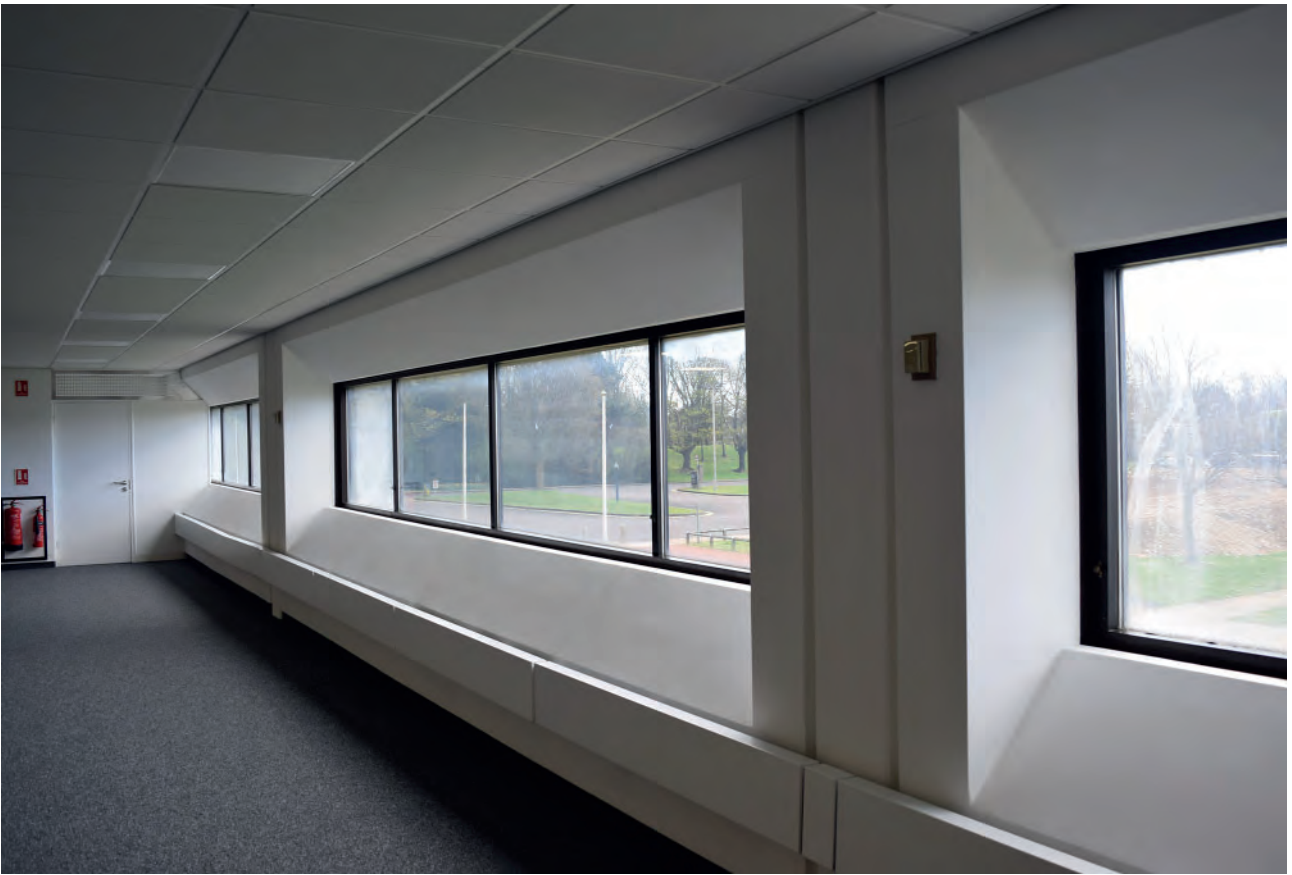
Plate 208: West wing of Building 6000, south office space, looking south- east.
