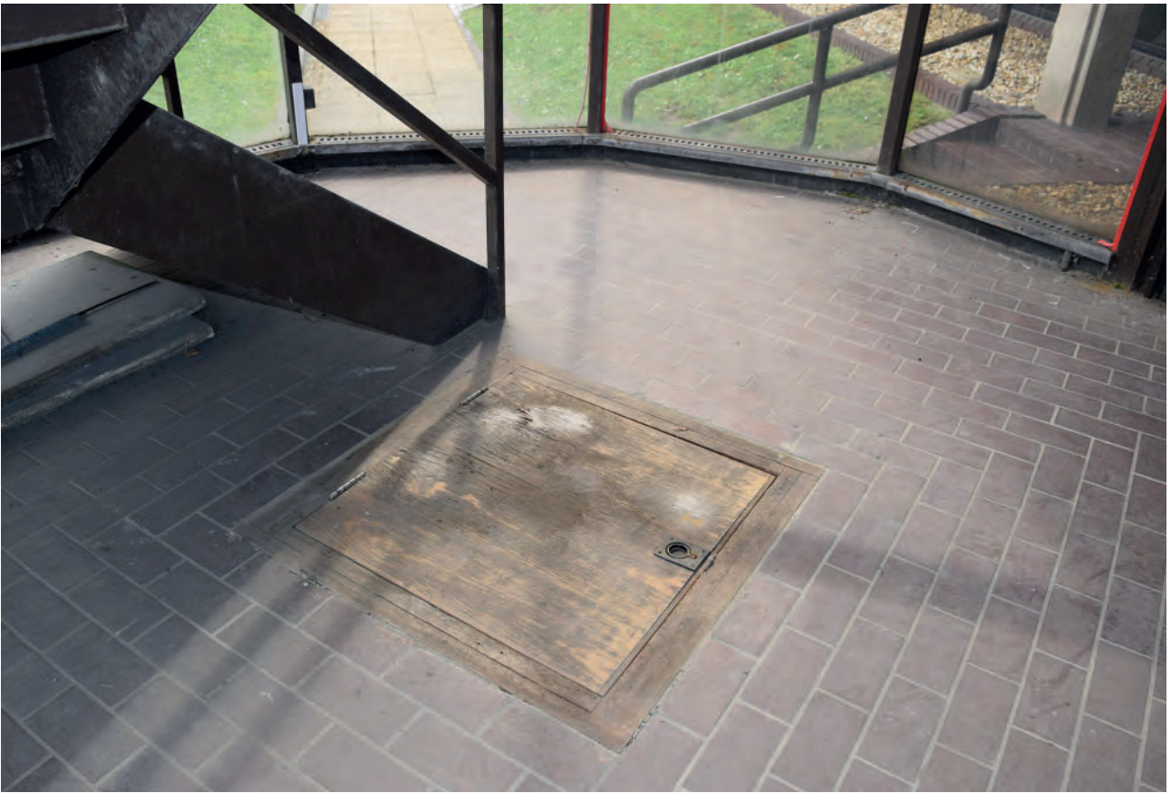
Plate 461: Base of staircase, looking south.
