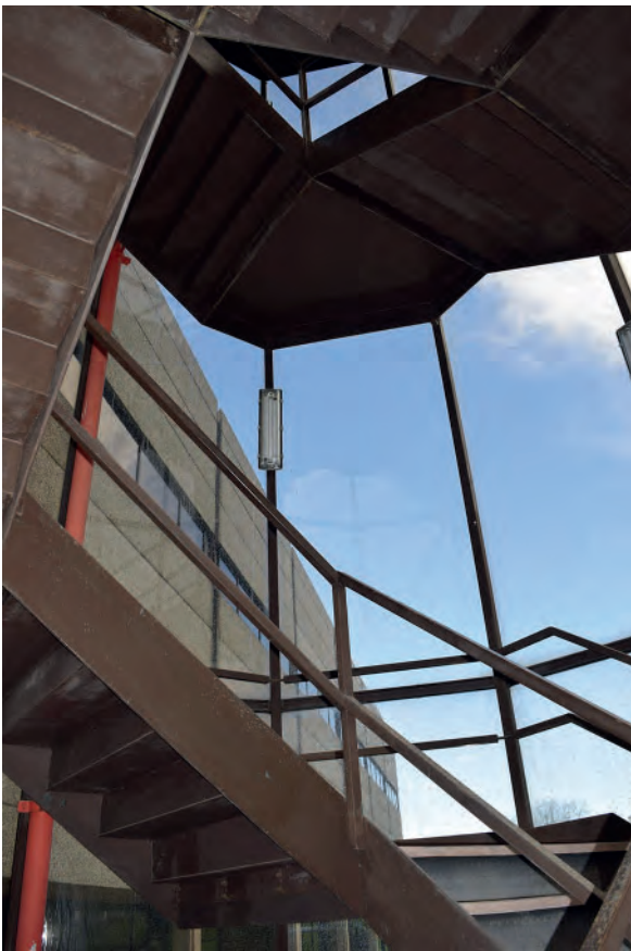
Plate 457: Construction of stairs, looking north.
