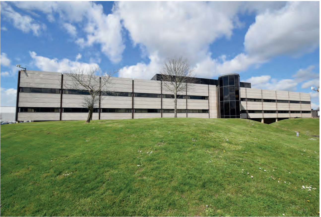
Plate 35: East elevation of Building 6000, looking north- west.
