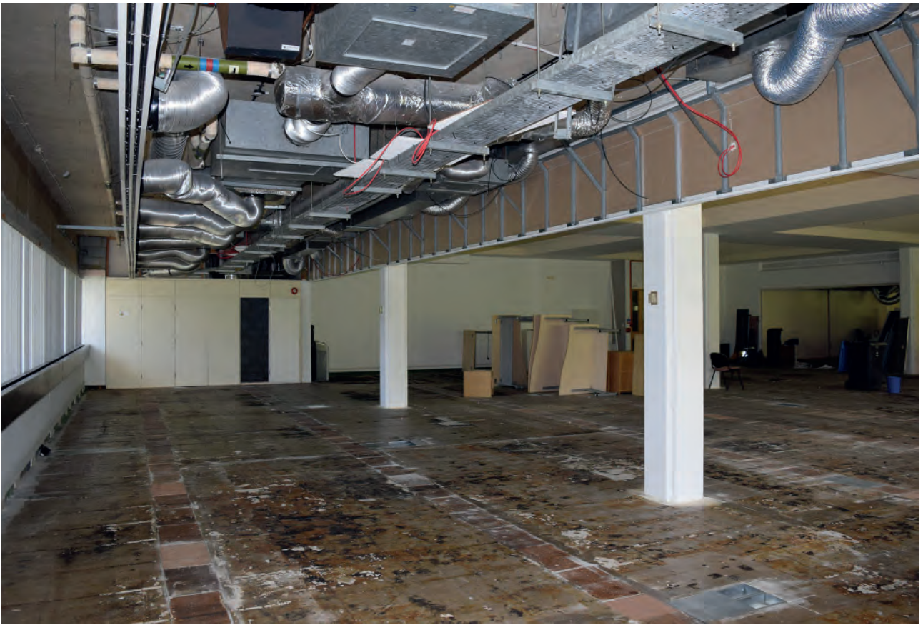
Plate 94: East wing of Building 6000, south office south office space, looking west.
