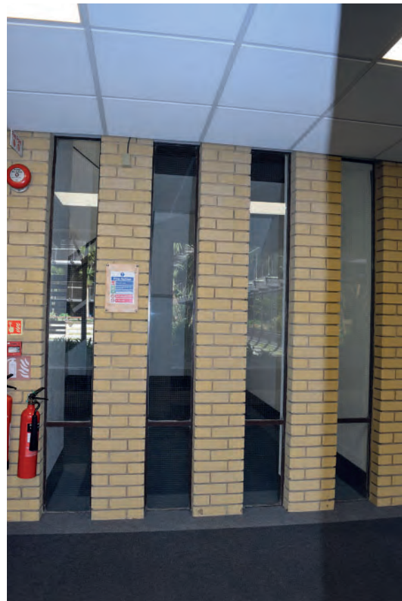
Plate 86: South part of Building 6000, south corridor, staircase glazing, looking south.
