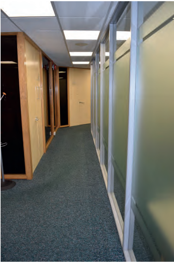
Plate 251: East wing of Building 6000, north office space, looking north.
