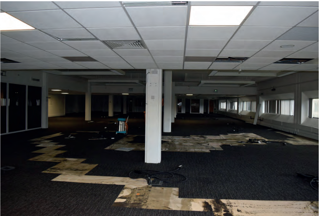
Plate 222: East wing of Building 6000, south office space, looking north.
