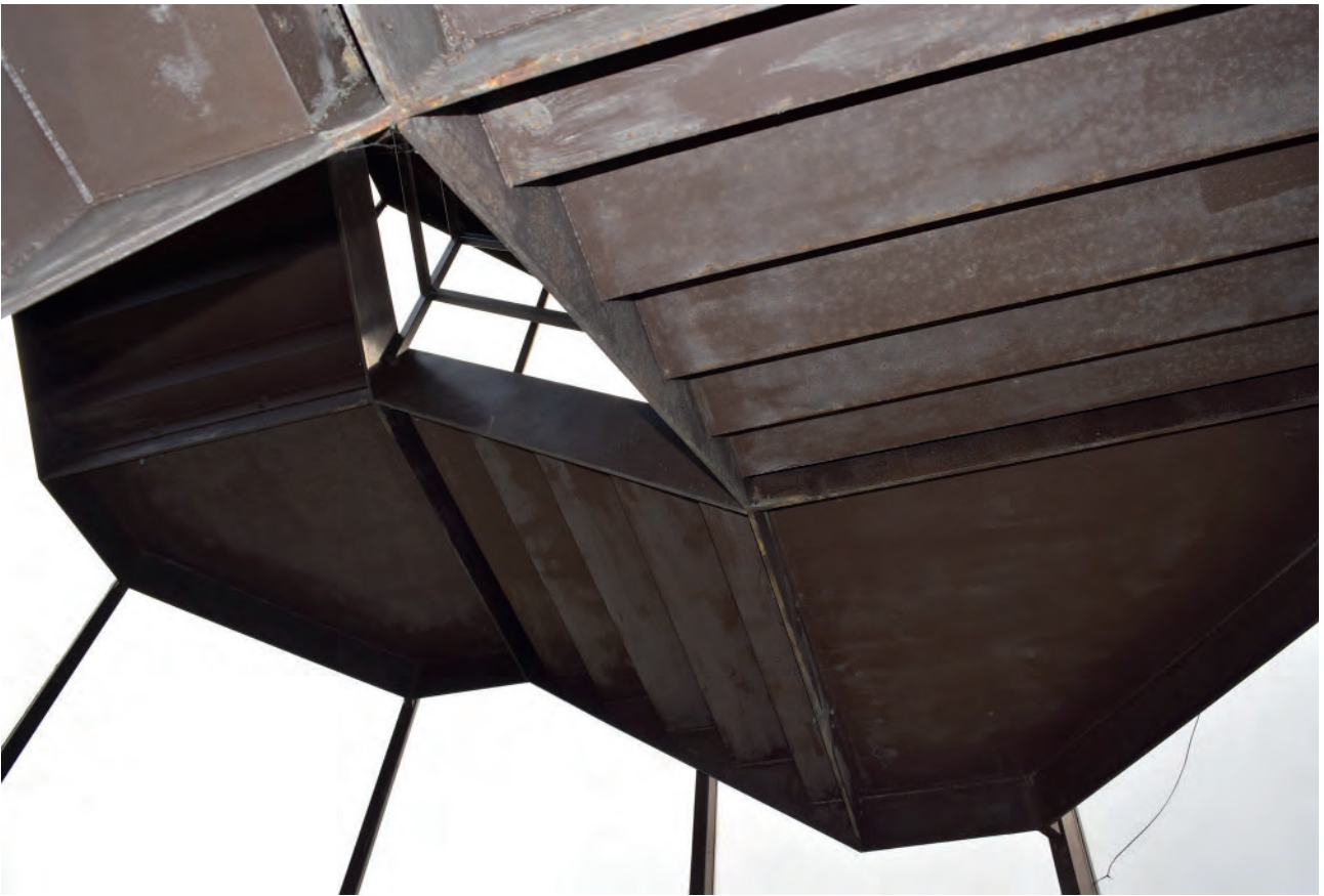
Plate 456: Construction of stairs.
