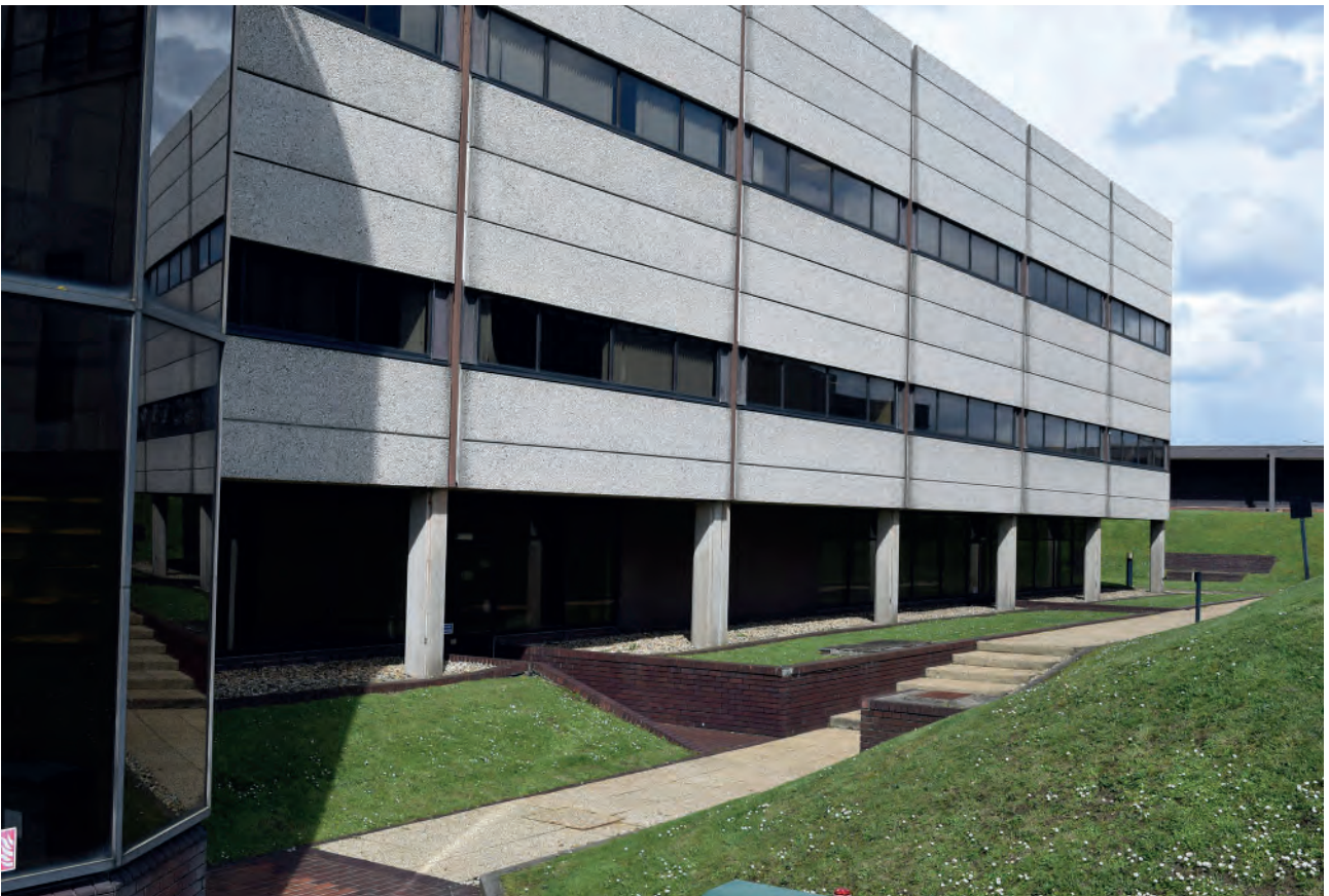
Plate 40: East elevation of Building 6000, looking north- west.
