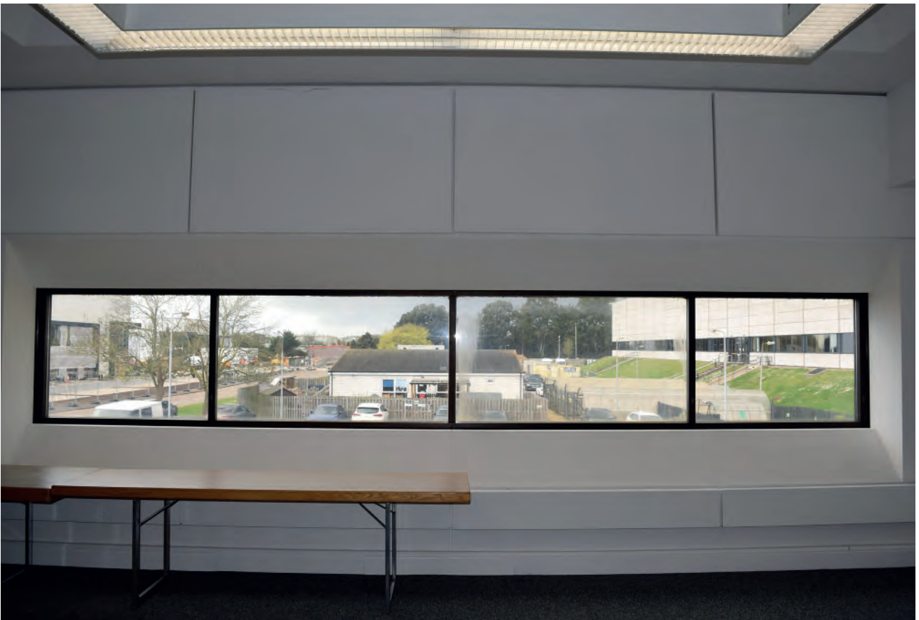
Plate 205: West wing of Building 6000, south office space, looking west.
