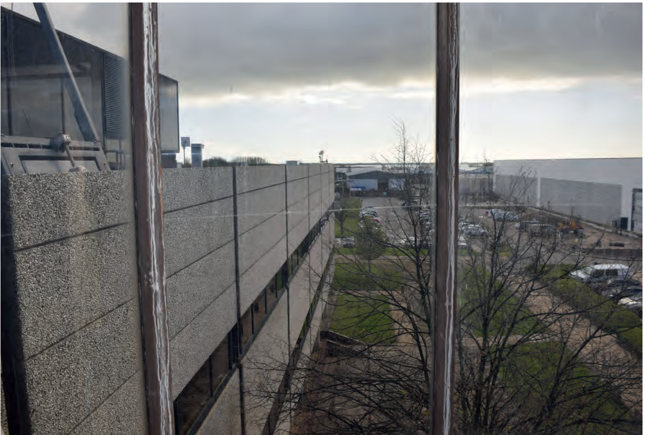
Plate 491: Roof level, looking south.
