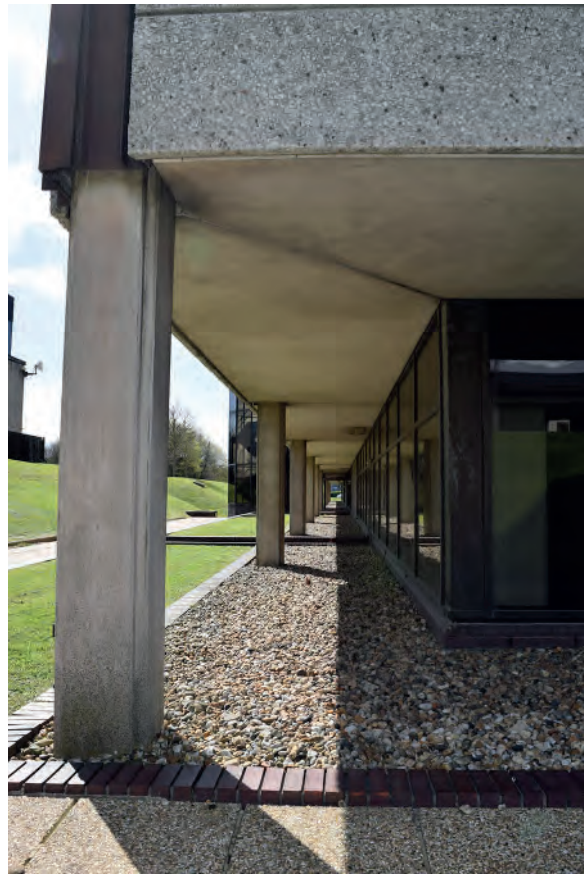
Plate 55: East concrete portico with glazing of the offices, looking south.
