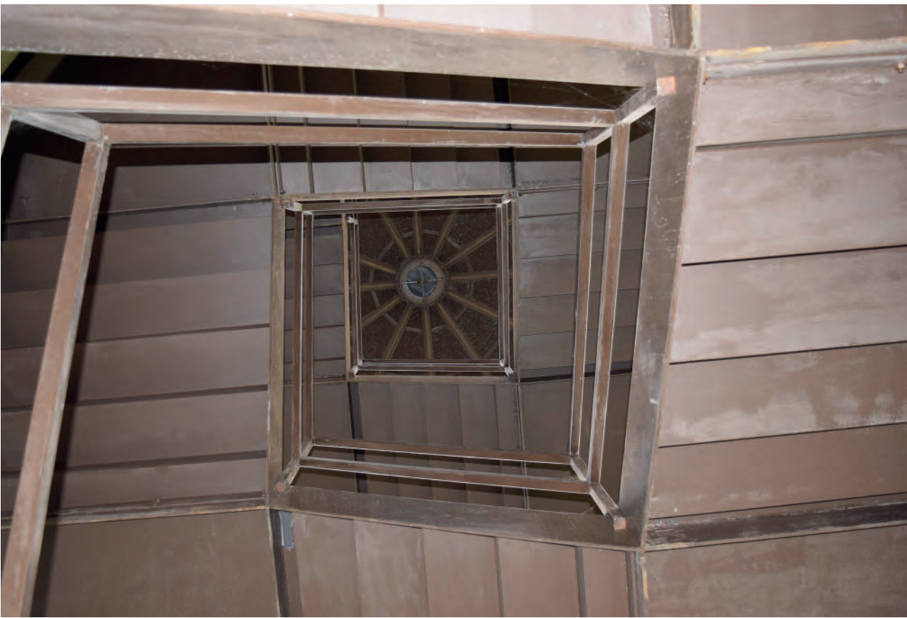
Plate 454: Construction of stairs, ceiling view.
