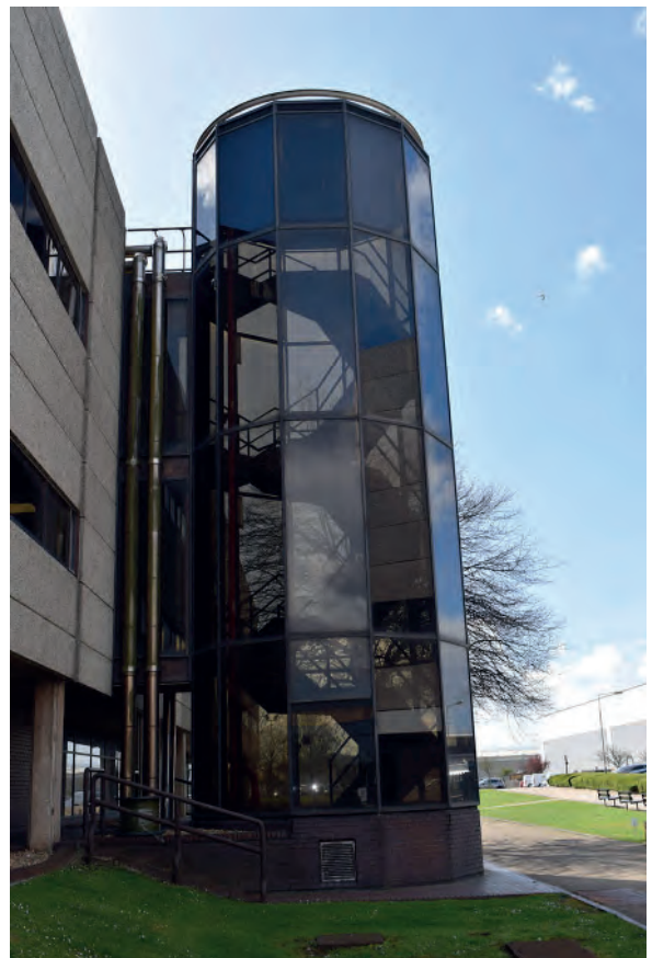
Plate 62: West staircase tower, looking south.
