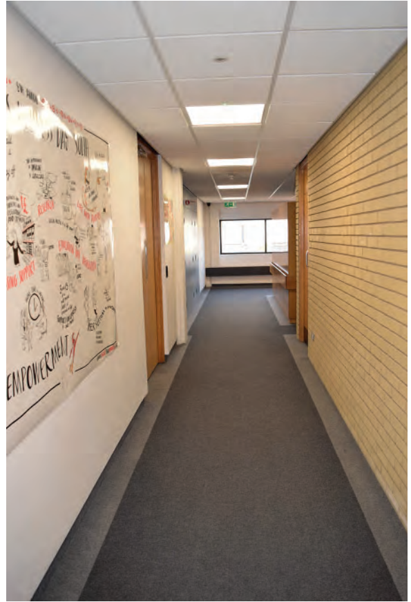
Plate 391: North part of Building 6000, west corridor, looking north.
