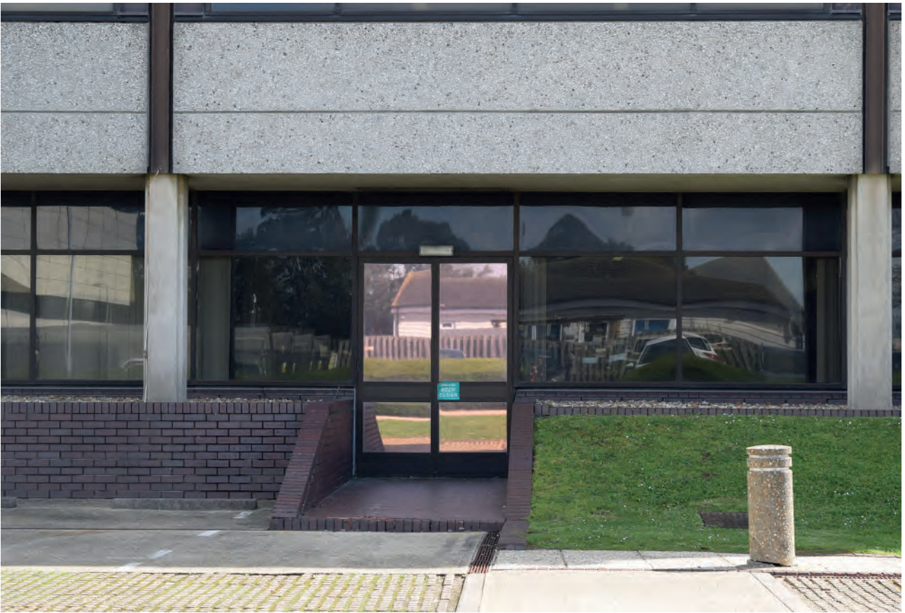
Plate 59: West elevation, one of the glazed emergency exits, looking east.
