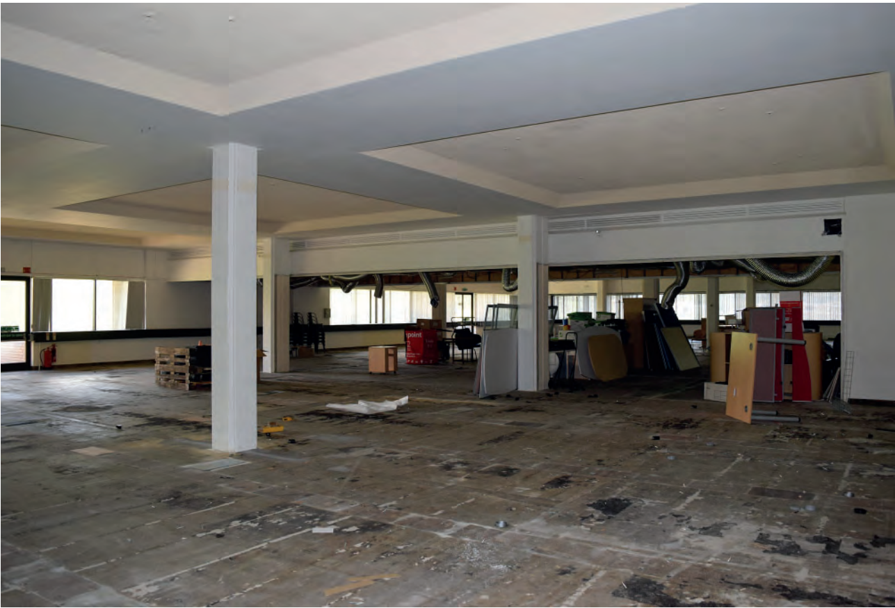
Plate 104: East wing of Building 6000, middle office space, looking south- east.
