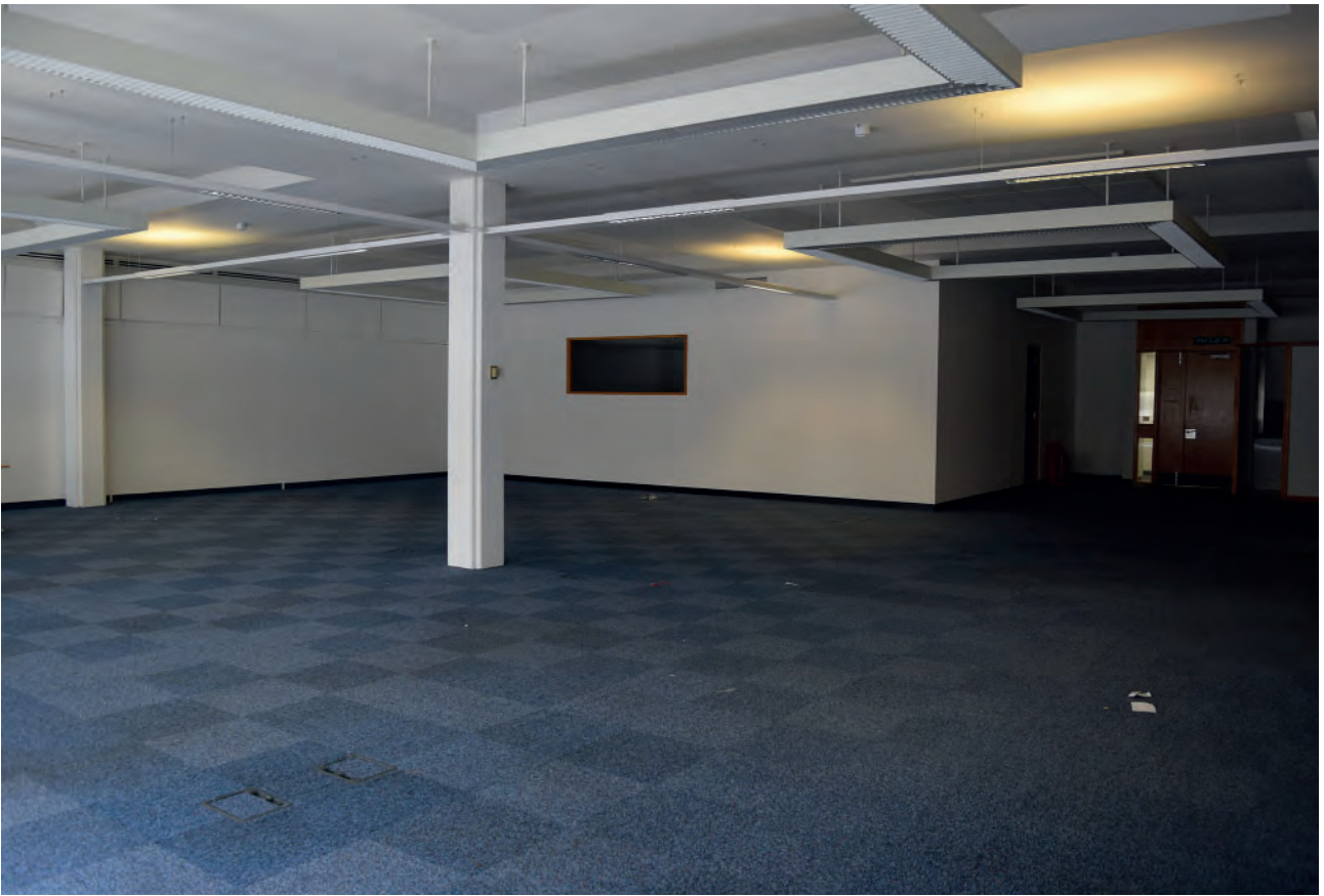
Plate 290: West wing of Building 6000, north office space, looking north- east.
