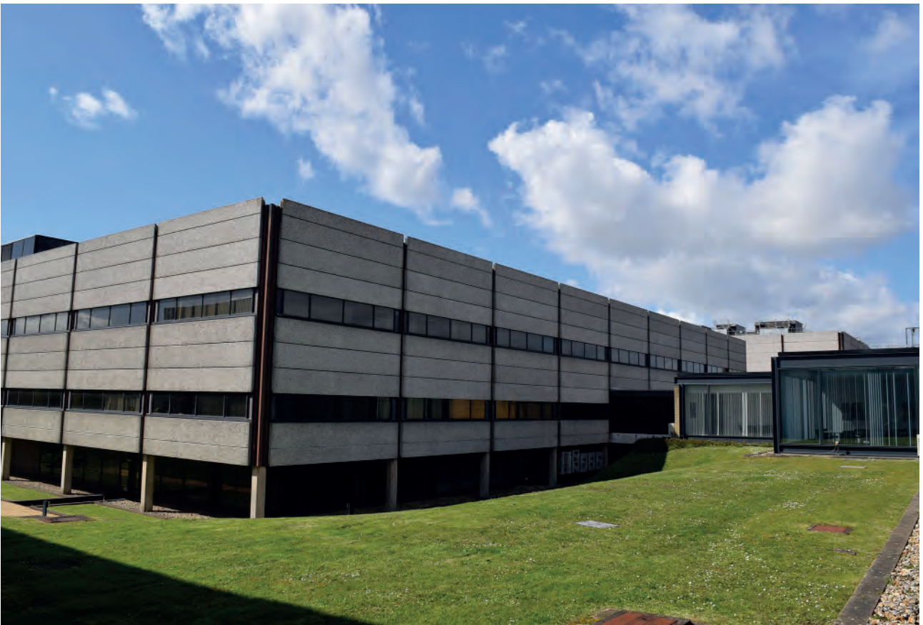
Plate 48: North elevation of Building 6000, looking south- west.
