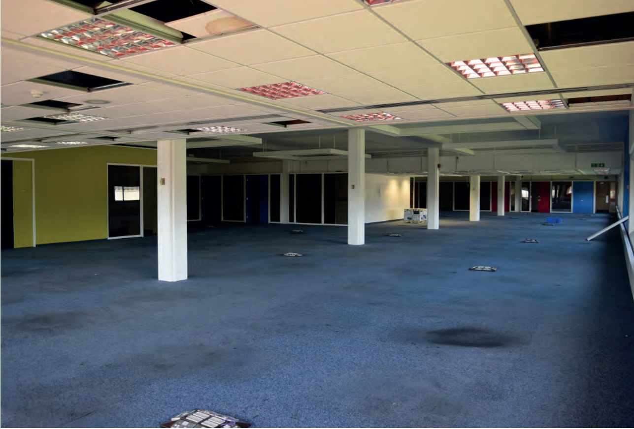
Plate 352: East wing of Building 6000, south office space, looking north- west.
