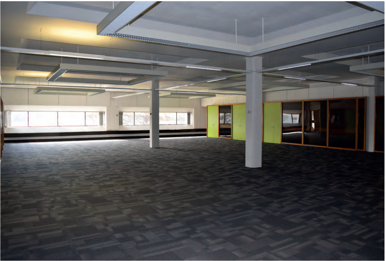
Plate 312: West wing of Building 6000, middle office space, looking north- west.
