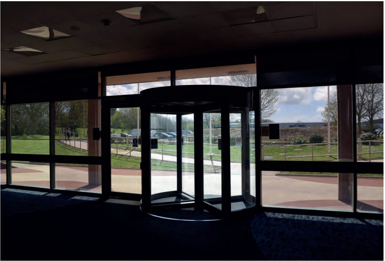
Plate 72: South part of Building 6000, main entrance, looking south.
