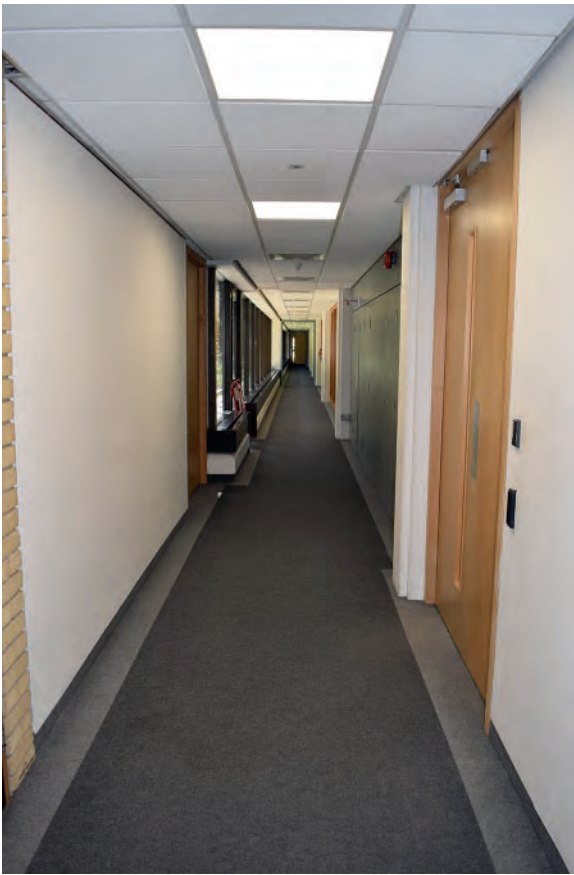
Plate 136: West wing of Building 6000, middle part of west corridor, looking south.
