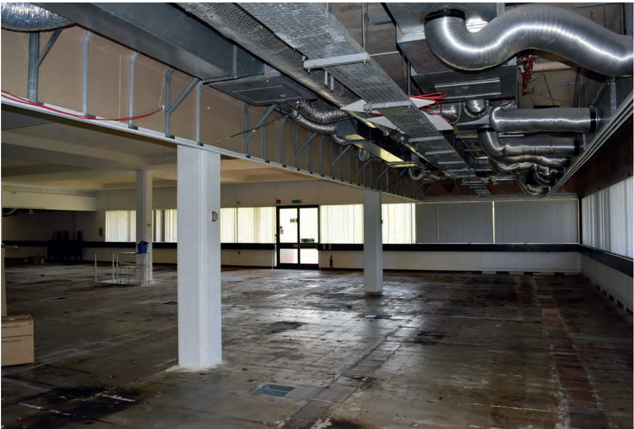
Plate 97: East wing of Building 6000, south office south office space, looking east.
