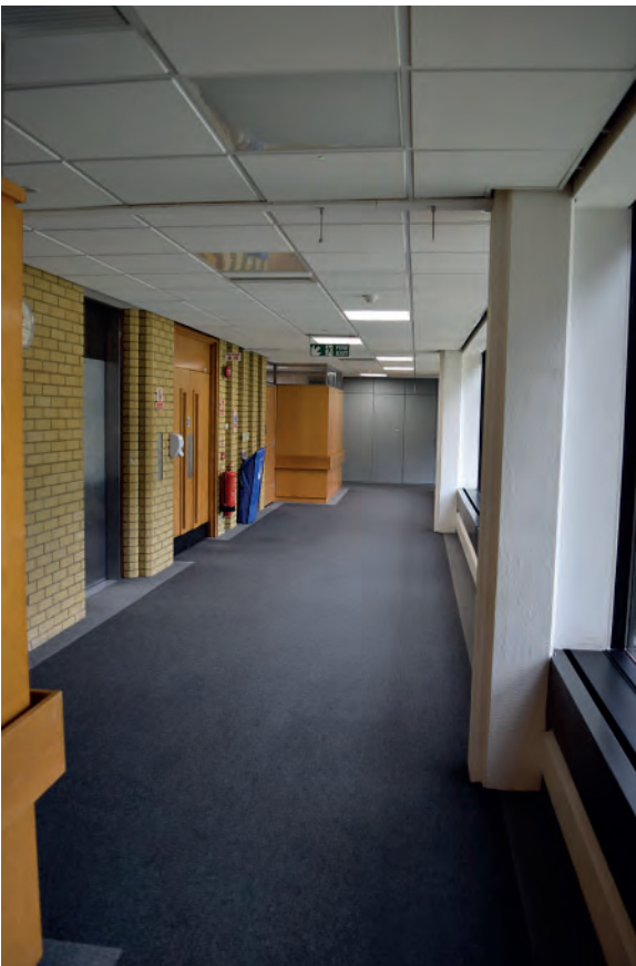
Plate 195: South part of Building 6000, south corridor, looking west.
