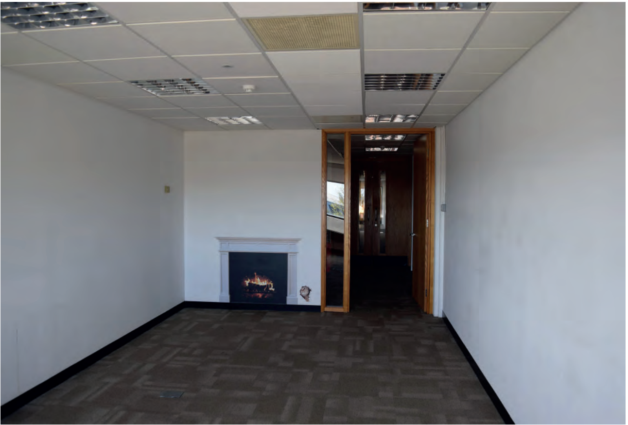
Plate 345: South part of Building 6000, south office space, looking north.
