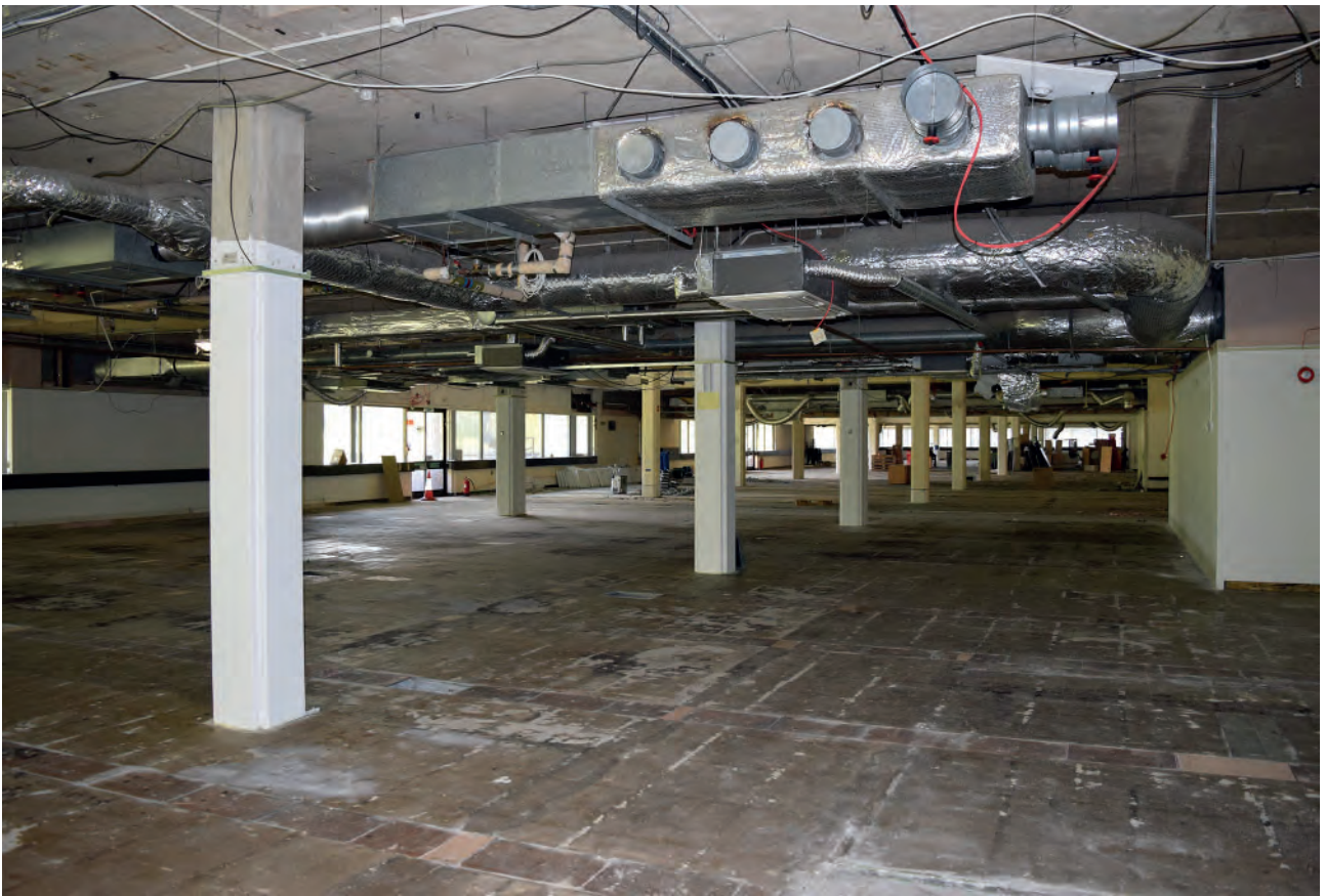
Plate 111: East wing of Building 6000, north office space, looking south-east.
