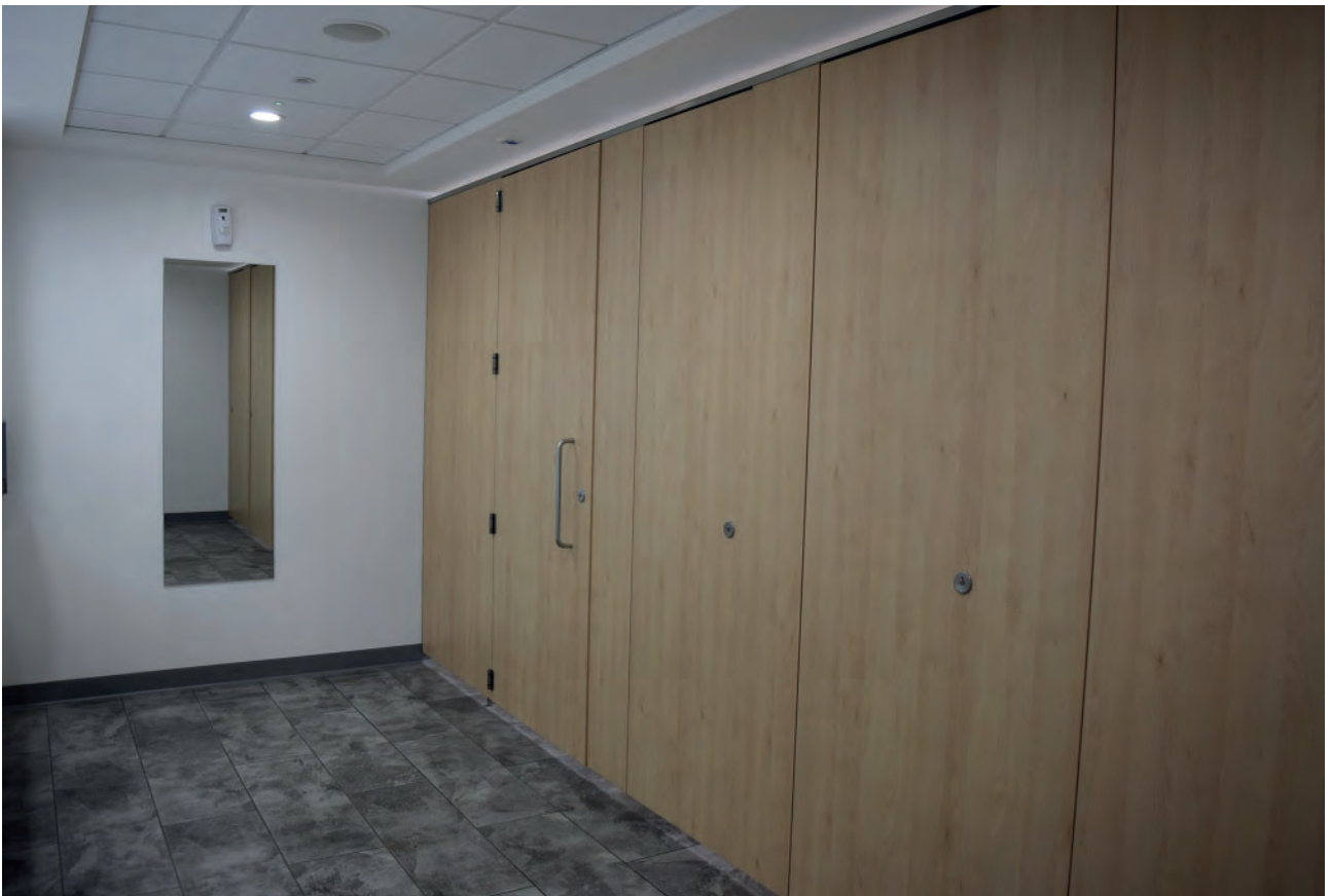
Plate 199: South part of Building 6000, west corridor, women's toilet, looking south-east.
