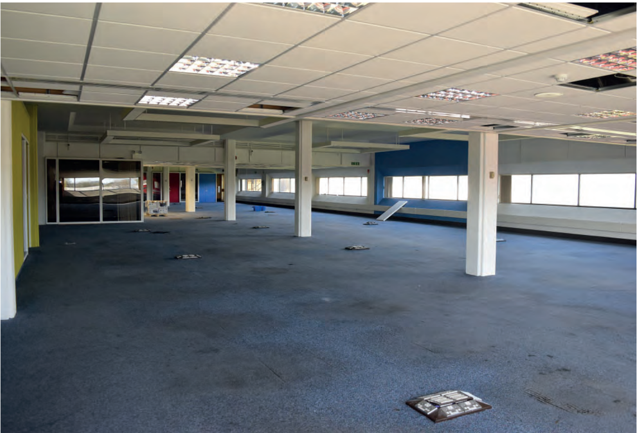
Plate 350: East wing of Building 6000, south office space, looking north-east.
