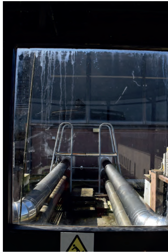
Plate 468: Roof, looking west.
