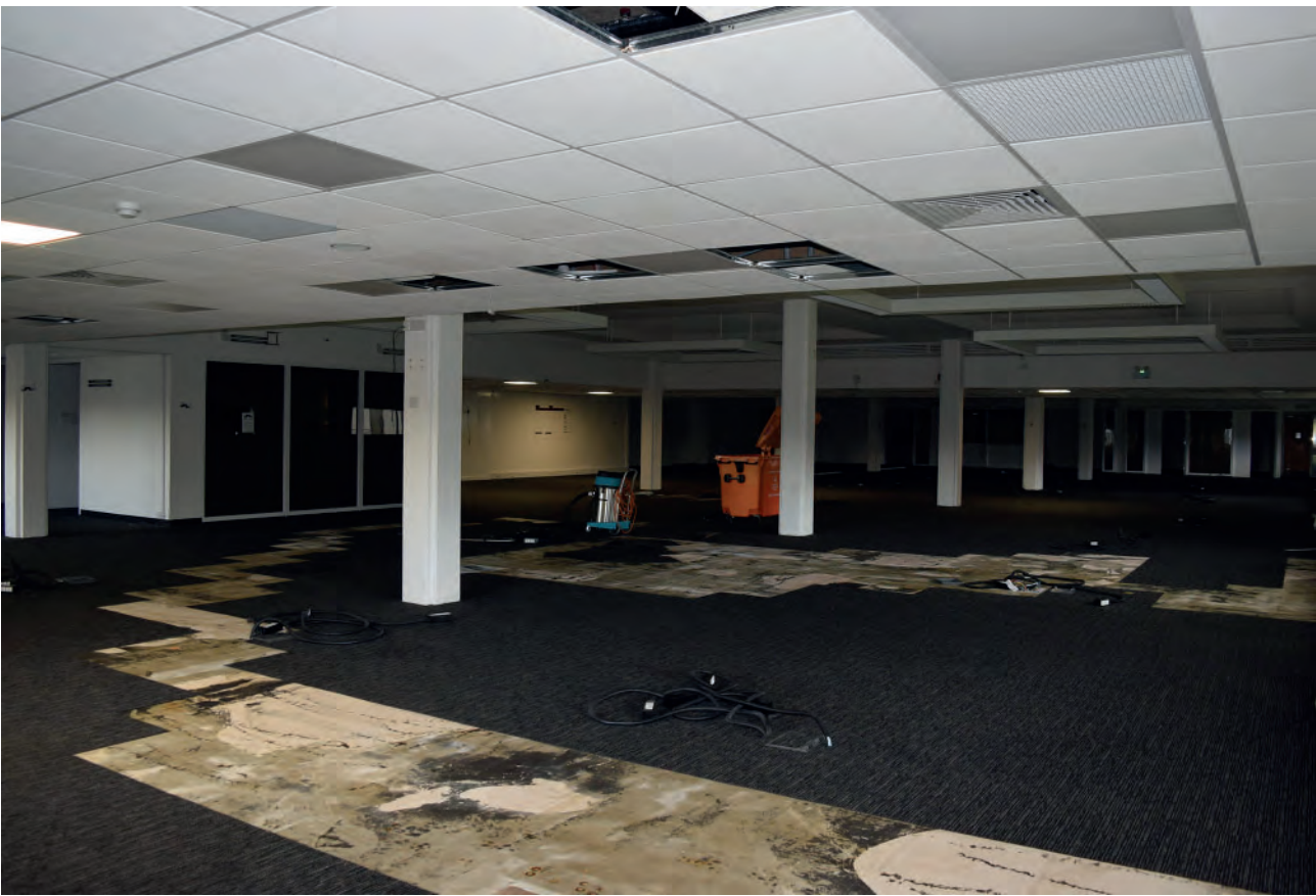
Plate 223: East wing of Building 6000, south office space, looking north- west.
