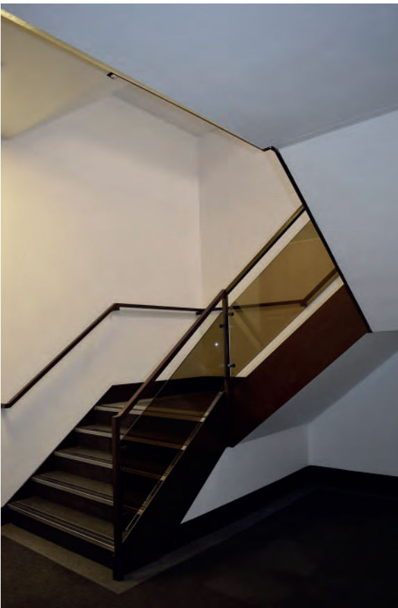
Plate 158: North part of Building 6000, staircase, looking south- east.
