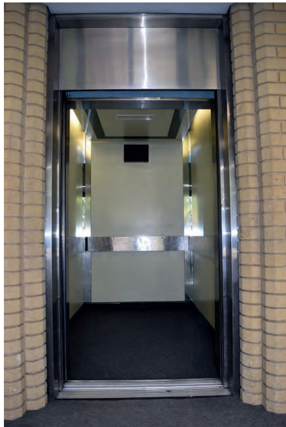
Plate 84: South part of Building 6000, south corridor, elevator entrance, looking south.
