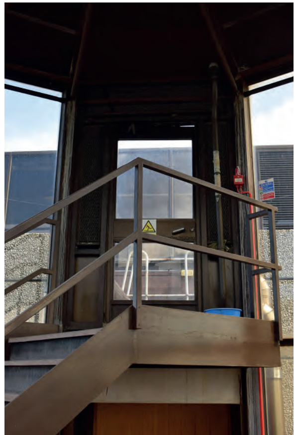
Plate 485: Roof door, looking east.
