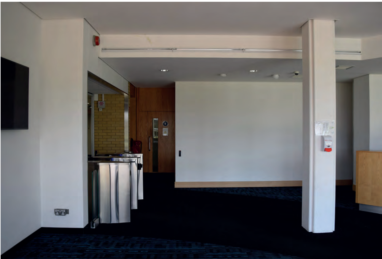
Plate 75: South part of Building 6000, west part of the main reception, looking north.
