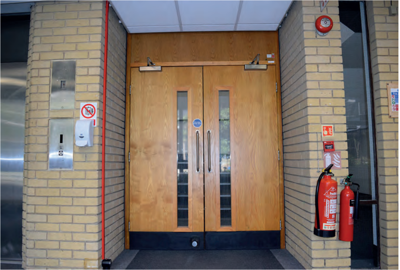
Plate 85: South part of Building 6000, south corridor, stairway entrance, looking south.
