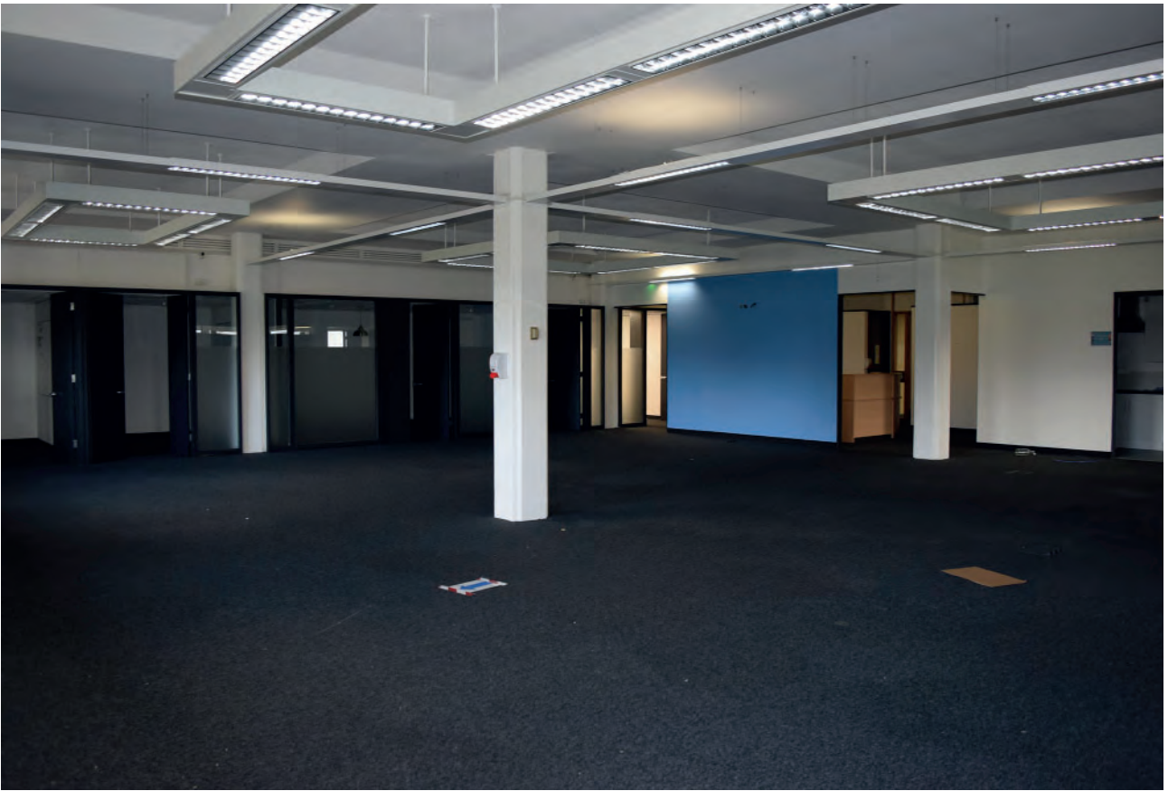
Plate 118: West wing of Building 6000, south office space, looking north- east.
