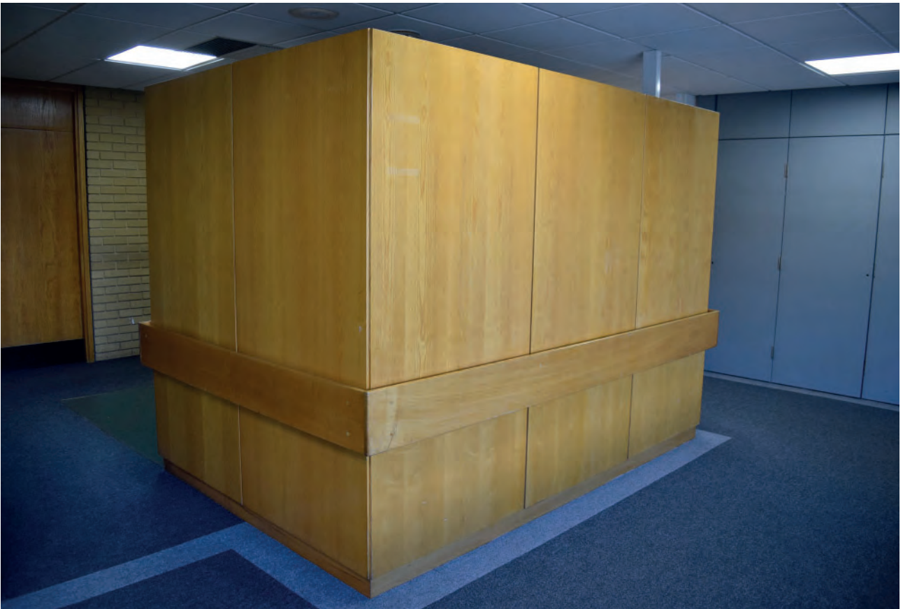
Plate 332: South part of Building 6000, south corridor, west wooden structure, looking south- west.
