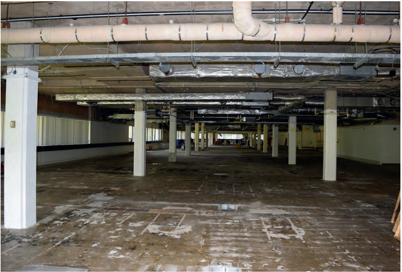
Plate 110: East wing of Building 6000, north office space, looking south.
