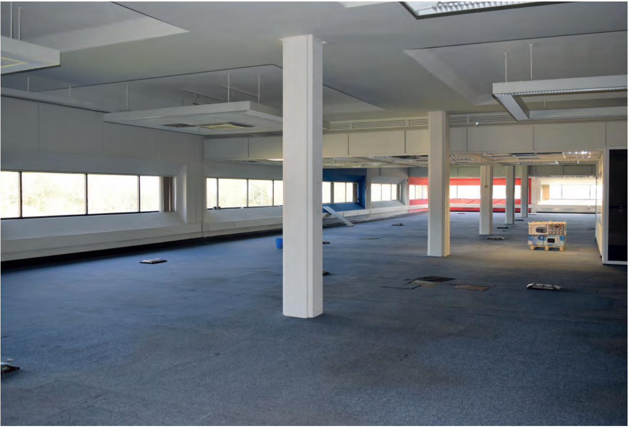
Plate 358: East wing of Building 6000, middle office space, looking south- east.
