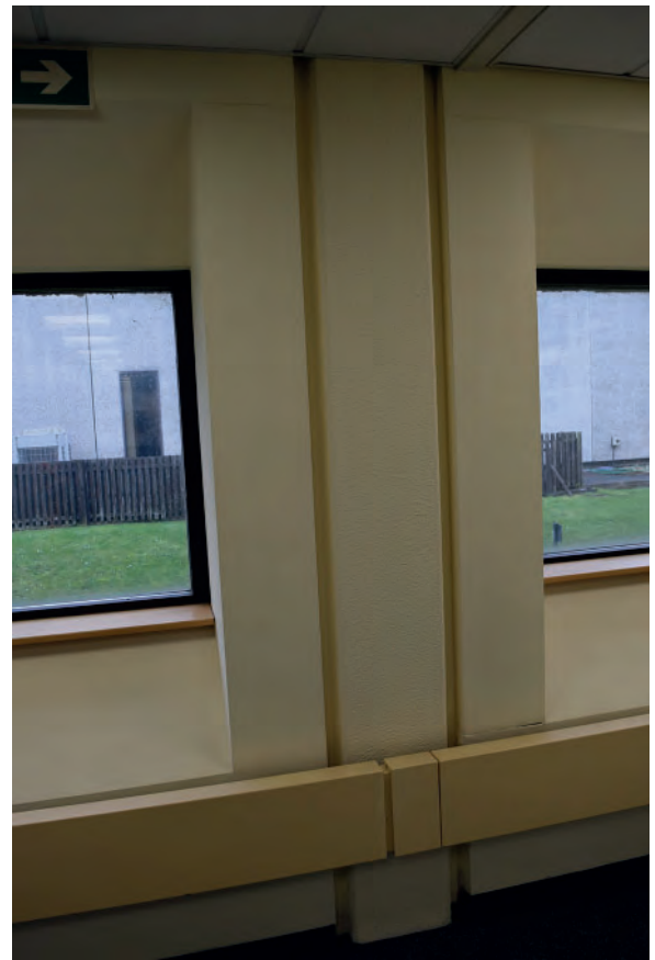
Plate 261: East wing of Building 6000, north office space, steel beam, looking east.
