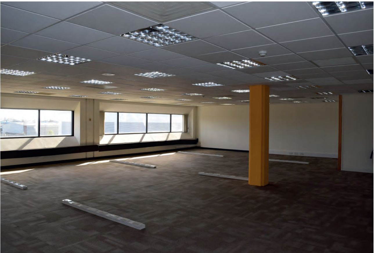
Plate 346: South part of Building 6000, south office space, looking south- west.
