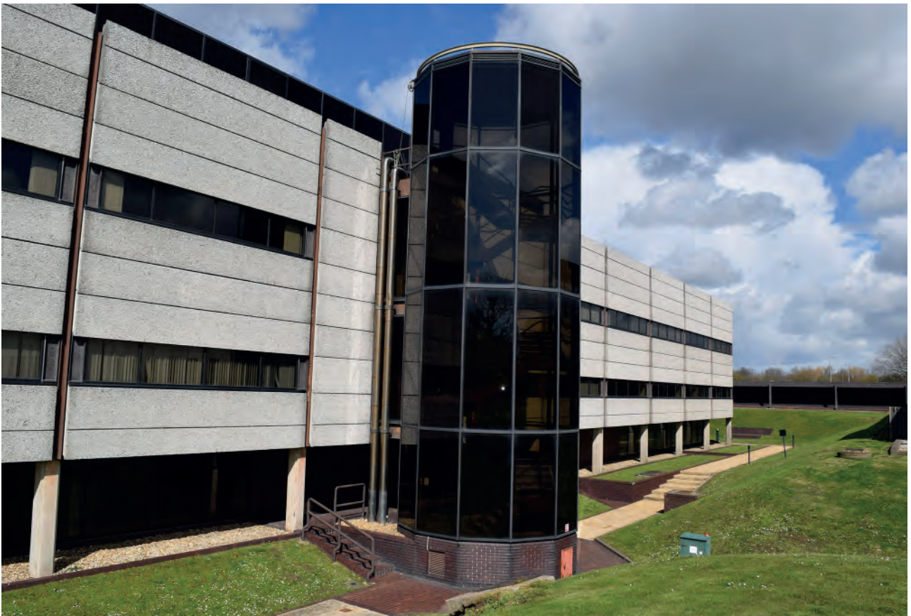
Plate 38: East elevation of Building 6000, looking north- west.
