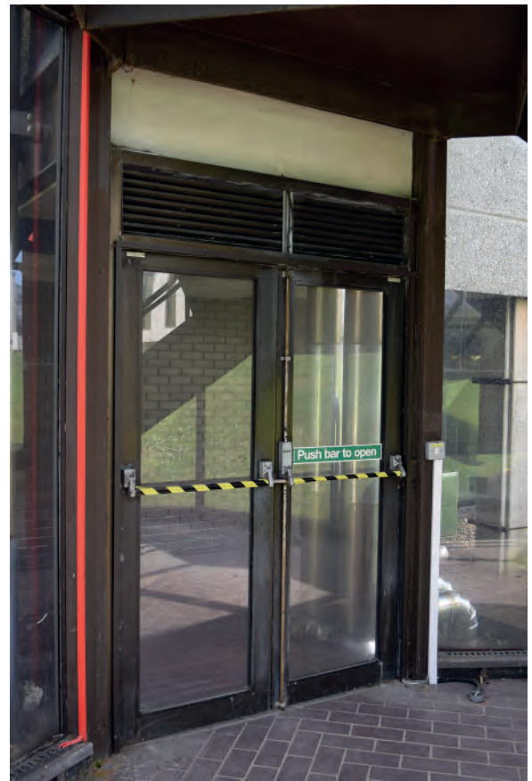
Plate 458: Ground Floor, emergency door, looking north- west.
