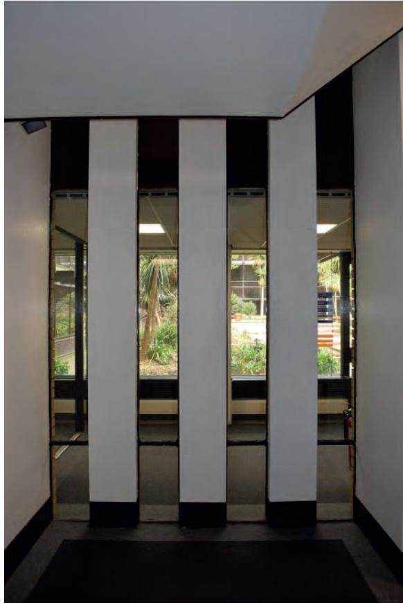
Plate 167: South part of Building 6000, staircase glazing, looking north.
