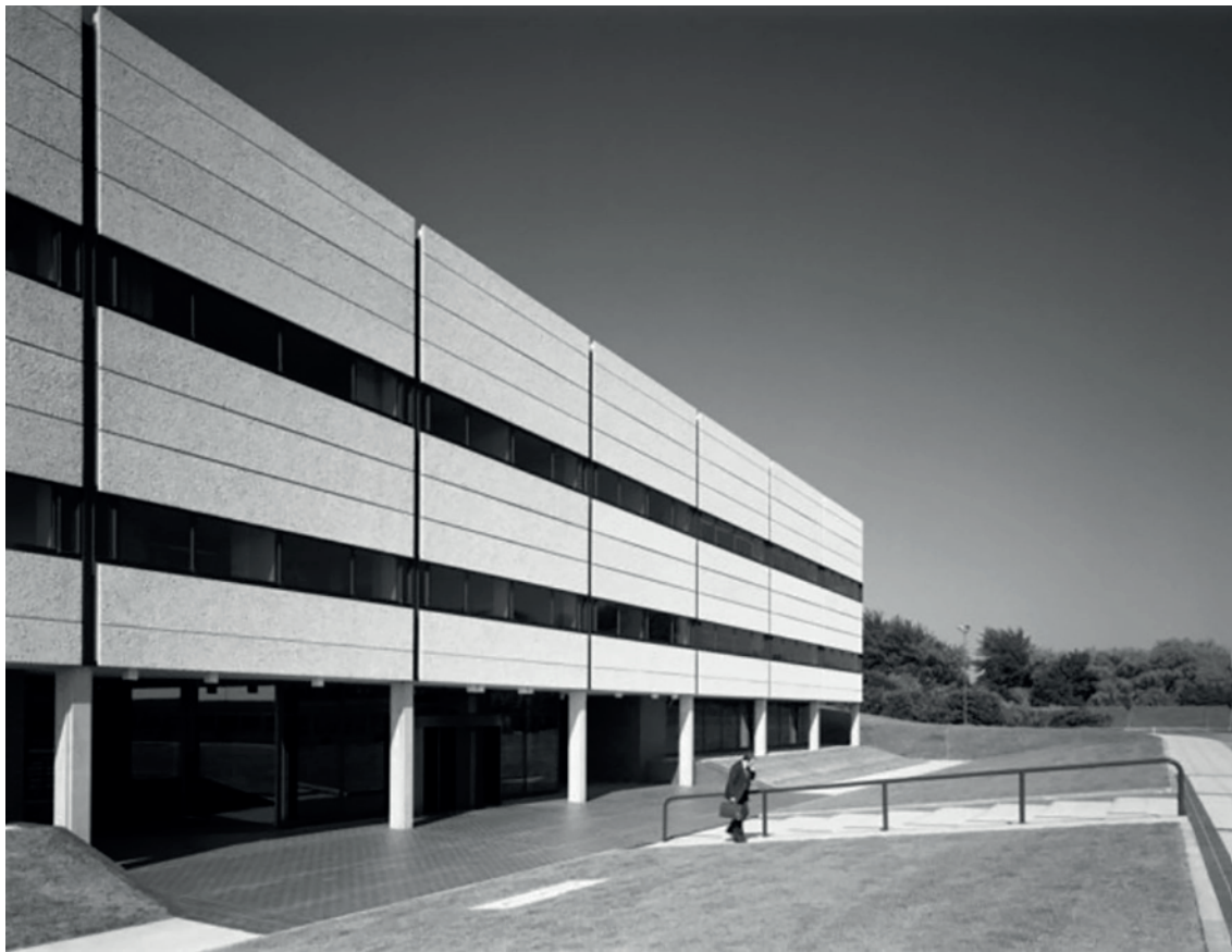
Plate 2: Main entrance to Building 6000, looking north- east, 1980.
