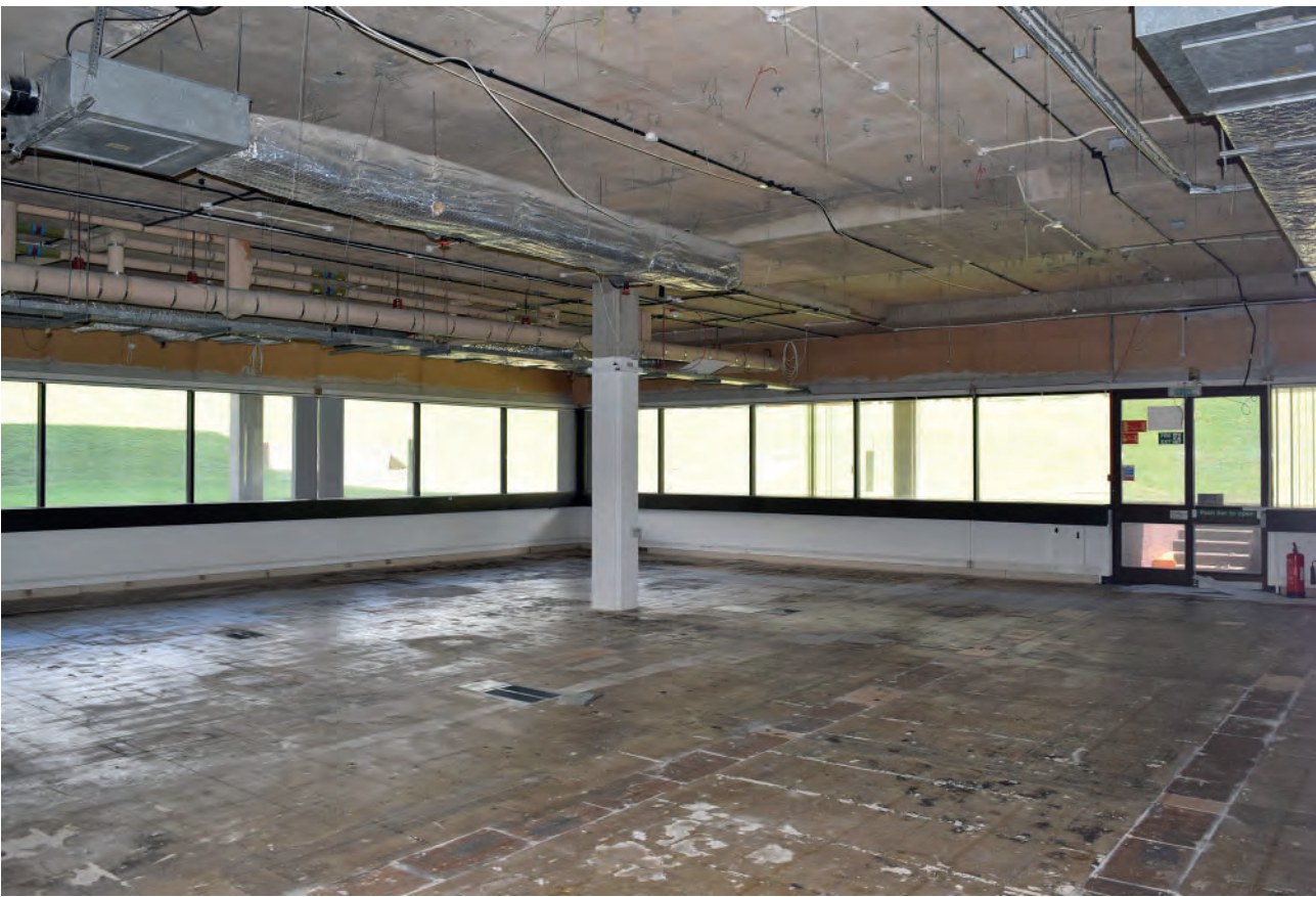
Plate 112: East wing of Building 6000, north office space, looking north- east.
