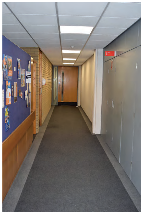
Plate 285: North part of Building 6000, west corridor, looking south.
