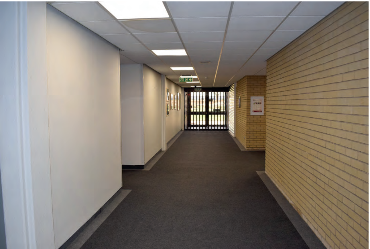
Plate 82: South part of Building 6000, east corridor of, looking south.
