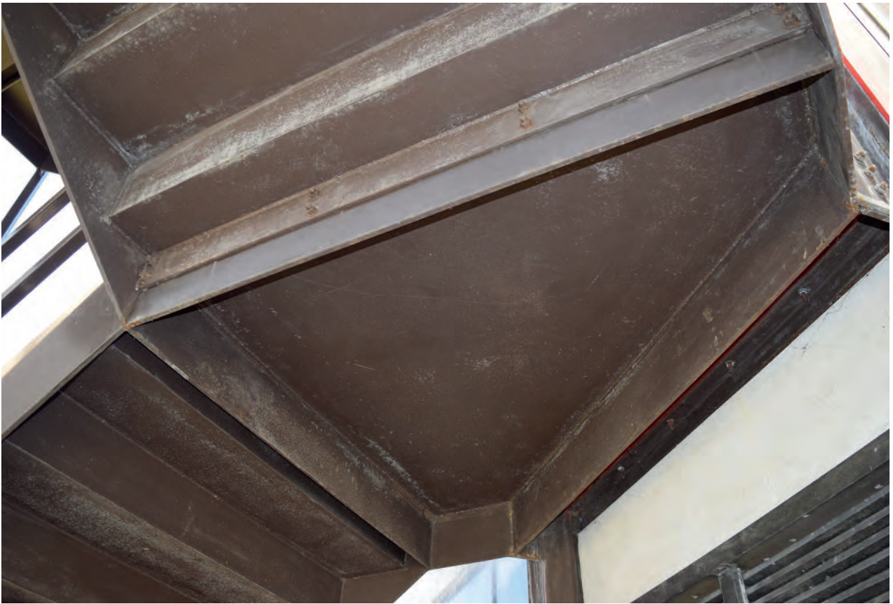
Plate 479: Construction of stairs, landing.
