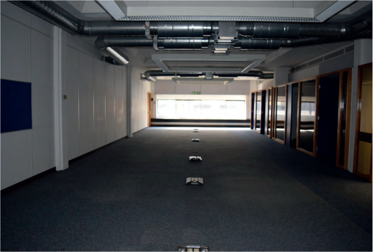
Plate 303: West wing of Building 6000, middle office space, looking west.
