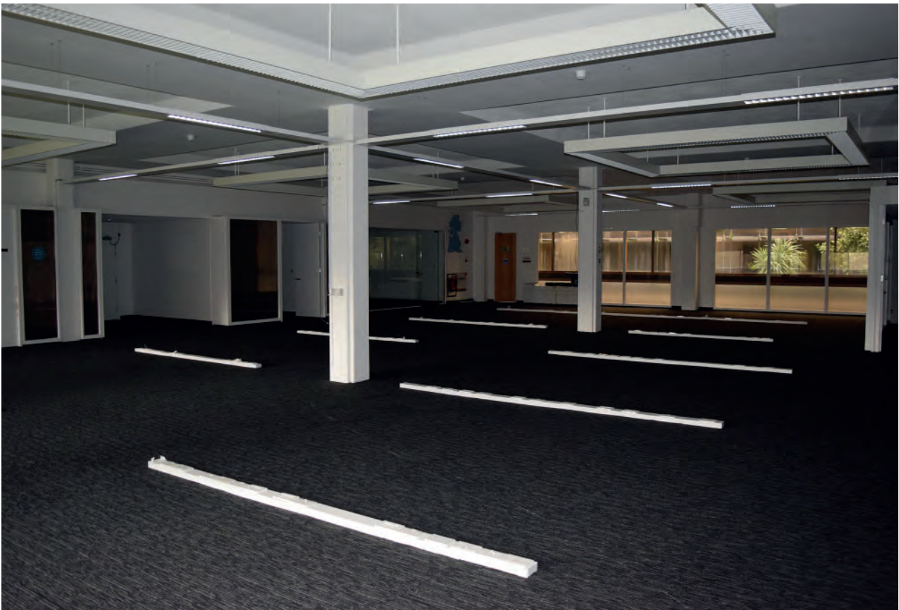
Plate 240: East wing of Building 6000, middle office space, looking south- west.
