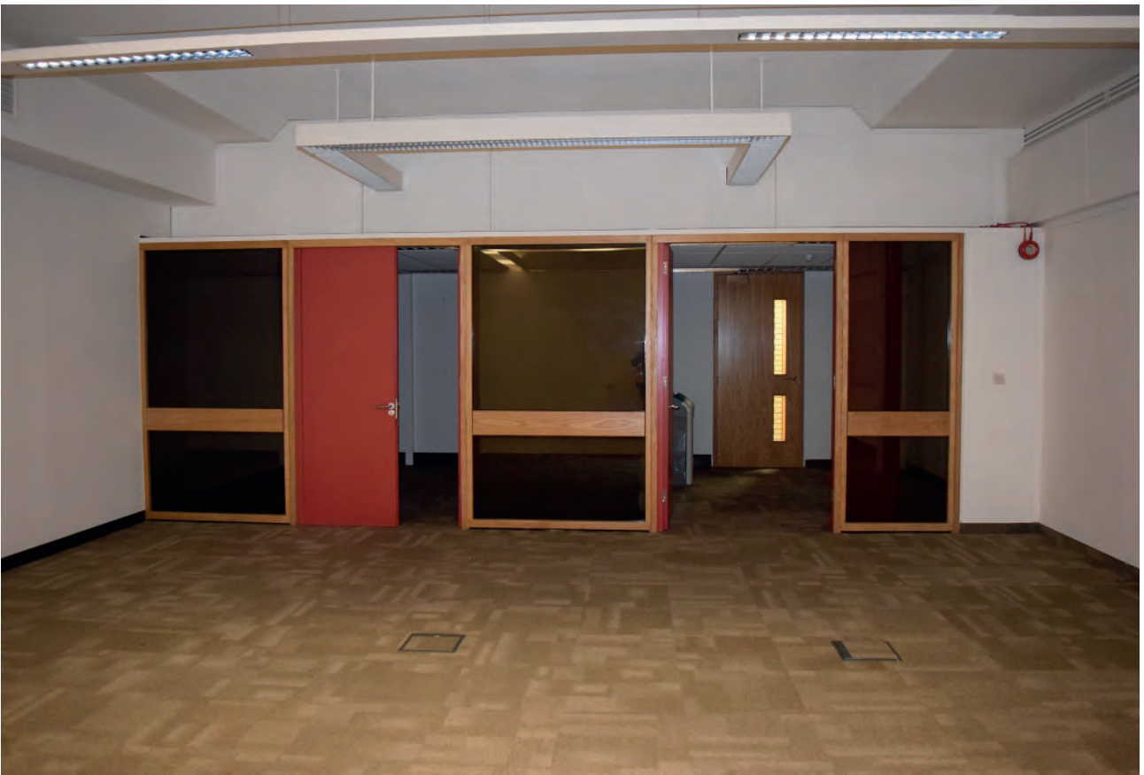
Plate 383: East wing of Building 6000, north office space, looking west.
