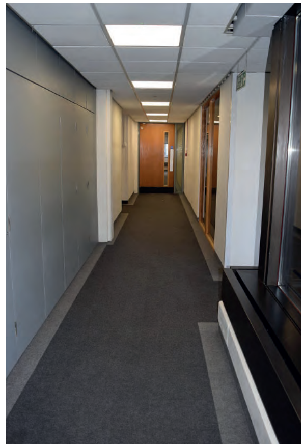
Plate 401: North part of Building 6000, west corridor, looking north.
