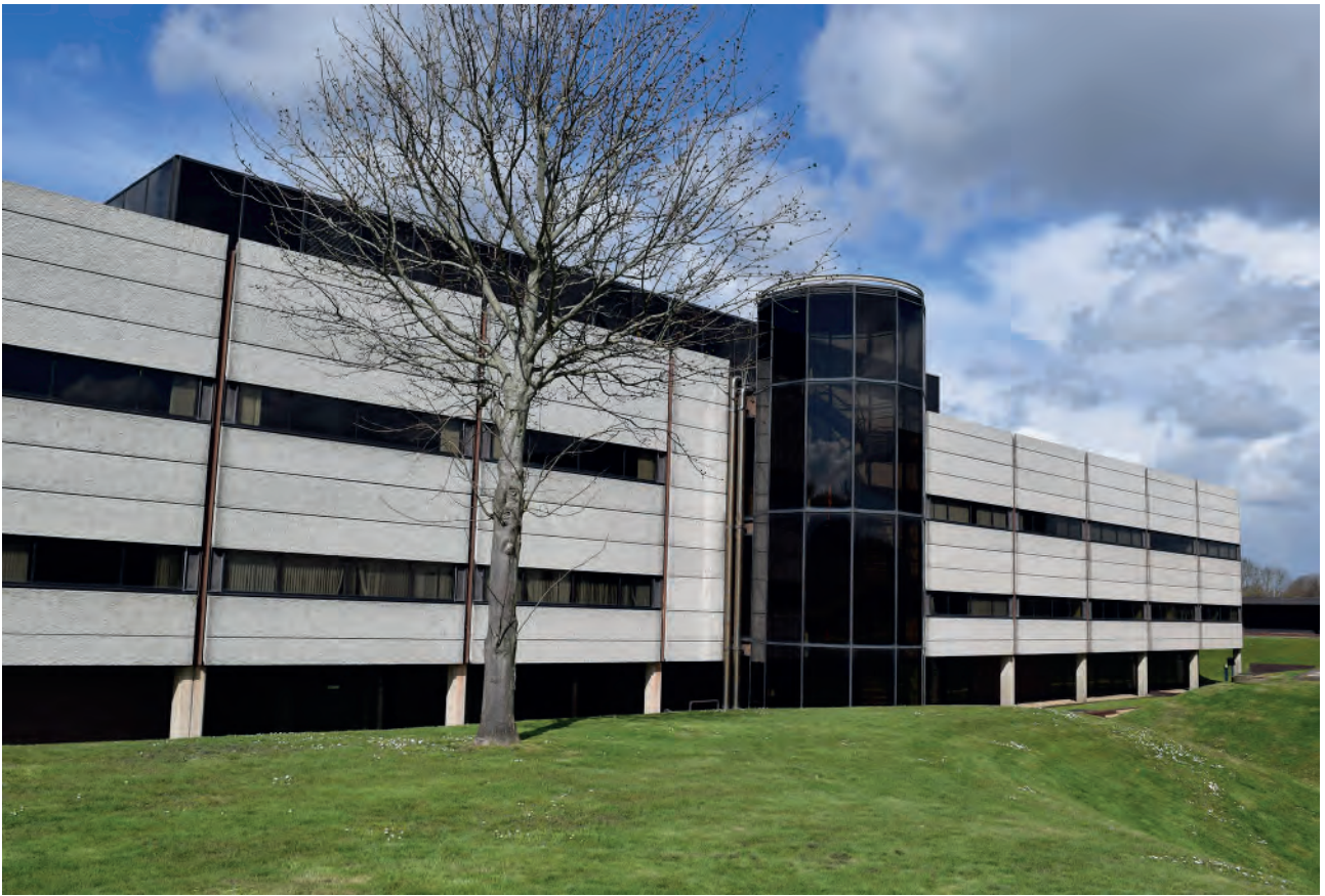
Plate 37: East elevation of Building 6000, looking north- west.
