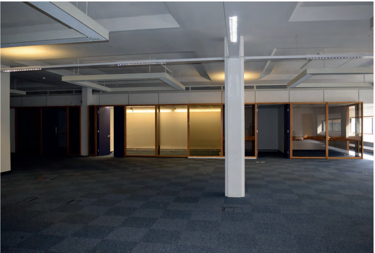
Plate 293: West wing of Building 6000, north office space, looking south.
