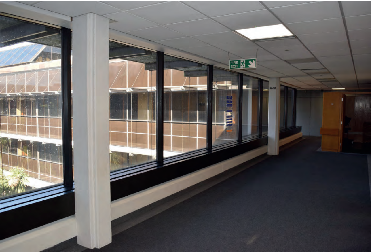
Plate 330: South part of Building 6000, south corridor, looking north- east.
