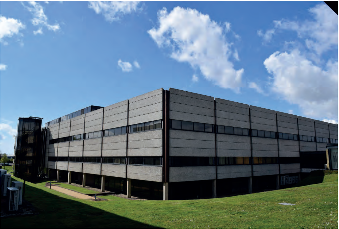
Plate 47: North- east corner of Building 6000, looking south- west.
