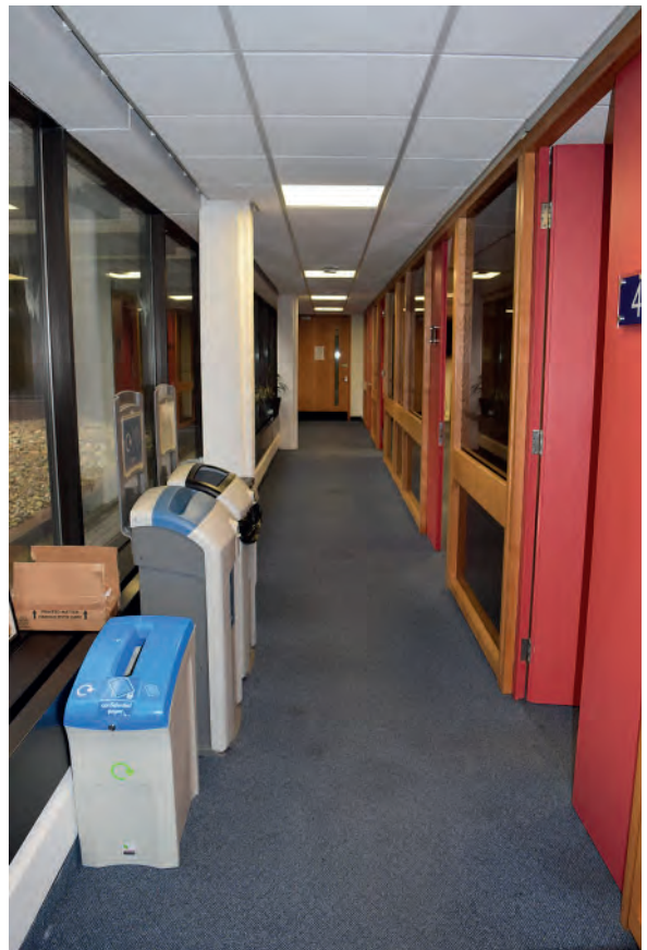
Plate 172: North part of Building 6000, corridor along the north side of the courtyard, looking west.
