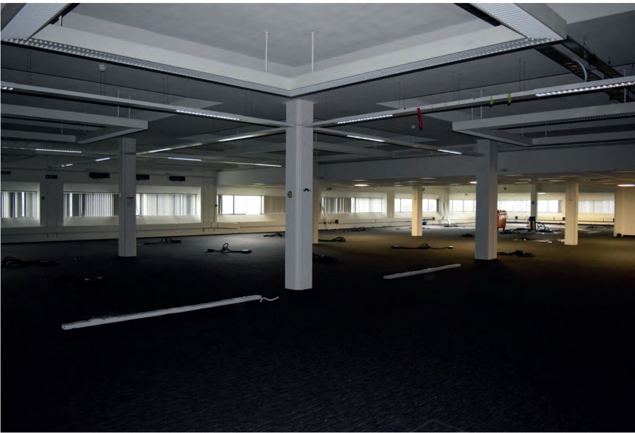
Plate 231: East wing of Building 6000, middle office space, looking south- east.
