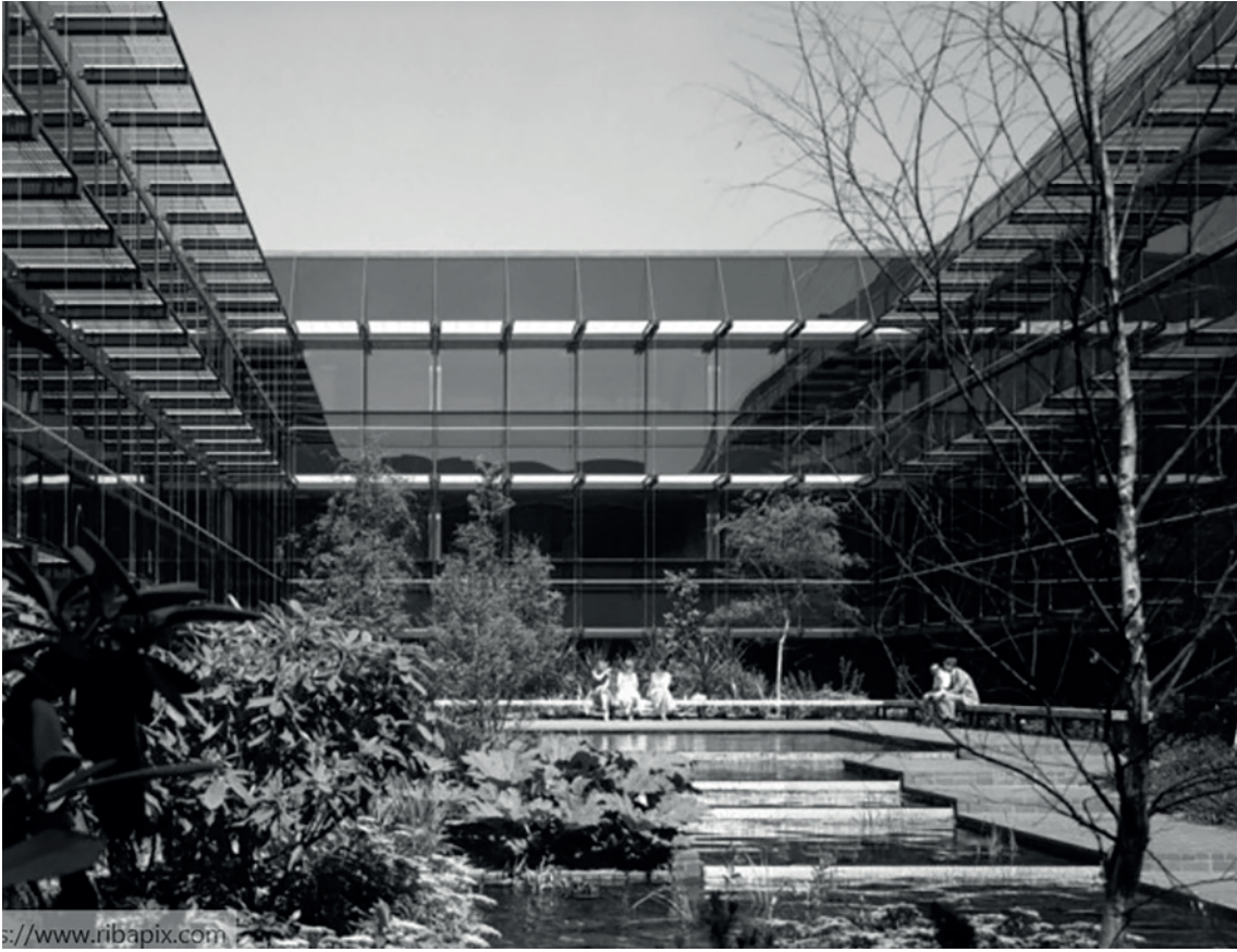
Plate 19: Ground Floor, courtyard, looking north, 1980.
