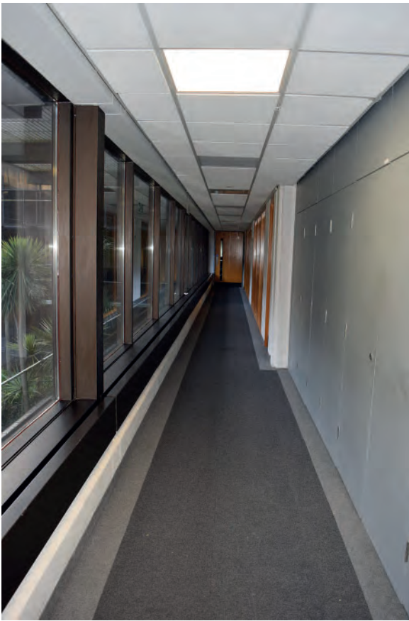
Plate 309: West wing of Building 6000, middle part of west corridor, looking south.
