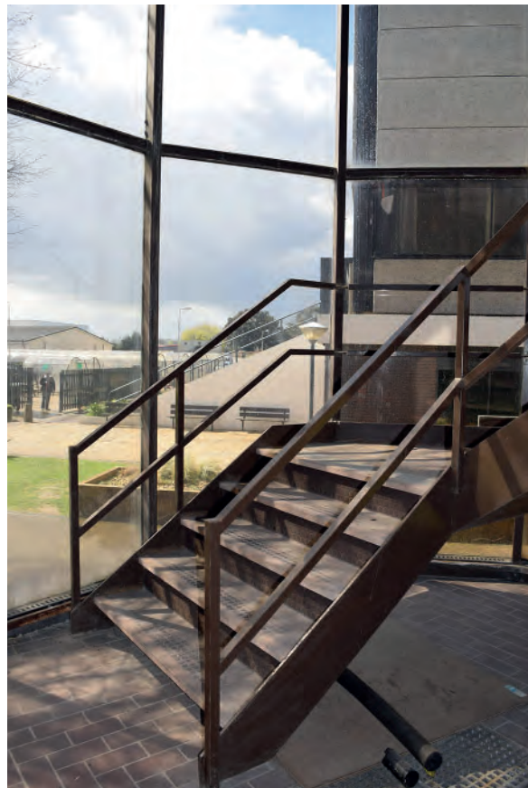
Plate 480: Construction of stairs, looking west.
