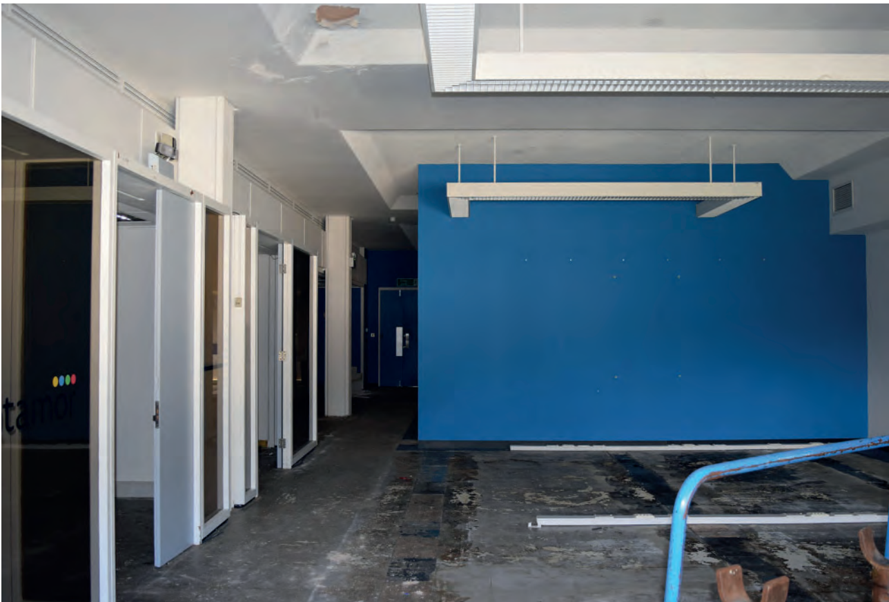
Plate 360: East wing of Building 6000, middle office space, looking west.
