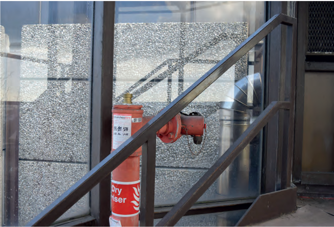
Plate 488: Roof level, hydrant, looking east.
