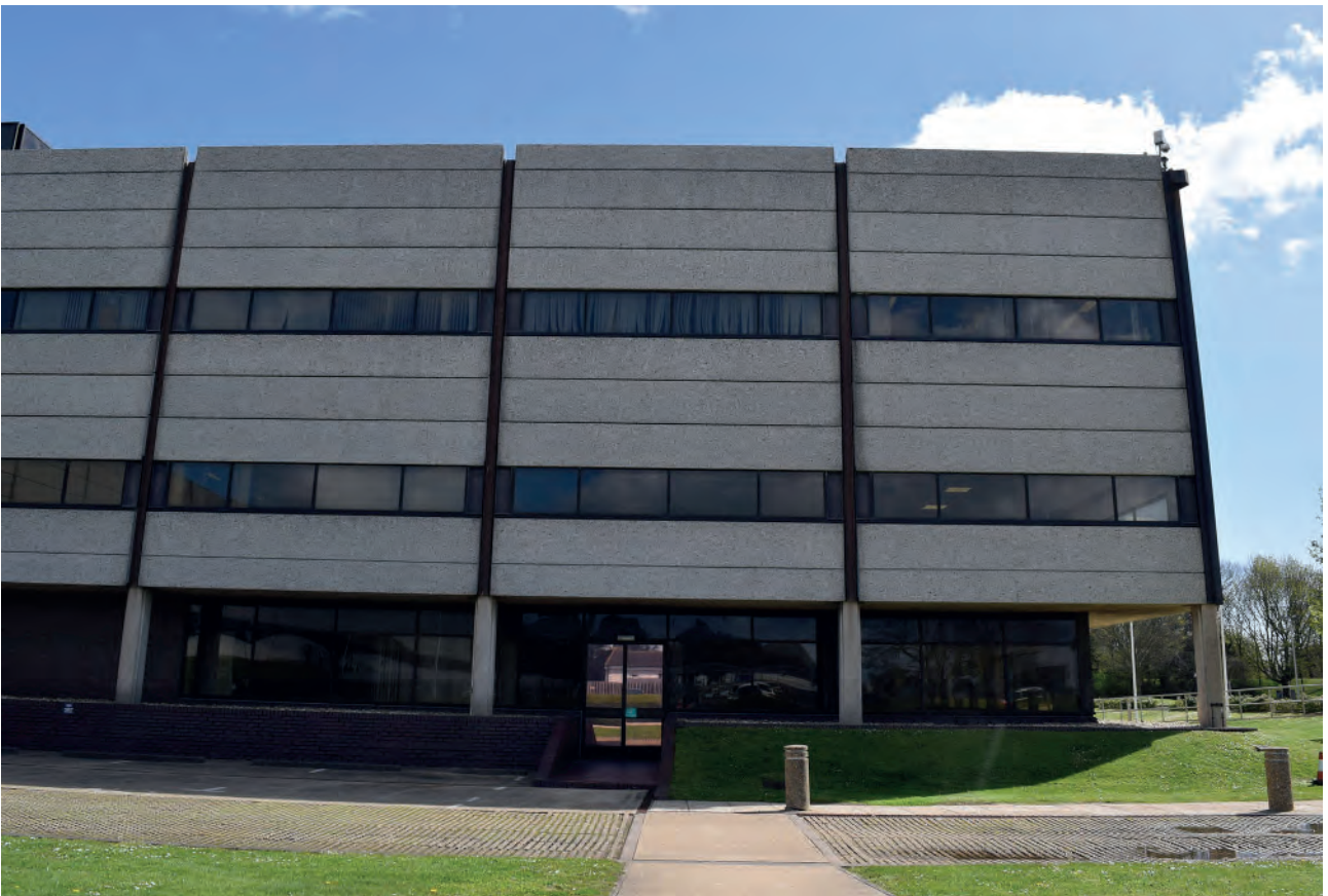
Plate 60: West elevation, one of the glazed emergency exits, looking east.
