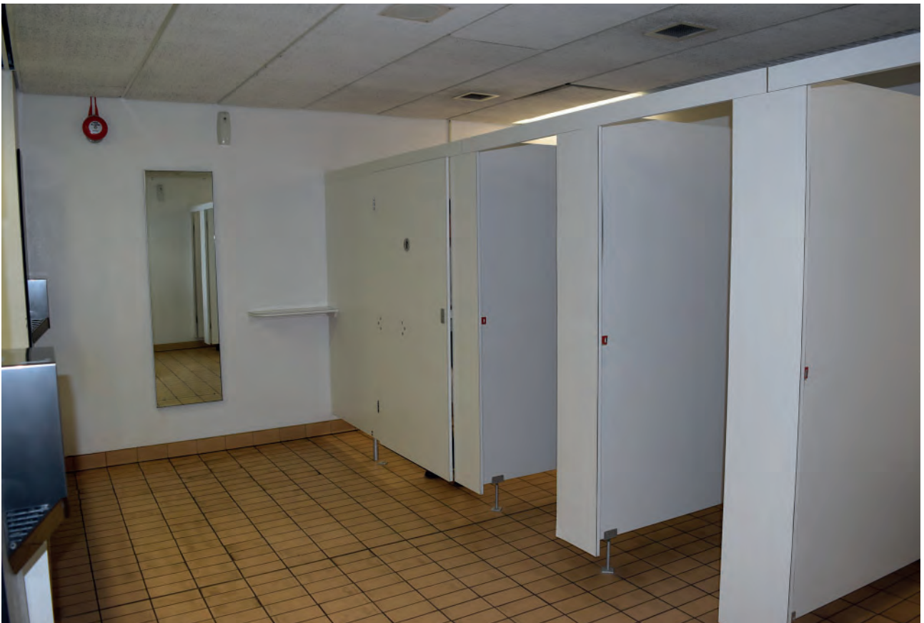
Plate 140: North part of Building 6000, west corridor, women's toilet, looking south-east.
