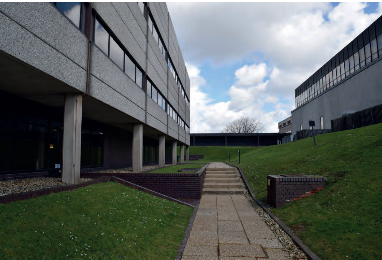
Plate 41: Walkway between buildings 6000 and 7000, looking north.
