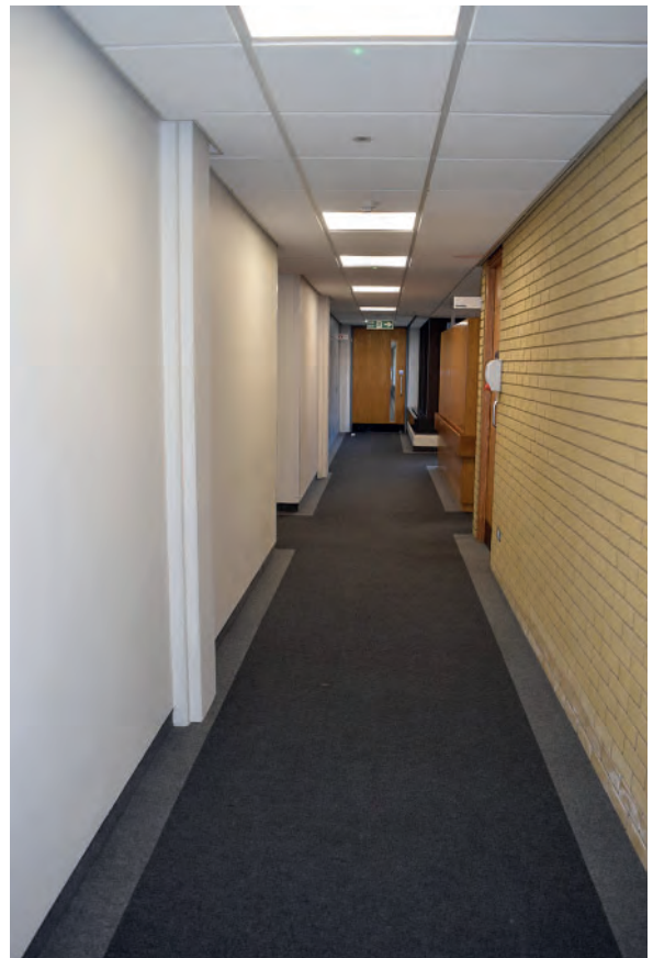
Plate 334: South part of Building 6000, west corridor, looking north.
