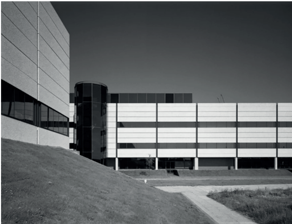
Plate 10: West staircase tower, looking east, 1980.
