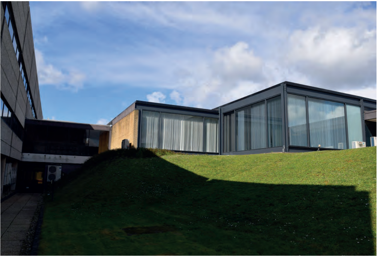
Plate 51: Connection between buildings 6000 and 4000, looking west.
