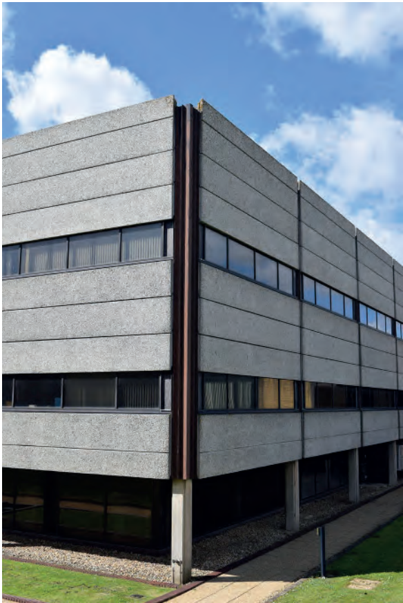
Plate 46: North- east corner of Building 6000, looking south- west.
