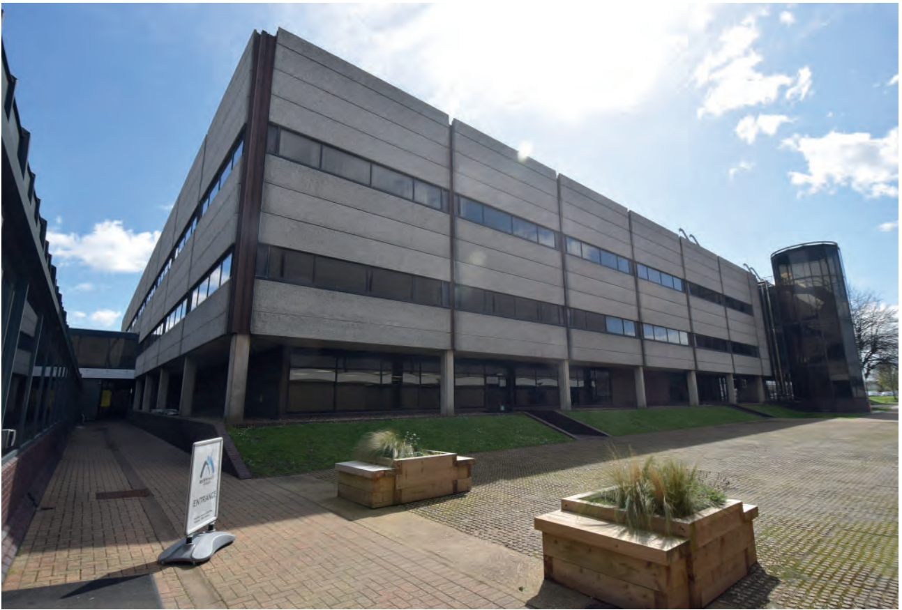
Plate 66: Northwest corner of Building 6000, looking south- east.
