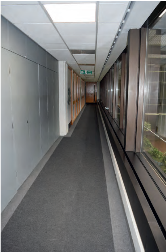
Plate 245: East wing of Building 6000, middle part of east corridor, looking south.
