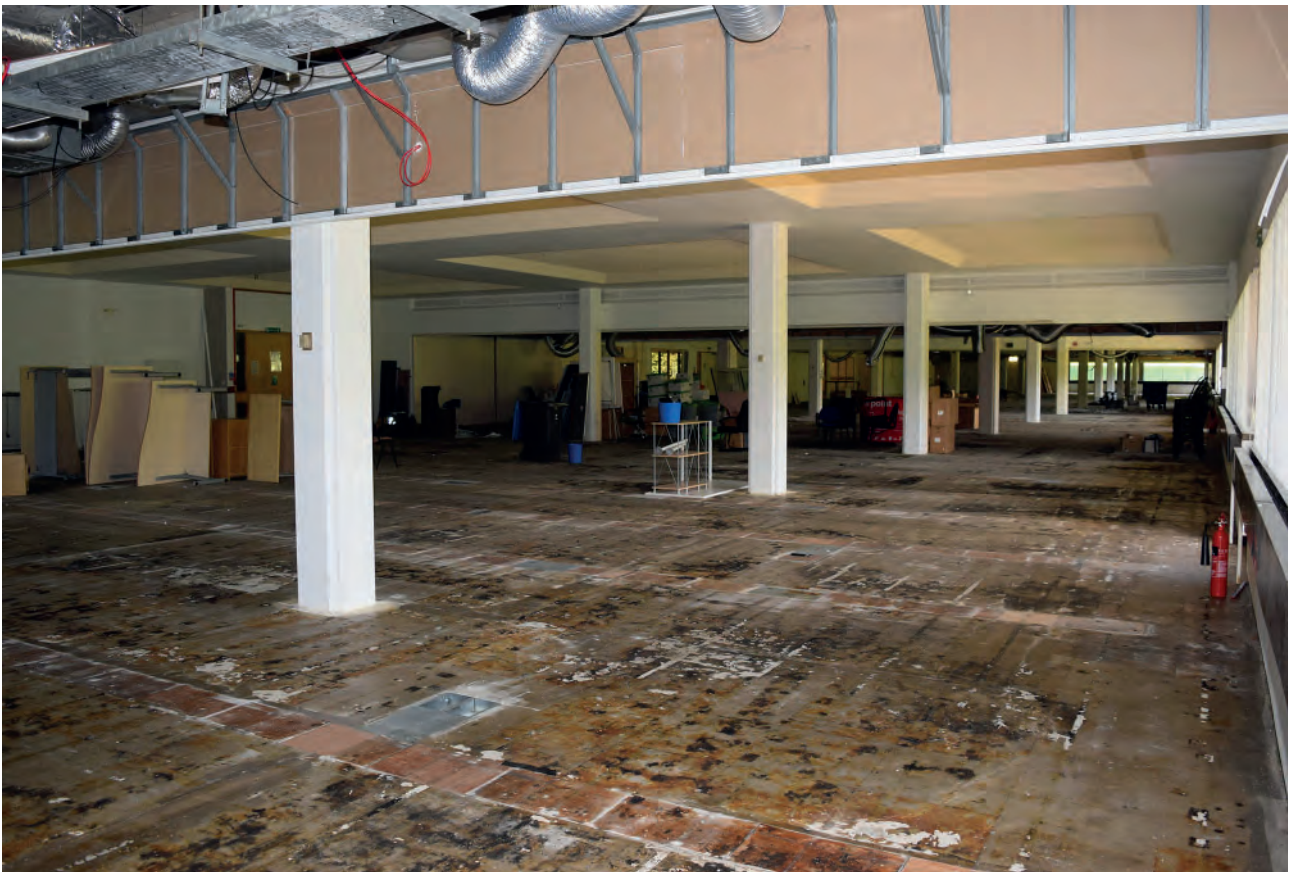
Plate 93: East wing of Building 6000, south office space, looking north-west.
