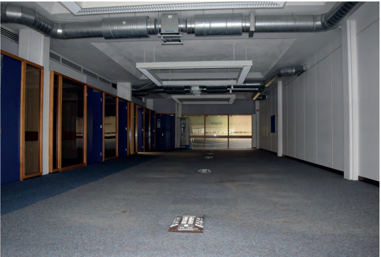
Plate 304: West wing of Building 6000, middle office space, looking east.
