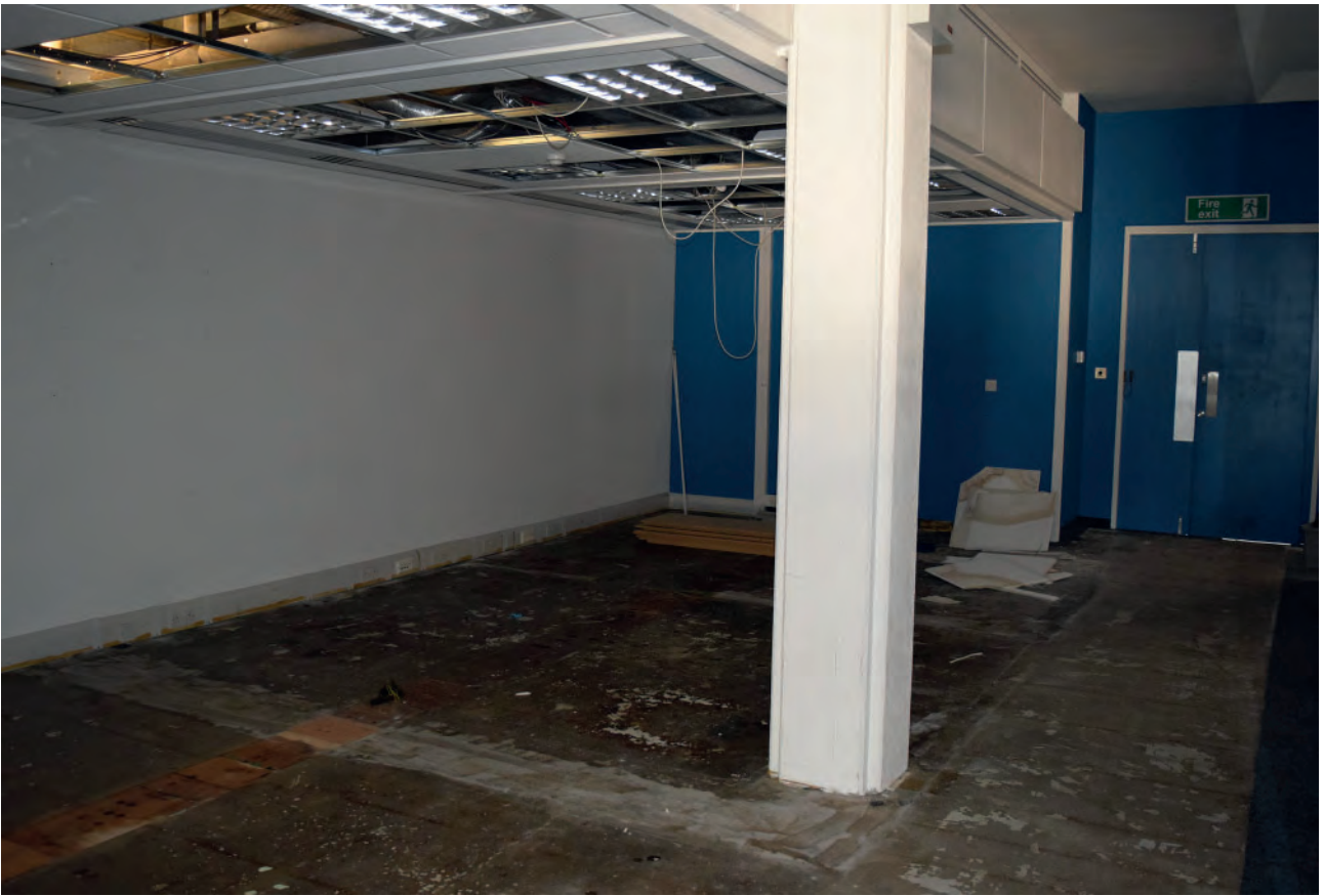
Plate 363: East wing of Building 6000, middle office space, looking south- west.
