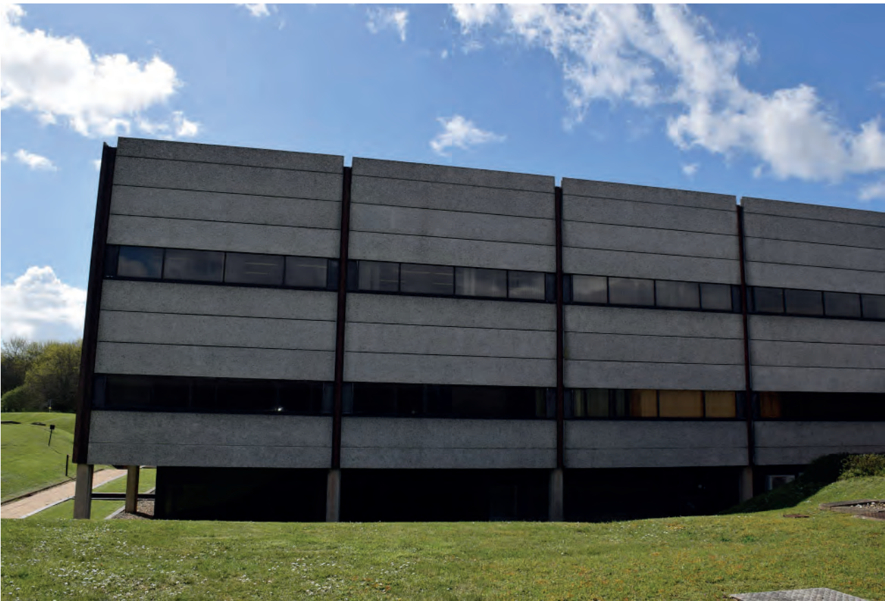
Plate 50: North elevation of Building 6000, looking south.
