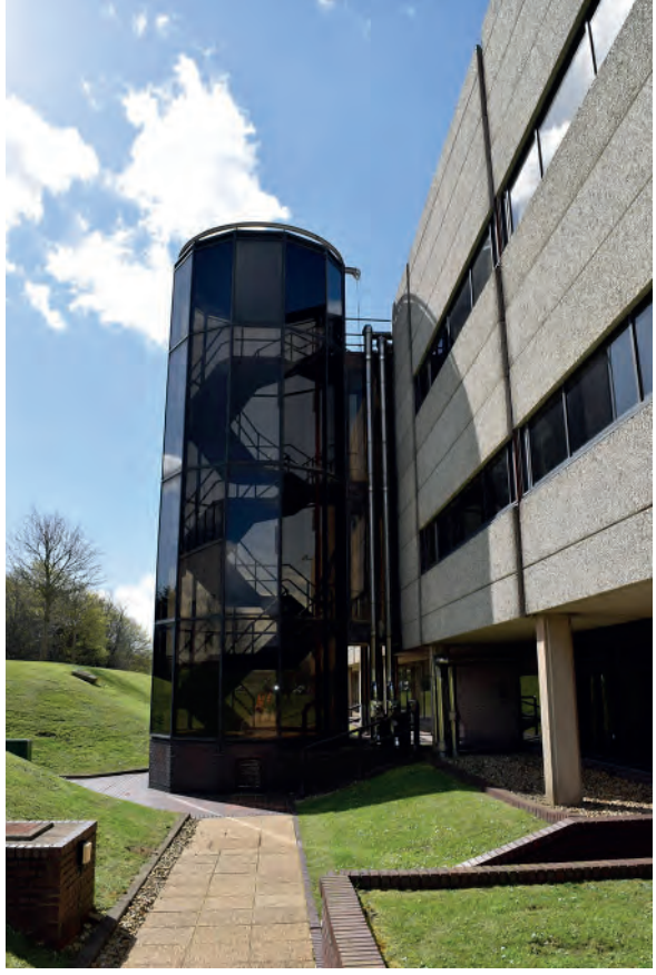
Plate 42: East staircase tower, looking south.
