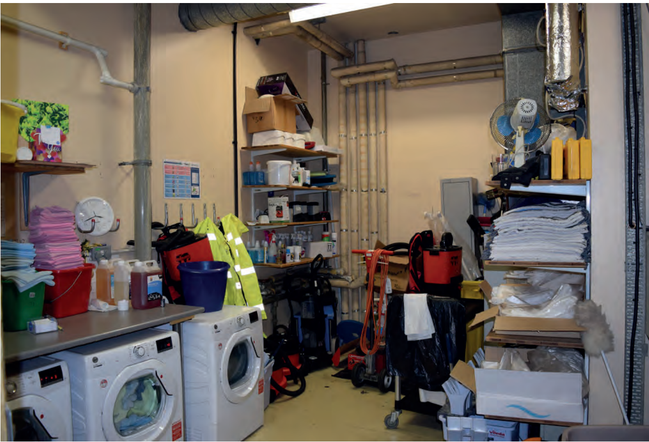
Plate 280: North part of Building 6000, north corridor, utility room, looking south- west.
