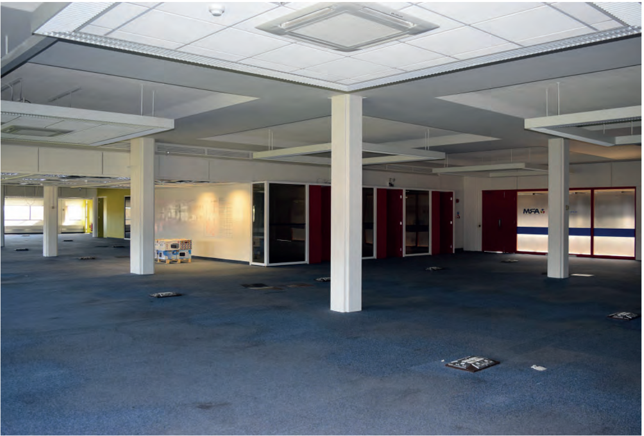
Plate 357: East wing of Building 6000, middle office space, looking south- west.
