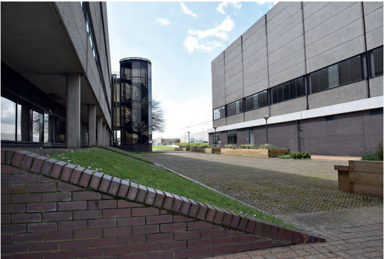
Plate 65: West staircase tower, looking south.
