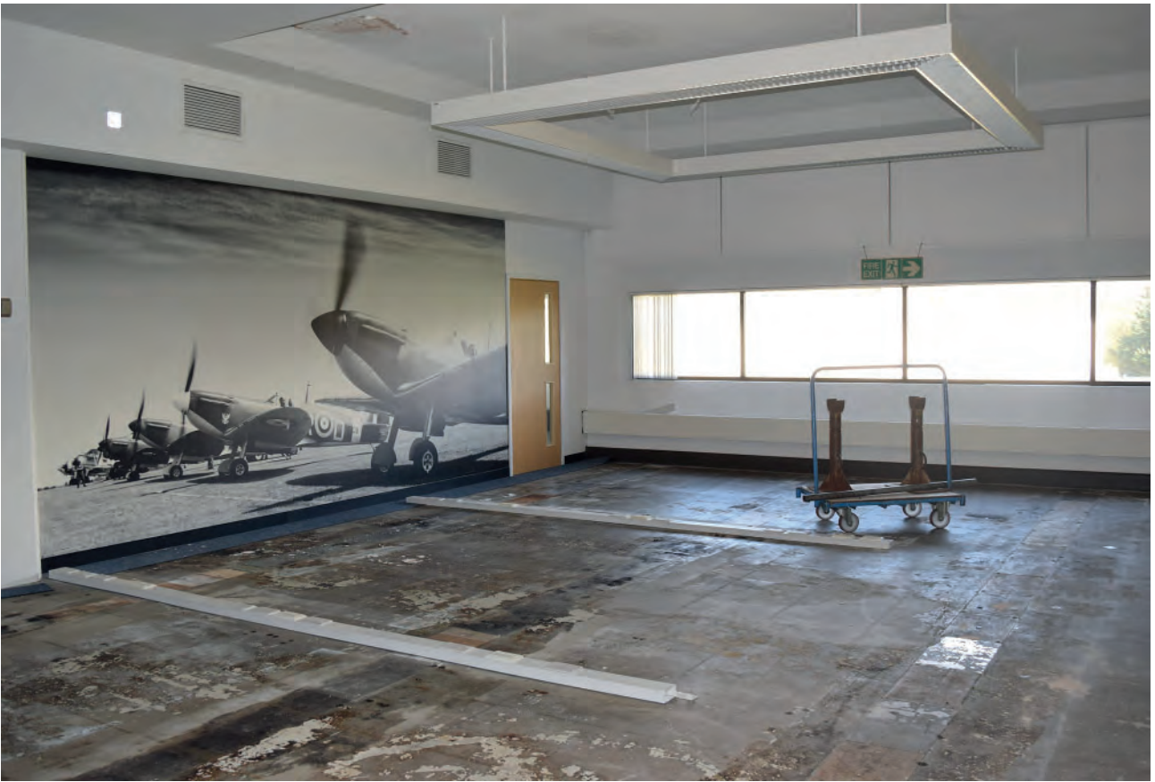
Plate 361: East wing of Building 6000, middle office space, looking east.
