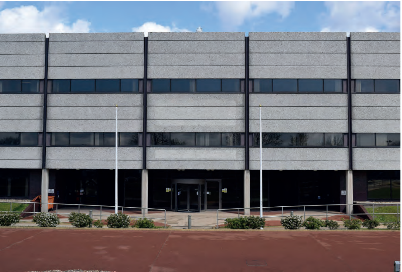
Plate 31: Main entrance to Building 6000, looking north.
