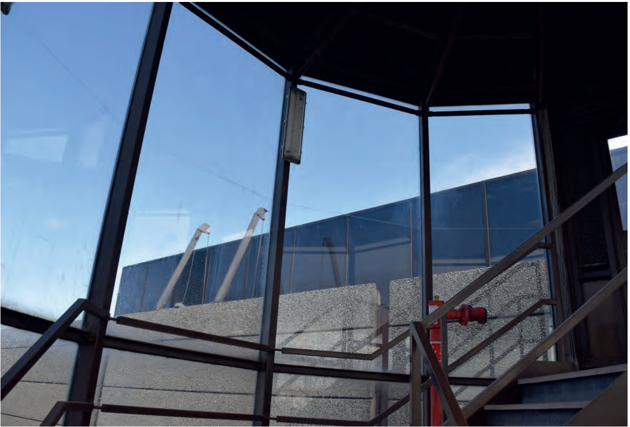
Plate 486: Roof, crane arms, looking north- east.
