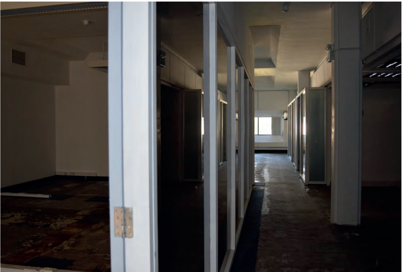
Plate 362: East wing of Building 6000, middle office space, looking east.
