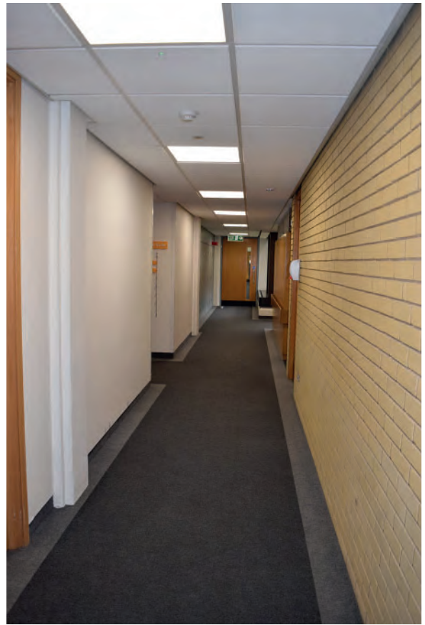
Plate 198: South part of Building 6000, west corridor, looking north.
