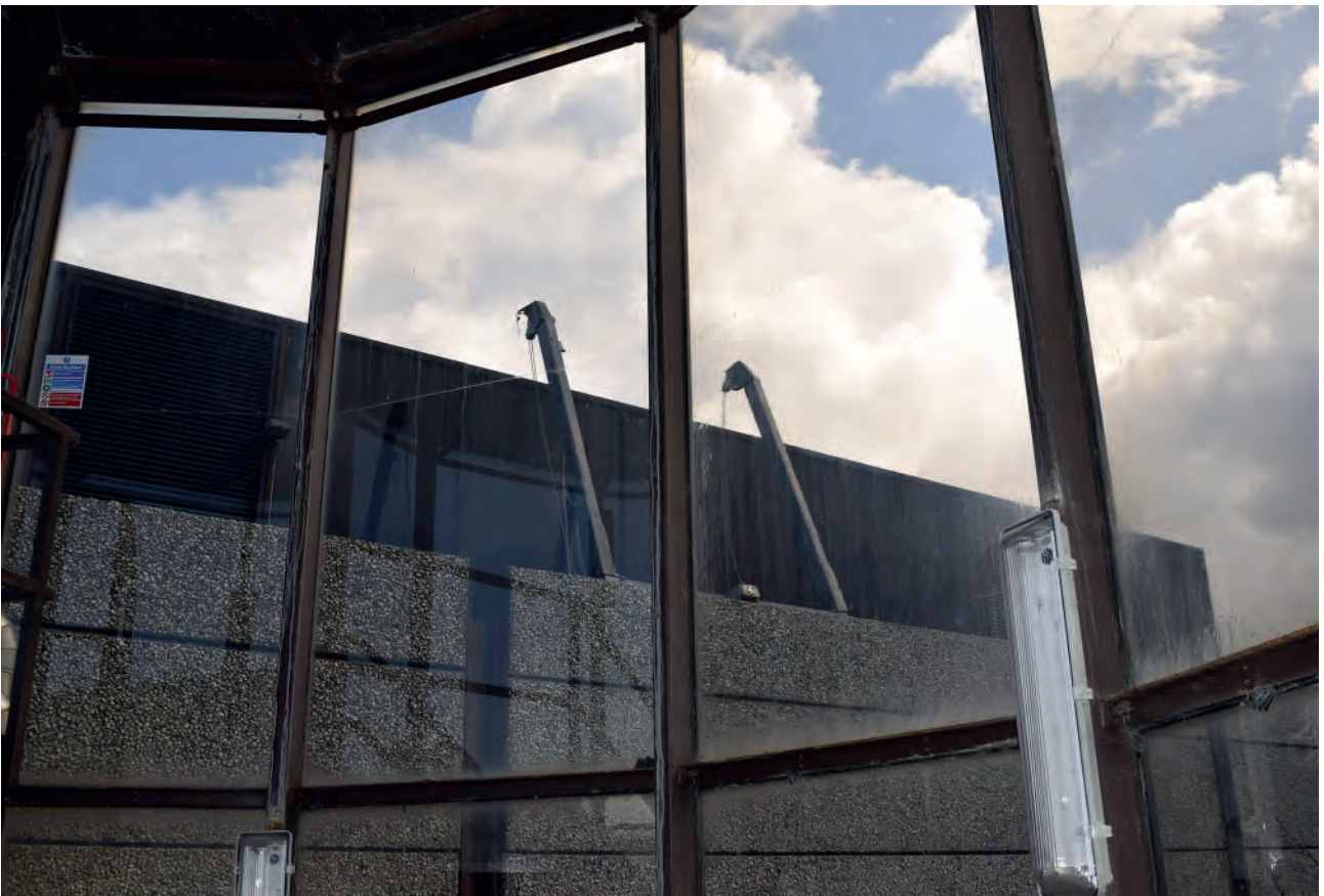
Plate 487: Roof, crane arms, looking south- east.
