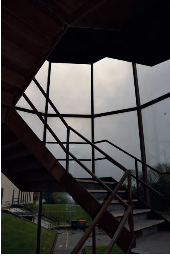
Plate 466 :First Floor, construction of stairs, looking east.
