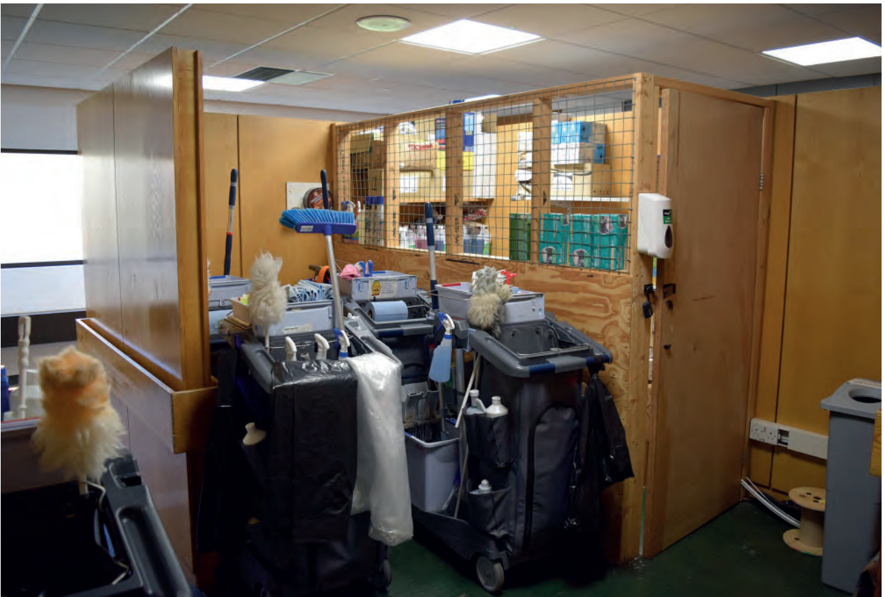
Plate 279: North part of Building 6000, north corridor, wooden structure converted into a utility room, looking north- east.
