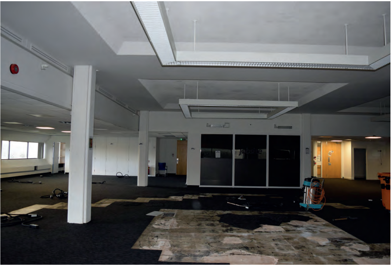
Plate 225: East wing of Building 6000, south office space, looking west.
