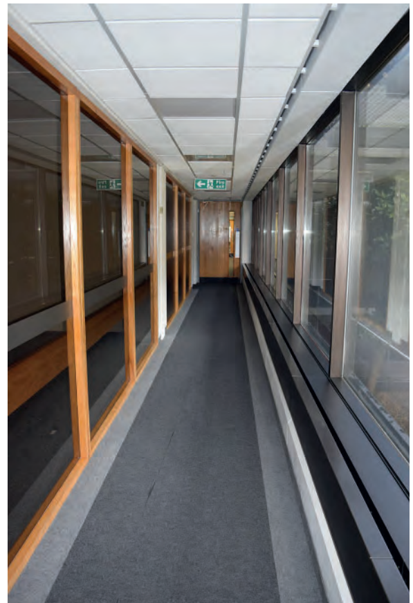
Plate 302: West wing of Building 6000, middle part of west corridor, looking north.
