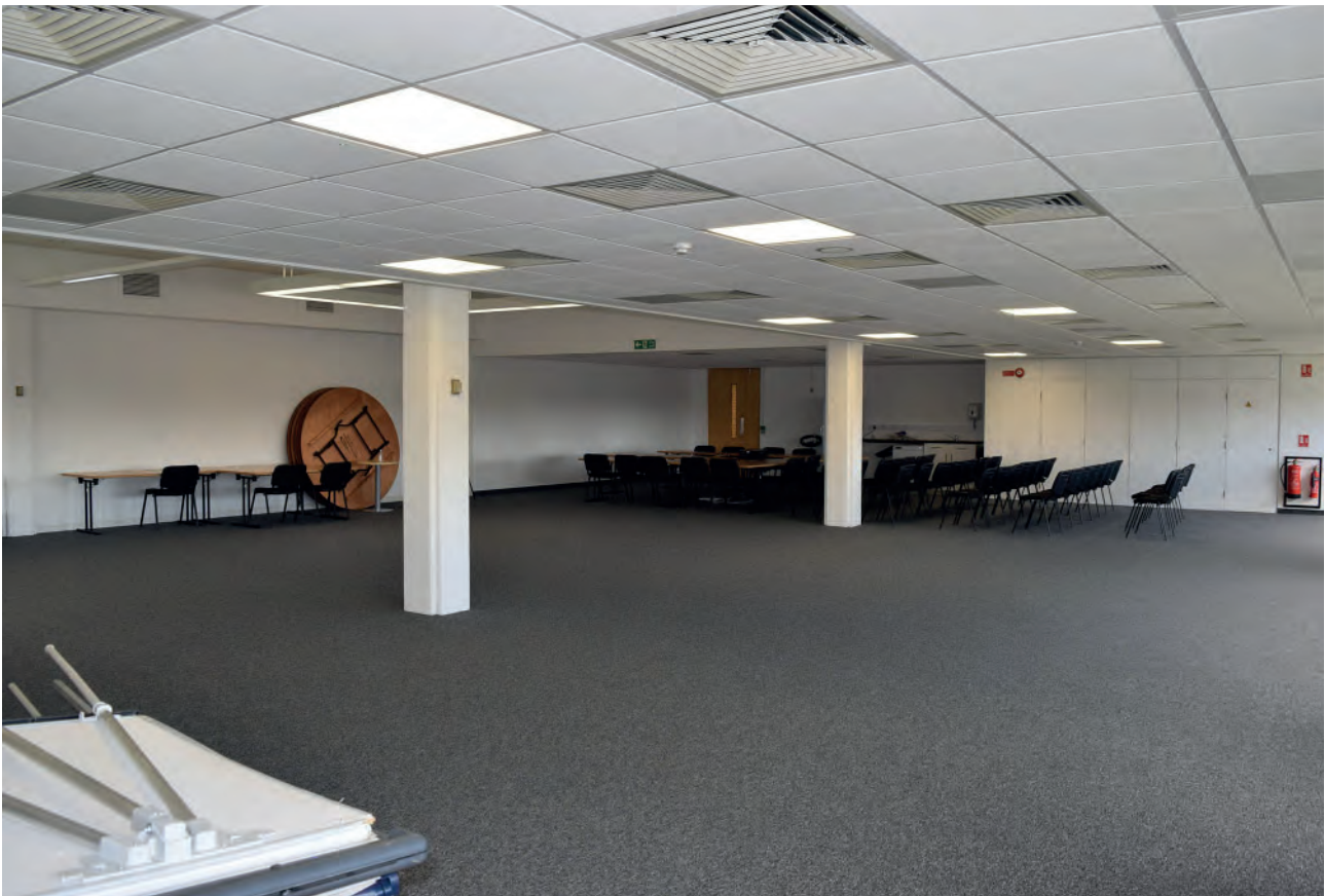
Plate 203: West wing of Building 6000, south office space, looking north- east.
