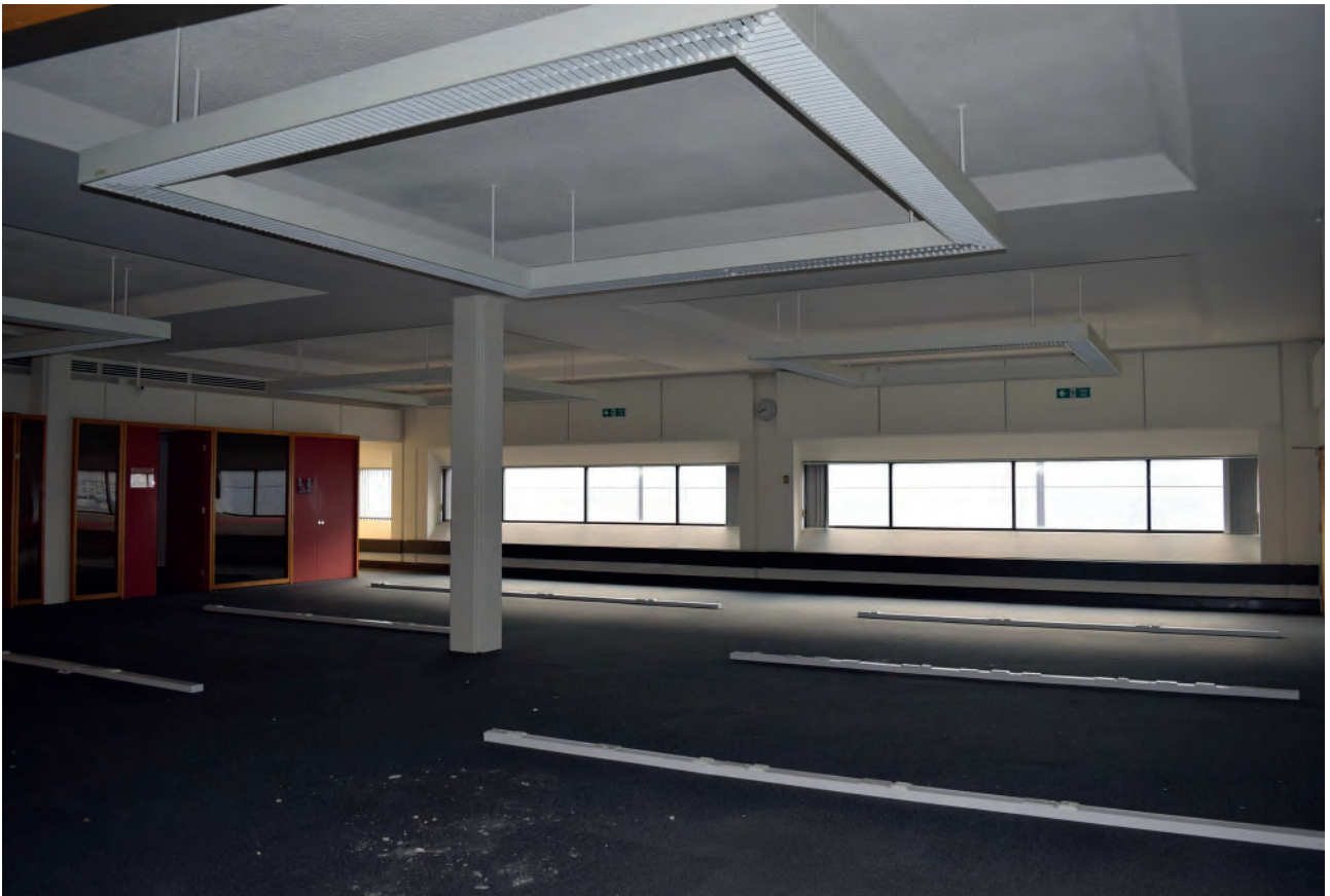
Plate 406: West wing of Building 6000, north office space, looking south- west.
