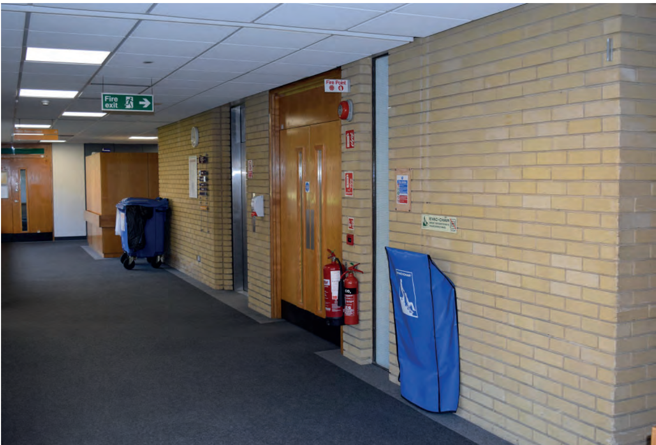
Plate 284: North part of Building 6000, north corridor, looking south- east.
