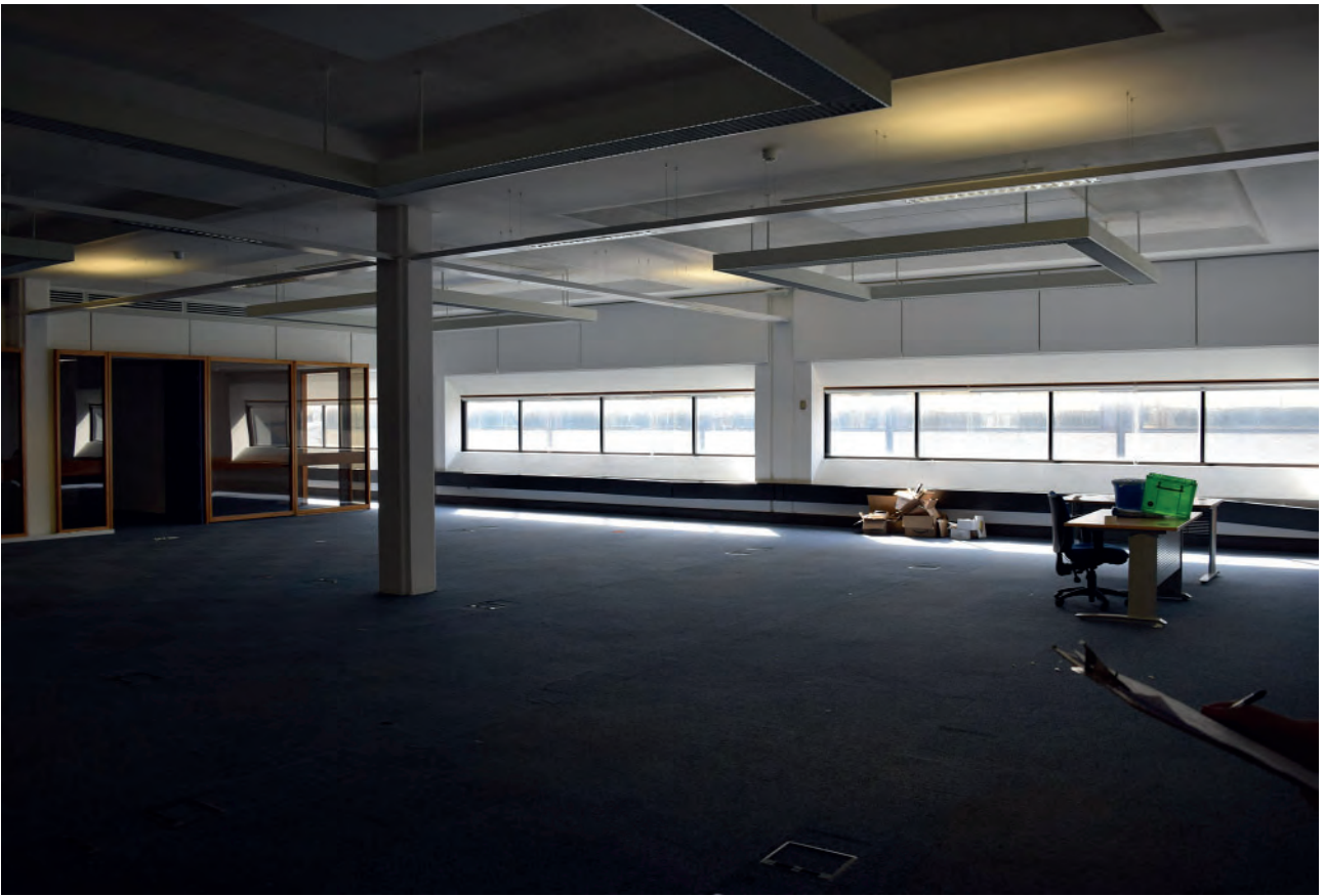
Plate 294: West wing of Building 6000, north office space, looking south- west.
