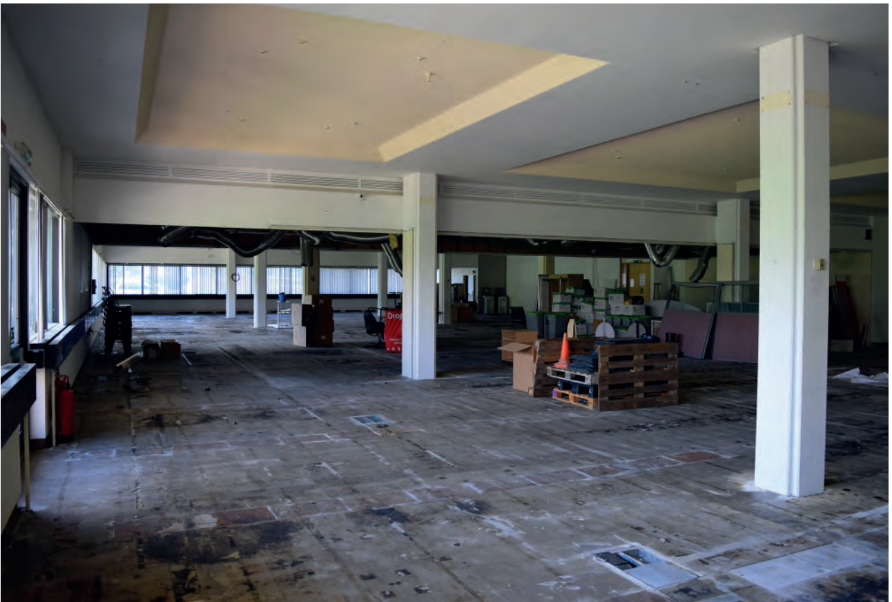
Plate 103: East wing of Building 6000, middle office space, looking south- west.
