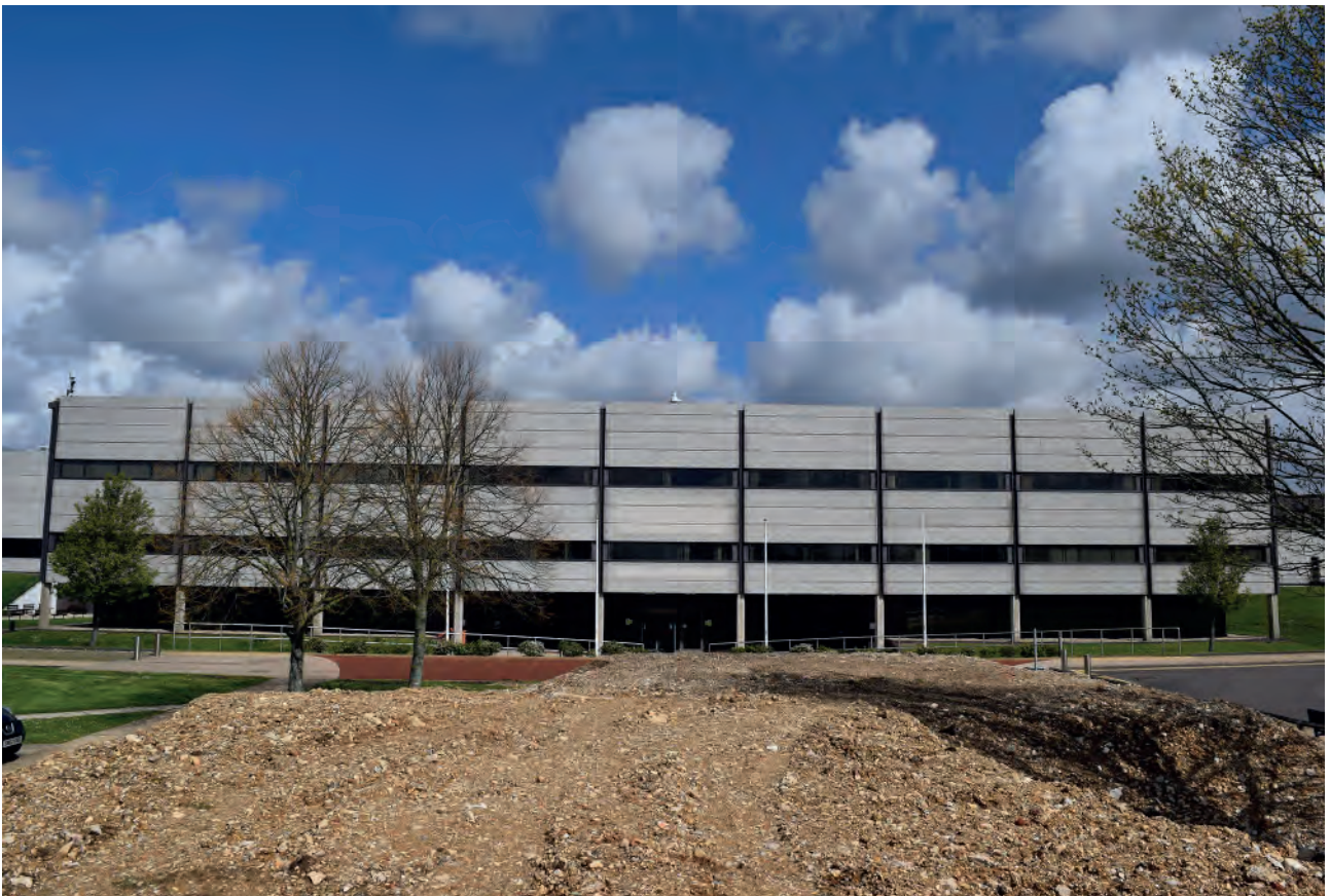
Plate 30: South façade of Building 6000, looking north.
