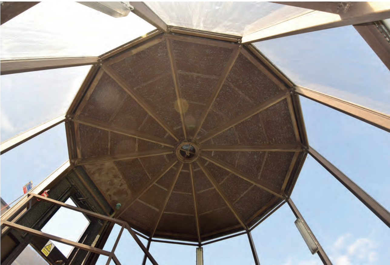
Plate 475: Construction of staircase ceiling.
