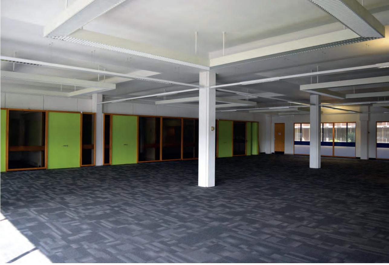
Plate 315: West wing of Building 6000, middle office space, looking north-east.
