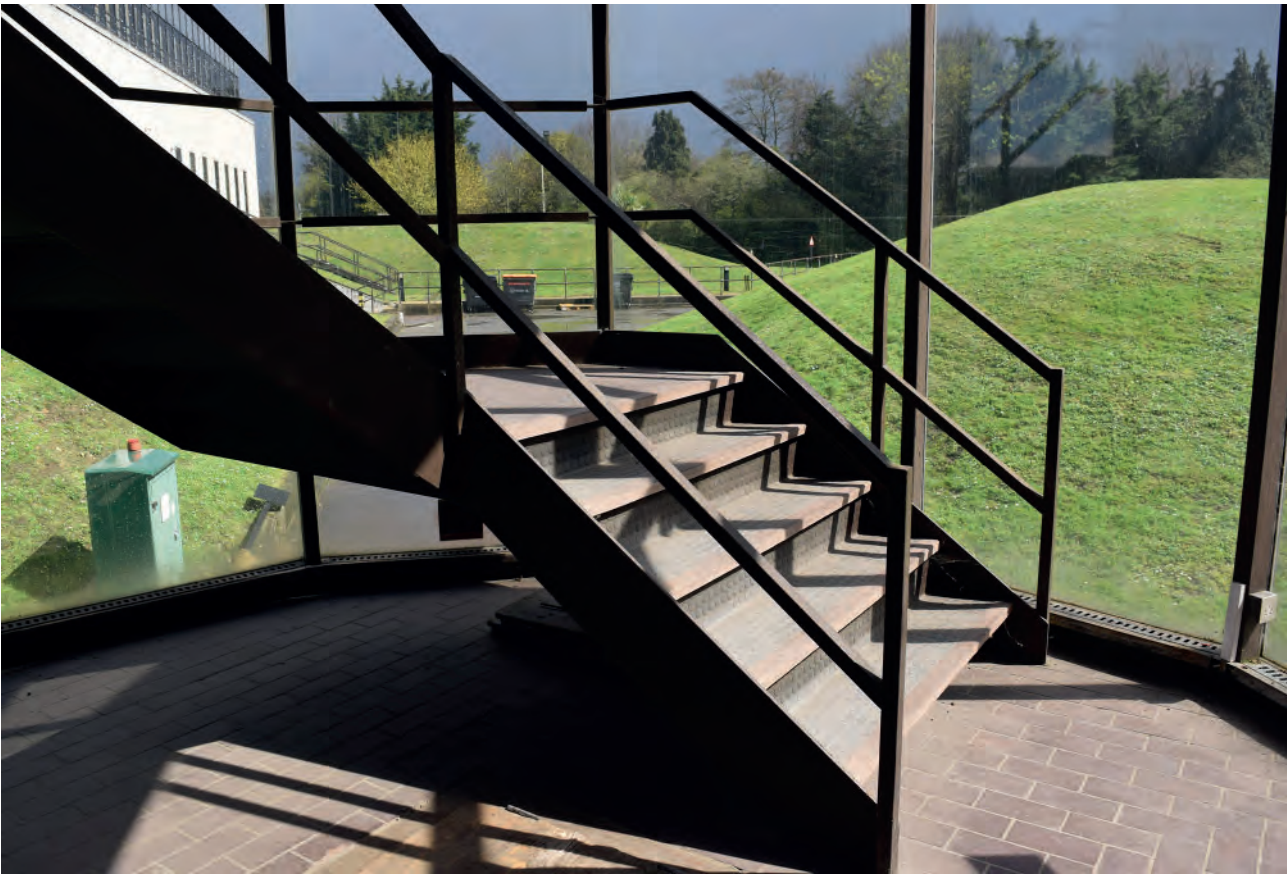
Plate 459: Construction of stairs, looking east.
