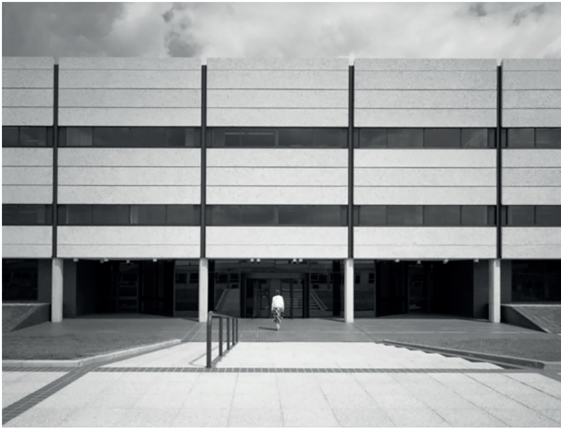
Plate 1: Main entrance to Building 6000, looking north, 1980.
