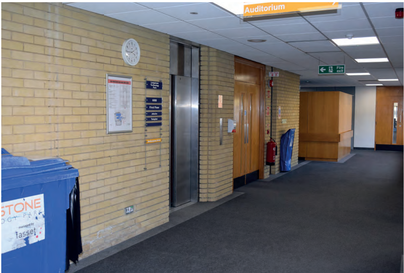
Plate 283: North part of Building 6000, north corridor, looking south- west.
