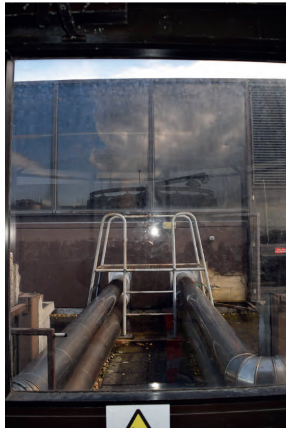
Plate 489: Roof, looking east.
