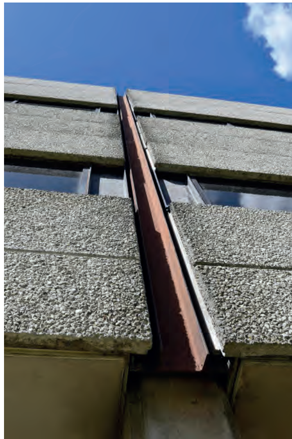
Plate 44: Example of steel channel beam, east elevation, looking west.
