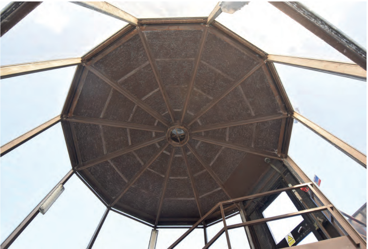
Plate 496: Construction of staircase ceiling.
