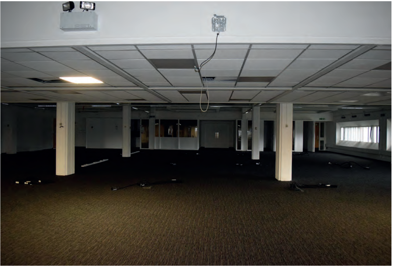
Plate 229: East wing of Building 6000, middle office space, looking north.
