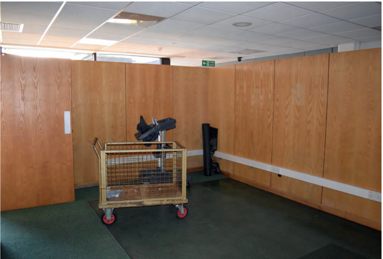
Plate 338: South part of Building 6000, south corridor, wooden structure, looking north- east.
