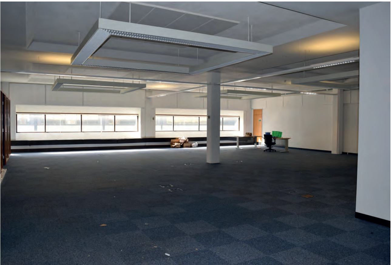
Plate 289: West wing of Building 6000, north office space, looking north- west.
