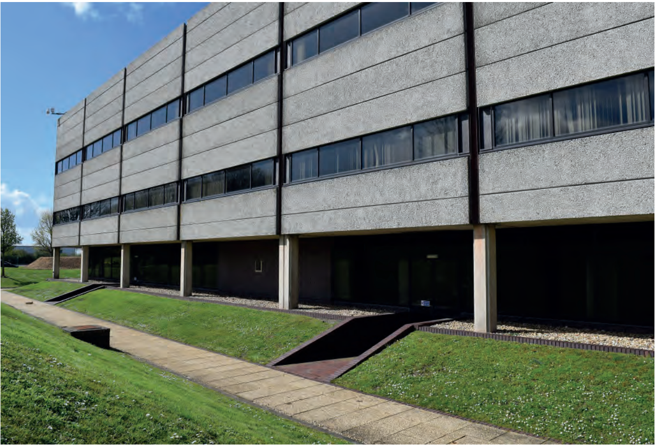
Plate 39: East elevation of Building 6000, looking south- west.
