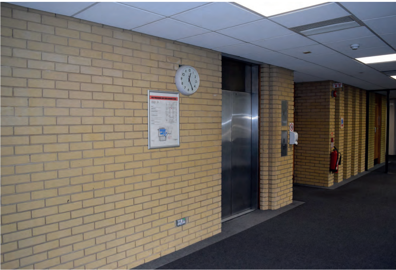
Plate 83: South part of Building 6000, south corridor, looking south- west.
