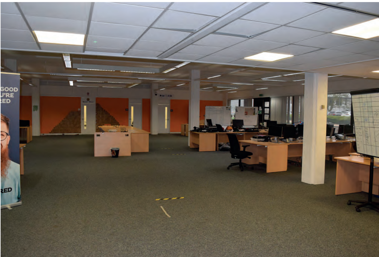
Plate 184: West wing of Building 6000, middle office space, looking north- west.
