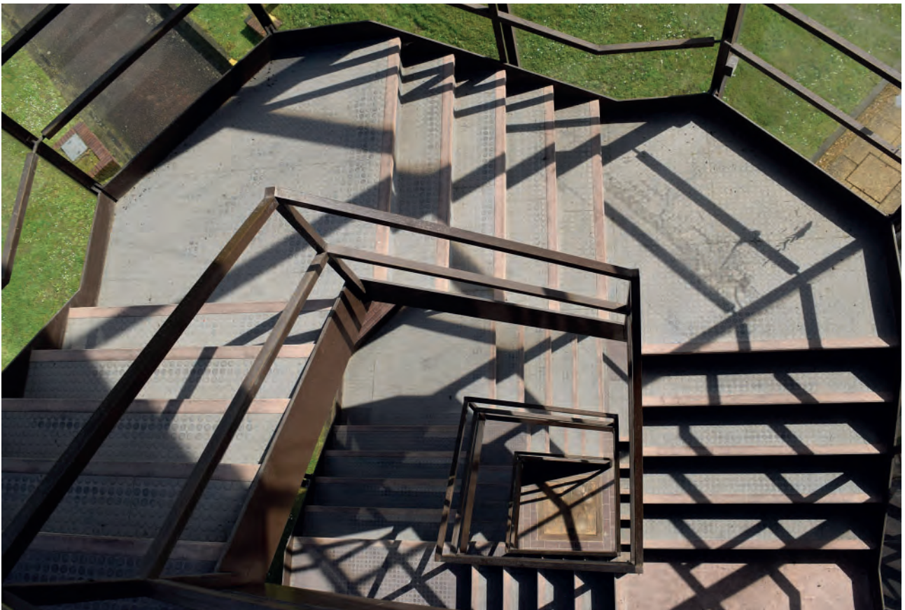
Plate 469: Construction of stairs, ground floor view.
