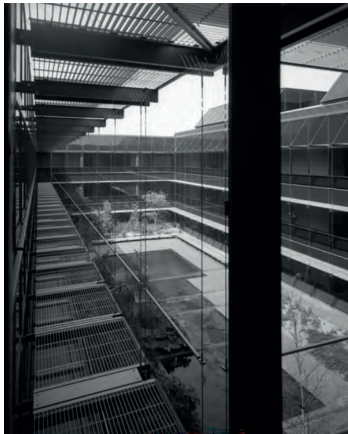
Plate 29: Second Floor, courtyard, looking north- east, 1980.
