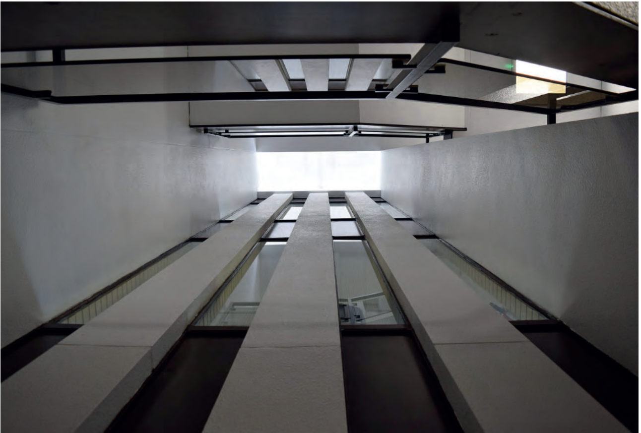
Plate 168: South part of Building 6000, staircase skylight.
