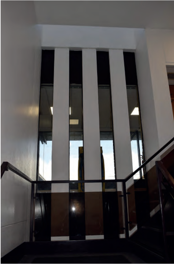
Plate 327: South part of Building 6000, staircase glazing, looking north.
