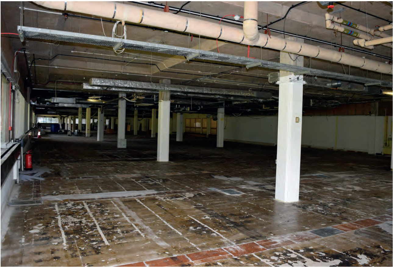
Plate 108: East wing of Building 6000, north office space, looking south- west.
