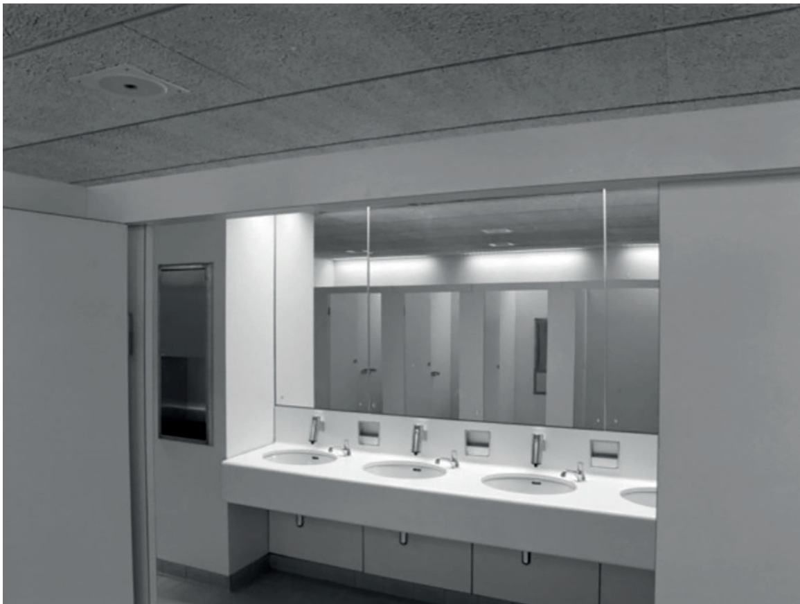
Plate 18: Ground Floor, south part of Building 6000, men's toilet, looking north- west, 1980.
