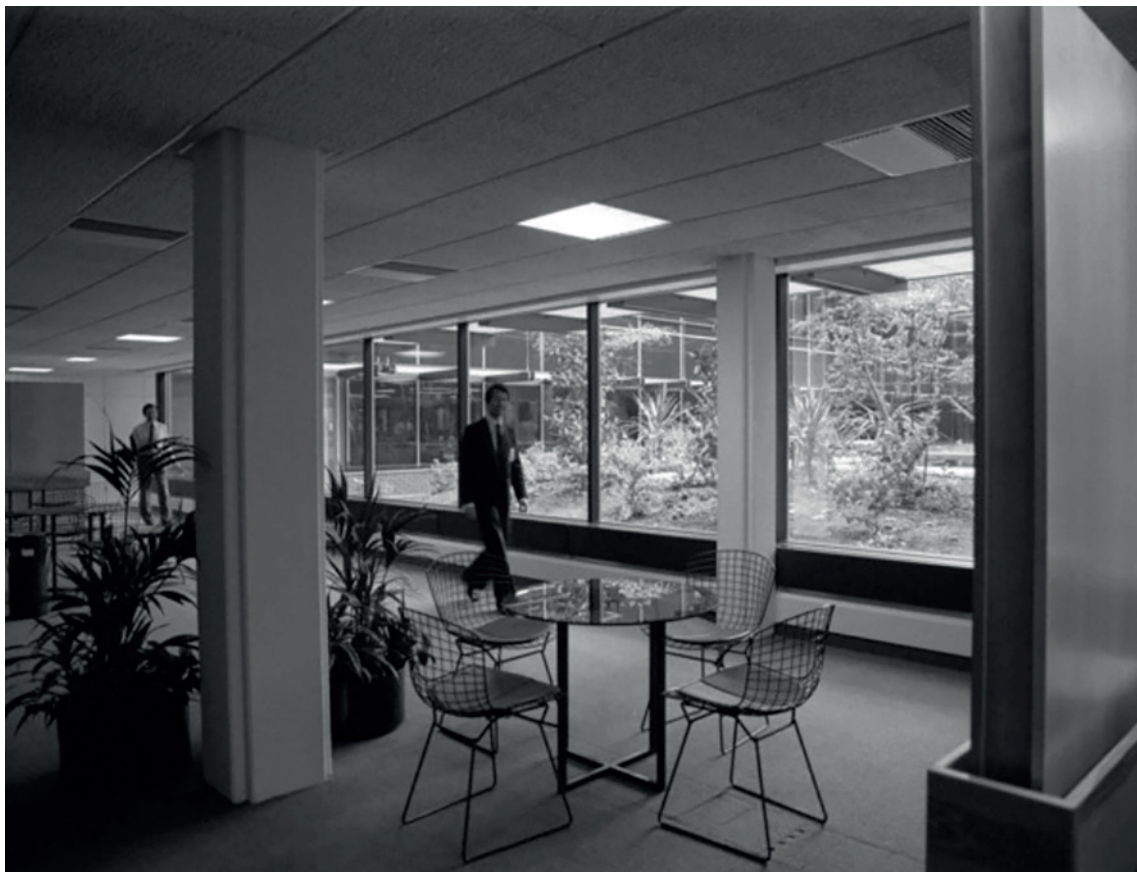
Plate 13: Ground Floor, east corridor, looking south- west, 1980.
