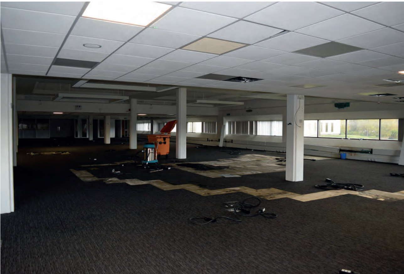
Plate 220: East wing of Building 6000, south office space, looking north- east.
