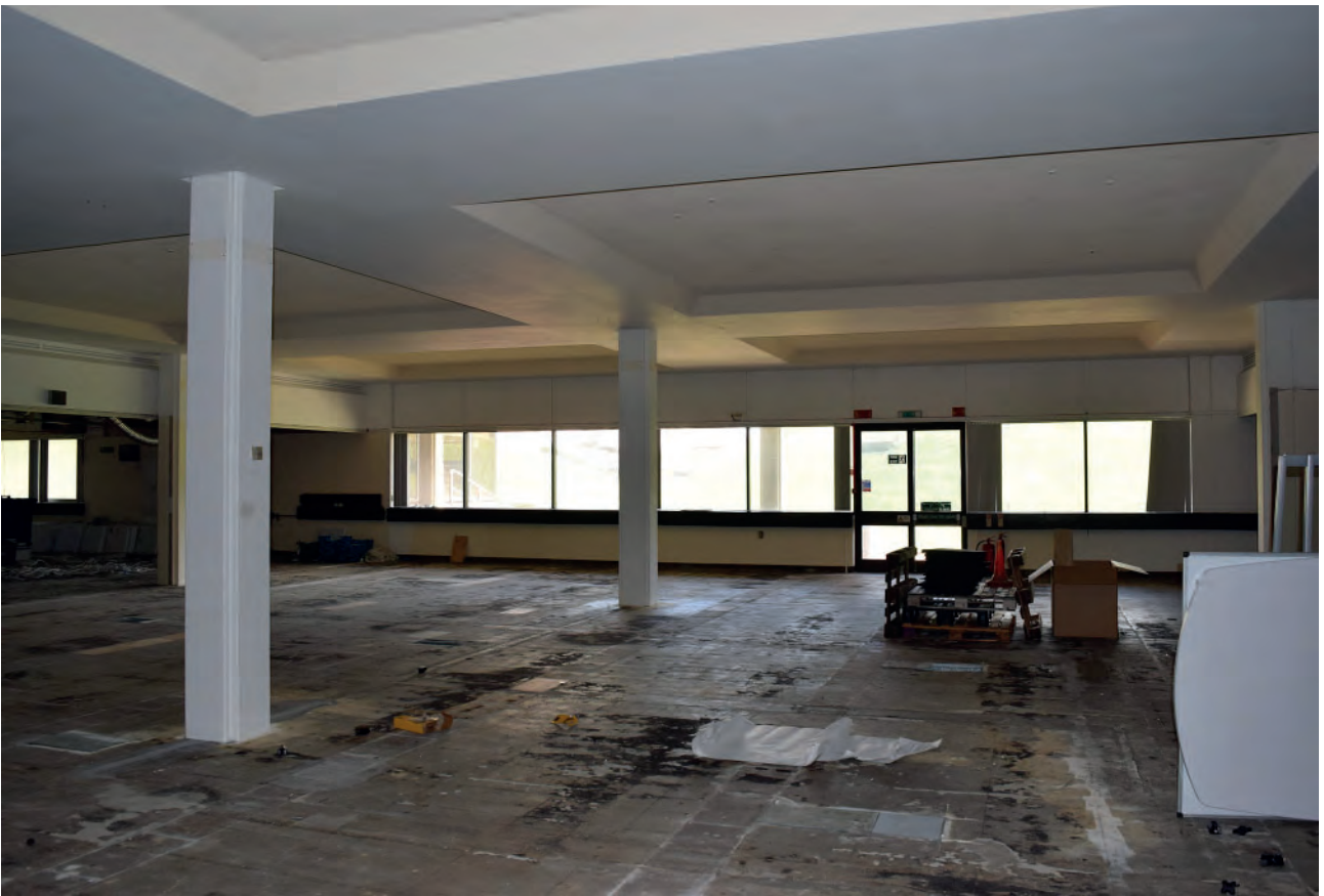
Plate 99: East wing of Building 6000, middle office space, looking east.
