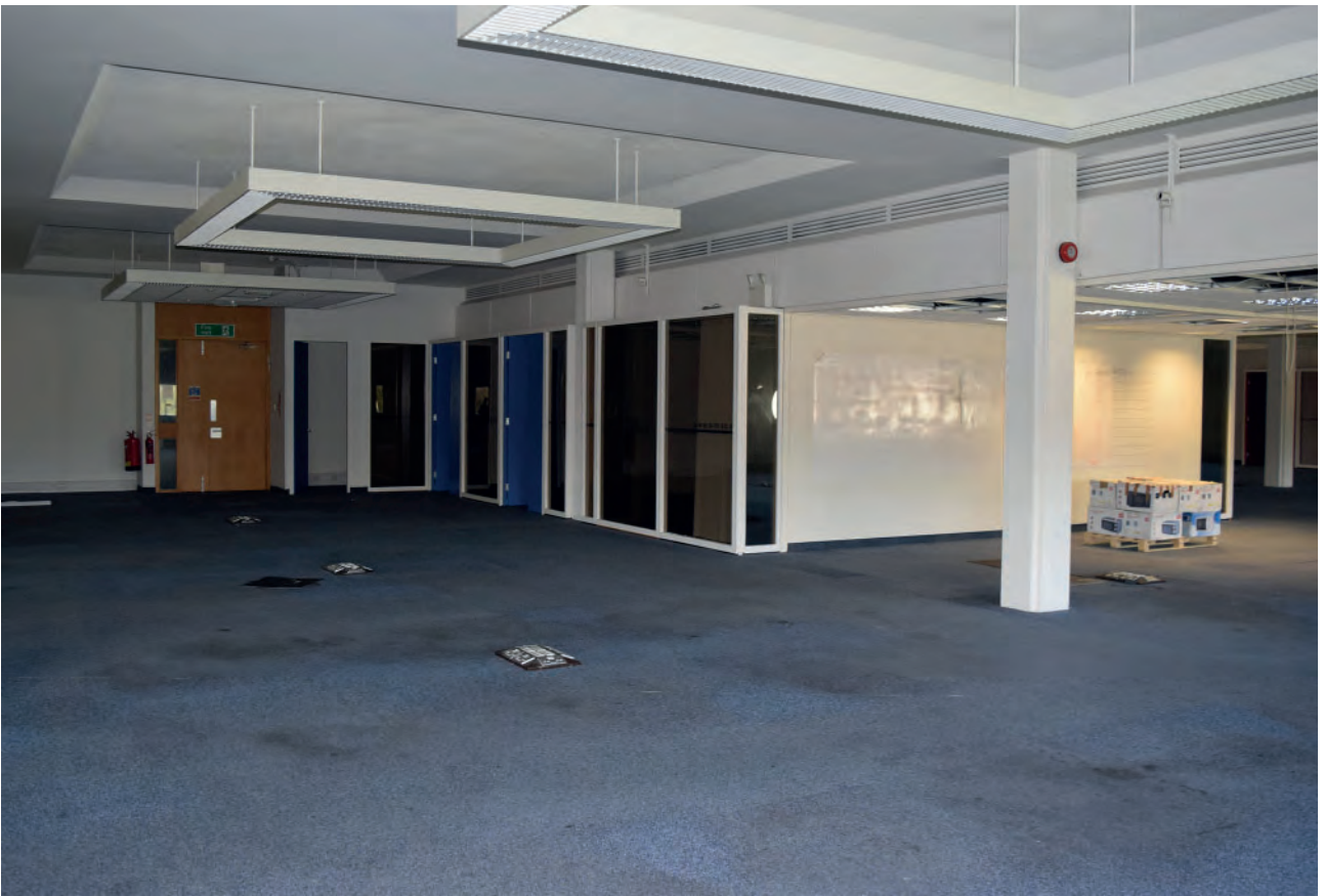
Plate 354: East wing of Building 6000, south office space, looking north- west.
