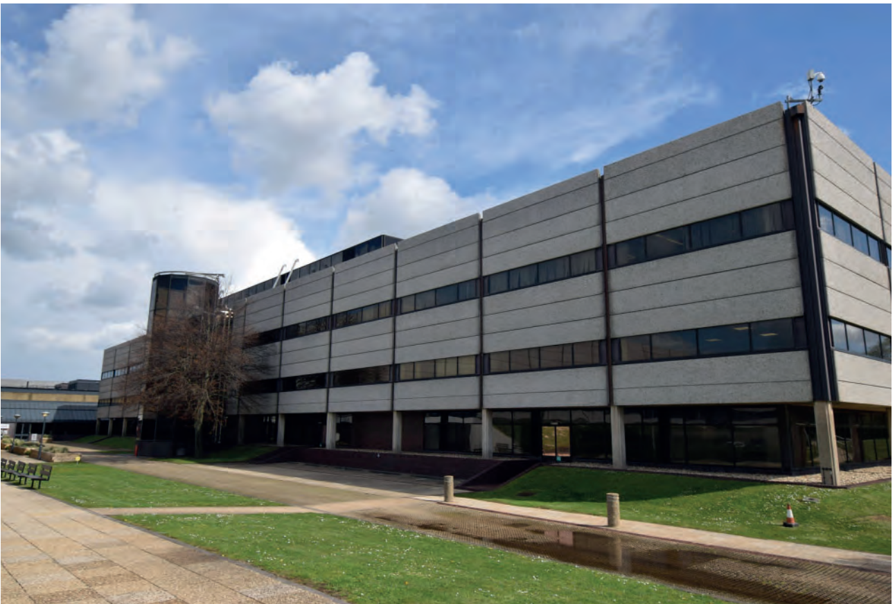
Plate 58: West elevation of Building 6000, looking north-east.
