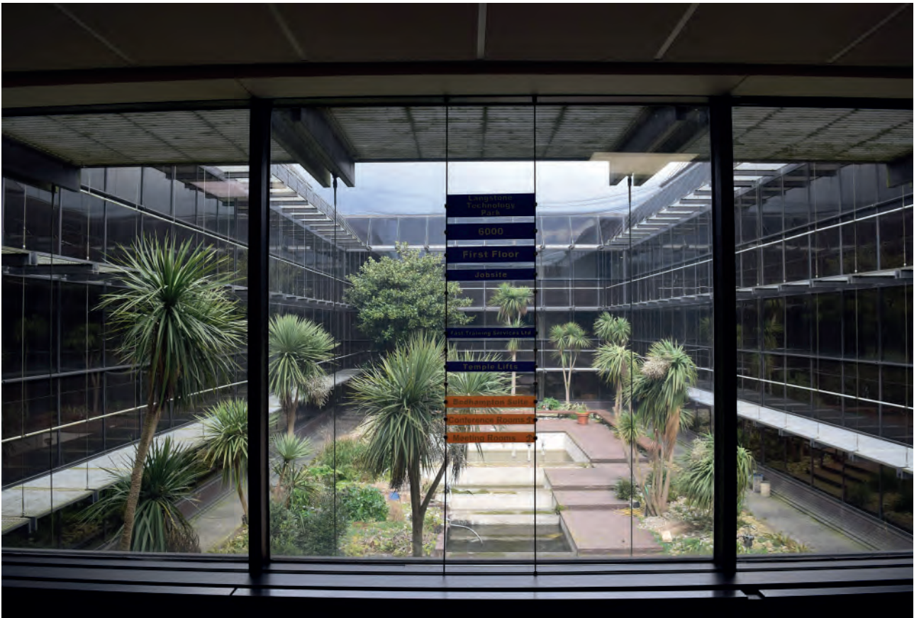
Plate 192: South part of Building 6000, courtyard, looking north.
