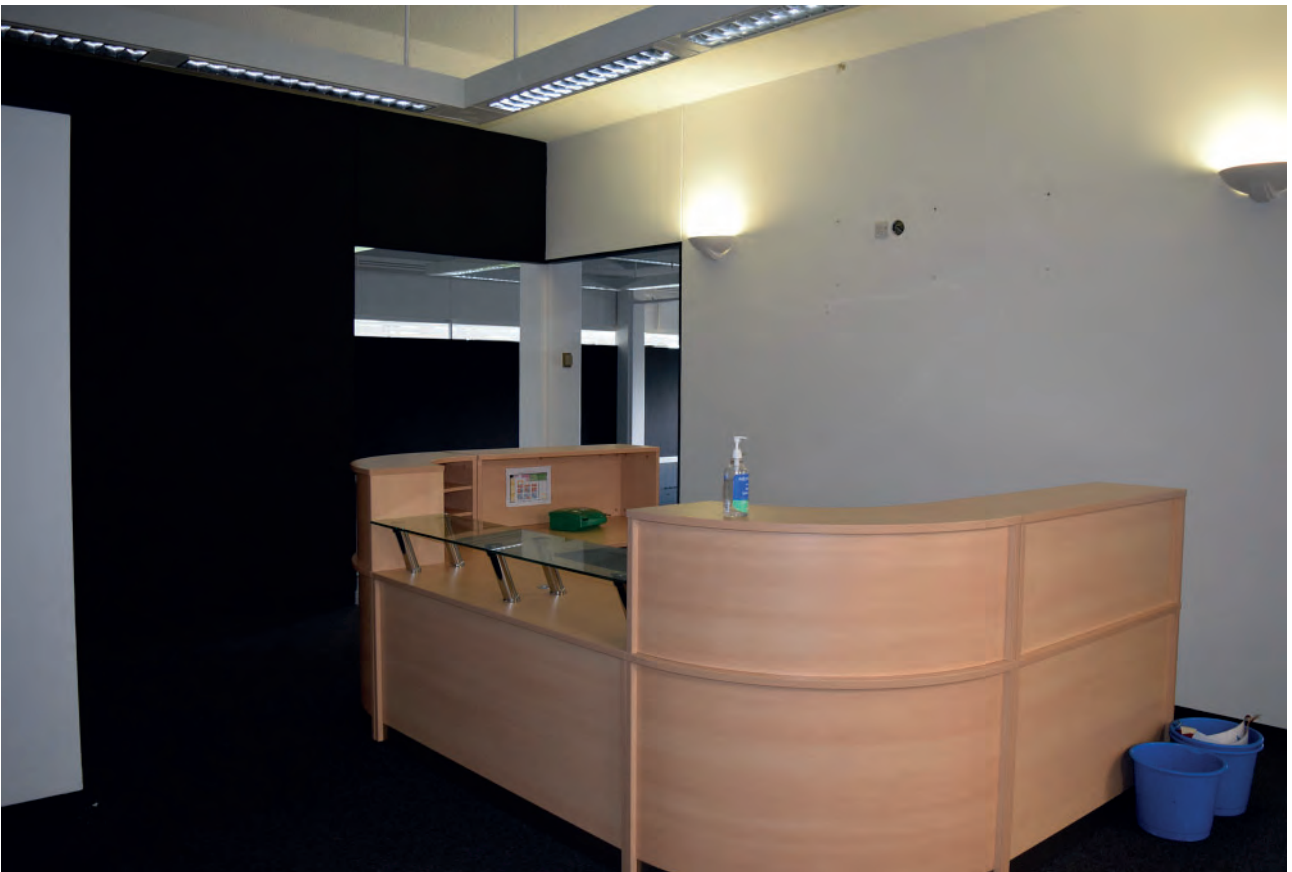
Plate 115: West wing of Building 6000, south office space, office reception, looking south-east.
