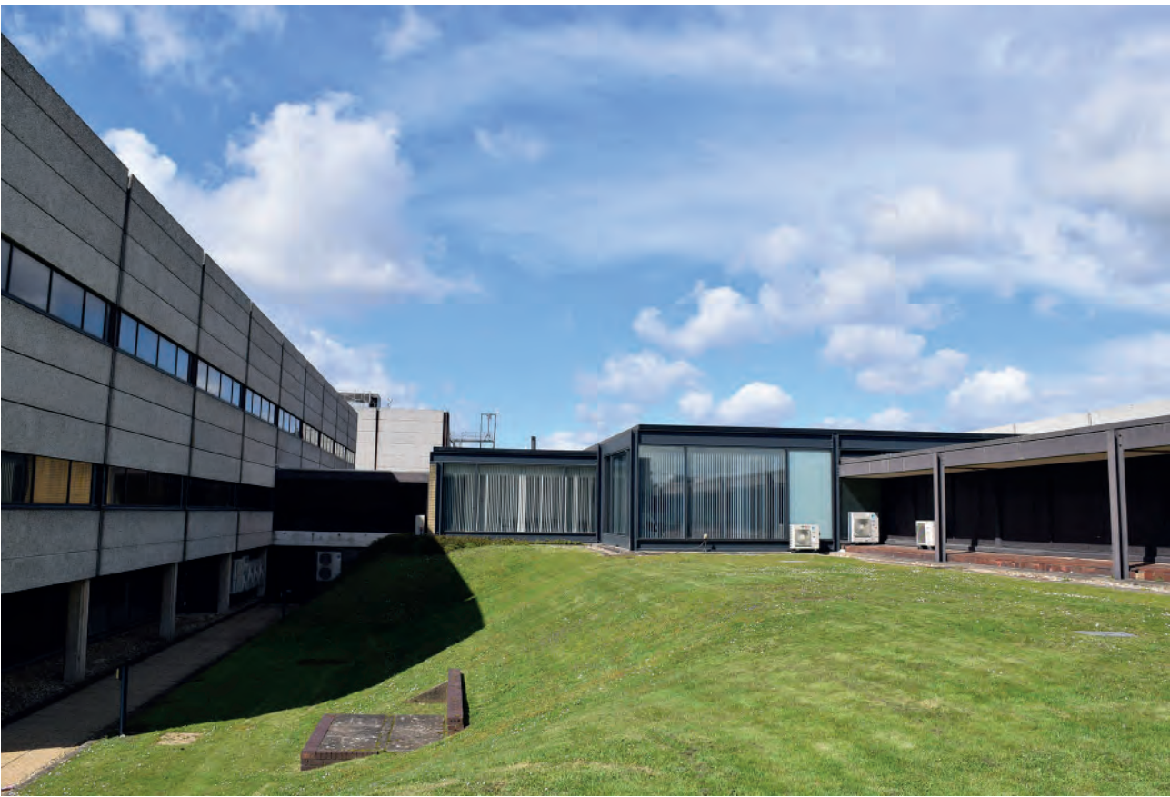
Plate 49: Connection between Buildings 6000 and 4000, looking west.
