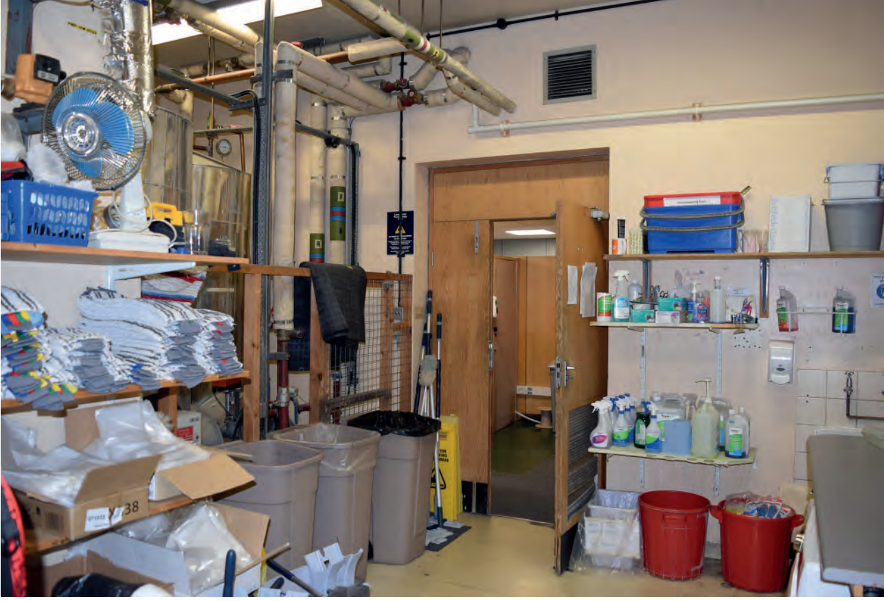
Plate 281: North part of Building 6000, north corridor, utility room, looking north- east.
