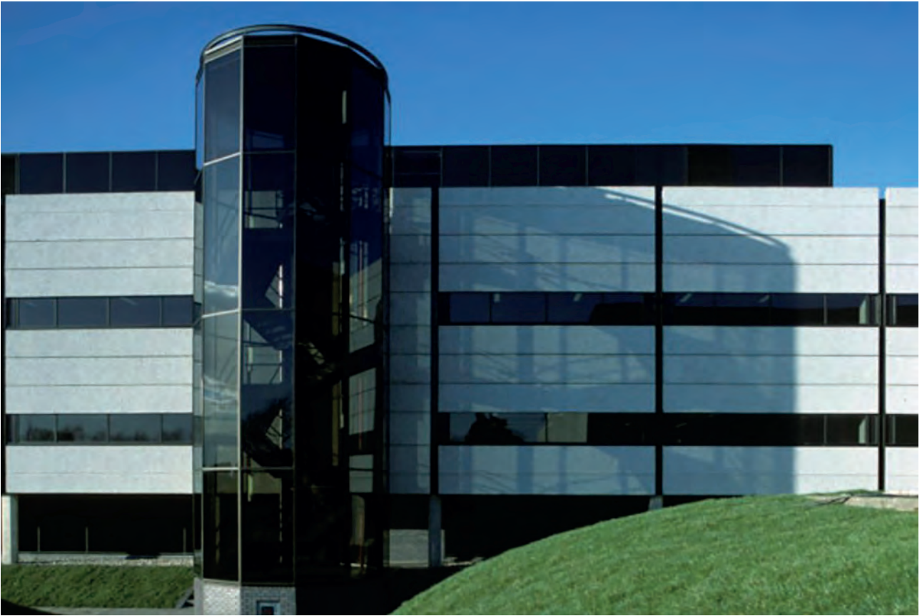
Plate 7: East staircase tower, looking west, 1979.
