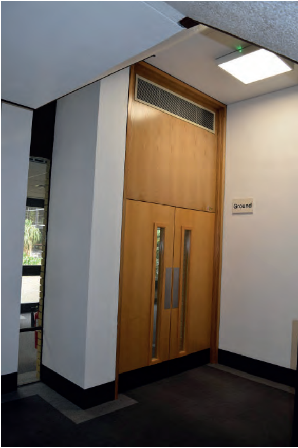
Plate 169: South part of Building 6000, staircase, looking north- west.
