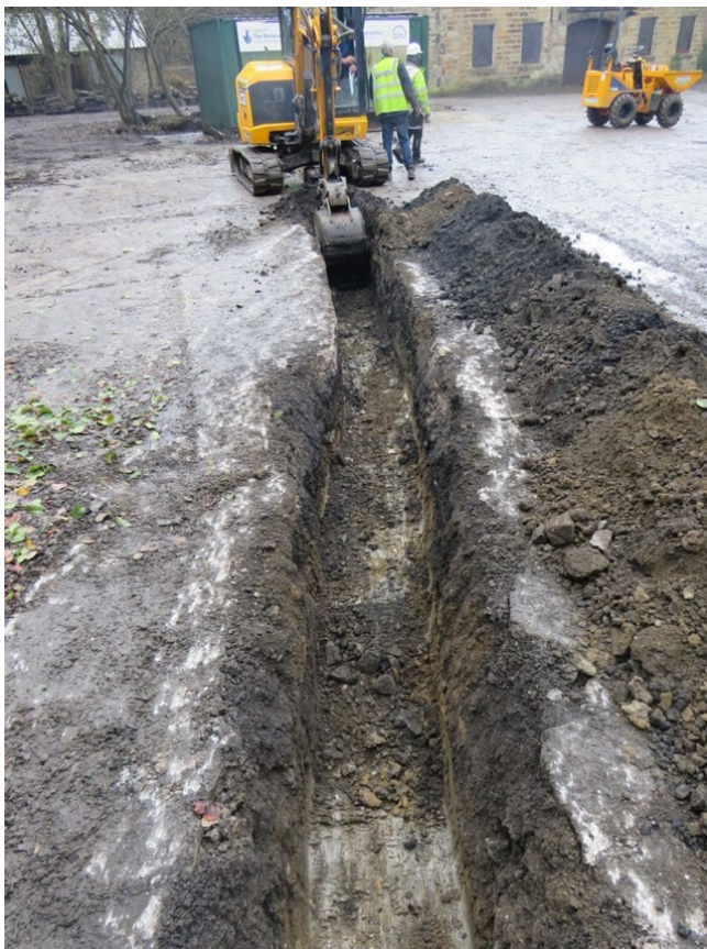
Plate 16. Excavation of a service trench from the site entrance towards Buildings 7-9.
