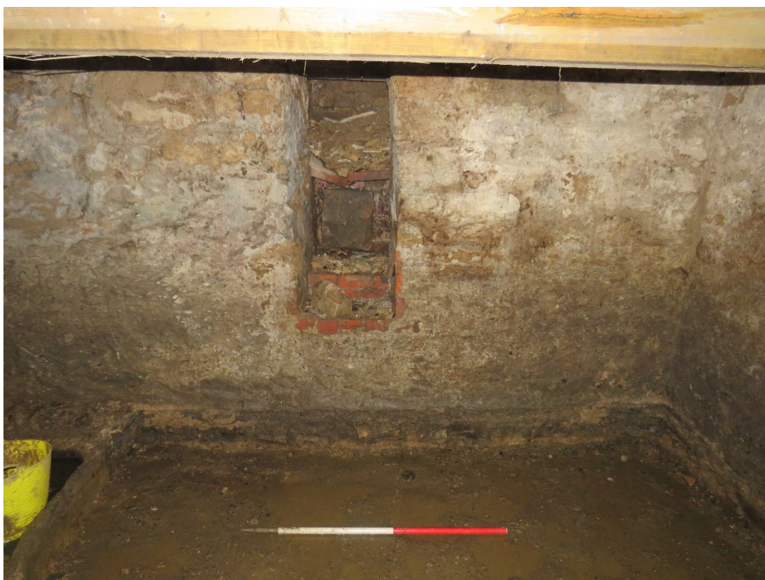
Plate 1. West facing cellar wall showing ground reduction within Building 1
