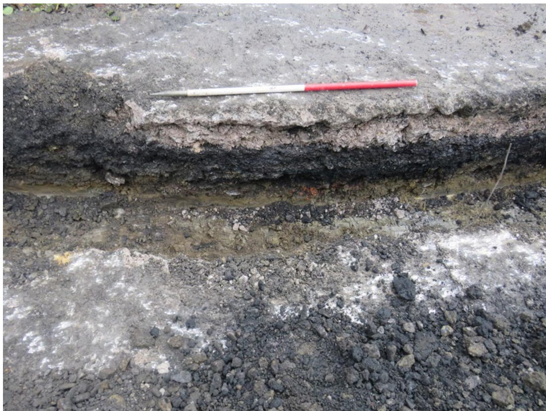
Plate 17. West facing section of the north-south aligned service trench, showing composition of modern surface deposits.
