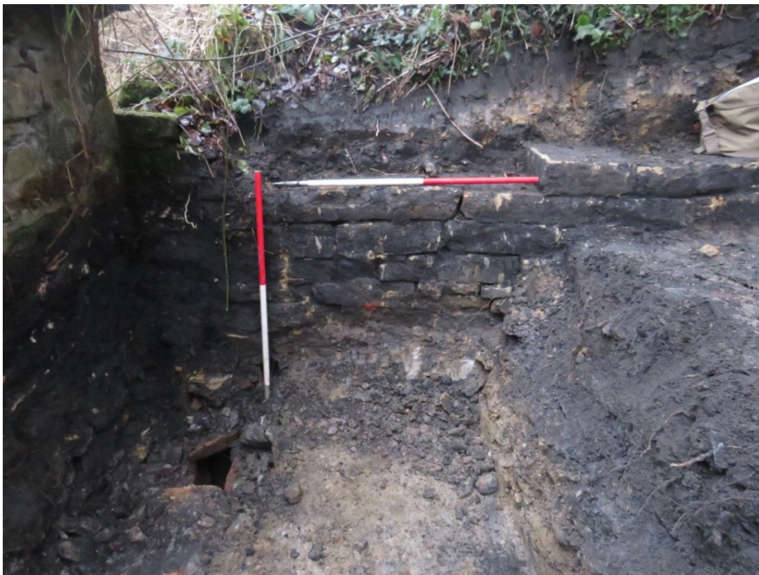
Plate 12. Retaining wall 201 to rear of the forge, and culvert 202 partially exposed
