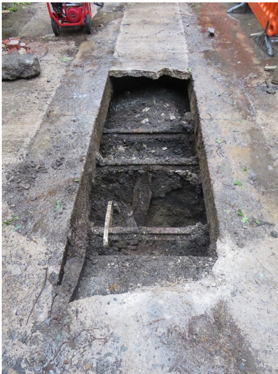
Plate 3. The potential saw pit within Building 9. Viewed facing north post excavation.
