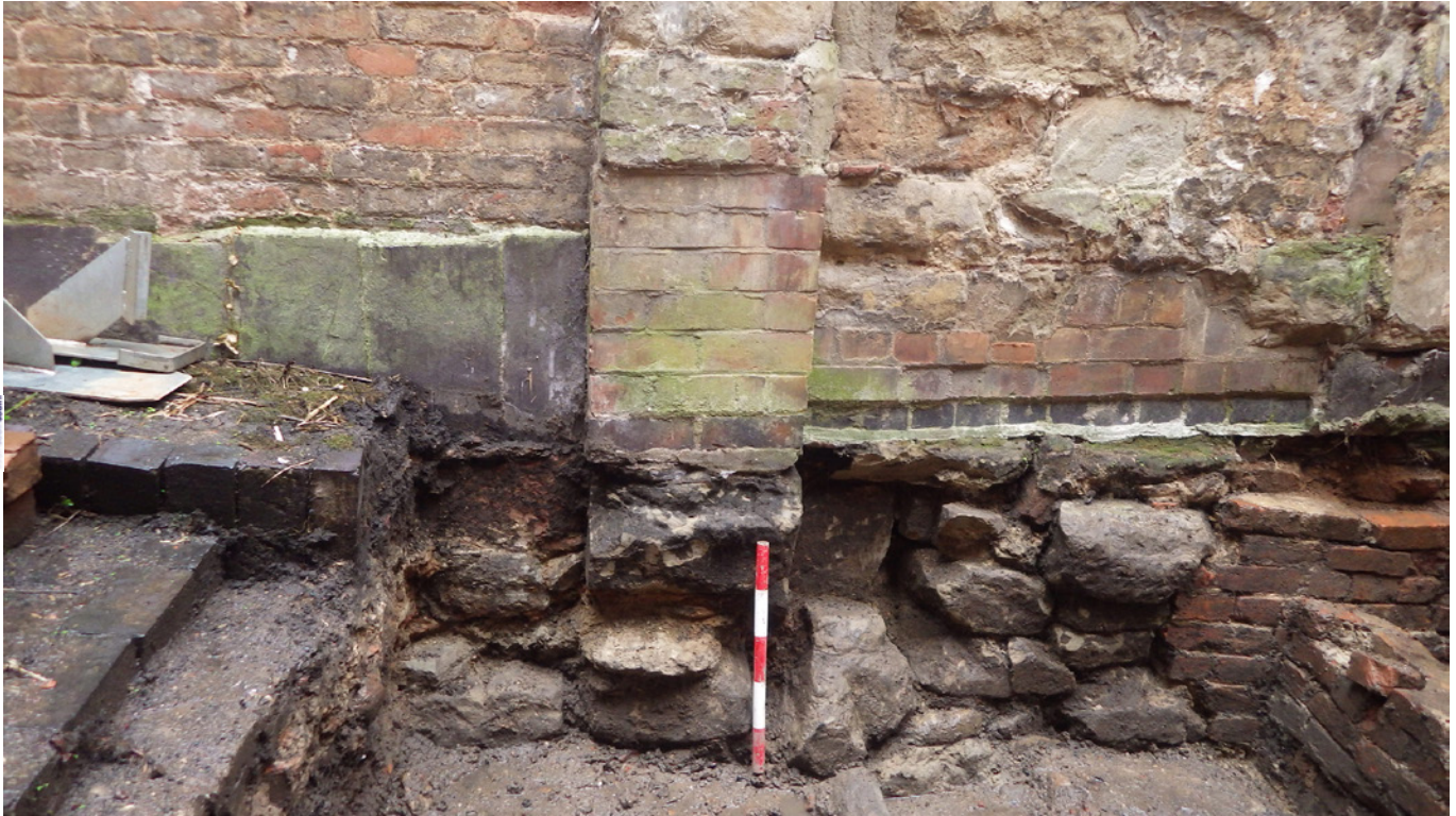
Plate 1: Sandstone wall/foundation 5 with wall 11 above , looking west
