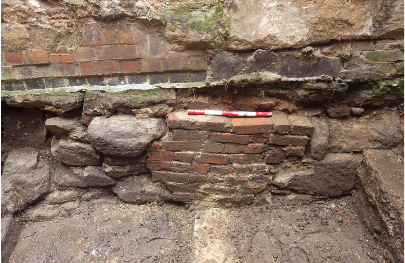
Plate 4: Brick infill 12 in sandstone wall/foundations 5 after removal of wall 6, looking west
