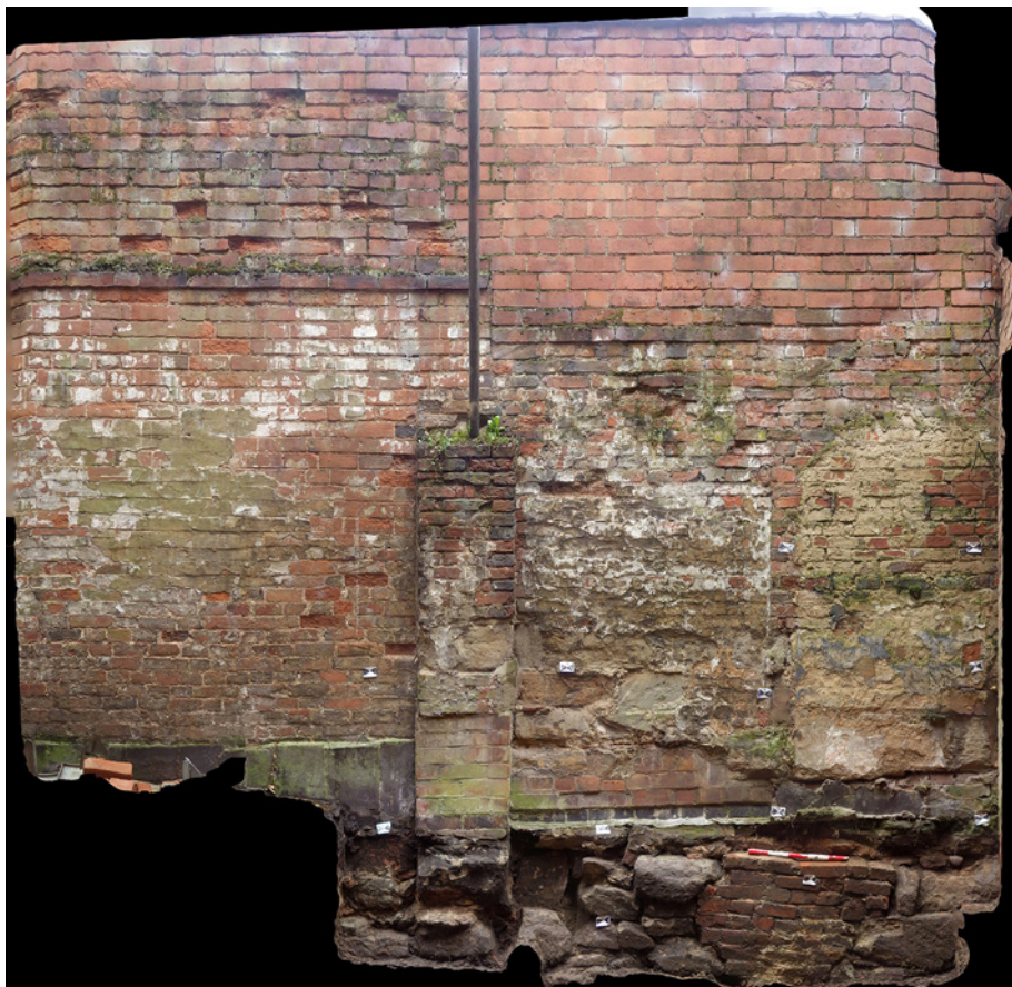
Plate 8: Walls 5, 9, 12 and 11 showing scar of lean-to and multiple phasing on wall 11
