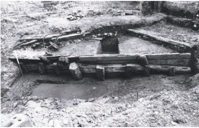
Plate 13 Timber revetment at Rainham Creek
