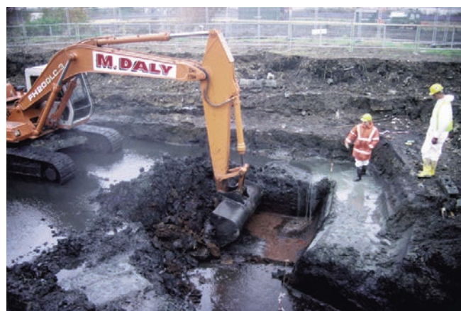
Plate 10 Excavations at the Goresbrook diversion
