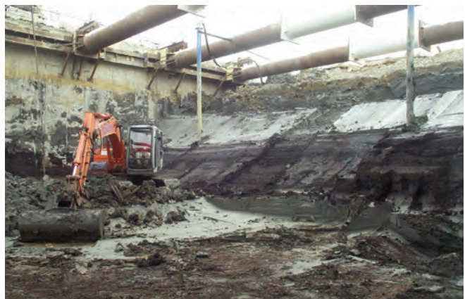
Plate 8 Peat and clay-silt within alluvium, HSI Swanscombe
