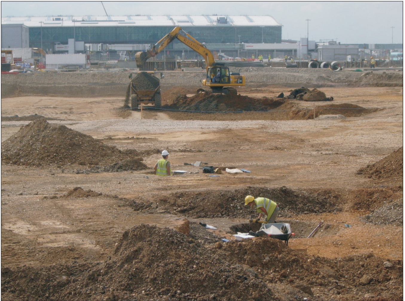
Plate 1.3: Working shot of excavations at Terminal 5
