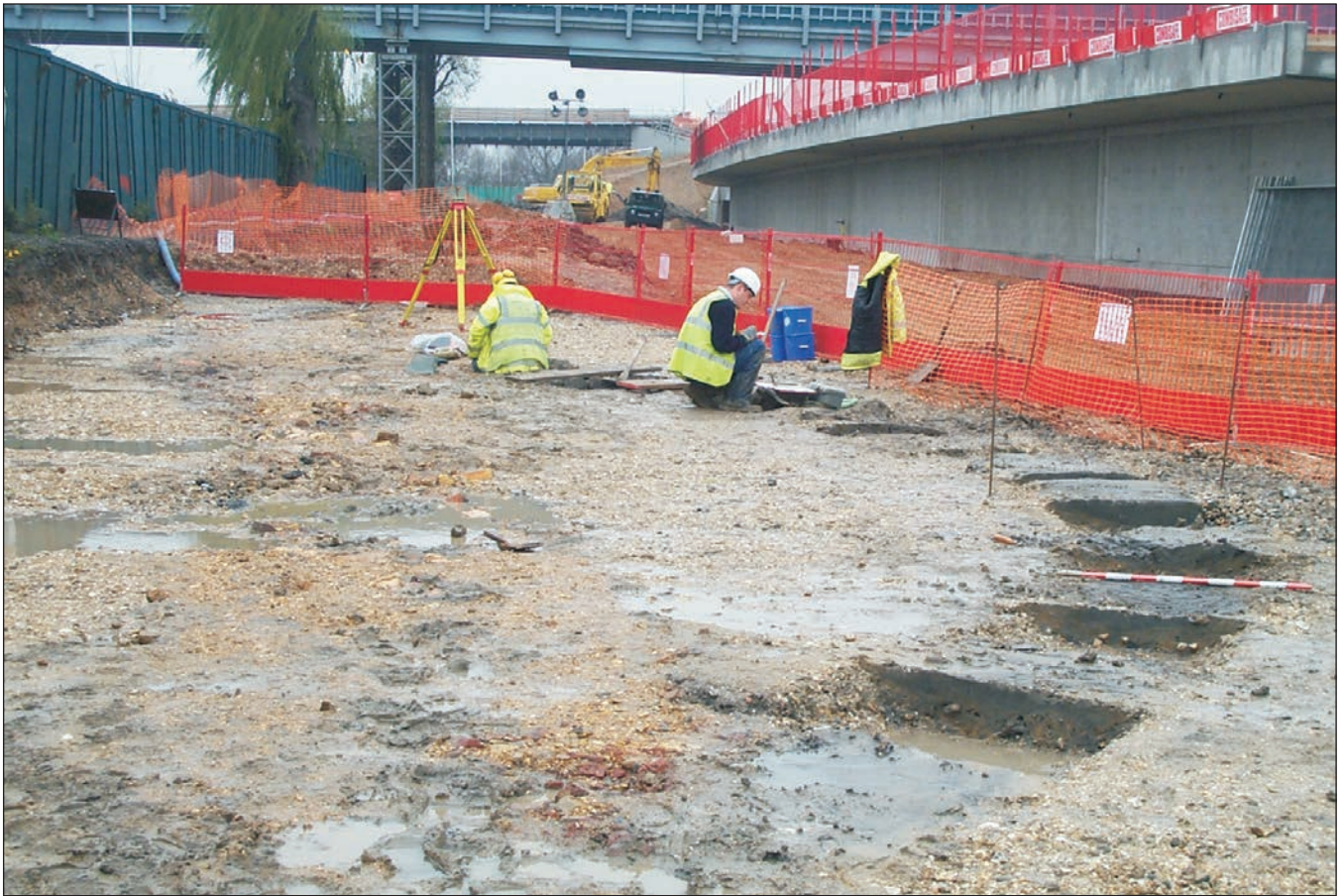
Plate 2.34: HE3 enclosure under excavation
