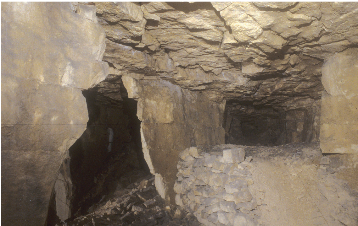
Fig. 2.7 Sailed pillars – the result of a fault running through north Firs
