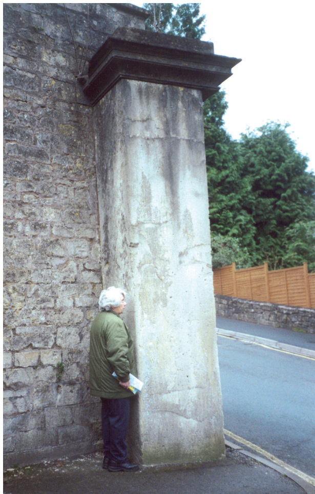
Fig. 2.5 One of the two Priory Close gateposts, nominally 3.7 m (above ground) x 0.9 m sq. The pair are the largest extant blocks of Combe Down freestone
