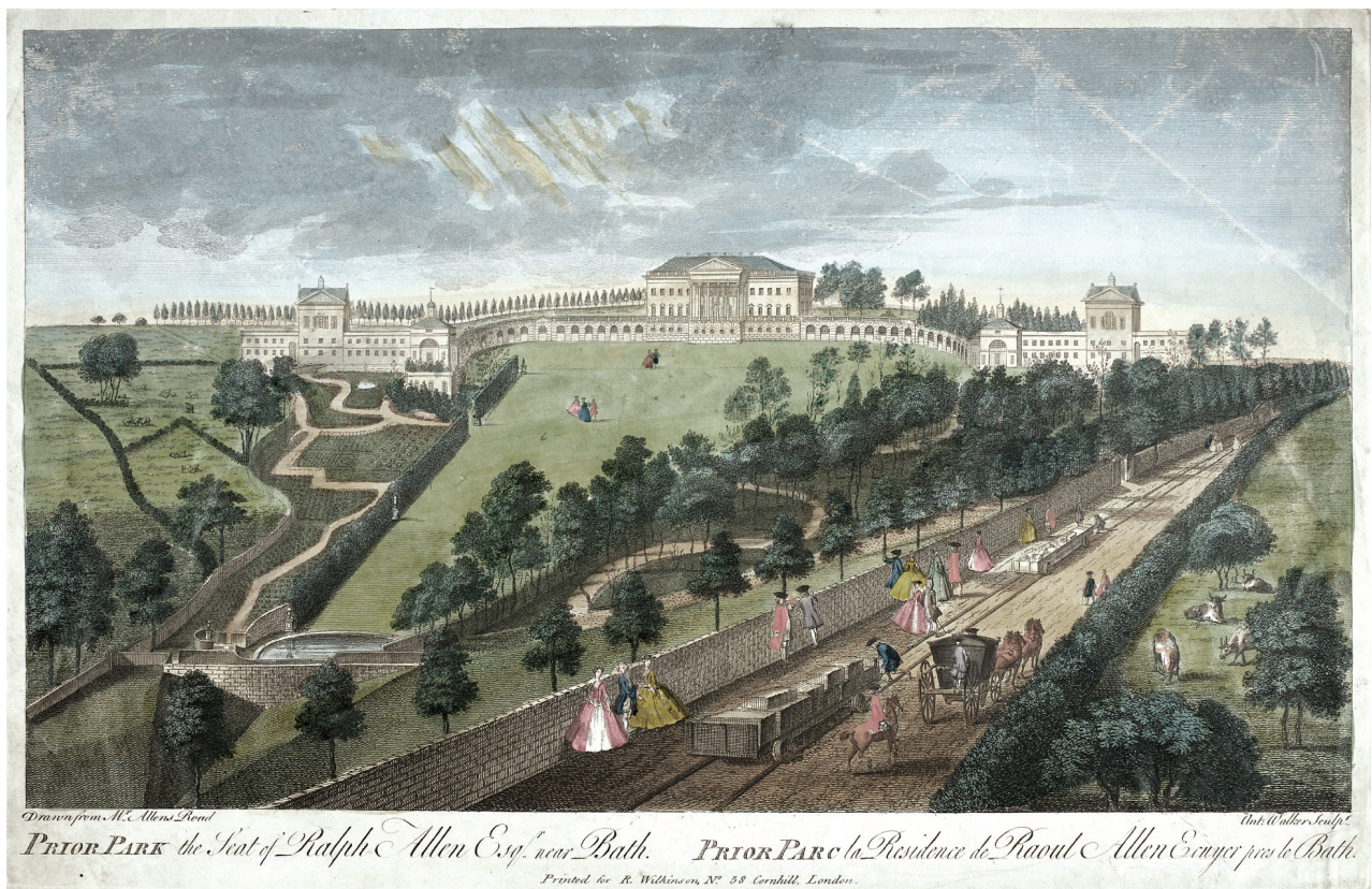
Fig. 3.6 Allen's wooden railway, at the lower end of Prior Park about 1750. The nearer carriage contains block stone, the other seems to contain walling stone. From an engraving by Anthony Walker Prior Park: The Seat of Ralph Allen (courtesy of The Building of Bath Museum)
