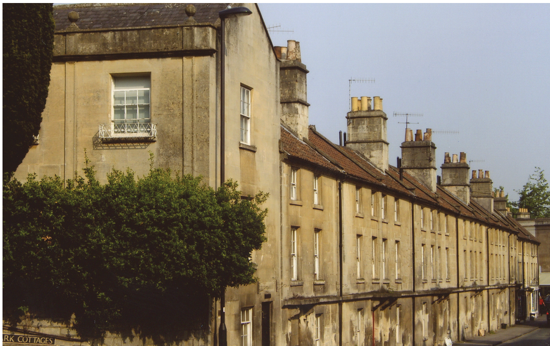
Fig. 3.9 The cottages built for the stoneyard workers at Dolemead, at the lower end of the railway
