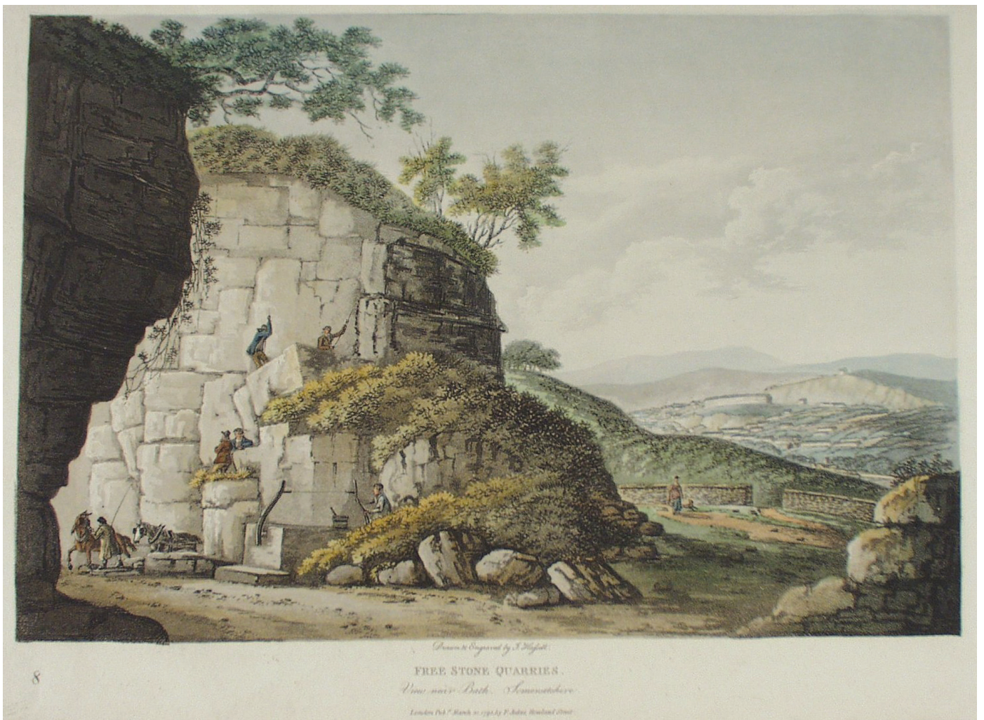
Fig. 3.12 Freestone Quarries near Bath by J. Hassall, about 1800. The site may be near Entry Hill. Note the use of bow-sawing and the wagon awaiting loading. (copyright Victoria Art Gallery, Bath & North East Somerset Council)
