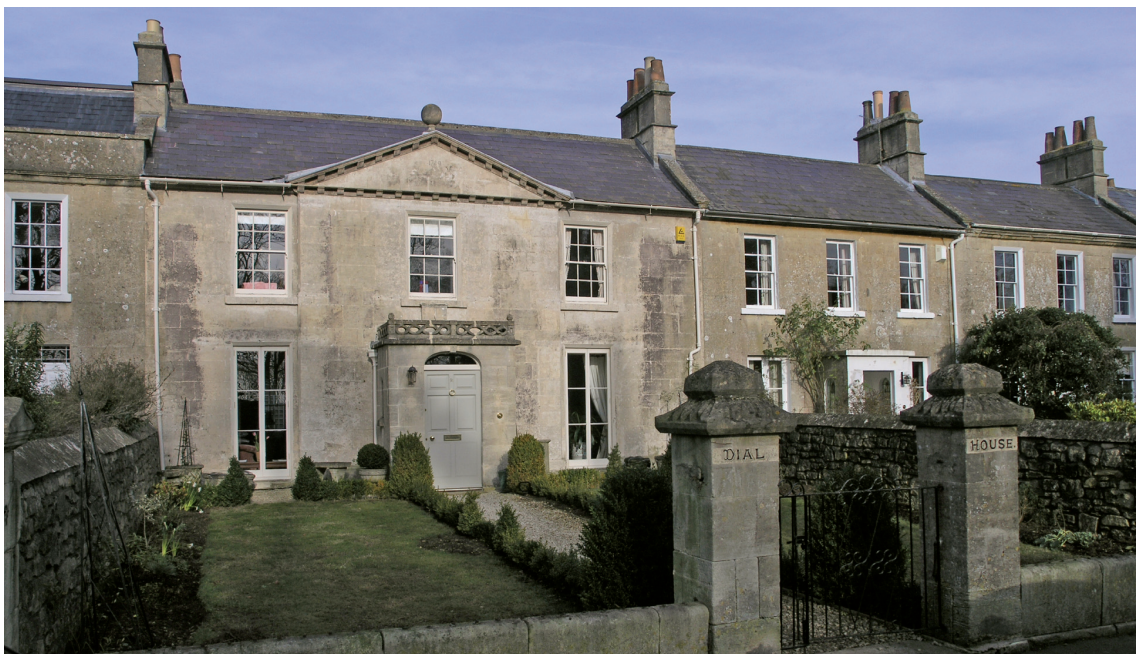
Fig. 3.8 The Old Rank of the eleven cottages at Combe Down, designed by Wood for Allen's workmen 1729-30
