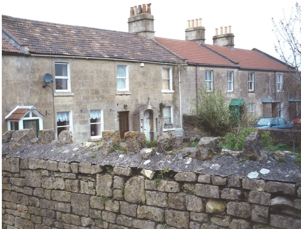
Fig. 4.4 The Farris Lane Cottages built on the quarry dump. The second from the right was the first to be built
