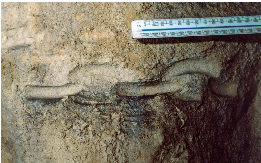
Fig. 7.14 Mould of chain formed by links pressing into the stone. The chain, wrapped around a pillar, was part of a crane anchor, late 19th century, Central Firs (Quarry 2201)
