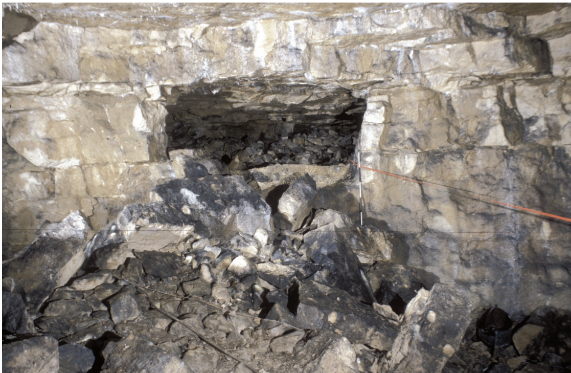
Fig. 7.10 Window used to throw out high-level spoil from Long Room working beyond, just north of Firs Shaft
