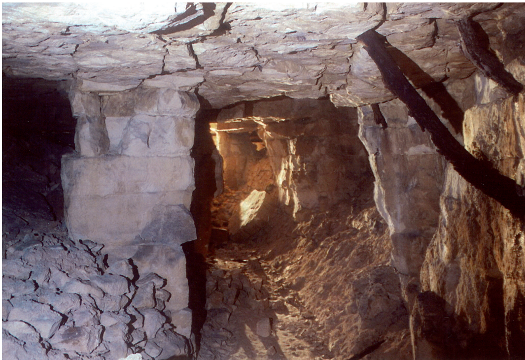
Fig. 7.12 Partially sawn pillar with timber sprag (or scorter) to tighten blocks in the roof (Photo by Paul Deakin)
