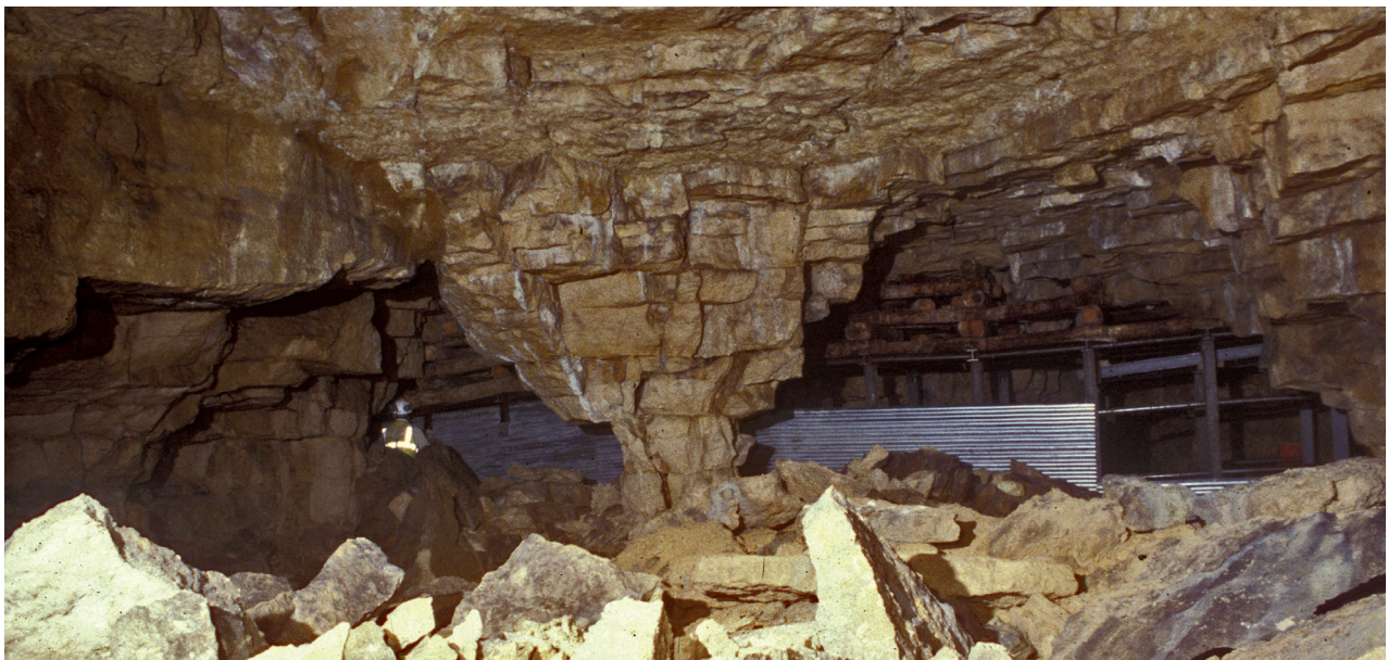
Fig. 8.36 The most extreme example seen of the reworking of a pillar, in East Firs (2203)
