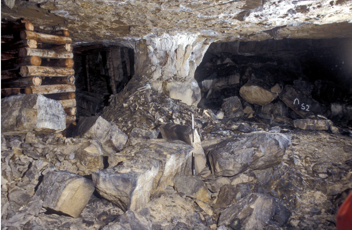
Fig. 8.5 Apophygate pillar showing the area picked and broken-out at the top, with a small lip below where the freestone beds were removed (Quarry 505)
