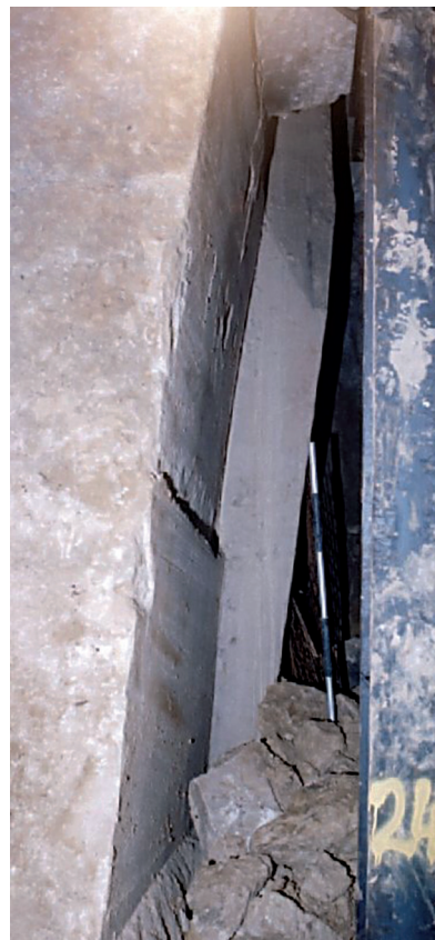
Fig. 8.32 Sawn face showing the slot left by a saw end penetrating into the rock at the far end (Shaft Road)
