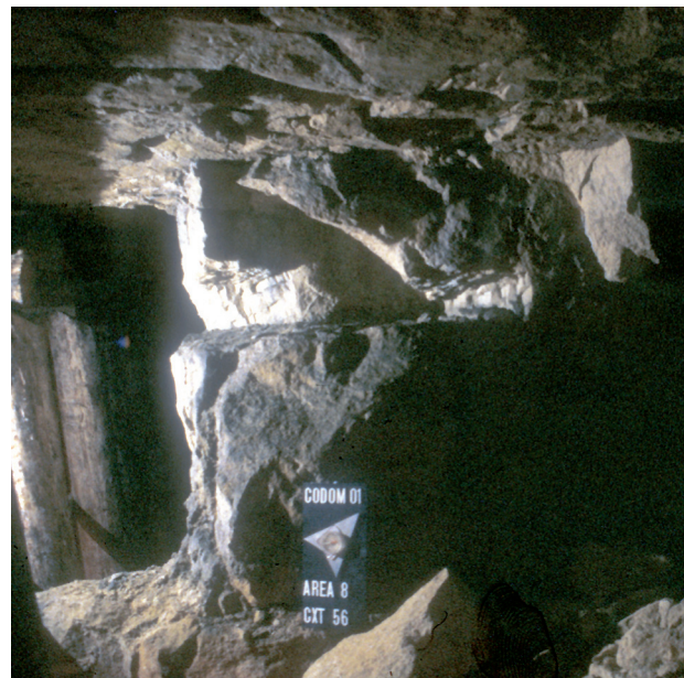
Fig. 8.7 Dressed block in situ showing use of a chamfered jad to assist removal. The use of the chamfered jad may be just the choice of the workman, but was probably mainly used for shallower depths
