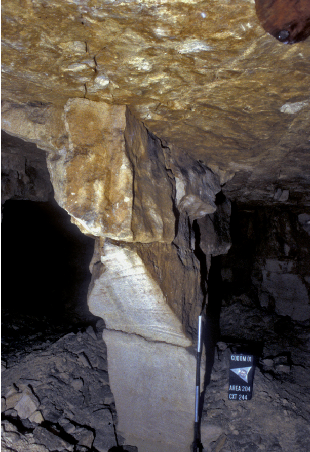
Fig. 8.29 Curved face (at top) made using a bow saw, to allow access to vertical saw cut below. Probably part of a secondary working, pillar robbing activity, Central Firs Quarry (2203)
