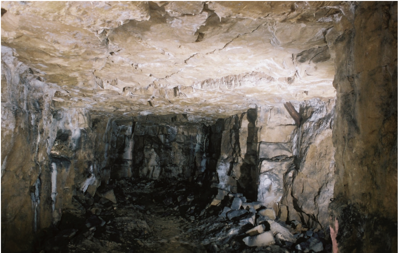
Fig. 8.9 Long Room developed just west of Firs Shaft (Quarry 2200). Note the window in the left wall, and the almost continuous side walls and the end wall which would greatly assist stability
