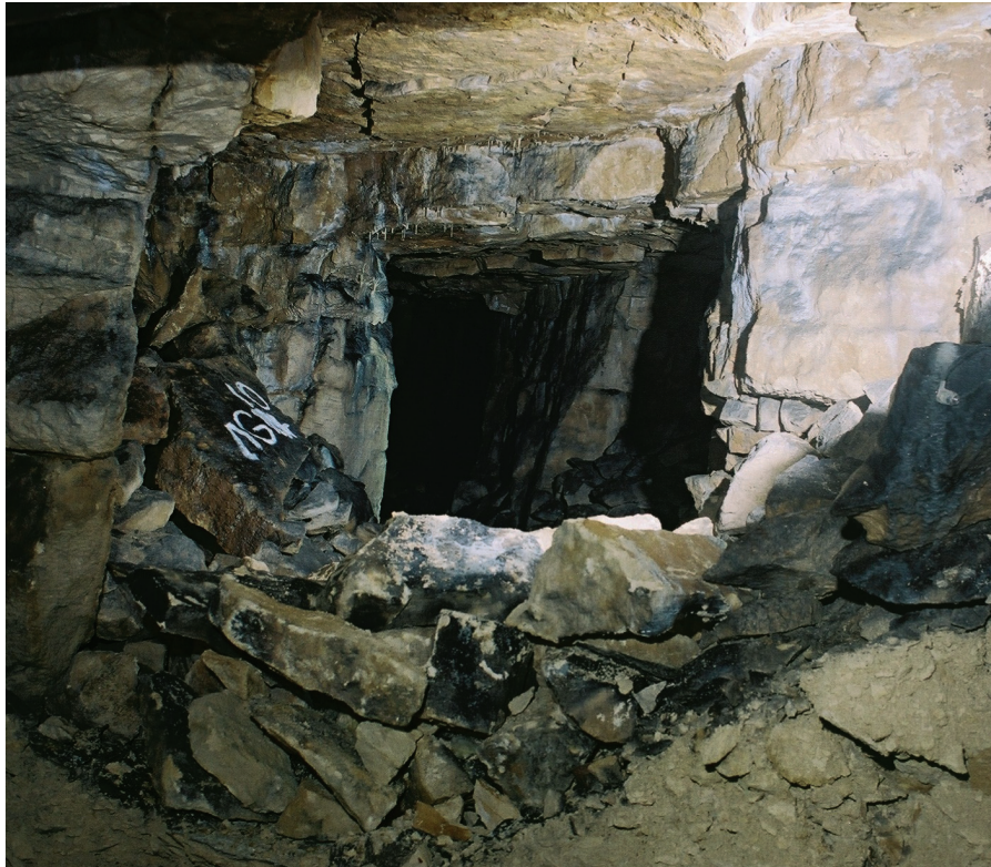
Fig. 8.10 Window used to dump spoil from the Long Room just beyond, north of Firs Shaft (Quarry 2201)
