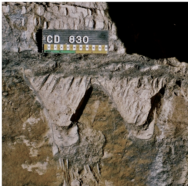
Fig. 8.20 Wedge pit impressions left from cutting down a pillar
