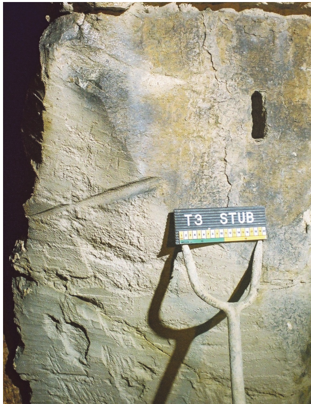
Fig. 8.26 Marks left by a scappling axe on a face, with wedge slots, south-east Byfield
