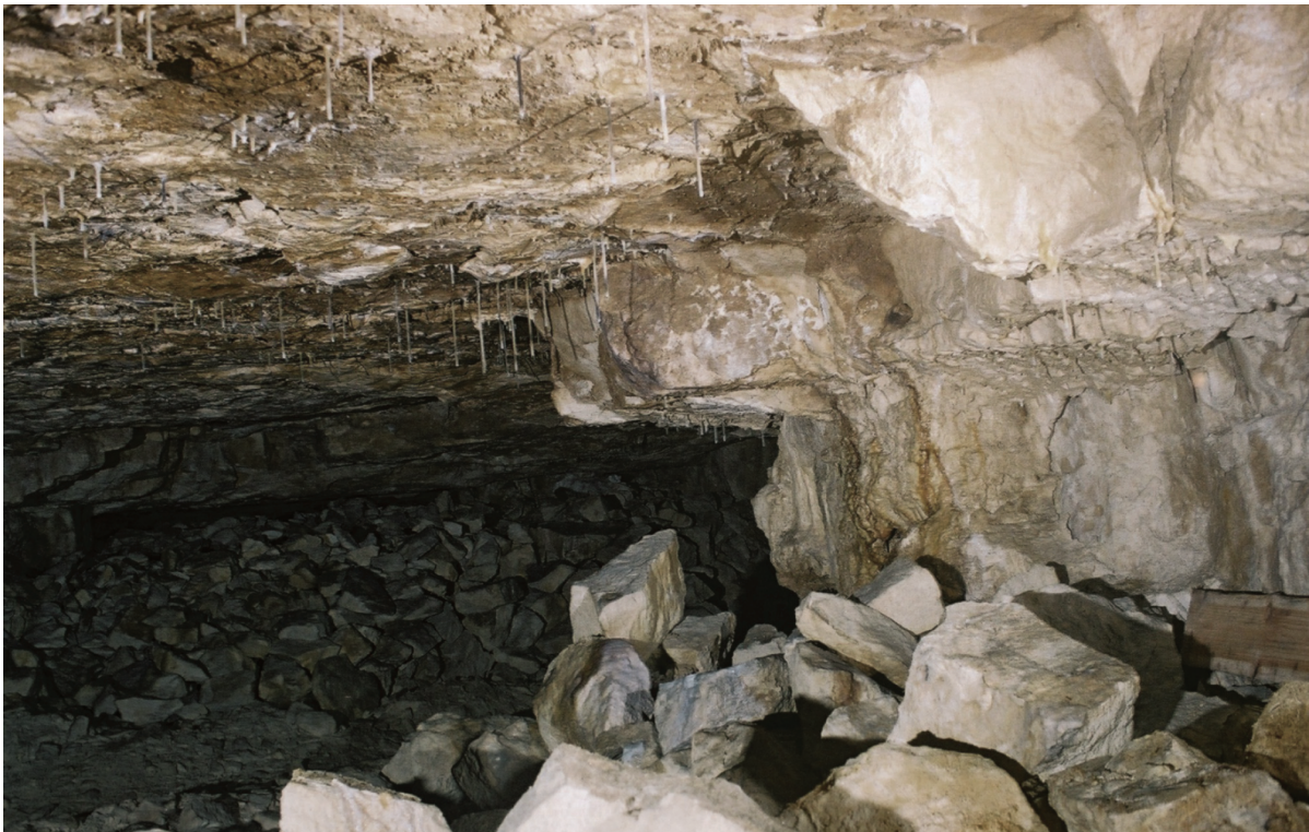
Fig. 8.8 Corbelled pillar in Firs Quarry (2201) Quarry Area 2211
