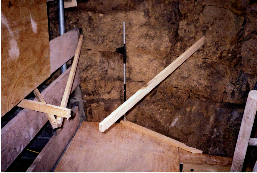
Fig. 9.37 Probable mast crane position inside the Firs Shaft indicated by wooden slats projecting from an arrangement of Lewis slots
