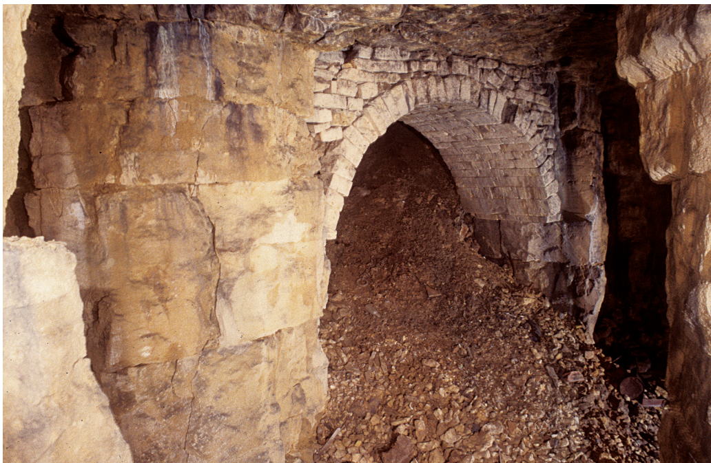
Fig. 9.15 The arch supporting the shaft on the Firs-Hadley Arms cartway
