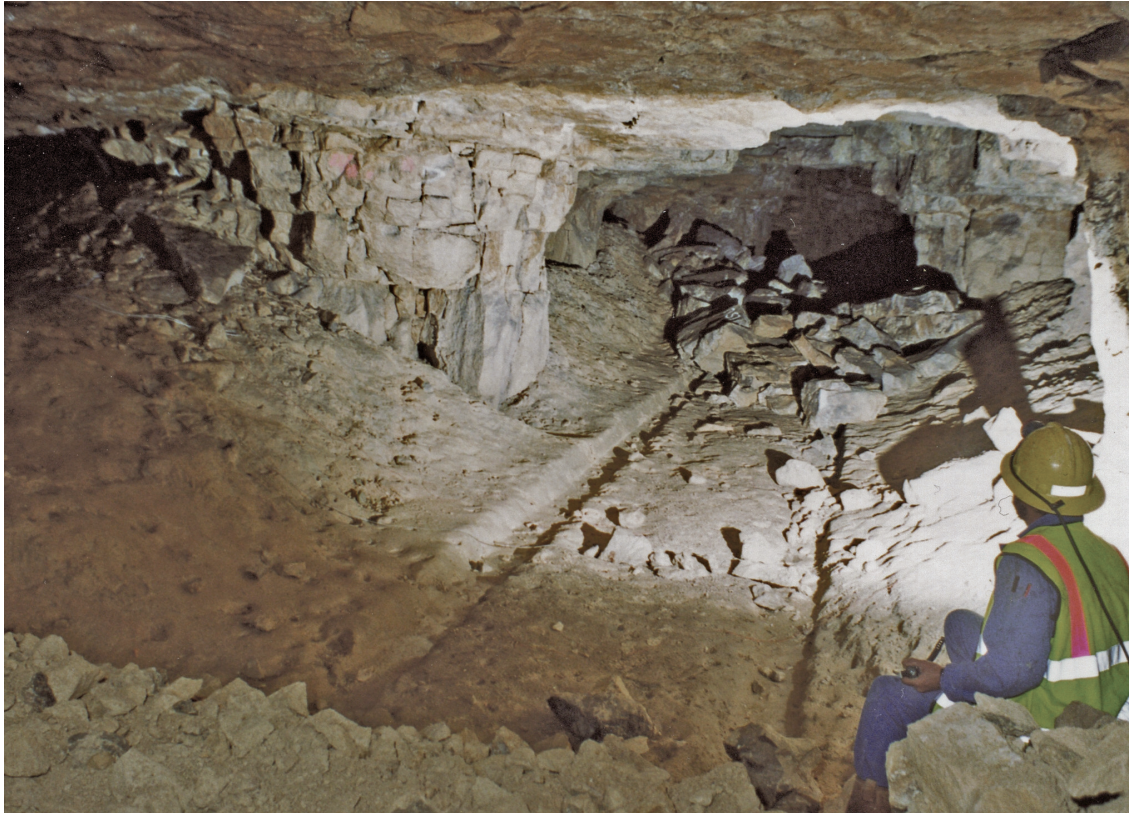
Fig. 9.4 Upper section of Allen's western cartway in central Byfield showing a roof-fall which is below a wide joint or "gull" in the roof. The seated figure is mine manager, John Lister
