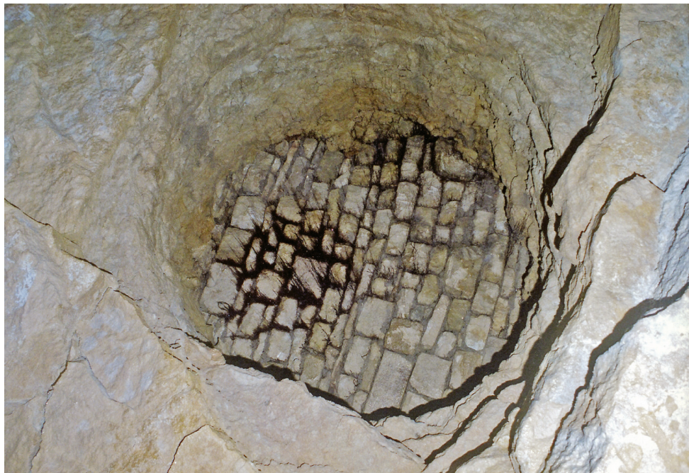
Fig. 9.40 Underside of barrel-arched shaft-cap in East Firs
