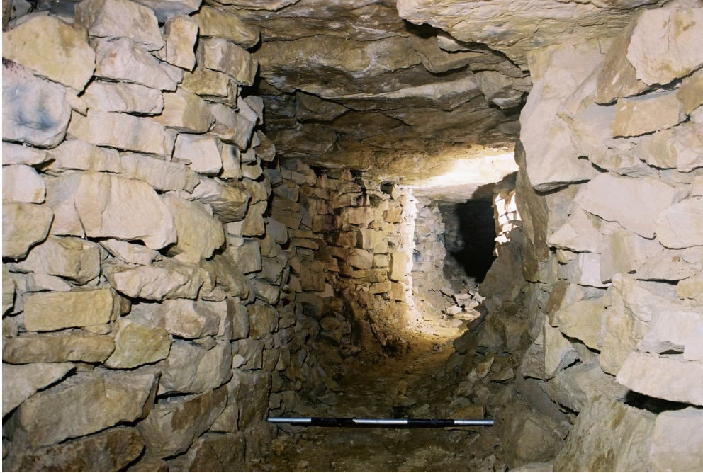
Fig. 9.20 Barrow-way in Far East Firs (Quarry 2365)
