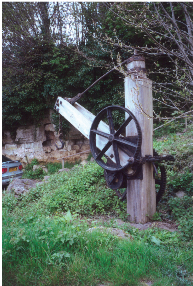
Fig. 9.36 Preserved underground crane at Combe Manor Hotel
