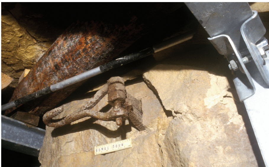
Fig. 9.33 A Lewis in situ in north Central Firs, used to hold a crane stay
