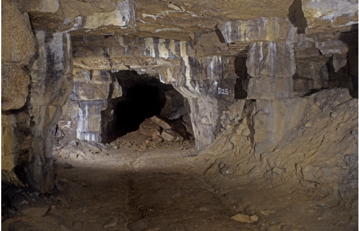
Fig. 9.5 Allen's east cartway in Central Firs. Note the remains of an apophygate pillar, on the left, the original roof destroyed by a fall. The heap is a cone of debris from the narrow shaft above. The passage with light from the left links to the west cartway
