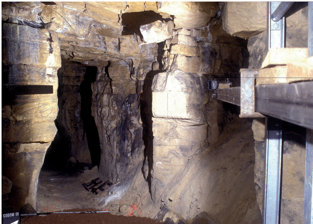
Fig. 9.14 Cartway near Firs Shaft leading towards the Hadley Arms. Note rub-marks from a cable on the left side-pillar and a corbel with a post-working fracture on the right-side pillar
