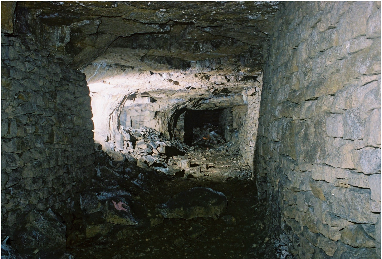
Fig. 9.6 Allen's west side cartway in Central Firs showing apophygate pillars and support packs alongside
