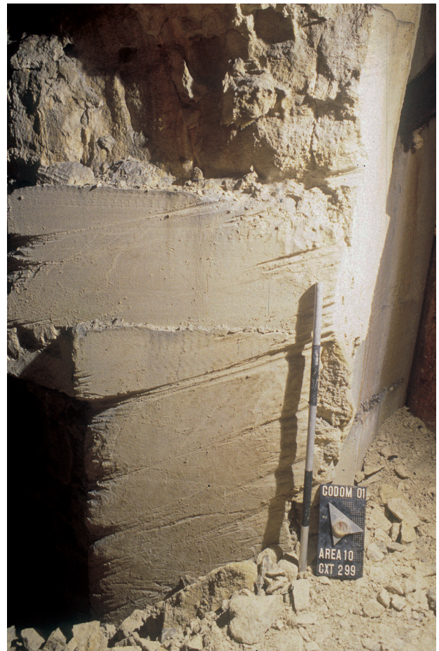
Fig. 9.30 Grooves in the side of a pillar at Allen's east side entry at Jones Quarry (Ralph Allen Yard), the nearly horizontal grooves suggesting the crane cable was diverted up the cartway to draw-out carts or wagons
