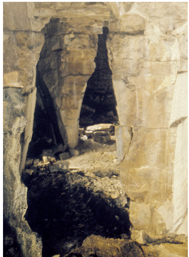
Fig. 10.11 Tapered sawn pillars in north Central Firs (Quarry 2215)
