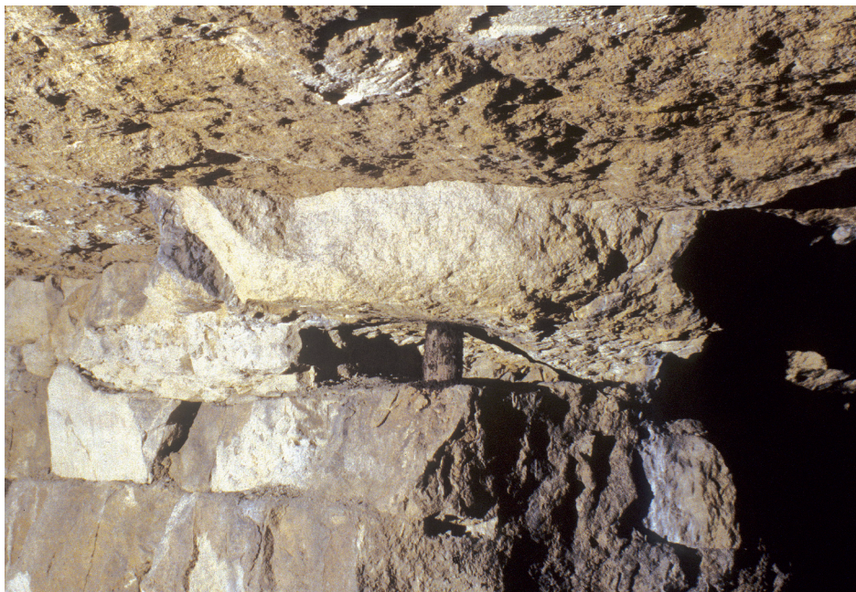
Fig. 10.23 Vertical prop placed on a pack
