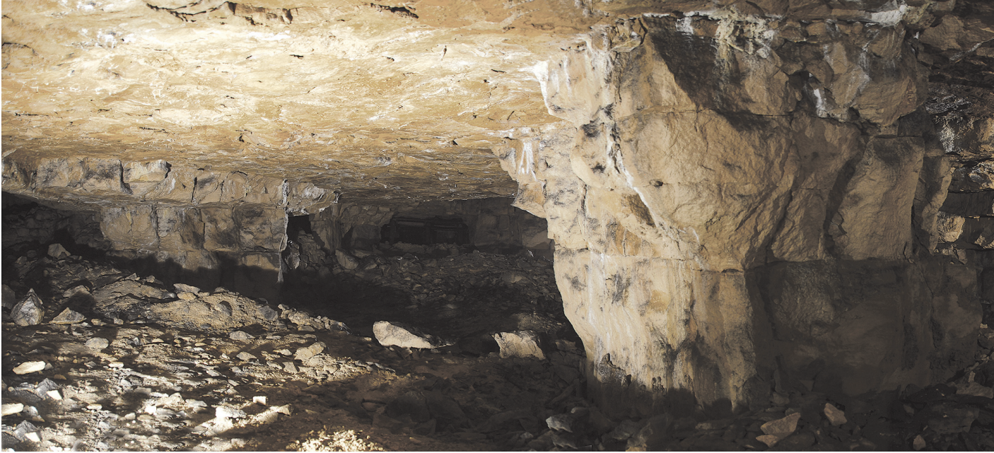
Fig. 10.2 Apophygate pillars within Central Byfield (Quarry 505). The pillar on the left is severely degraded
