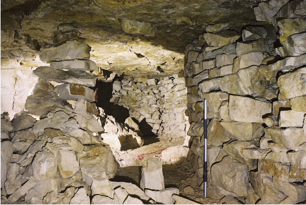
Fig. 10.30 Conical pack in East Firs (Quarry 2364)
