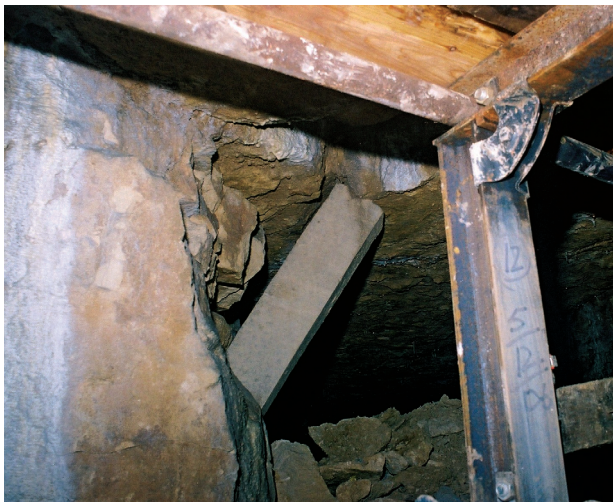
Fig. 10.31 Sawn stone used as a sprag in West Firs (Quarry 2342)
