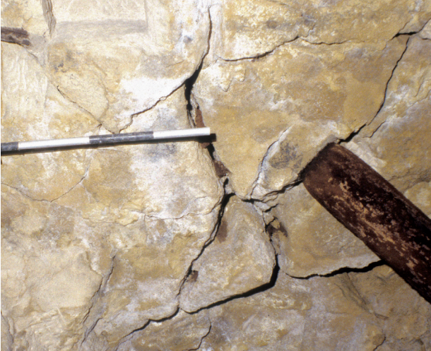
Fig. 10.21 Wooden wedges or cleats inserted to tighten roof blocks
