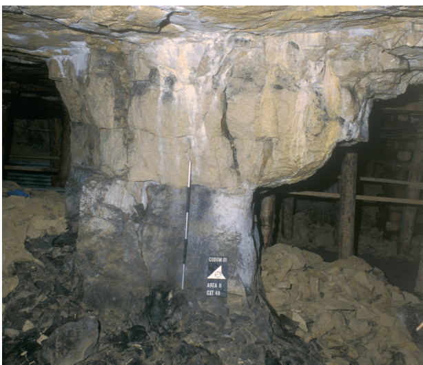
Fig. 10.7 Transitional form of apophygate and corbelled pillar in Central Byfield (Quarry 505)
