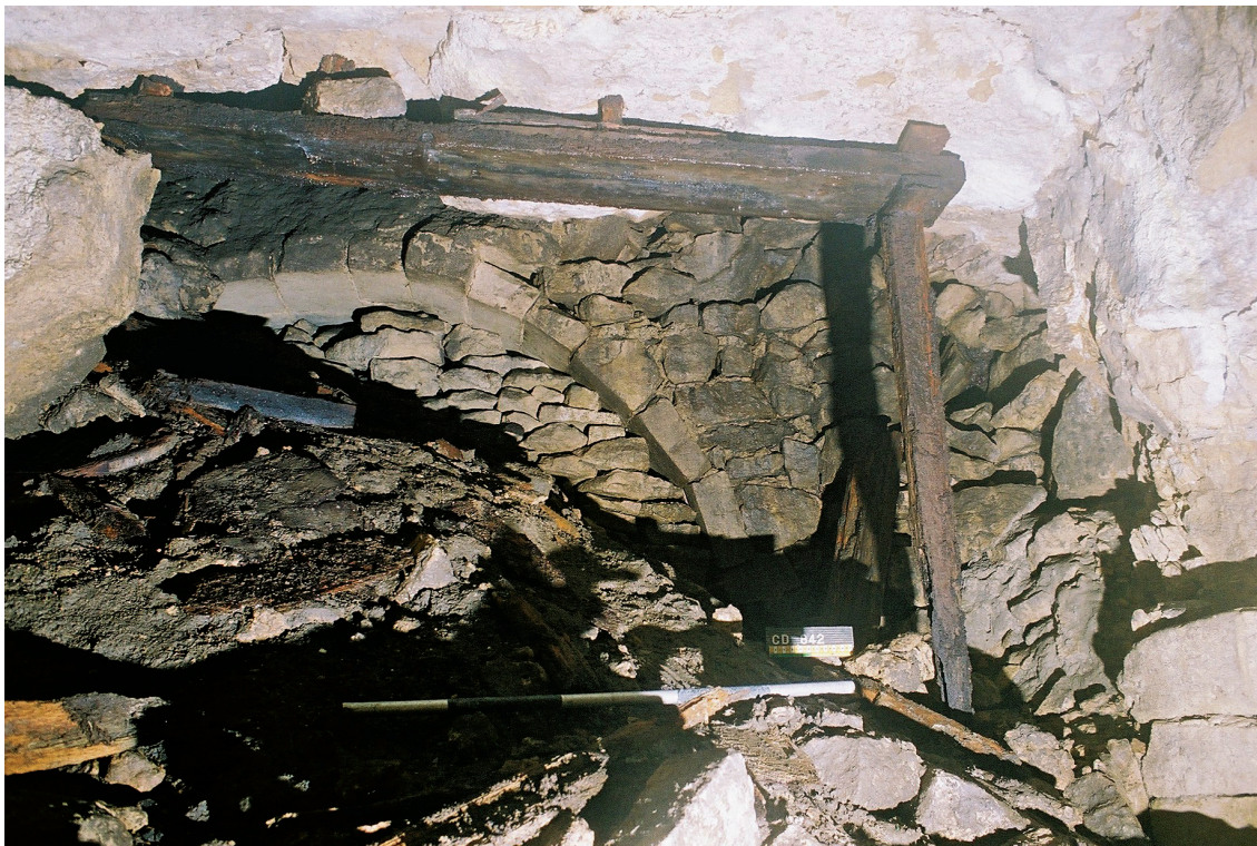
Fig. 10.24 Stone arch at a West Byfield entry (Quarry 505) with sawn voussoirs
