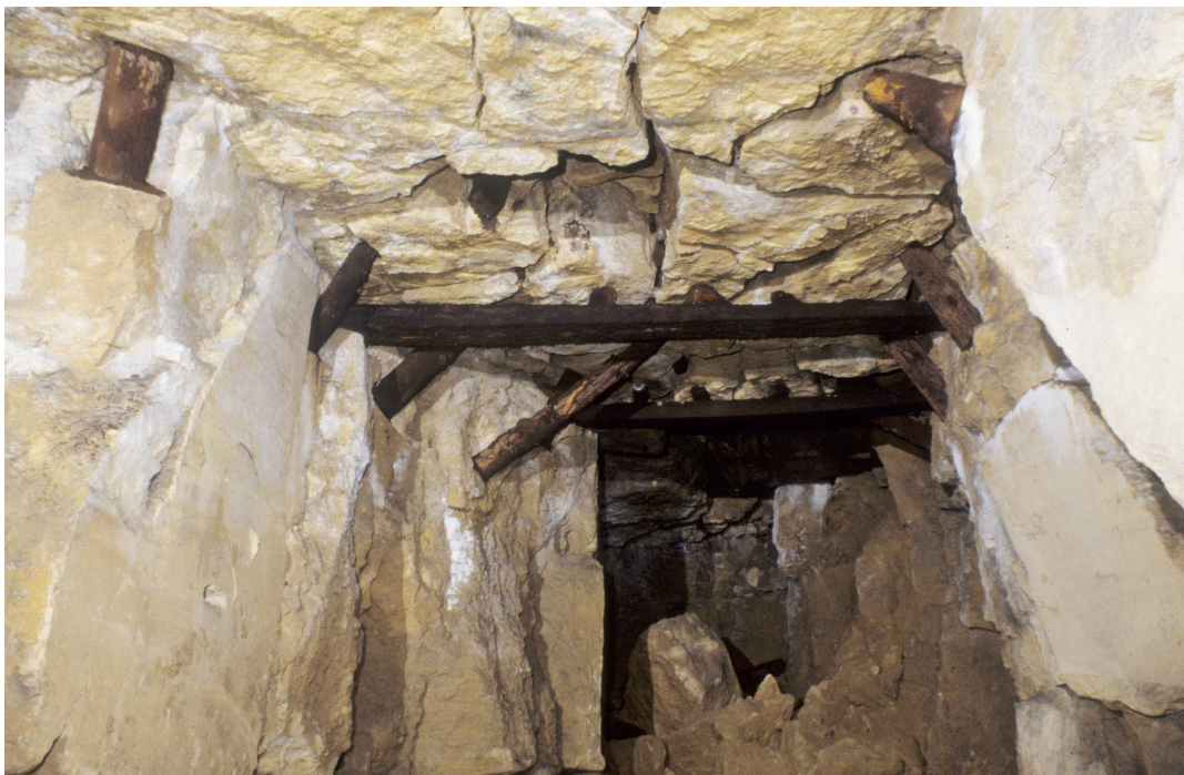
Fig. 10.22 Horizontal timber used for roof support under Shaft Road.
