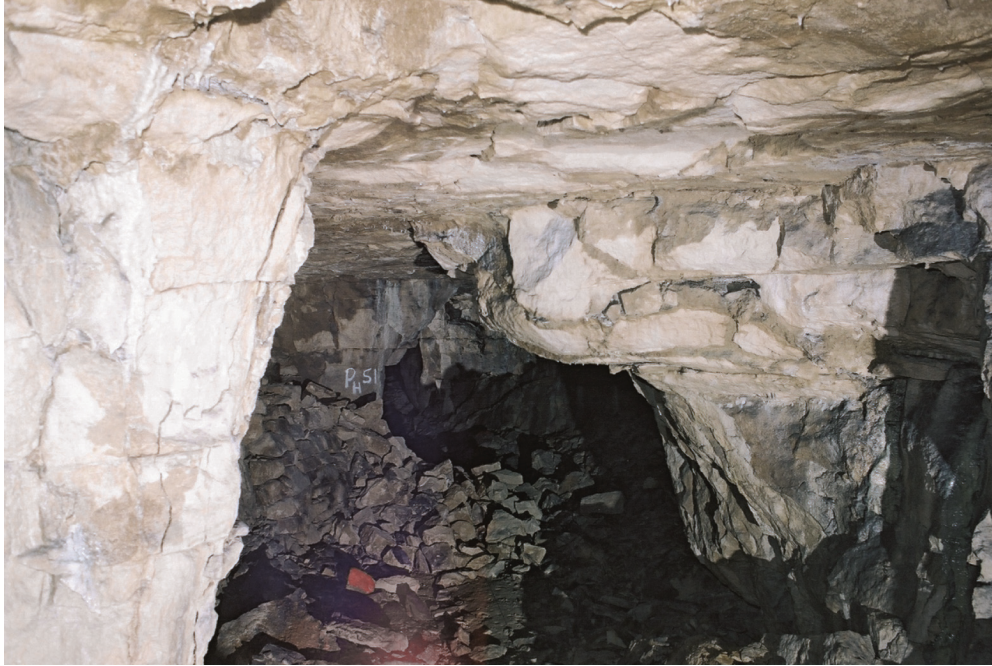
Fig. 10.6 Corbelled pillar in Byfield
