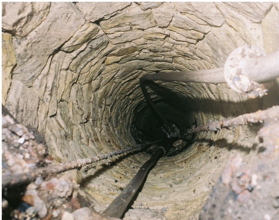
Fig. 11.2 The Carriage Inn well, in the pre-Allen E4 stub workings, (Central Firs, Quarry 2347). The two pump rods and pipes are visible, but the pumps themselves appear to be buried
