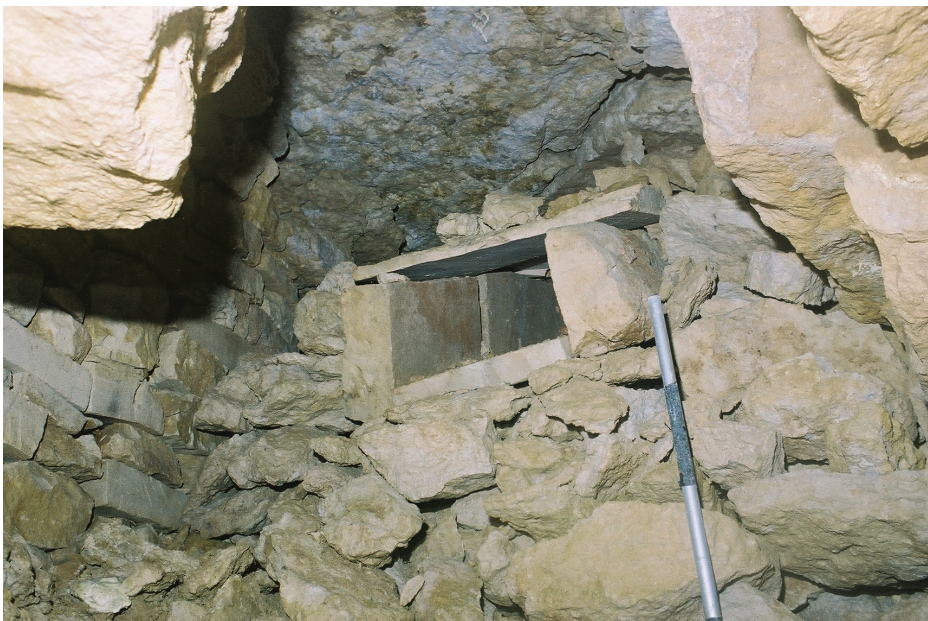
Fig. 11.5 The probable drain in Quarry 2392 in Far East Firs, projecting through the roof. Made of thin-sawn stone slabs, there was no sign of it ever having been used
