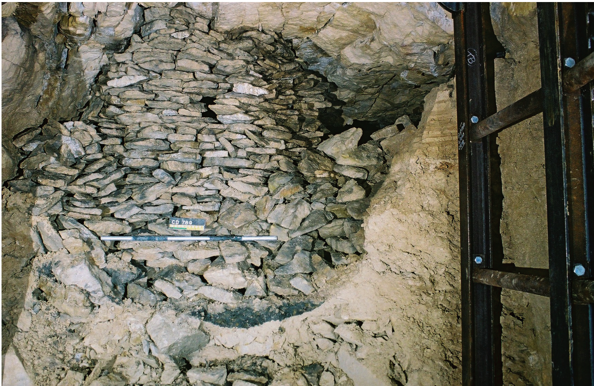
Fig. 11.3 The well in Byfield (Quarry 911) just east of Ralph Allen Yard, was sunk through pre-existing workings but, unusually, had been lined from within the well shaft, resulting in the 'inside-out' pack seen here
