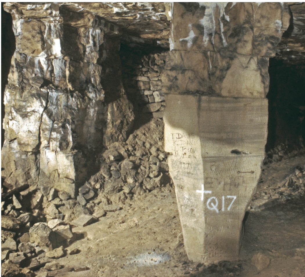
Fig. 11.8 Tapered pillar in north-east Byfield Quarry (308) with a wide range of inscriptions including the date 1816 (faint and high to the right), giving a fairly reliable earliest date for the sawn face and other activity in the area
