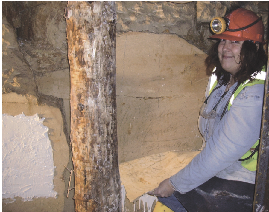
Fig. 11.10 Successful stripping of the Knowles and Prescott graffiti using silicon rubber. Far East Firs (Quarry 2363)
