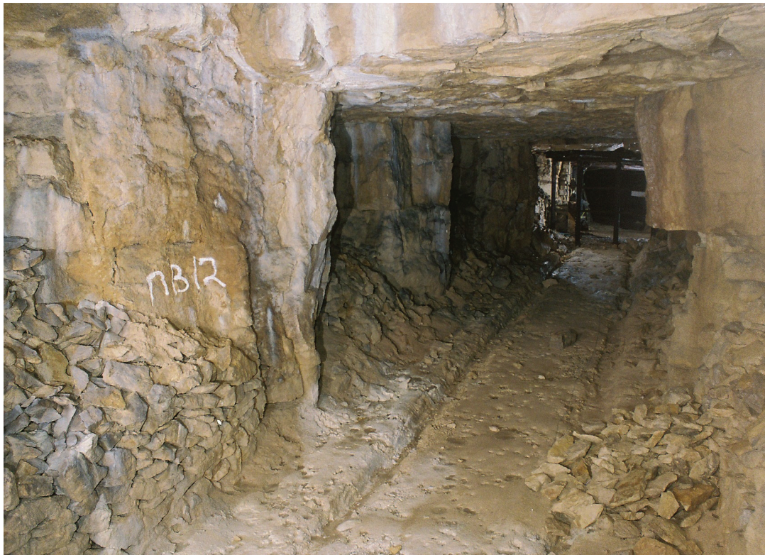
Fig. 12.19 Late 18th- to 19th-century cartway with cart ruts in West Firs (Quarry 2342) which belonged to Samuel and John Pearce
