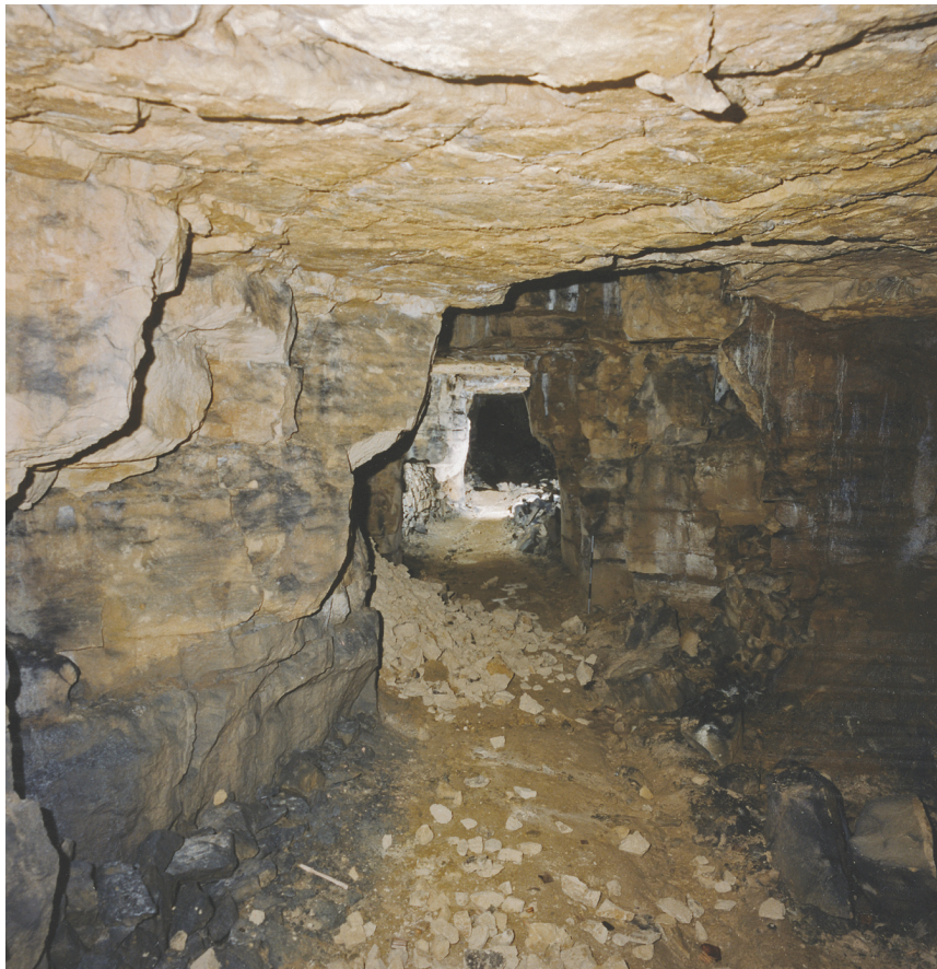
Fig. 12.14 View down the eastern cartway near the Firs Shaft
