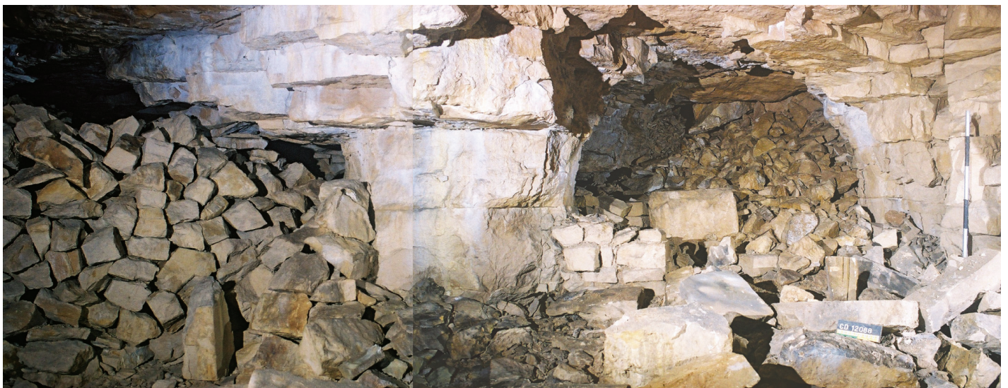
Fig. 12.3 Apophygate arches and supporting packs with masons working area in the foreground
