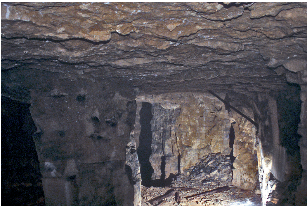
Fig. 12.37 Pillar with scorter recesses
