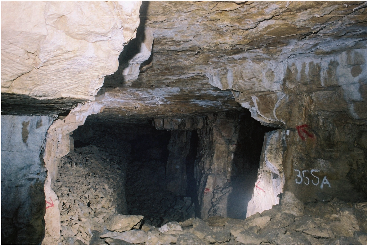
Fig. 12.6 The partially infilled cartway suggesting an entry from the north-west side (in Sheeps House Quarry)
