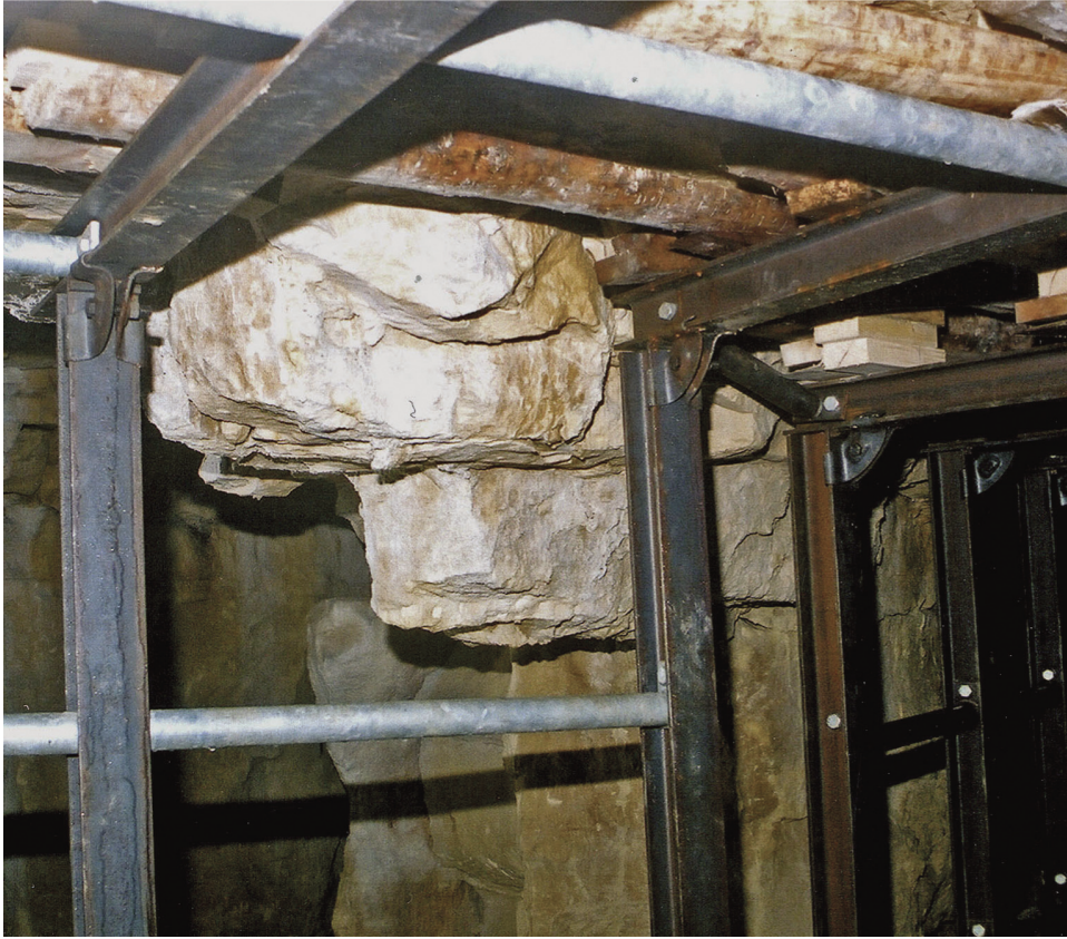
Fig. 12.8 Long corbels on a pillar in the E4 Stub
