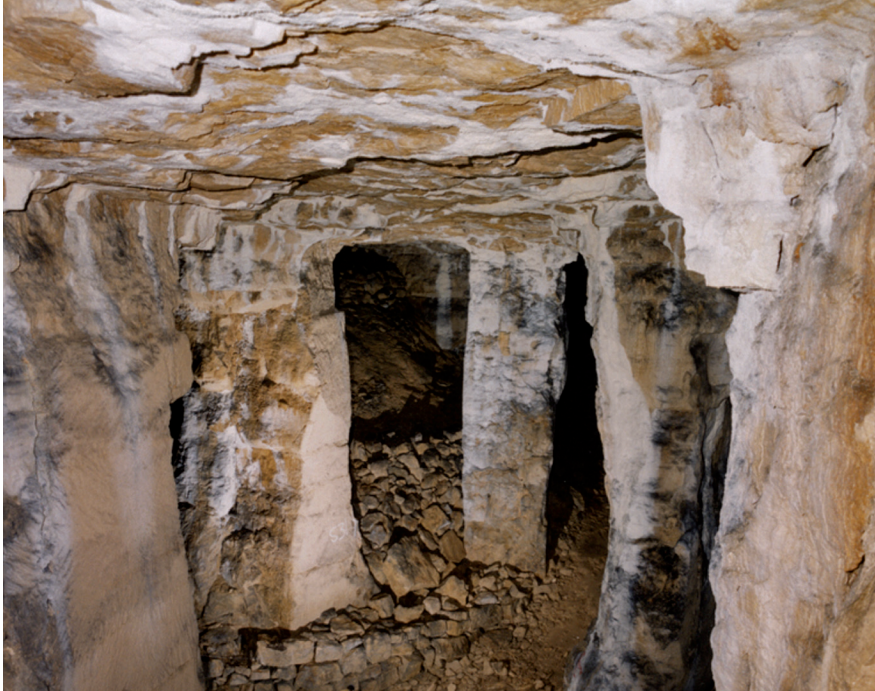
Fig. 12.21 High pillars in William Hulonce's Quarry (West Byfield)
