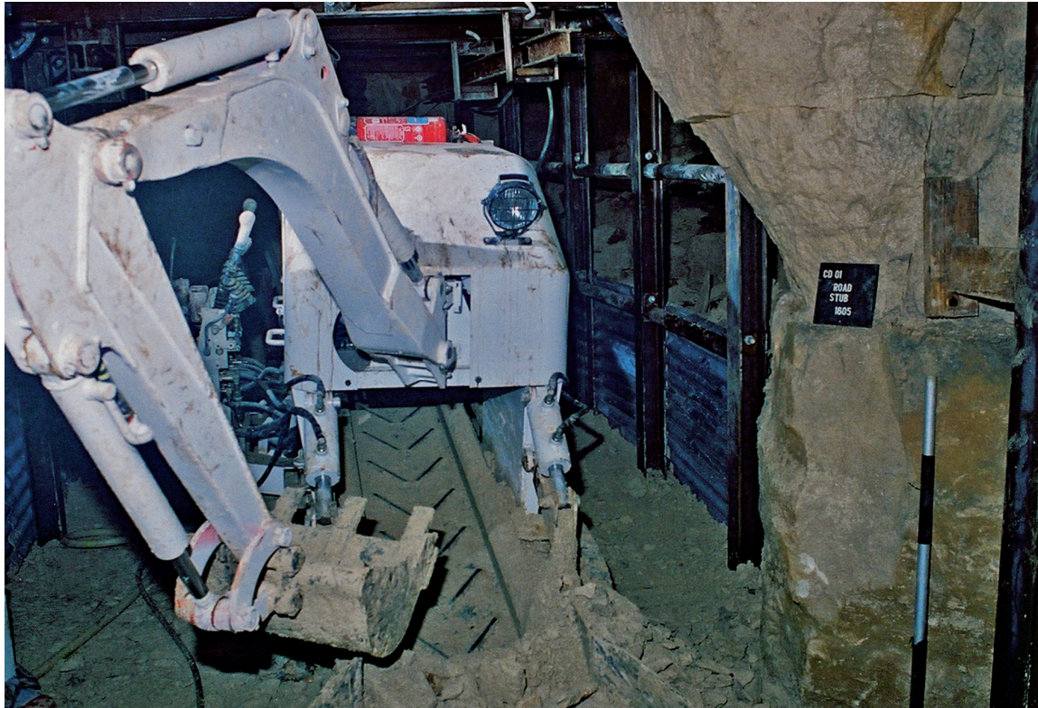
Fig. 1.8 Modern roadway heading with tracked mini-excavator – East Firs
