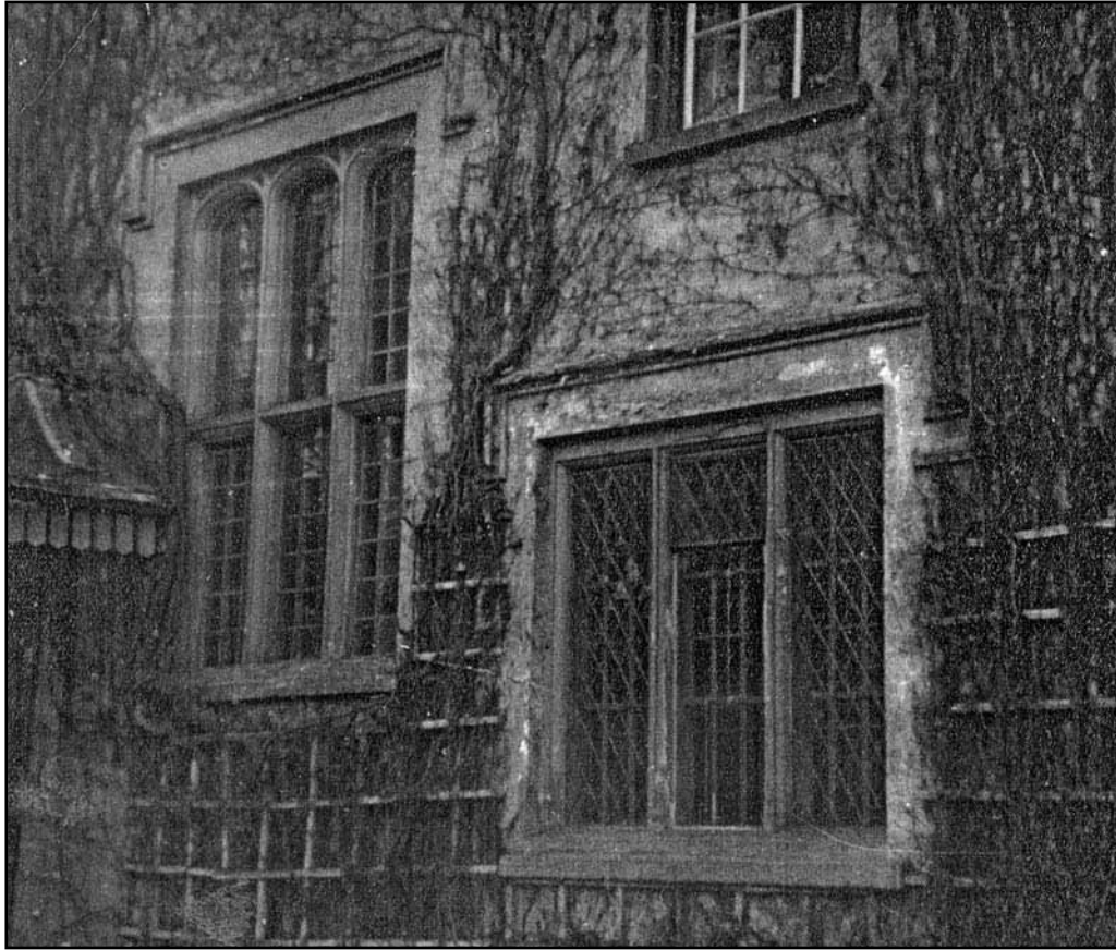
Plate 6: Mullioned windows of Old Palace House c.1968
