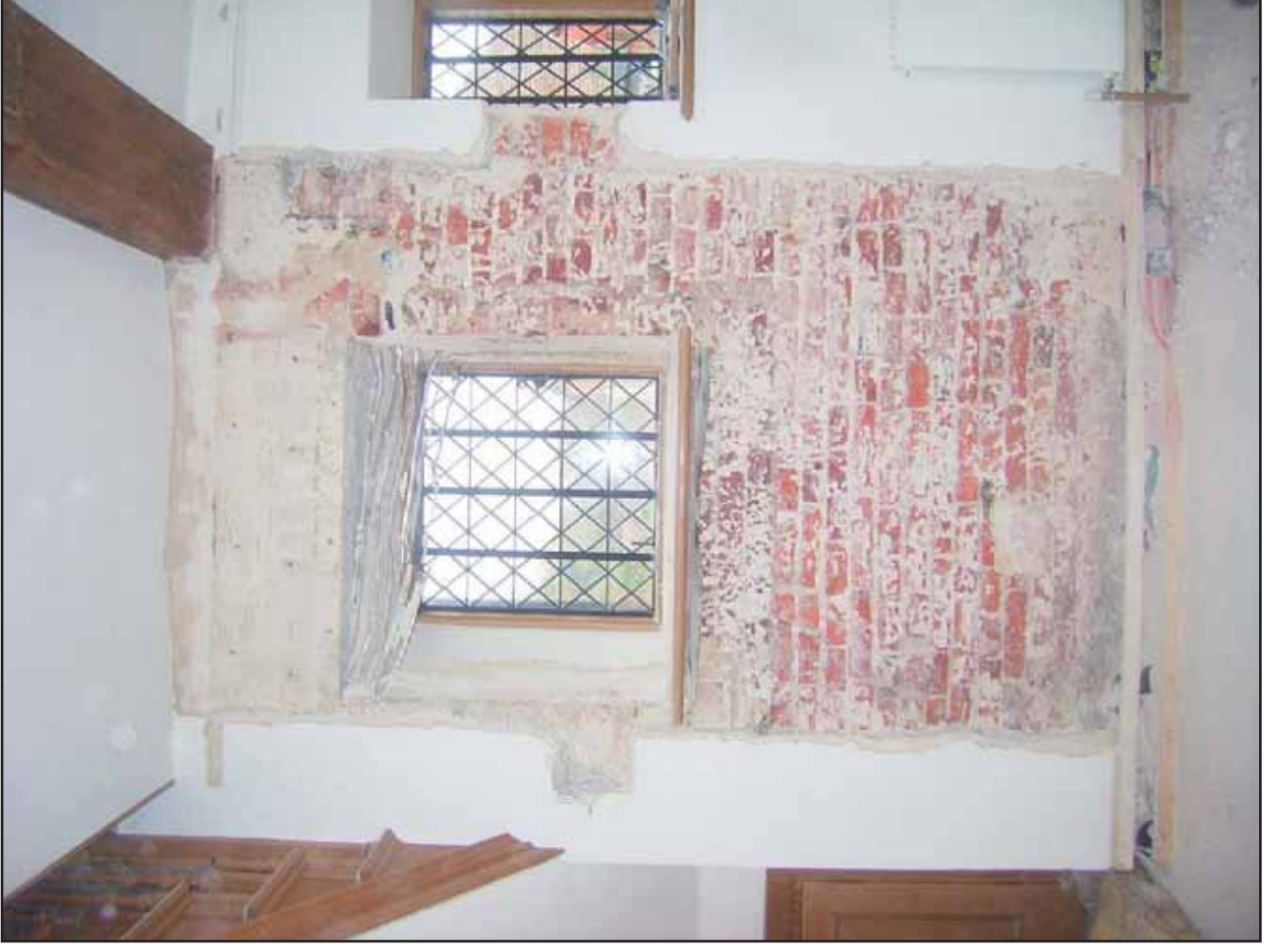
Plate 8: Sutton Place, Opening WWG7 prior to removal of walling (W elevation)
