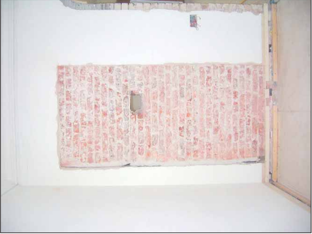
Plate 7: Sutton Place, Opening DF70 prior to removal of walling (N elevation)
