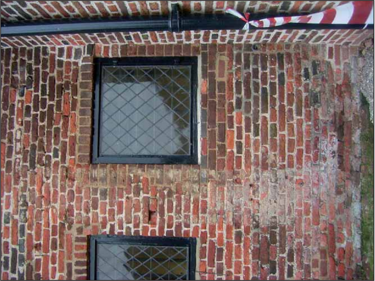
Plate 9: Sutton Place, Opening WWG7 prior to removal of walling (E elevation)
