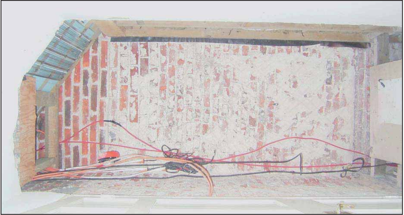
Plate 1: Sutton Place, Opening DF53 prior to removal of walling (W elevation)
