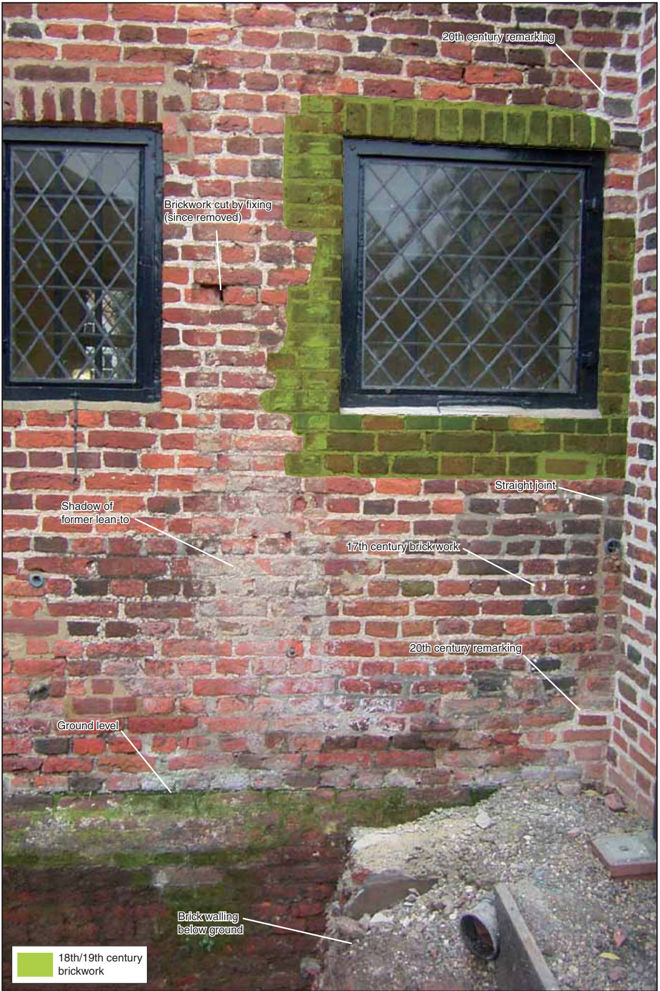
Figure 5: Sutton Place – Opening WWG7 as seen from exterior (west facing)
