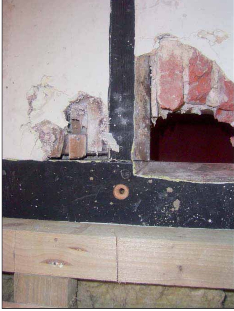
Plate 4: Sutton Place, Opening DF66 detail of chamfered timbers and infill (SE elevation)
