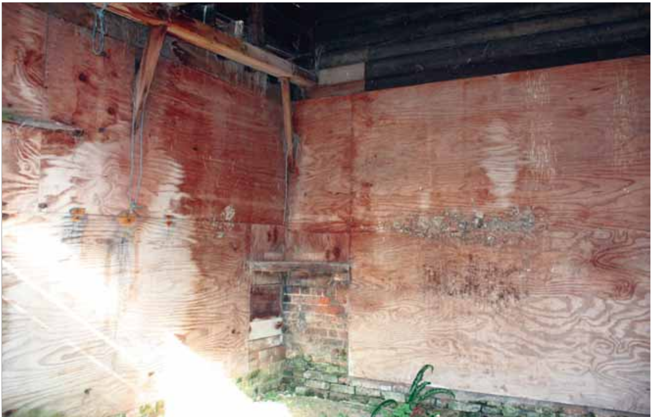
Plate 9: Internal view, Building 2
