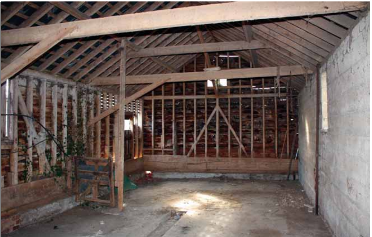
Plate 6: Internal view, Building 1
