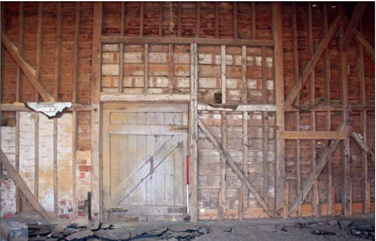
Plate 27: Detail of door from inside Building 5
