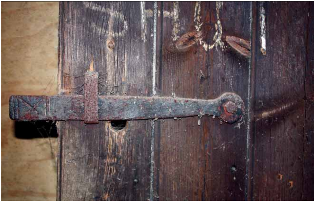
Plate 36: Detail of latch on internal door, Building 6
