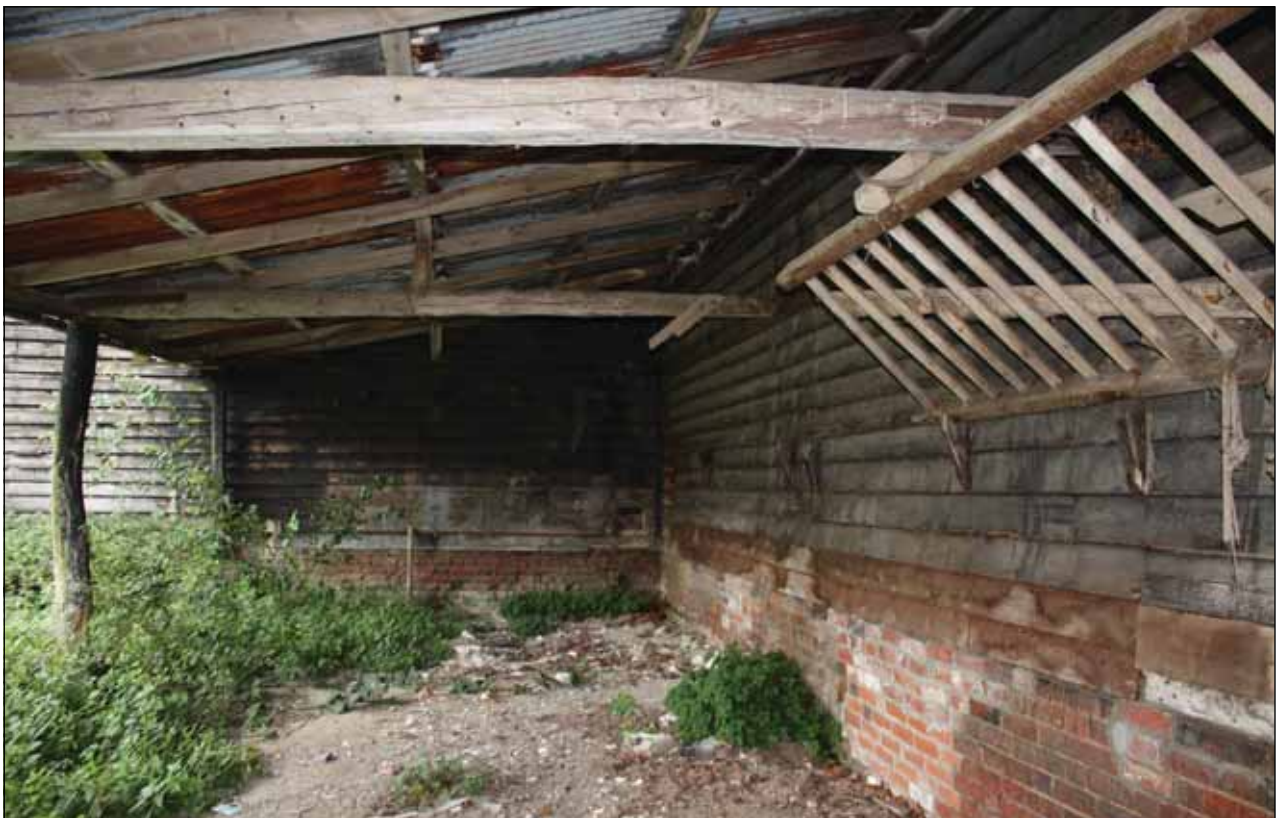
Plate 39: Internal view, Building 7
