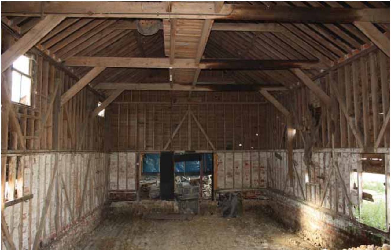
Plate 20: Internal view, Building 4
