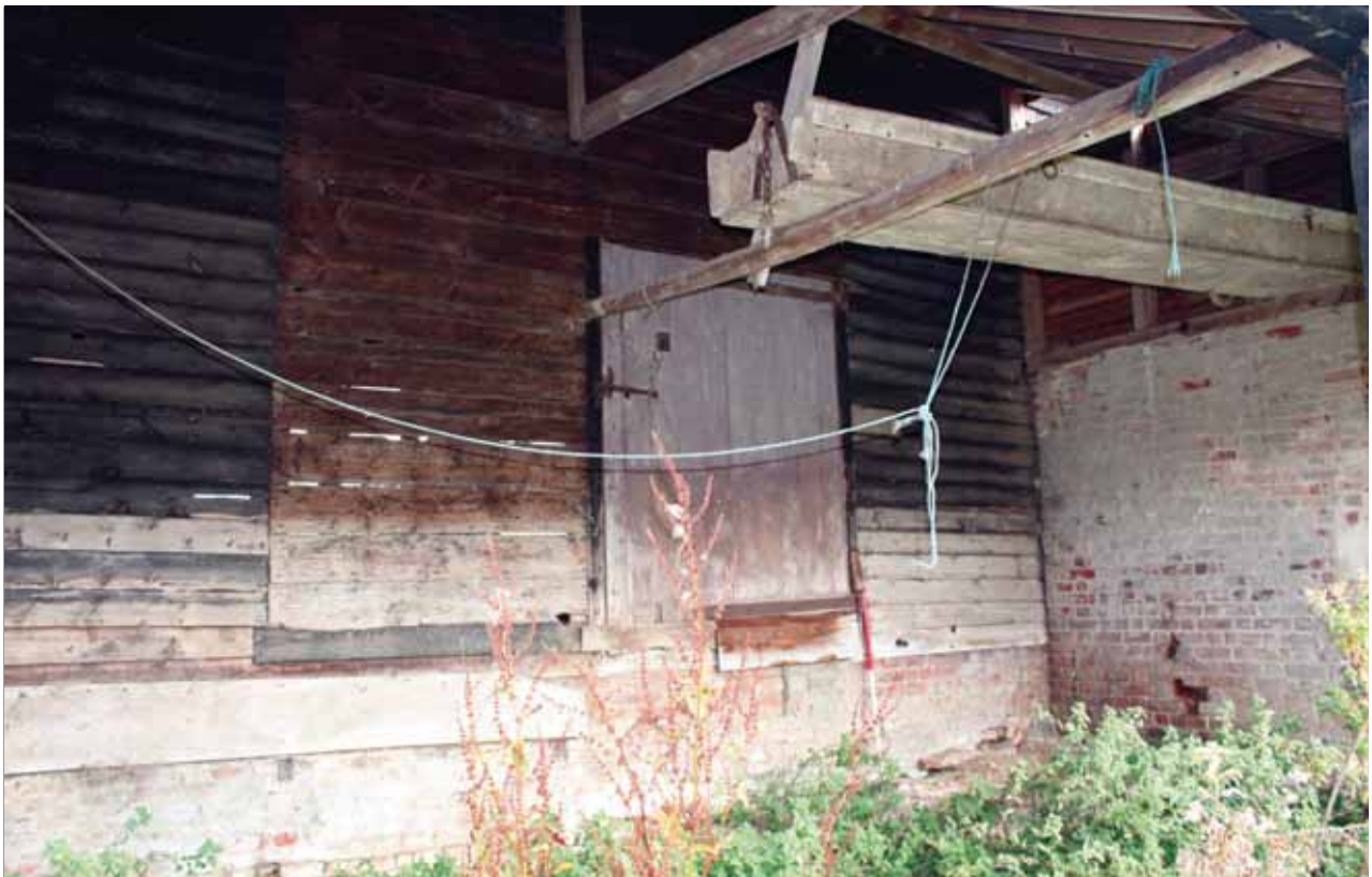
Plate 10: Detail of door on south-facing elevation of Building 5 (from inside Building 2)
