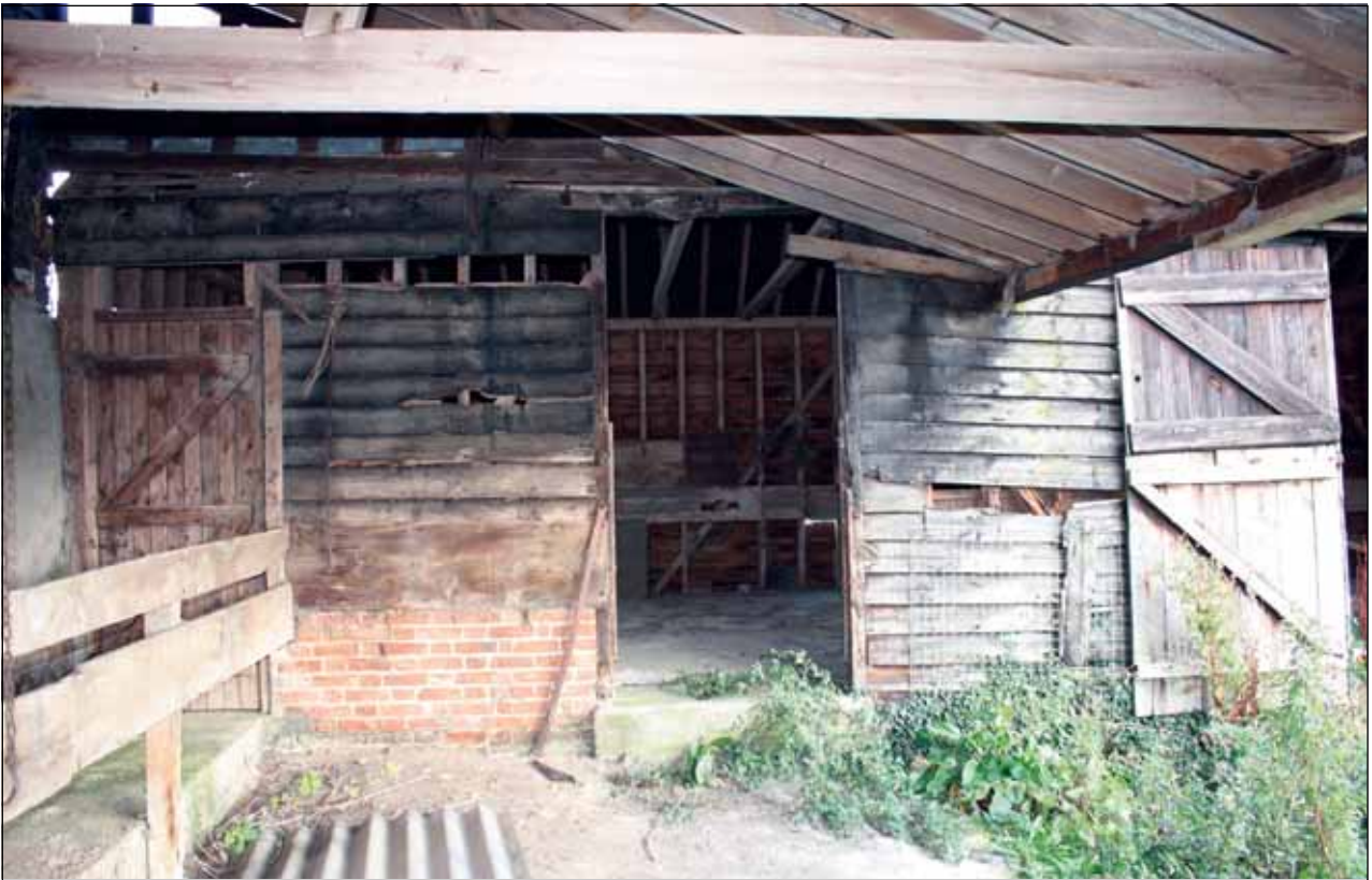
Plate 22: Internal view, Building 4b
