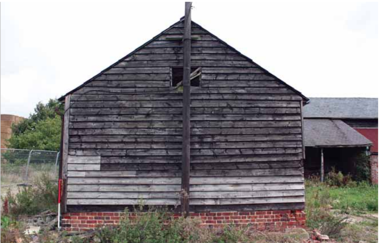
Plate 2: North-facing gable-end, Building 1
