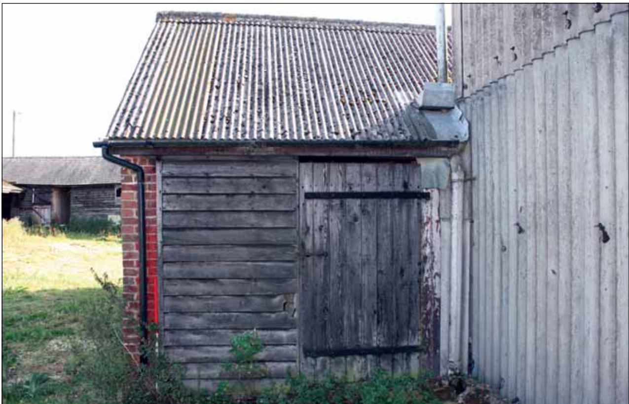
Plate 50: West-facing elevation, Building 9
