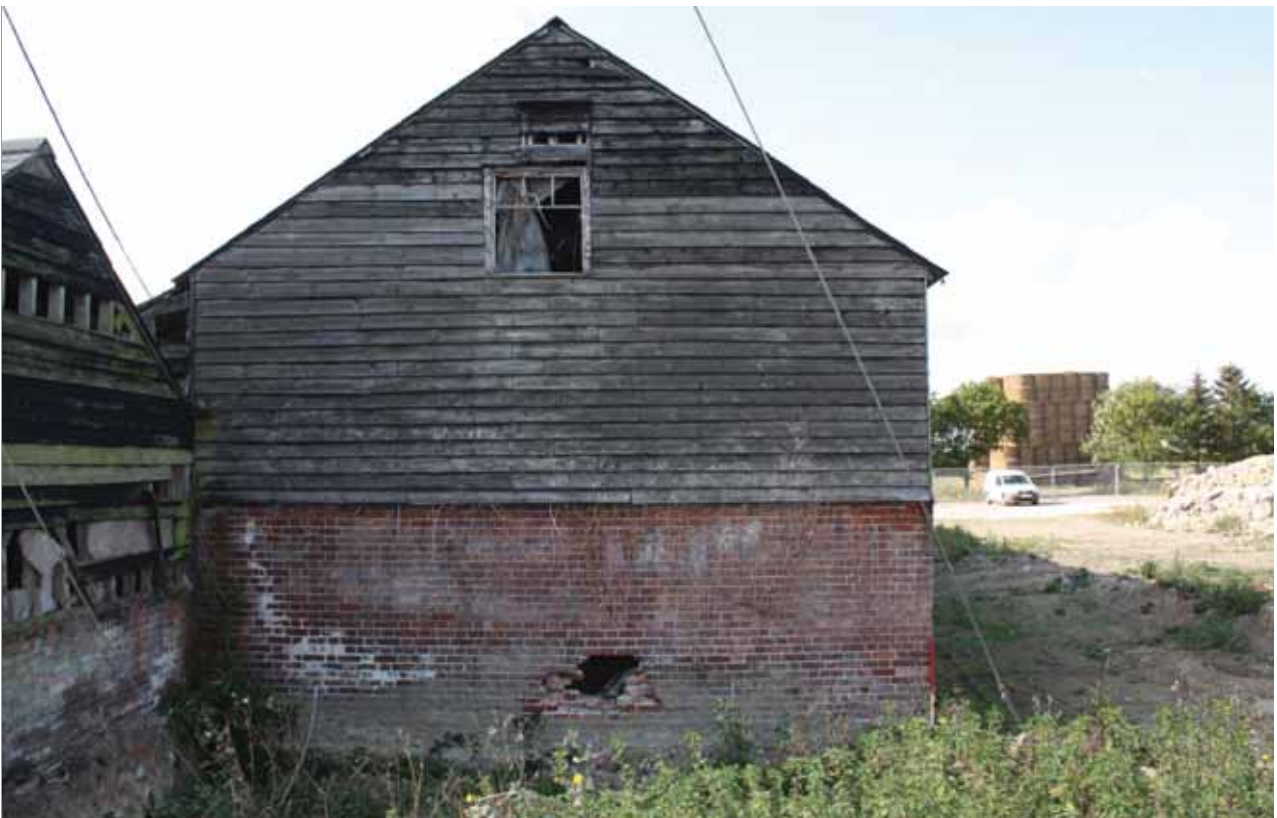
Plate 16: East-facing elevation, building 4
