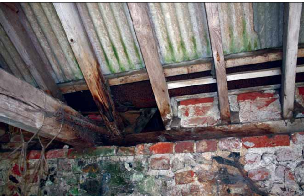
Plate 45: Detail of wall-plate, tie beam and common rafters inside Building 8
