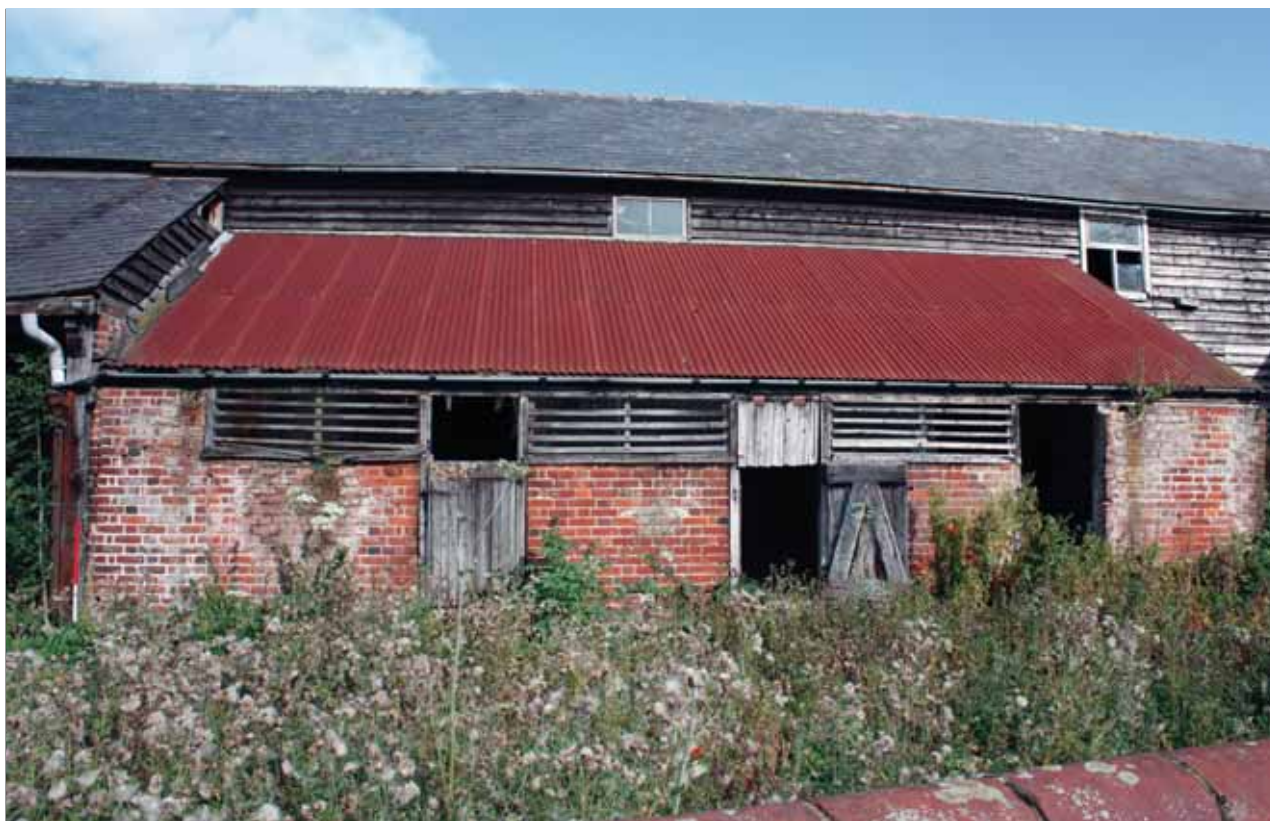
Plate 11: South-facing elevation, Building 3
