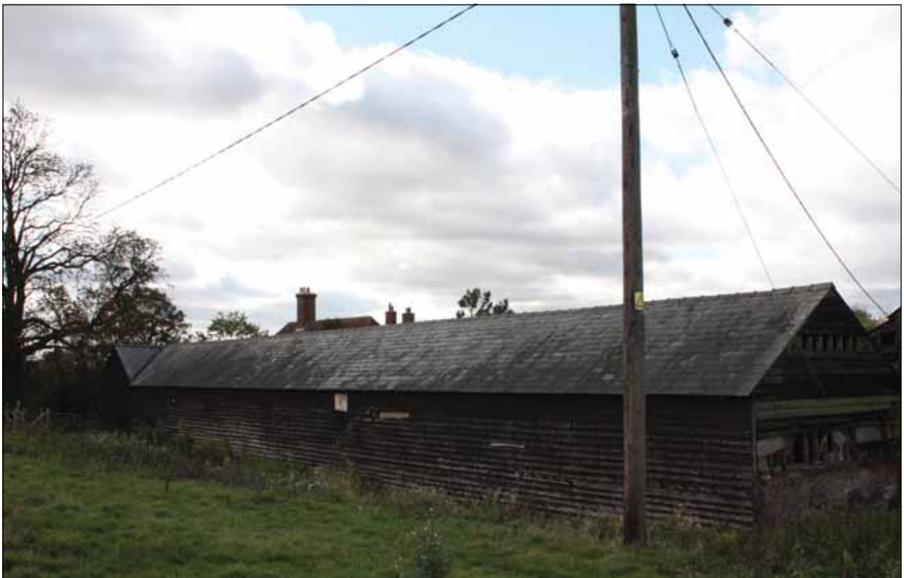
Plate 32: East-facing elevation, Building 6
