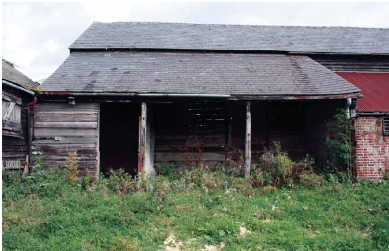
Plate 8: South-facing elevation, Building 2
