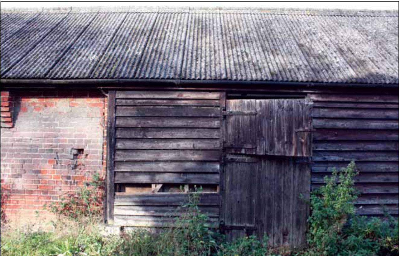
Plate 41: Detail of weatherboard and door on Building 8
