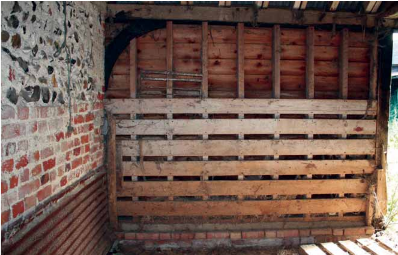
Plate 49: In-filled former opening, from inside Building 8
