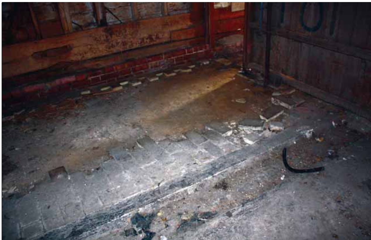
Plate 7: Detail of drainage gully and brick floor, Building 1
