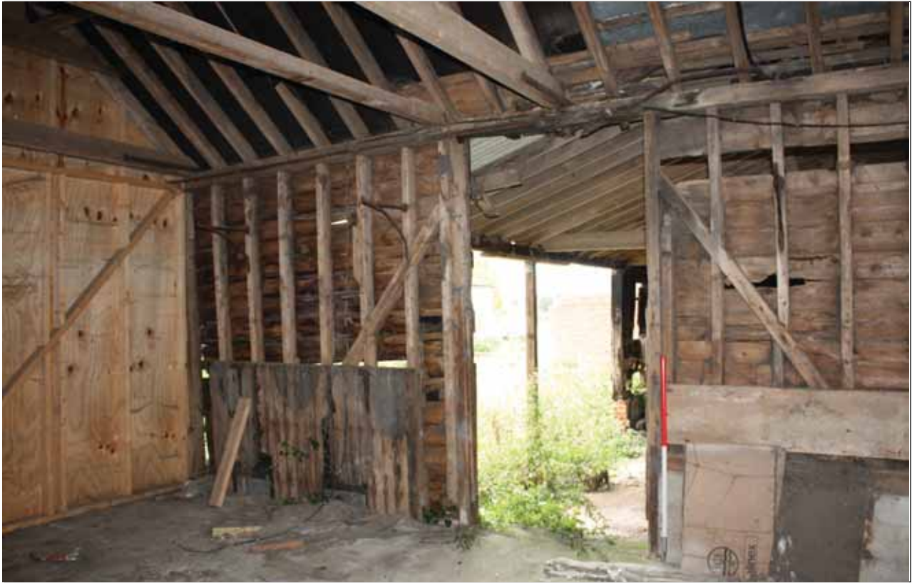
Plate 34: Internal view, Building 6
