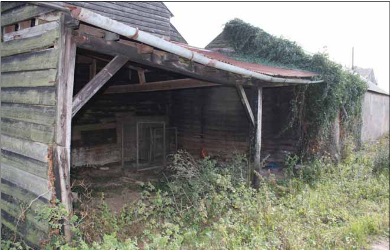
Plate 24: Detail of west-facing elevation, Building 5
