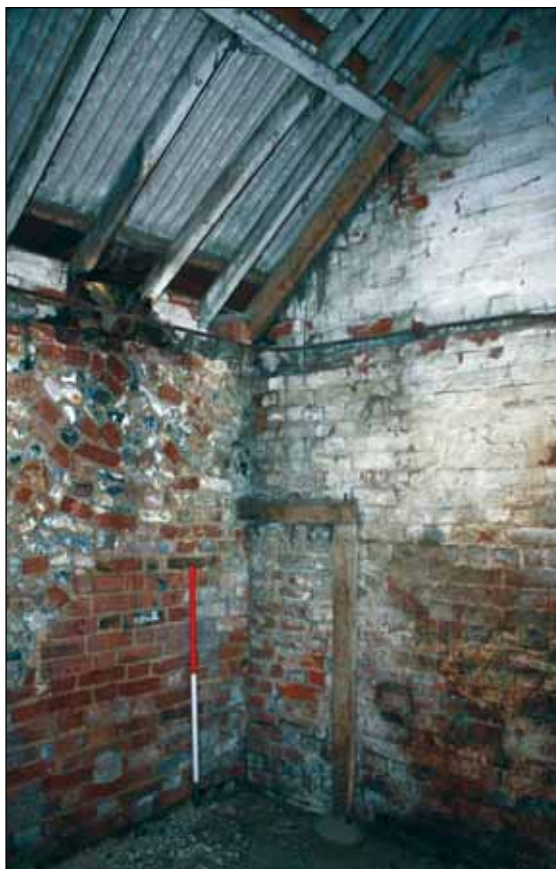
Plate 54: Internal detail, Building 9
