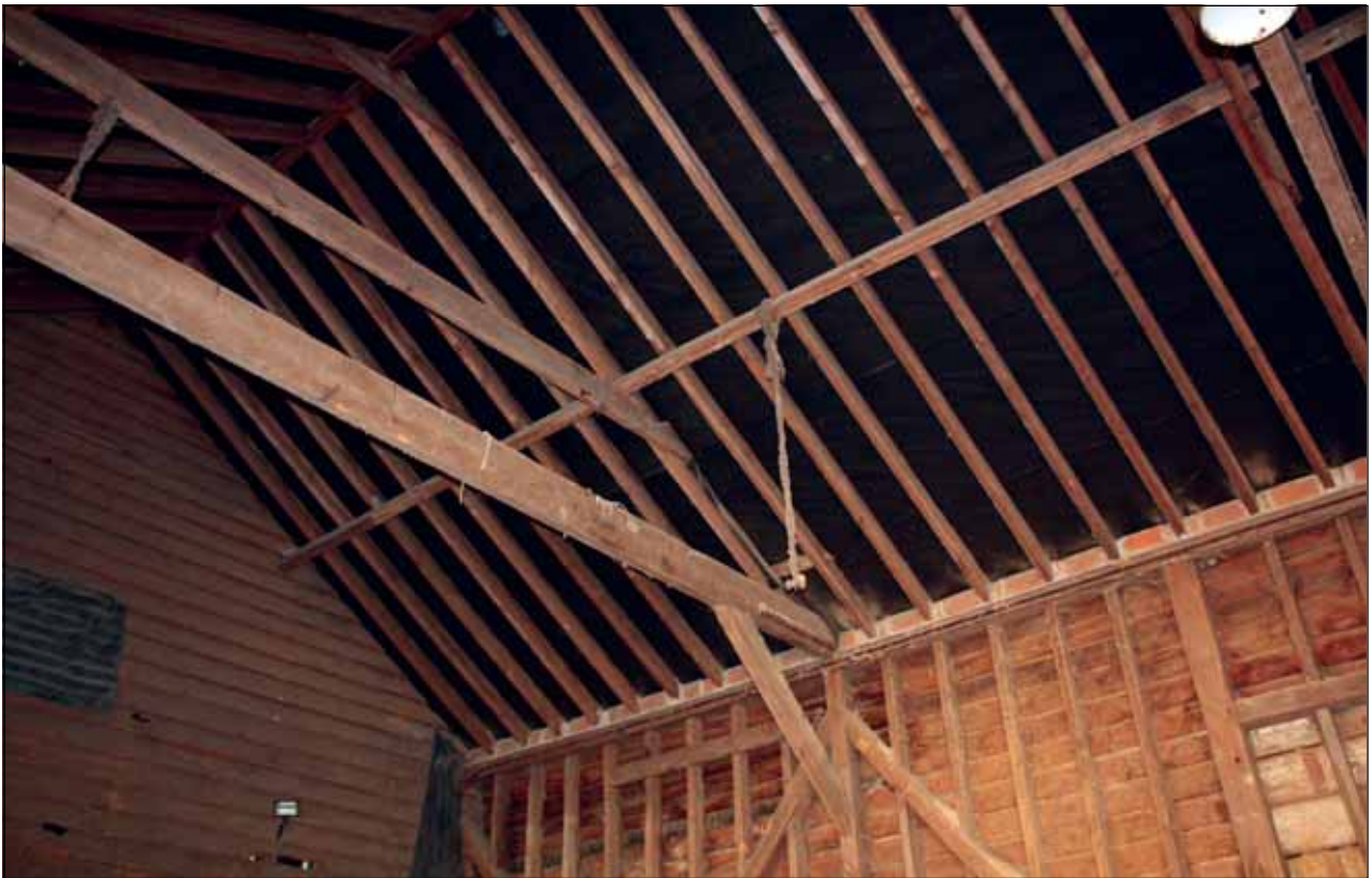
Plate 28: Detail of roof from inside Building 5
