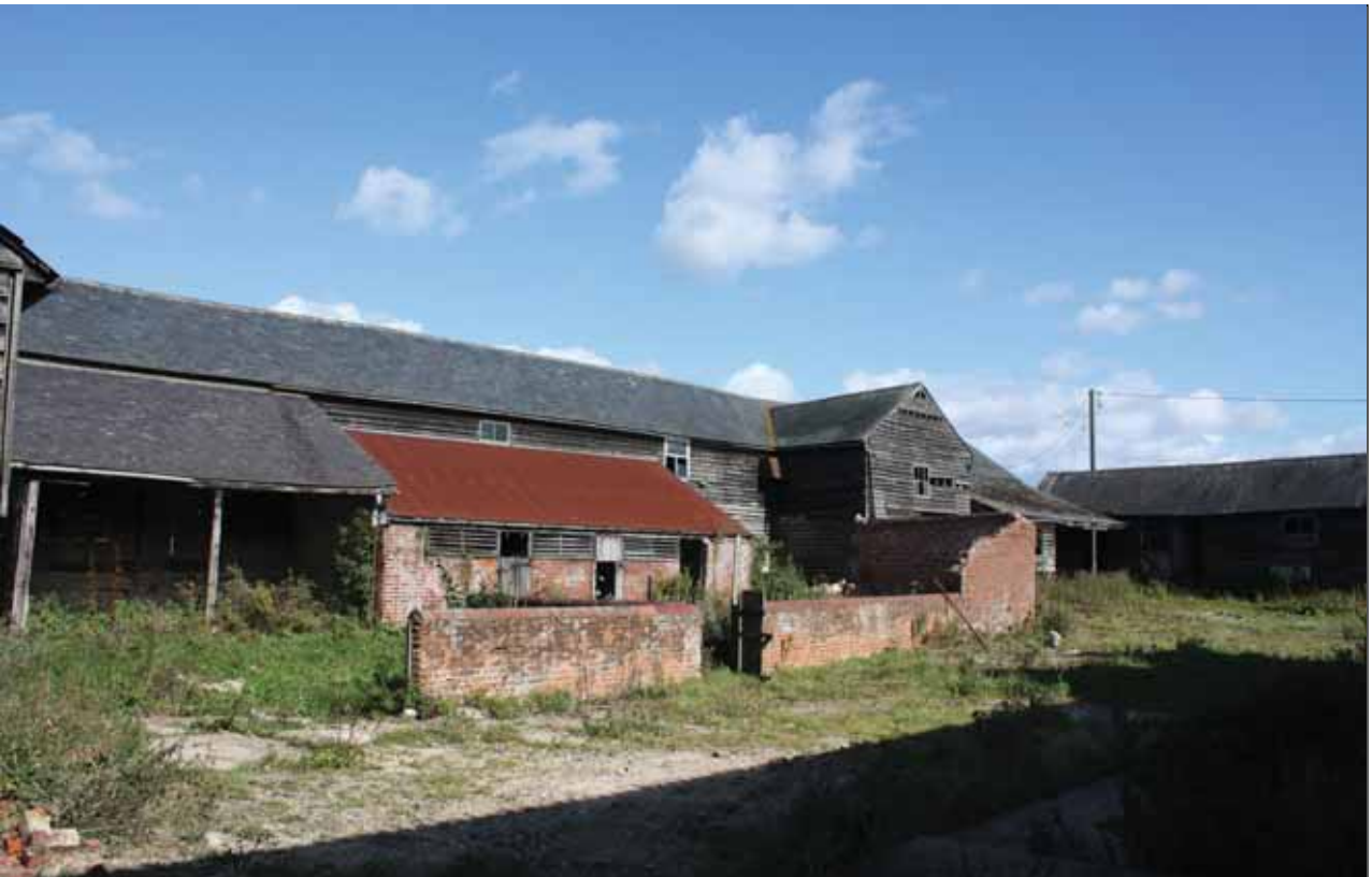
Plate 23: View of south-facing elevation, Building 5, showing relationship with Buildings 2 and 3
