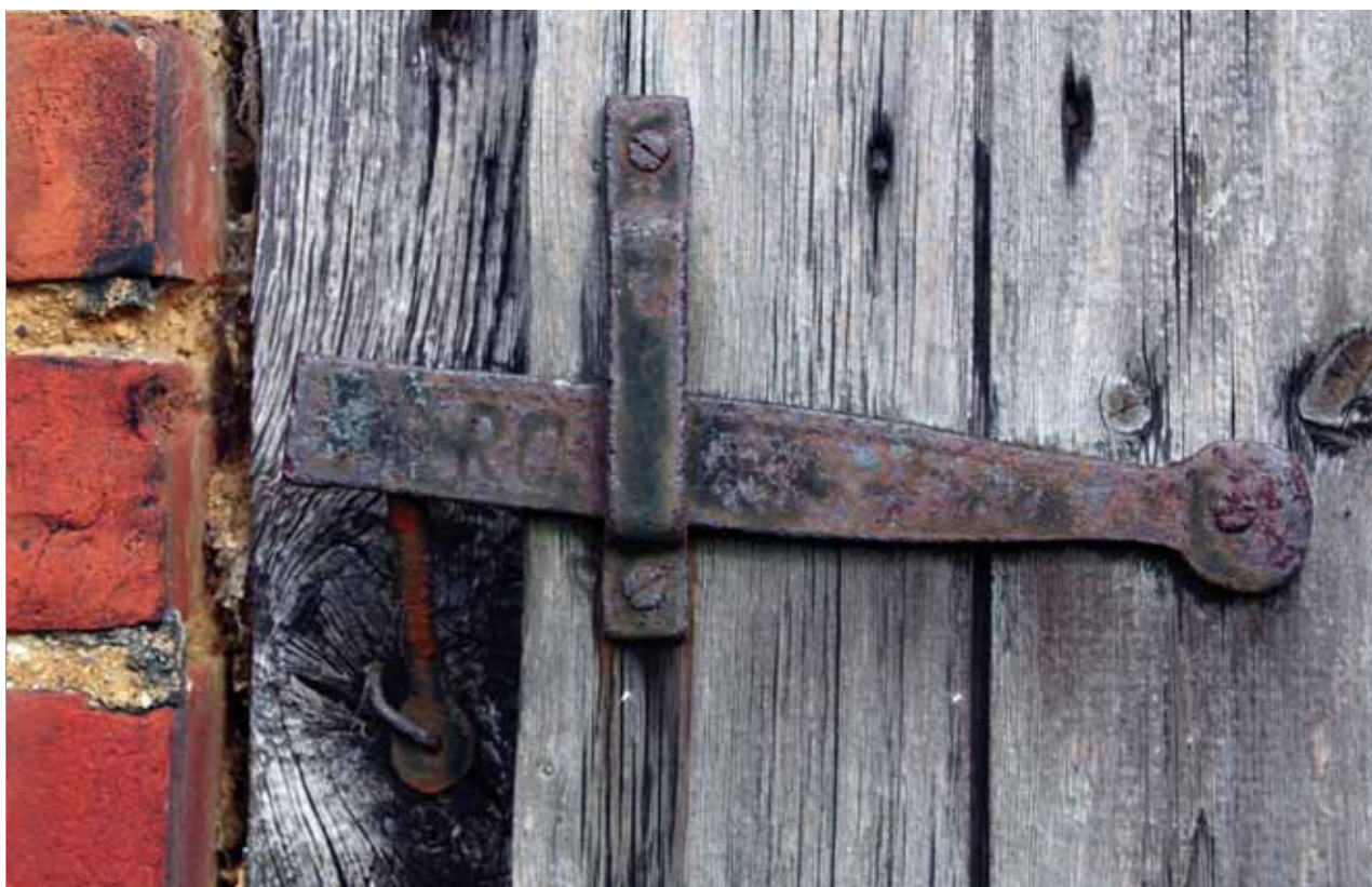
Plate 12: Detail of initials on door latch, Building 3
