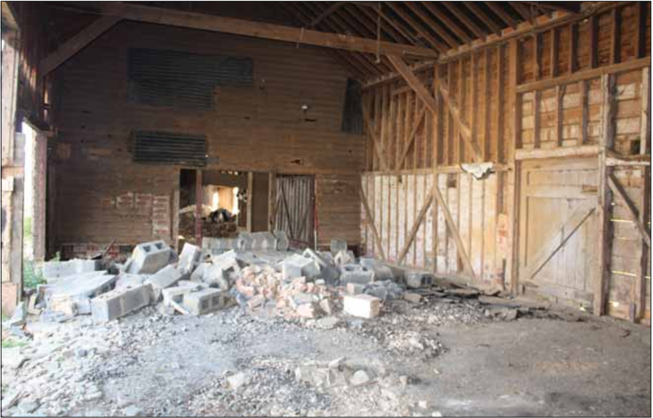
Plate 26: Internal view, Building 5
