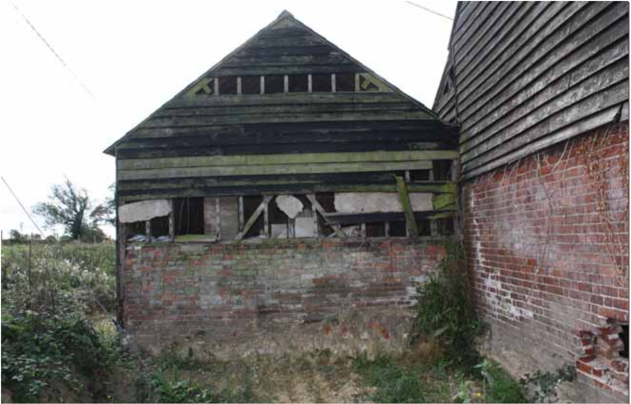
Plate 31: North-facing gable-end, Building 6
