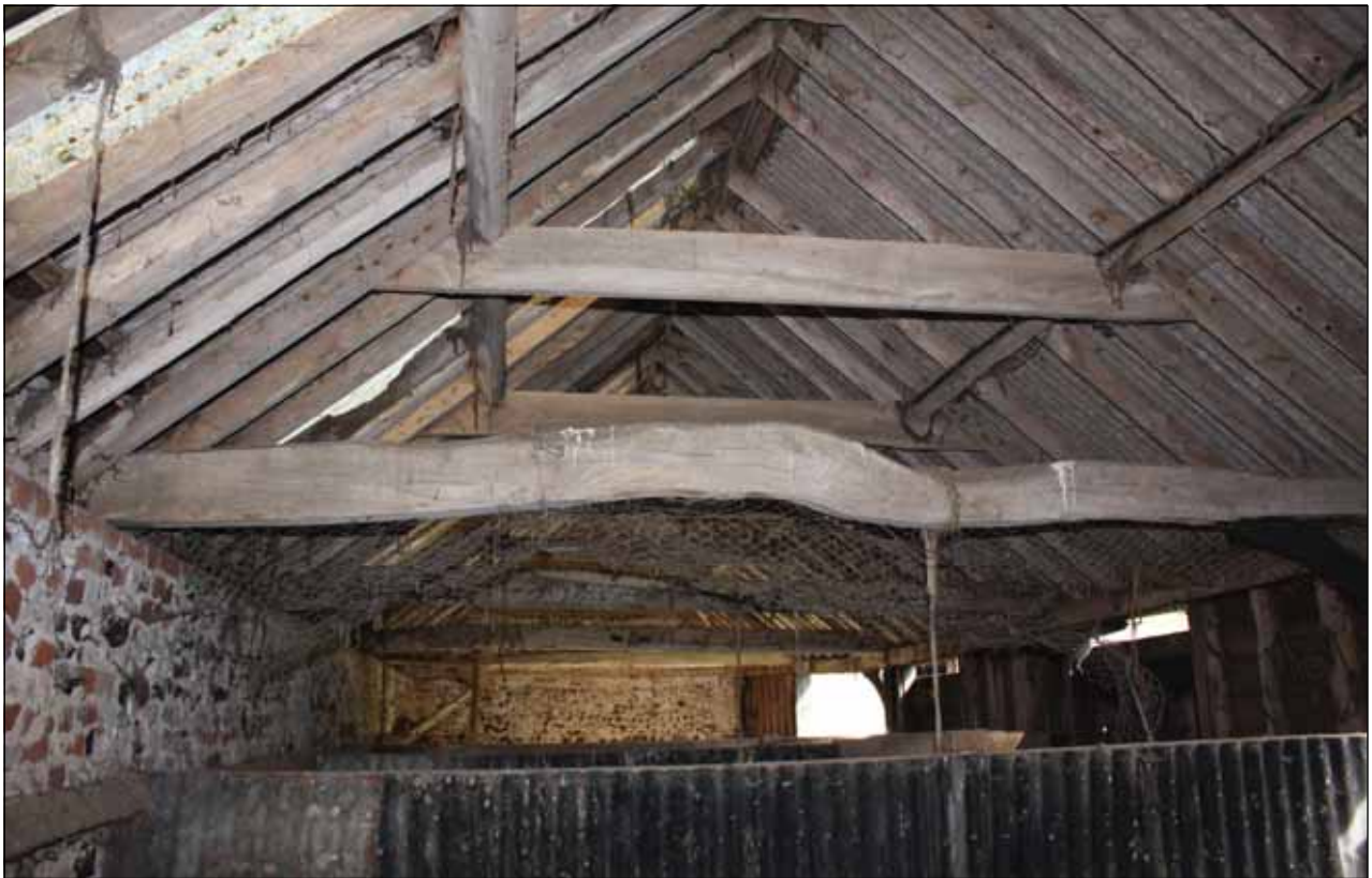
Plate 44: Internal view, Building 8
