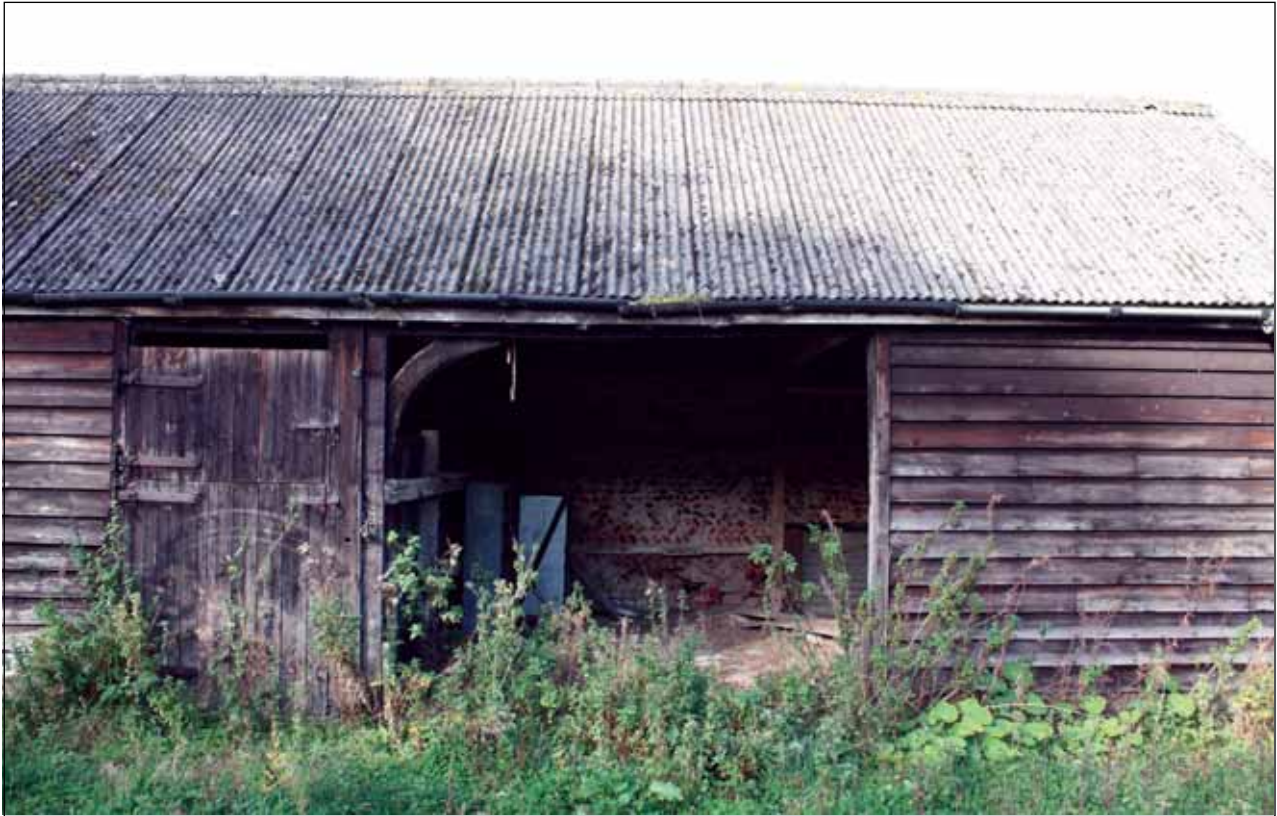
Plate 42: Detail of open-fronted northern end of east-facing elevation, Building 8
