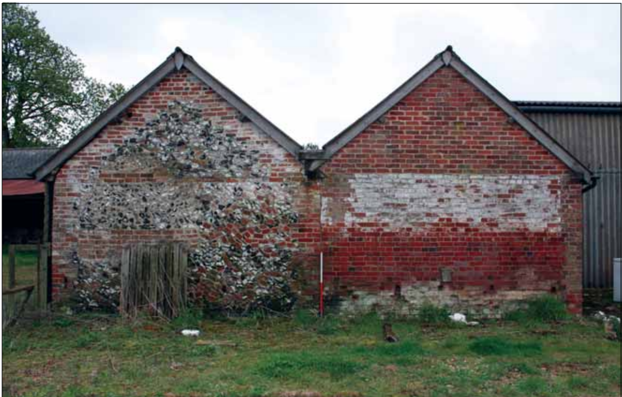
Plate 43: North-facing gable-ends, Buildings 8 and 9
