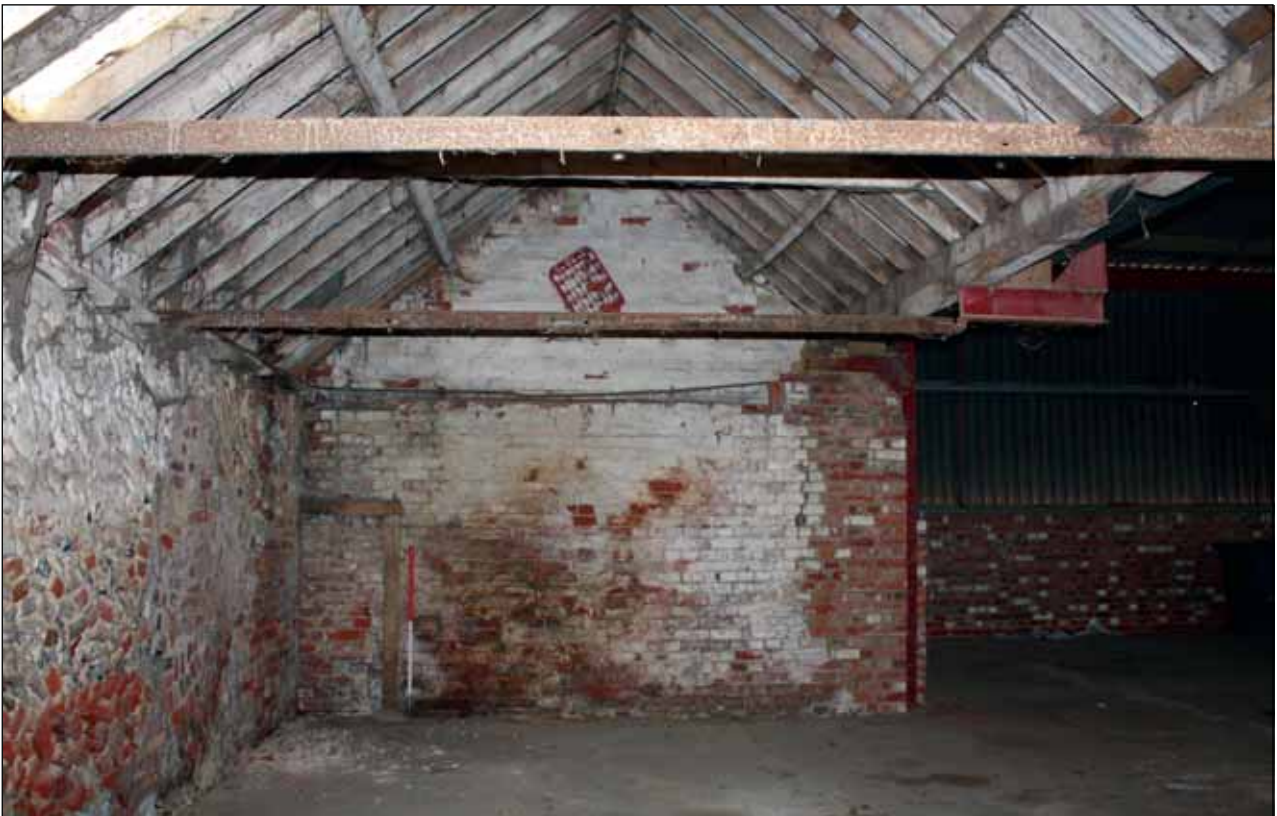
Plate 52: Internal detail, Building 9
