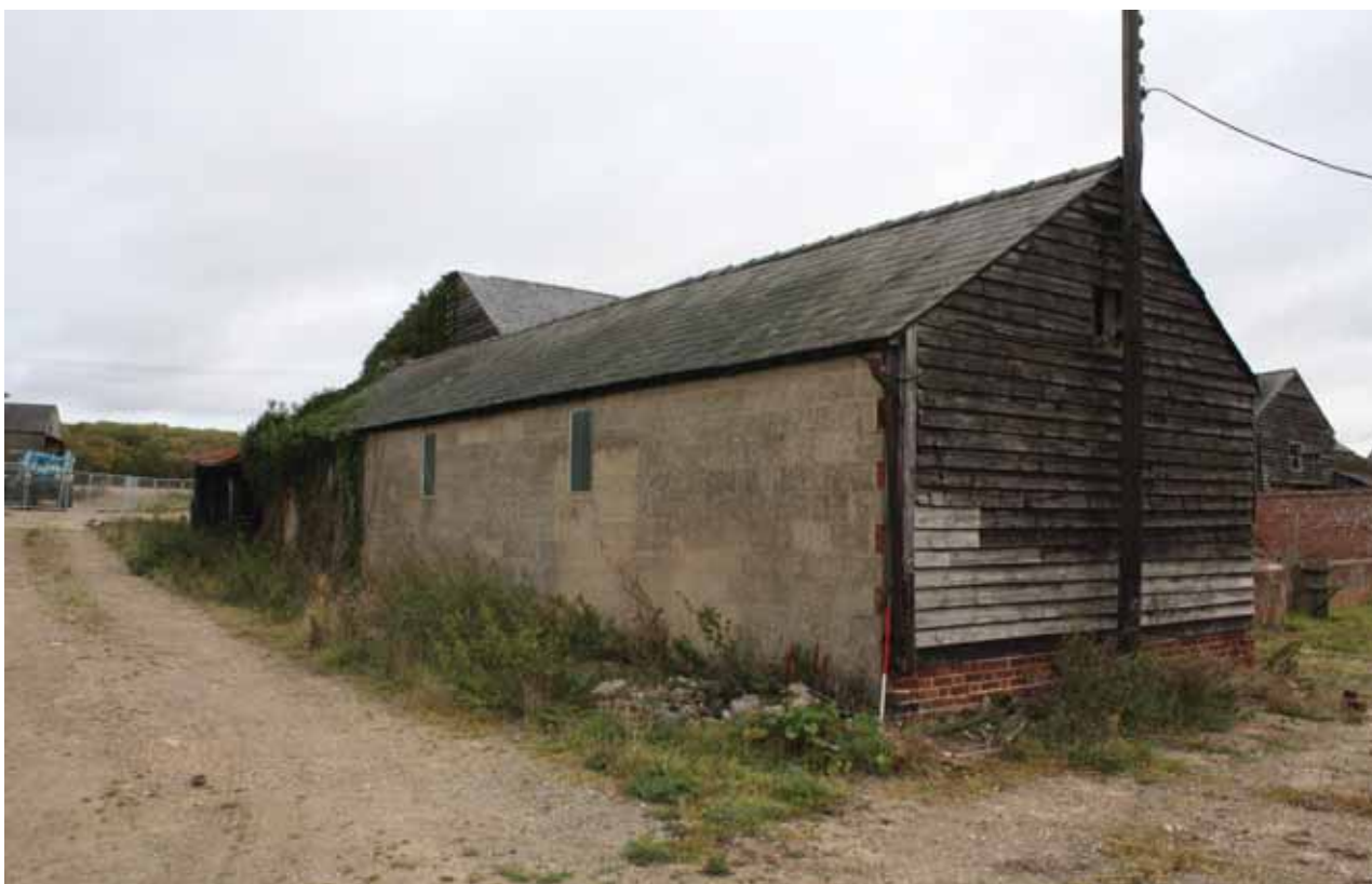
Plate 4: West and south-facing elevation, Building 1
