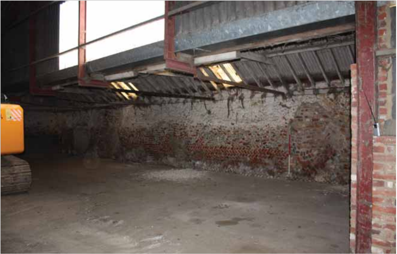
Plate 51: Building 9 from inside modern steel unit
