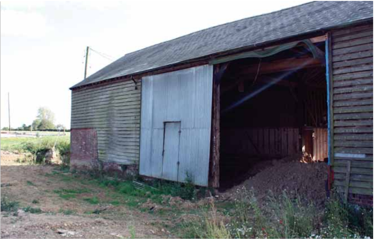
Plate 15: North-facing elevation, Building 4
