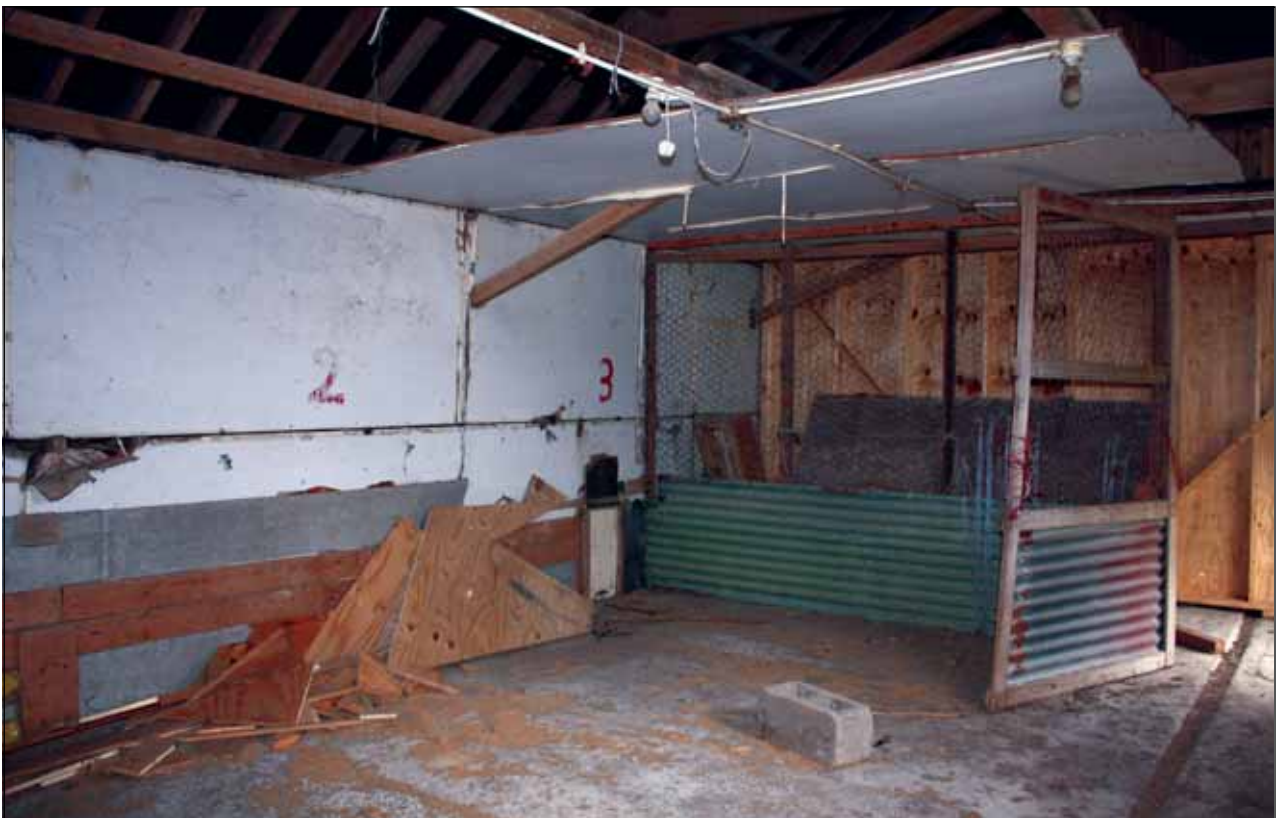
Plate 37: Internal view, Building 6
