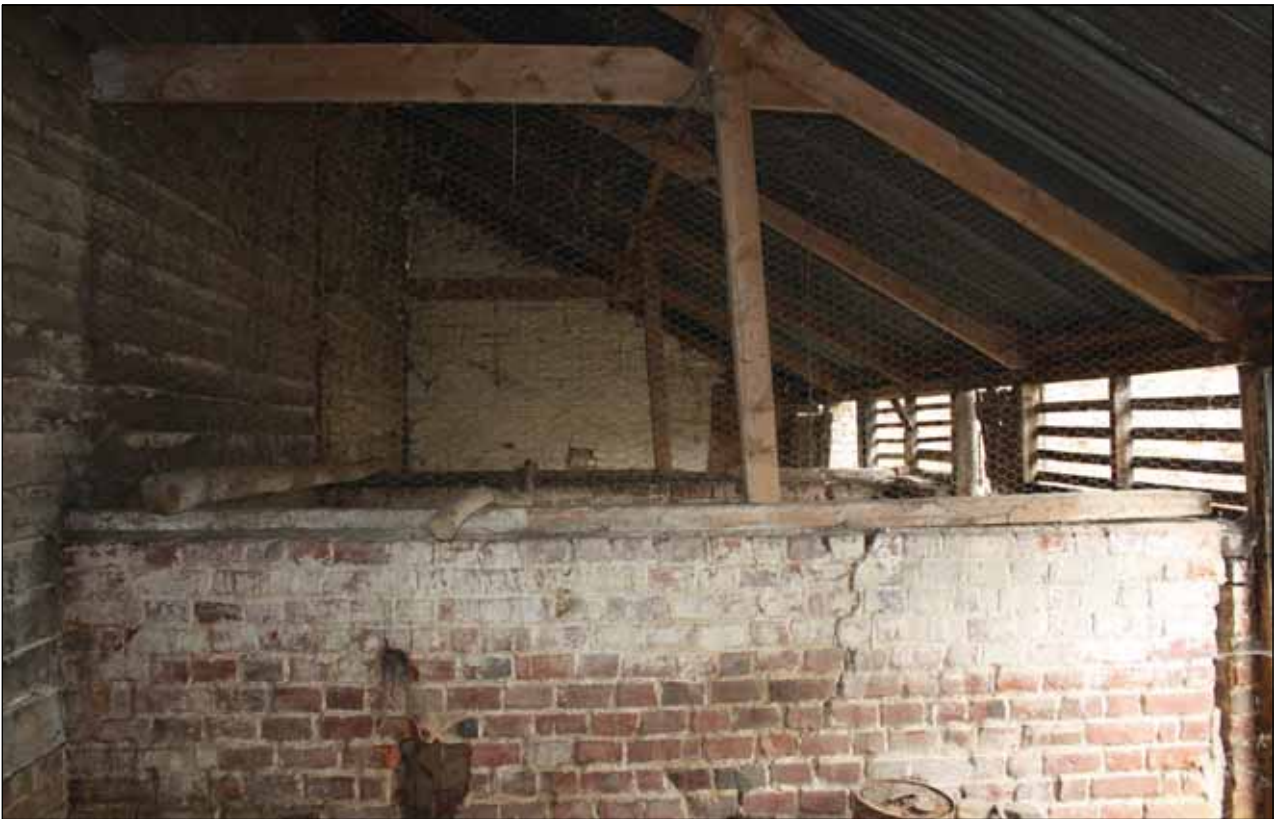
Plate 13: Internal view, Building 3
