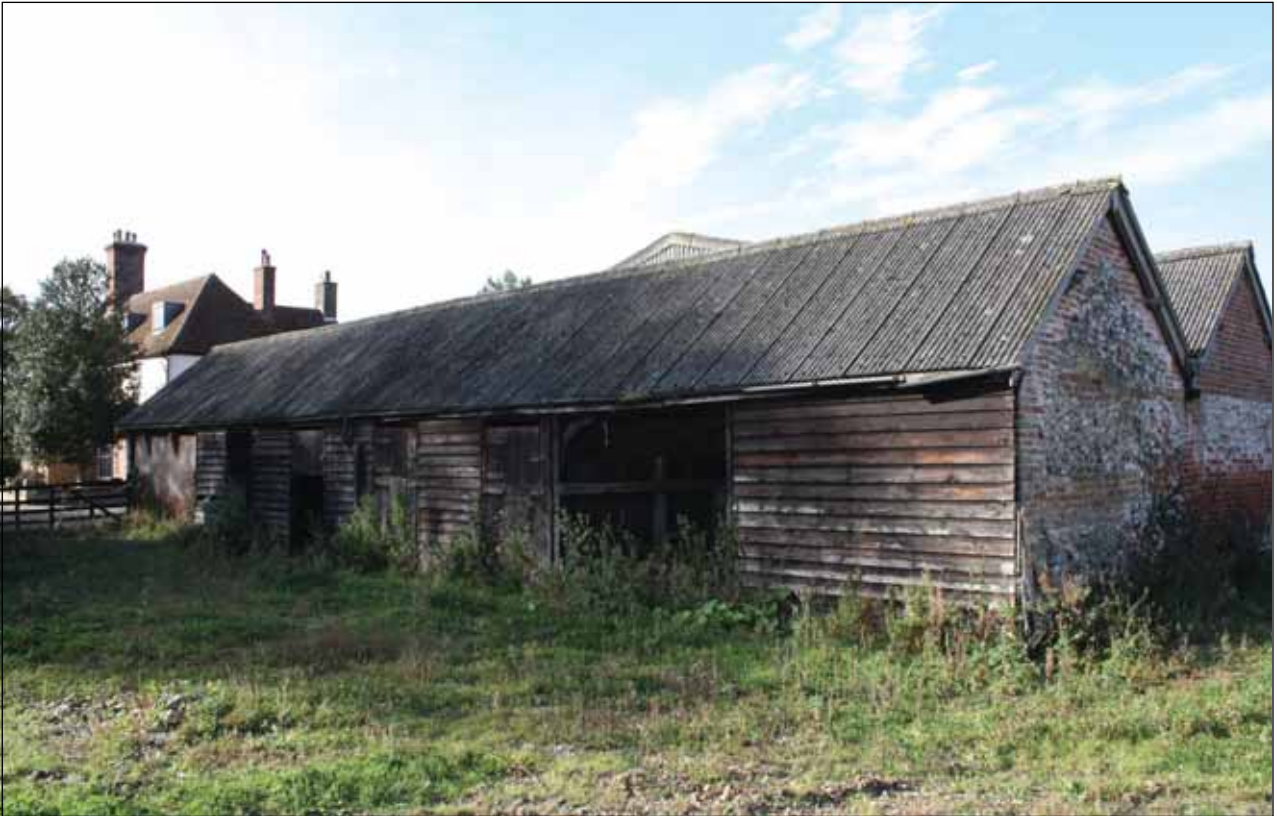
Plate 40: East-facing elevation, Building 8
