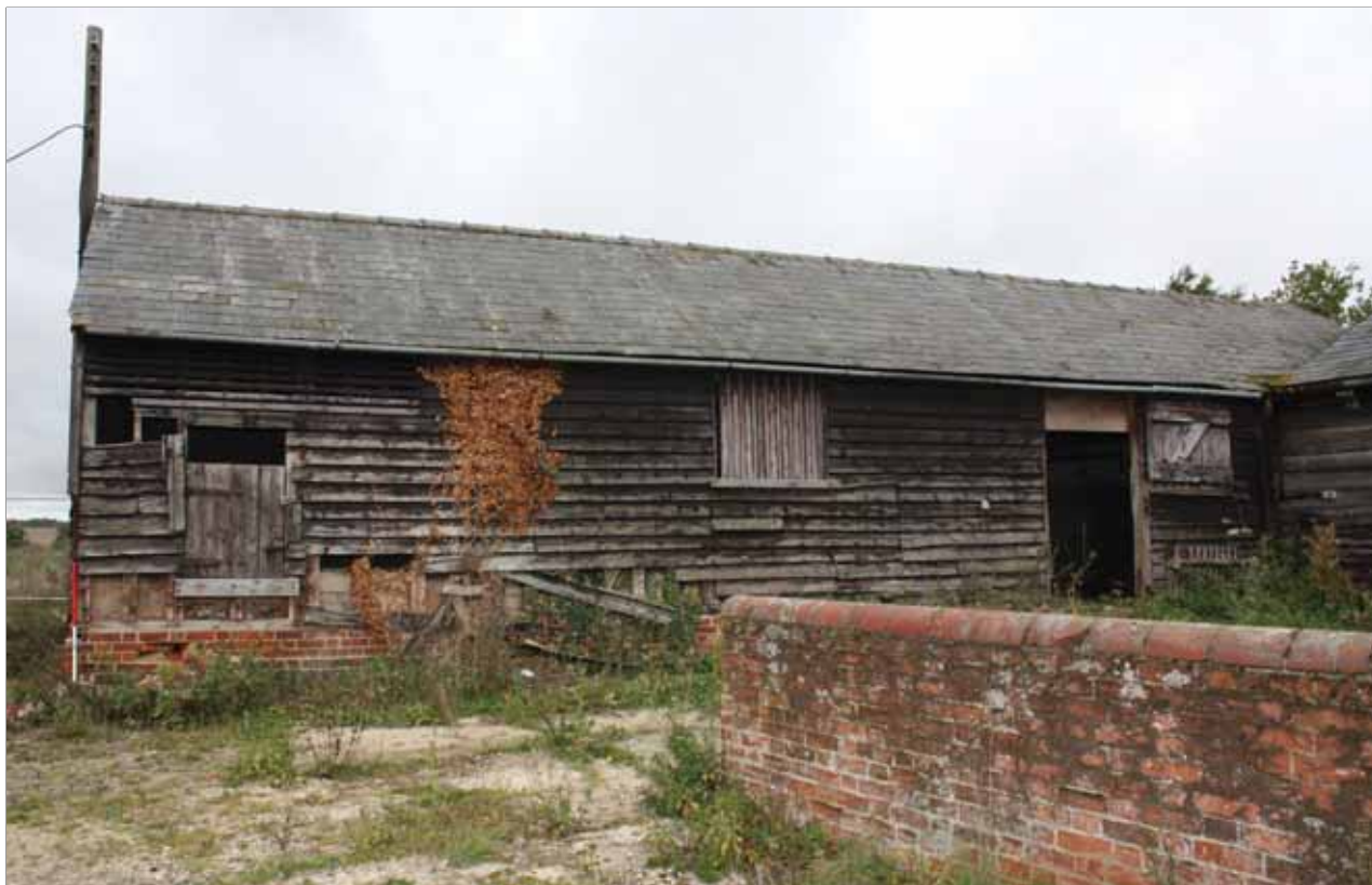
Plate 3: East-facing elevation, Building 1
