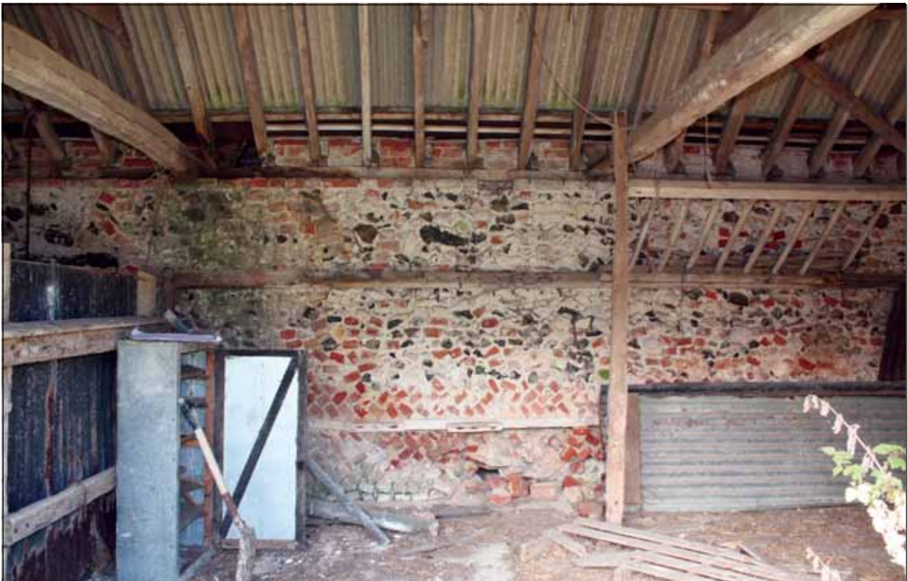
Plate 48: Detail of brick and flint wall and wooden stall, Building 8
