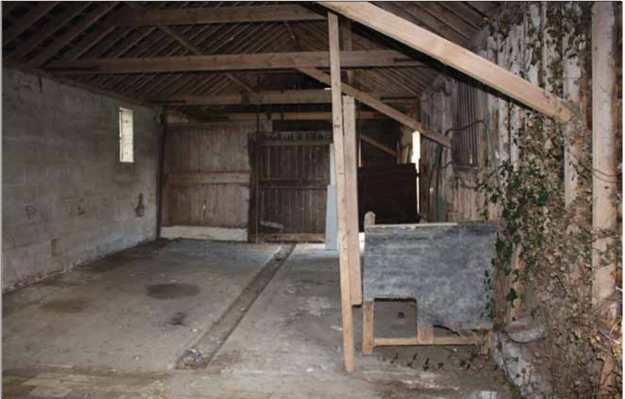
Plate 5: Internal view, Building 1
