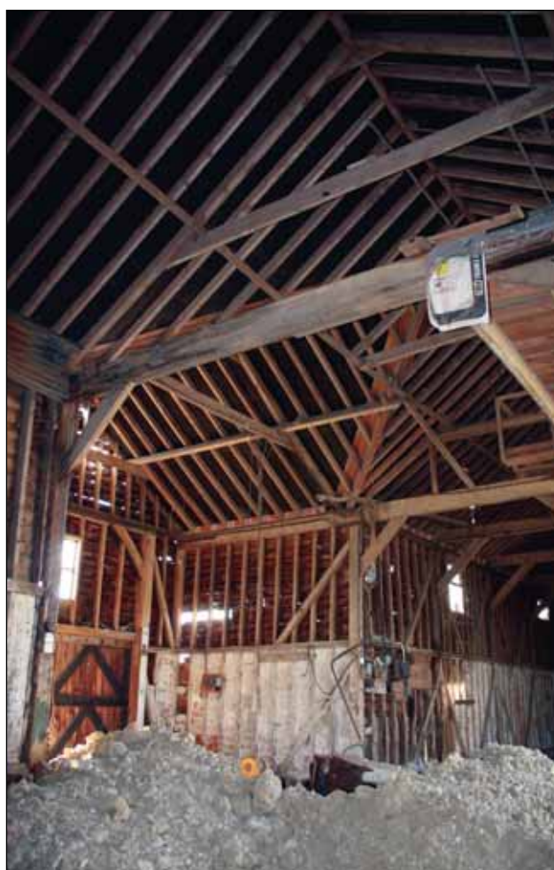
Plate 18: Internal view, Building 4
