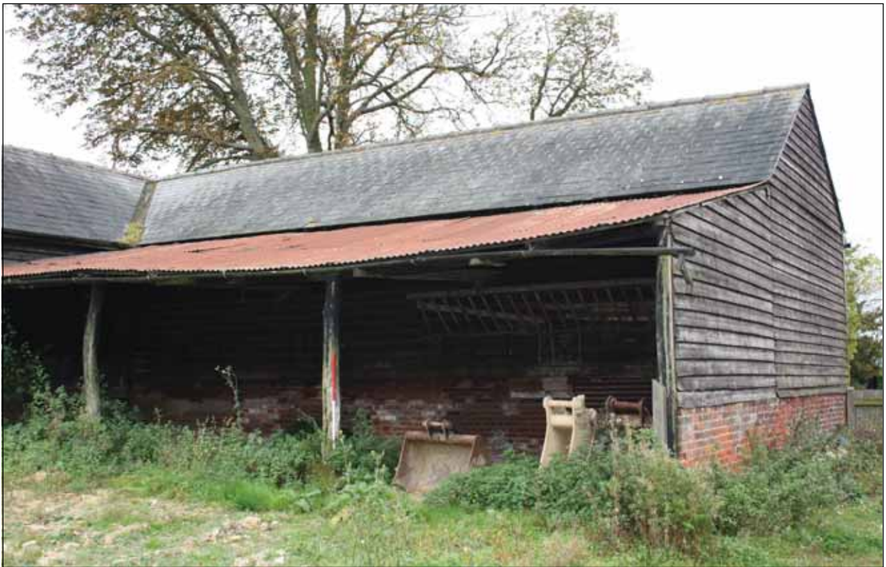
Plate 38: North-facing elevation, Building 7
