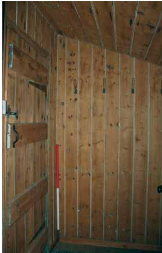
Plate 14: Internal view of entrance area G1
