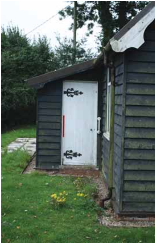
Plate 11: External entrance door on north-west facing elevation
