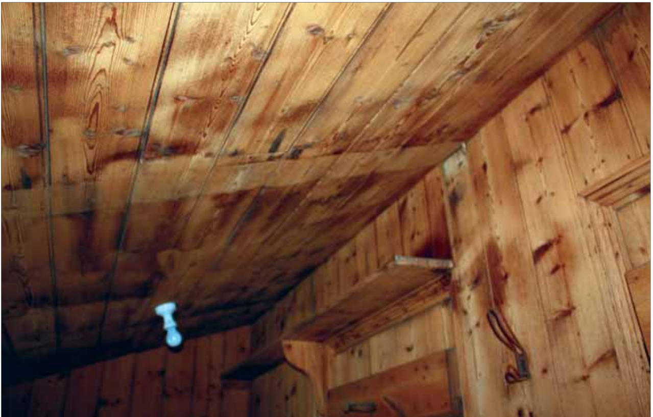
Plate 18: Evidence of removed internal partition, G2
