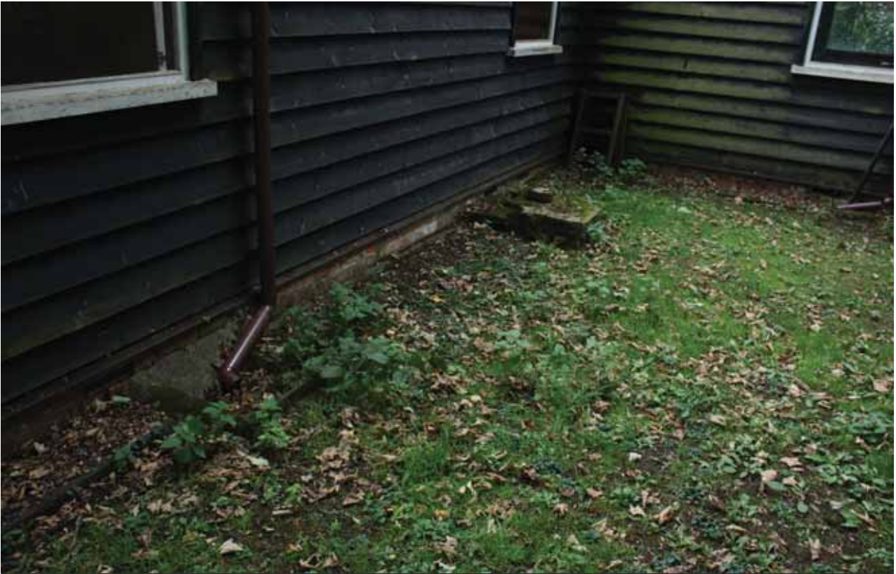
Plate 7: Remains of removed structure on south-west facing elevation
