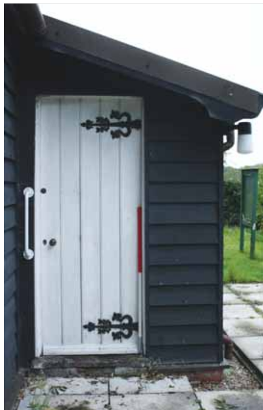
Plate 6: External door on south-east facing elevation
