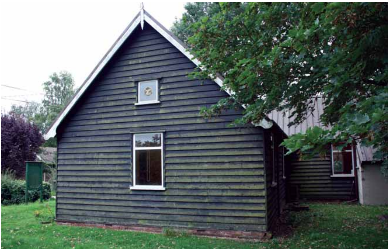
Plate 12: South-west facing elevation
