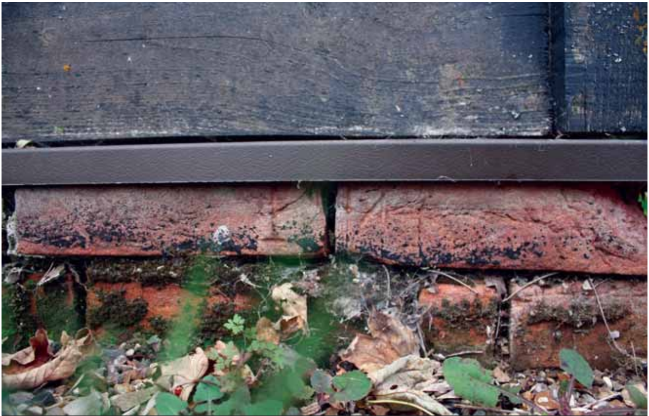
Plate 3: Detail of brick plinth on north-east facing elevation
