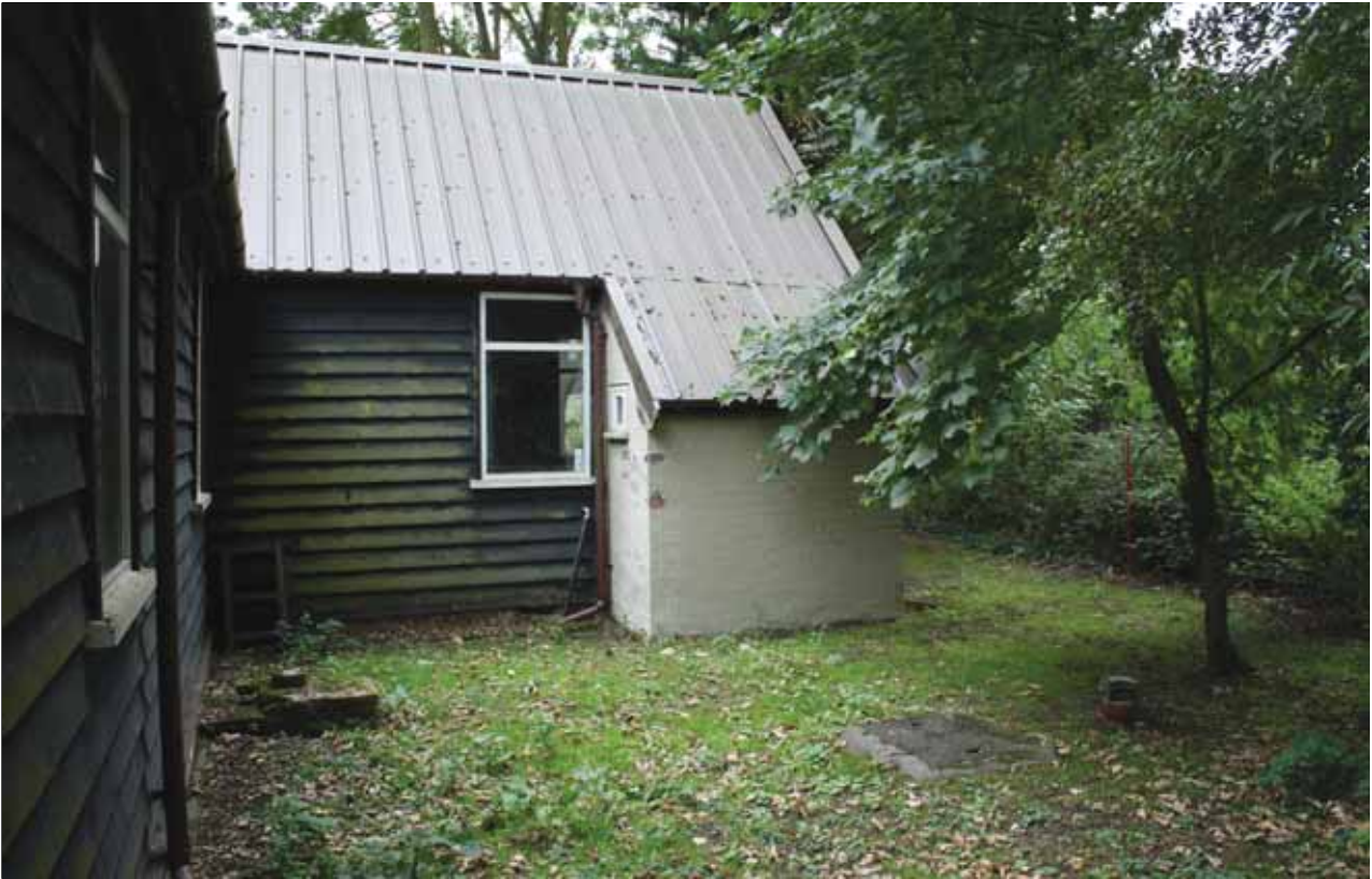
Plate 13: South-west facing elevation
