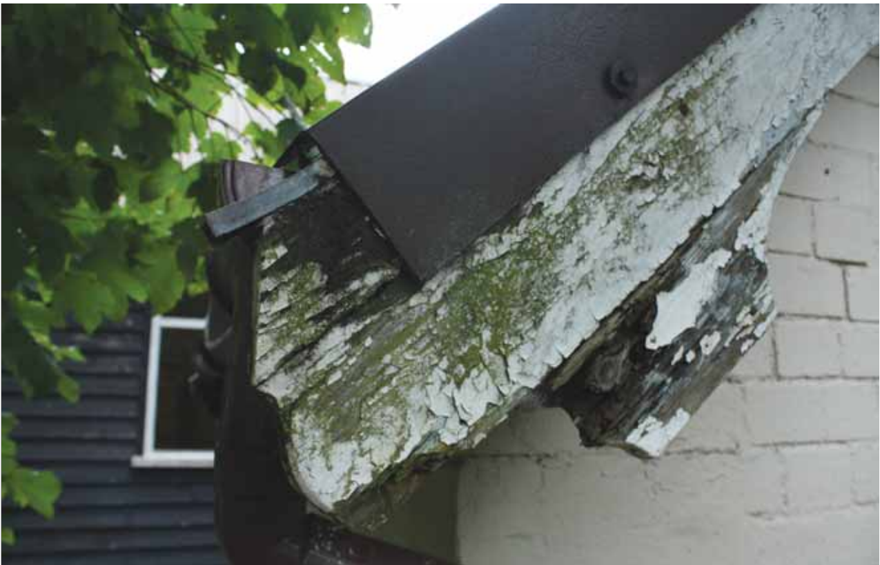
Plate 10: Detail of roof covering on eave of south-west facing elevation
